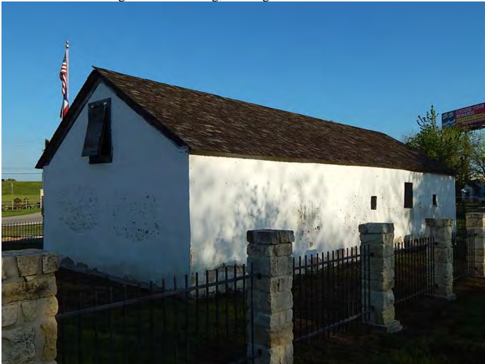
Photo 4: Selma Stagecoach Building, looking northwest.
