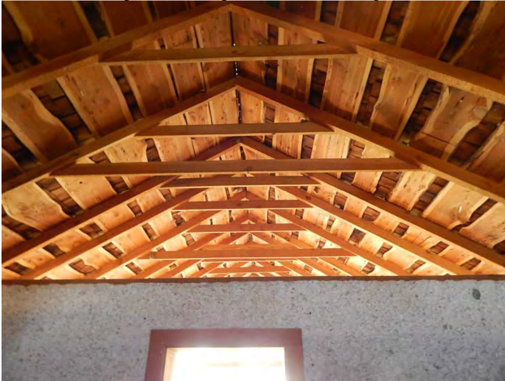
Photo 9: Selma Stagecoach Building detail of wall and ceiling construction
