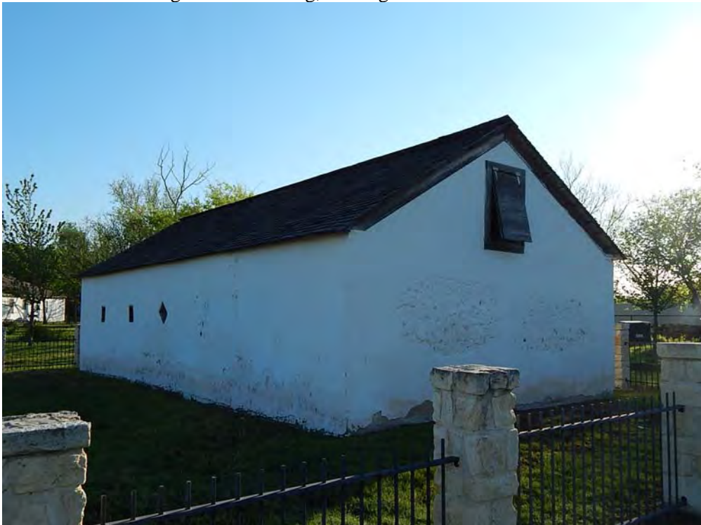
Photo 6: Selma Stagecoach Building, looking northeast
