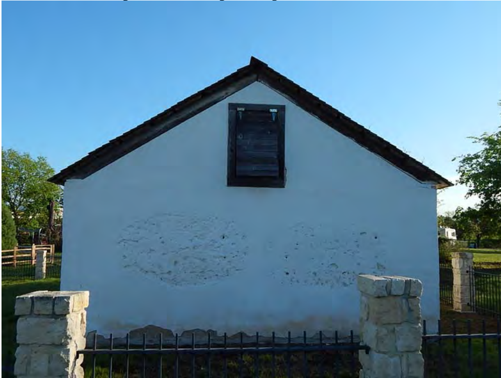
Photo 3: Selma Stagecoach Building, looking south.
