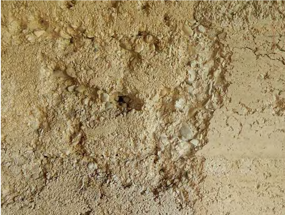
Photo 11: Selma Stagecoach Building detail of wall construction
