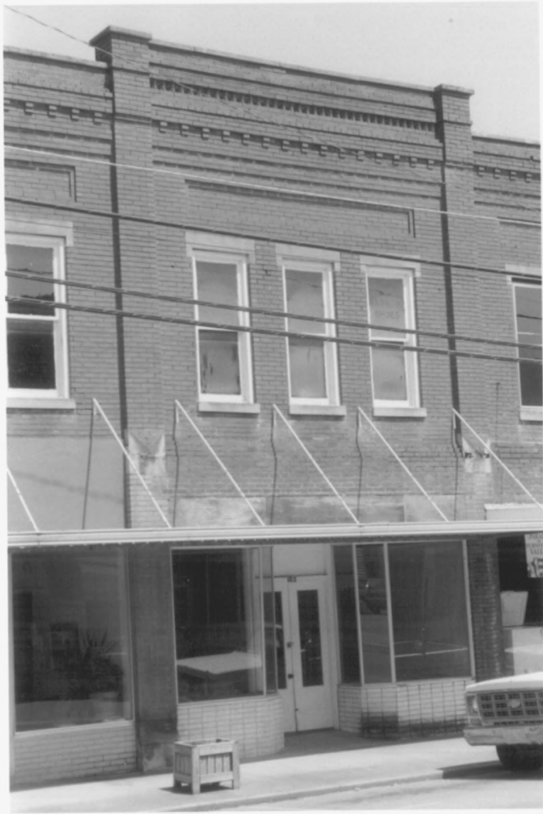
Hartsville Historic District Trosdale Co TN
