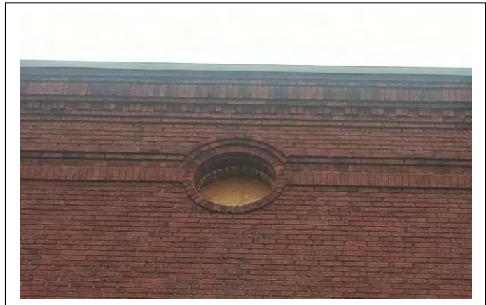
Figure 5: Detail of roundel window and brick corbeling on 2552 Marcy St.
