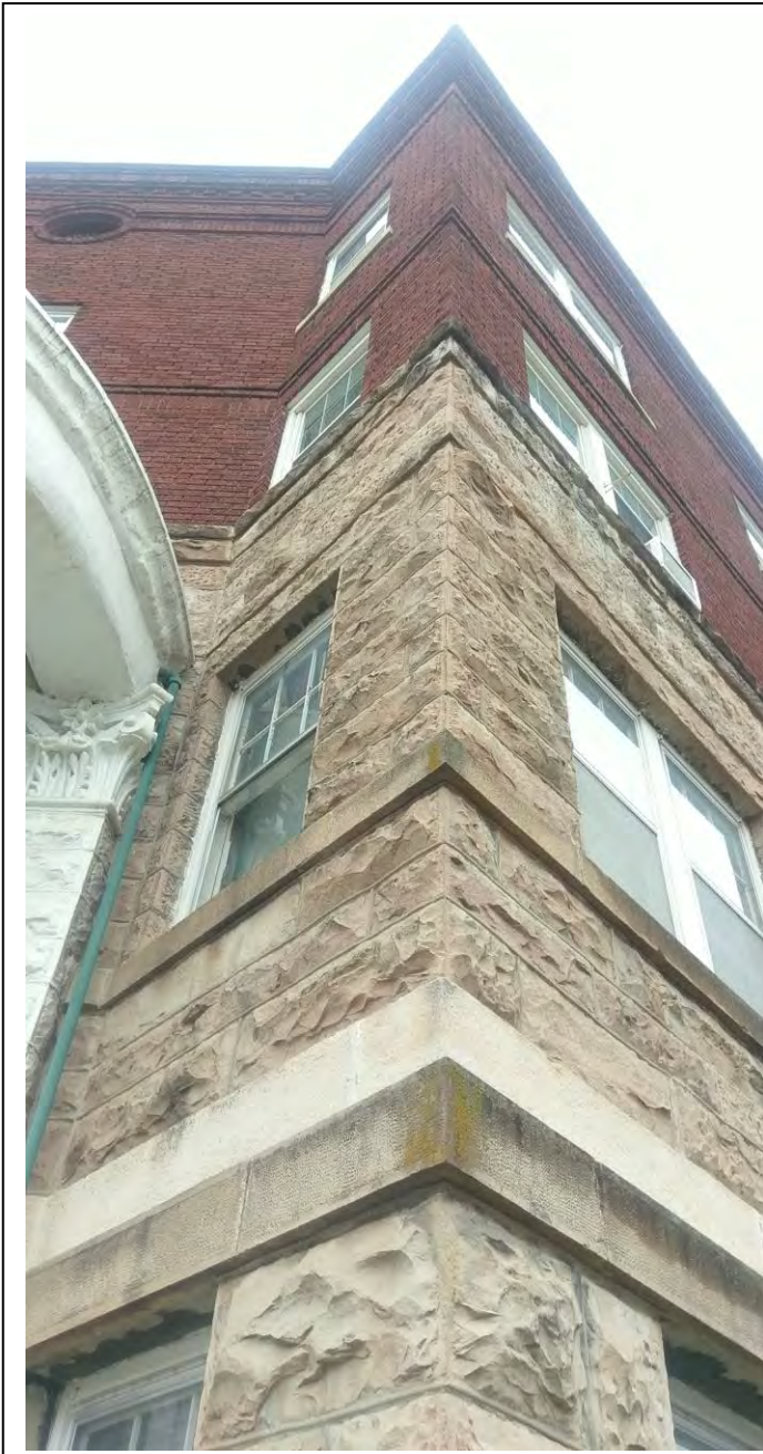
Figure 3: Detail of front façade stone work next to 2552 Marcy St. Portico.
