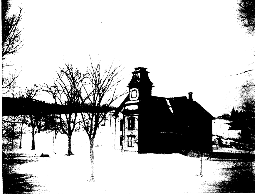
THE TOWN HALL IN 1894 WHOSE MAIN BUILDING, WITHOUT THE TOWER AND FRONT GABLE, WAS THE FIRST MEETING HOUSE, BUILT IN 1749
