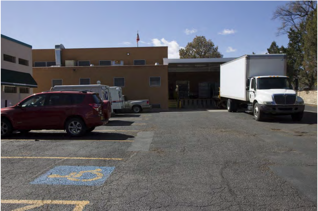
Photo: 9 of 13: Rear view with loading dock, photographer facing south.
