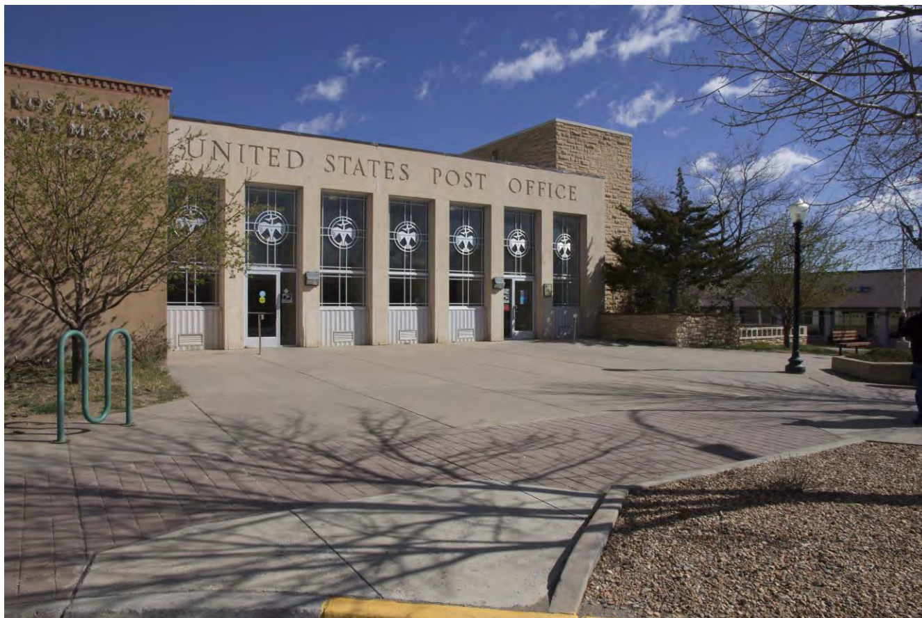
Photo 2 of 13: Main façade and plaza, photographer facing northeast.
