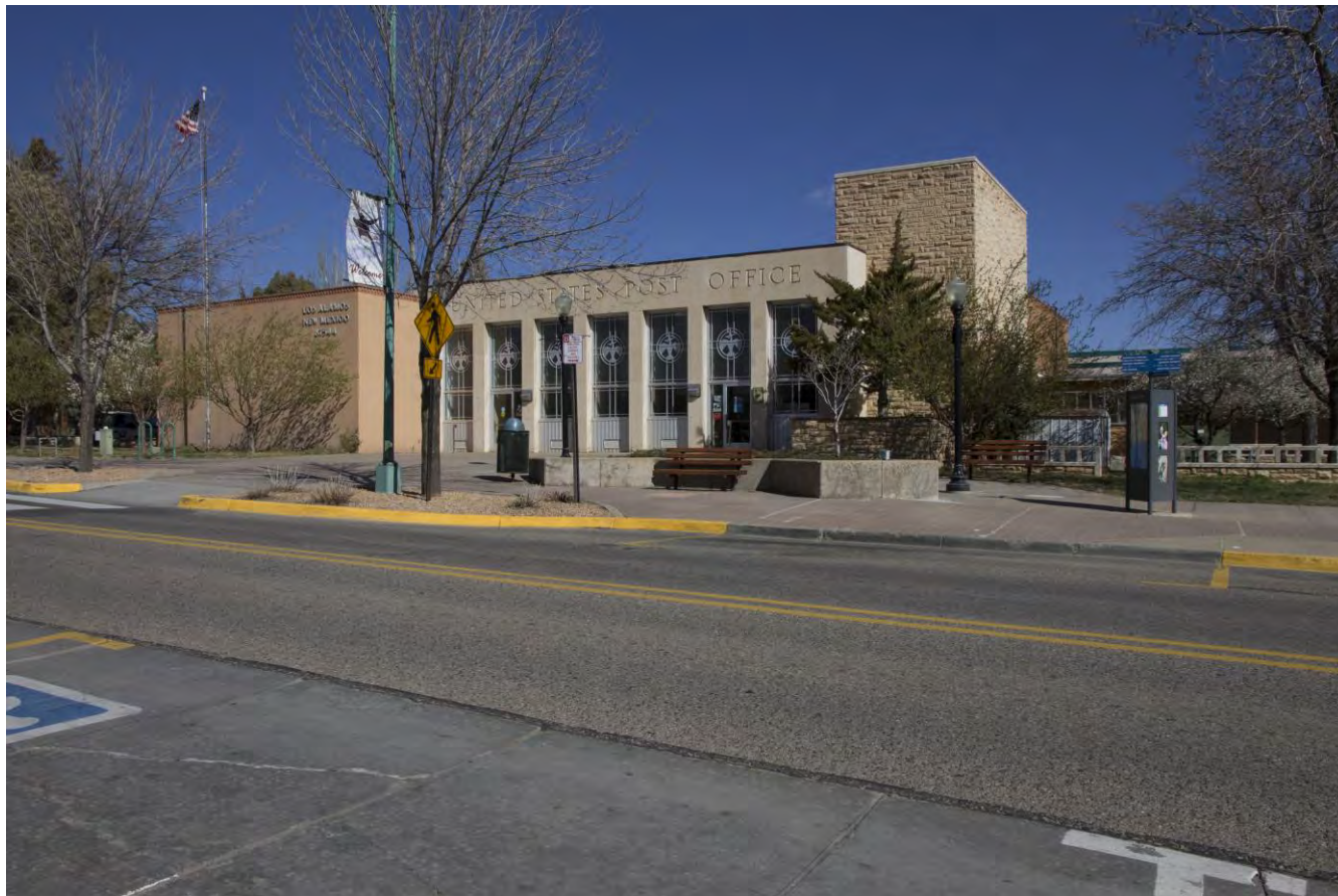
Photo 3 of 13: Main façade, photographer facing northwest.
