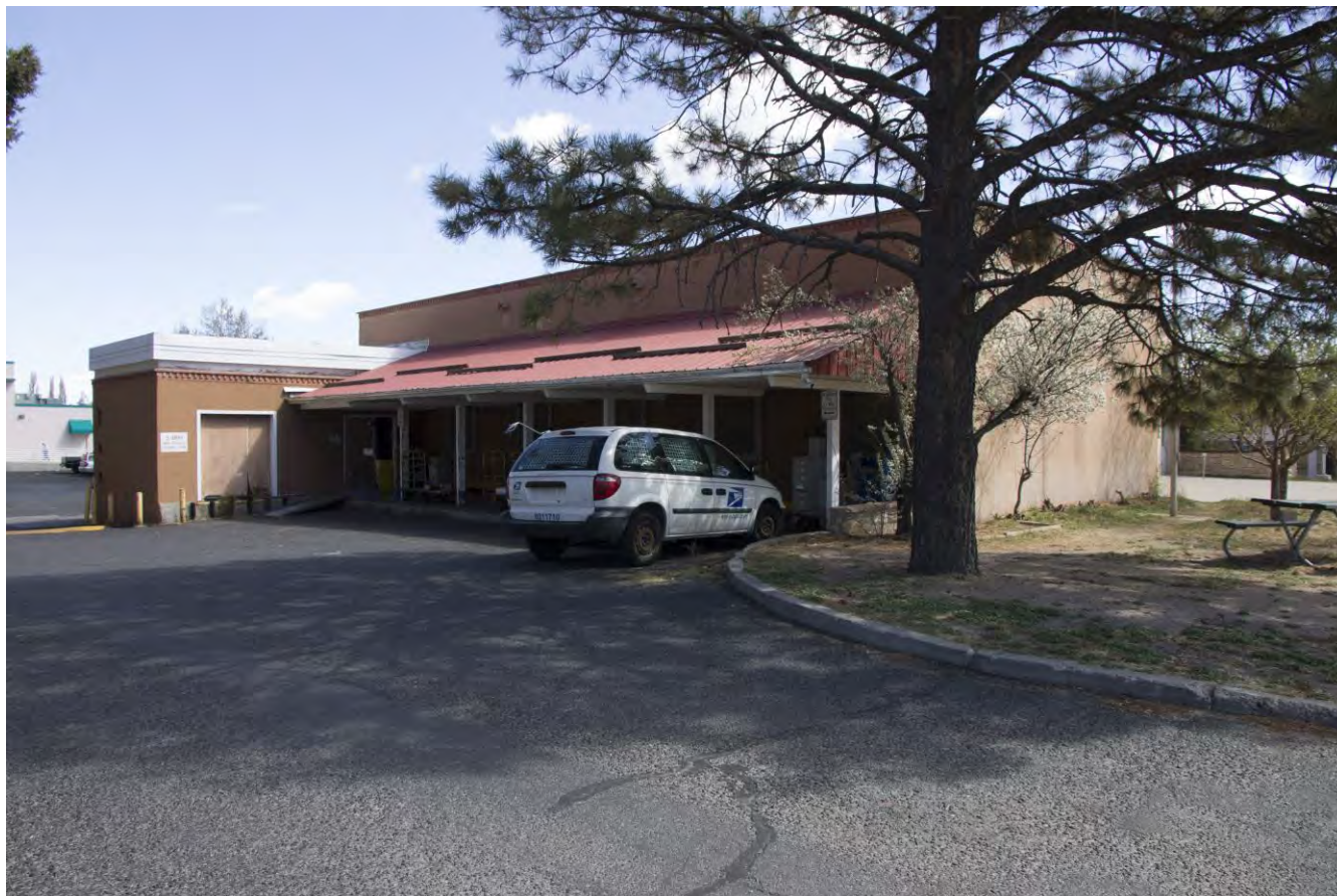
Photo: 10 of 13: West side with loading dock and nonhistoric roof awning, photographer facing northeast.
