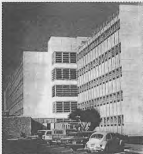
Eola Hall in 1972. Note the continuous band of steel sash security windows. Photo courtesy Salem Public Library Digital Photo Archive.
