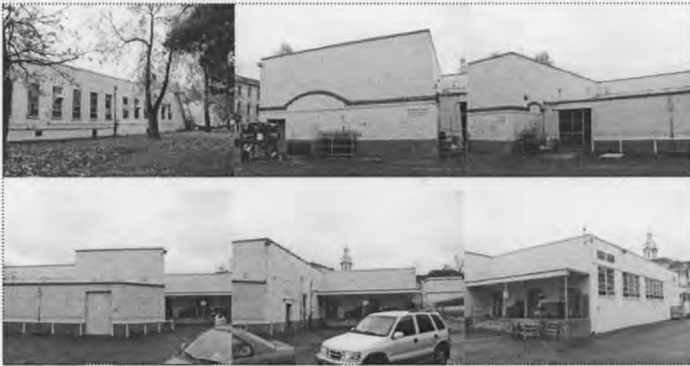
Series of photos demonstrating the haphazard way in which Building 31b has developed. Photos start with the south facade and progress in a counter-clockwise path around the building. Photos 2007 by ARG.
