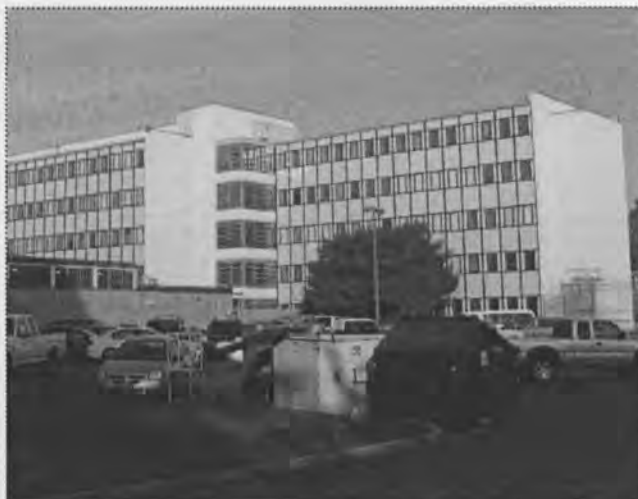
Eola Hall in 2007 showing the 1992 changes in window profile and configuration. Photo by ARG.
