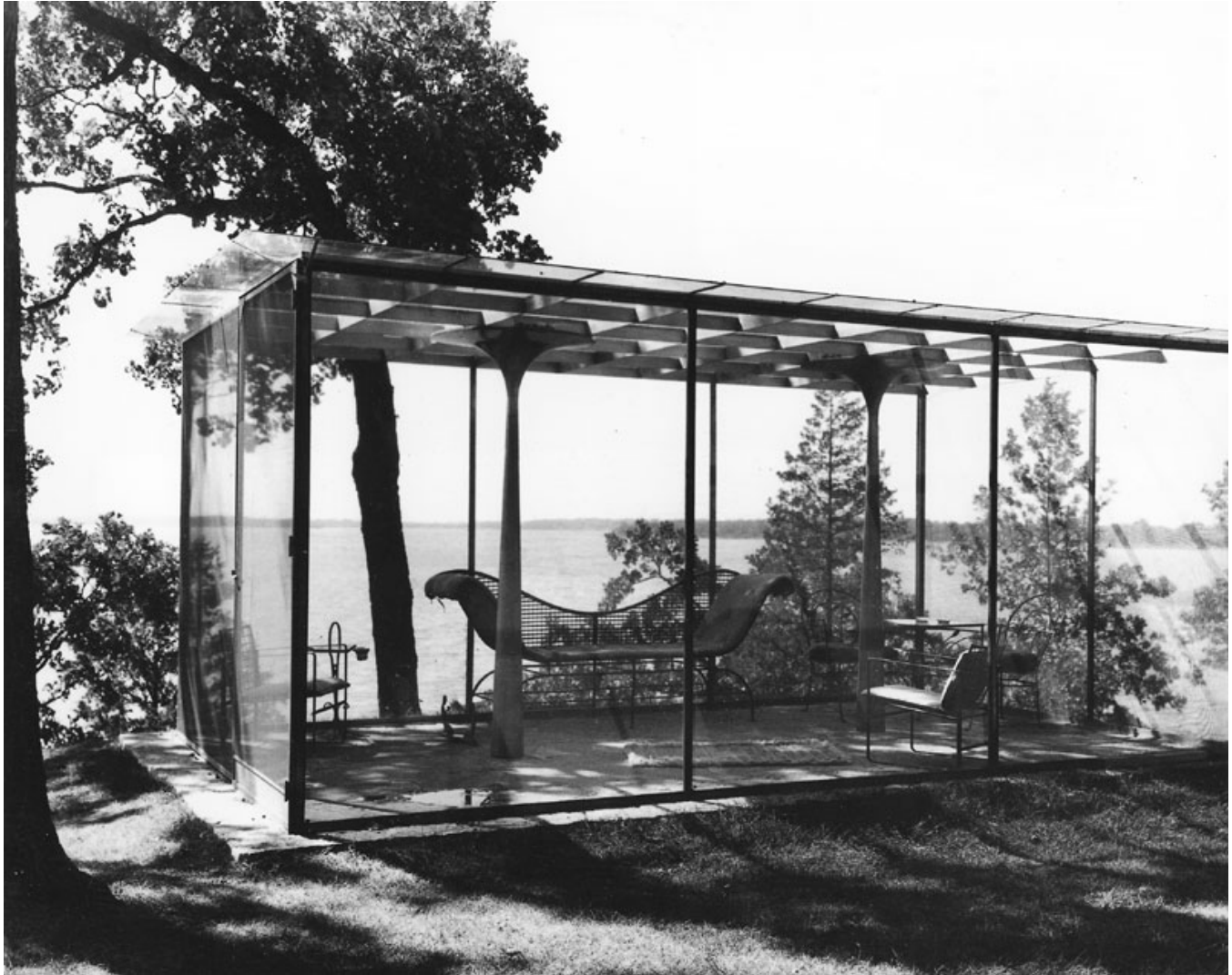
Historic view showing the Bertrand Goldberg designed “orangerie” (above) atop the bluff; view southwest. ( Bertrand Goldberg Archives – Art Institute of Chicago )
