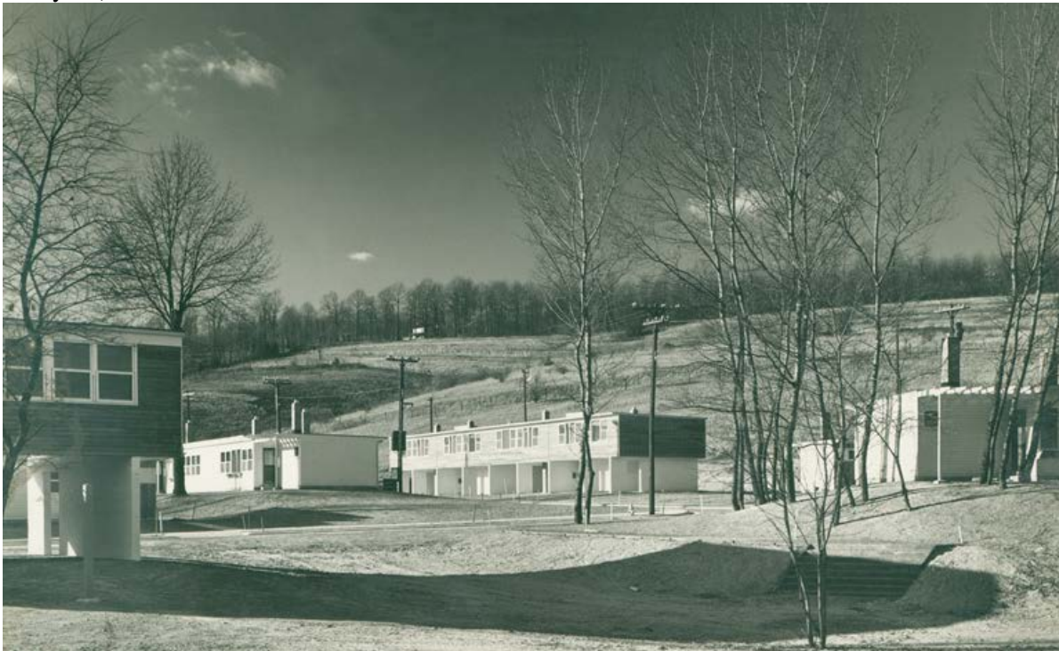
Figure 15: Facing Brook Lane, from the rear yard of 2-4 Foundry Street. The rear entrances to the B plan houses had pergola-like structures overhead, which were later replaced by other roof structures. (Barely visible in far right house and house in left-center.)
