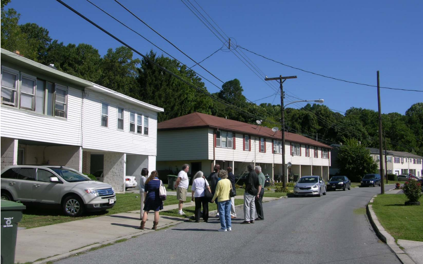
Photo 7: Three groups of CC houses on N side of Foundry St., camera facing NE. The first grouping (only partially visible, showing 37 and 35 in foreground) retains early low-pitch roof line.
