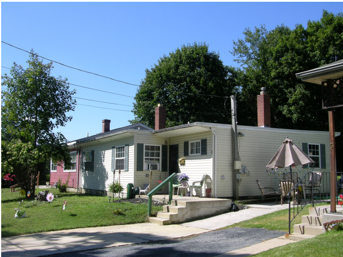
Photo 2: Plan B, north end (3) of 1-3 Foundry Street, Camera facing SW. Windows and siding replaced but prominent chimneys and flat roofline intact.
