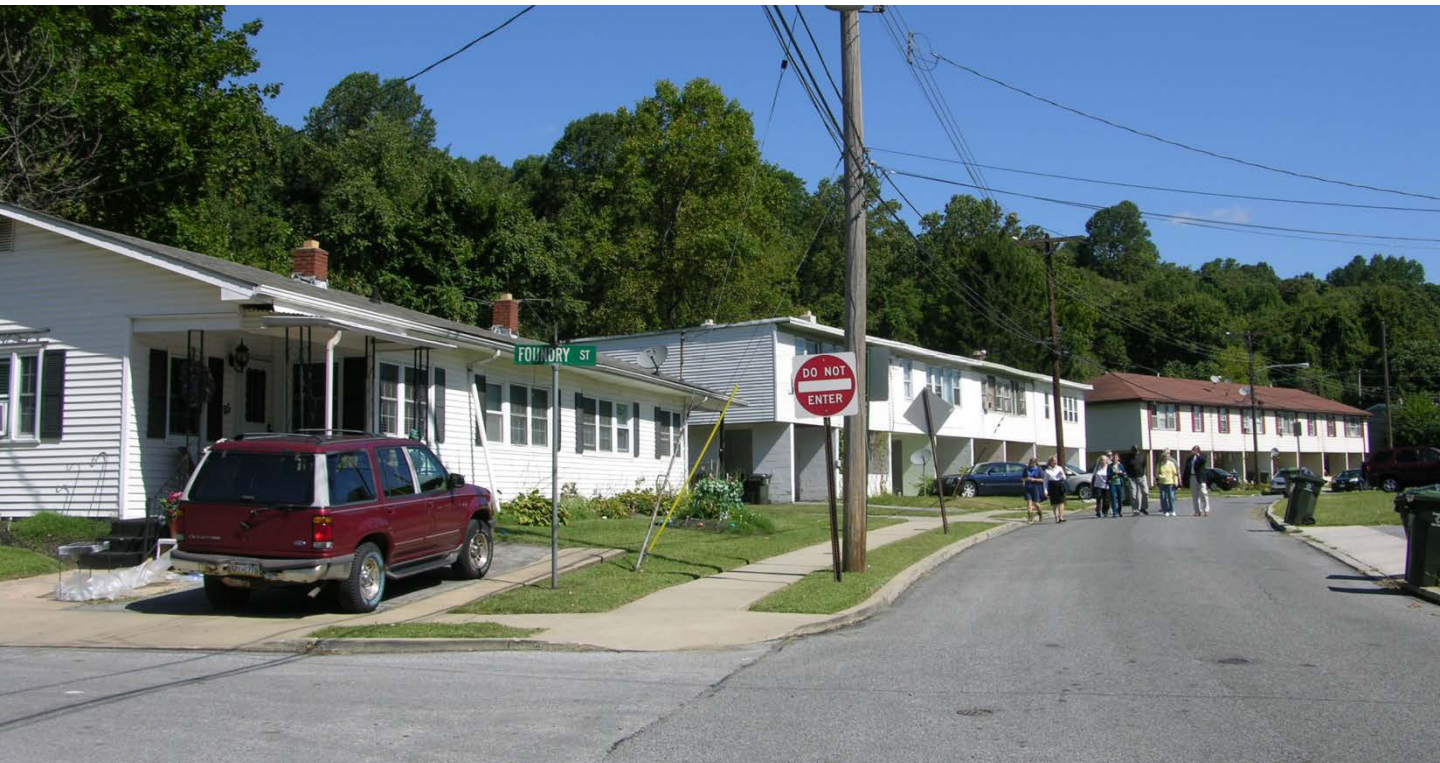
Photo 4: Looking NE from the intersection of Foundry St. and Brook Lane, at houses on the N side of Foundry St. (street sign is turned); Plan B (25-27 Foundry) in foreground; two Plan CCs in background.
