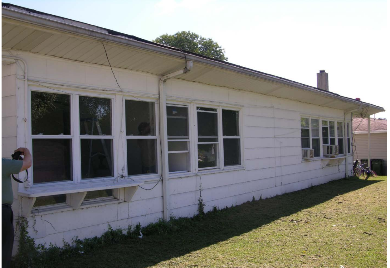
Photo 10: Rear elevation of 42 (left) and 44 Foundry Street, which retain original flower planter shelves with various size holes cut into shelf for pots. Original flat roof line. Plan B. Camera facing SE.
