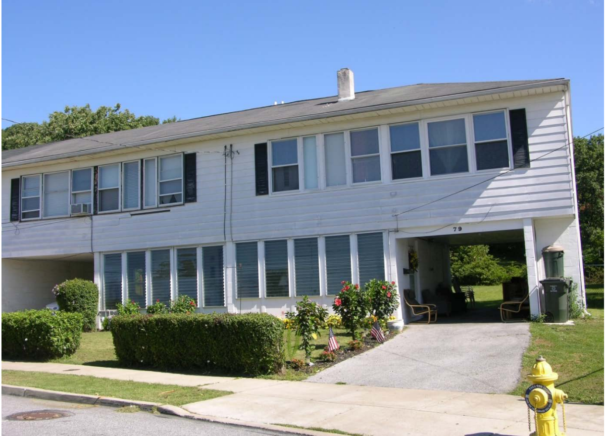
Photo 11: Plan CC; 73-79 Foundry Street. Photo shows 77 and 79; both porches enclosed, carports open. Camera facing N.
