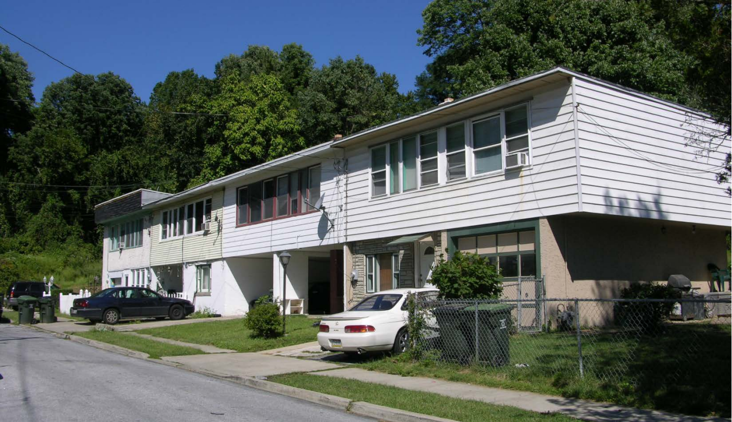
Photo 5: Houses on N side of Brook Lane; camera facing NW. Carport at E end has been enclosed as garage; some former porches enclosed. House at W end has a faux mansard roof. Plan CC.
