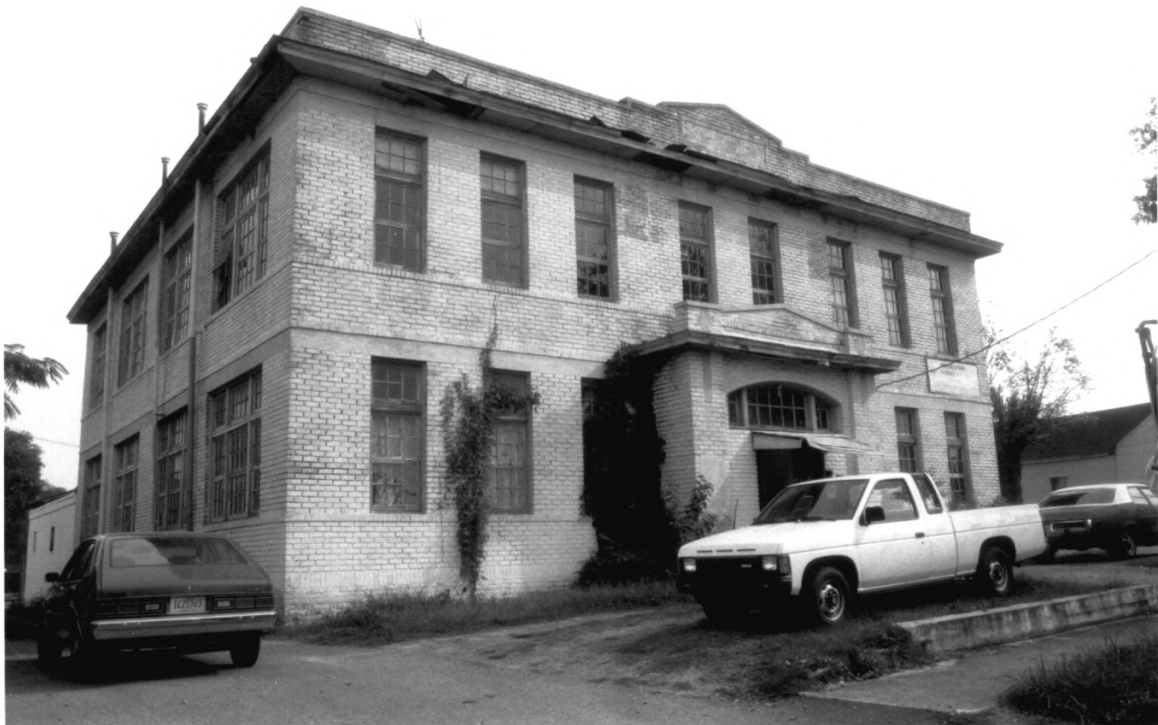
Bradley Academy Rutherford County TN
