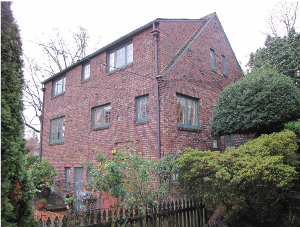
3 of 17 House exterior northeast corner.
