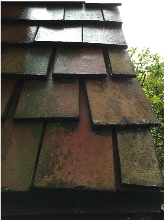
7 of 17 Detail of clay tile roof.
