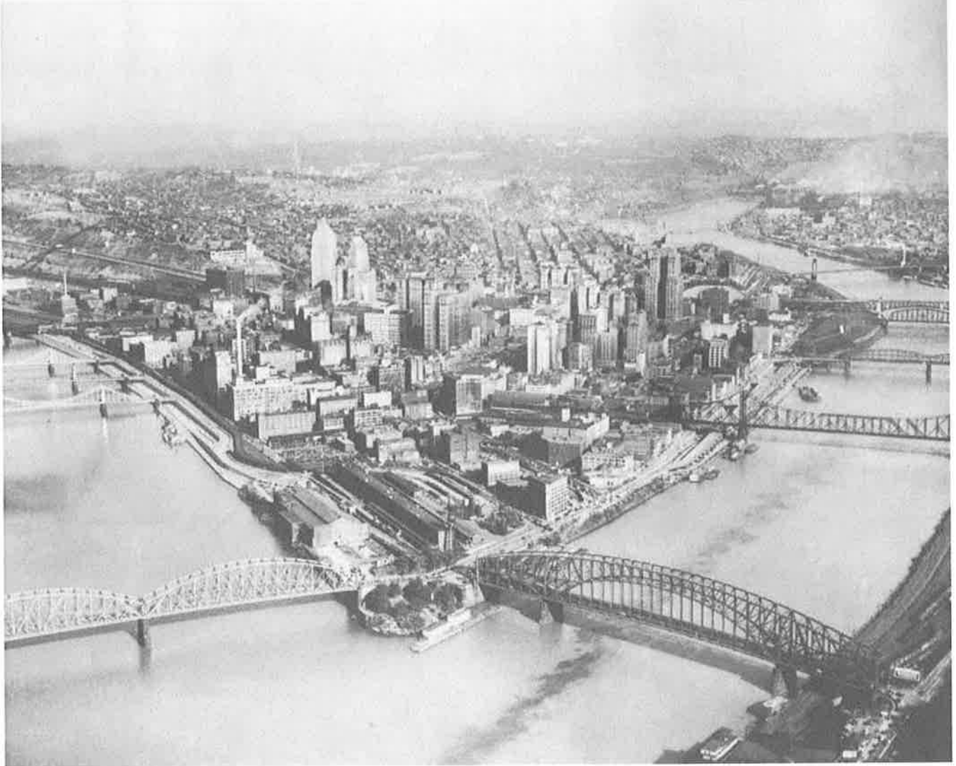
Figure 13: The Golden Triangle in 1947. The two point bridges and the 93 buildings in the foreground will be razed to make way for Gateway Center and Point State Park as the most dramatic and highly visible initiative of the Pittsburgh Renaissance (Allegheny Conference on Community Development 1956:4).
