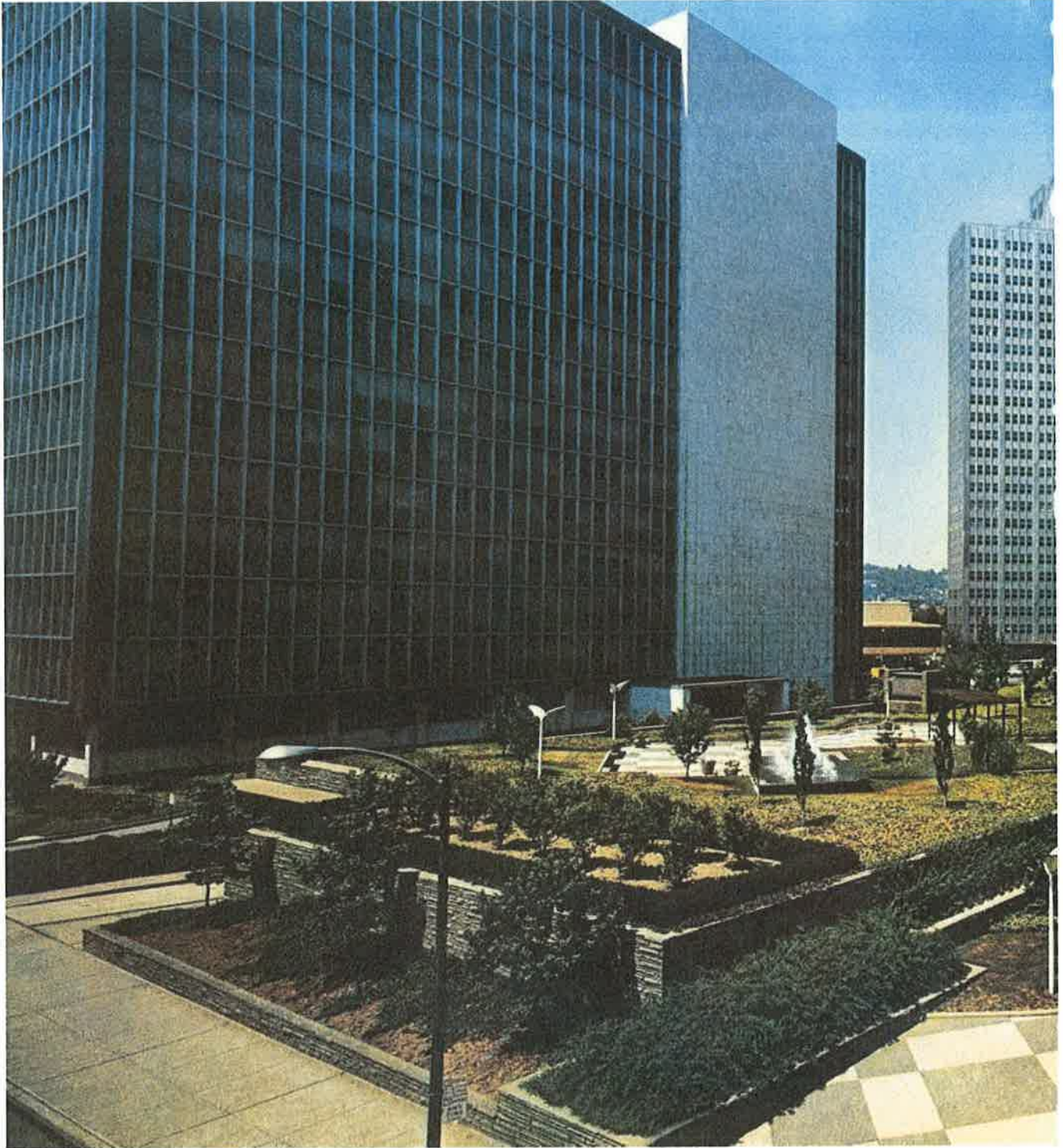
Figure 1: View of the State Office Building (left) and Equitable Plaza prior to the construction of the pedestrian bridge over the Boulevard of the Allies (bottom left corner). Note the original curtain wall configuration of the State Office Building (Ben Rosen Associates c. 1964:2).
