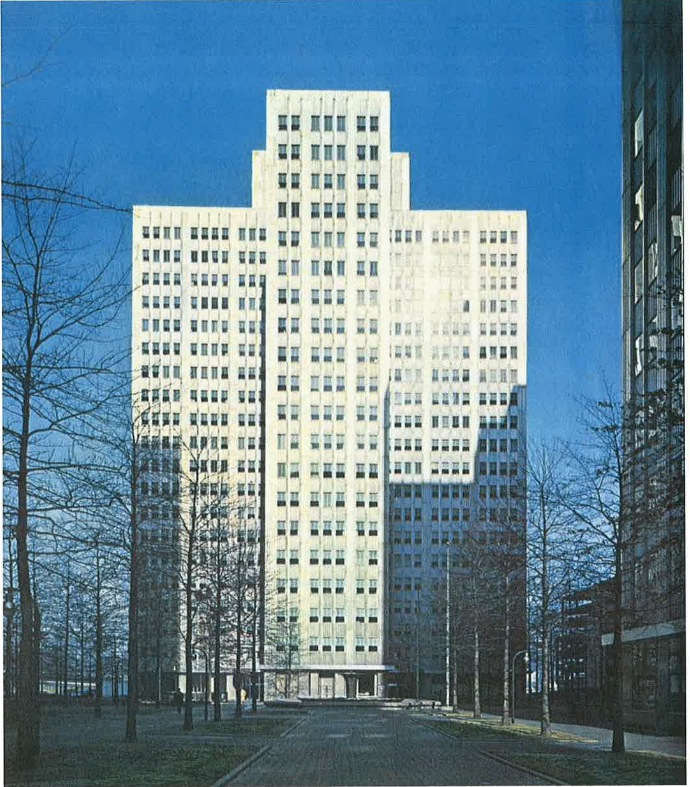
Figure 3: View of One Gateway Center with Gateway Plaza and fountain in the foreground (Ben Rosen Associates c. 1964:12).
