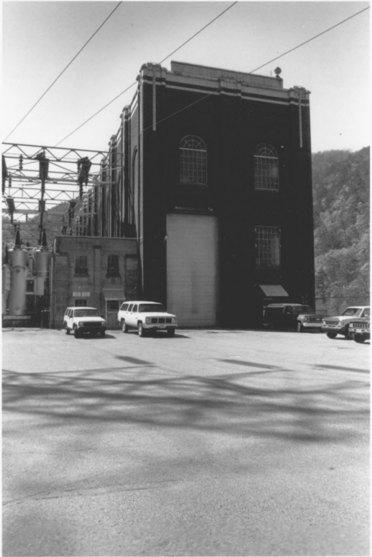
Calderwood Hydroelectric Station Calderwood vicinity, Blount & Monroe Cos., TN
