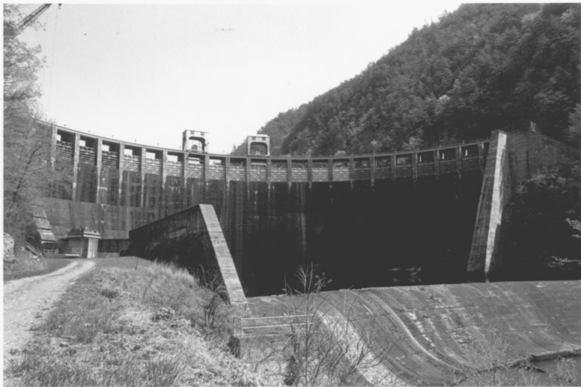
Calderwood Hydroelectric Station Calderwood vicinity, Blount & Monroe Co's, TN
