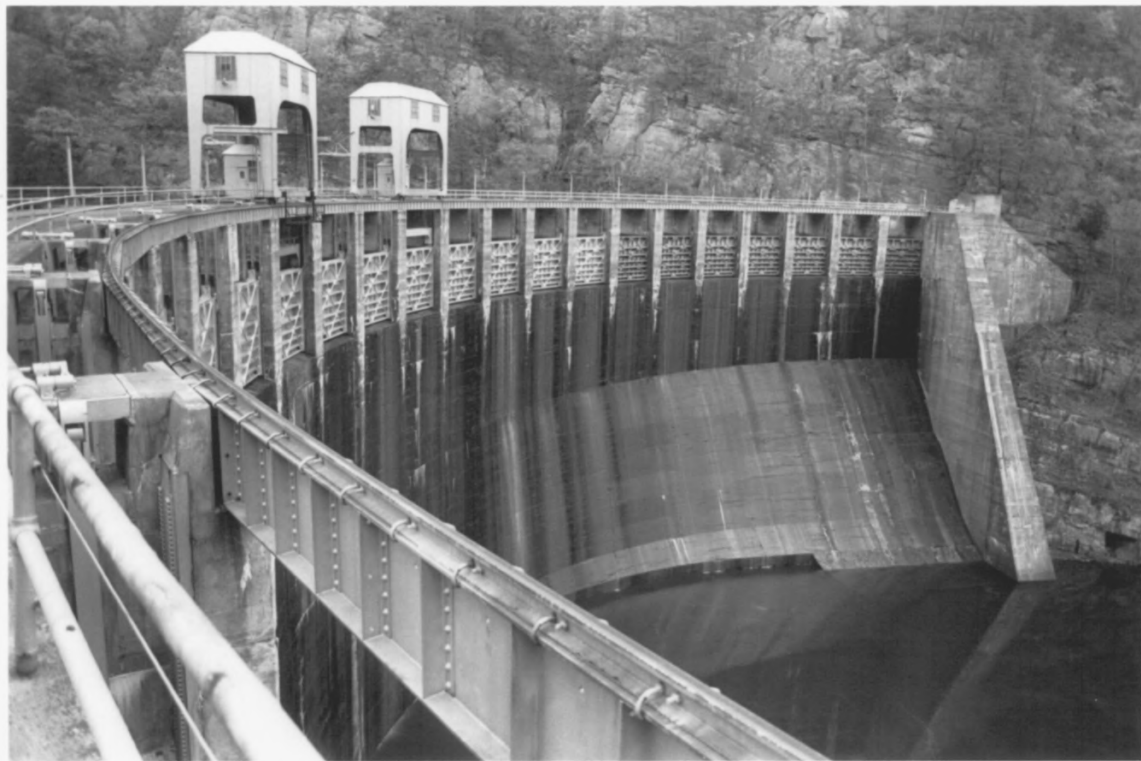
Calderwood Hydroelectric Station Calderwood vicinity, Blount & Monroe Co's, TN #9 of 9
