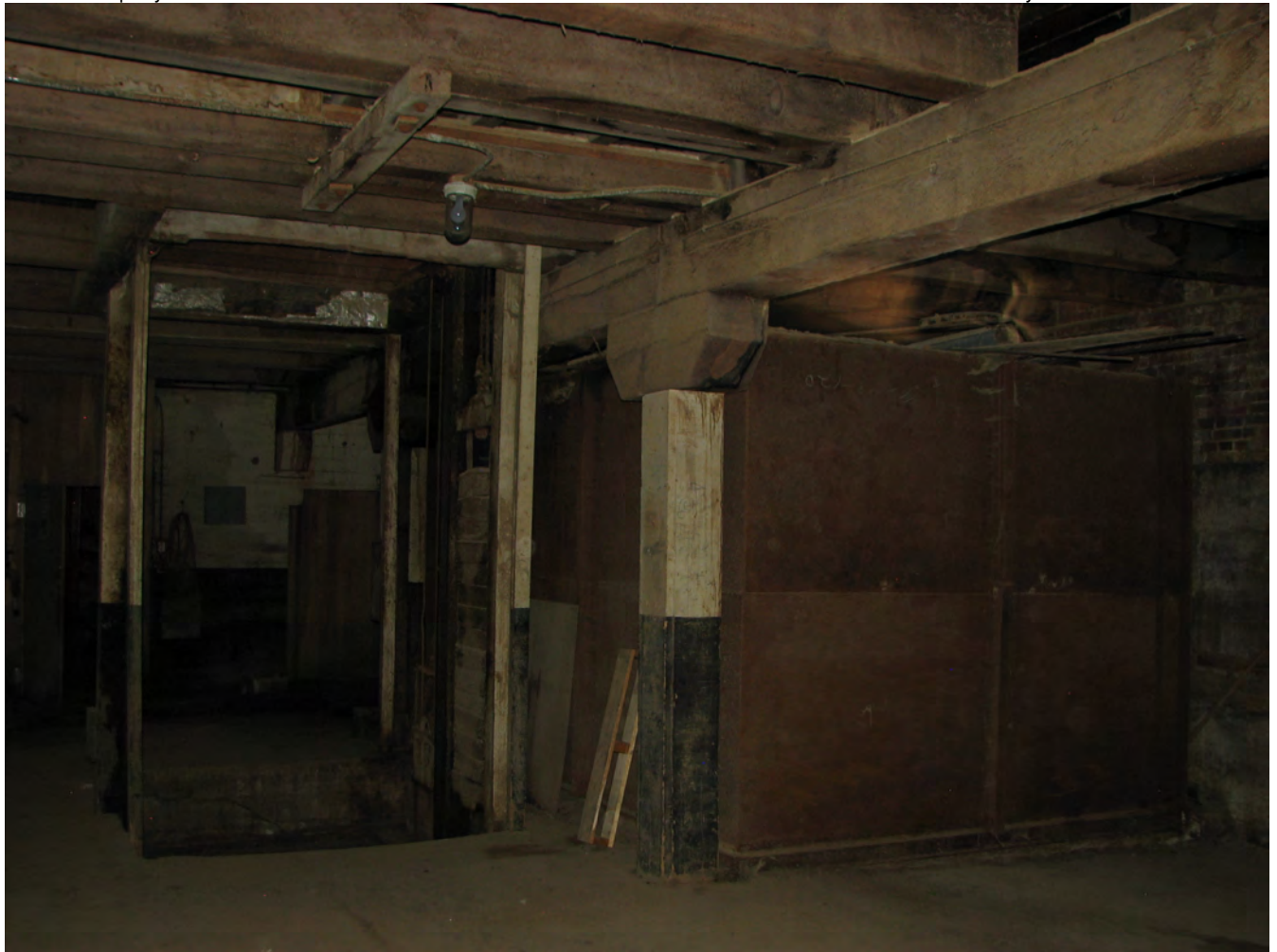
Photo MT_FergusCounty_Gamble-RobinsonCoWarehouse_0010. Interior, Basement with Freight Elevator, facing: N
