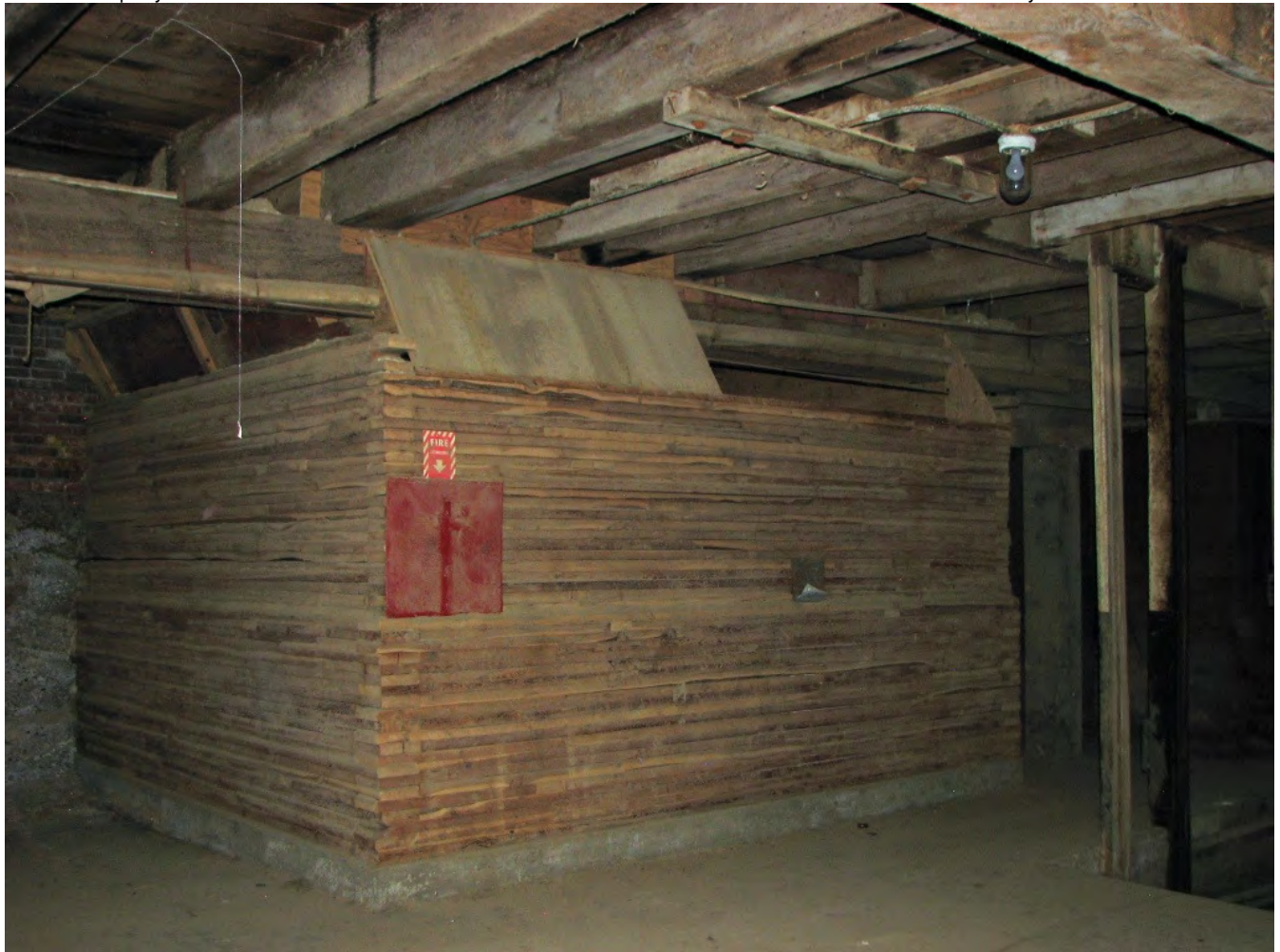
Photo MT_FergusCounty_Gamble-RobinsonCoWarehouse_0011. Interior, Wood Storage Crib in Basement, facing: S
