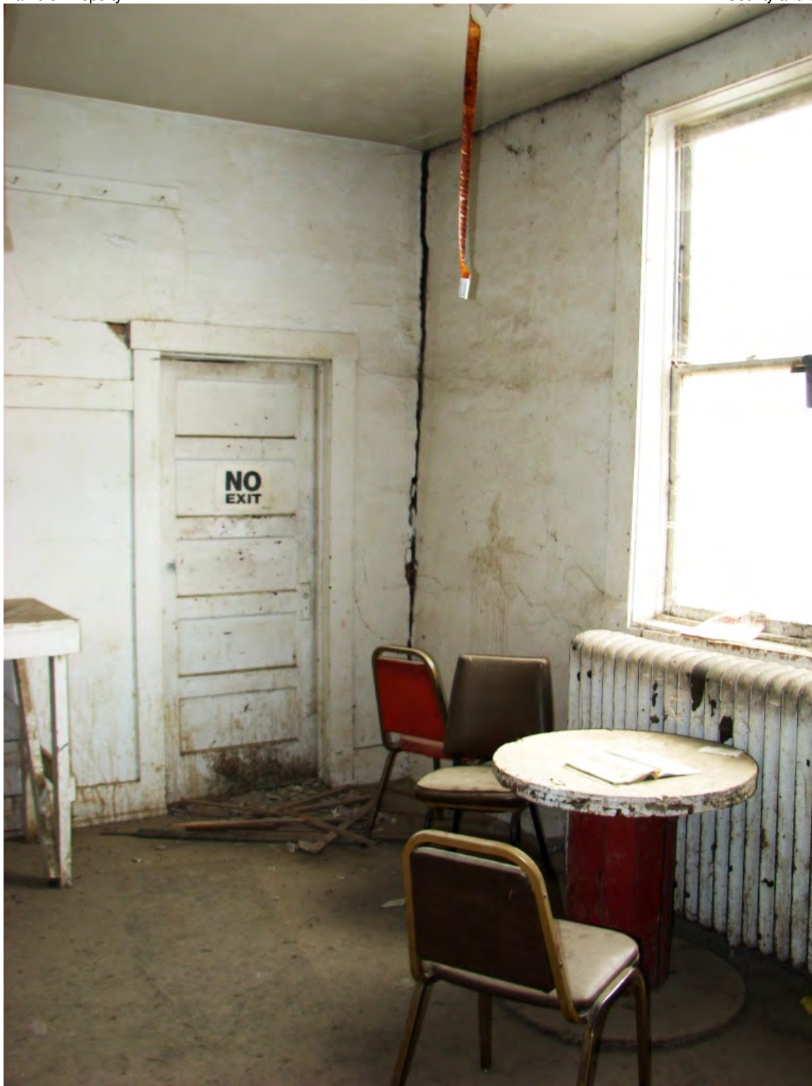
Photo MT_FergusCounty_Gamble-RobinsonCoWarehouse_0008. Interior, Detail of East Office, facing: SE
