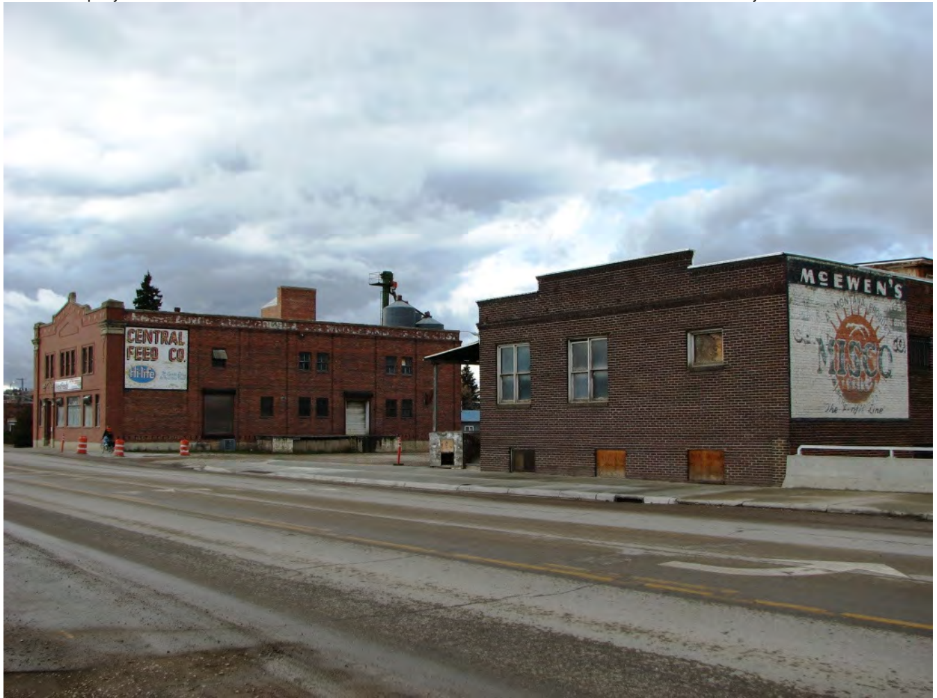
Photo MT_FergusCounty_Gamble-RobinsonCoWarehouse_0012. Overview of Gamble Robinson Co. Warehouse and Lewistown Mercantile Company (Nash-Finch Co), facing: W
