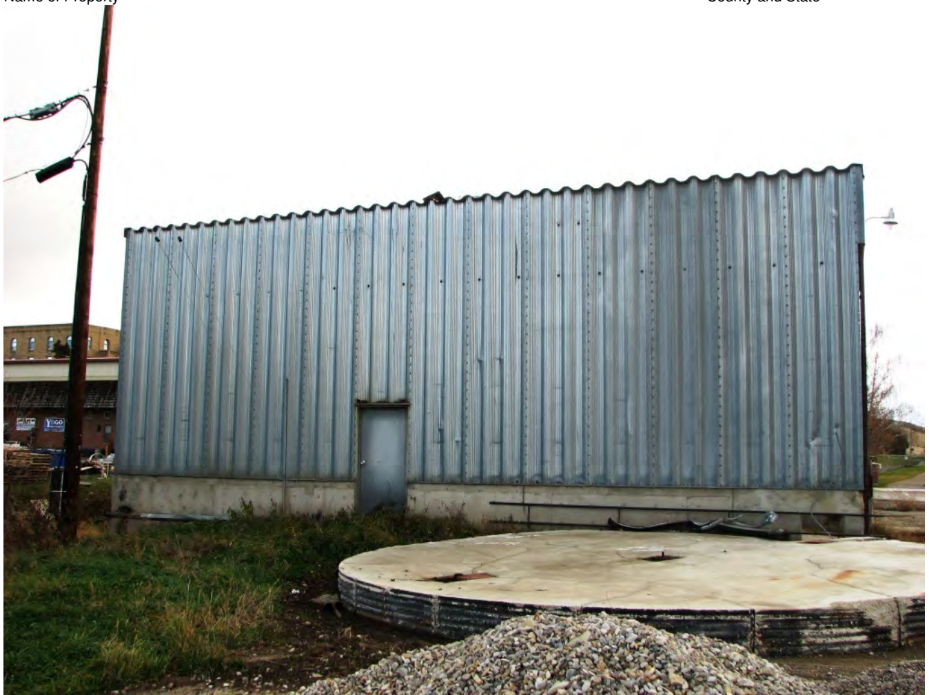
Photo MT_FergusCounty_Gamble-RobinsonCoWarehouse_0006. North "Rear" Elevation of Metal Addition, facing: SE
