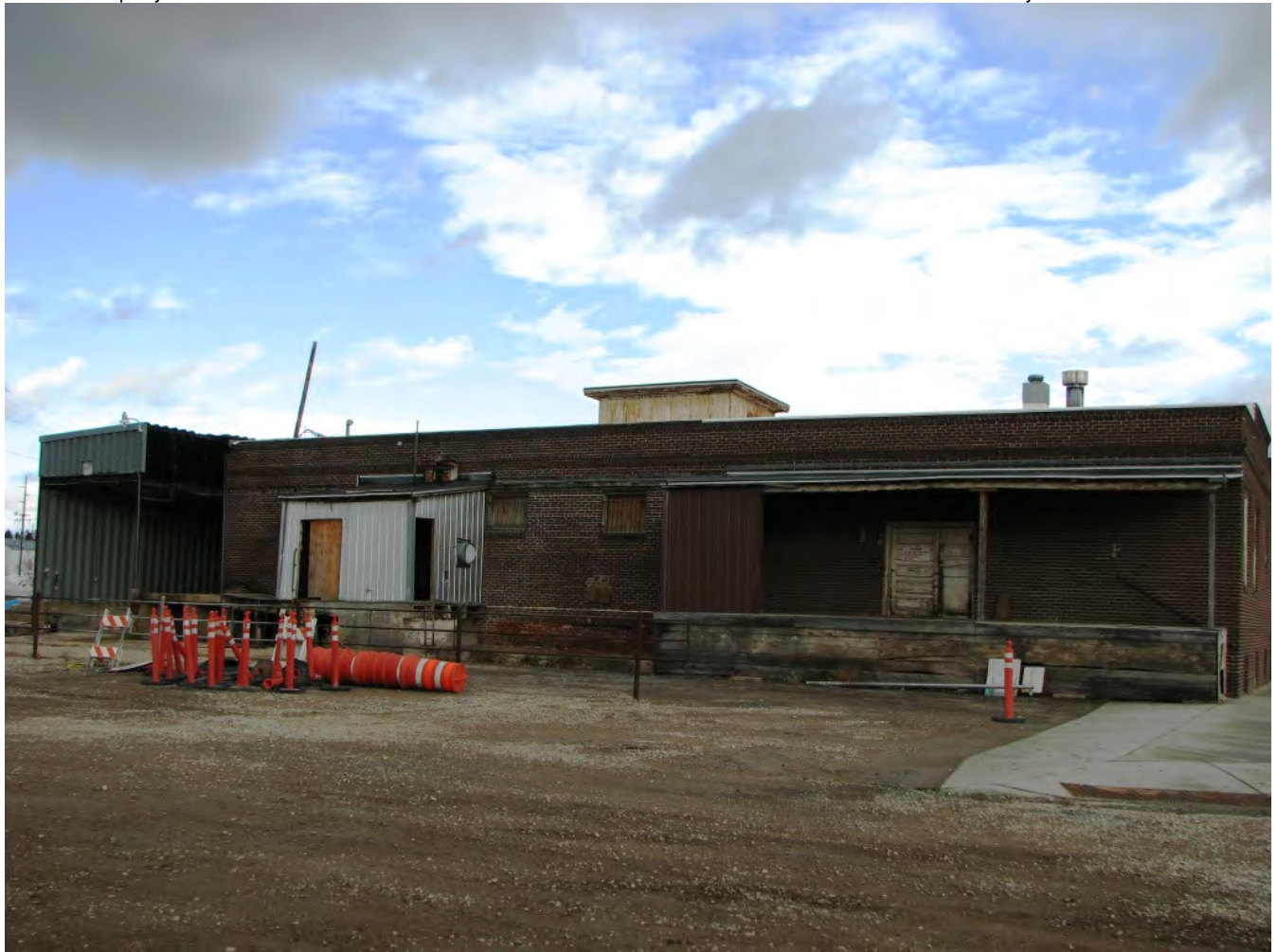
Photo MT_FergusCounty_Gamble-RobinsonCoWarehouse_0002. West "Rail-Side" Façade, facing: N
