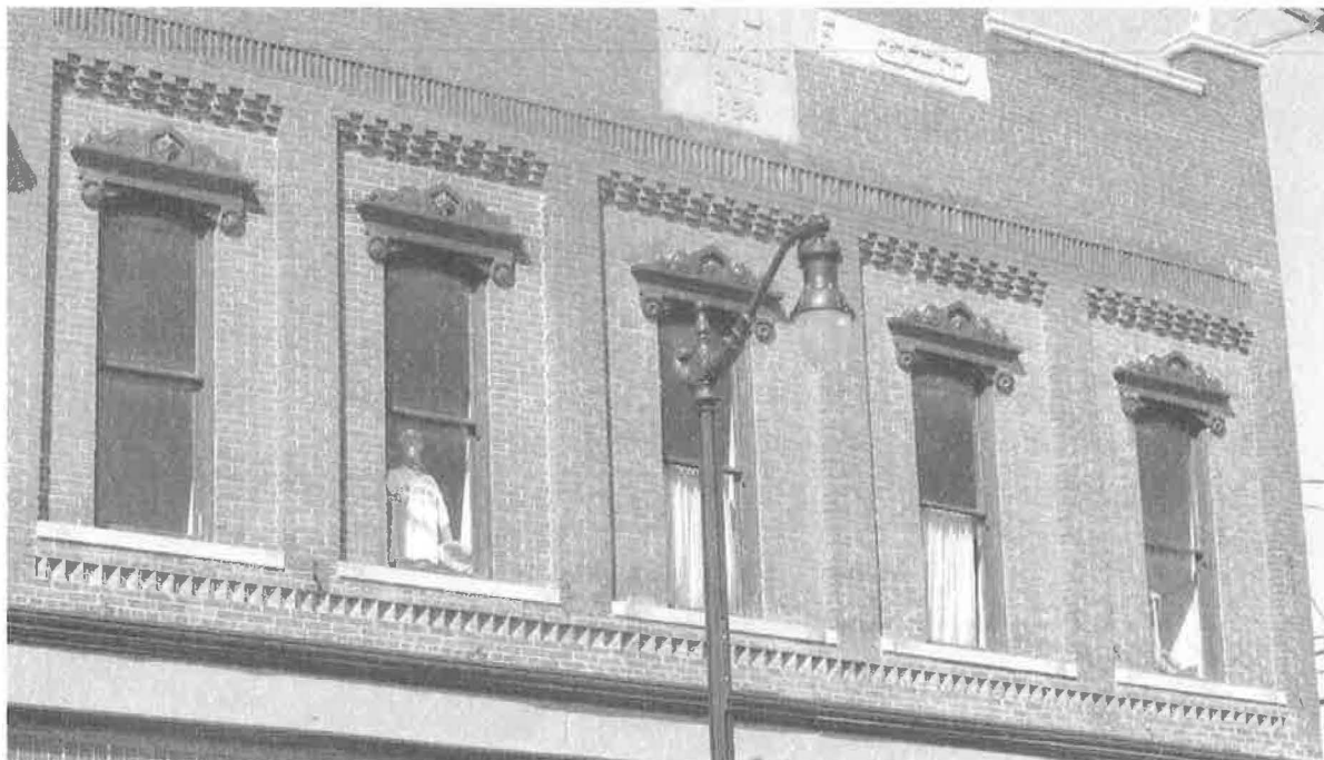
Figure 16. I.O.O.F. Hall constructed in 1892 and 1925. Note differences in cornices above second-story windows.
