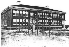
1910 ca. East Elevation, new addition. Tacoma Public Schools Collection
