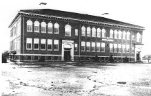
1928 East Elevation Boland Collection, Tacoma Public Library
