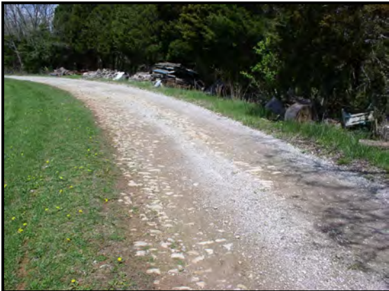
Turnpike roadbed section – 3 of 4
