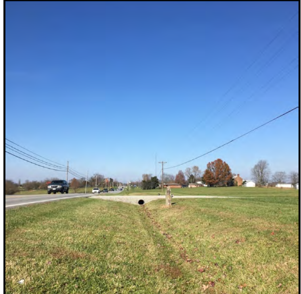
"34L 5B" location view – looking north
