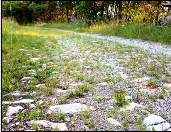
Turnpike roadbed section – 1 of 4
