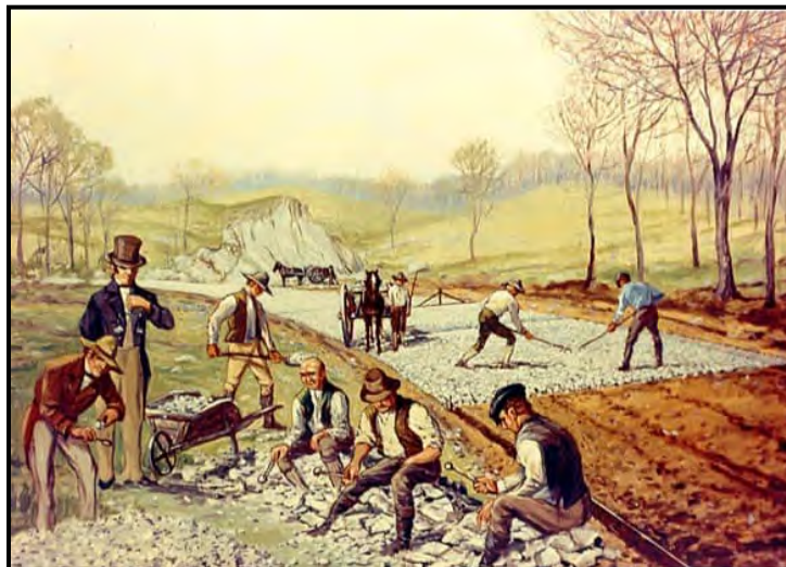
Road construction by the “McAdams Plan” “1823 – First American Macadam Road”, ( Painting by Carl Rakeman ) U.S. Department of Transportation, 2008
