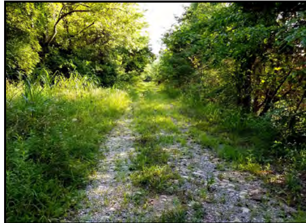
Turnpike roadbed section – 4 of 4
