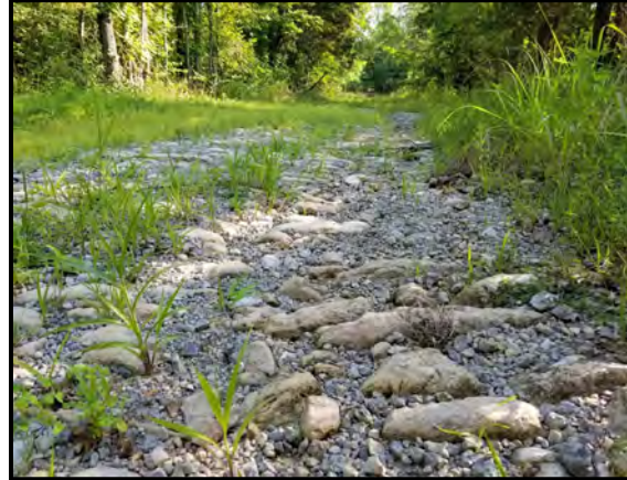
Turnpike roadbed section – 2 of 4
