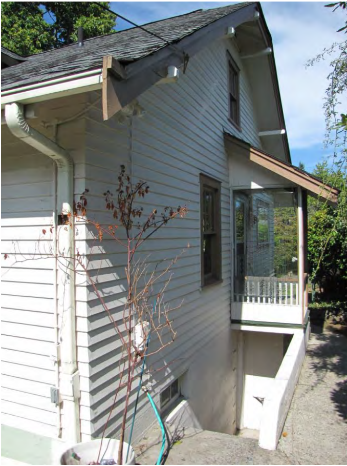
6 of 11 Southeast corner showing exterior basement entry.
