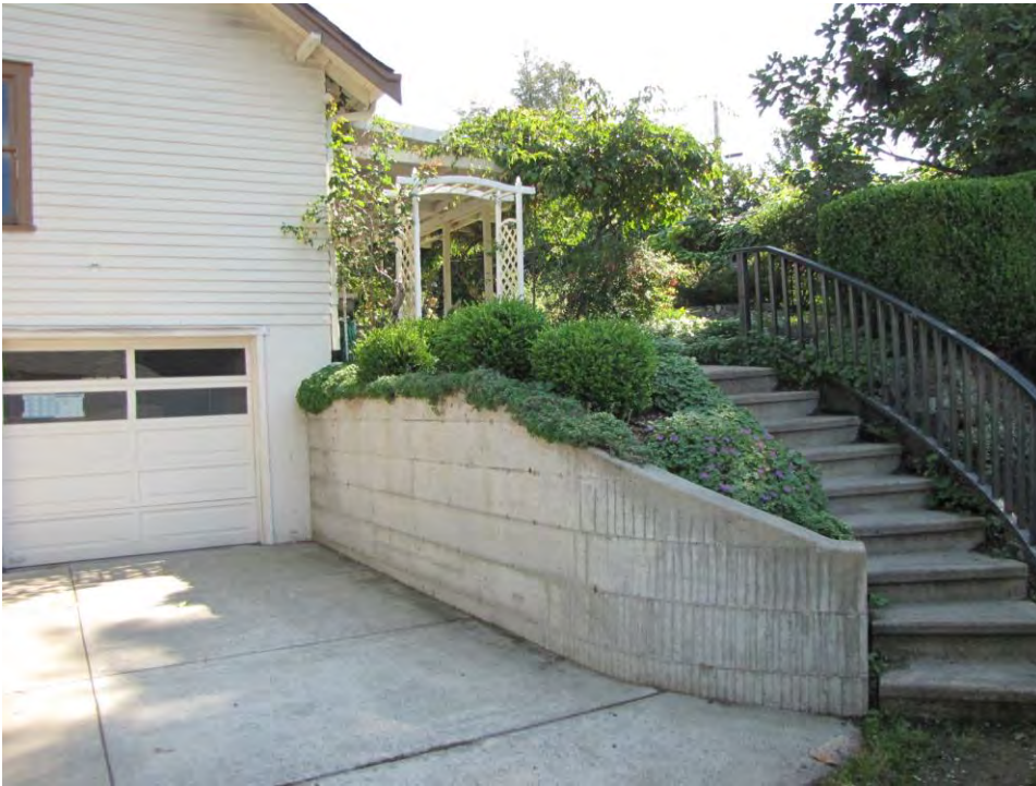
4 of 11 West Elevation retaining wall detail and backyard access
