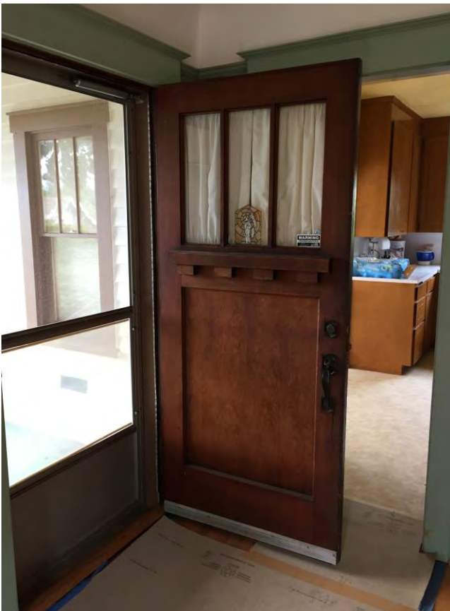
9 of 11 Entry door detail
