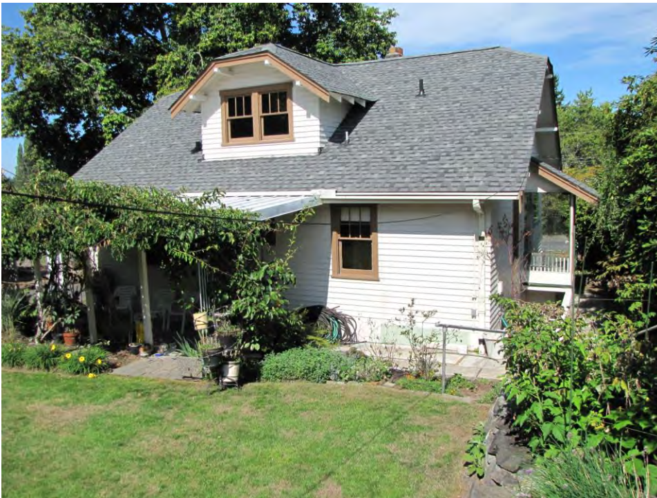
5 of 11 South/Rear Elevation
