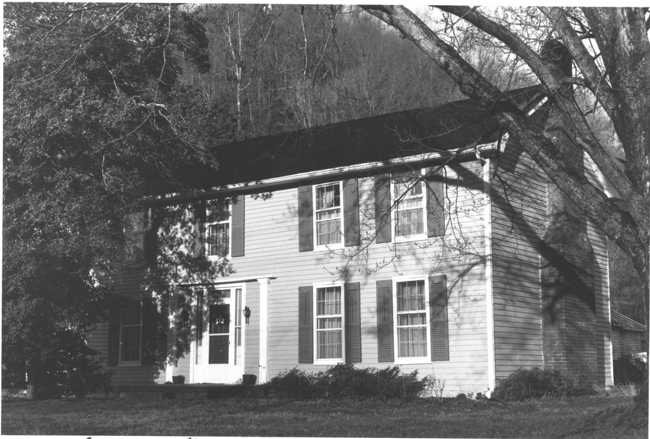
Aaron Atherton House, U-6 Lancaster County MRA
