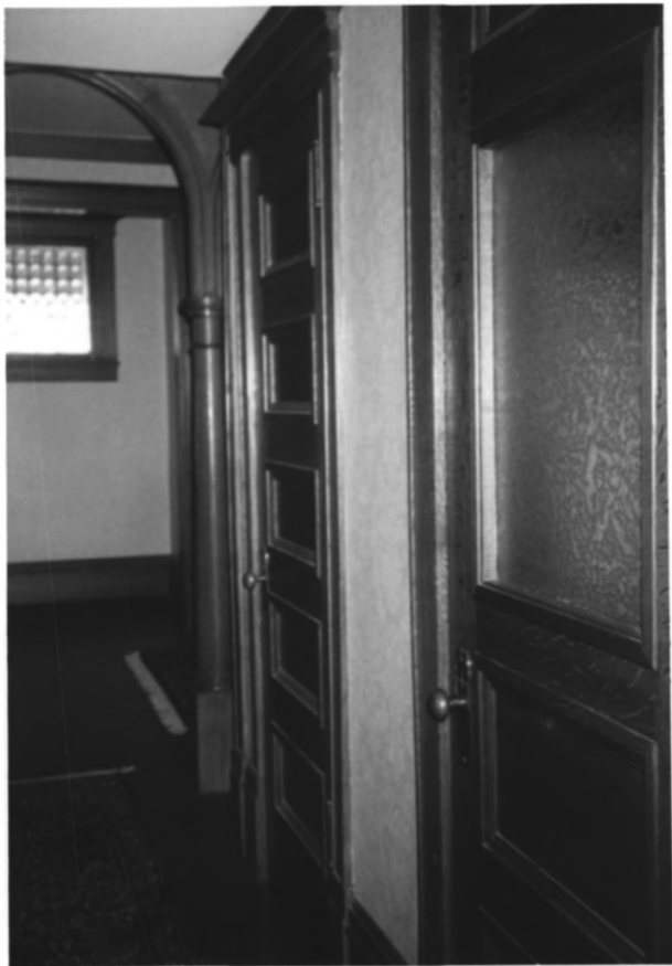
Nylius-Eaton House Woodbury County, Iowa 21
