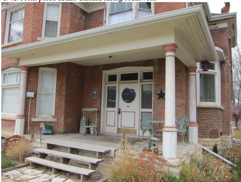
Photograph 9 of 19. Front porch detail. Camera facing southwest.
