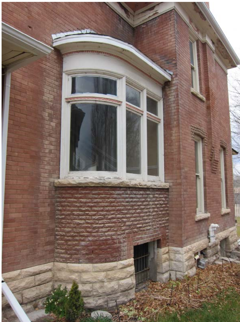
Photograph 11 of 19. Rounded projecting bay with staircase. Camera facing southwest.
