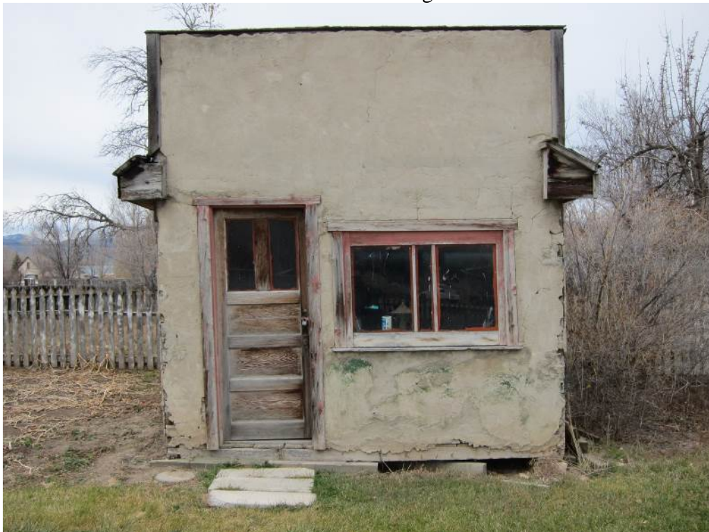
Photograph 7 of 19. View of shed East elevation. Camera facing west.
