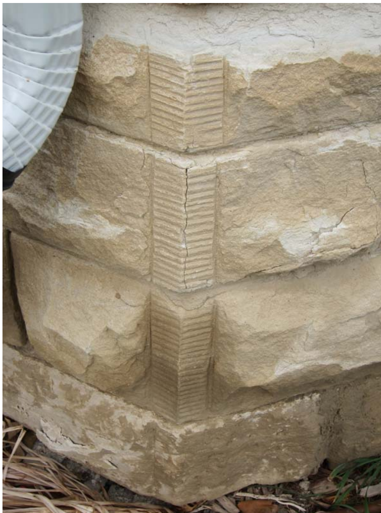
Photograph 10 of 19. Foundation stonework detail. Camera facing Northwest.
