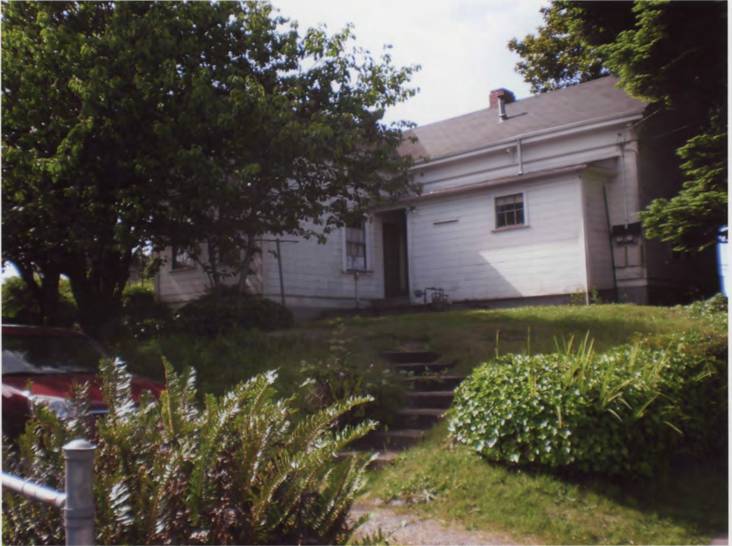
CA_Humboldt_Chapman House_0006.tif: Building rear showing 1874 building on right, facing southeast
