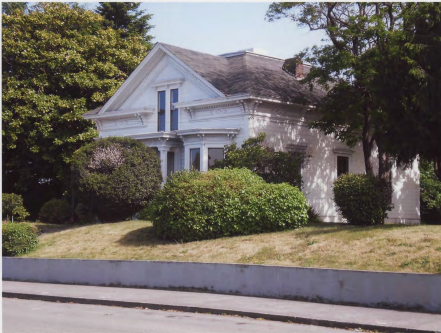
CA_Humboldt_Chapman House_0004.tif: Concrete retaining wall and primary façade, facing northwest
