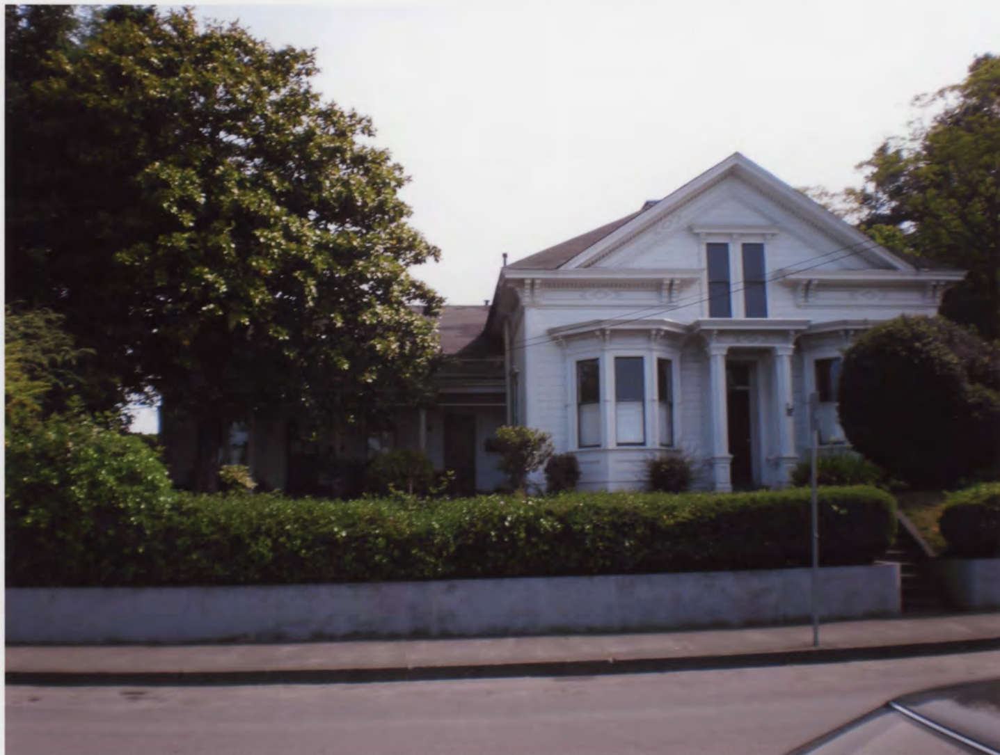
CA_Humboldt_Chapman House_0005.tif: Primary façade showing 1874 building on left, facing north
