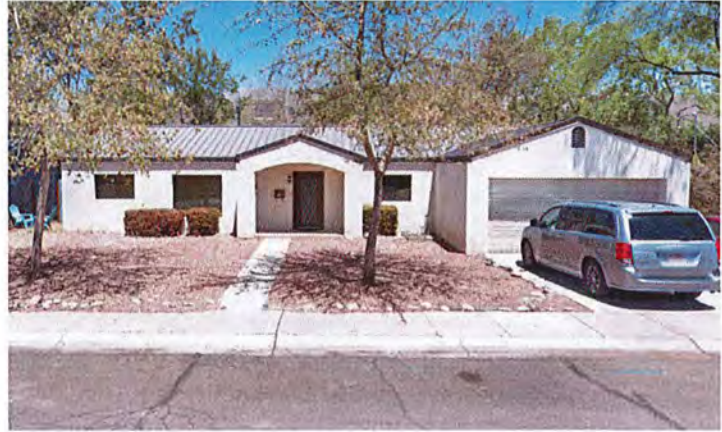
Figure 10. House at 312 E. 14th St. Source: Google, 2018.
