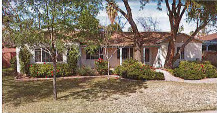
Figure 2. House at 32 E. 14th St. Source: Google, 2018.
