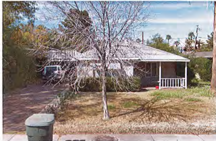
Figure 1. House at 8 E. 14th St. Source: Google, 2018.
