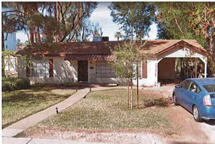
Figure 3. House at 126 E. 14th St. Source: Google, 2018.
