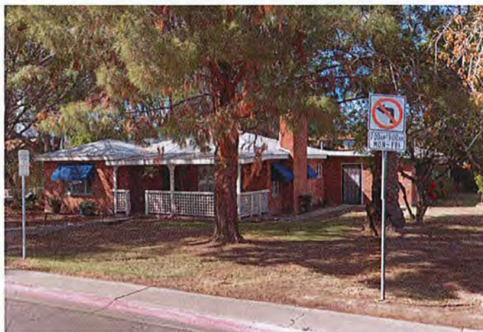
Figure 4. House at 130 E. 14th St. Source: Google, 2018.
