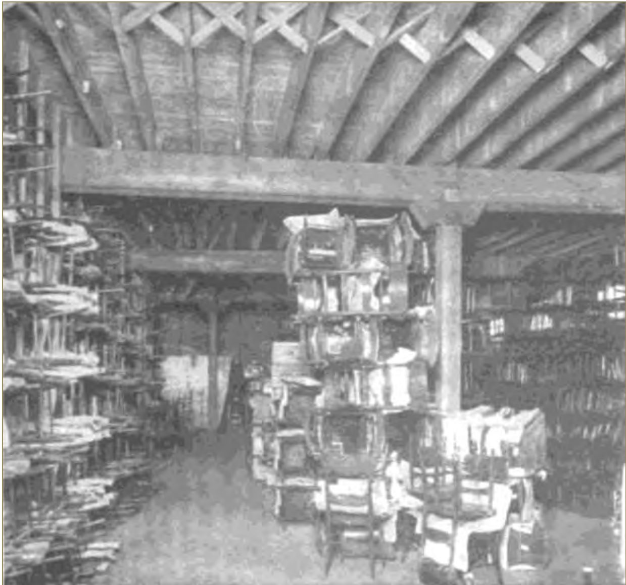
Figure 05. Peck and Hills Warehouse, Section B interior, 1911
