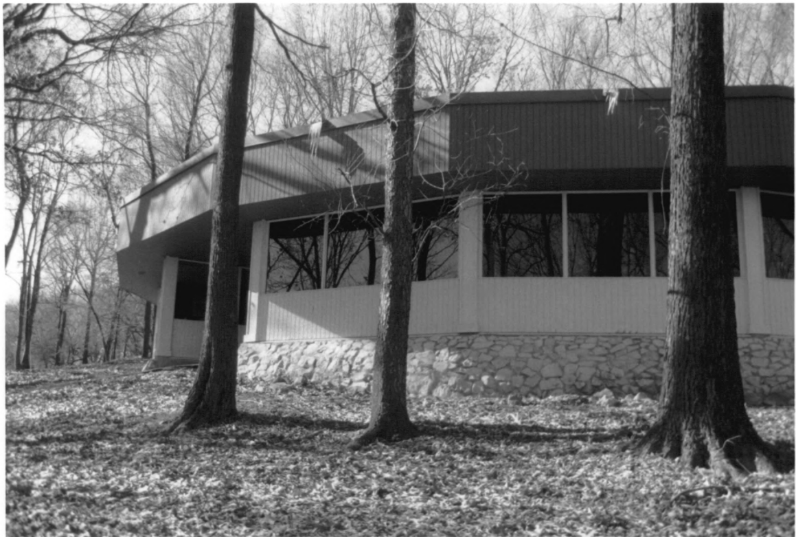
Johnsonville Historic District Humphreys Co. TN
