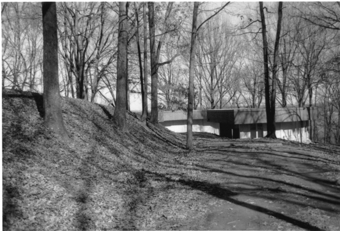
Johnsonville Historic District Humphreys Co. TN
