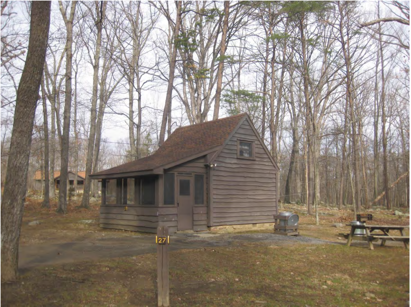
Photo 21: Cabin No. 27, camera facing west
