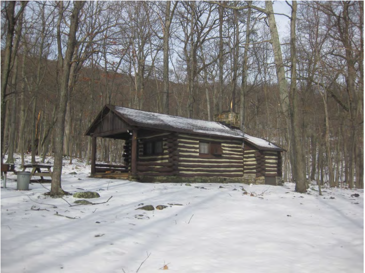
Photo 15: Cabin No. 7, camera facing north
