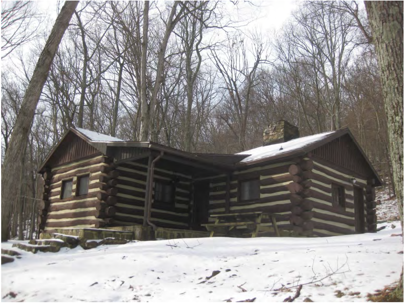
Photo 13: Cabin No. 2, camera facing south
