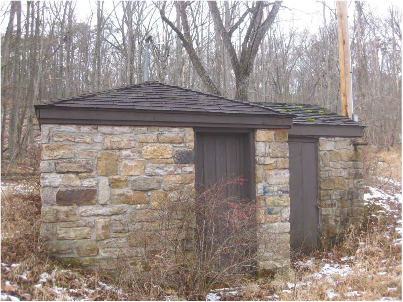
Photo 10: Springhouse, camera facing north
