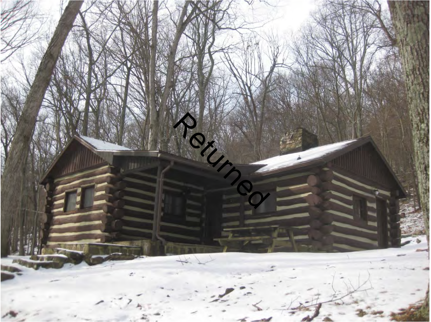
Photo 13: Cabin No. 2, camera facing north
