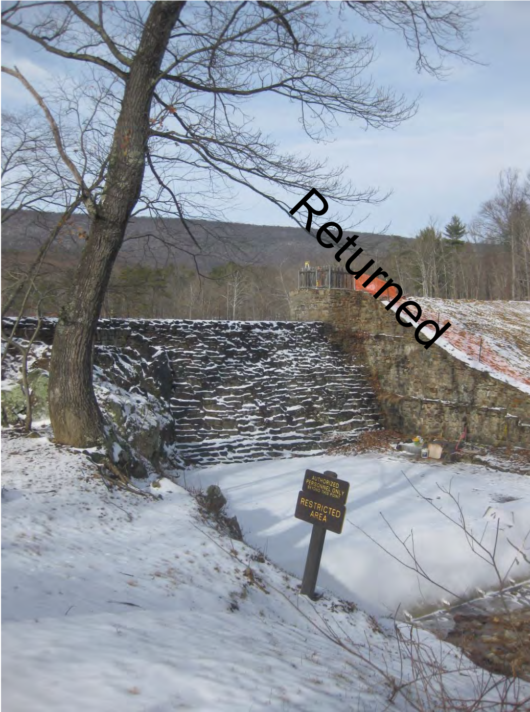
Photo 6: Cacapon Dam, camera facing west
