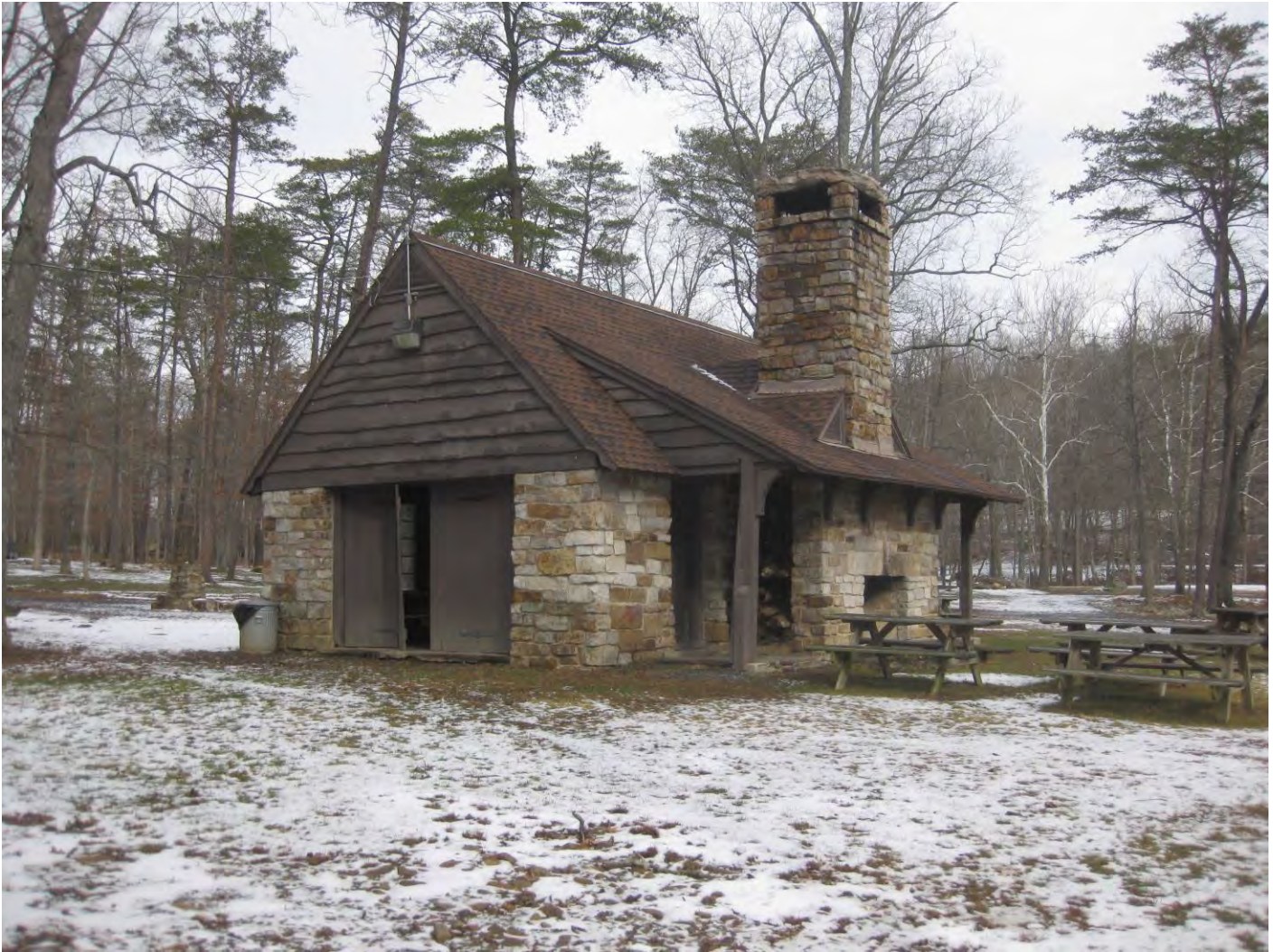
Photo 7: Lake Picnic Shelter, camera facing northeast
