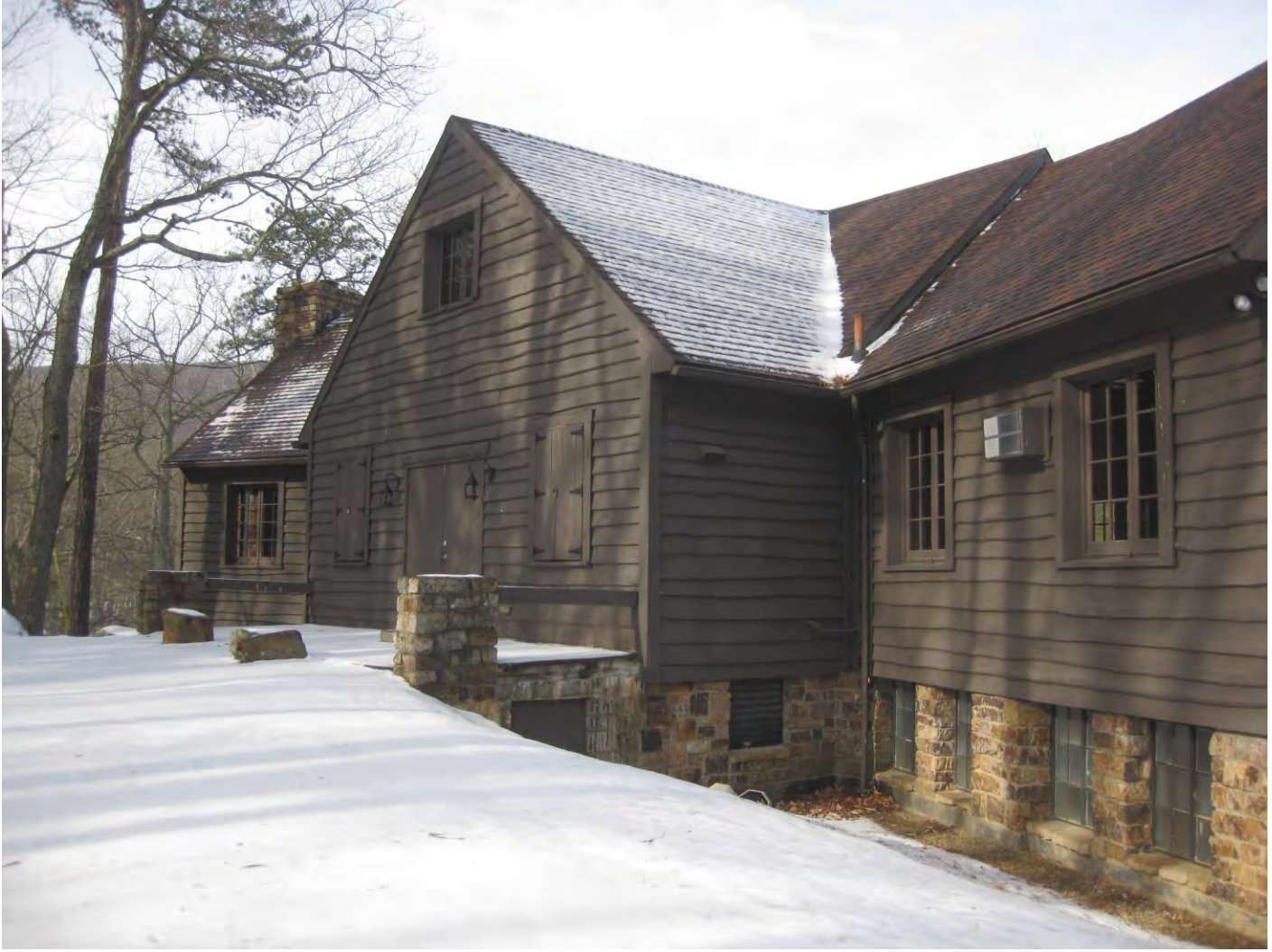
Photo 8: Lake Bathhouse, camera facing northwest
