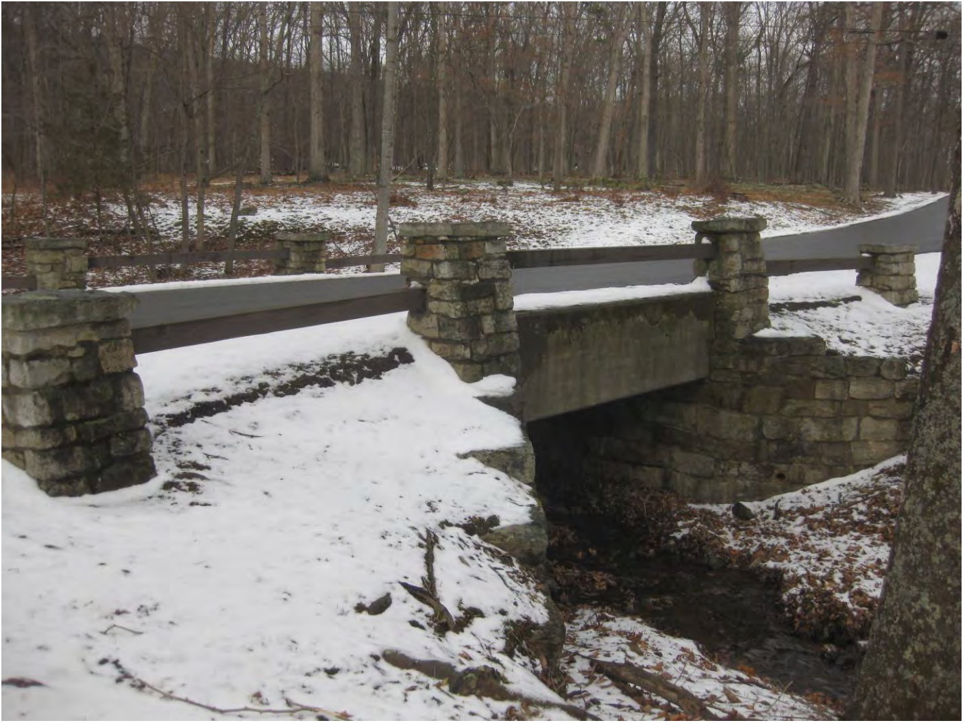
Photo 3: Vehicular Bridge, detail
