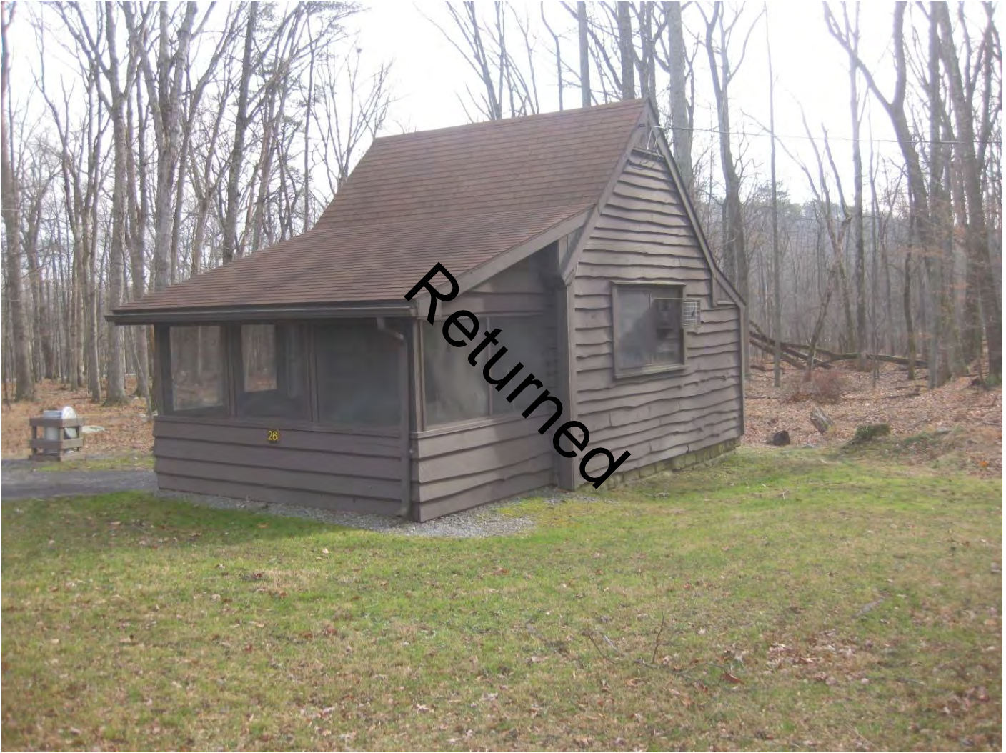
Photo 20: Cabin No. 26 camera facing south
