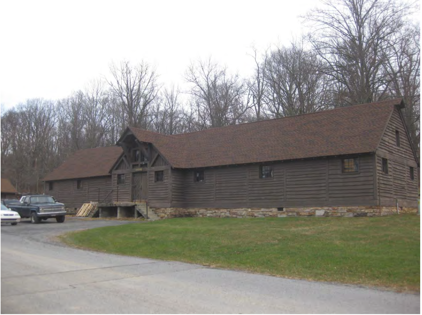
Photo 25: Main Supply House, camera facing northeast
