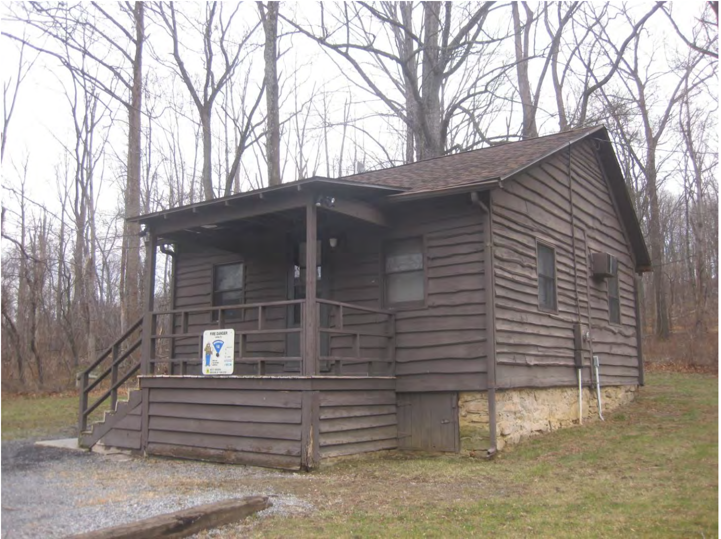
Photo 22: Park Headquarters - Ranger's Residence, camera facing east
