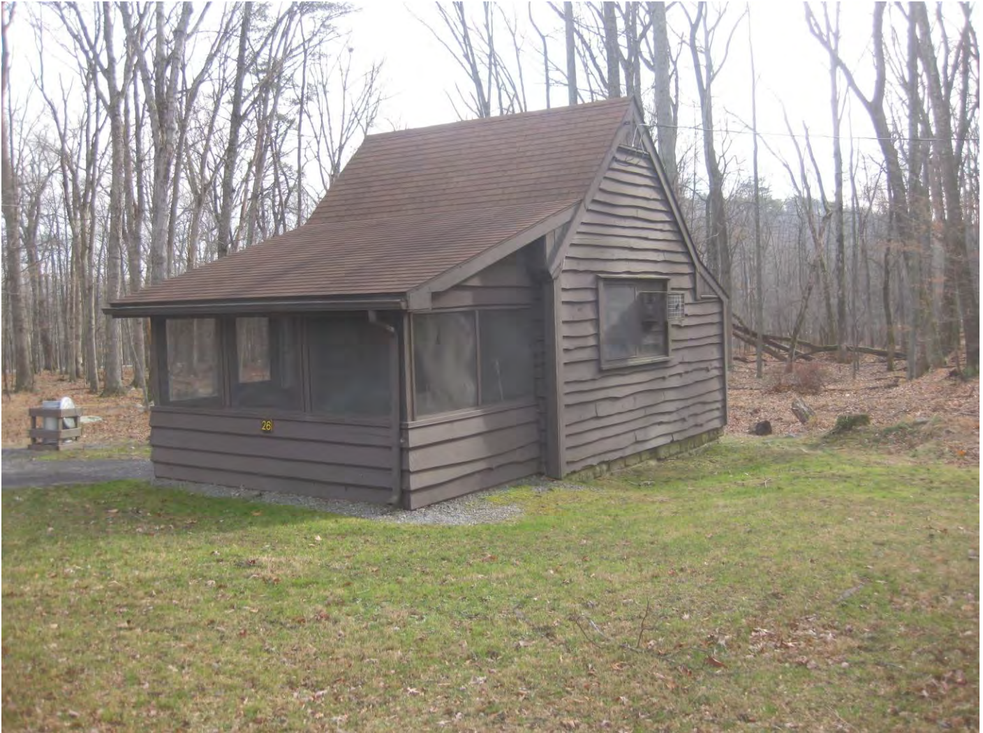
Photo 20: Cabin No. 26 camera facing south
