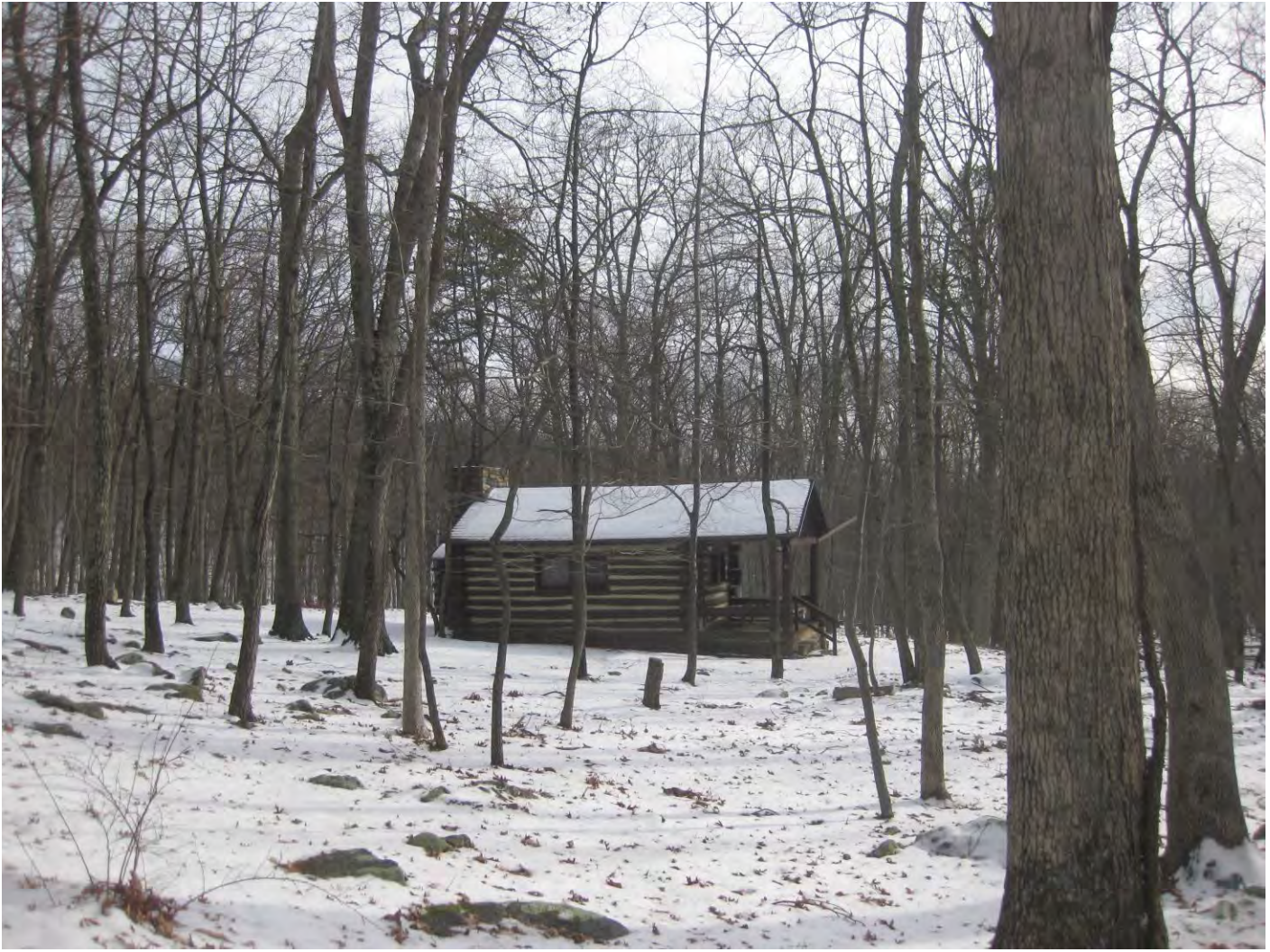
Photo 14: Cabin No. 5, camera facing south
