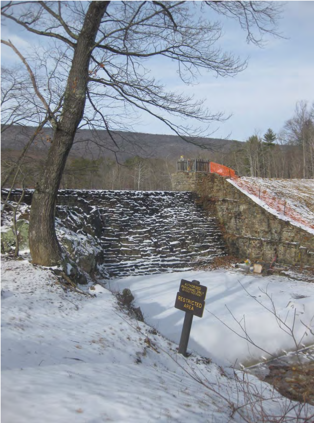
Photo 6: Cacapon Dam, camera facing west
