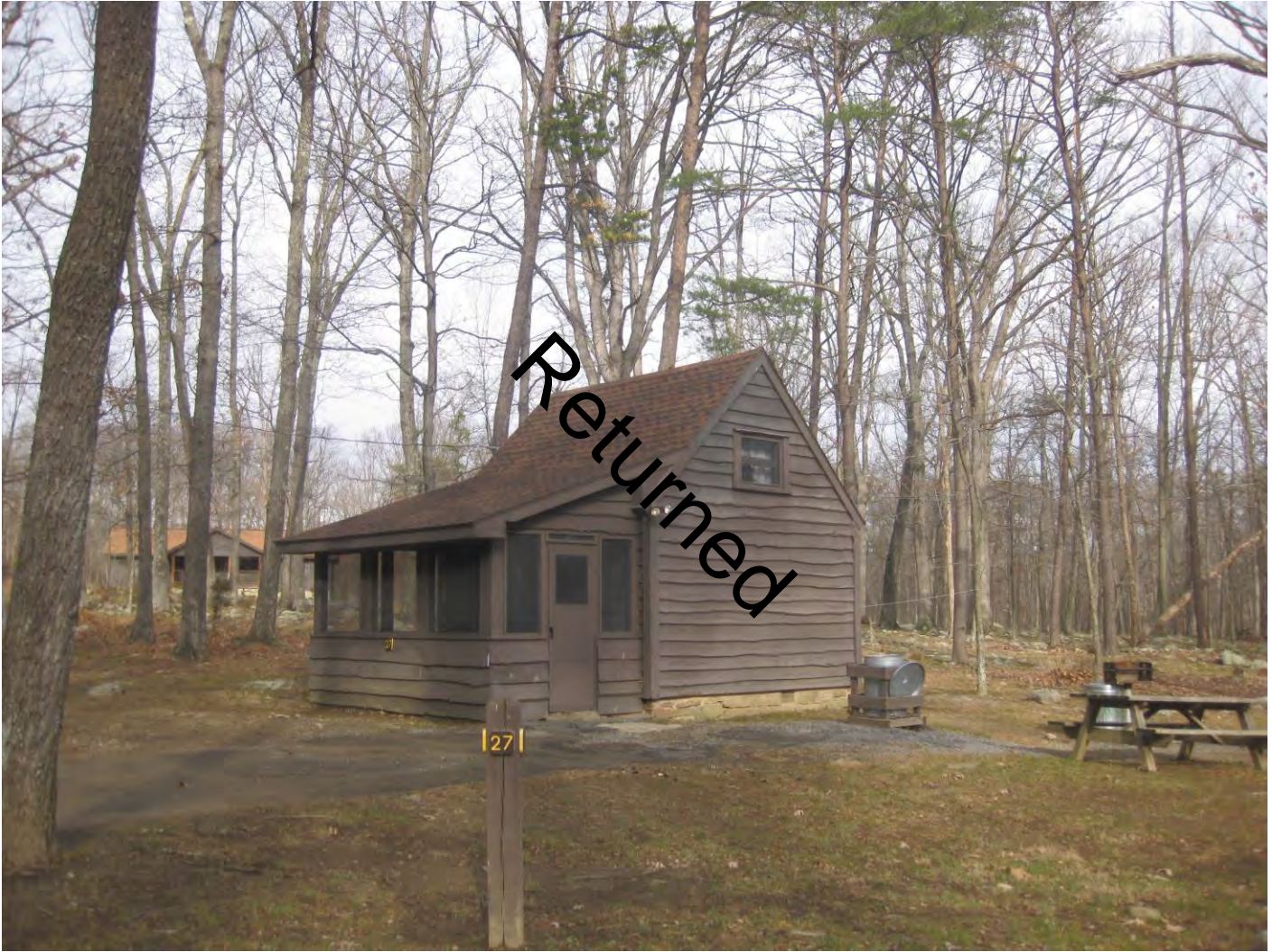
Photo 21: Cabin No. 27, camera facing west
