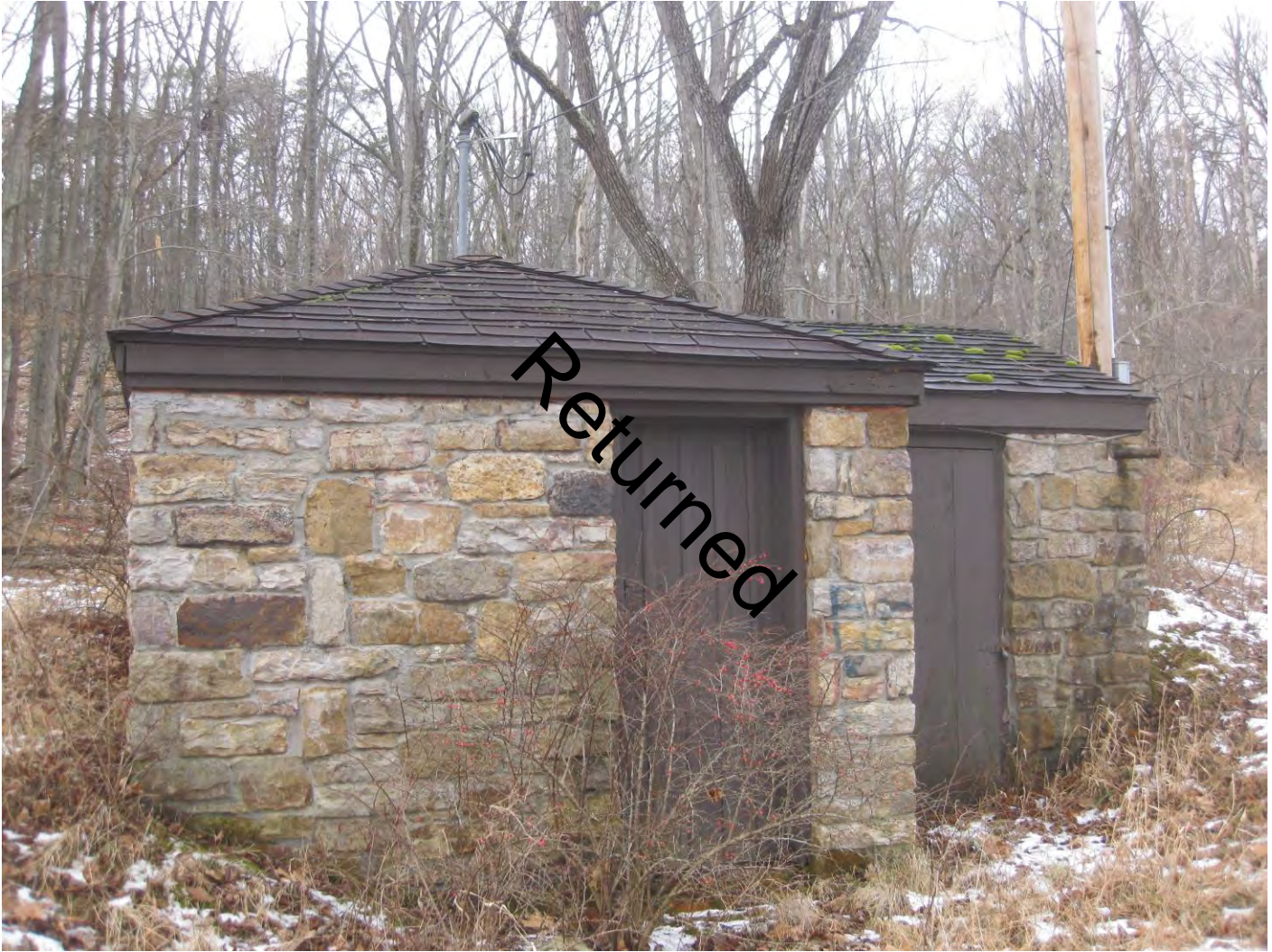
Photo 10: Springhouse, camera facing north
