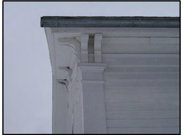
Figure 2. Paired brackets and corner boards.
