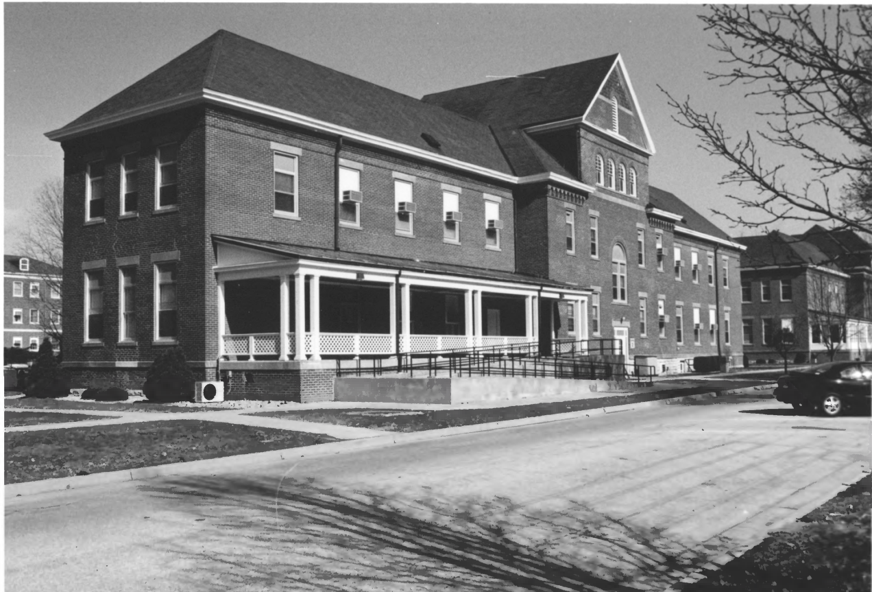
MARION BRANCH, NATIONAL HOME FOR DISABLED VOLUNTEER SOLDIERS HISTORIC DISTRICT, CLERMONT COUNTY, IN; PHOTO 5149
