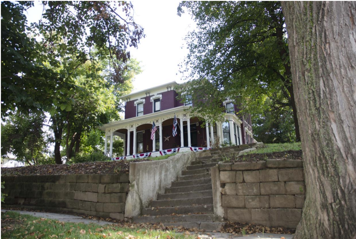
Figure 1: Block retaining wall, concrete steps, and west façade of home; September 2018.
