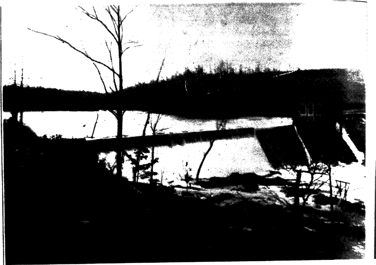
Historic View Lawrenceburg No. 2 Hydroelectric Station Lawrenceburg vicinity, Lawrence Co., TN
