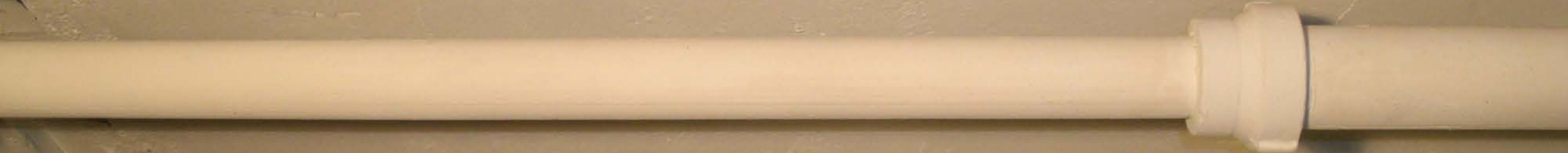
Original Electrical Wooden Raceway
