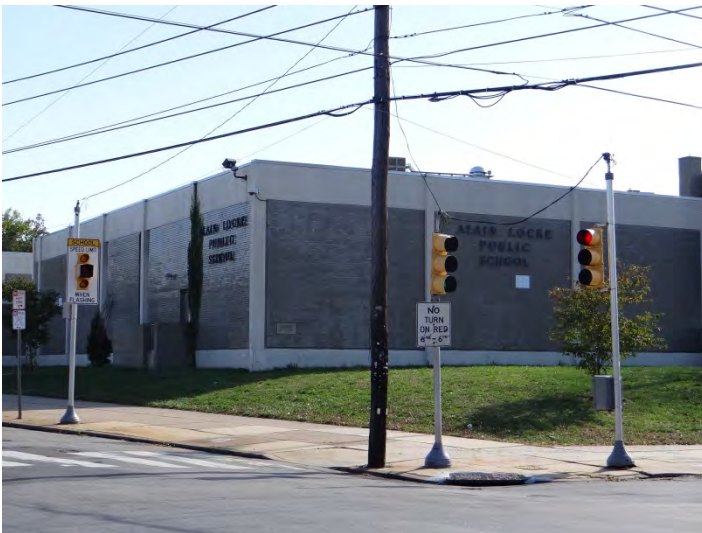
Photo 3: Looking SE at main (N, left) and W (right) facades
