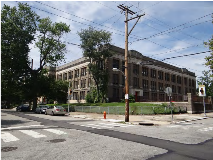
Photo 5: Looking NW at main (SE, left) and NE facades
