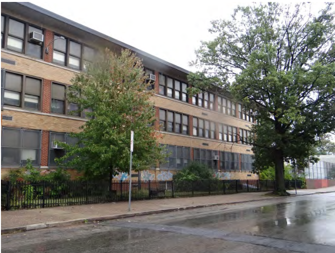
Photo 3: Looking NE at N end of main (SE) façade
