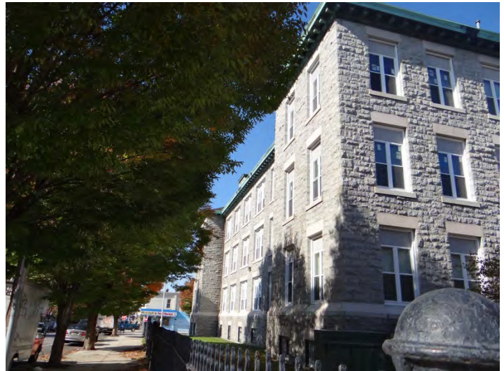
Photo 4: Looking W along S facade
