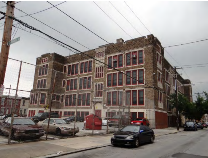
Photo 3: Looking SW at E façade
