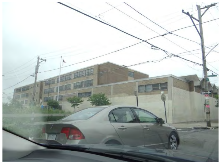
Photo 6: Looking SW at E façade
