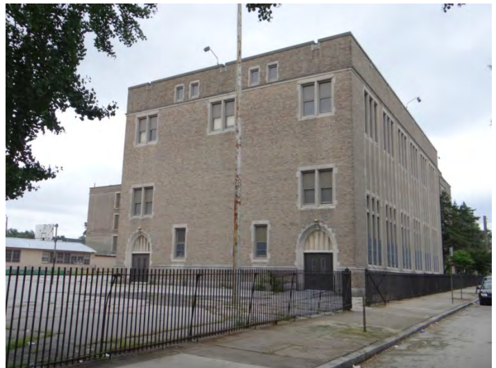
Photo 4: Looking S at NE end of addition
