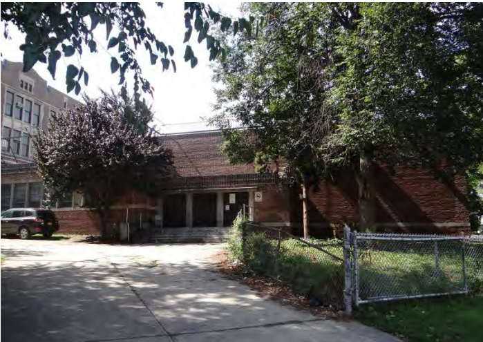
Photo 3: Looking W at main (E) façade, 1953 addition
