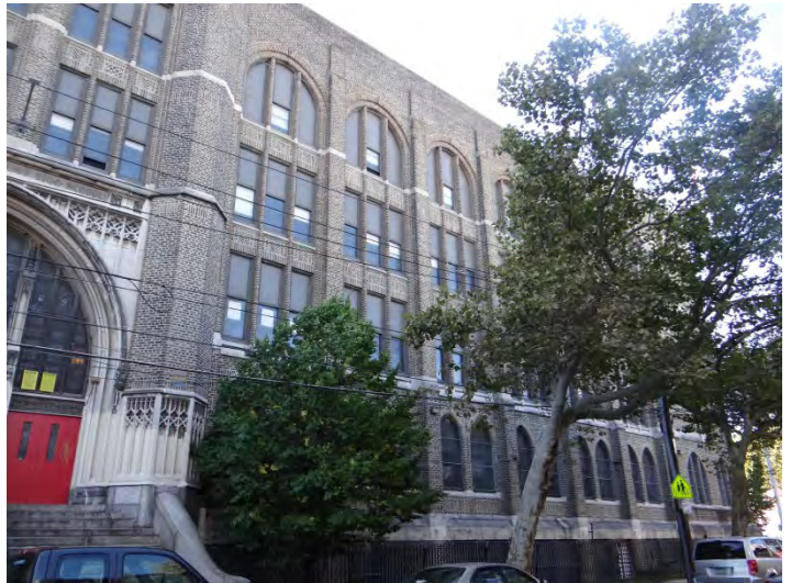
Photo 4: Looking SW at W end of main (N) façade
