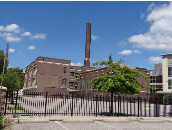
Photo 5: Looking N at rear (SE) façade
