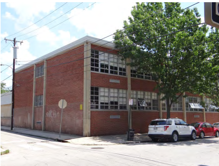
Photo 5: Looking SE at N (left) and W facades
