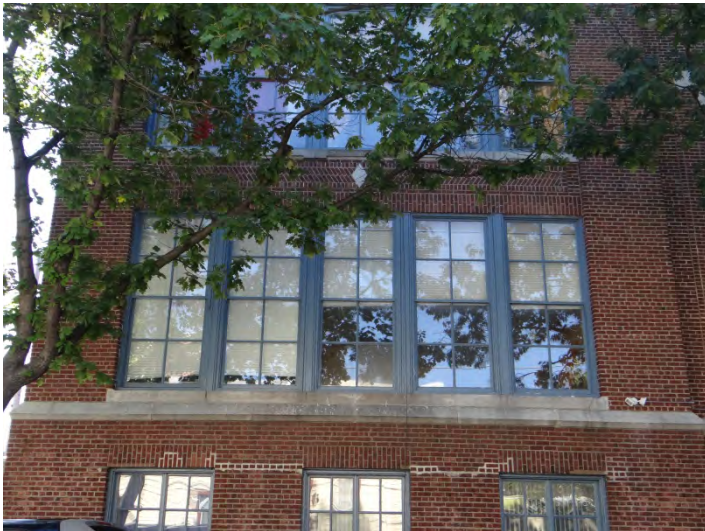
Photo 3: Looking S at E end of N facade
