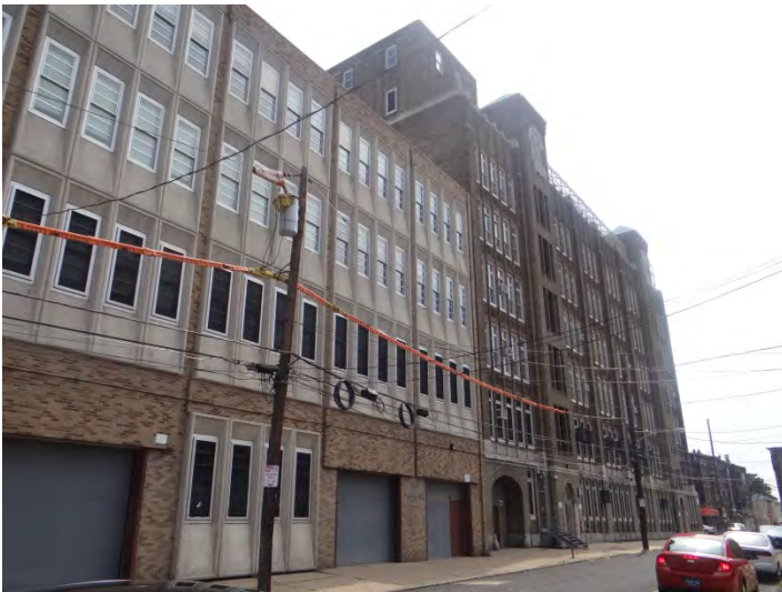
Photo 3: Looking E at center of SW facade
