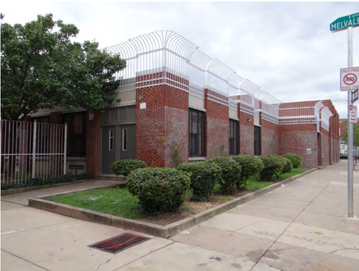
Photo 3: Looking NW at main (NE) façade
