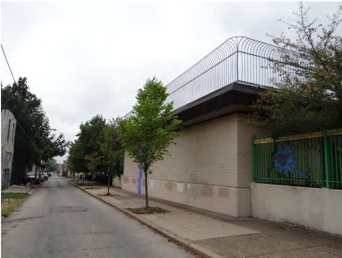
Photo 3: Looking SW at E facade
