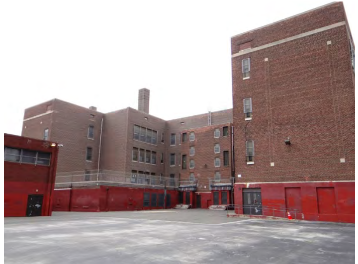
Photo 4: Looking NE at W facades
