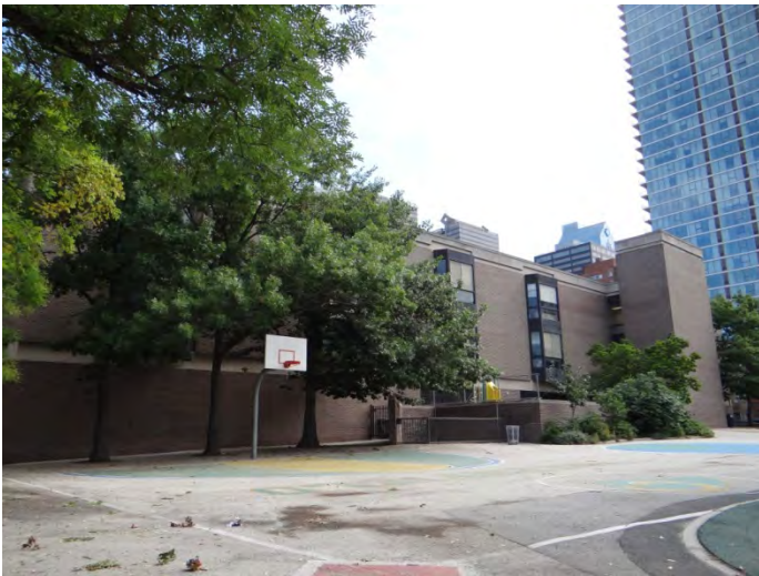
Photo 1: Looking NE at rear (S) facade
