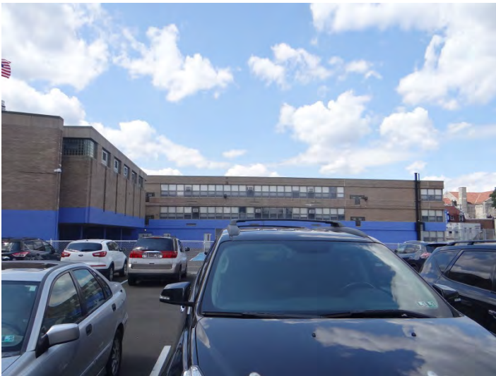
Photo 3: Looking NW at SE facade
