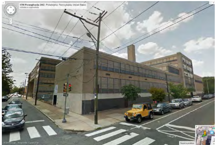
Photo 4: Looking SW at N (right) and E (left) facades. Source: Google Earth, August 2014
