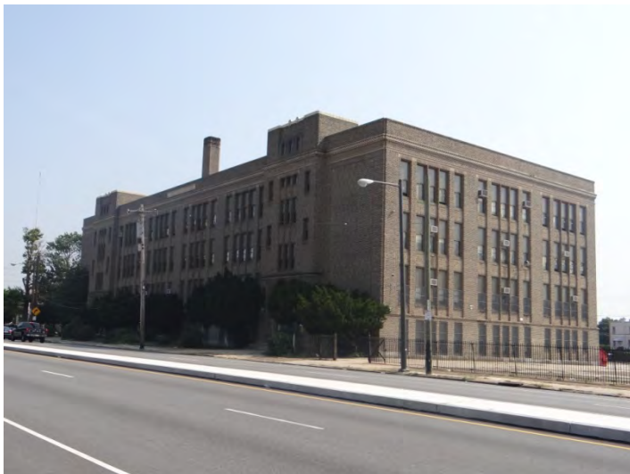
Photo 3: Looking NE at NW (left) and SW (right) facades
