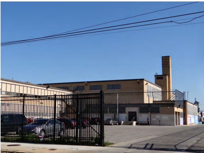
Photo 5: Looking NE at W corner of rear (S) facade
