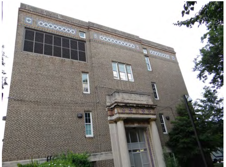
Photo 2: Looking N at S facade
