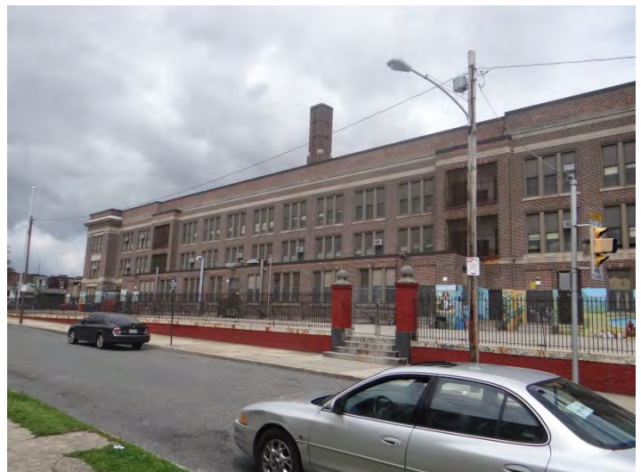
Photo 6: Looking NW at S facade
