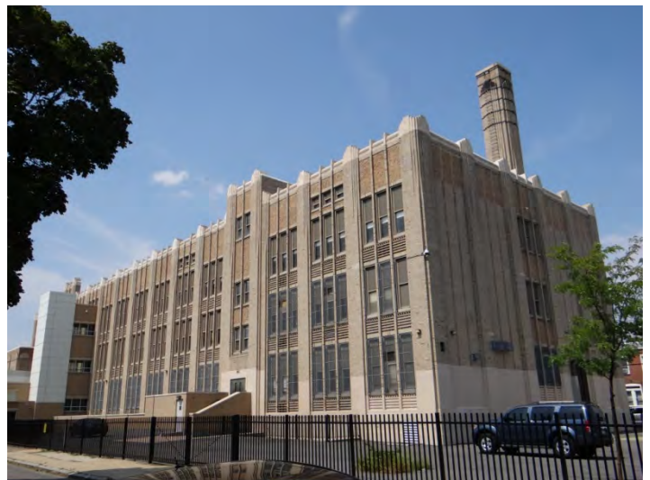
Photo 6: Looking NW at S facade
