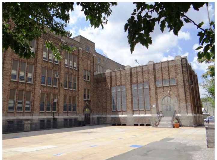
Photo 6: Looking SW at rear (N) facades
