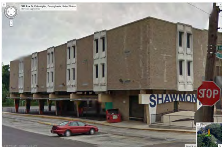
Photo 6: Looking NW at SE façade of addition
