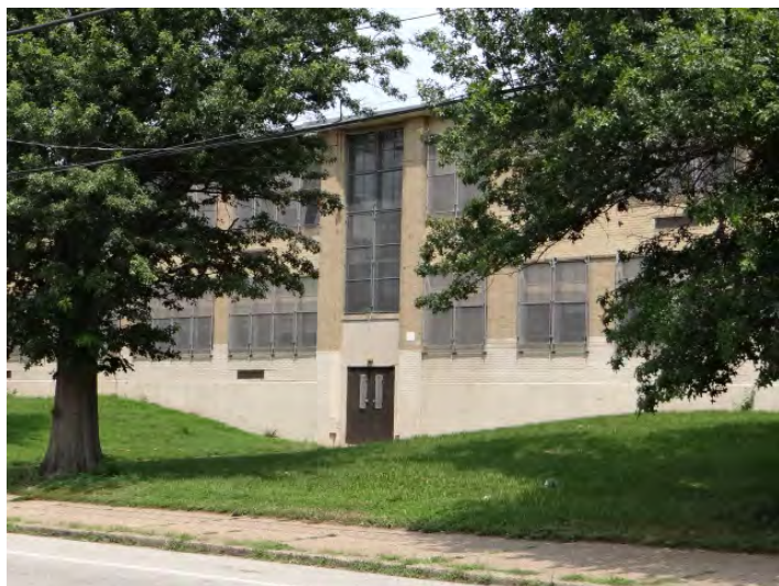
Photo 3: Looking N at center of SW façade
