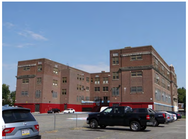
Photo 2: Looking NW at S facades
