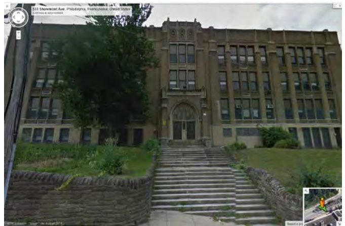
Photo 2: Looking SE at main (NW) facade
