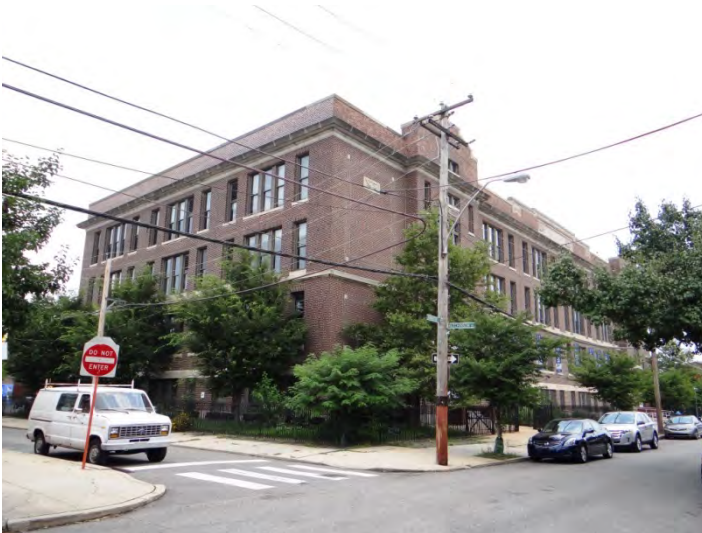
Photo 3: Looking NE at main (S, right) and W (left) facades
