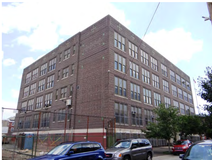
Photo 4: Looking NE at W (left) and main (S, right) facades
