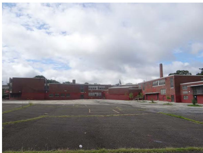
Photo 6: Looking SW at NE facades
