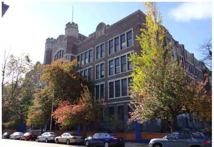
Photo 6: Looking SW at E facade
