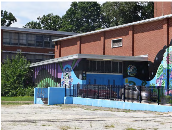
Photo 3: Looking W at main entrance of main (E) facade
