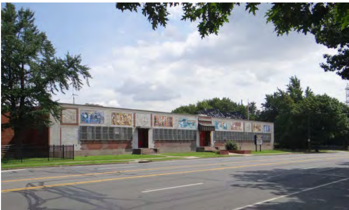
Photo 3: Looking SE at S end of main (W) facade
