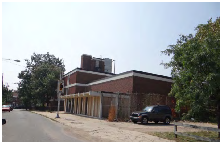
Photo 6: Looking S at NE (right) facade
