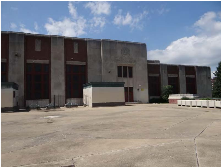
Photo 3: Looking W at N end of E façade
