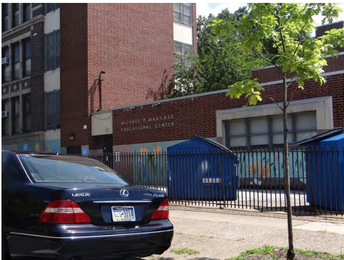
Photo 5: Looking NE at W façade
