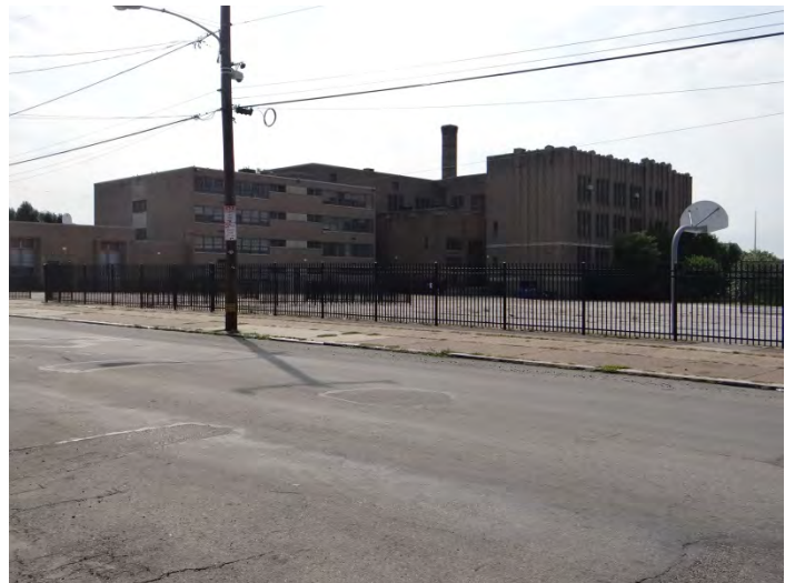
Photo 6: Looking SE at rear facades
