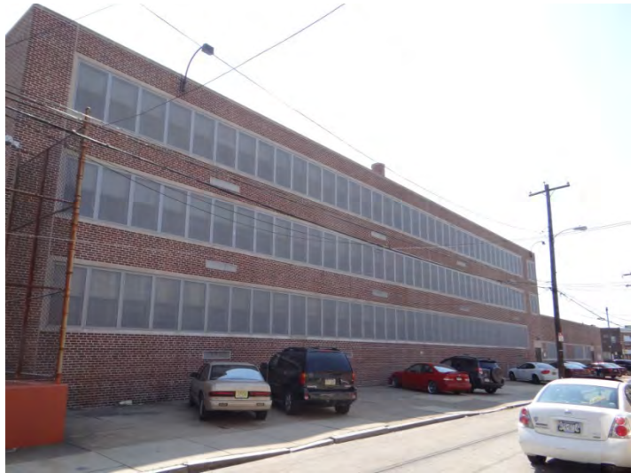
Photo 4: Looking SE at W facade
