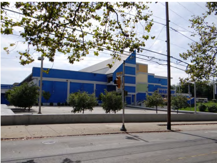
Photo 5: Looking SE at NW façade
