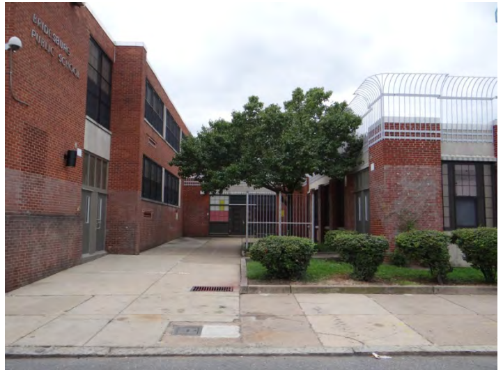
Photo 4: Looking SW at main (NE) façade at connection to 1966 addition
