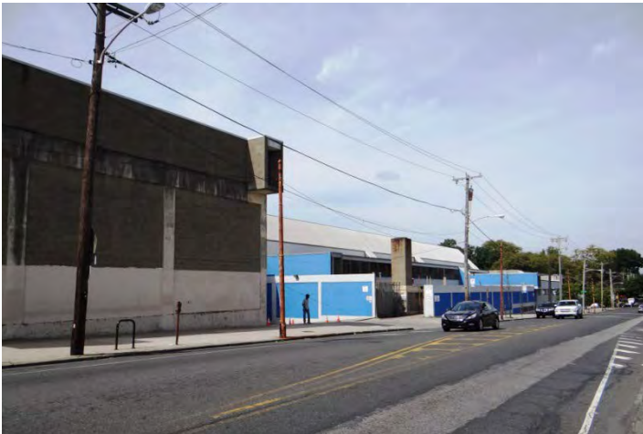
Photo 3: Looking E at W end of NE façade
