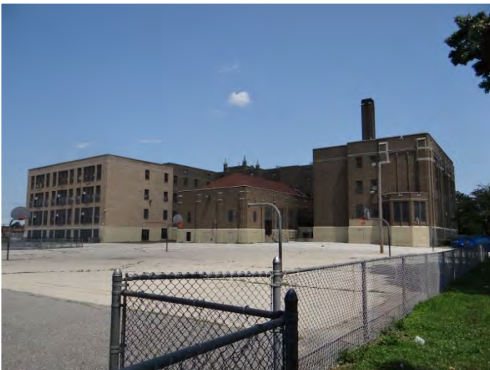
Photo 5: Looking N at rear (SW) facade
