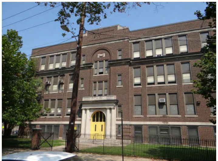
Photo 6: Looking N at SW façade
