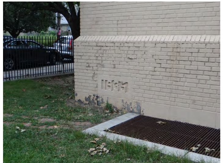
Photo 6: Datestone at SE corner of main (E) facade
