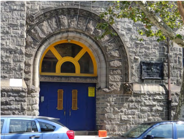
Photo 3: Looking E at W façade entrance
