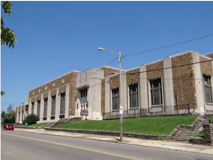
Photo 3: Looking NW at SW façade
