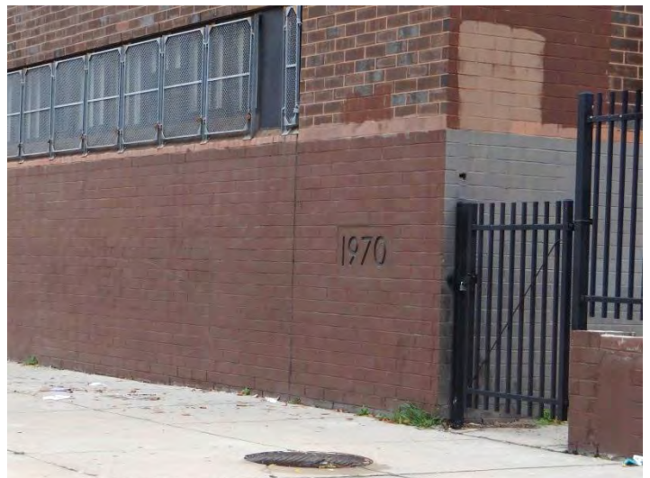
Photo 6: Datestone on main (SW) facade
