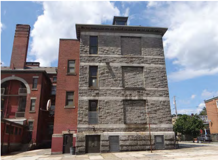
Photo 3: Looking NW at SE facade
