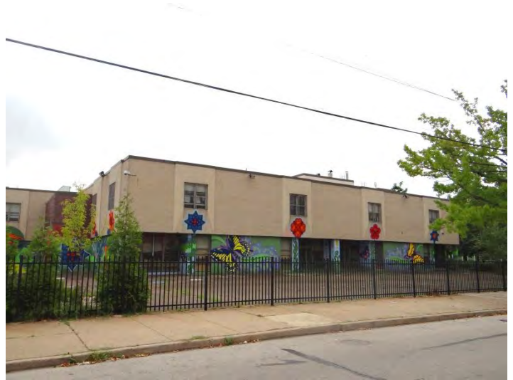
Photo 2: Looking SE at W façade
