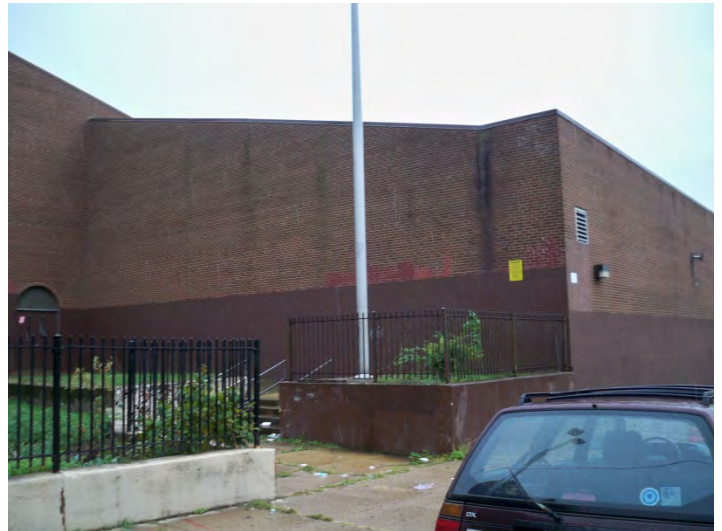
Photo 4: Looking SE at S end of W facade
