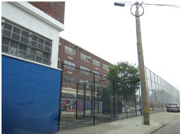
Photo 6: Looking SW at E end of N facade
