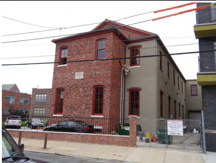
Photo 2: Looking W at N (right) and E (left) facades
