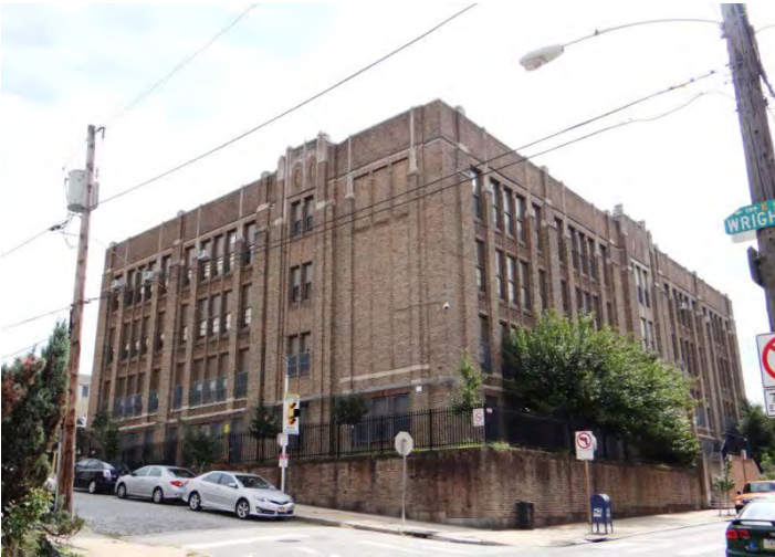
Photo 3: Looking E at NW (left) façade and main (SW) facade
