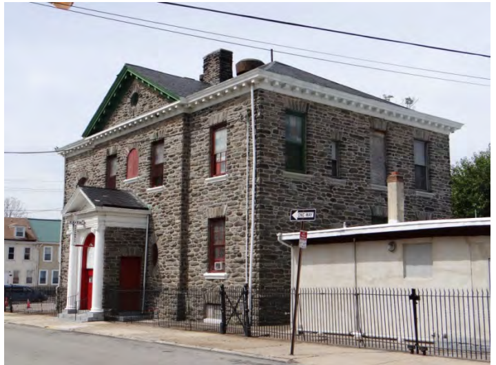
Photo 4: Looking SW at SE (left) and NE facades
