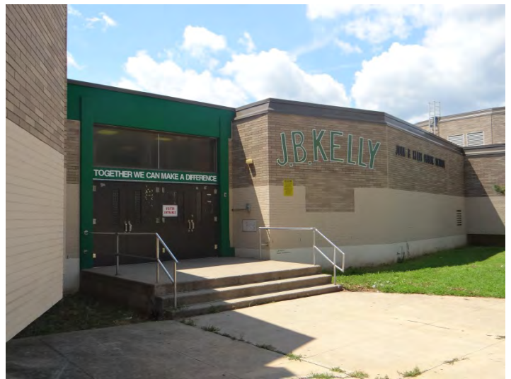
Photo 2: Main entrance, NE facade
