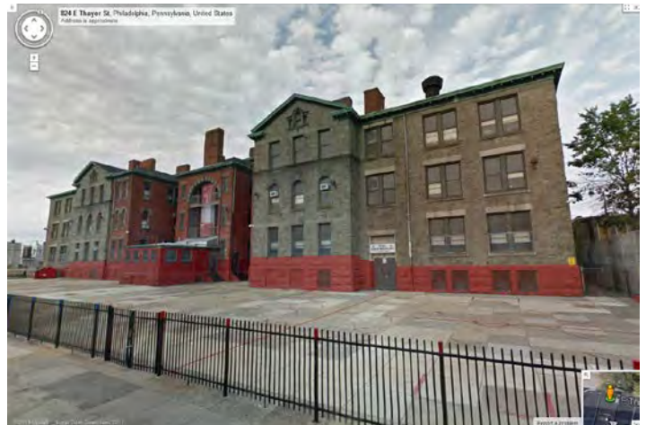
Photo 6: Looking NW at rear (S) façade. Source: Google Earth, September 2011
