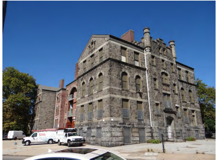
Photo 4: Looking NW at S (left) and E facades
