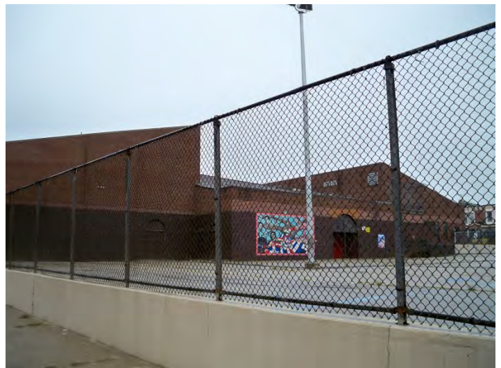
Photo 6: Looking NE at S facade
