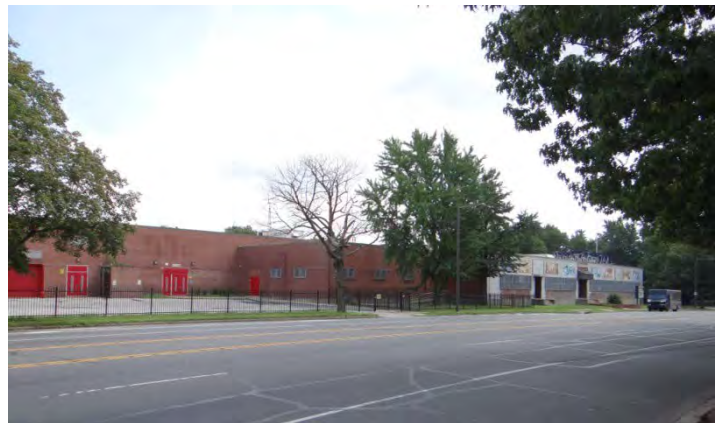
Photo 4: Looking SE at center of main (W) facades
