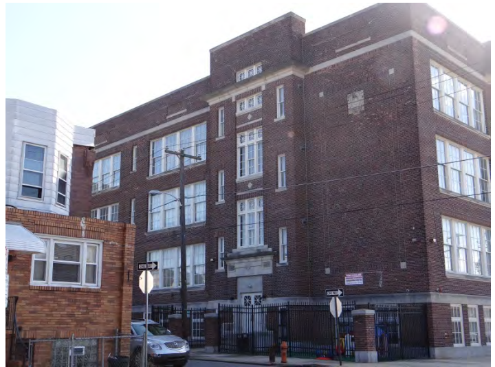
Photo 2: Looking SE at N facade
