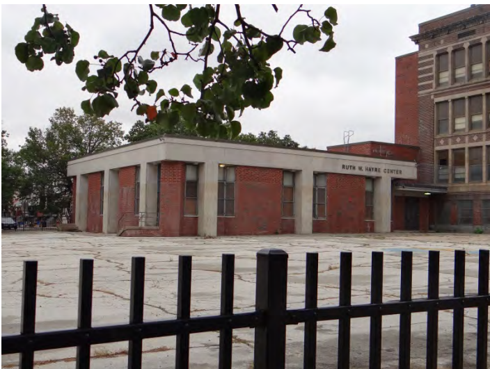
Photo 5: Looking SW at E façade of addition
