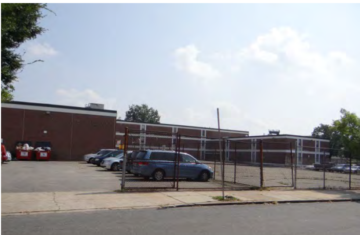
Photo 5: Looking SE at rear (NW) façade
