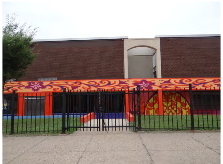
Photo 4: Looking N at S facade
