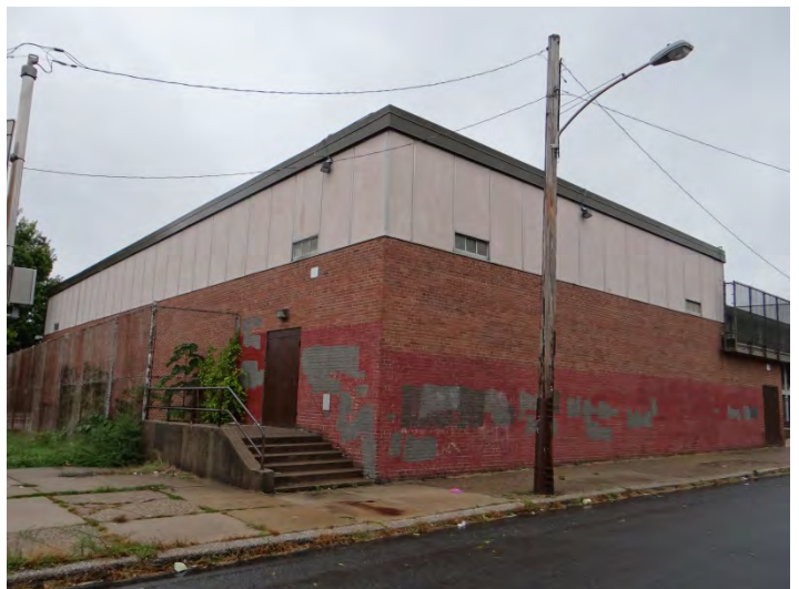
Photo 6: Looking NE at SW corner of school
