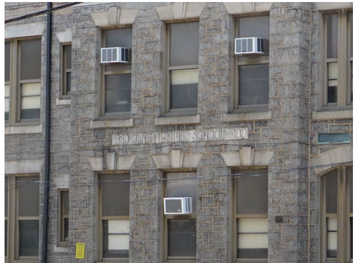
Photo 2: Looking S at main (N) façade
