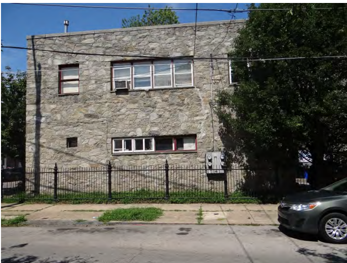
Photo 5: Looking NW at SE façade
