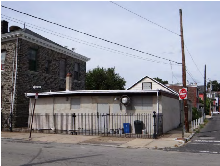
Photo 3: Looking N at NE facade
