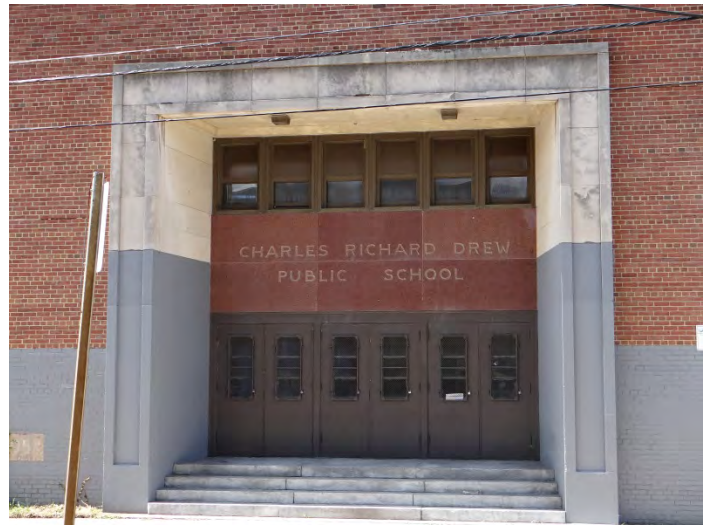
Photo 2: Detail, main (NE) façade
