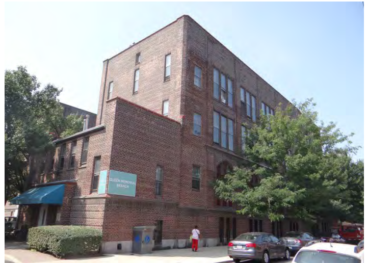
Photo 4: Looking SW at E (left) and N facades
