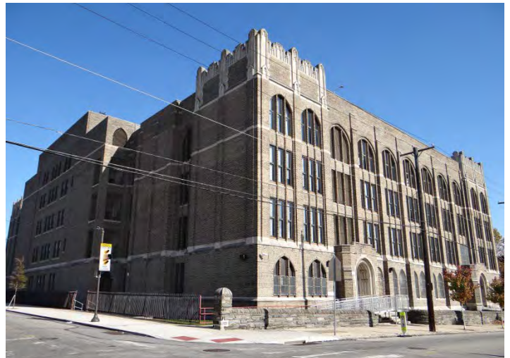
Photo 6: Looking NE at rear (W, left) and S (right) facades
