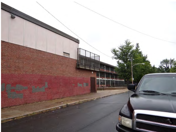
Photo 5: Looking NE at S facade
