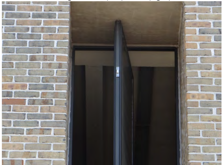
Photo 6: Detail, window opening
