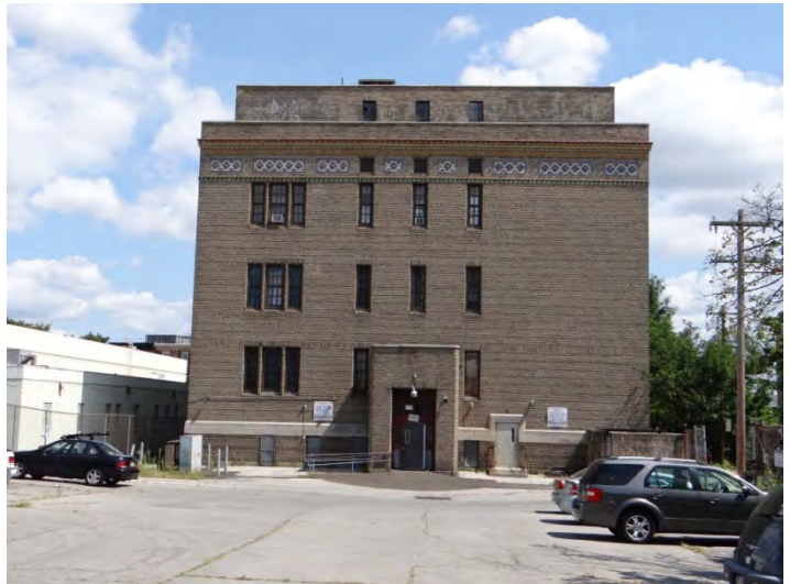
Photo 4: Looking E at rear (W) facade
