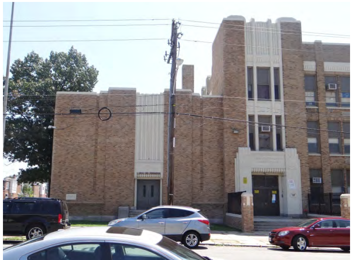
Photo 2: Looking SE at NE end of NW facade
