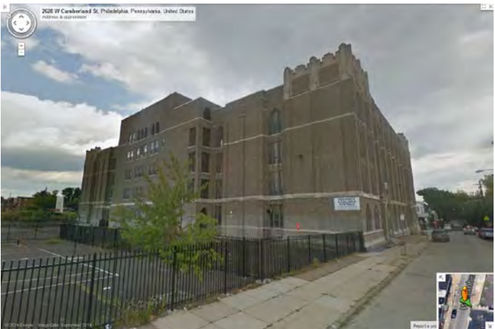
Photo 5: Looking SE at rear (N, left) and W facades
