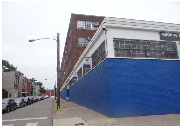
Photo 2: Looking NW at main (S, left) and E (right) facades
