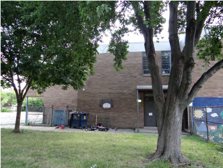
Photo 3: Looking E at NW facade
