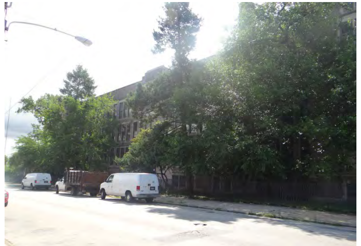
Photo 2: Looking SE at N façade
