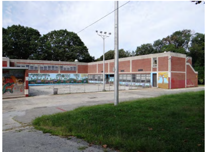
Photo 4: Looking W at N end of NE facade
