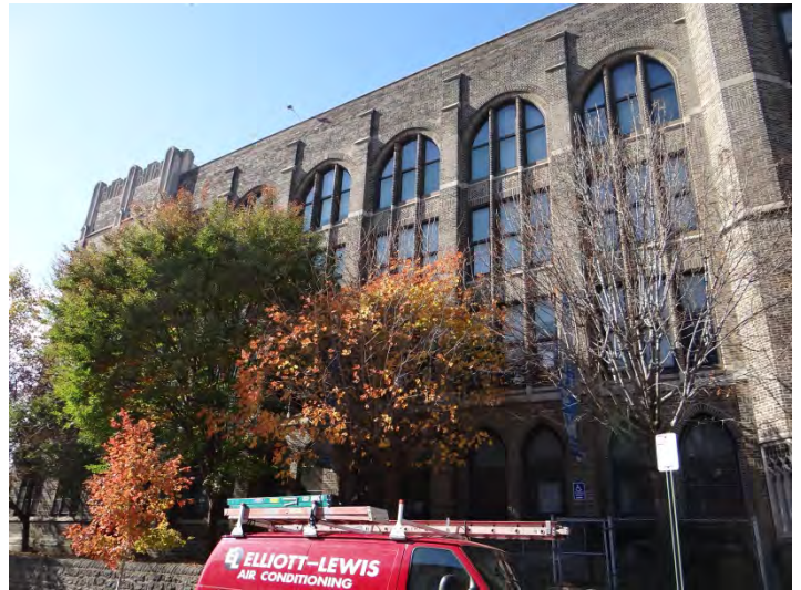
Photo 4: Looking SW at S end of main (E) facade
