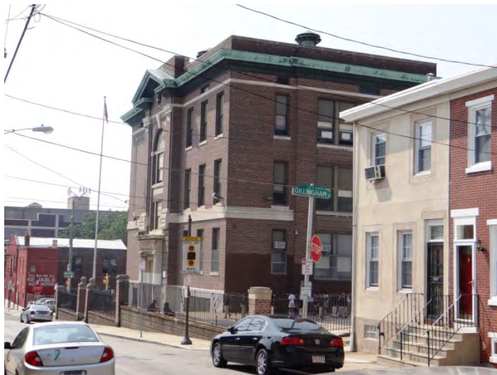
Photo 2: Looking SW at SE (left) and NE (right) facades
