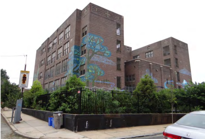
Photo 5: Looking NW at rear (E) facade
