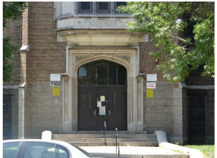
Photo 4: Looking SW at main entrance on main (NE) facade
