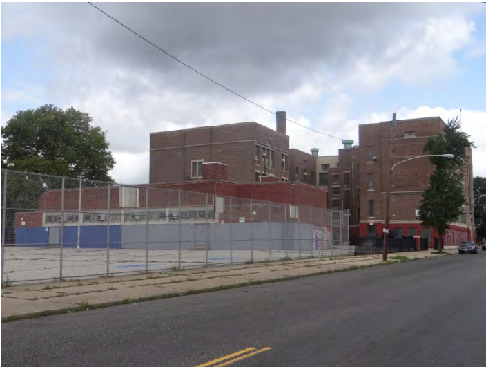
Photo 3: Looking NW at S façade
