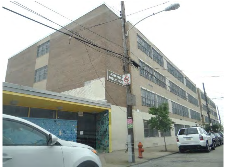
Photo 2: Looking SE at entrance on main (W) façade
