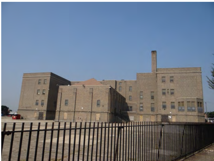
Photo 5: Looking NW at SE façade
