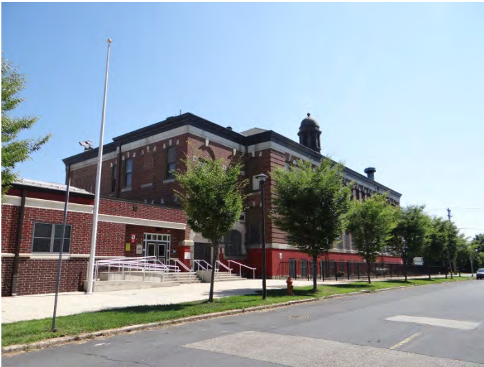
Photo 3: Looking NE at main (SW) façade
