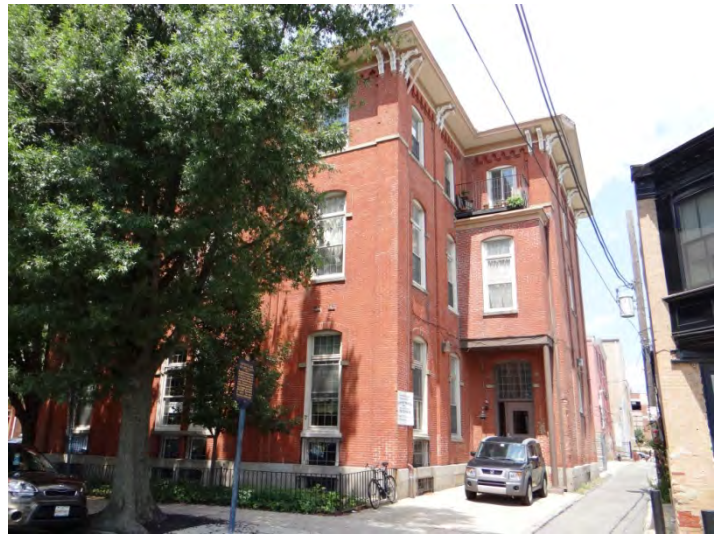
Photo 2: Looking N at E facade
