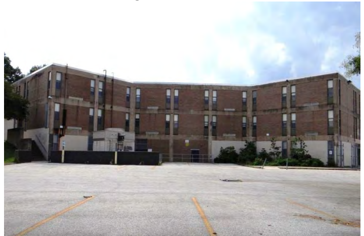
Photo 6: Looking W at E facade
