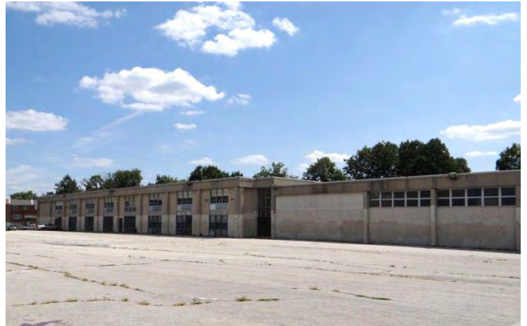
Photo 4: Looking NE at rear (NW) facade
