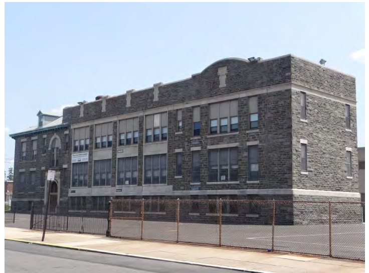
Photo 2: Looking NE at NW facade
