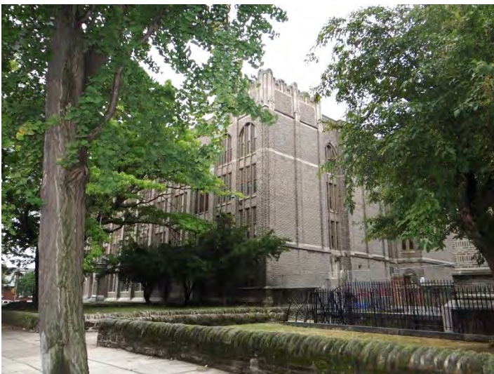
Photo 5: Looking W at N façade
