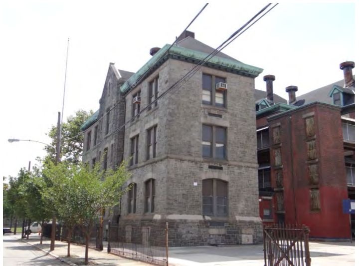
Photo 6: Looking S at E (left) and N facades
