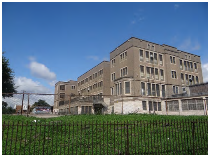
Photo 6: Looking NW at E (right) and S (left) facades
