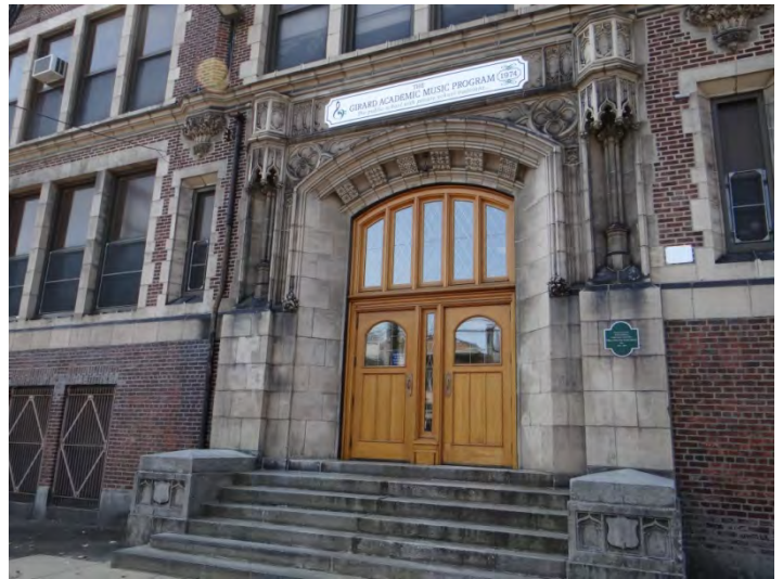
Photo 2: Detail, main entrance on main (N) facade
