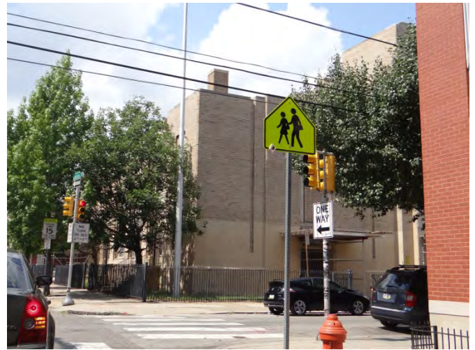
Photo 2: Looking NW at main (E) façade auditorium entrance
