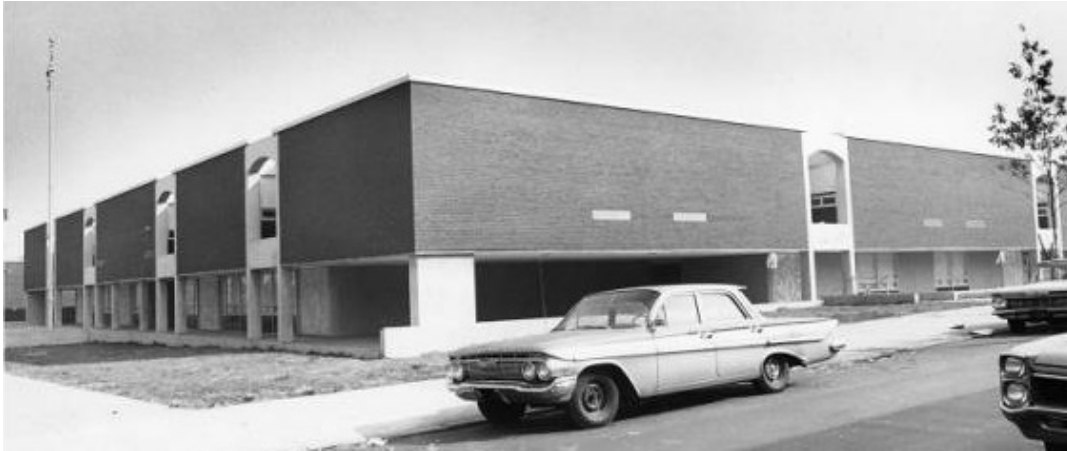
Potter-Thomas Elementary (1969), in North Philadelphia, is an example of the way urban crisis-era concern for security was reflected in inward facing school design.
