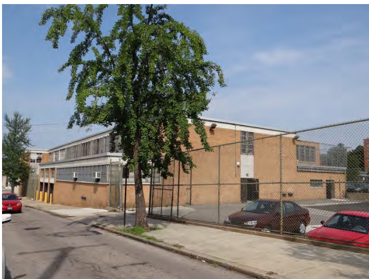
Photo 5: Looking NW at main (S, left) and E facades
