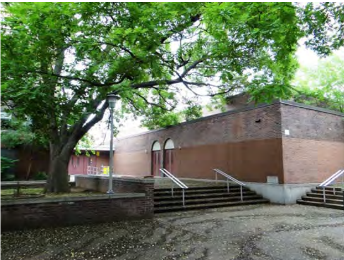
Photo 5: Looking NW at E side of addition
