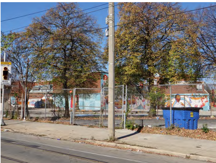
Photo 5: Looking NW at E facade
