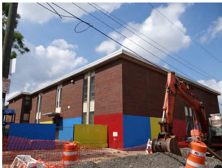
Photo 6: Looking NW at E (right) and main (S, left) facades
