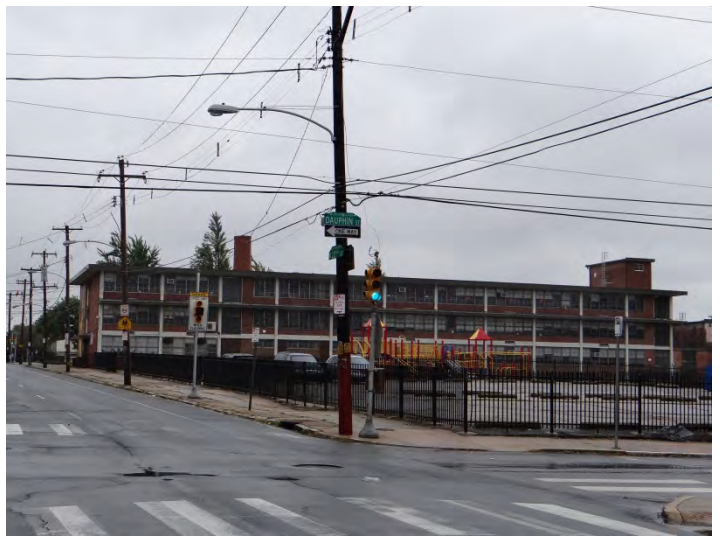
Photo 2: Looking S at N facade
