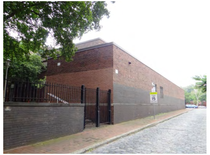
Photo 6: Looking N at E facade of addition
