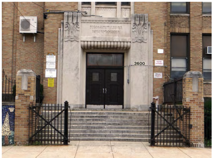
Photo 2: Looking W at entrance on main (NE) facade
