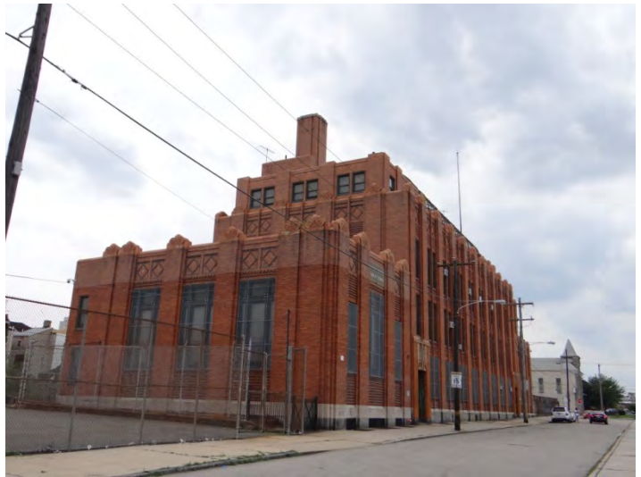
Photo 2: Looking SW at main (N, right) and E (left) facades
