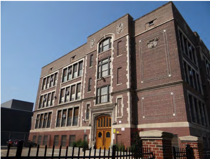
Photo 3: Looking W at E façade
