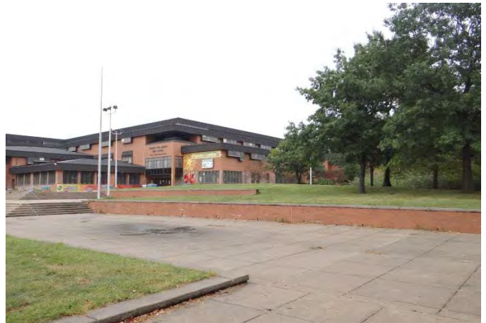
Photo 2: Looking NW at S (left) and E (right) facades
