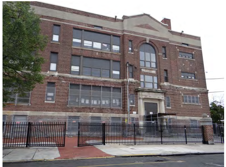
Photo 2: Looking W at N facade
