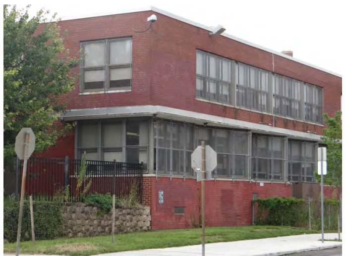
Photo 6: Looking S at E corner of the NE facade
