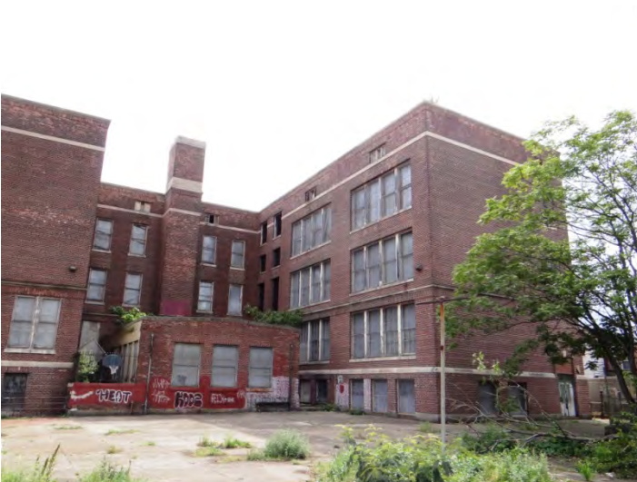
Photo 5: Looking SW at rear (N) façade
