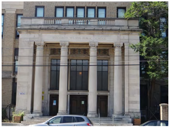
Photo 2: Looking SW at main entrance, main (NE) facade
