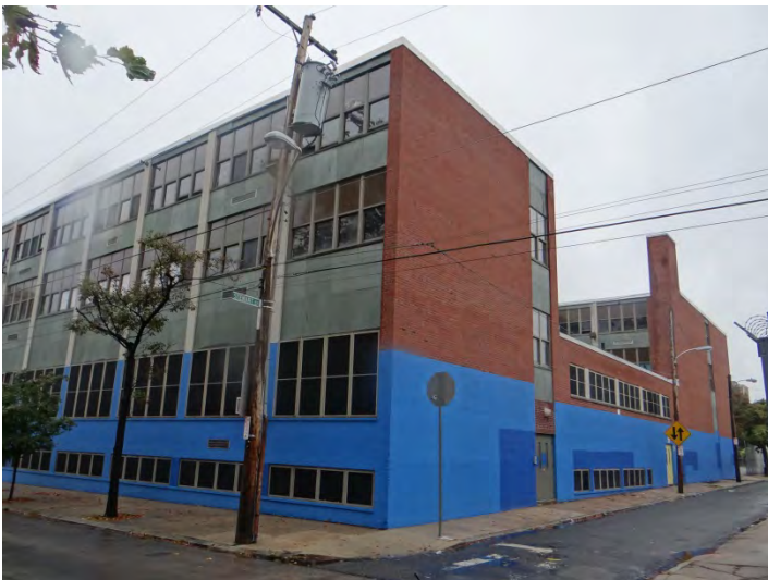
Photo 5: Looking NE at W (left) and rear (S, right) facades
