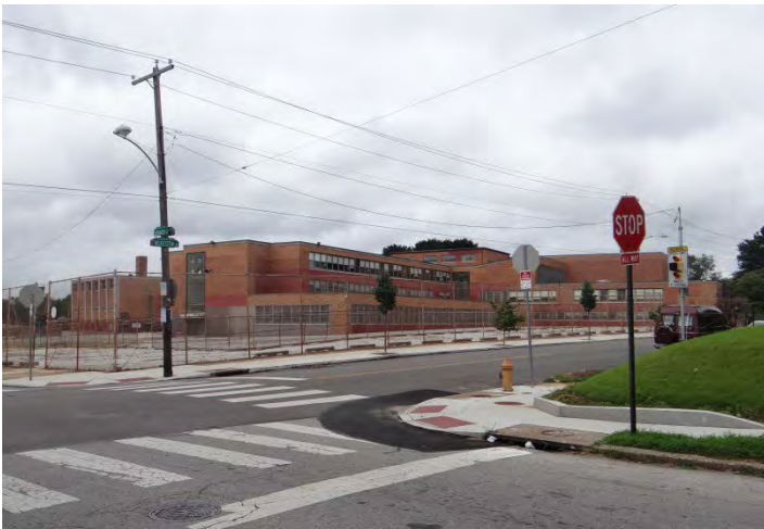
Photo 5: Looking W at E façade
