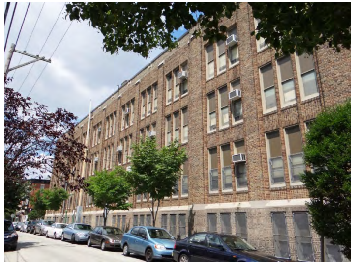
Photo 2: Looking NW at S facade
