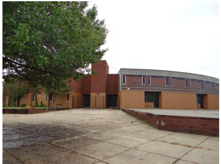
Photo 2: Looking SE at NW corner entrance
