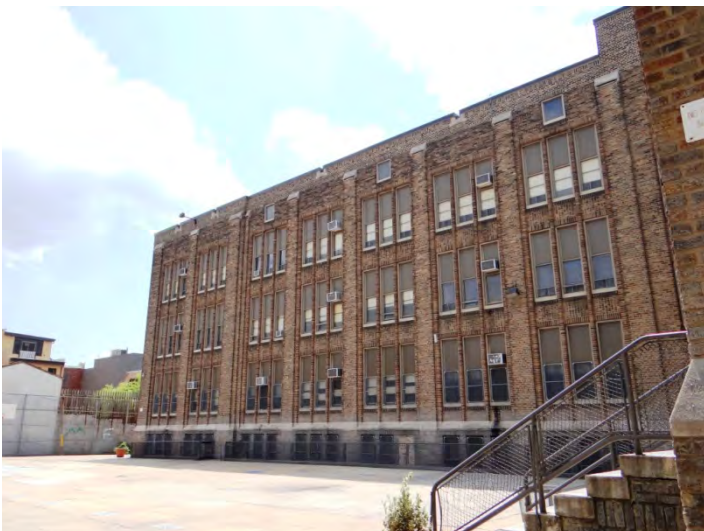
Photo 5: Looking S at N façade
