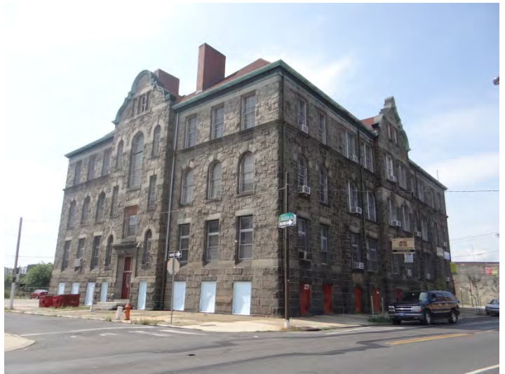
Photo 2: Looking SW at NE (left) and NW (right) facades
