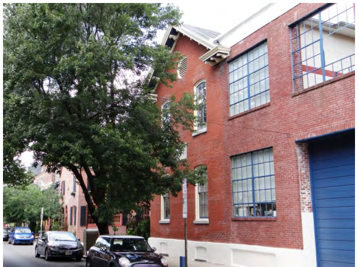
Photo 2: Looking NW at S facade
