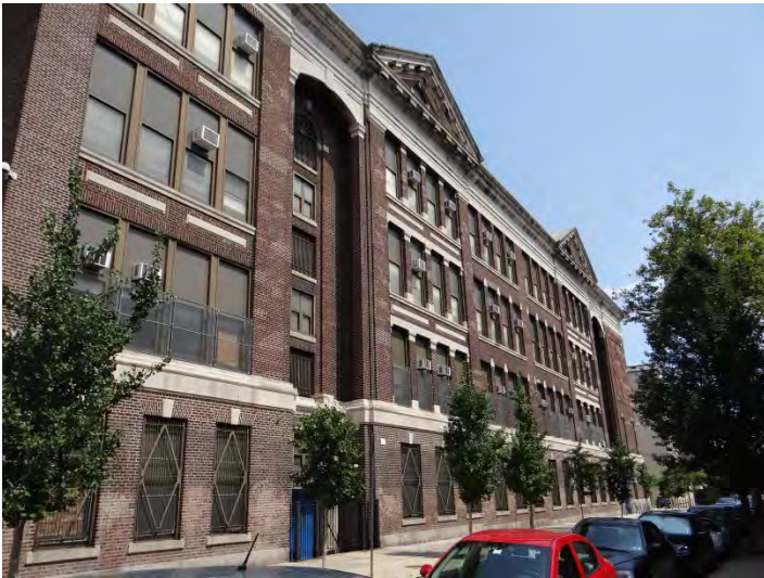
Photo 3: Looking NE at S facade
