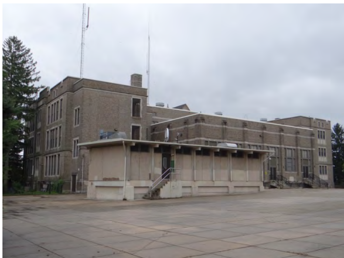
Photo 5: Looking E at N end of rear (NW) facade
