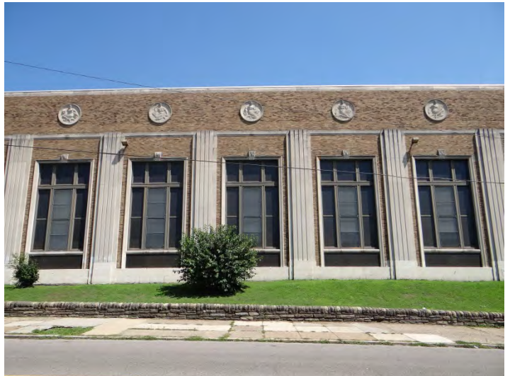
Photo 4: Looking NE at center of SW facade
