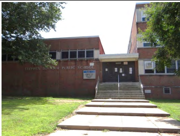
Photo 2: Looking SW at main (NE) facade
