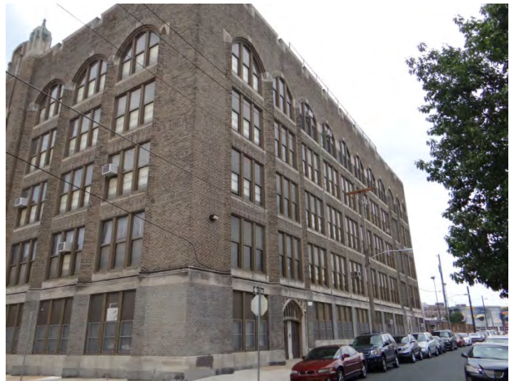
Photo 4: Looking SW at N façade
