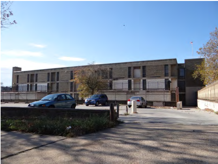
Photo 3: Looking W at E façade
