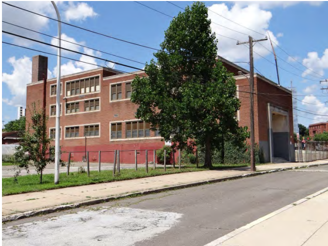
Photo 3: Looking W at SE façade
