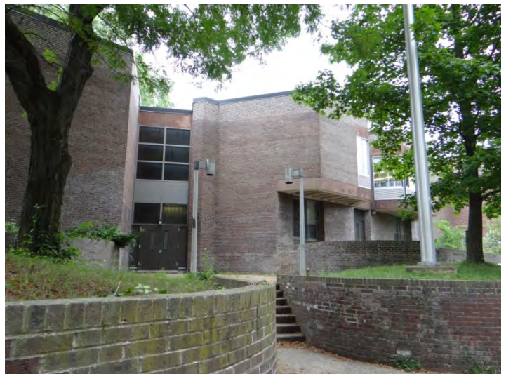
Photo 6: Looking NW at SE façade of ca. 1966 addition
