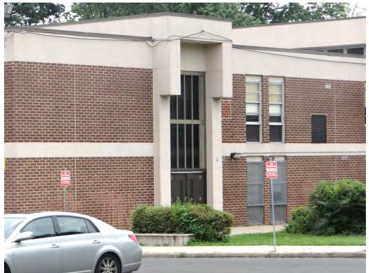
Photo 4: Looking E at entrance in NE wing
