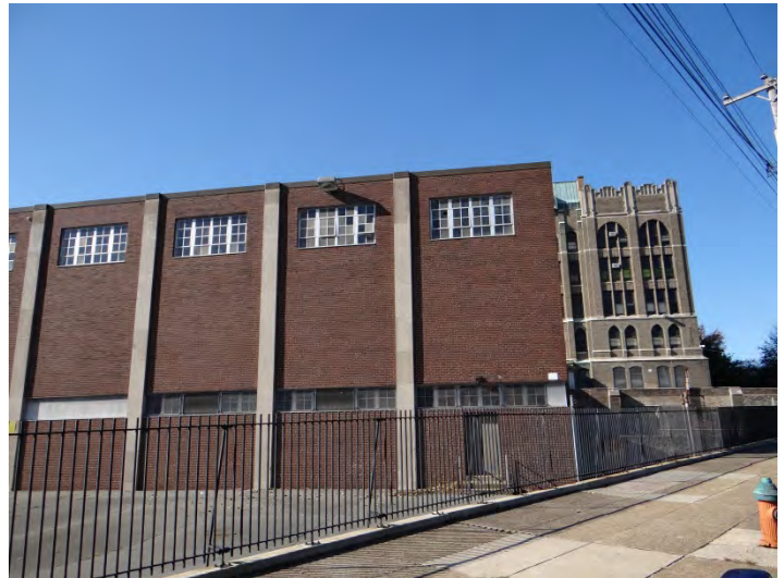
Photo 4: Looking SW at E façade of addition
