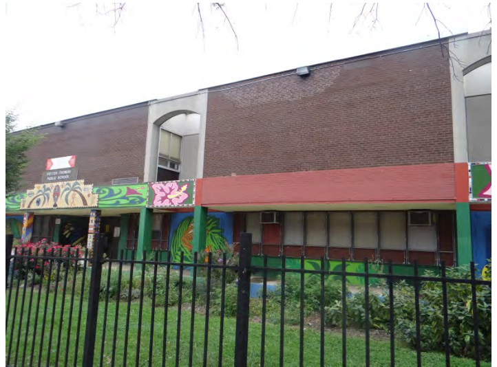
Photo 2: Looking NE at S end of main (W) facade
