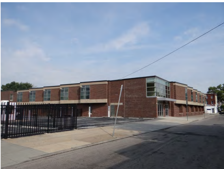
Photo 5: Looking NW at S façade
