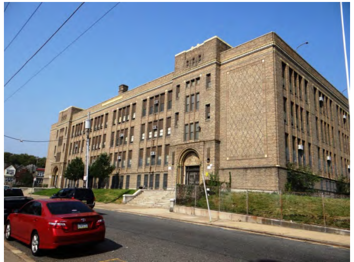
Photo 2: Looking NW at main (SE) facade
