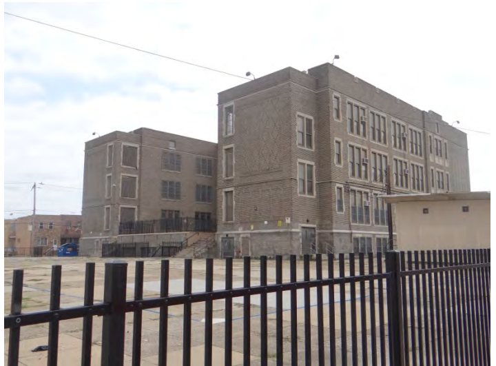
Photo 4: Looking SE at rear (NW, left) and SW (right) facades
