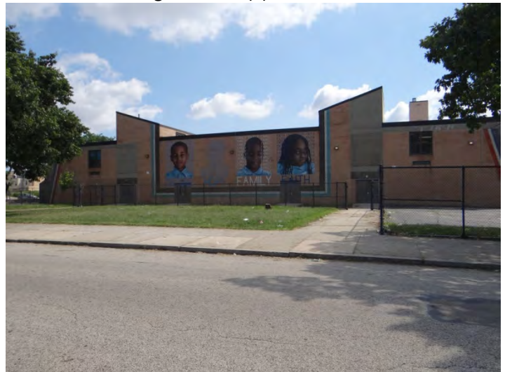
Photo 6: Looking E at W facade
