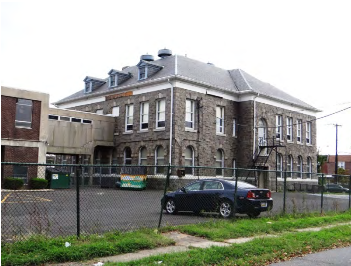
Photo 3: Looking S at NW façade
