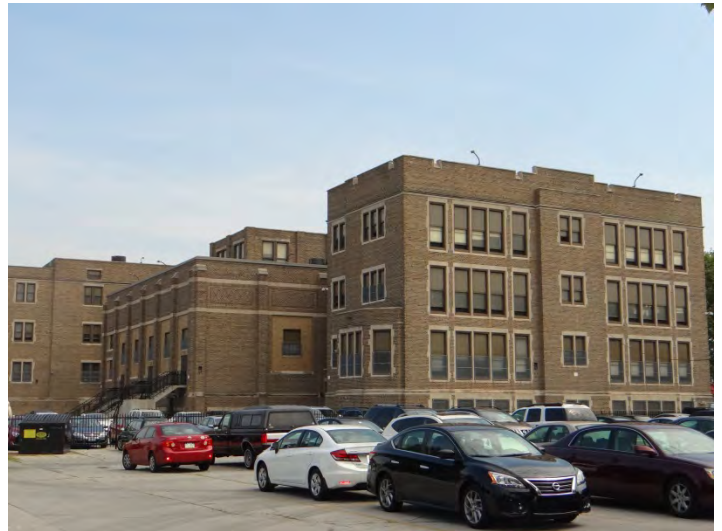
Photo 4: Looking NE at W facade
