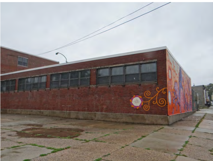
Photo 5: Looking SE at W end of main (N) façade
