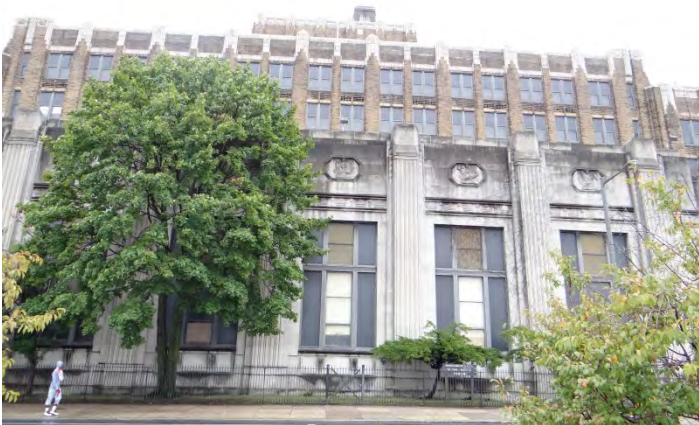
Photo 3: Looking S at center bays of main (N) façade
