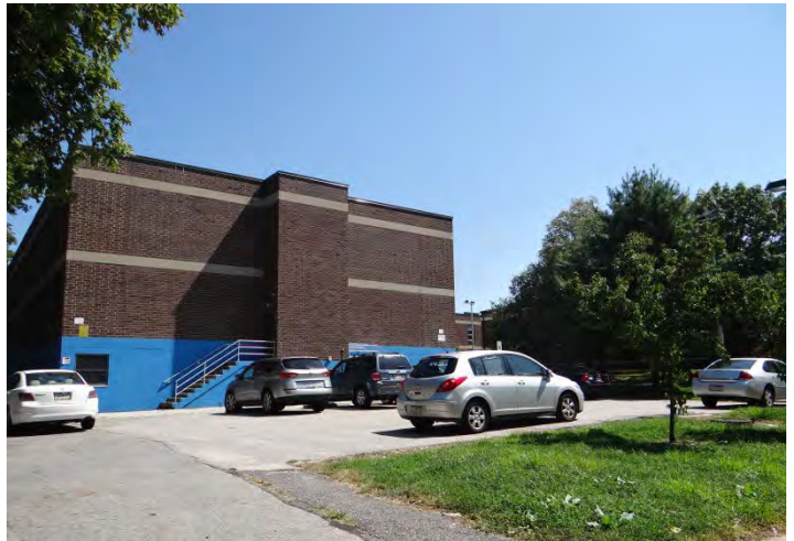
Photo 4: Looking N at SW facade
