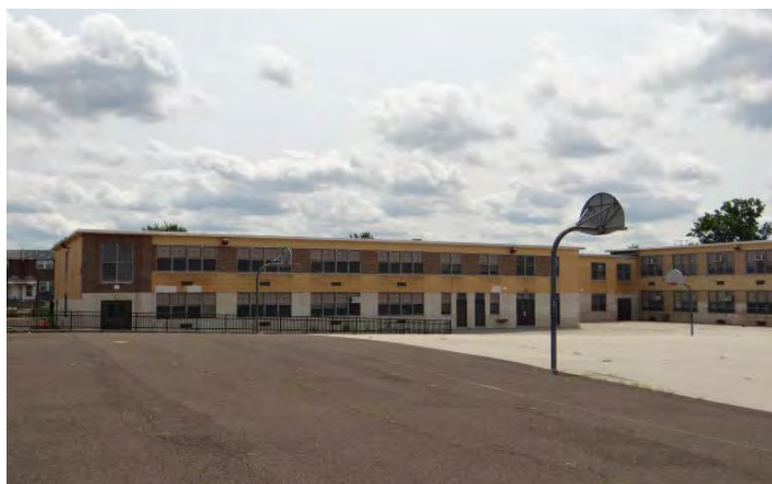
Photo 5: Looking SE at NE facades
