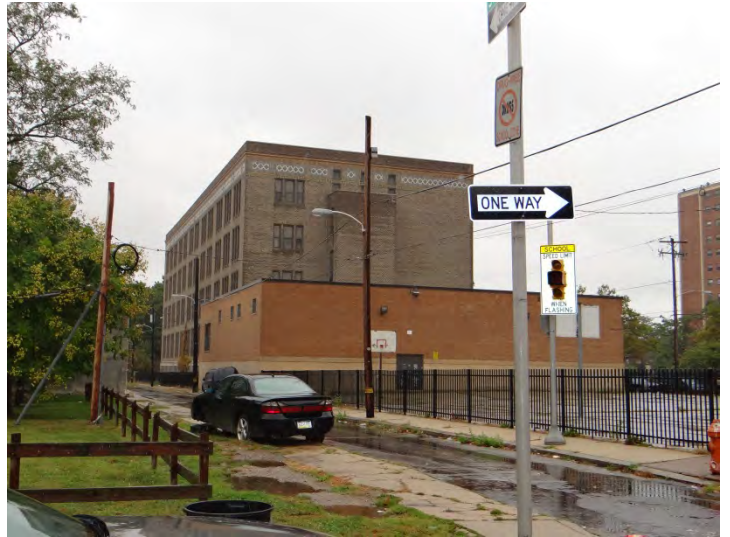
Photo 4: Looking NW at S (left) and rear (E, center) facades
