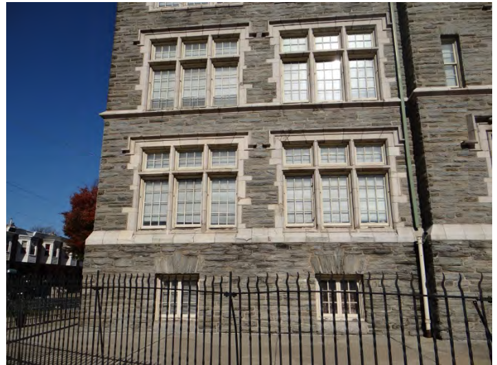
Photo 4: Looking N at window bays at W side of S facade
