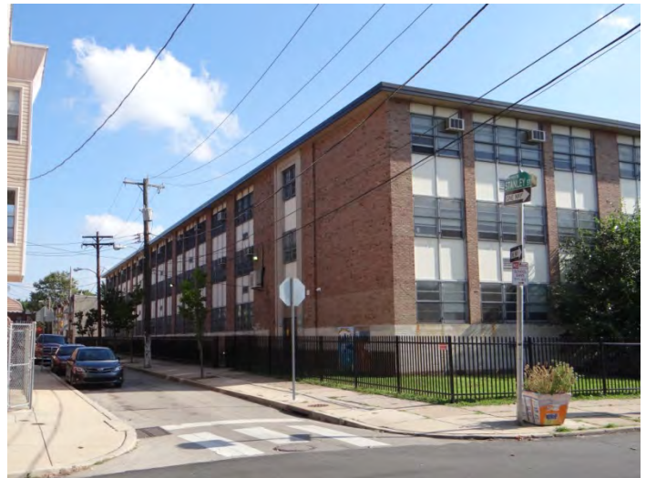
Photo 4: Looking N at W façade
