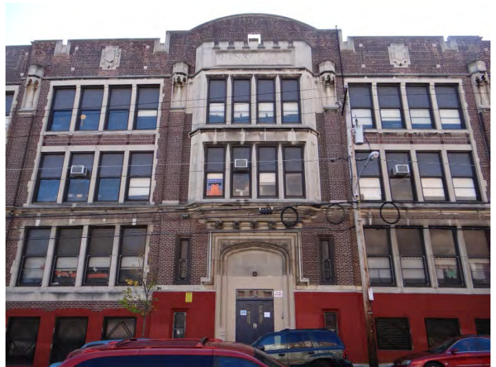
Photo 2: Looking S at main (N) facade
