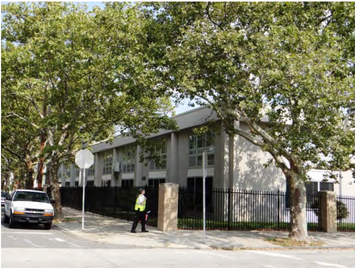
Photo 3: Looking E at NW facade
