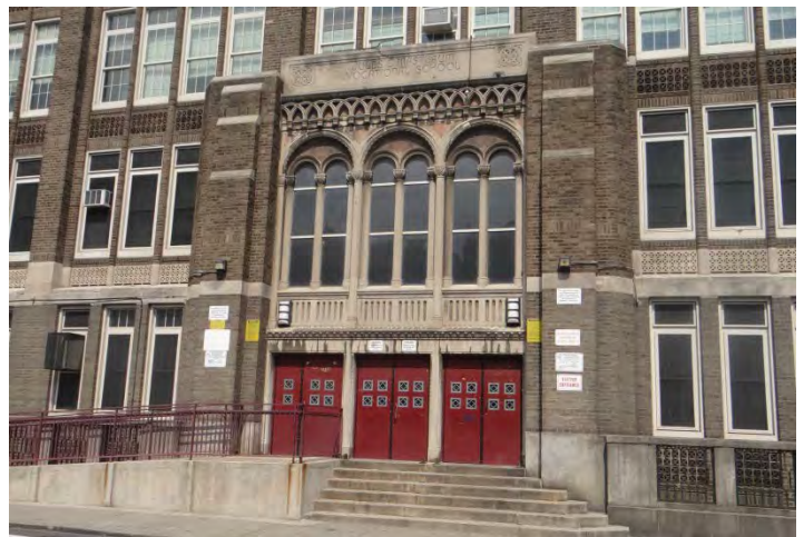
Photo 2: Looking N at main entrance on main (SE) facade
