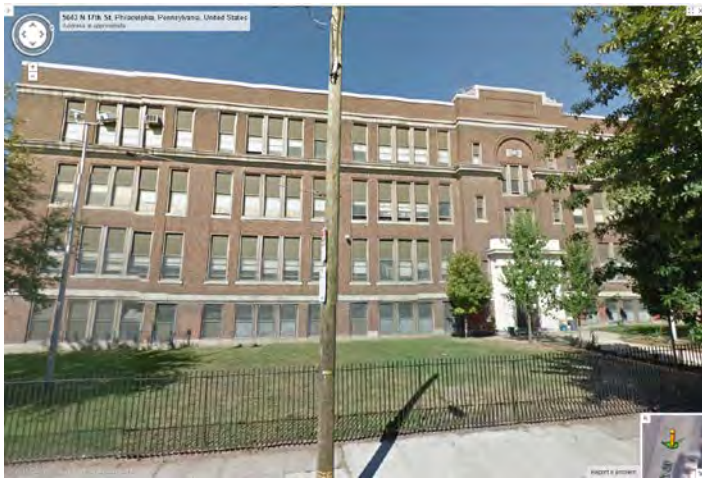
Photo 3: Looking SW at E façade
