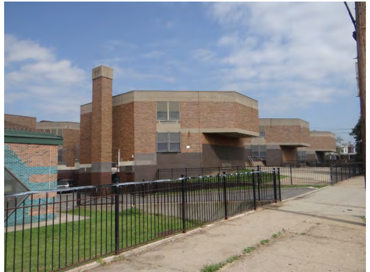
Photo 4: Looking N at E facade
