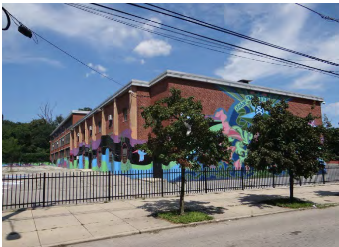
Photo 5: Looking NW at SW façade
