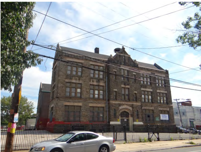
Photo 5: Looking SE at NW façade
