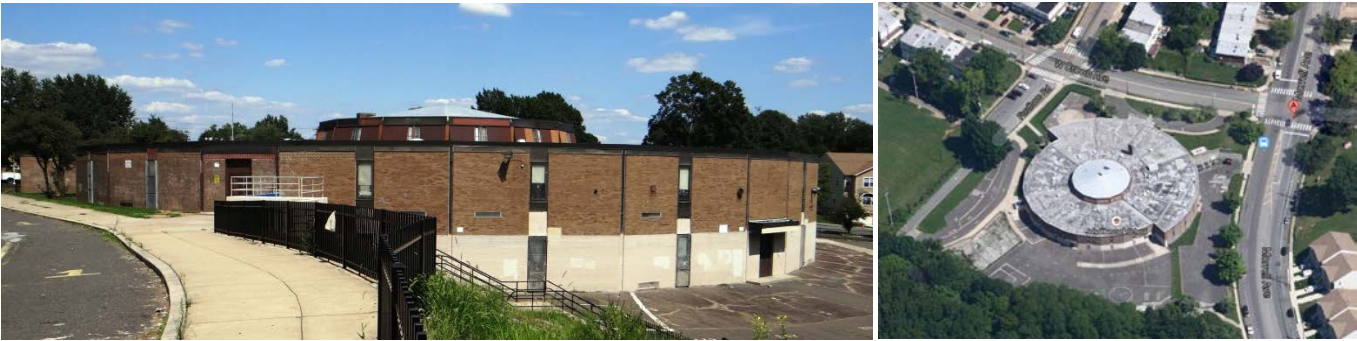
John Hancock Elementary, Northeast Philadelphia (1967, Sabatino & Fishman) current views here, and historic image above on the prior page. Photo directly above, 2013 PA SHPO; aerial view Google Earth 2014.
