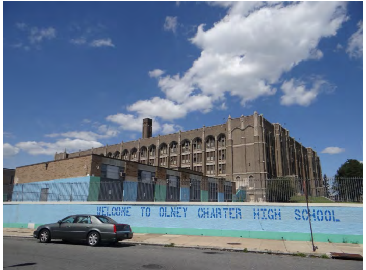
Photo 4: Looking NW at E façade
