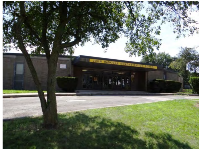
Photo 2: Looking SW at main entrance at N facade
