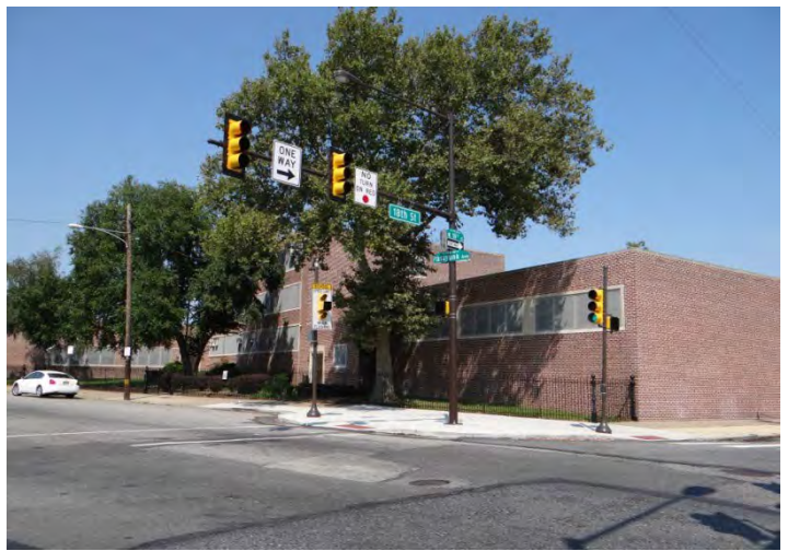
Photo 2: Looking NW at S facade
