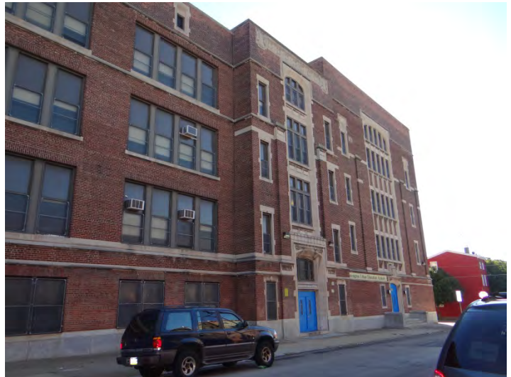
Photo 4: Looking SE at S corner of main (SW) façade
