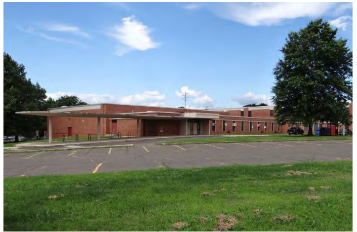
Photo 2: Looking W at E facade
