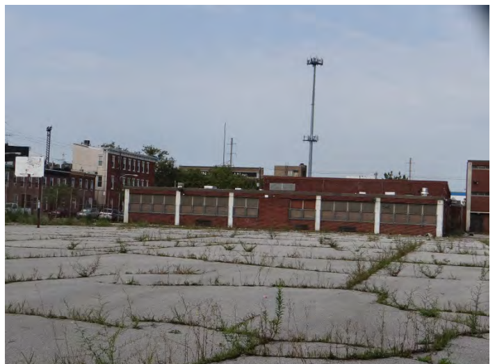
Photo 6: Looking W at E facade
