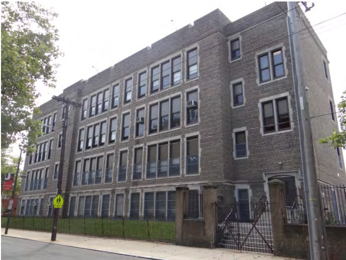
Photo 3: Looking E at N façade
