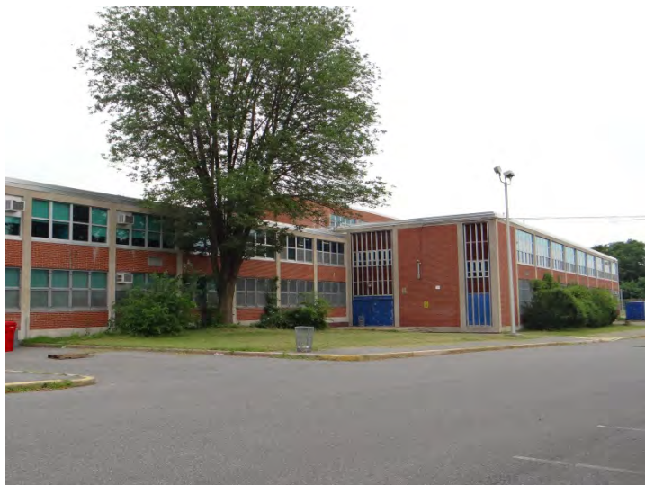
Photo 3: Looking NE at S facade
