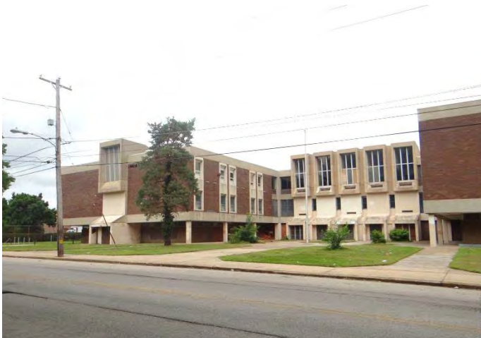
Photo 5: Looking NW at main (SW) façade
