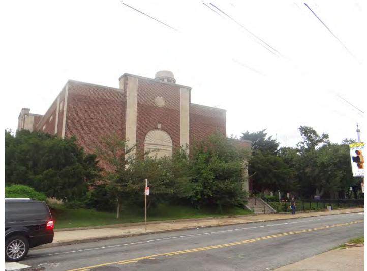
Photo 4: Looking N at W end of S facade
