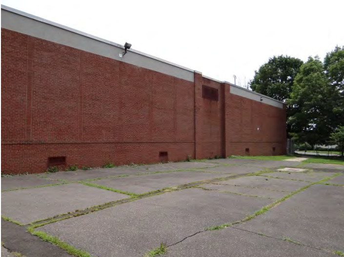
Photo 5: Looking E at W facade
