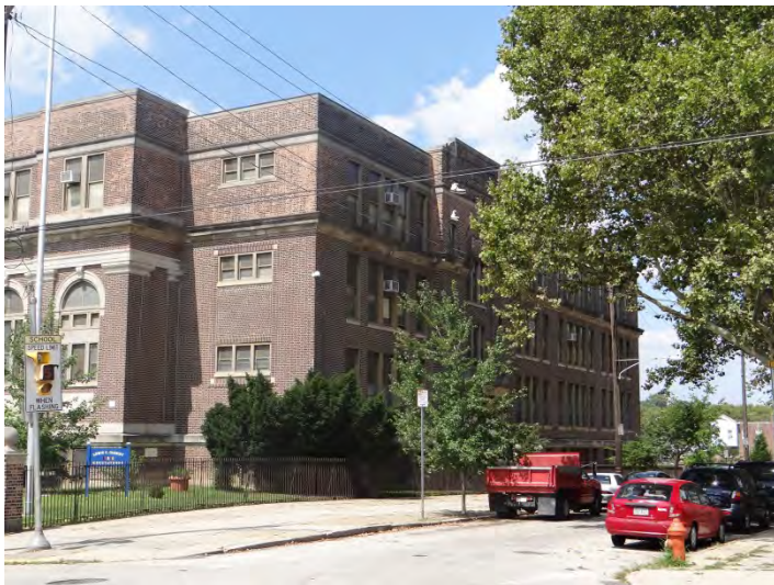
Photo 3: Looking N at E facade
