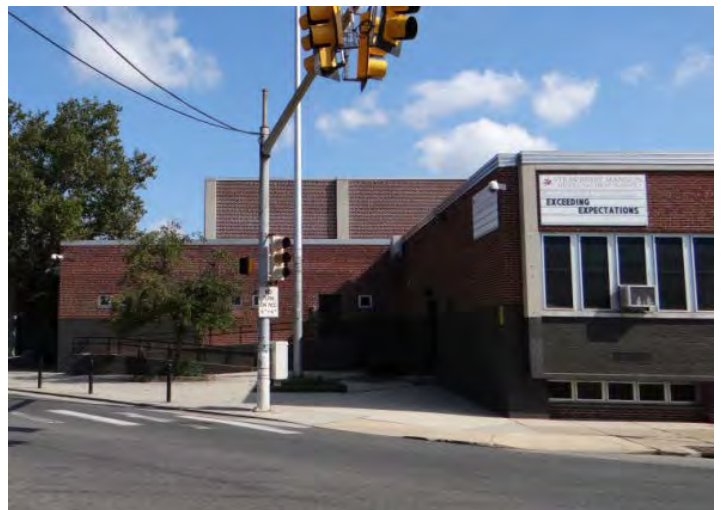
Photo 6: Looking N at W end of S facade
