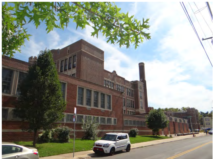
Photo 6: Looking S at NW facade
