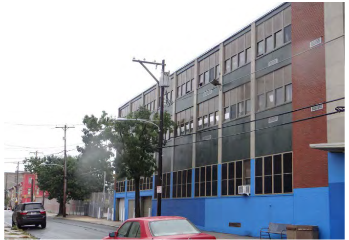
Photo 2: Looking E at E end of main (N) façade
