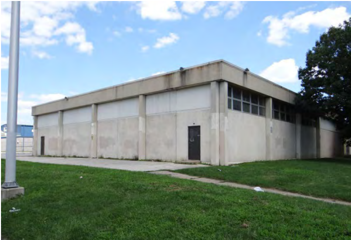
Photo 3: Looking N at SW (left) and SE (right) facades
