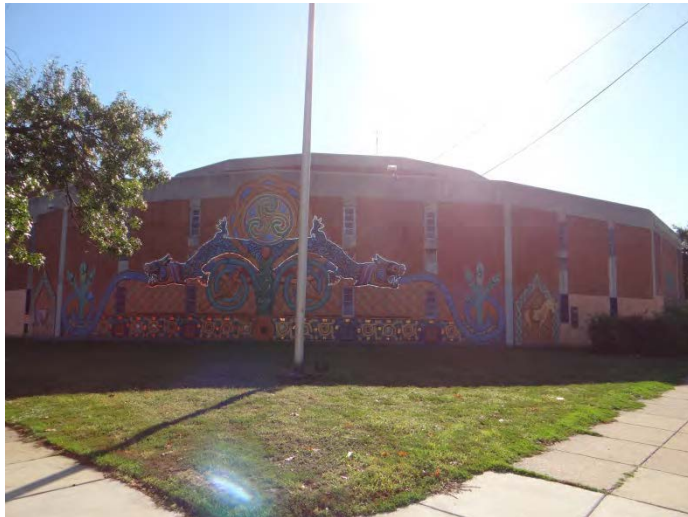
Photo 3: Looking E at NW facade
