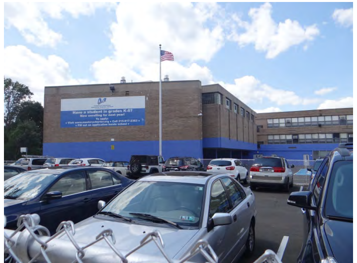
Photo 4: Looking W at NE (right) and SE (left) facades of rear wing
