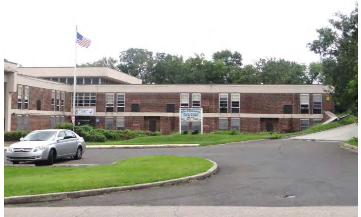
Photo 2: Looking SW at N façade of NW wing
