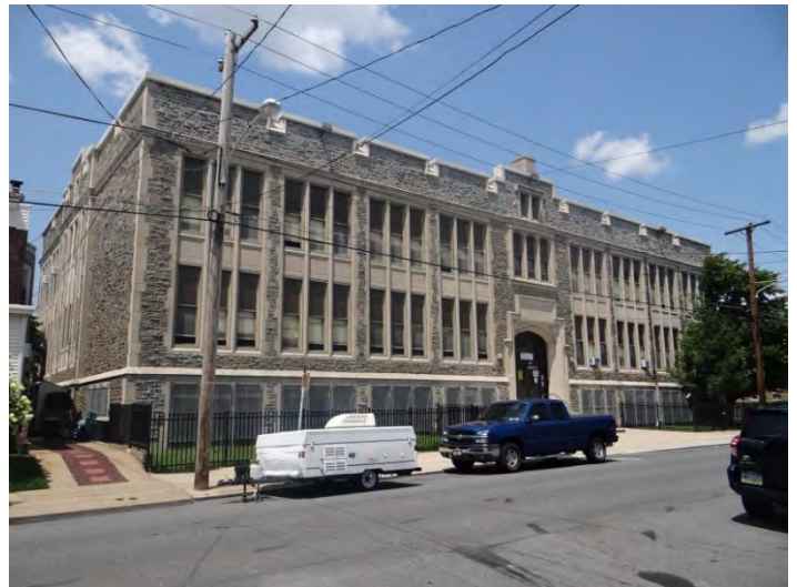
Photo 2: Looking N at main (SE) facade
