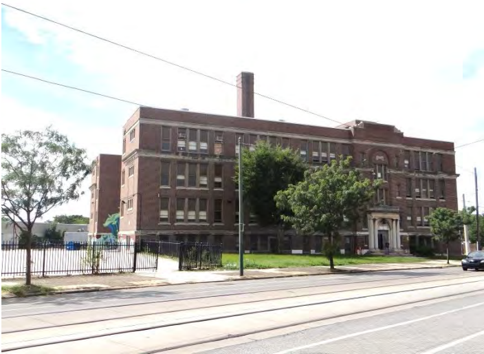
Photo 3: Looking SW at N façade
