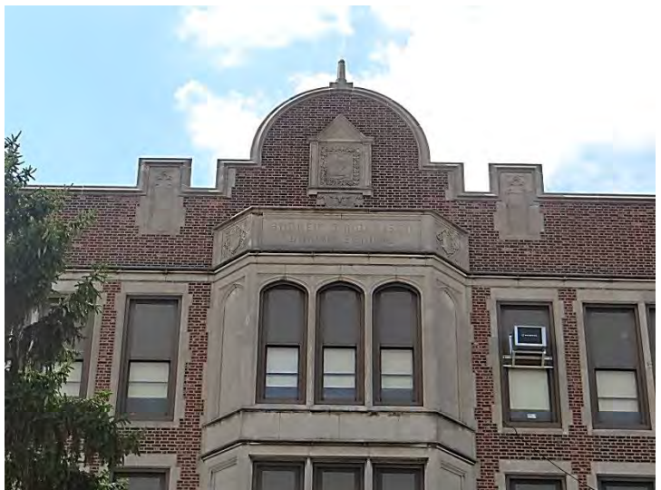
Photo 6: Looking W at nameplate in center of main (E) façade
