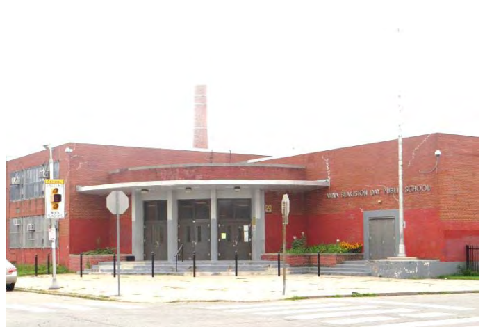
Photo 2: Looking S at main entrance at N end of building
