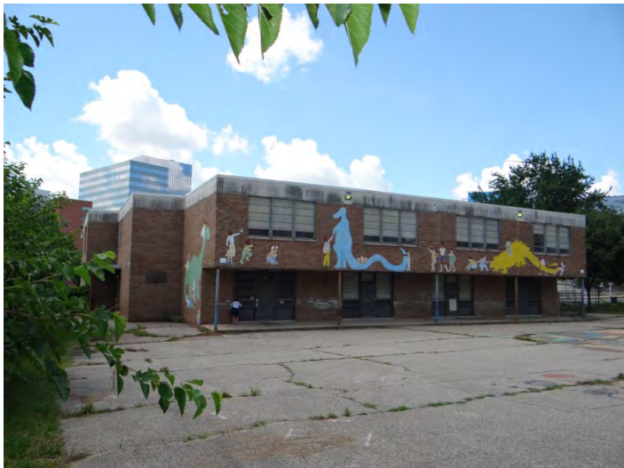
Photo 5: Looking SW at NE facade
