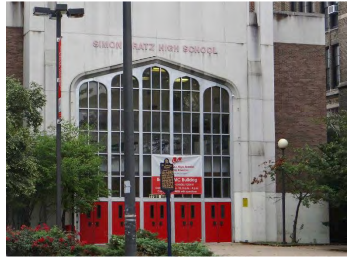
Photo 4: Looking E at main entrance on NW façade of addition
