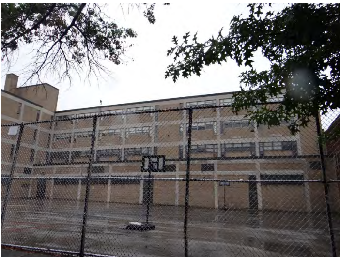
Photo 5: Looking E at W facade
