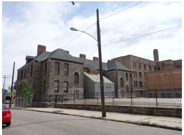
Photo 6: Looking N at rear (SW) facade
