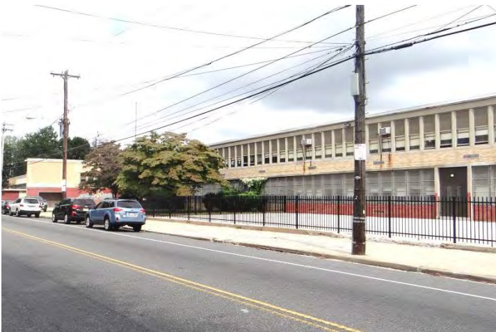
Photo 3: Looking NW at main (SW) facade
