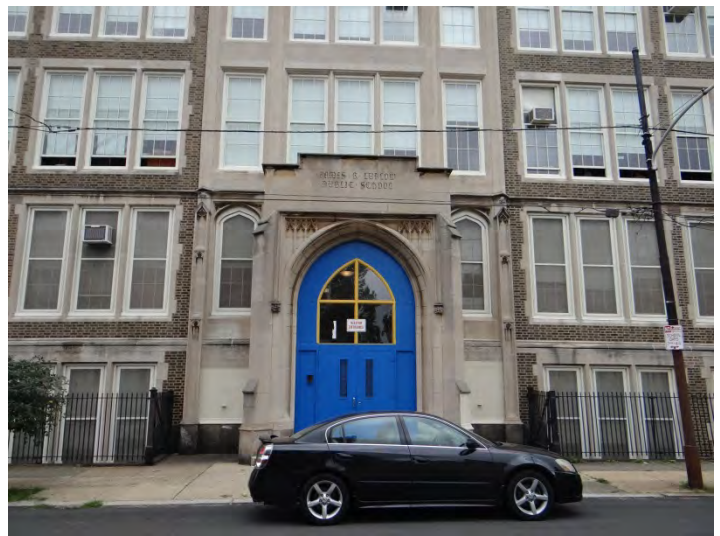
Photo 2: Looking E at main entrance on main (W) façade
