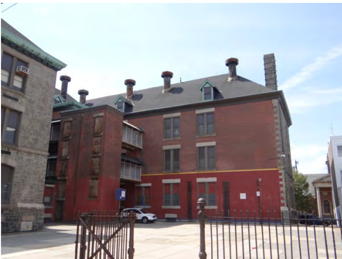
Photo 5: Looking SW at rear (E) facade
