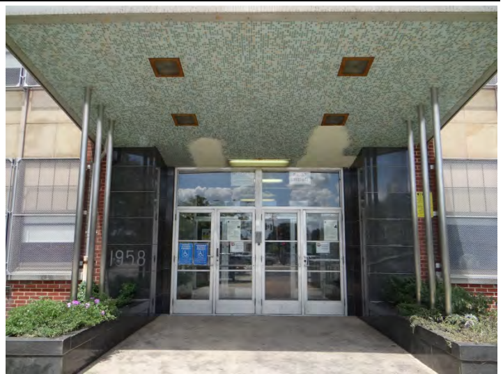
Photo 2: Looking NE at main (SE) entrance
