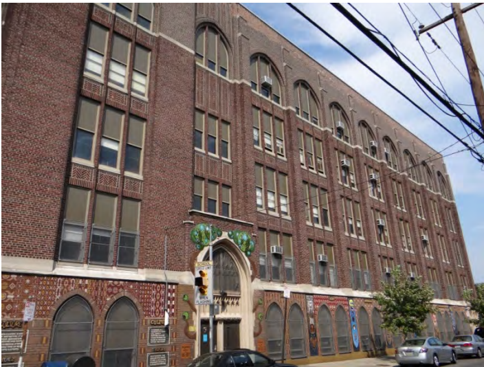
Photo 3: Looking N at S façade
