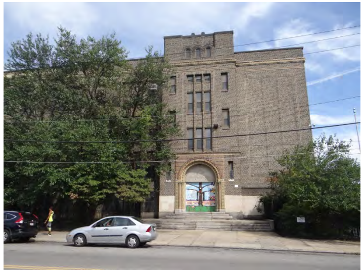
Photo 2: Looking E at W façade, S end
