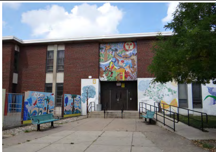
Photo 2: Looking N at main entrance on main (S) façade
