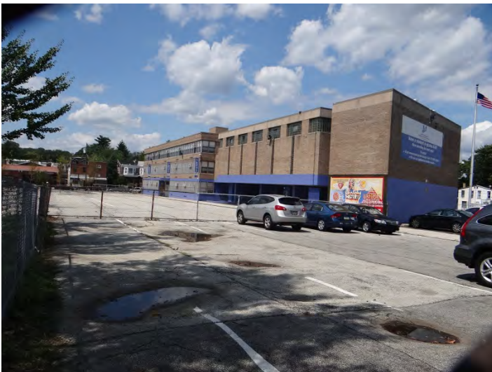
Photo 5: Looking N at SW facade
