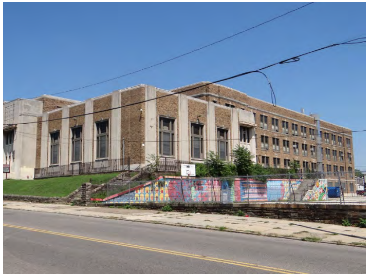
Photo 2: Looking N at SW (left) and SE (right) facades
