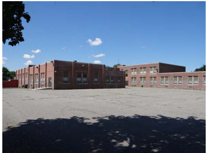
Photo 4: Looking SW at NE facade
