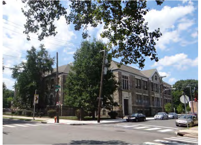
Photo 2: Looking W at SE corner, main (NE) façade to right
