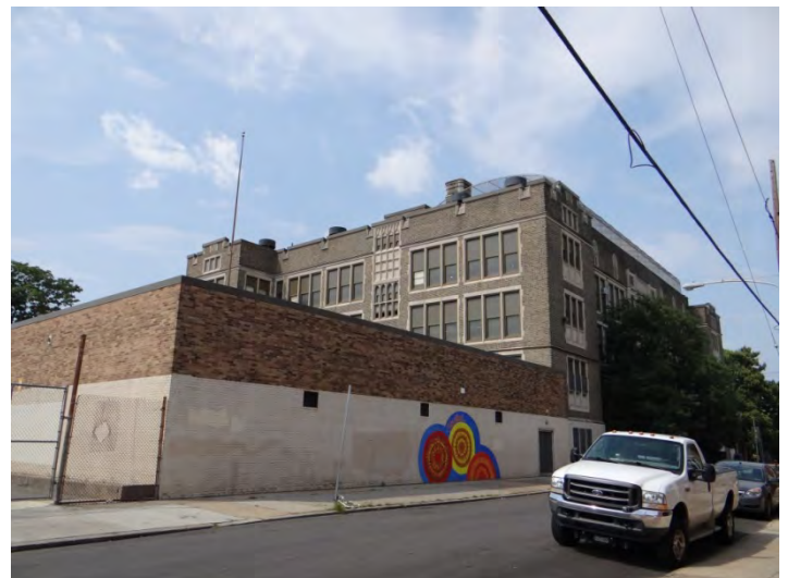
Photo 6: Looking NW at E facade
