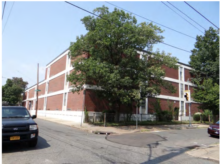
Photo 2: Looking N at main (SE, right) and SW (left) facades
