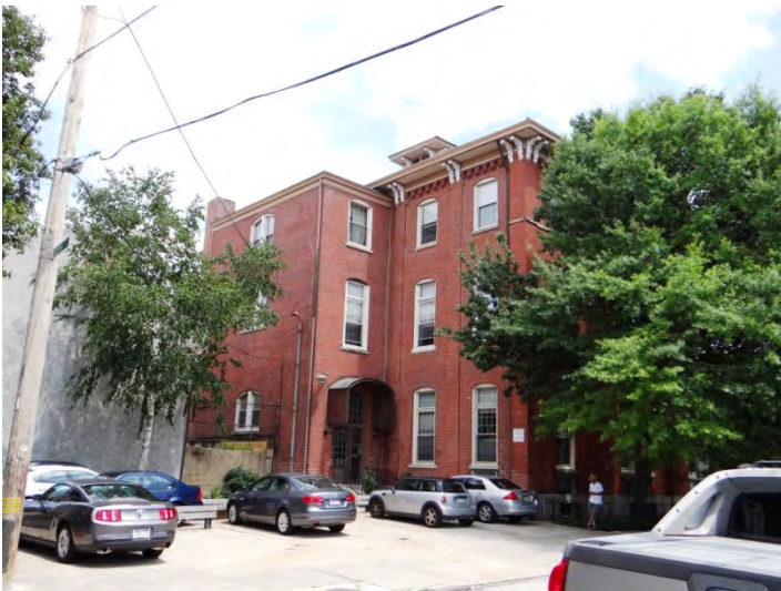
Photo 3: Looking NE at W façade
