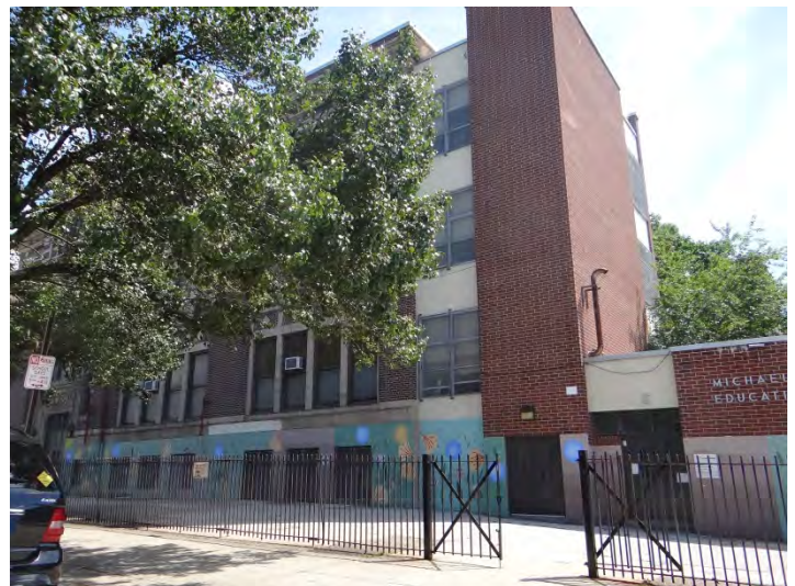
Photo 6: Looking NE at W façade
