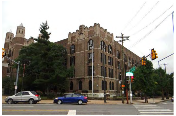
Photo 2: Looking SE at N (left) and W (right) facades
