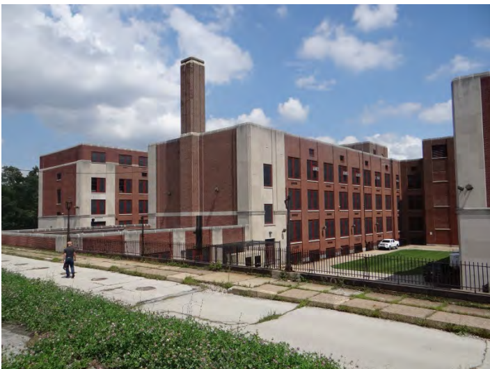
Photo 5: Looking NE at W facade
