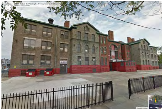
Photo 5: Looking NE at rear (S) façade. Source: Google Earth, September 2011
