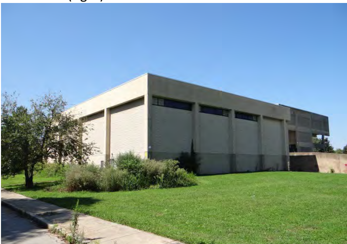
Photo 5: Looking SW at NE corner
