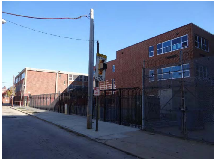
Photo 4: Looking N at SW facade
