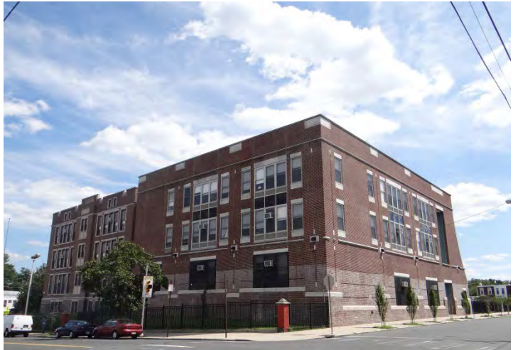
Photo 4: Looking SE at N (left) and W (right) facades
