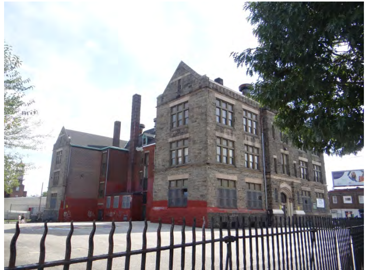
Photo 4: Looking S at NW (right) and NE (left) façades
