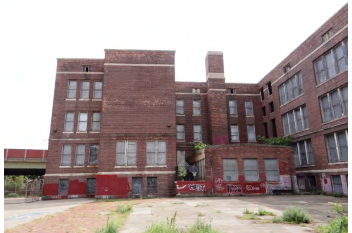
Photo 4: Looking S at rear (N) façade
