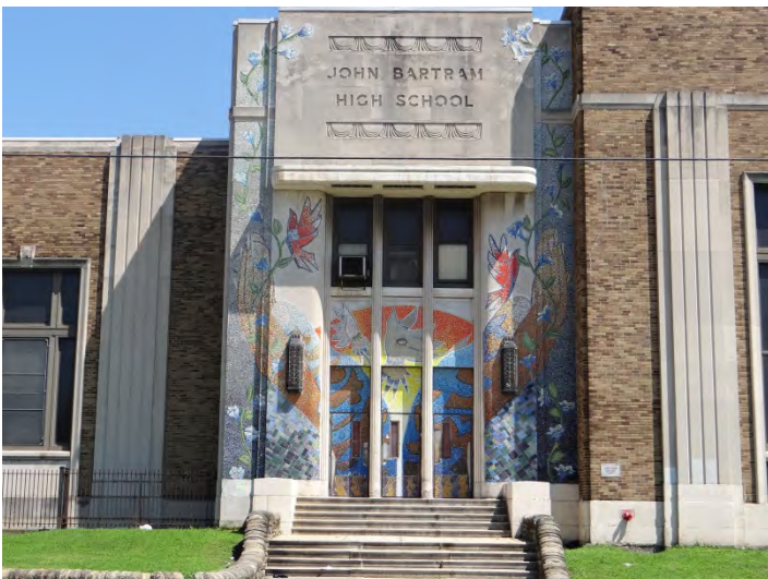
Photo 5: Looking NE at entrance at NW end
