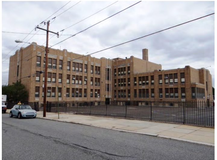
Photo 4: Looking SE at rear (NW) facade
