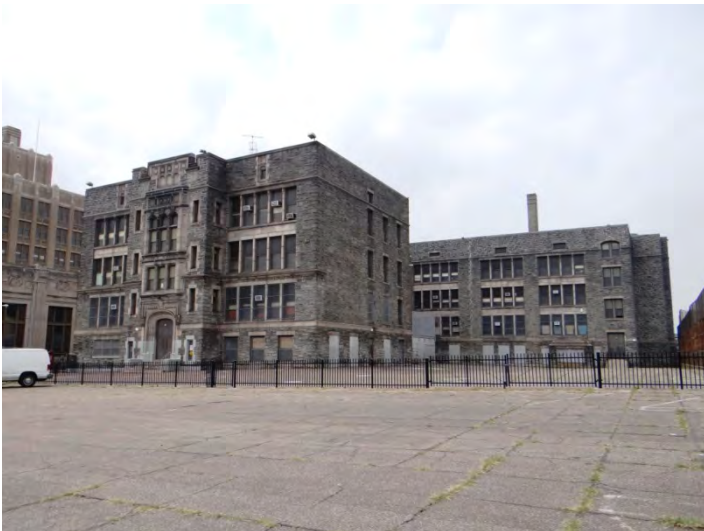
Photo 5: Looking SW at E facades
