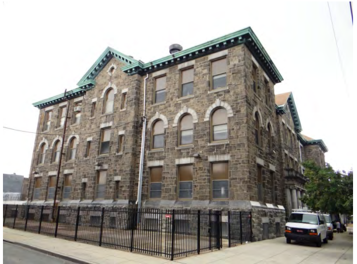
Photo 4: Looking S at N(left) and W (right) facades
