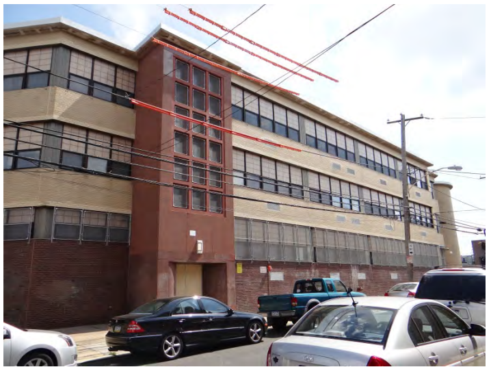
Photo 2: Looking SE at NW façade
