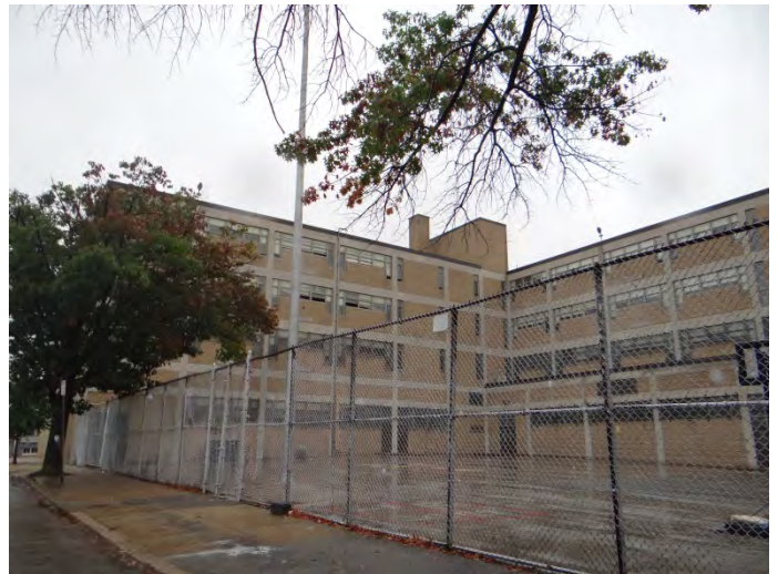
Photo 4: Looking NE at rear N (left) and W (right) facades
