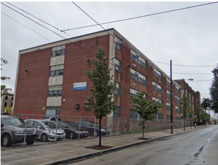
Photo 5: Looking N at rear (S, left) and E (right) facades
