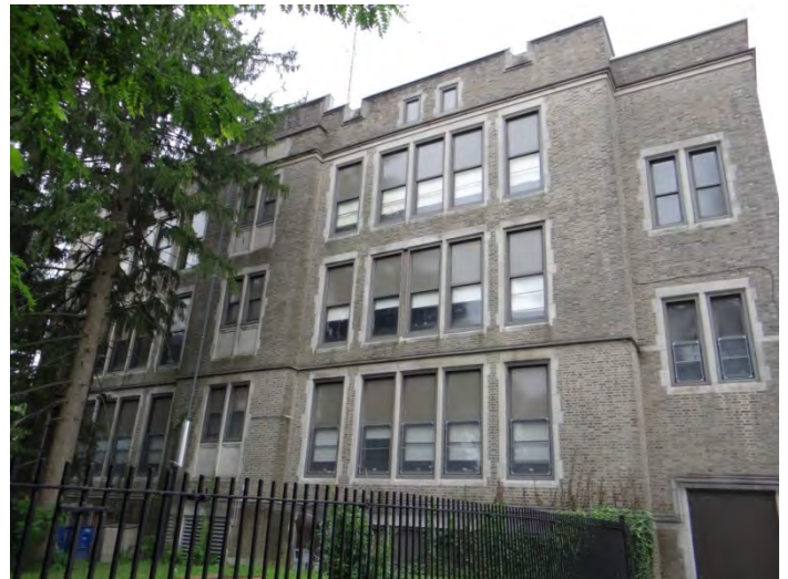
Photo 4: Looking SW at NE facade
