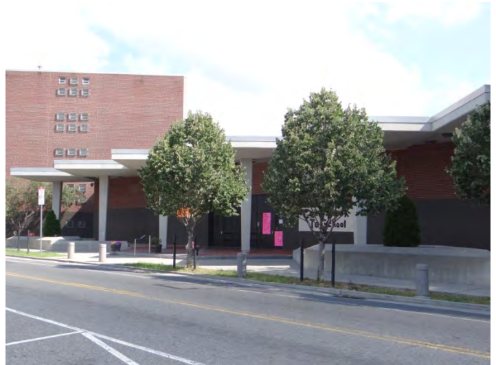
Photo 4: Looking NE at SW facade
