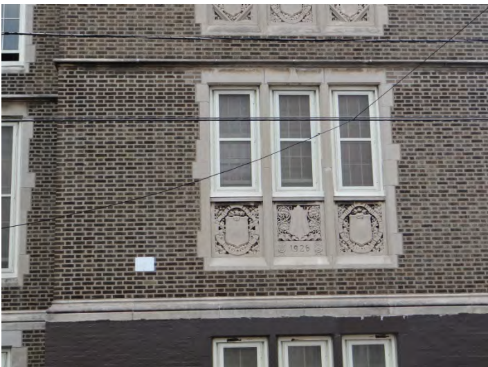
Photo 5: Window detail, main (W) façade
