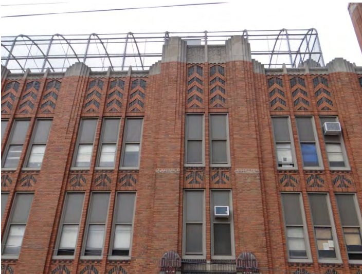
Photo 3: Looking W at brick and terra cotta details on main (E) façade
