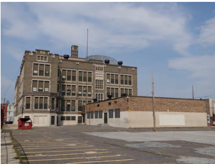
Photo 5: Looking N at S façade
