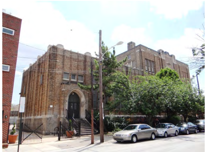
Photo 4: Looking SE at main (W) facade
