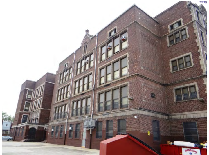
Photo 2: Looking NW at S facade
