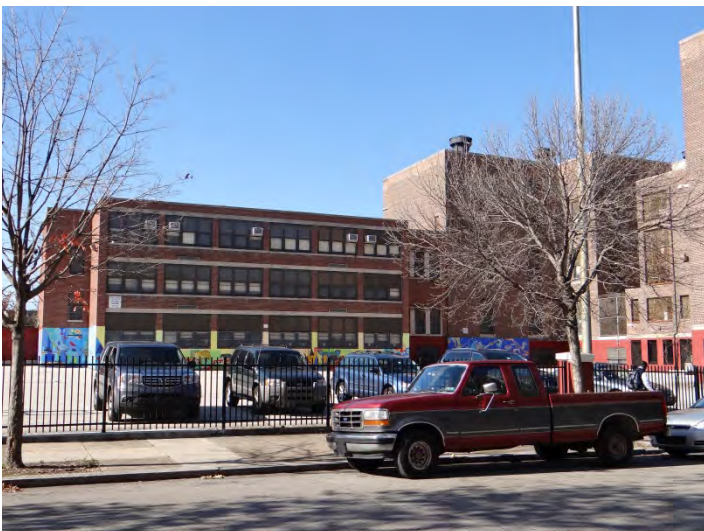
Photo 5: Looking W at E façade
