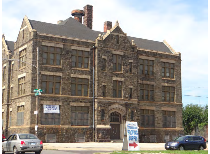
Photo 2: Looking N at SE façade
