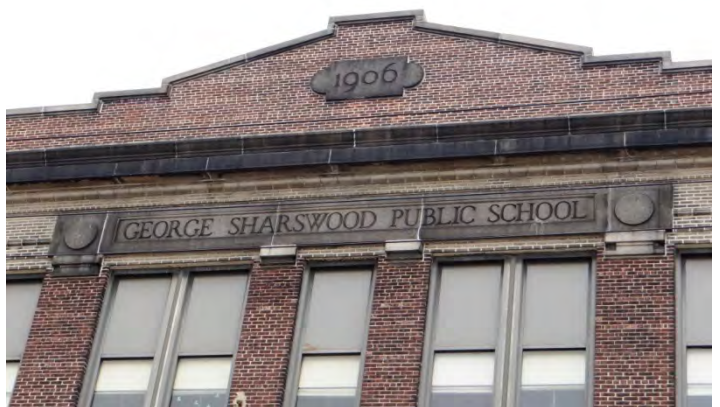
Photo 6: Looking W at E facade
