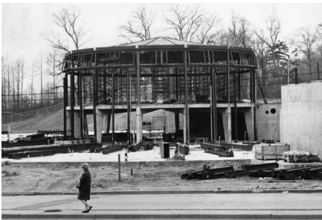
John Hancock Elementary in Northeast Philadelphia (1967, Sabatino & Fishman), shown under construction in the photo to the left. The school's round design reflects the experimental pedagogy explored at this demonstration school.
