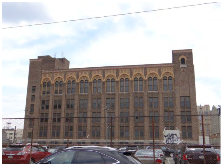
Photo 6: Looking S at rear (N) façade
