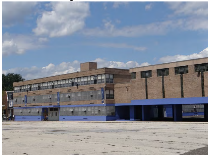
Photo 6: Looking N at NW half of SW facade
