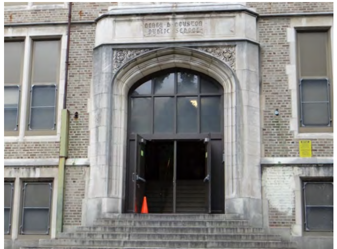
Photo 2: Looking N at main entrance, SE façade
