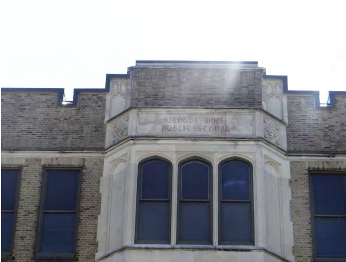
Photo 3: Detail, main (NW) façade
