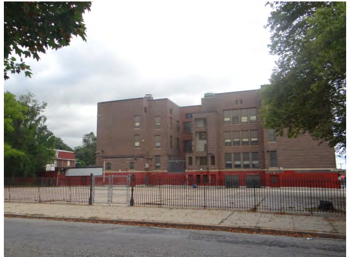
Photo 4: Looking E at W facade
