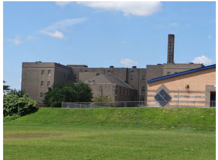
Photo 4: Looking W at rear (E) façade
