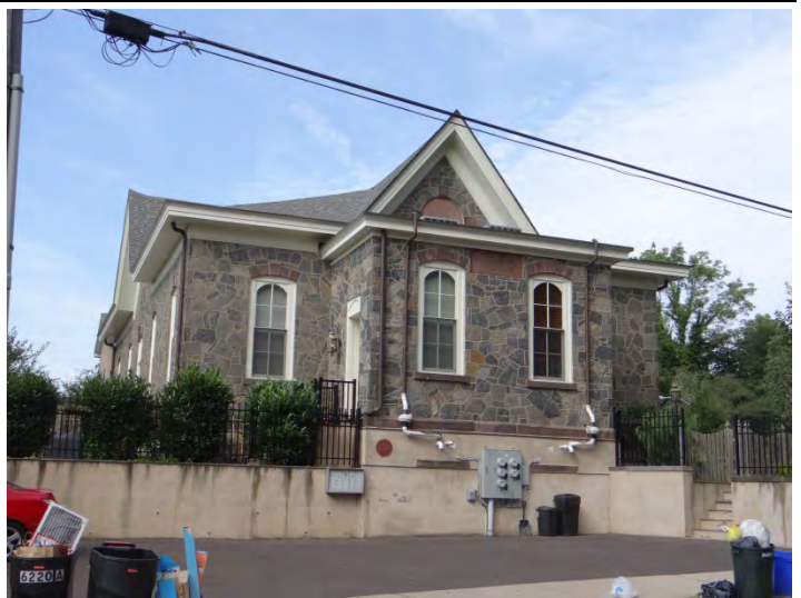
Photo 2: Looking SW at NE facade
