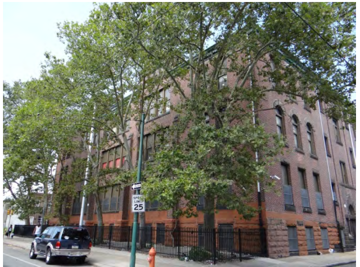
Photo 2: Looking NW at S façade
