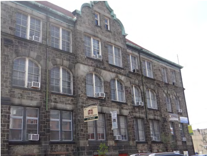
Photo 3: Looking S at NW façade
