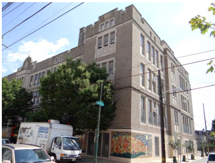
Photo 3: Looking NE at main (W, left) and S (right) facades
