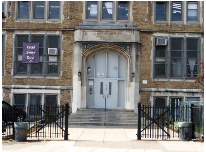
Photo 2: Looking SW at main entrance on NE façade
