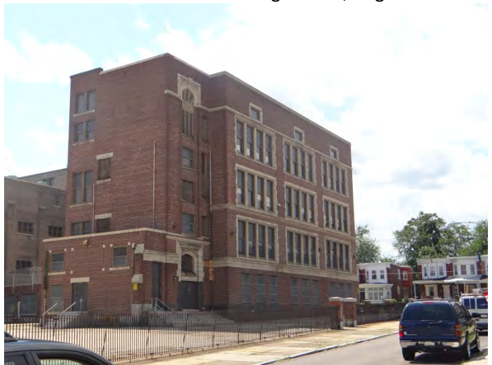
Photo 4: Looking SW at N façade
