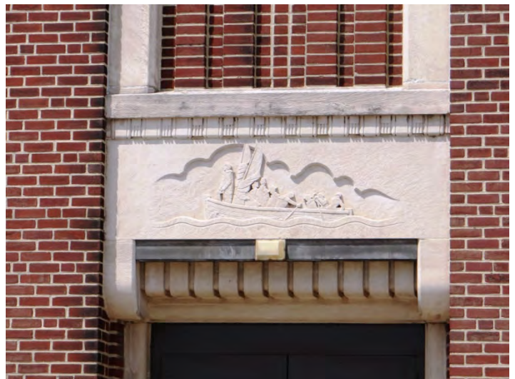
Photo 6: Detail, main entrance on main (E) facade
