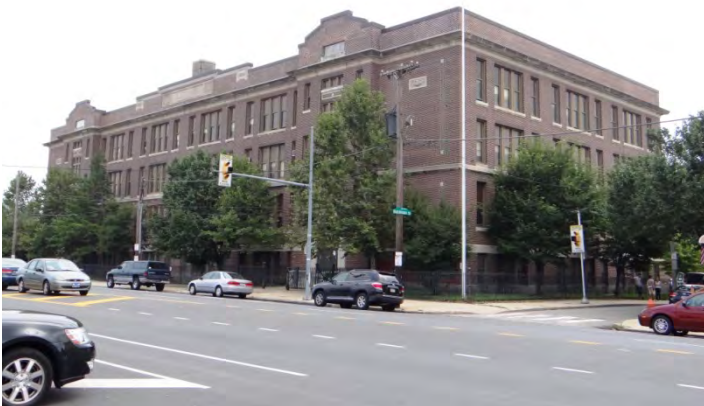
Photo 3: Looking SE at main (N, left) and W (right) facades
