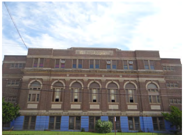
Photo 6: Looking E at W facade
