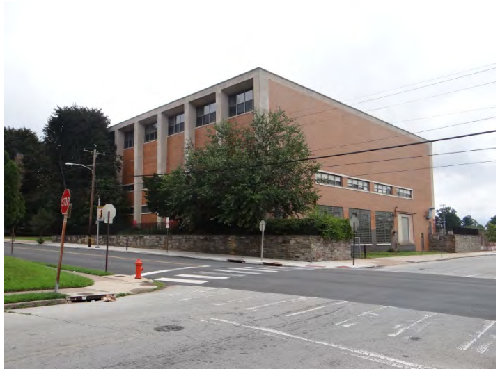
Photo 2: Looking NE at NW (left) and SW (right) facades
