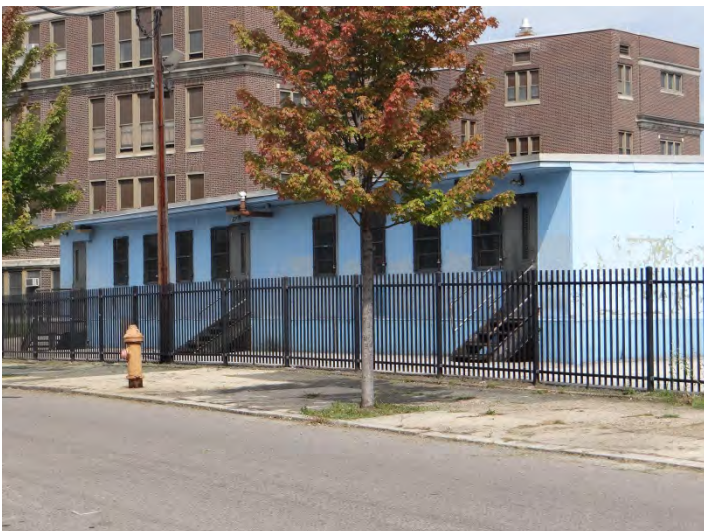
Photo 5: Looking NW at SW façade of portable
