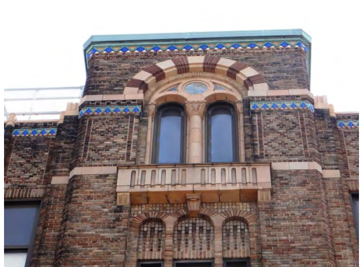
Photo 6: Looking S at N façade tower
