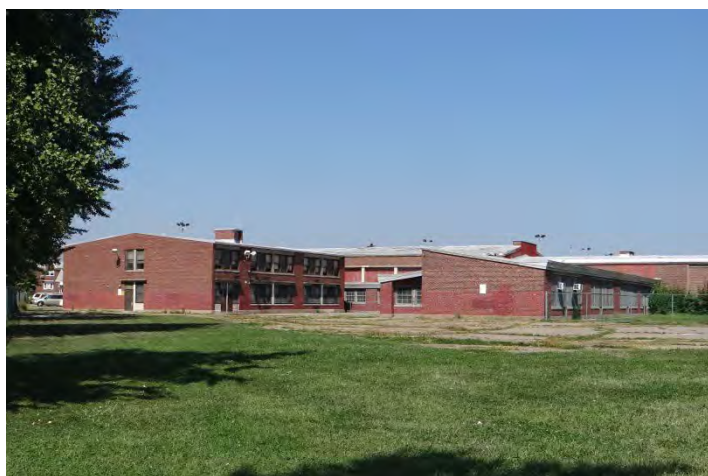
Photo 3: Looking N at westernmost wings on S façade
