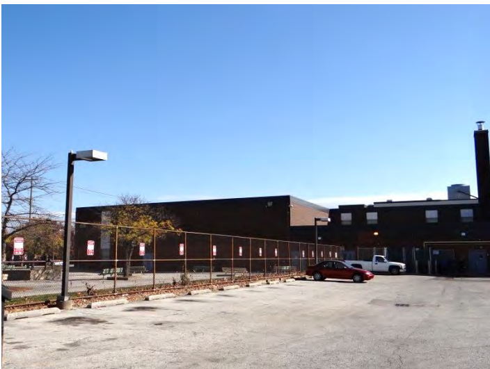
Photo 5: Looking E at N end of W facade
