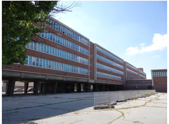
Photo 4: Looking SE at W facade
