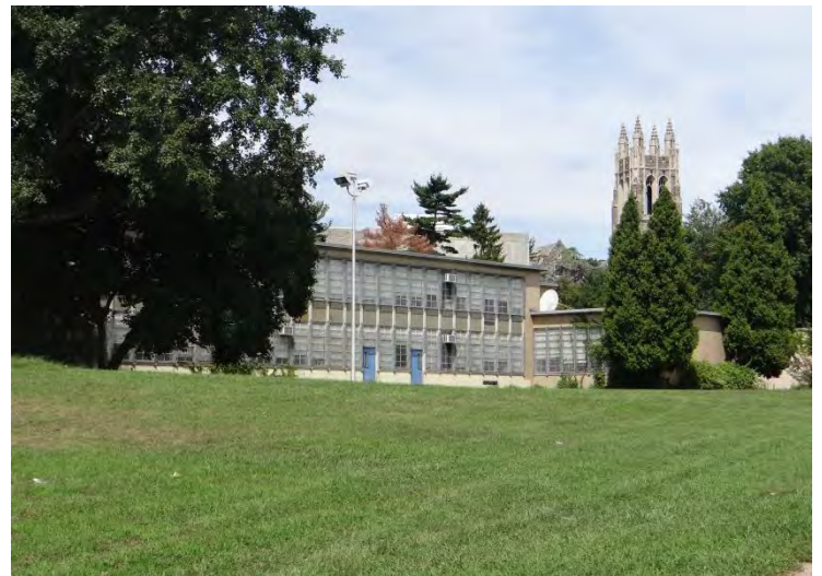
Photo 4: Looking N at NE end of main (SE) facade
