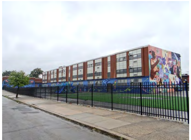
Photo 4: Looking SW at N (right) and E (left) facades
