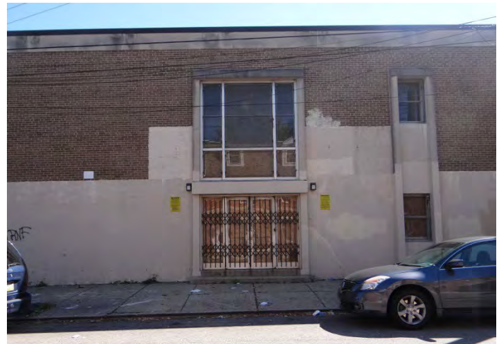
Photo 6: Looking E at entrance to secondary building, W façade
