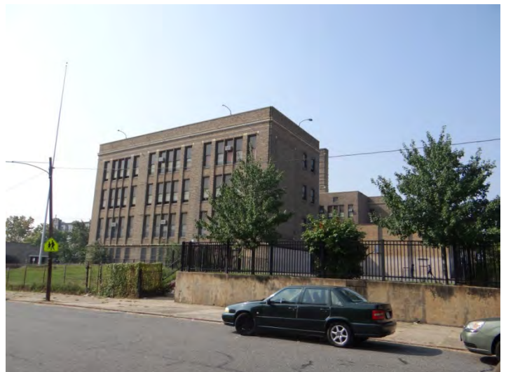
Photo 6: Looking S at NE facade
