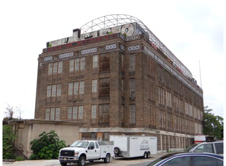
Photo 4: Looking SW at E (left) and N (right) facades
