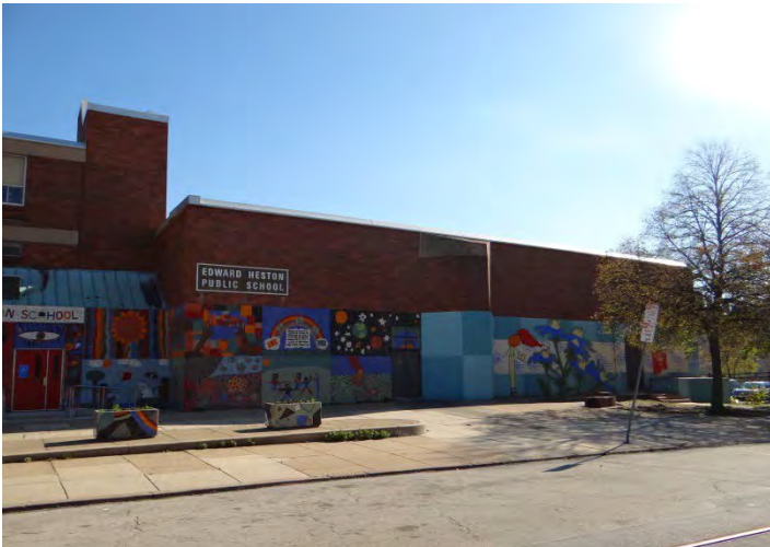
Photo 3: Looking SE at S end of main (W) façade
