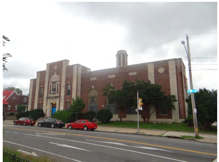
Photo 2: Looking NE at main (W) facade
