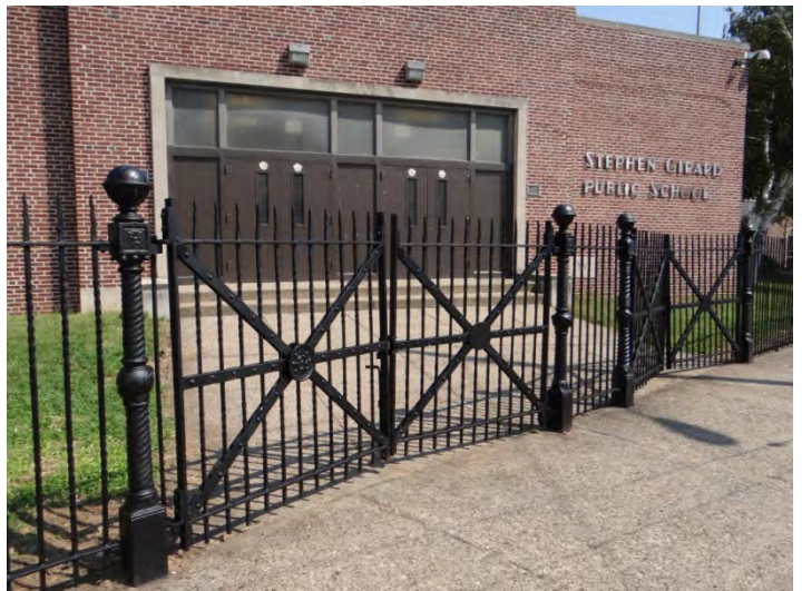
Photo 6: Looking N at main entrance on S facade
