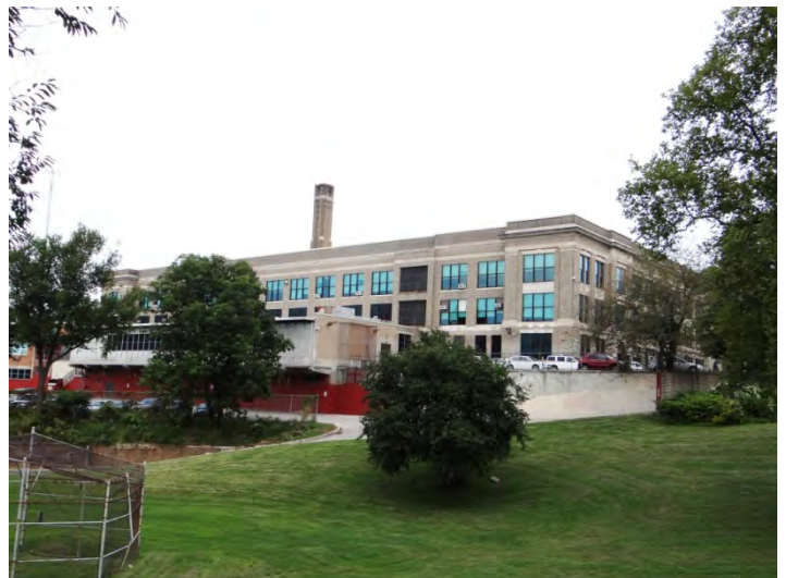
Photo 6: Looking NW at rear (S) facade
