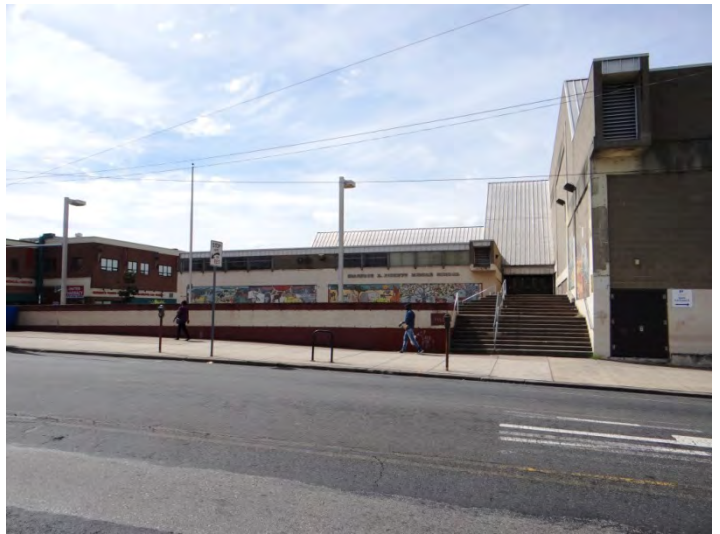
Photo 2: Looking SW at center of NE façade
