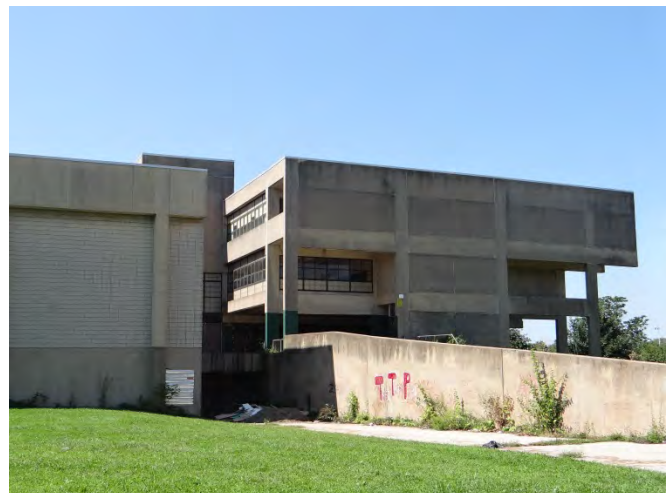
Photo 6: Looking SW at NE facade
