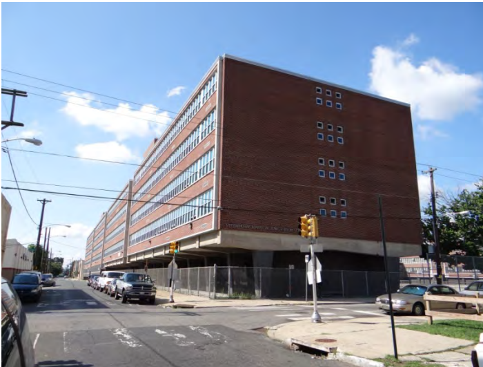
Photo 3: Looking SW at E (left) and N (right) facades
