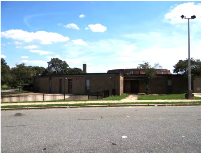
Photo 3: Looking E at W facade
