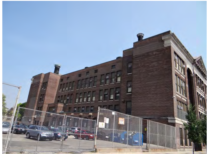
Photo 4: Looking NE at rear (W) facade
