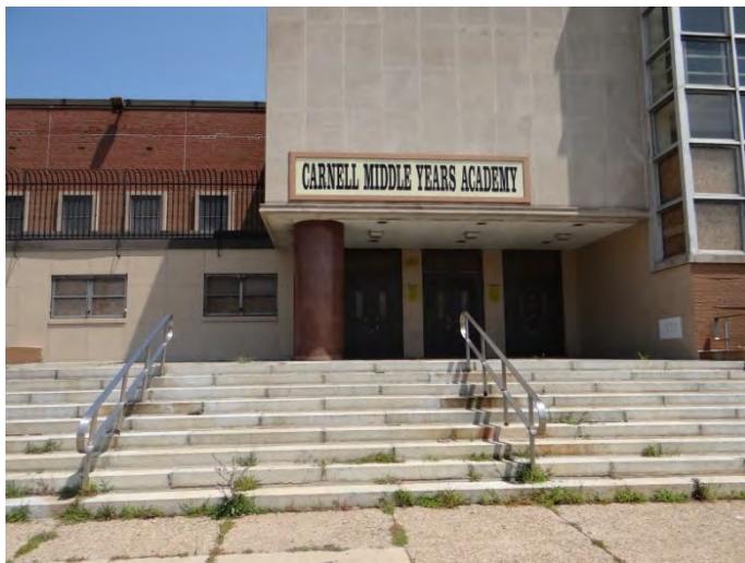
Photo 3: Looking NE at entrance on main (SW) facade
