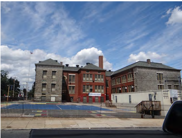
Photo 5: Looking N at rear (S) facade
