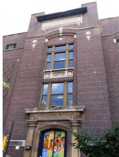
Photo 2: Looking S at N façade entrance
