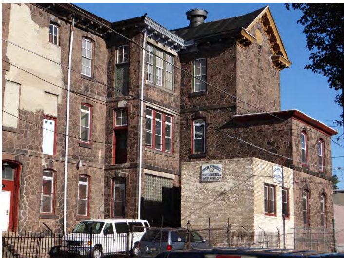
Photo 5: Looking NW at N half of E facade
