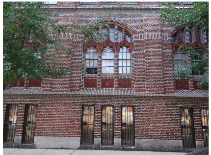
Photo 6: Detail, window/masonry design, typical
