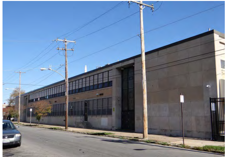
Photo 4: Looking NE at W facade
