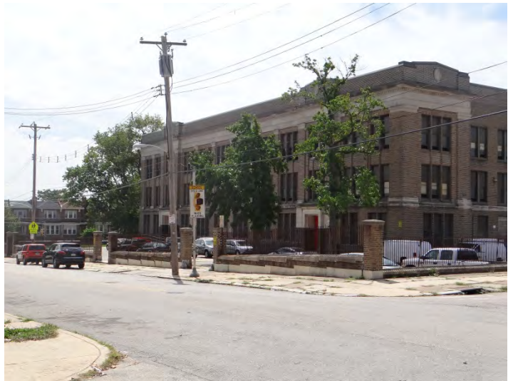
Photo 2: Looking S at NE facade
