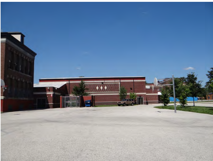
Photo 5: Looking NW at E façade, new addition
