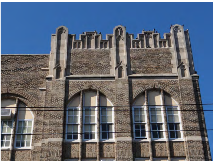
Photo 5: Detail, looking S at 4 th floor windows/parapet
