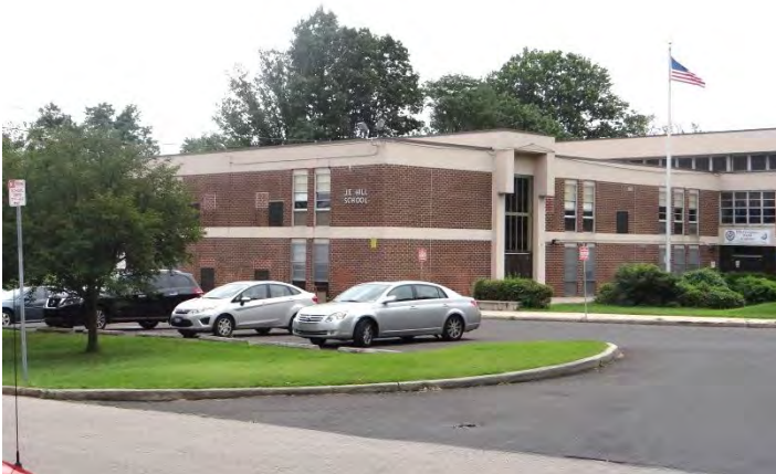
Photo 3: Looking SE at N façade of NE wing
