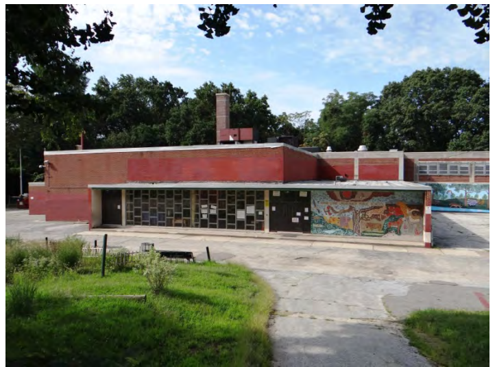
Photo 2: Looking SW at S end of NE facade
