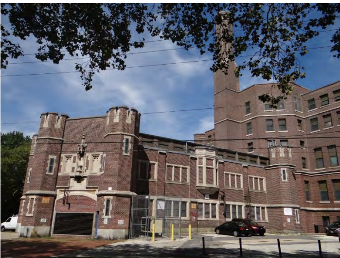
Photo 5: Looking NE at rear (S) façade
