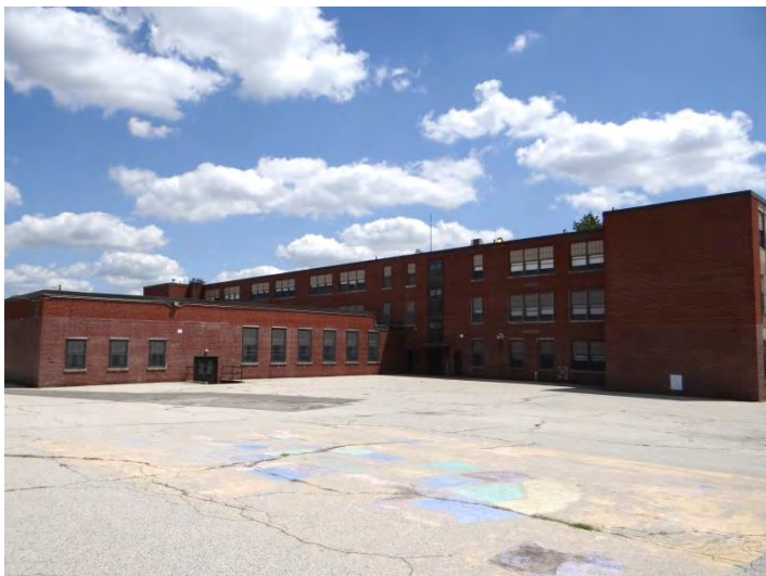
Photo 5: Looking E at rear (NW) façade
