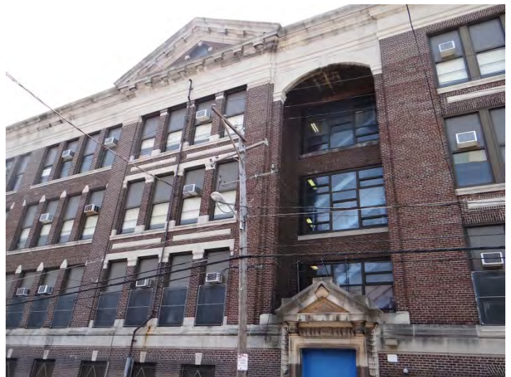
Photo 6: Looking S at W end of N facade
