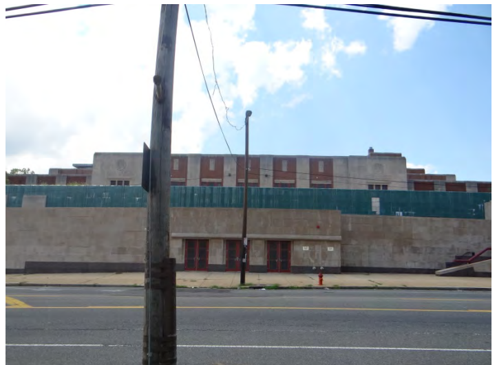
Photo 6: Looking W at E façade
