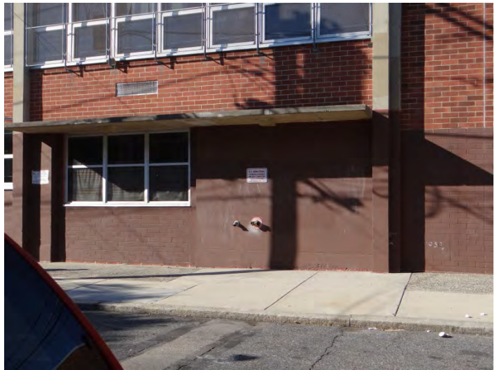
Photo 2: Looking W at entrance at N end of NE facade
