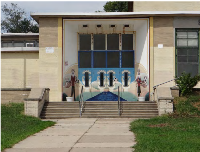
Photo 3: Looking NW at main entrance on main (SE) facade
