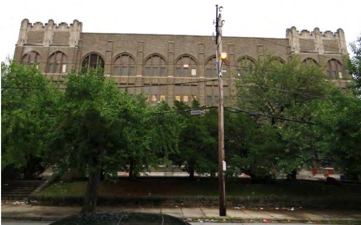
Photo 3: Looking E at W facade
