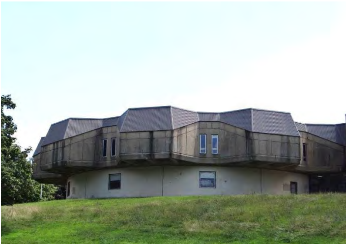
Photo 3: Looking S at N wing on NW facade
