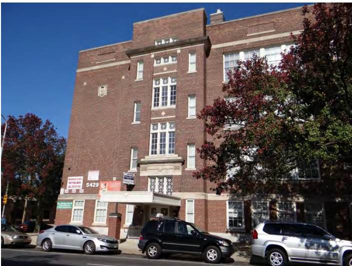
Photo 5: Looking N at S façade
