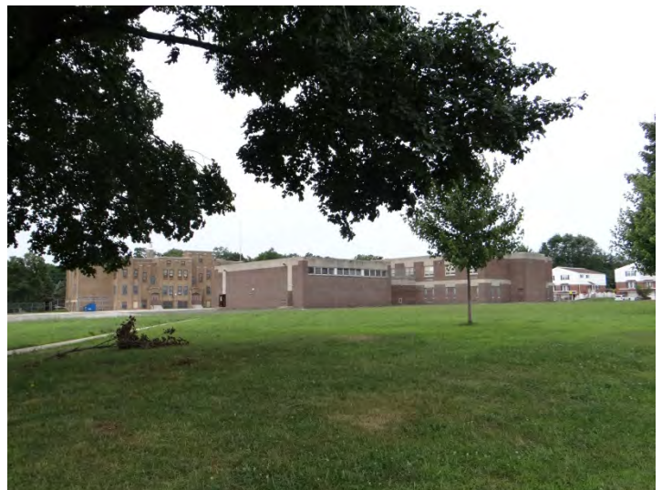
Photo 6: Looking SW at NE facades
