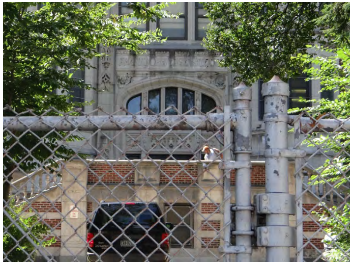
Photo 2: Looking W at main entrance on main (E) façade
