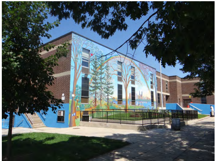
Photo 2: Looking N at SE wall
