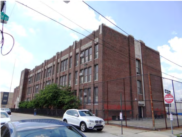
Photo 3: Looking SW at main (E, left) and N (right) facades
