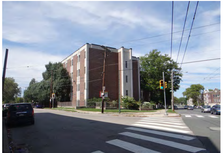
Photo 4: Looking NW at SW (left) and SE (right) facades of 1960s addition
