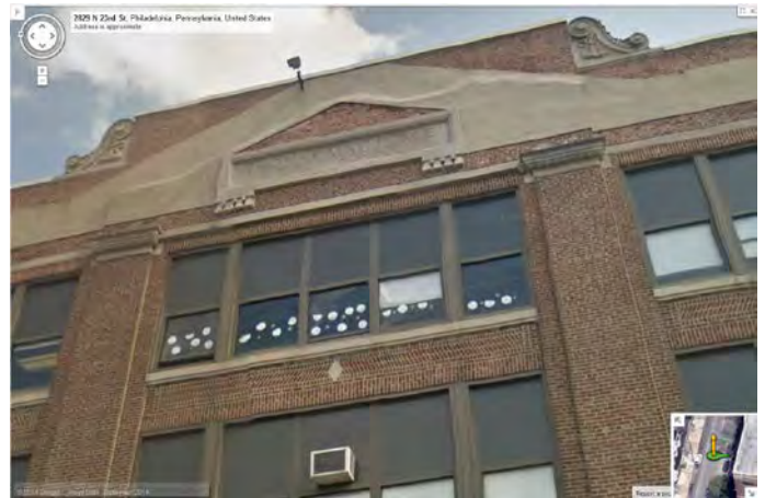
Photo 4: Looking NE at center bay of W façade. Source: Google Earth
