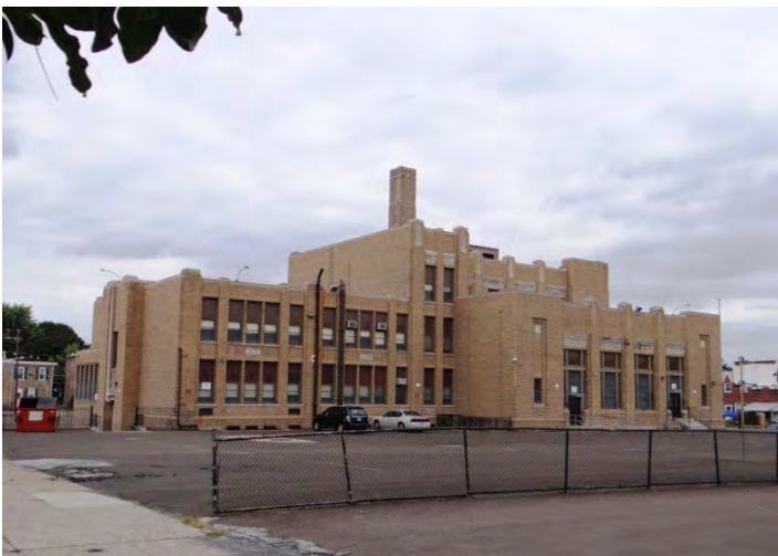
Photo 5: Looking NE at SE facade
