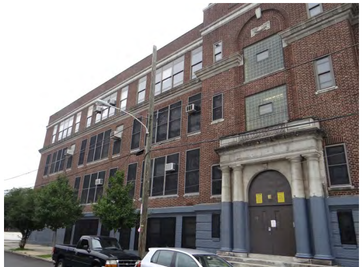
Photo 6: Looking SE at W façade
