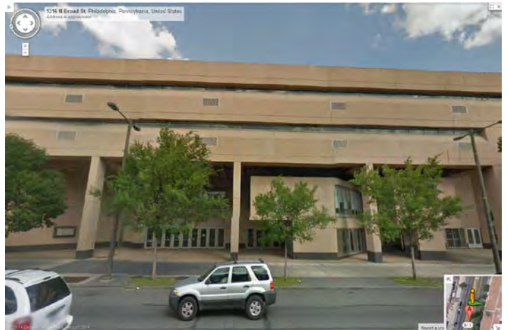
Photo 4: Looking E at main (W) façade and main entrance
