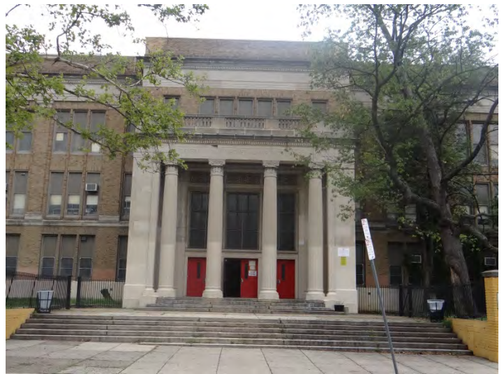
Photo 2: Looking N at main entrance on S facade
