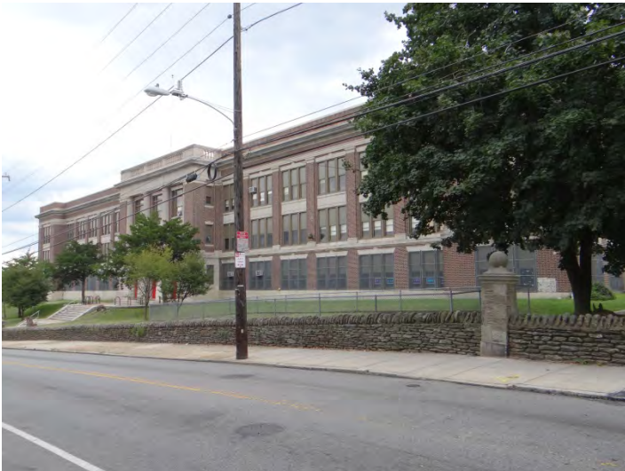
Photo 3: Looking NE at main (NW) facade
