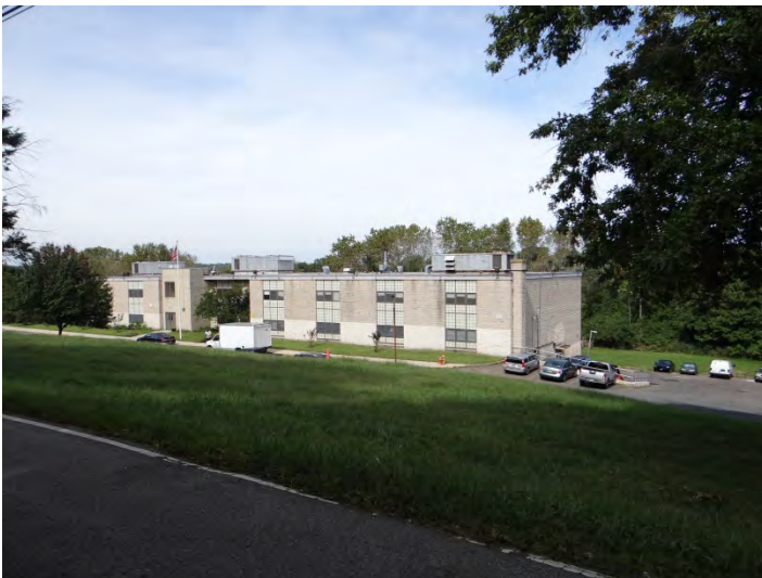
Photo 3: Looking SW at main (SE, left) and NE facades
