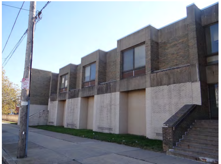
Photo 2: Looking SE at N facade
