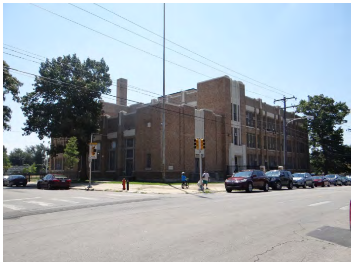
Photo 6: Looking S at NW (right) and NE (left) facades
