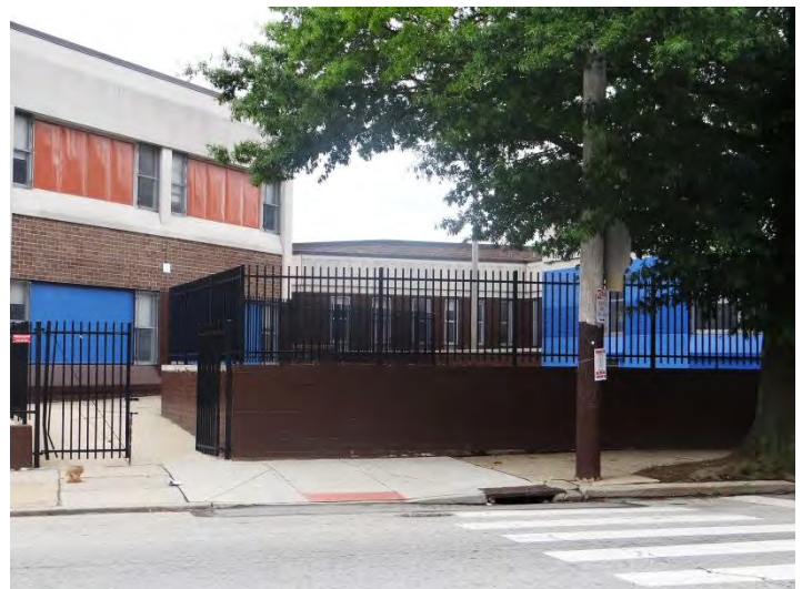
Photo 6: Looking S at N façade
