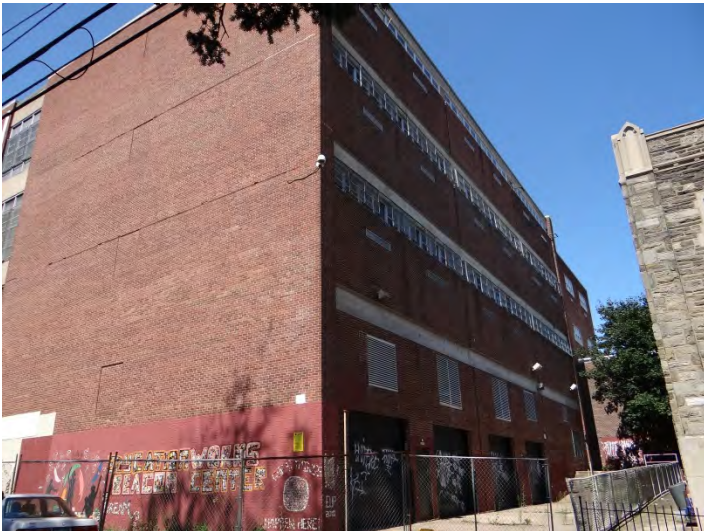
Photo 3: Looking W at N wing of SE facade
