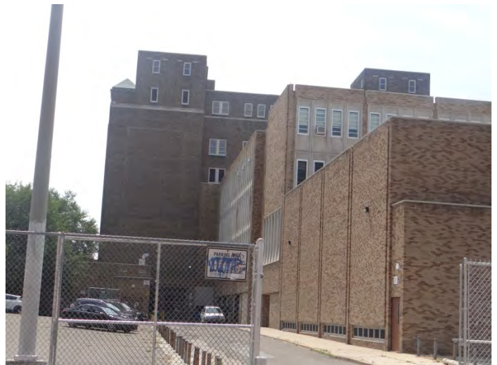
Photo 6: Looking S at NE facade
