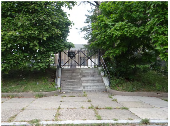
Photo 6: Looking W at steps to playground
