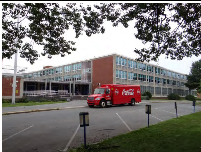
Photo 2: Looking SE at main entrance on main (W) facade
