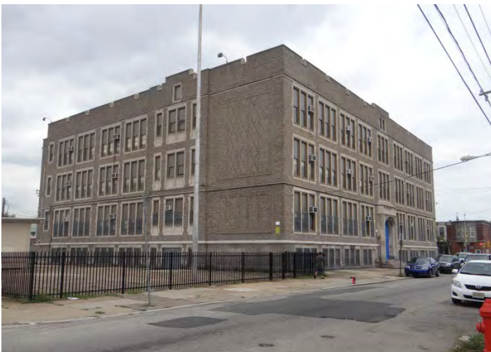
Photo 5: Looking NE at SW (left) and main (SE, right) facades
