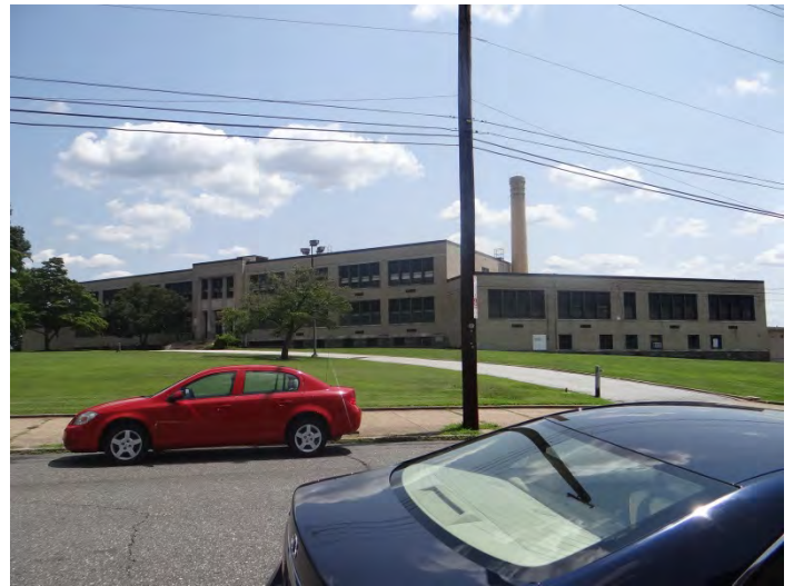
Photo 2: Looking S at main (N, left) and NE (right) facades
