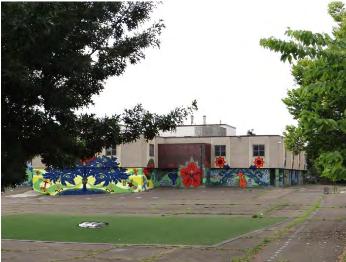
Photo 3: Looking SE at rear (N) façade
