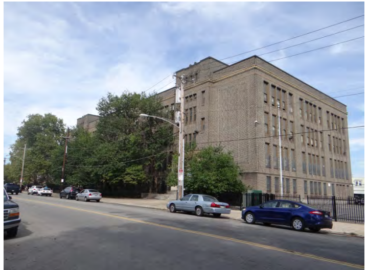
Photo 4: Looking NE at W (left) and S (right) facades
