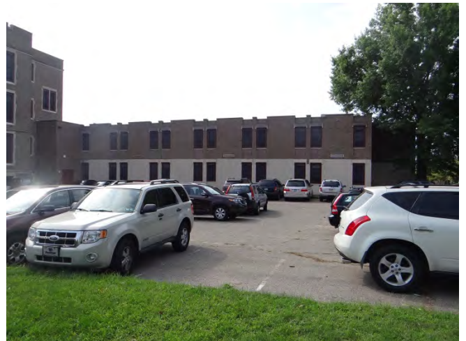
Photo 4: Looking S at N façade of addition
