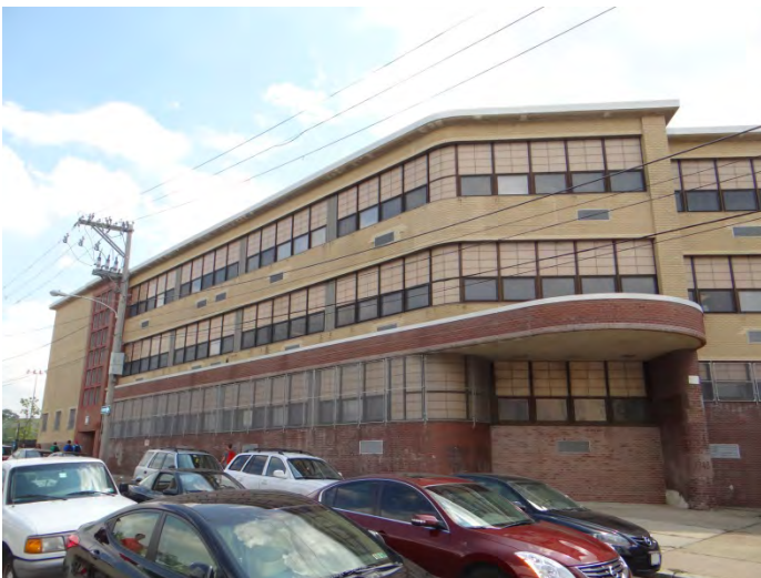
Photo 5: Looking SE at NE façade
