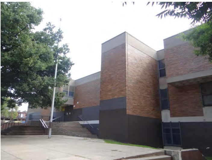
Photo 5: Looking NE at N end of W facade
