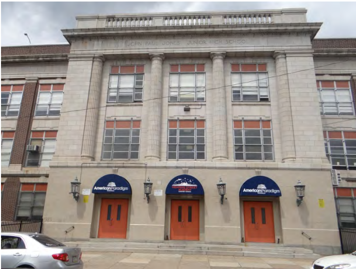
Photo 3: Looking N at main entrance on main (SE) facade
