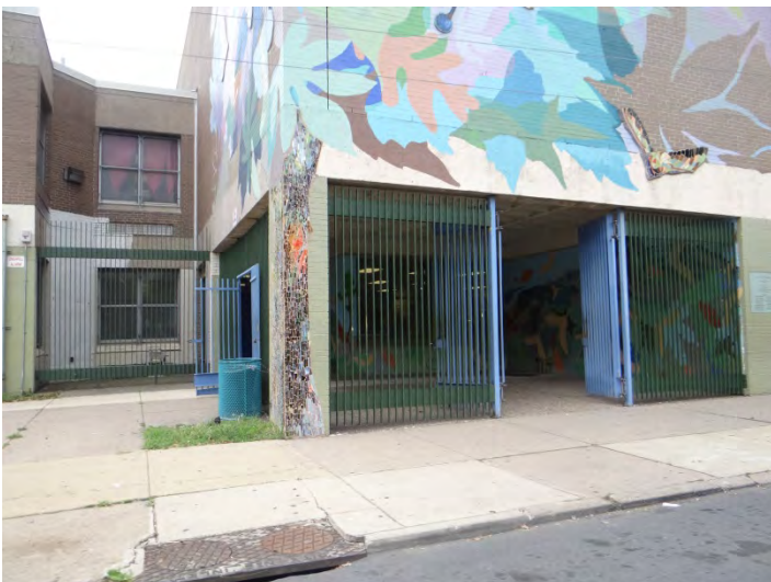
Photo 5: Looking S at entrance in center of N facade
