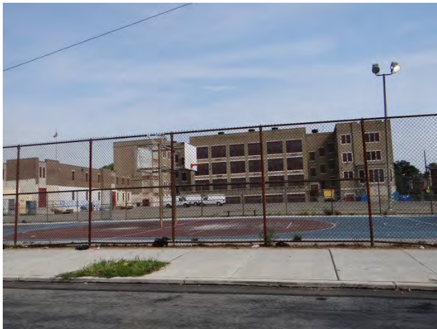
Photo 3: Looking N at rear (S) façade
