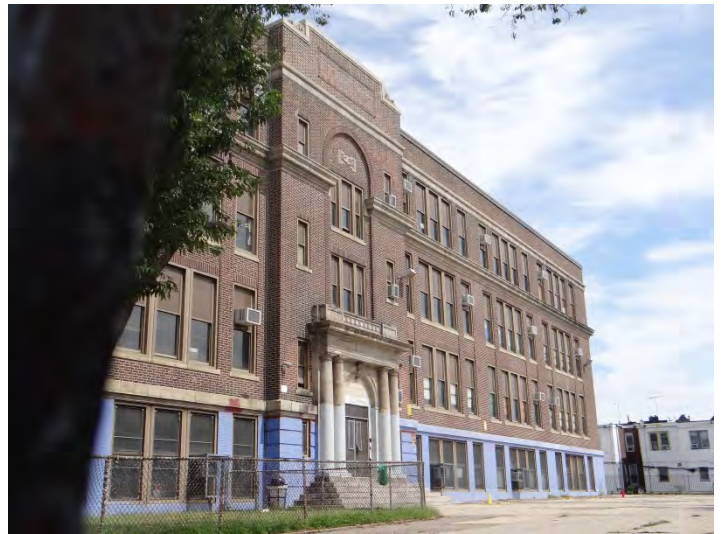
Photo 2: Looking NE at S facade
