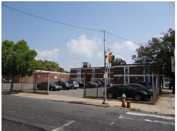
Photo 4: Looking E at rear (NW) façade
