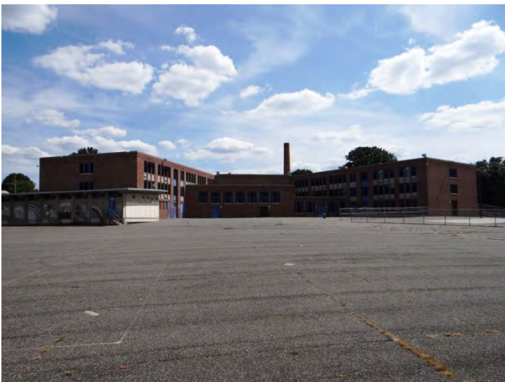
Photo 5: Looking S at rear (NW) facade
