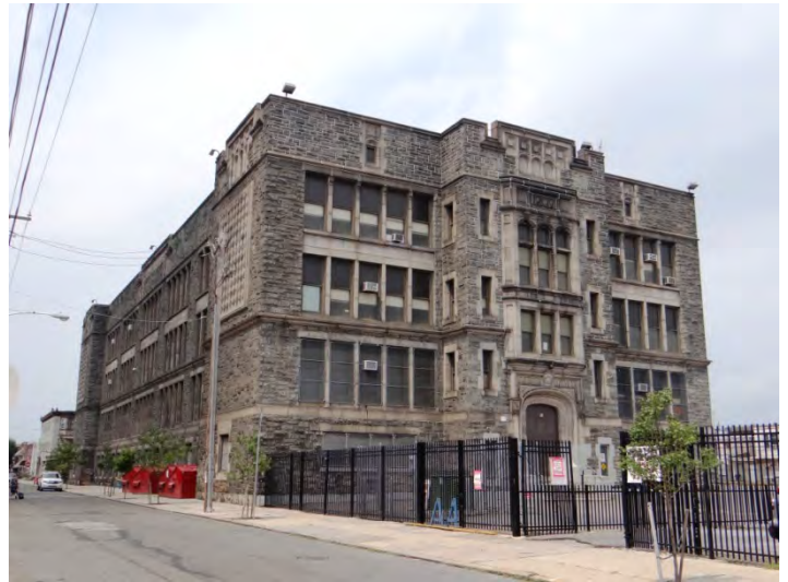
Photo 4: Looking W at S (left) and E (right) facade
