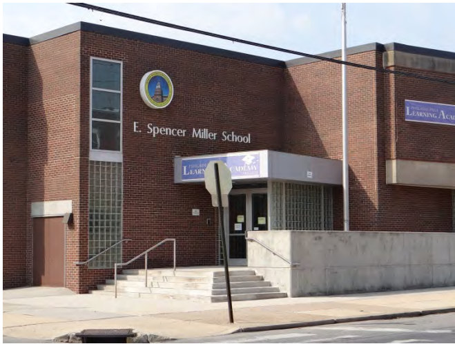
Photo 1: Looking S at N façade entrance
