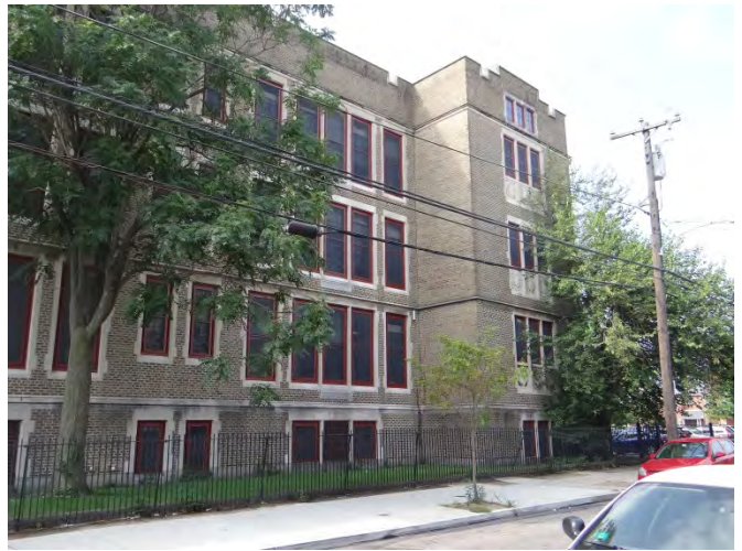
Photo 2: Looking SW at W end of main (N) façade
