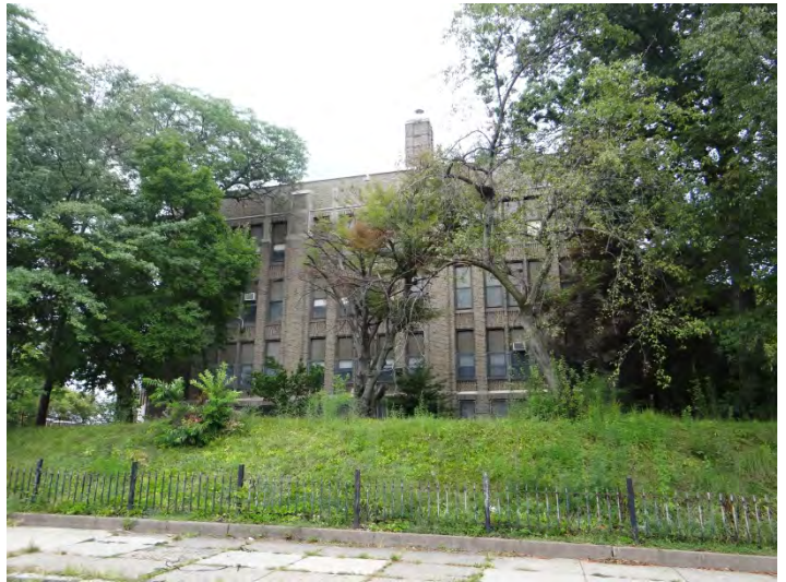
Photo 4: Looking NW at SE facade
