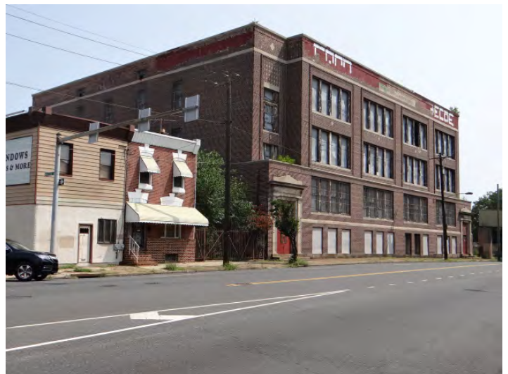
Photo 6: Looking NE at W (left) and main (S, right) façade
