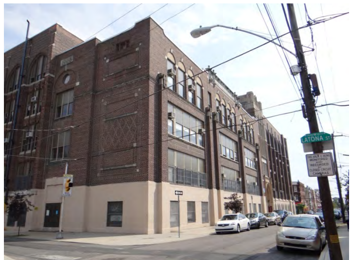
Photo 6: Looking W at N facade
