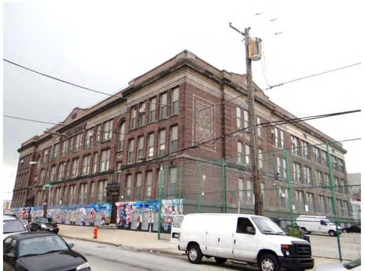
Photo 2: Looking SW at main (E, left) and N (right) facade
