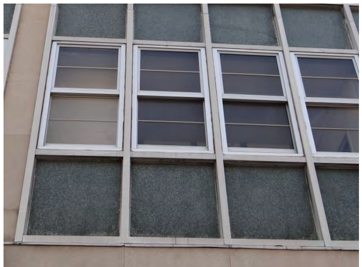
Photo 6: Detail, typical window bay
