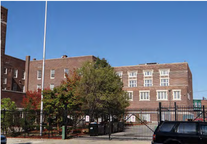
Photo 3: Looking N at S façade of N wing
