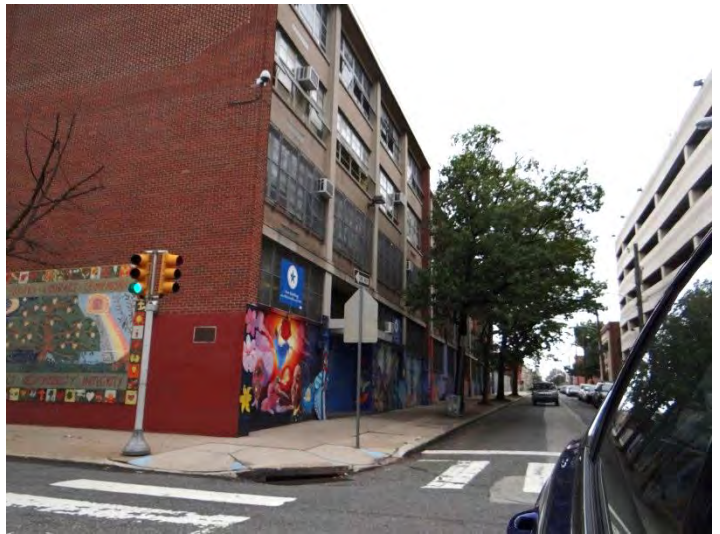
Photo 2: Looking N at E facade
