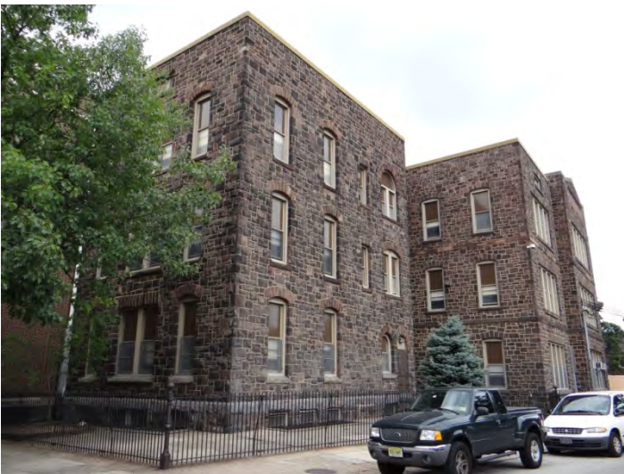
Photo 5: Looking E at S façade
