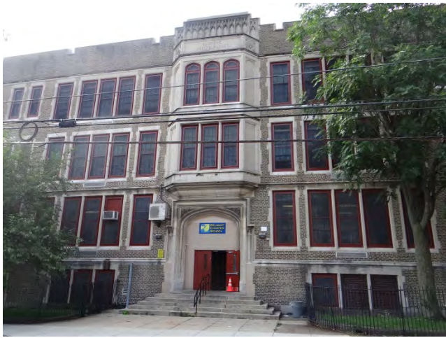
Photo 1: Looking S at main (N) façade
