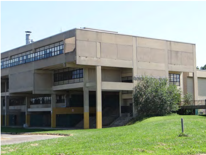
Photo 3: Looking NE at SW corner, NW (left) and SW (right) facades
