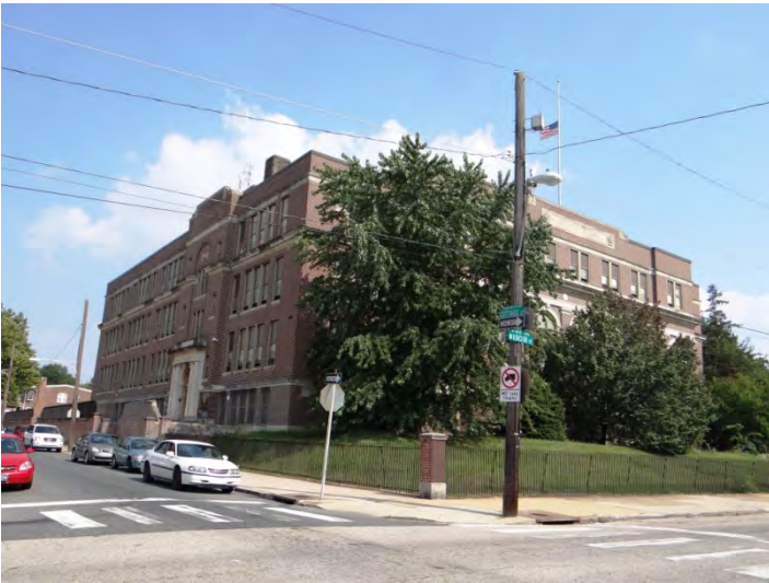
Photo 3: Looking SE at SW (right) and NW (left) facades
