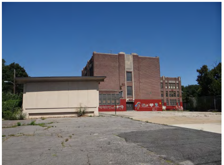
Photo 6: Looking NW at SE facades
