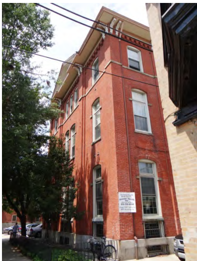
Photo 5: Looking W at S facade
