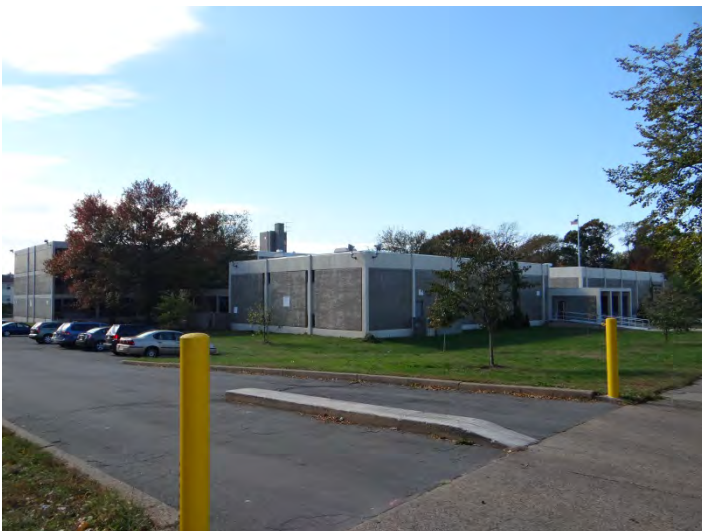
Photo 5: Looking SW at main (N, right) and E facades
