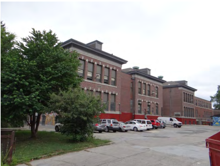
Photo 3: Looking S at rear (NW) facade
