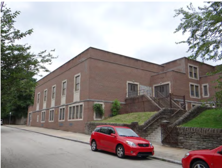
Photo 5: Looking N at SW façade of 1954 addition
