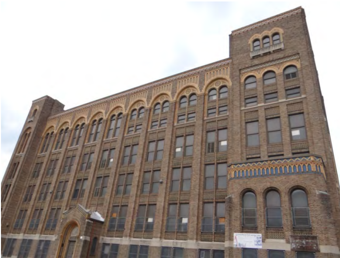
Photo 3: Looking NW at S facade
