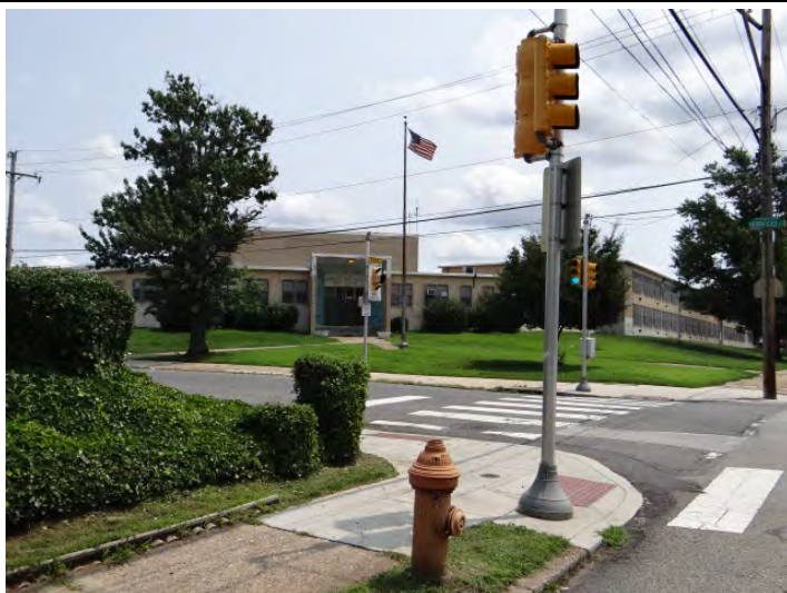
Photo 2: Looking SE at main (E, center) and SW facades
