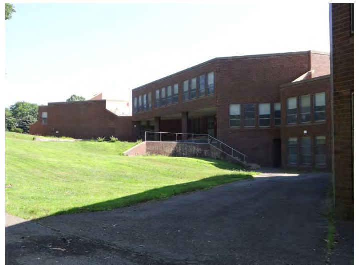
Photo 6: Looking Ne at center of W facade
