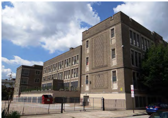
Photo 5: Looking SW at rear (E) façade
