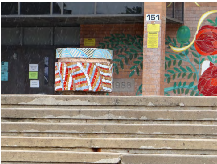
Photo 5: Looking N at entrance main entrance on S façade
