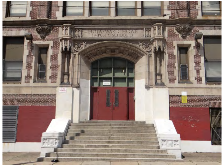
Photo 2: Looking W at main entrance on E facade
