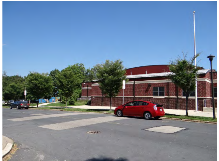
Photo 4: Looking N at SW façade, new addition
