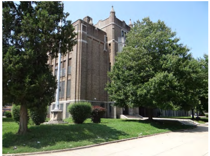
Photo 2: Looking SW at main (NE, right) and SE facades
