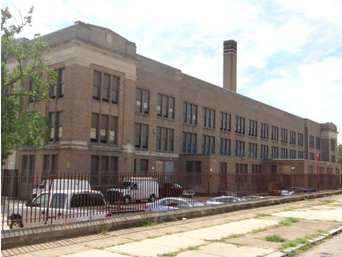
Photo 3: Looking SW at rear (NW) façade
