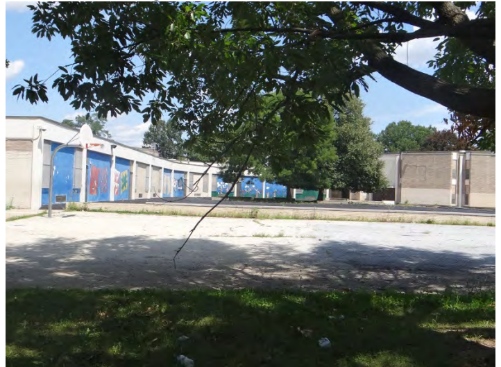
Photo 6: Looking NW at SE facade
