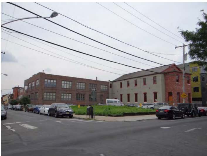
Photo 3: Looking NW at school and connected factory building
