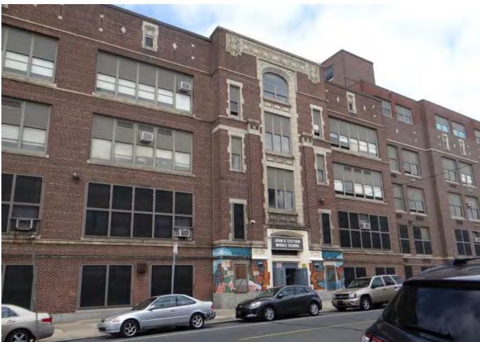
Photo 5: Looking W at main entrance in center of main (E) facade
