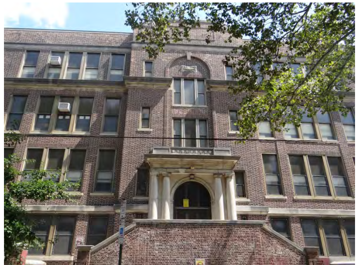
Photo 4: Looking W at S end of E facade
