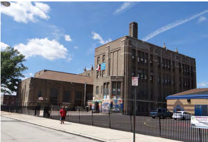
Photo 5: Looking SW at rear (SE, left) and NE (right) facades
