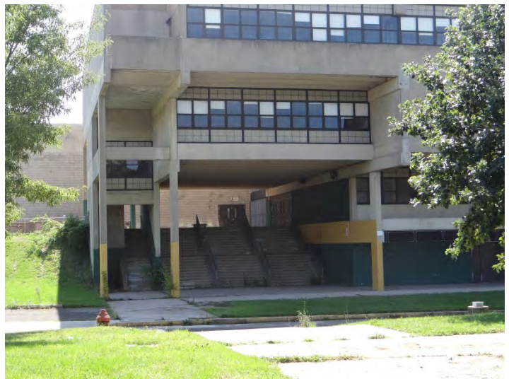
Photo 2: Looking SE at N end, NW facade
