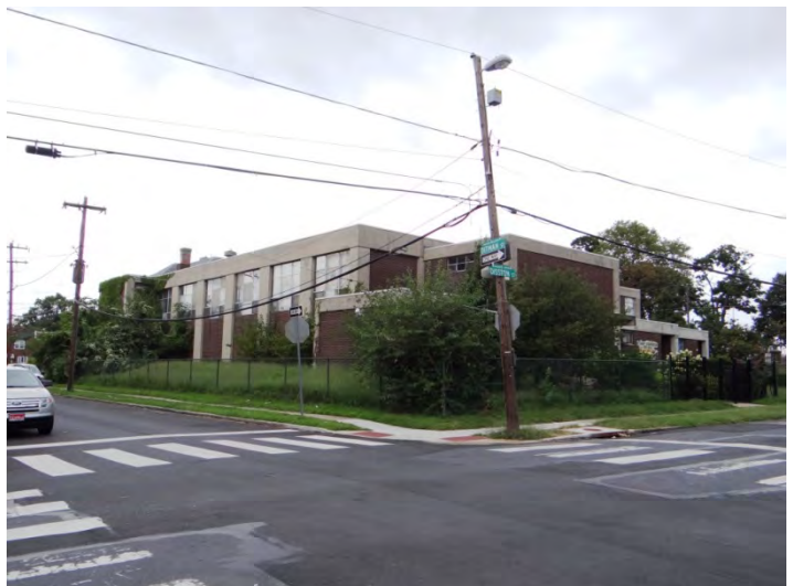
Photo 6: Looking W at SE facade
