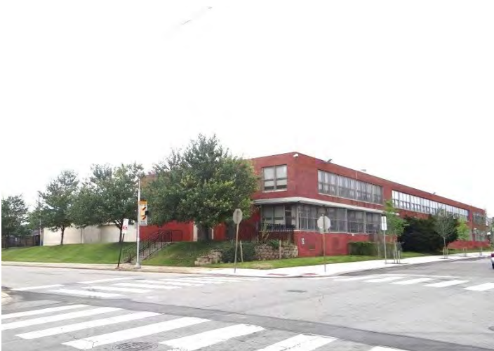
Photo 5: Looking SW at SE (left) and NE (right) facades
