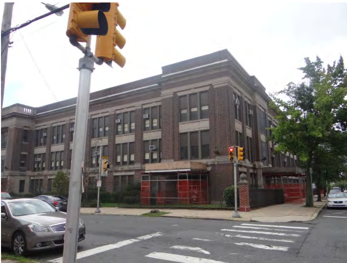
Photo 3: Looking SE at N (left) and W (right) facades
