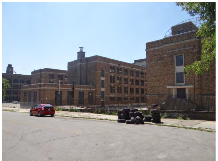
Photo 6: Looking SE at NE facade
