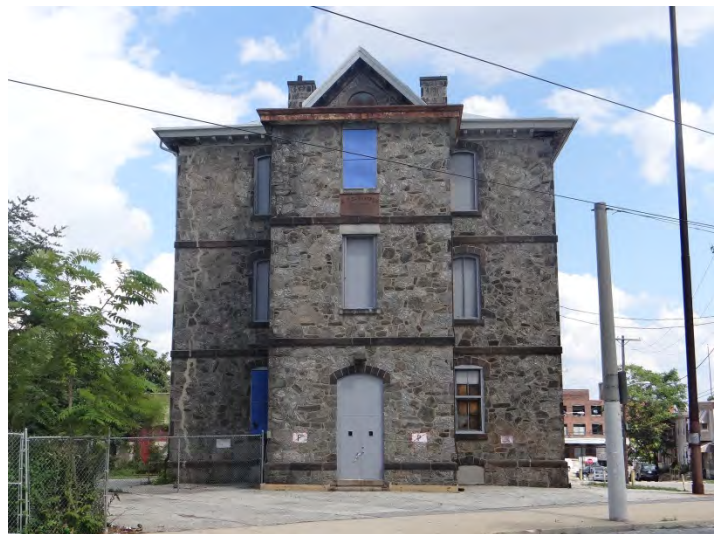
Photo 2: Looking E at W façade
