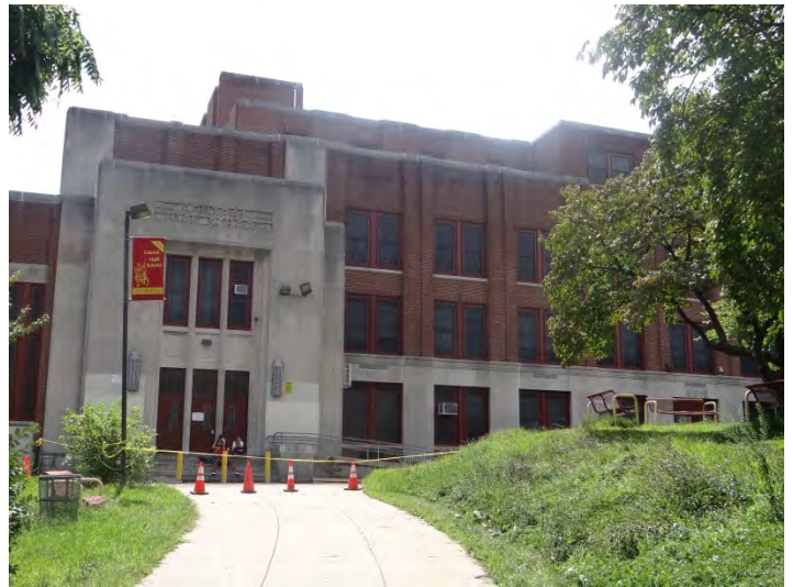
Photo 2: Looking S at N facade
