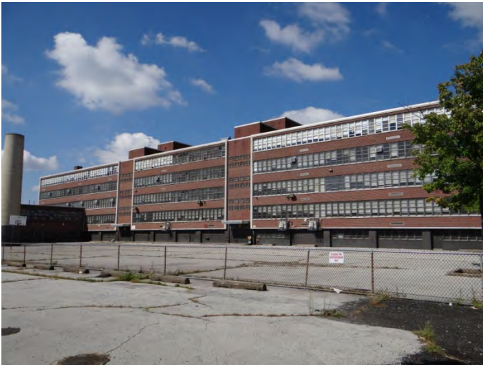
Photo 3: Looking SW at E facade
