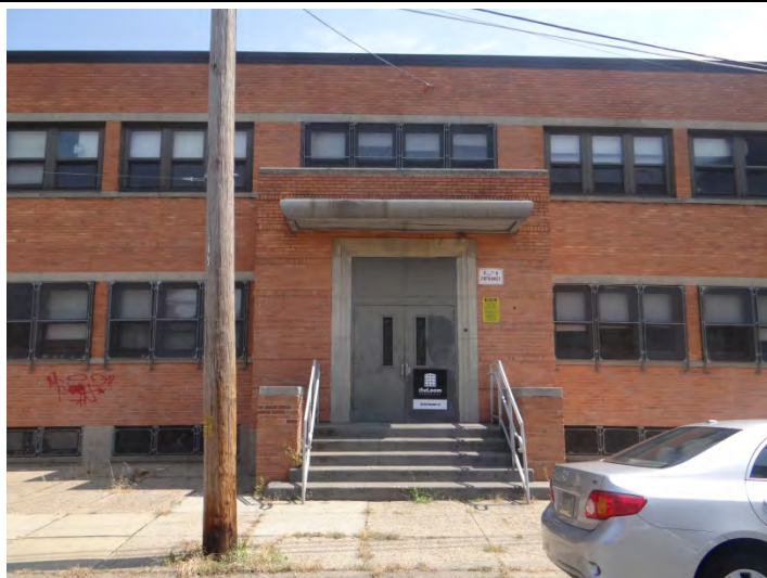
Photo 2: Looking NE at main entrance on main (SW) façade
