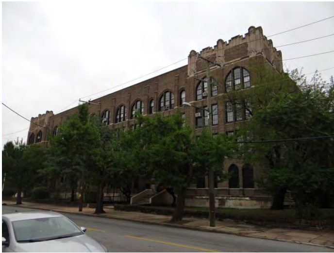
Photo 3: Looking E at W facade
