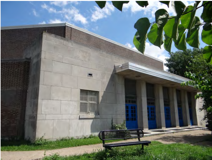
Photo 3: Looking SE at N facade
