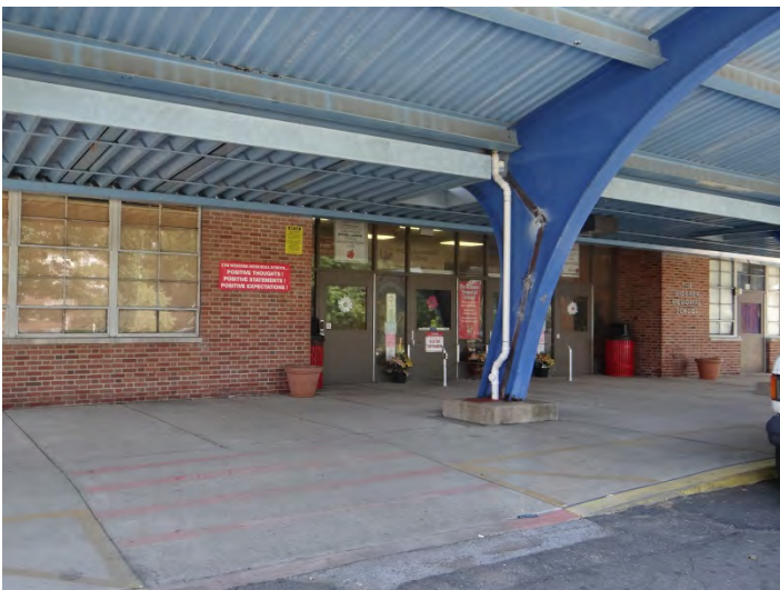
Photo 5: Looking S at main entrance on N façade
