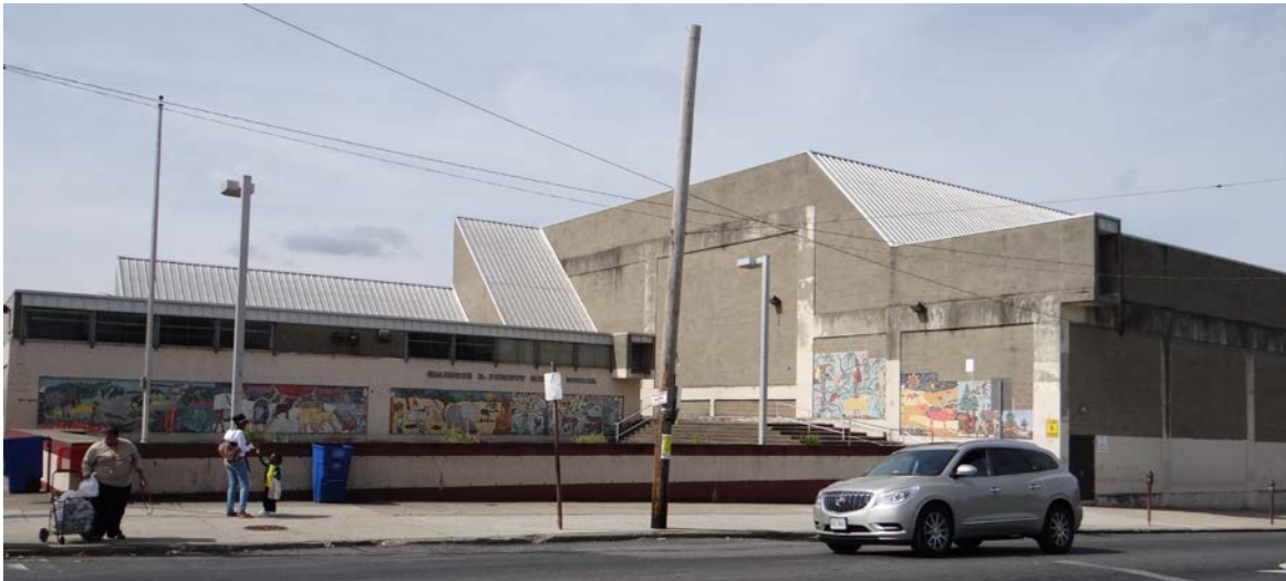
Clarence Pickett Middle School, 1968, a Brutalist design by prominent local firm Geddes, Brecher, Qualls, Cunningham. PA SHPO, 2013.
