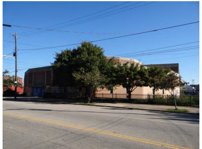
Photo 2: Looking N at S/SE facade
