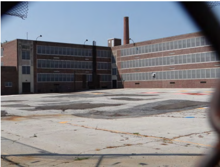
Photo 3: Looking SW at NW facades
