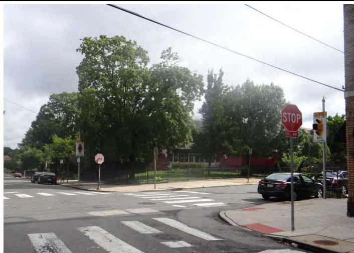
Photo 2: Looking NE at SW facade
