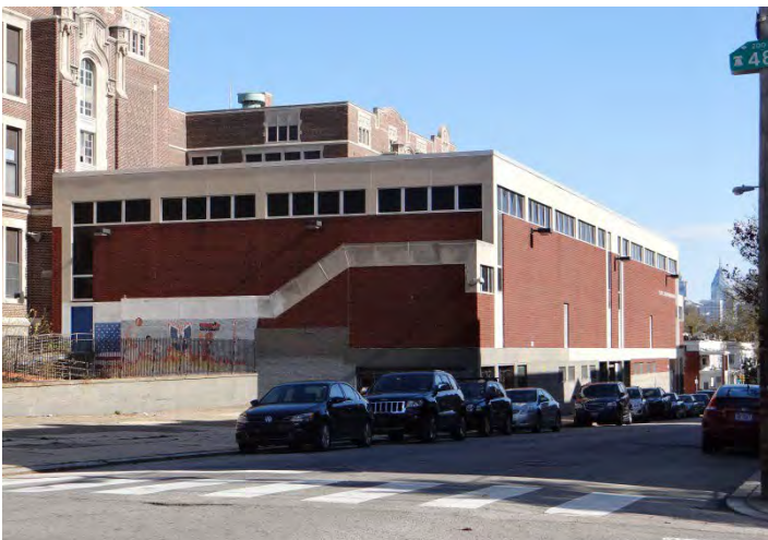
Photo 5: Looking NE at rear gym addition W (left) and S facades
