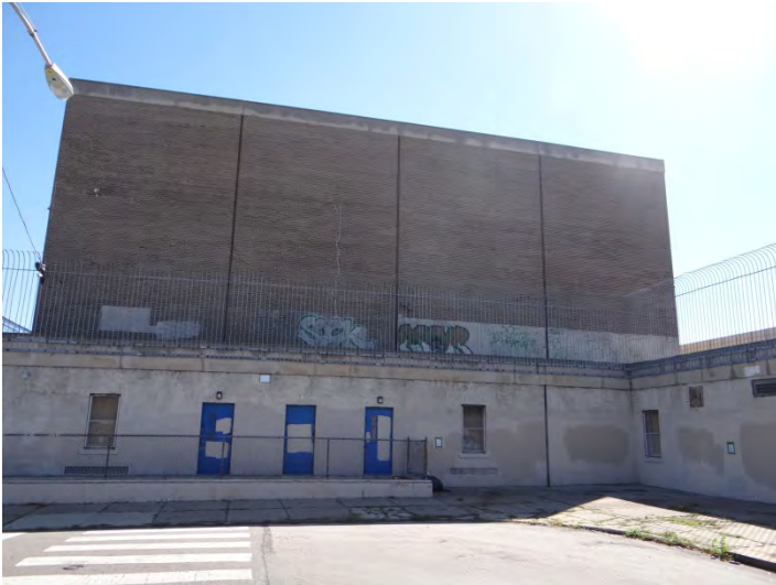
Photo 3: Looking E at W façade
