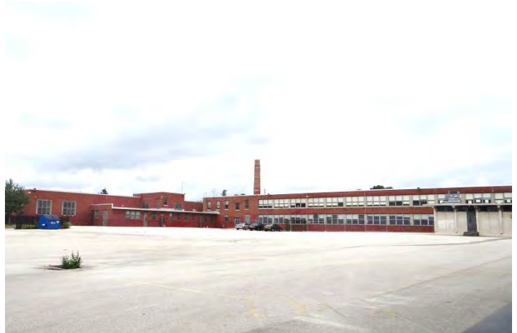
Photo 4: Looking N at rear facades
