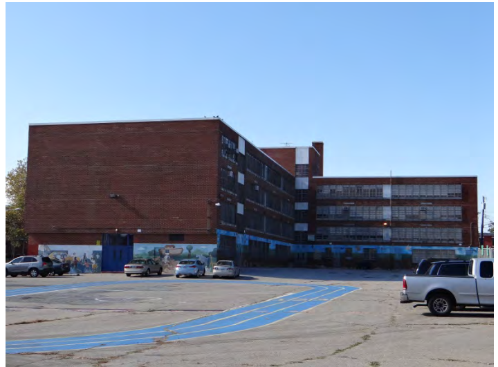
Photo 4: Looking W at E facades
