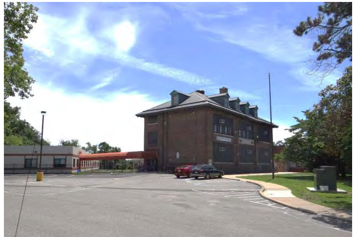
Photo 2: Looking SE at historic school and additions to NE
