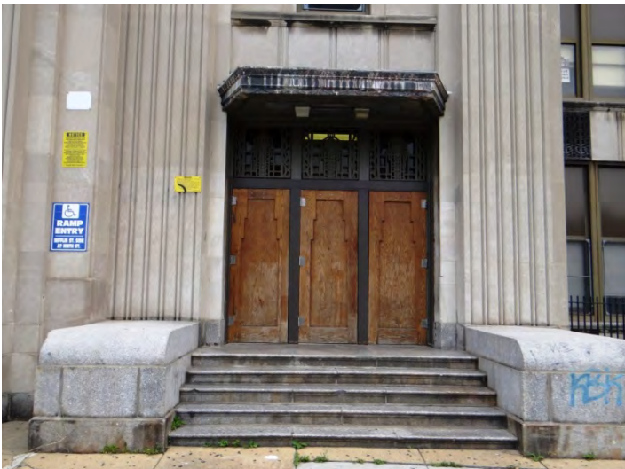
Photo 5: Looking S at E corner of main (N) facade
