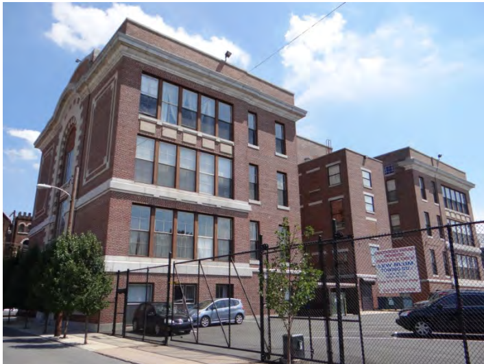
Photo 3: Looking SE at W façade
