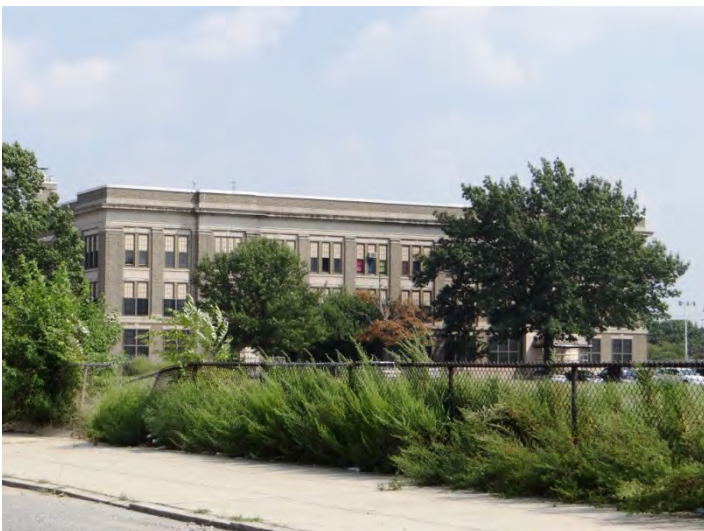
Photo 5: Looking SE at W façade
