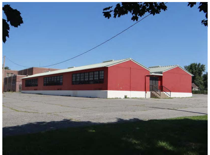
Photo 6: Looking N at rear of property
