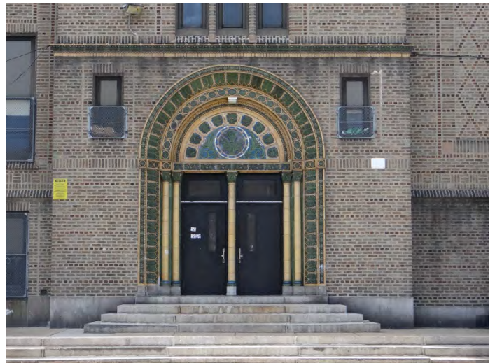
Photo 2: Looking W at entrance on main (E) façade
