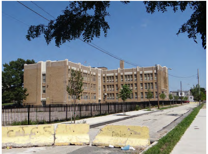
Photo 4: Looking N at SW and SE facades
