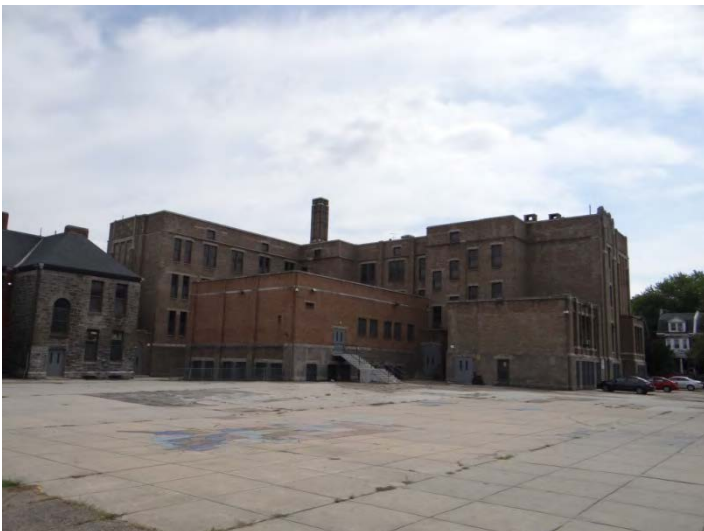
Photo 5: Looking E at rear SE (right) and SW facades
