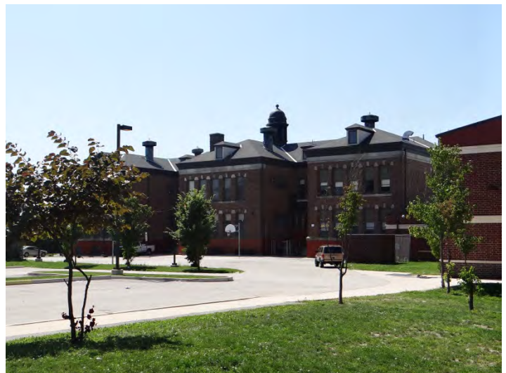
Photo 6: Looking S at rear (NE) facade
