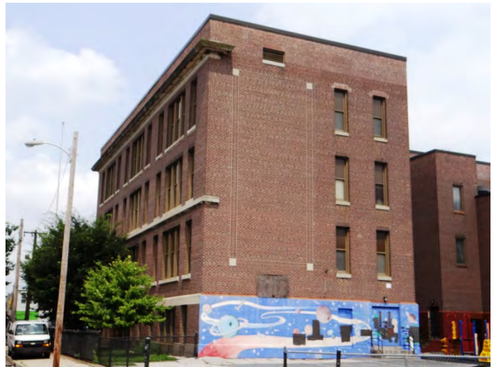
Photo 2: Looking NE at W (left) and rear (S) facades
