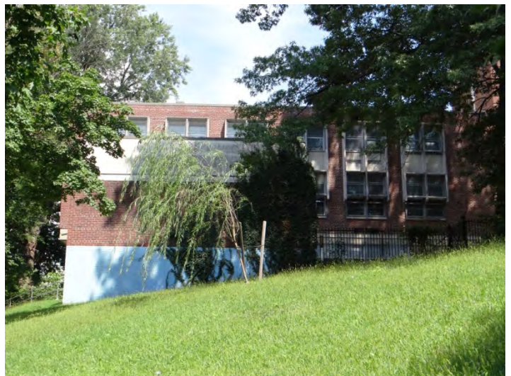
Photo 6: Looking NE at SW facade
