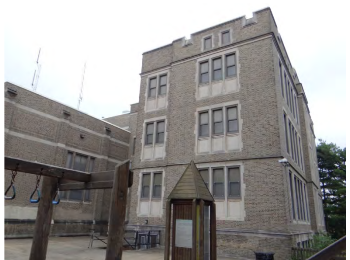
Photo 6: Looking SE at S end of rear (NW) facade
