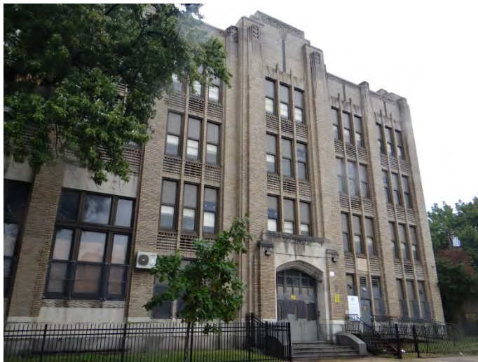
Photo 3: Looking W at E façade
