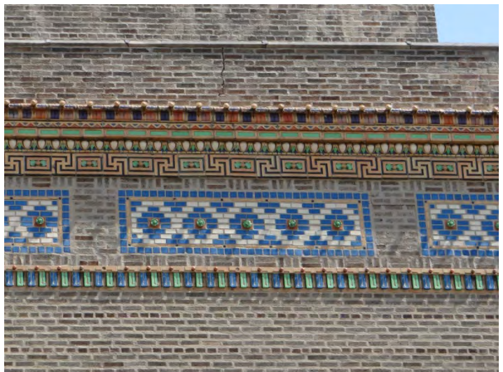
Photo 6: Detail, terra cotta cornice
