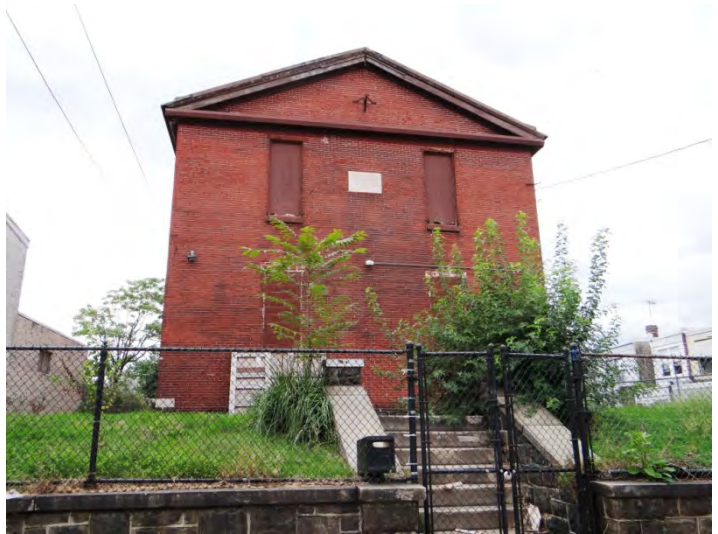
Photo 2: Looking SW at main (NE) facade
