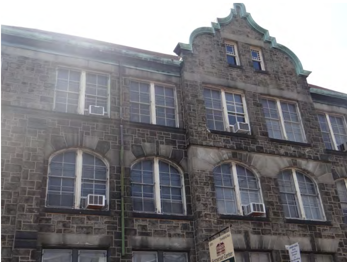
Photo 5: Looking S at wood windows on NW façade
