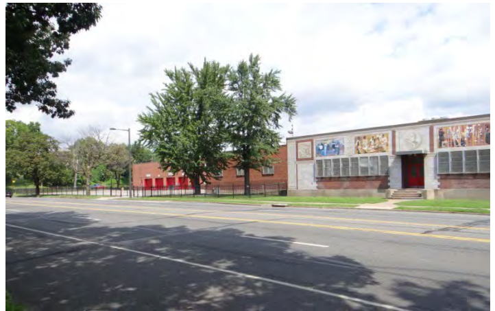
Photo 2: Looking NE at N end of main (W) facade
