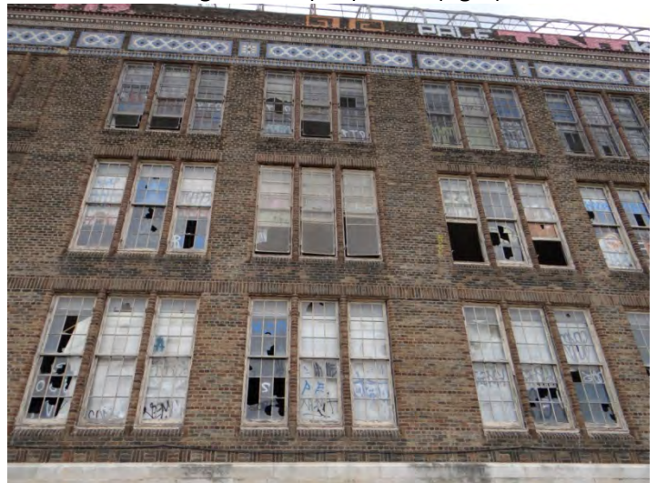
Photo 6: Detail, looking S at original windows on N facade
