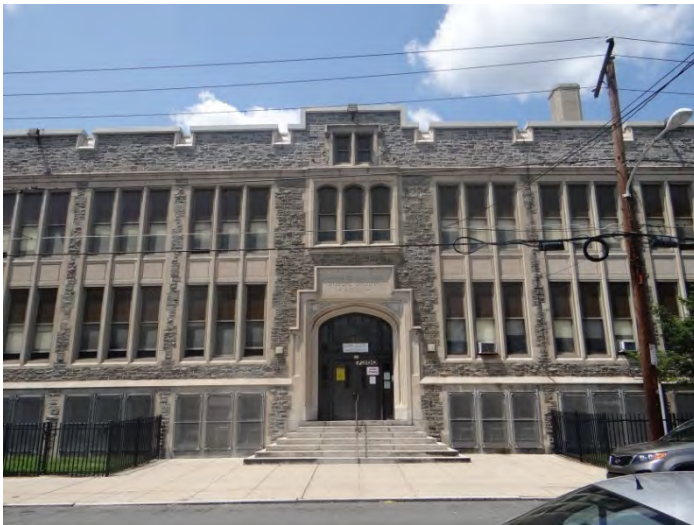
Photo 3: Looking NW at main (SE) facade
