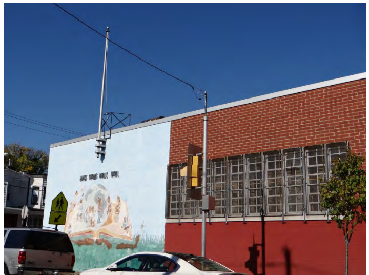
Photo 2: Looking NW at main (S) facade
