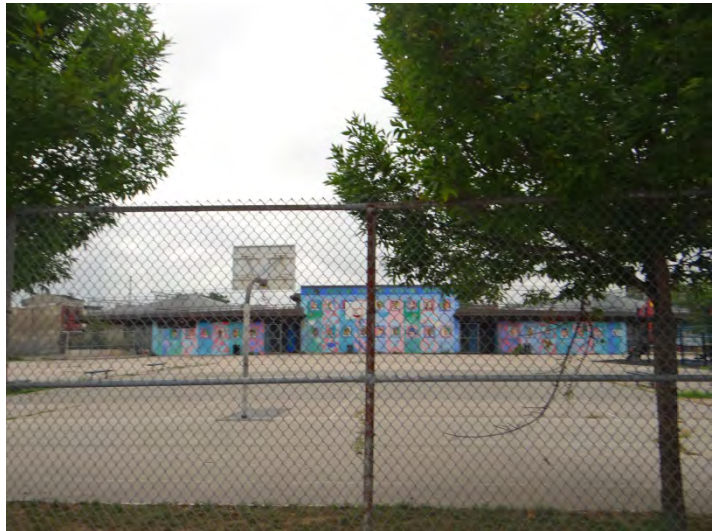
Photo 4: Looking S at N façade
