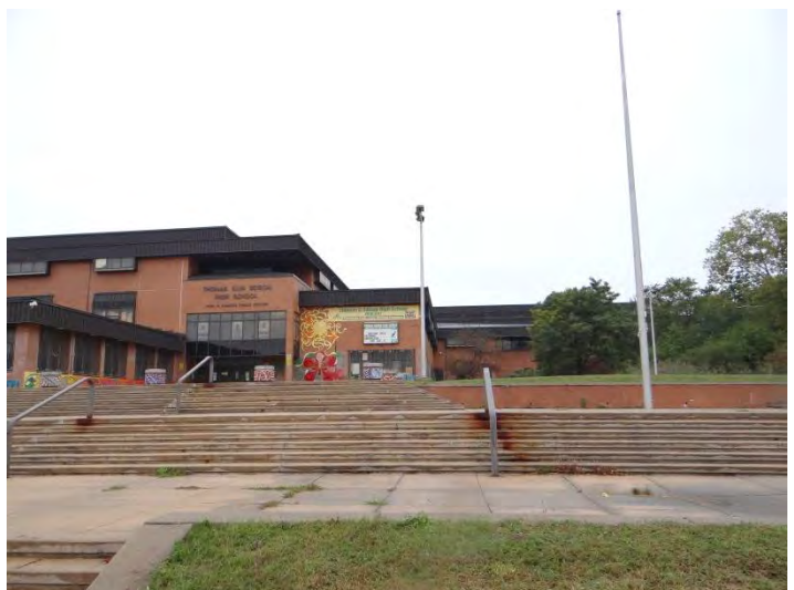
Photo 6: Looking N at S facade
