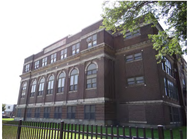
Photo 4: Looking E at N facade
