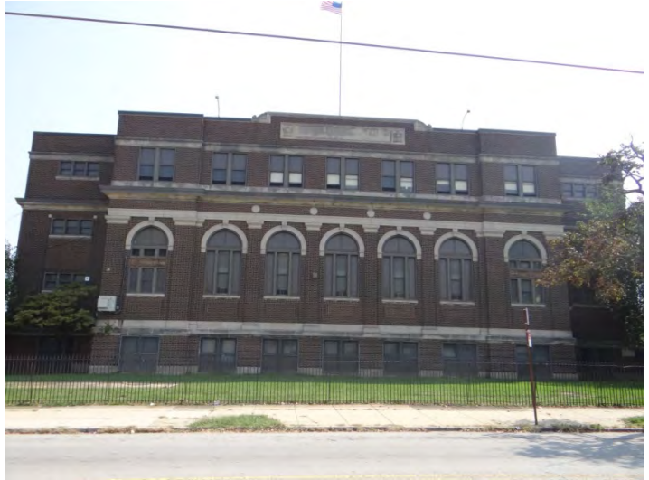
Photo 2: Looking SE at NW façade
