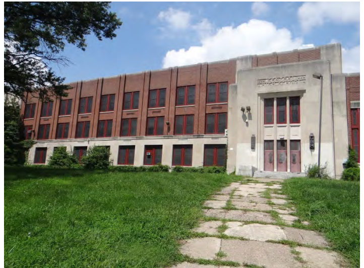
Photo 4: Looking N at S facade
