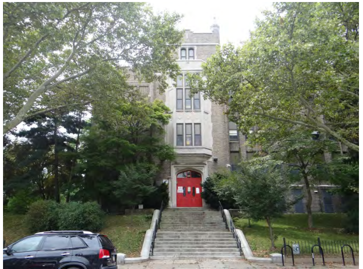
Photo 2: Looking SW at entrance at E end of NE facade
