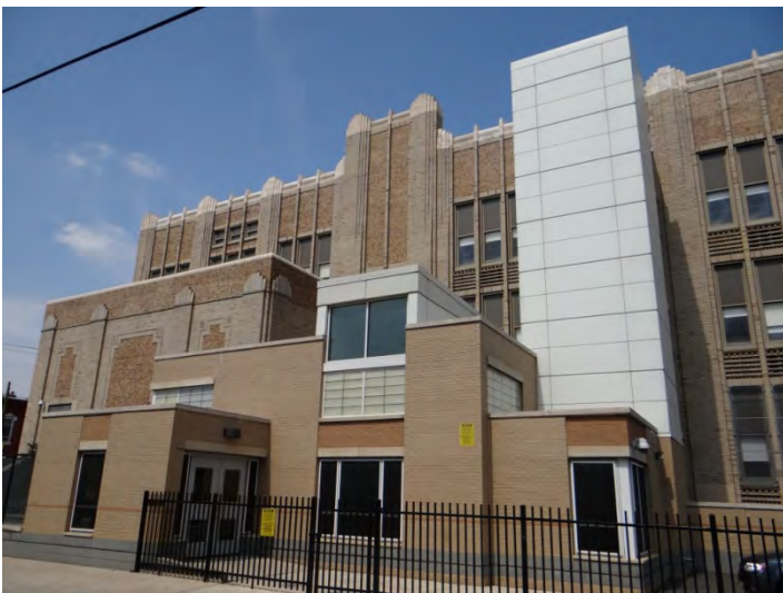
Photo 5: Looking N at S façade
