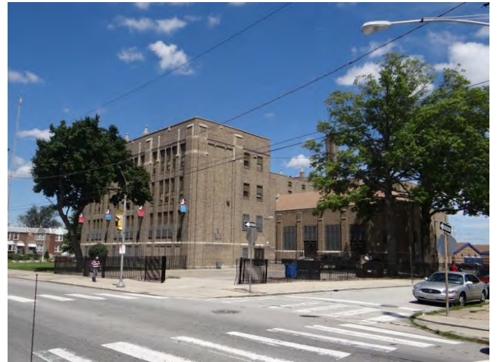
Photo 4: Looking N at SW (left) and rear (SE, right) facades
