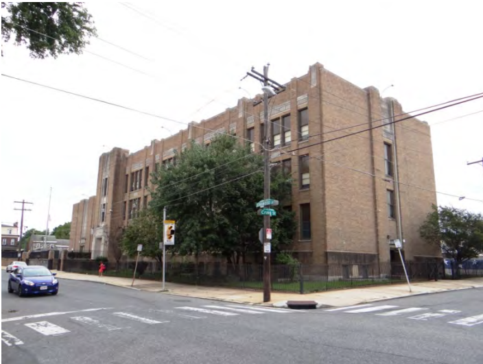
Photo 3: Looking S at main (NE, left) and NW facades
