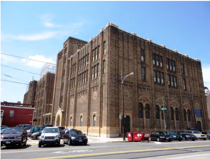
Photo 3: Looking NW at E (right) and S (left) facades
