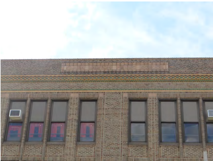
Photo 3: Looking W at nameplate on main (E) façade
