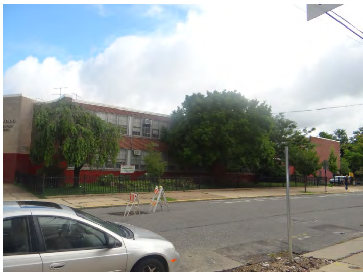
Photo 3: Looking NE at S facade
