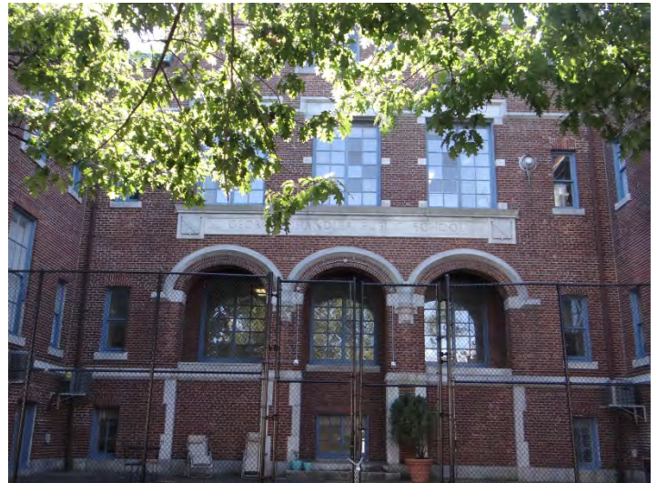
Photo 4: Looking S at center bays of N façade
