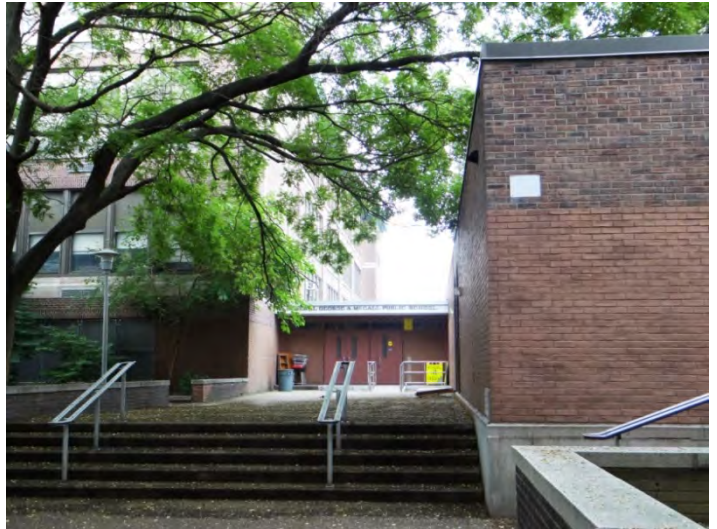
Photo 4: Looking W at addition entrance
