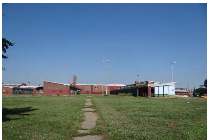
Photo 4: Looking N at easternmost wings on S façade
