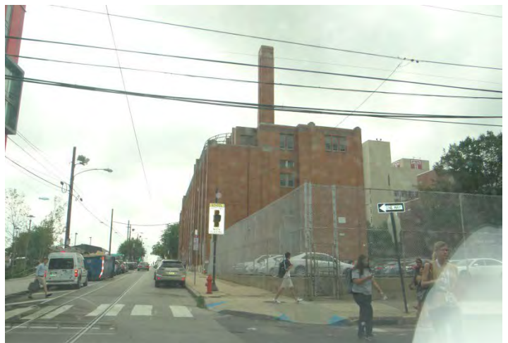
Photo 6: Looking S at N facade
