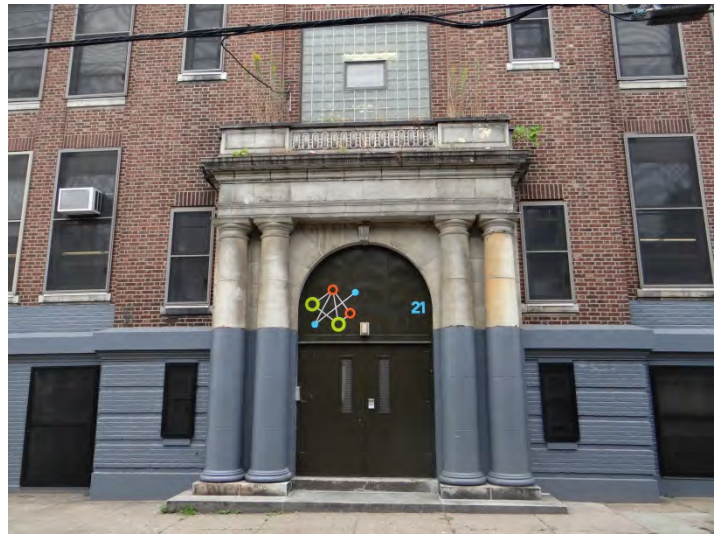
Photo 2: Looking W at E façade entrance
