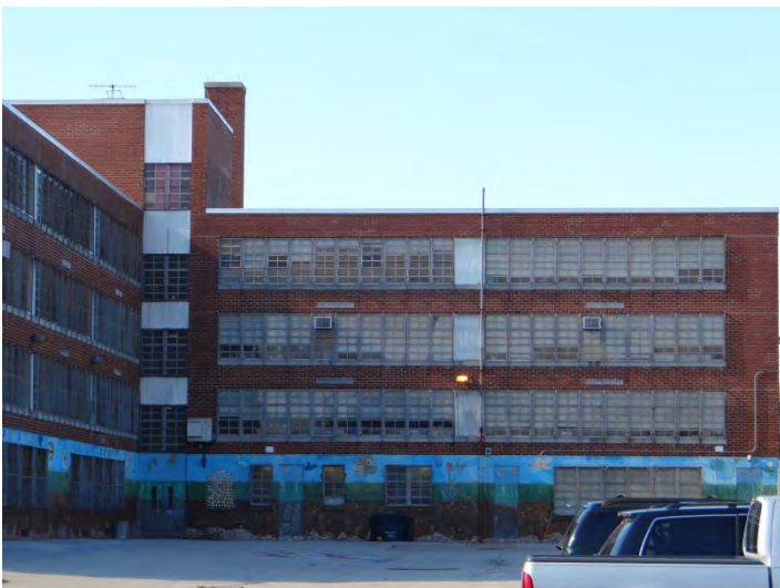
Photo 5: Looking W at E façade
