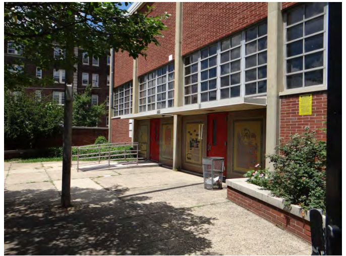
Photo 2: Looking NW at main (S) facade
