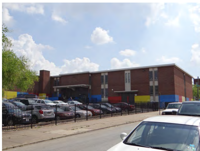
Photo 4: Looking SW at E façade
