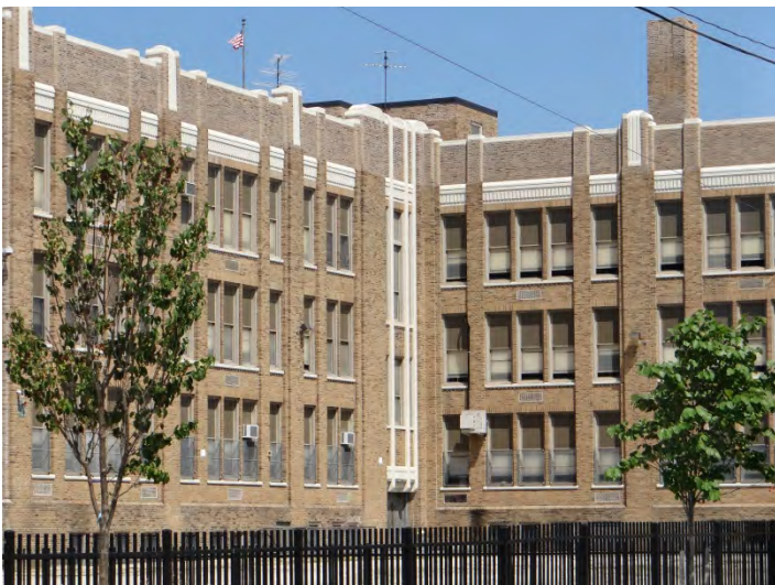
Photo 5: Looking N at SW (right) and SE (left) facades
