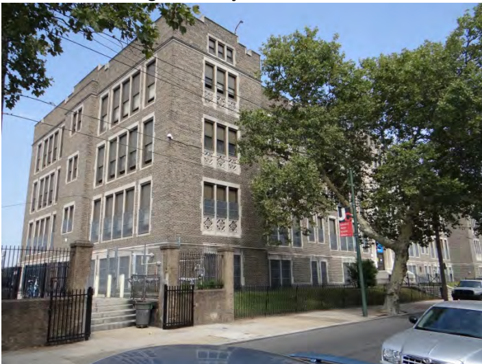
Photo 5: Looking NW at S (left) and E facades
