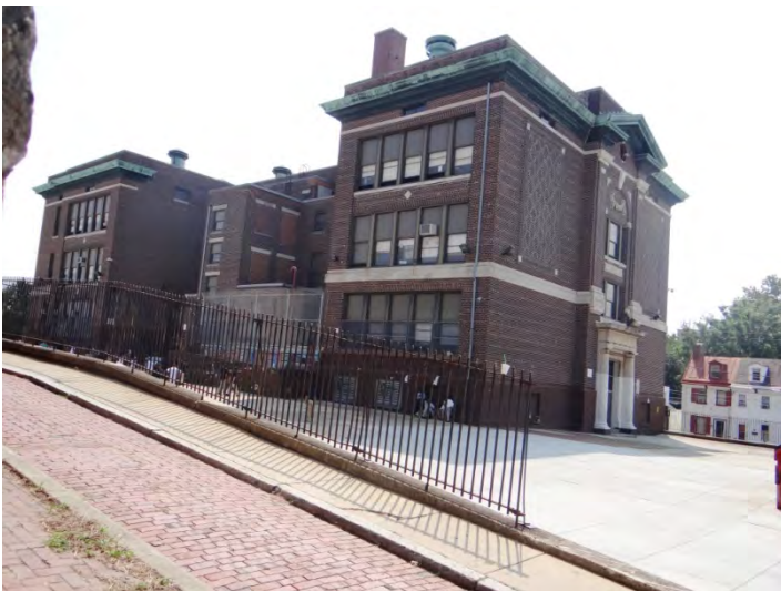
Photo 3: Looking SE at NE (left) and NW (right) facades
