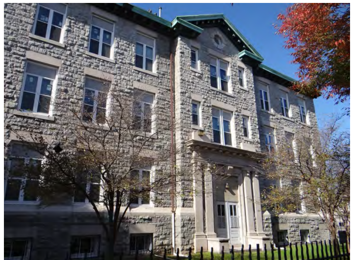
Photo 6: Looking N at E facade
