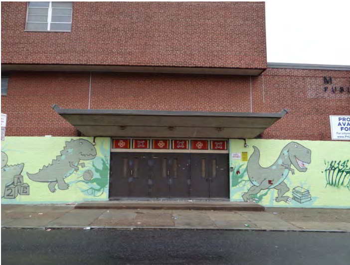
Photo 3: Looking E at main entrance on W facade
