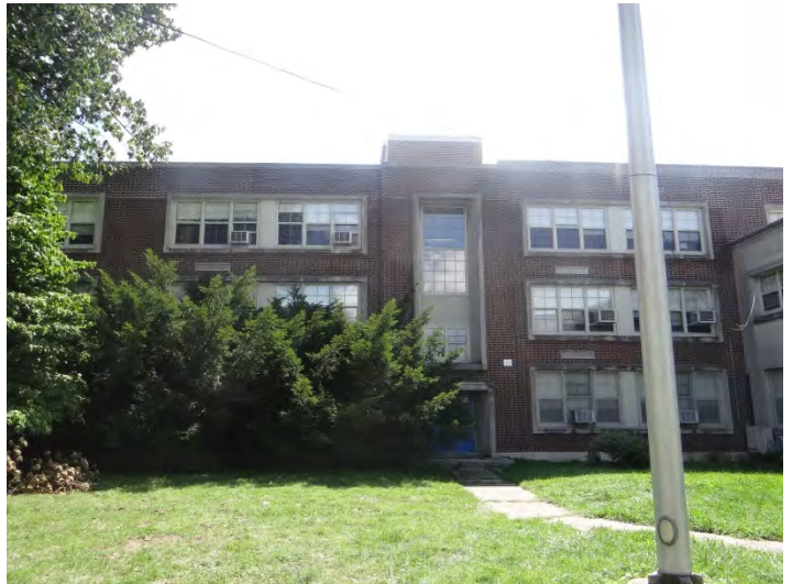
Photo 4: Looking S at E end of N facade
