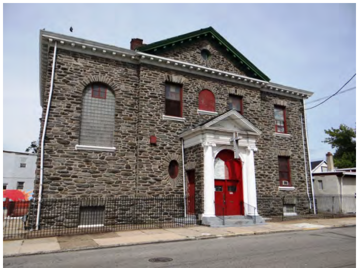
Photo 2: Looking NW at SE facade
