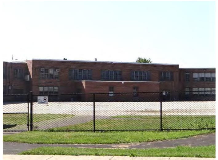
Photo 4: Looking S at rear (N) facade
