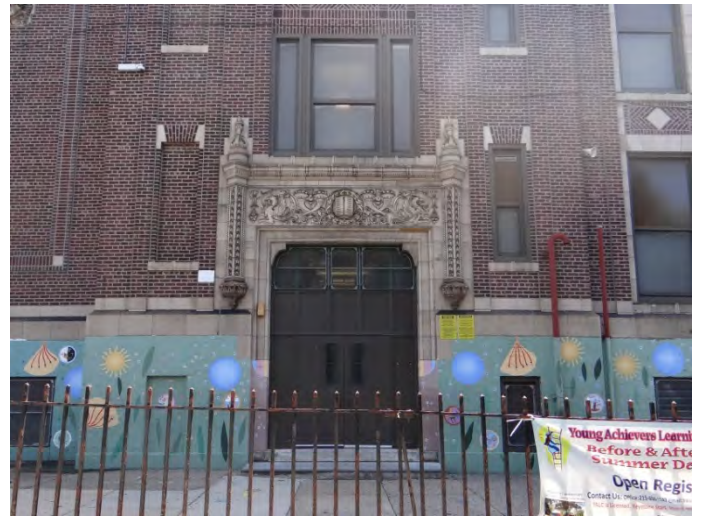
Photo 2: Looking E at main entrance on W façade
