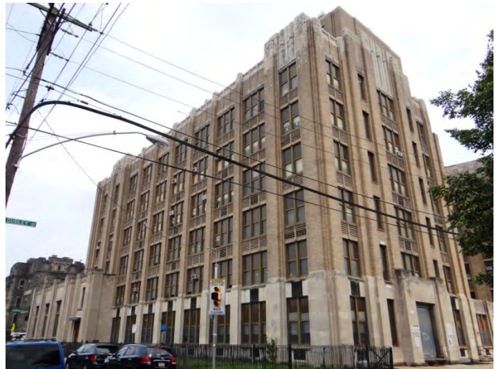
Photo 2: Looking NE at W (left) and rear (S, right) facades
