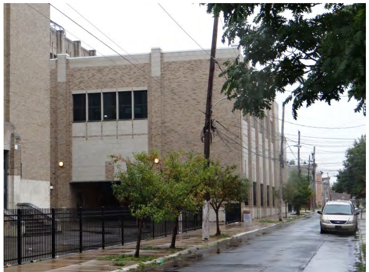
Photo 6: Looking NE at rear (S) façade addition
