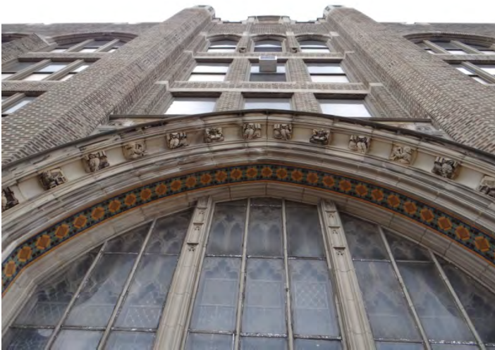
Photo 3: Detail, looking W at E façade entrance surround
