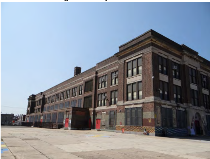
Photo 5: Looking SW at E (left) and N (right) facades
