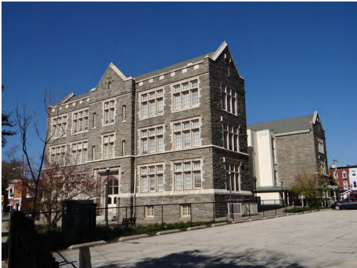
Photo 3: Looking NW at S (left) and E (right) facades
