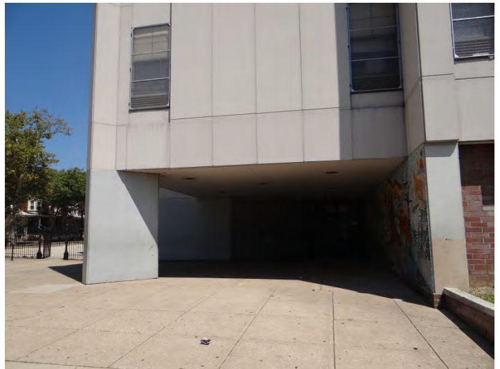
Photo 4: Looking NE at entrance at NW corner of building
