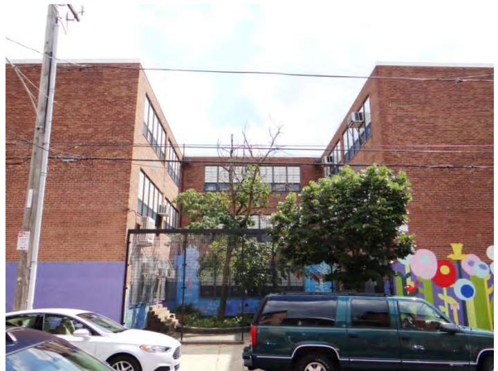
Photo 2: Looking S at W end of N façade
