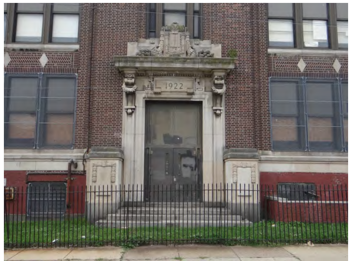
Photo 2: Looking SW at entrance on main (NE) facade
