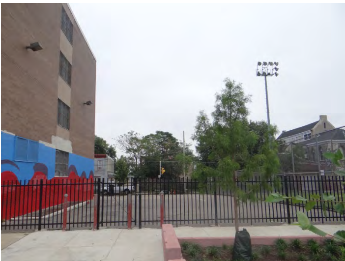
Photo 5: Looking E along S façade
