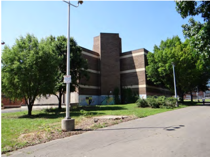
Photo 3: Looking S at N facade
