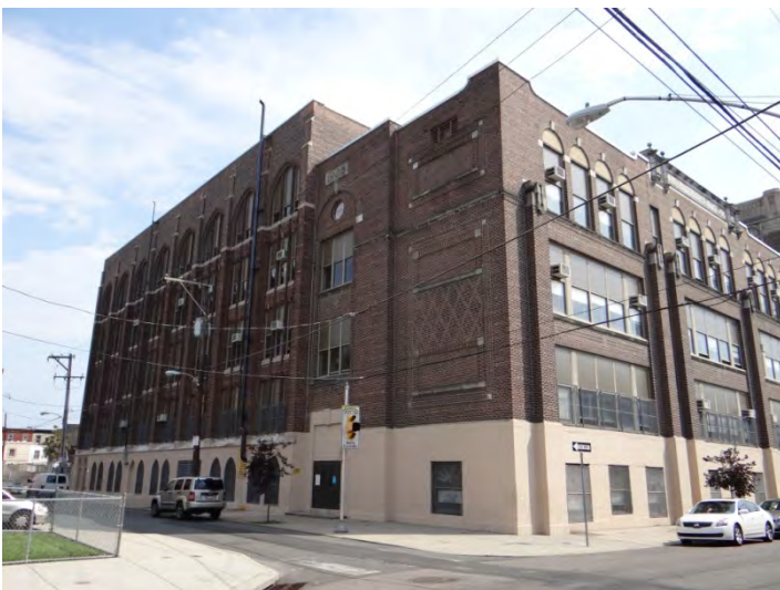
Photo 5: Looking SW at E (left) and N facades
