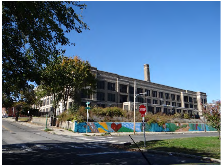
Photo 4: Looking NW at rear (E) facade
