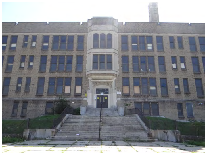
Photo 2: Looking SE at main (NW) facade
