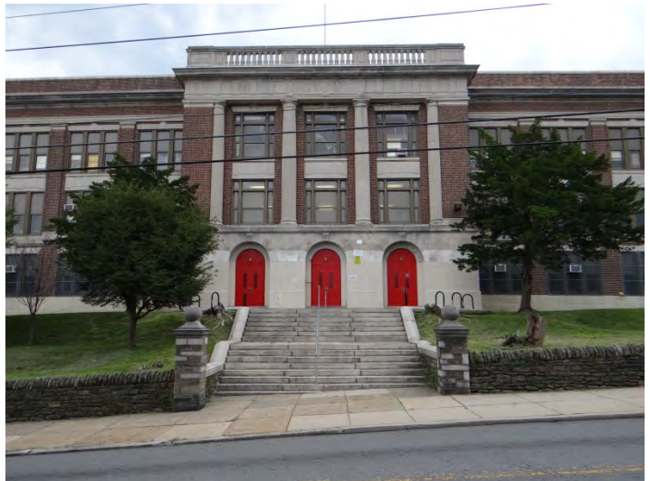
Photo 2: Looking SE at main (NW) facade
