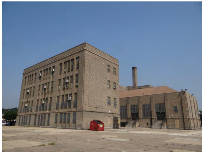
Photo 4: Looking N at S facades
