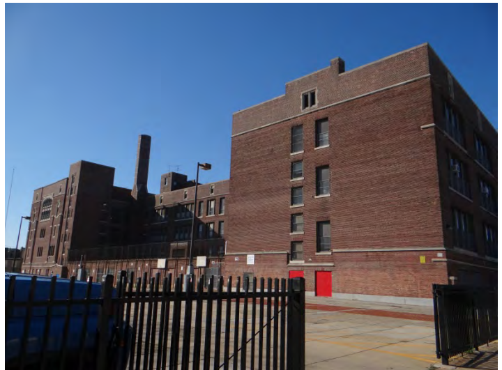
Photo 6: Looking S at rear (NE) façade
