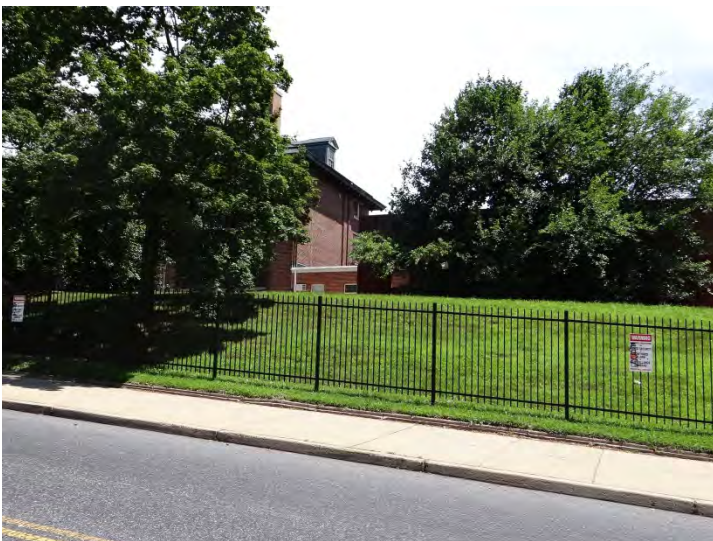
Photo 5: Looking S at NW façade of addition to SW
