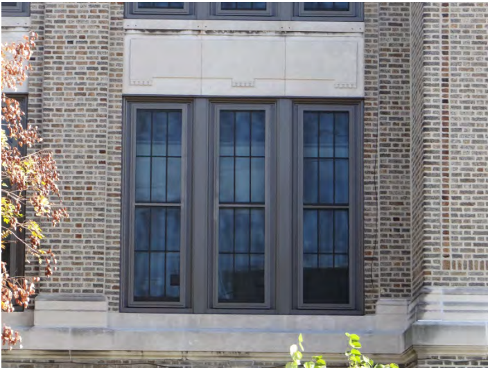
Photo 3: Looking E at main (W) façade, typical window bay
