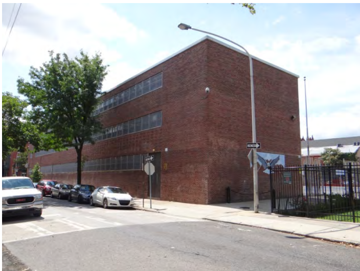
Photo 5: Looking SW at N (center) and E (left) facades
