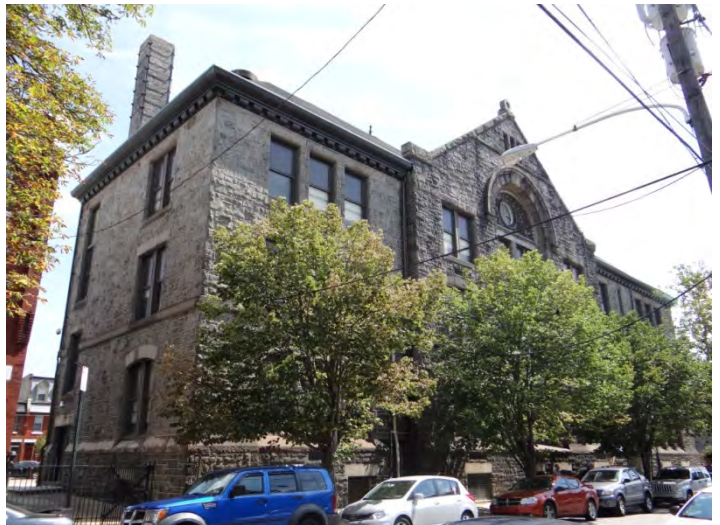
Photo 2: Looking S at N (left) and W facades
