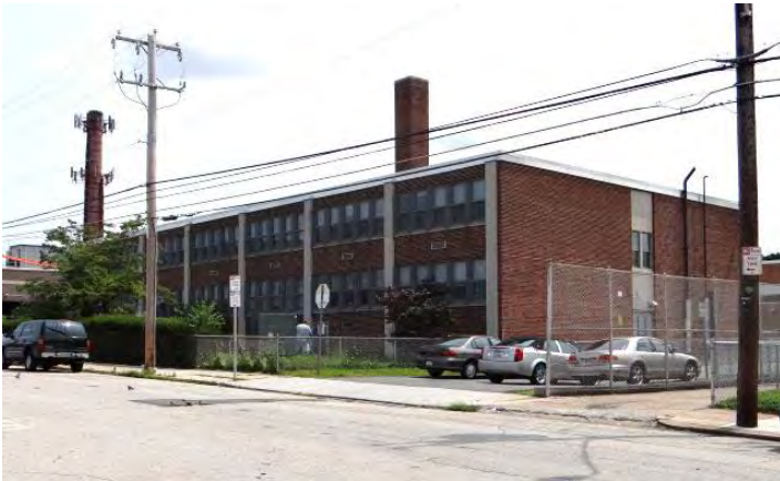
Photo 3: Looking NE at main (N) facade
