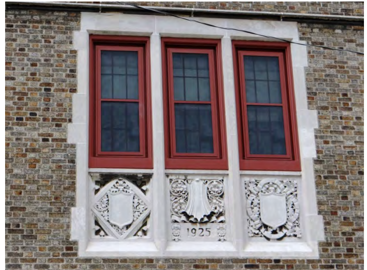
Photo 4: Looking S at main (N) facade
