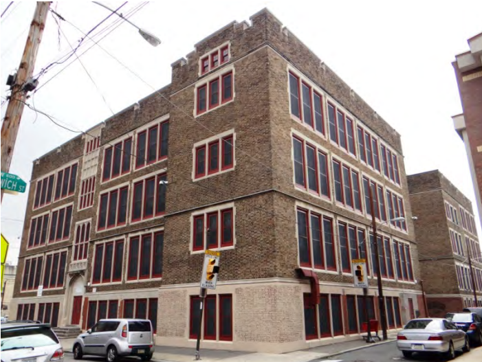
Photo 5: Looking NE at W (left) and S (right) facades
