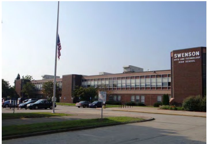
Photo 2: Looking S at S end of main (NE) facade
