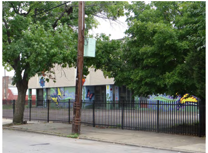
Photo 6: Looking SW at E façade
