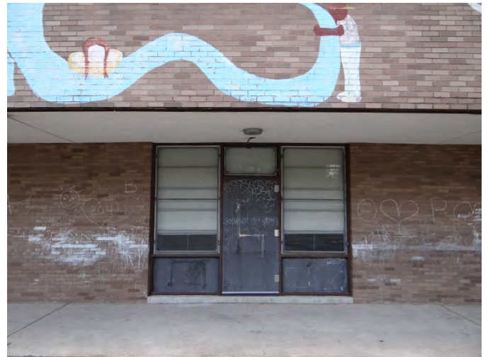
Photo 6: Looking SW at NE façade entrance
