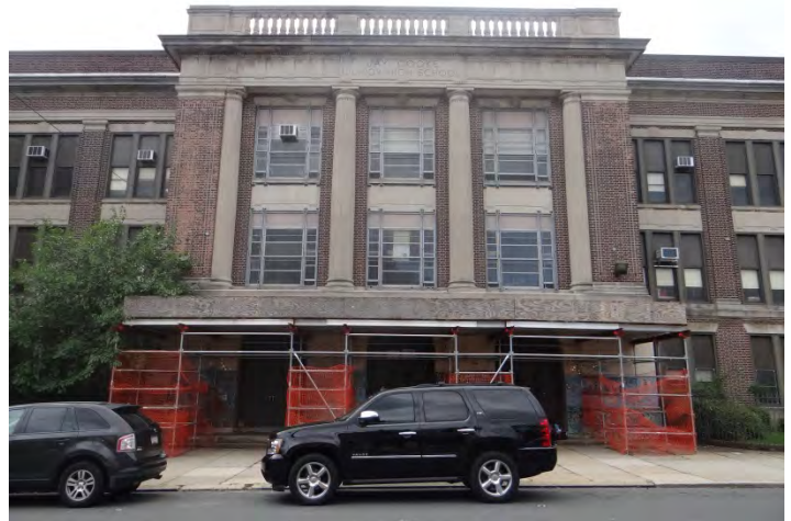
Photo 2: Looking S at main entrance on N facade
