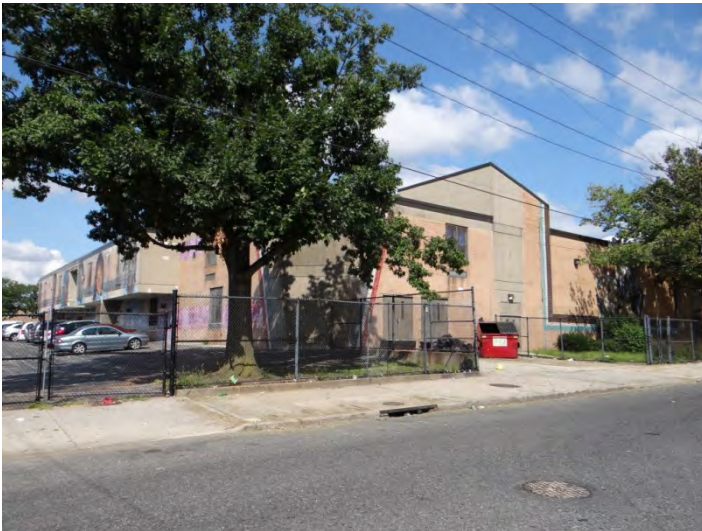
Photo 3: Looking NW at E (right) and rear (S, left) facade
