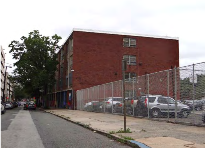
Photo 5: Looking S at N facade
