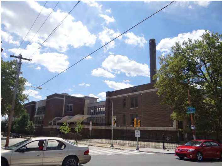
Photo 3: Looking SE at NE façade
