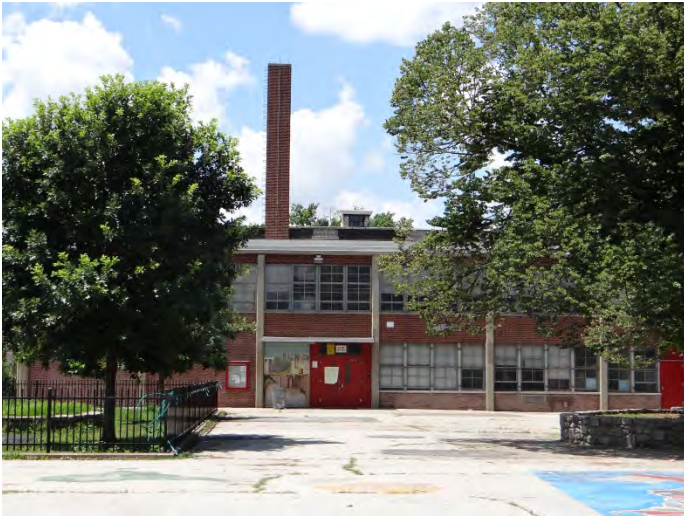
Photo 3: Looking W at E facade
