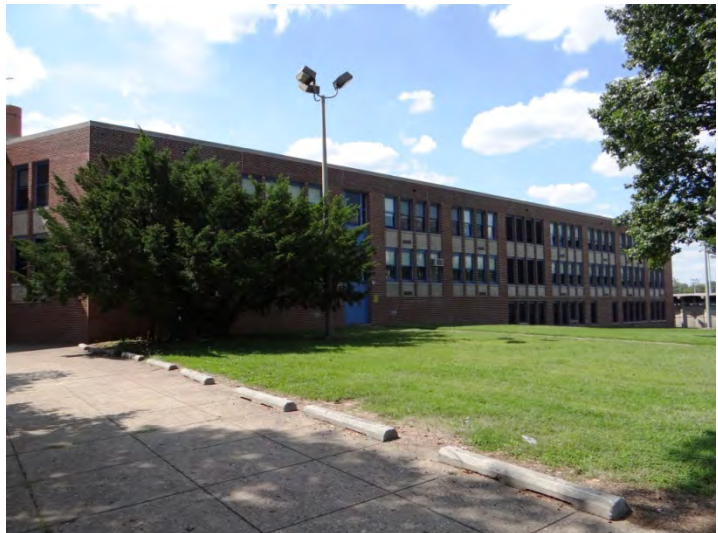
Photo 4: Looking N at E facade
