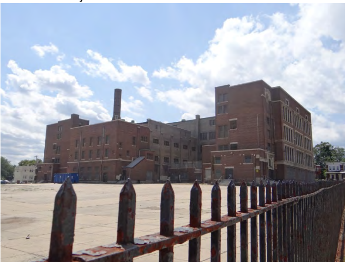
Photo 5: Looking SW at rear (E) façade
