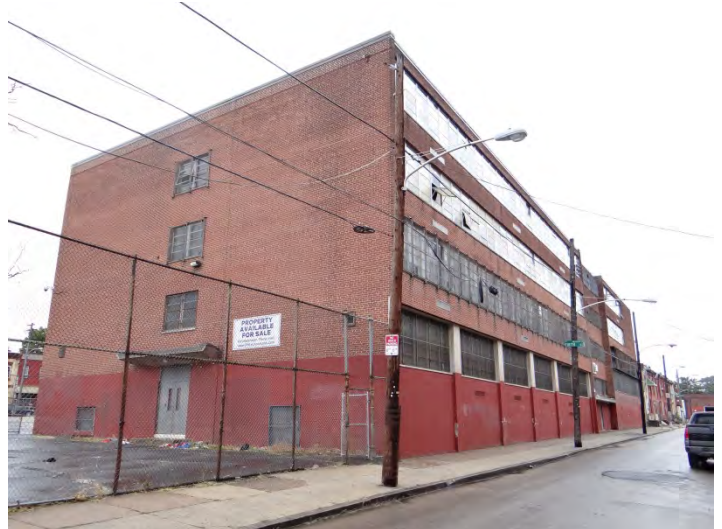
Photo 6: Looking NW at S (left) and E (right) facades
