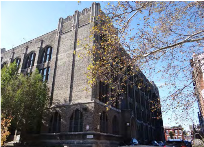
Photo 5: Looking W at N facade
