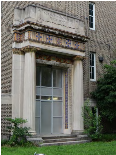
Photo 3: Looking NE at former main entrance on S facade
