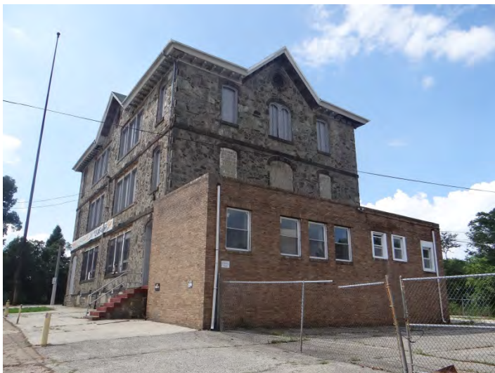
Photo 5: Looking SW at E (center) and N facades
