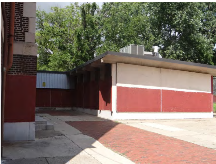
Photo 5: Looking W at addition on N facade
