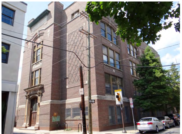
Photo 6: Looking NW at S (left) and E facades
