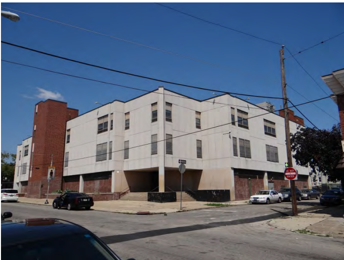
Photo 5: Looking N at SW (left) and SE (right) facades
