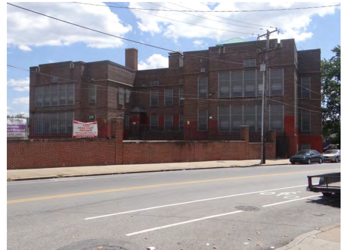
Photo 6: Looking SE at rear (N) facade
