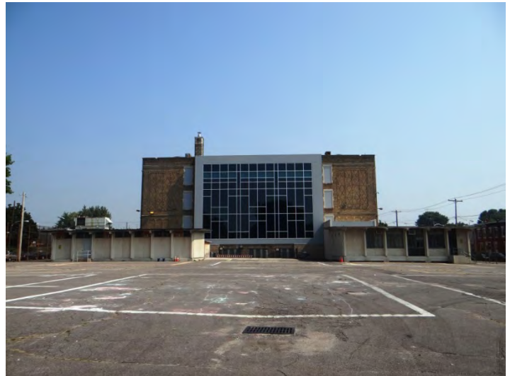
Photo 4: Looking NE at SW façade
