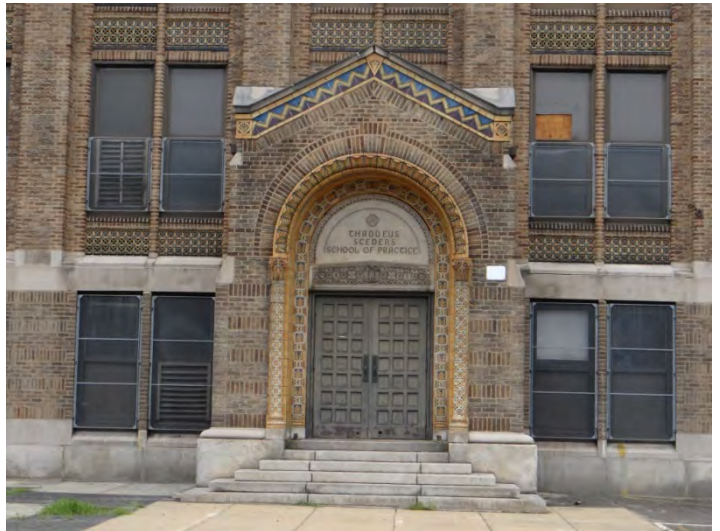
Photo 4: Detail, looking N at entrance on main (S) façade
