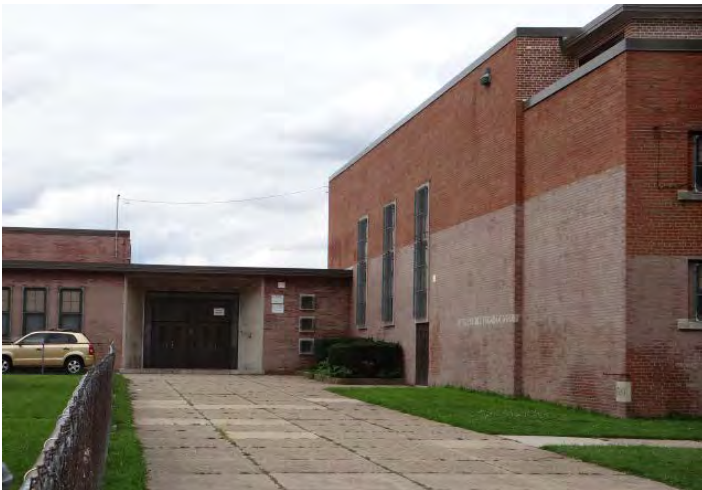
Photo 3: Looking NW at main entrance on main (S) facade
