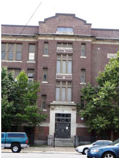
Photo 5: Looking S at E corner of main (N) façade
