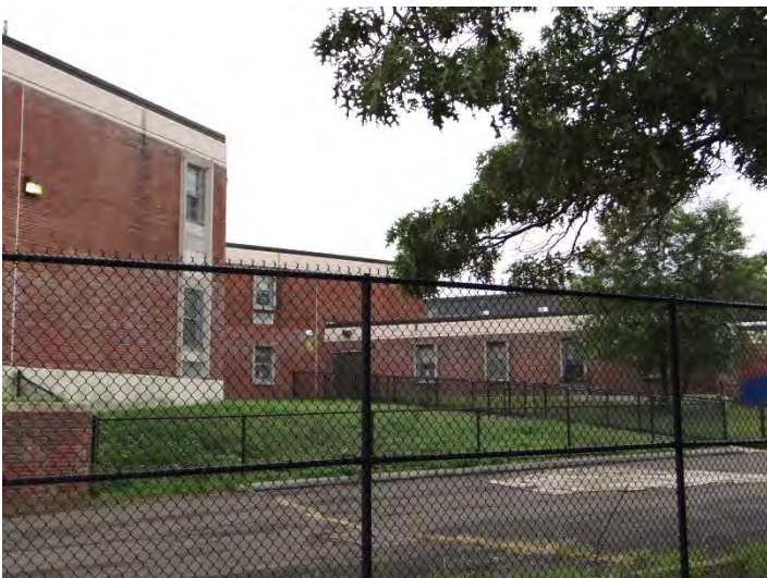
Photo 5: Looking S at W end of N facade
