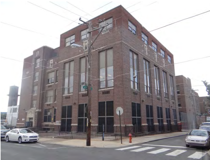
Photo 3: Looking SE at N (left) and W (right) facades
