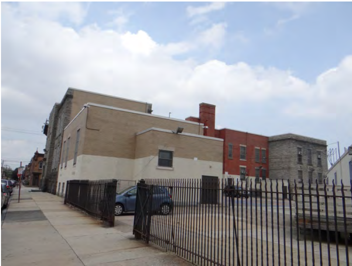
Photo 3: Looking N at S façade
