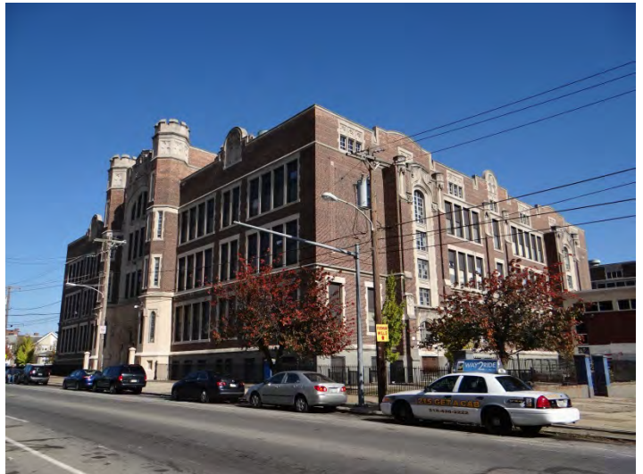
Photo 4: Looking NE at W (left) and S (right) facade
