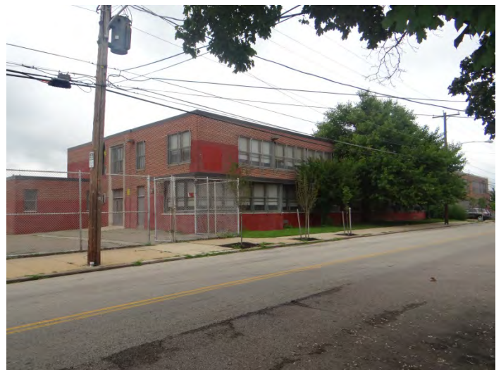
Photo 4: Looking N at SW (left) and SE (right) facades
