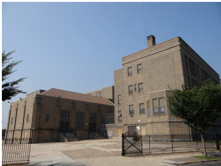
Photo 6: Looking SW at E facades
