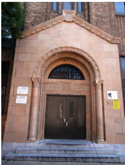
Photo 5: Looking N at S façade entrance at E end
