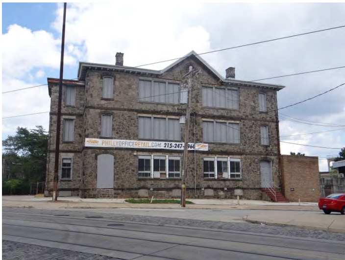
Photo 3: Looking N at S façade
