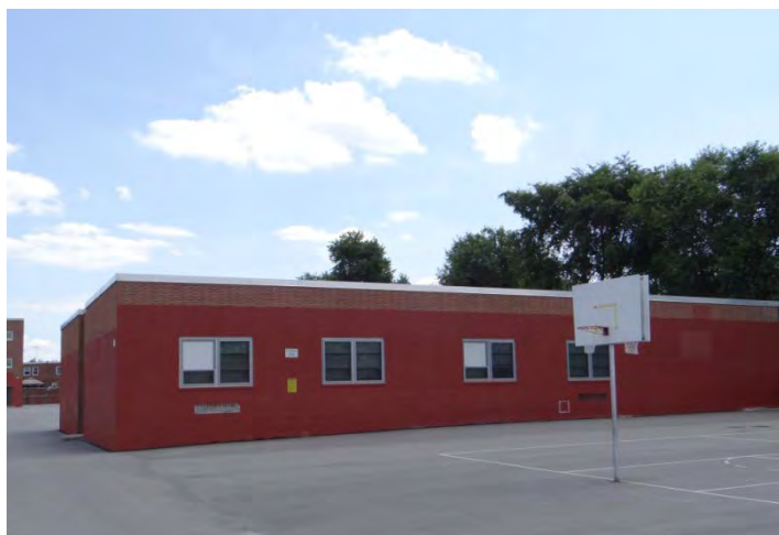
Photo 5: Looking SW at NE facade, rear building
