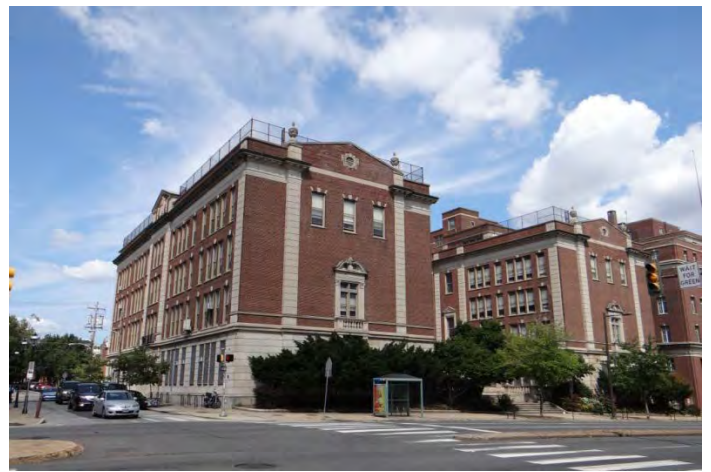
Photo 2: Looking NE at W (left) and S (right) facades
