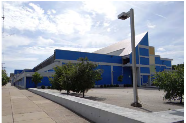
Photo 4: Looking S at NW facade
