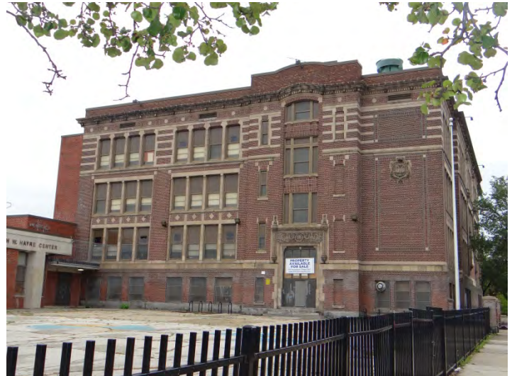
Photo 4: Looking SW at E facade
