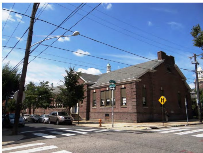
Photo 6: Looking W at S facade
