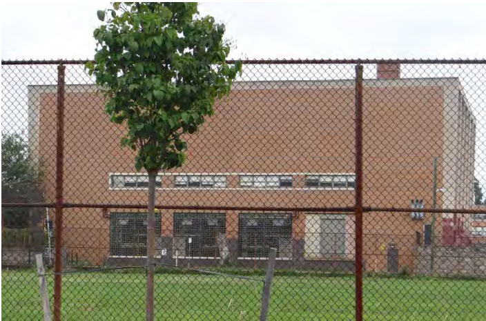
Photo 3: Looking N at S façade
