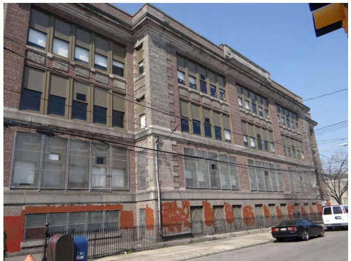
Photo 2: Looking NW at center of NE façade
