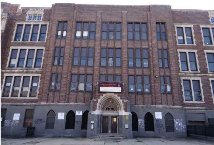
Photo 3: Looking S at 1930s center infill on N facade
