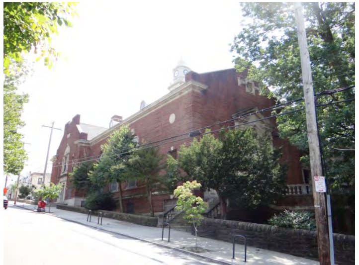
Photo 4: Looking S at NE (left) and NW facades
