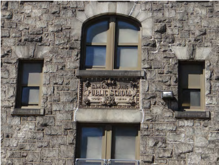
Photo 3: Looking W at nameplate on E façade
