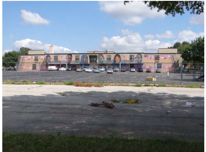
Photo 4: Looking N at rear (S) facade
