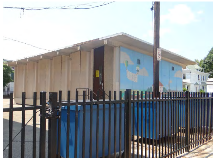
Photo 6: Looking S at portable addition
