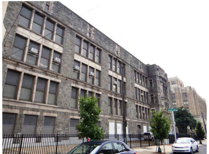
Photo 2: Looking SE at main (W) facade
