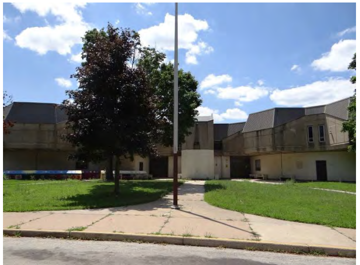
Photo 6: Looking W at NE facade
