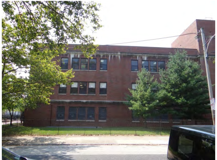
Photo 4: Looking SW at addition NE façade
