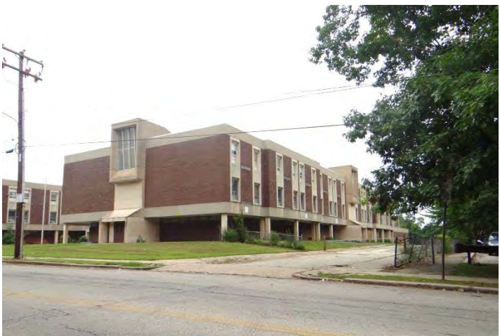
Photo 6: Looking N at main (SW, left) and SE (right) facades
