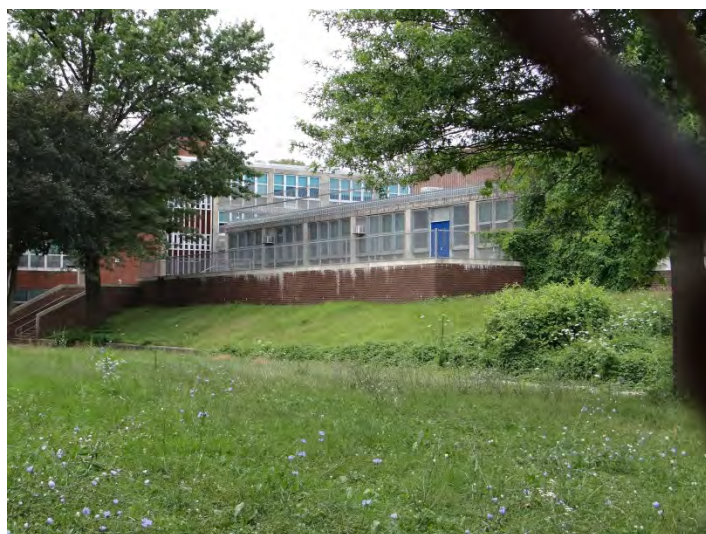
Photo 6: Looking S at N facade
