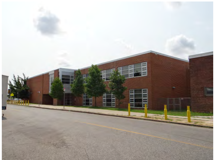
Photo 6: Looking SE at NE facade
