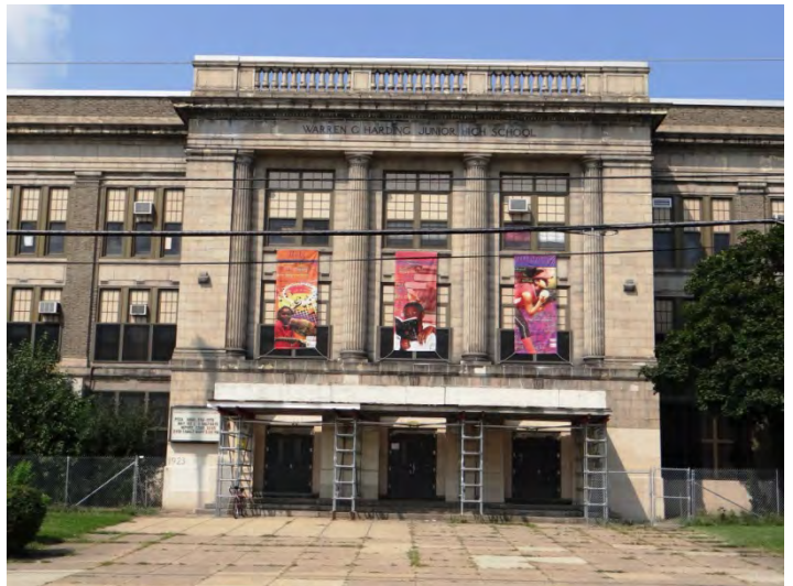
Photo 2: Looking N at main entrance on main (S) façade
