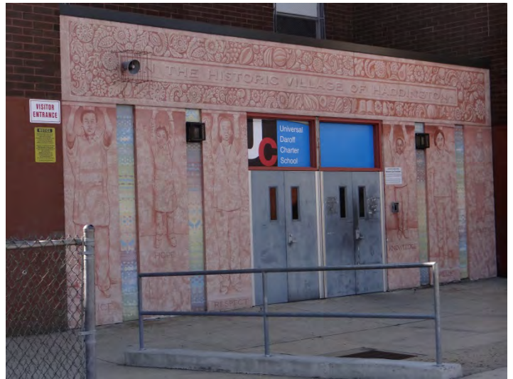
Photo 2: Looking SW at main entrance on main (N) facade
