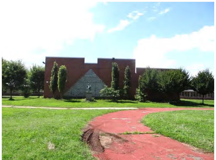
Photo 6: Looking W at E façade
