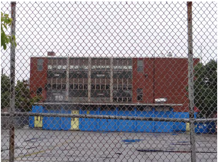
Photo 6: Looking W at E facade
