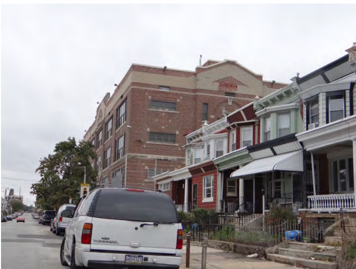
Photo 5: Looking NE at S facade
