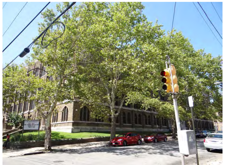
Photo 6: Looking W at SE (left) and NE (right) facades
