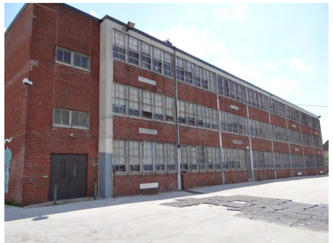
Photo 6: Looking W at N facade
