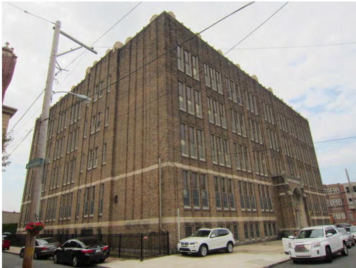
Photo 3: Looking NW at S (left) and E facades
