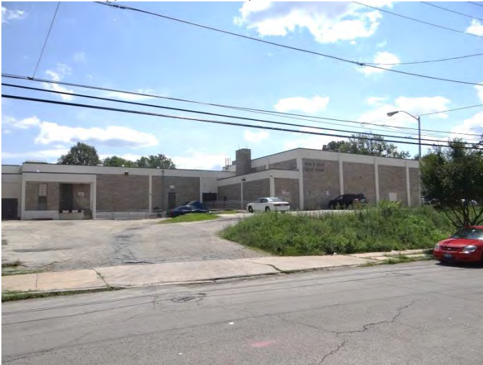
Photo 5: Looking S at NW facade
