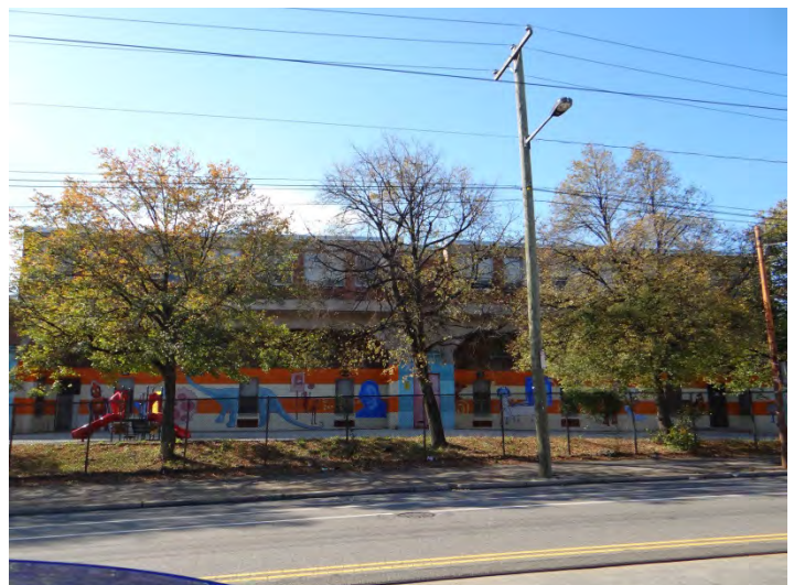
Photo 6: Looking SW at NE facade
