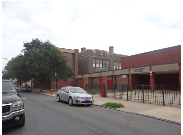
Photo 4: Looking E at NW facade
