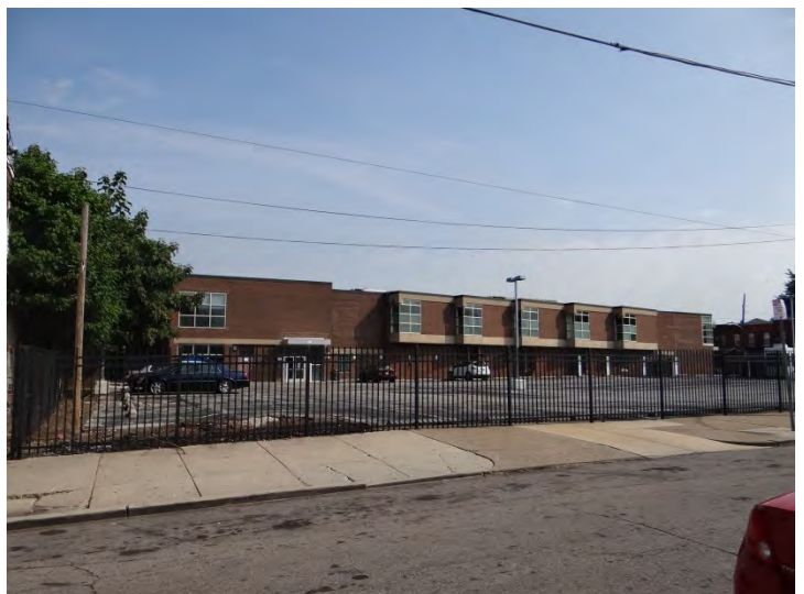
Photo 6: Looking N at S façade
