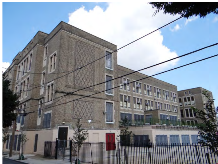
Photo 4: Looking NW at rear (E) facade
