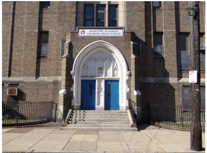
Photo 2: Looking SW at main (NE) facade
