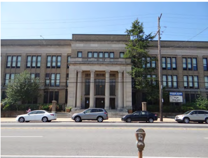
Photo 1: Looking SW at main (NE) facade
