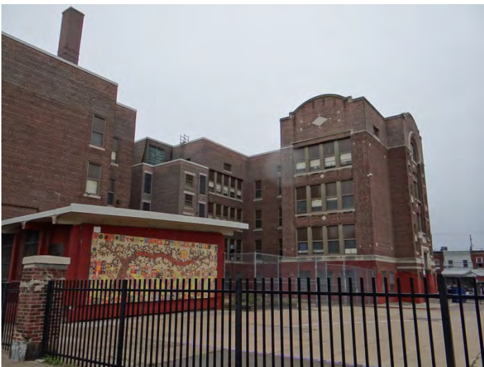
Photo 5: Looking E at W facades
