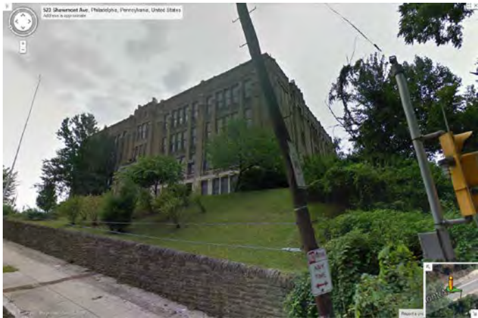
Photo 3: Looking SE at main (NW, left) and SW facades
