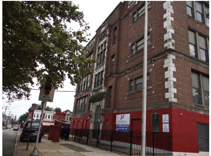
Photo 4: Looking S at N facade
