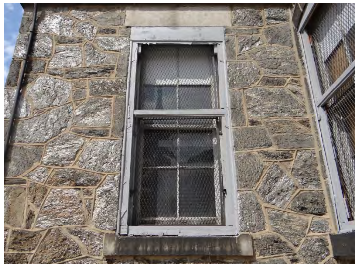
Photo 6: Detail, original wood windows
