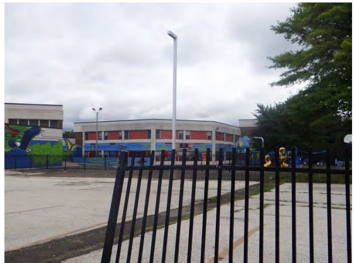
Photo 4: Looking NW at SE facade
