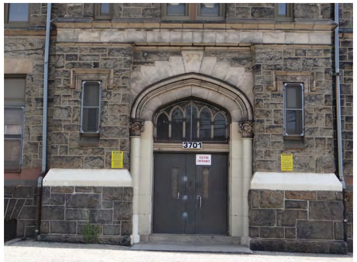
Photo 6: Looking SE at NW façade entrance
