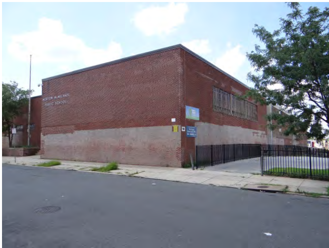
Photo 3: Looking NW at main (S, left) and E (right) facades
