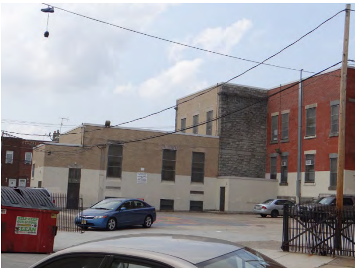
Photo 5: Looking W at S facades
