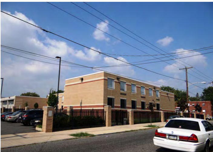
Photo 5: Looking NE at SE end of addition
