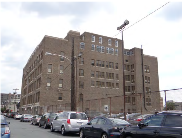
Photo 5: Looking E at W façade
