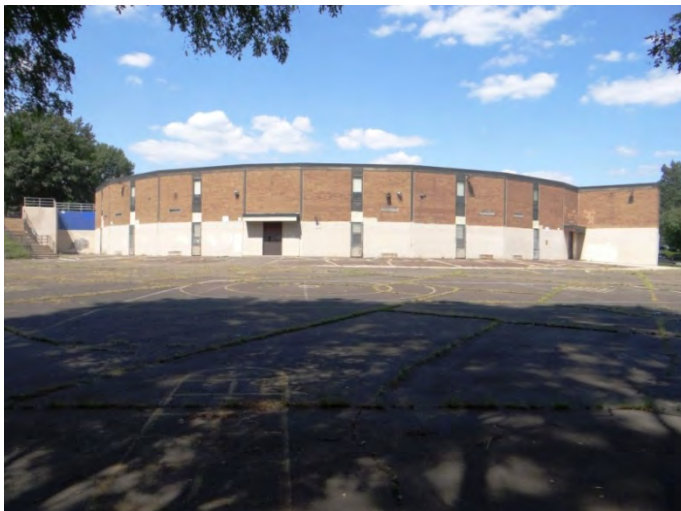
Photo 5: Looking N at S facade
