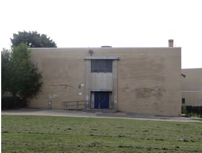
Photo 5: Looking SE at N façade
