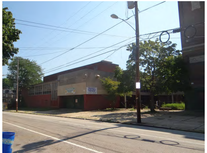
Photo 2: Looking NE at N end of NW facade
