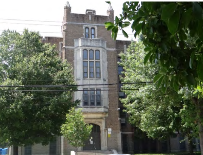
Photo 3: Looking SW at main (NE) facade
