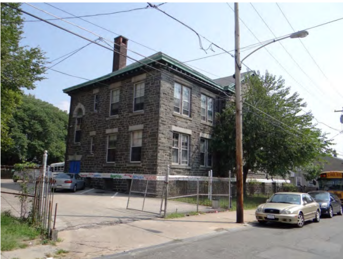
Photo 5: Looking E at NW (left) and SW (right) facades
