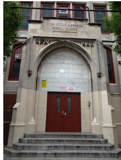
Photo 2: Looking S at main entrance on main (N) facade
