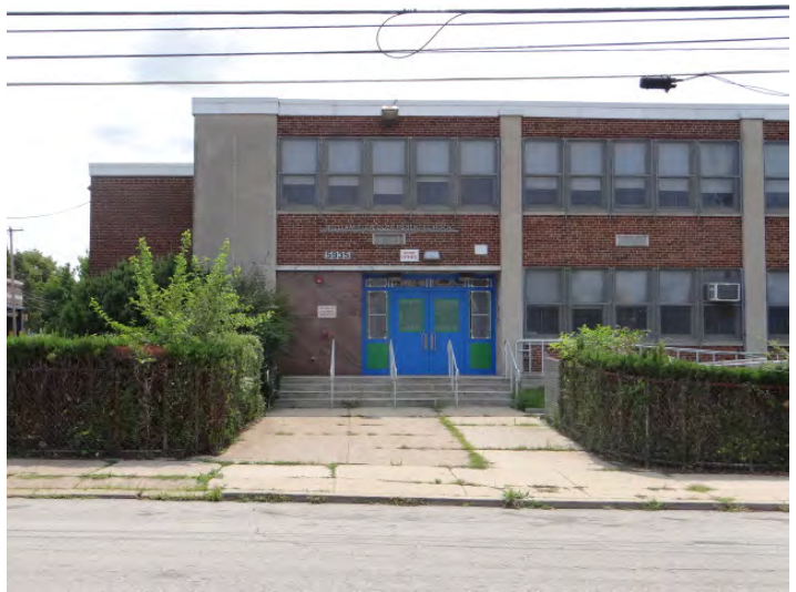
Photo 2: Looking SE at main (NW) facade
