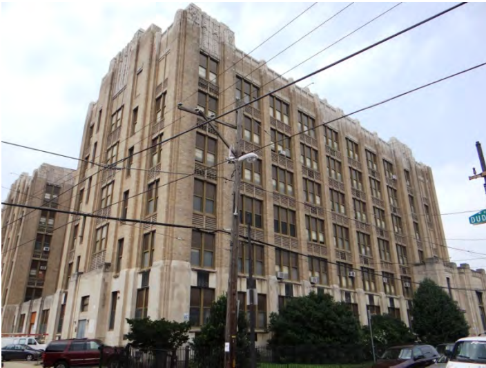
Photo 3: Looking NW at rear (S, left) and E (right) facades
