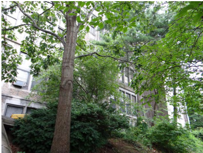
Photo 3: Looking N at N end of main (SE) facade
