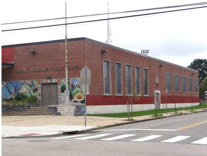
Photo 3: Looking W at NE façade
