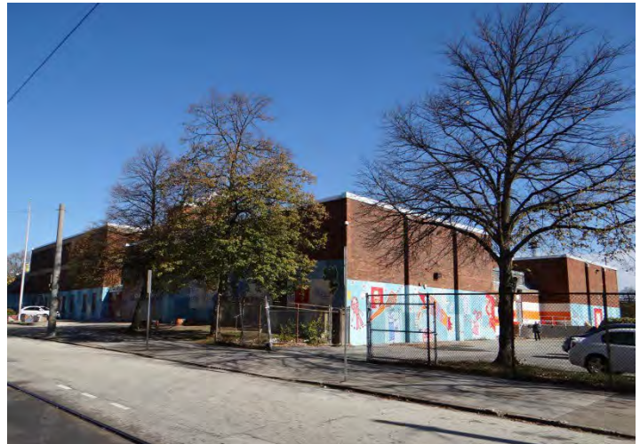
Photo 4: Looking NE at S facade
