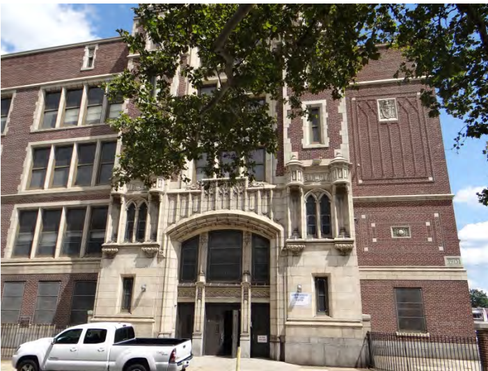
Photo 3: Looking E at entrance at S end of main (W) façade
