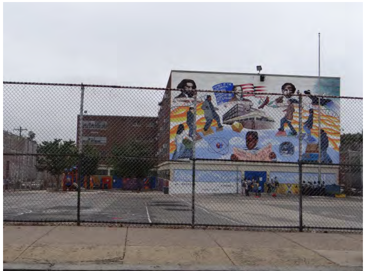
Photo 4: Looking E at W facade
