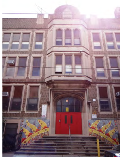
Photo 2: Looking E at main entrance on main (W) facade
