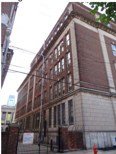
Photo 5: Looking SW at E facade
