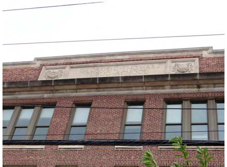
Photo 6: Looking N at main (S) facade
