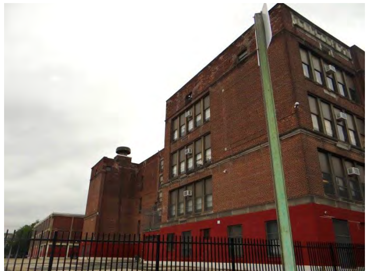
Photo 6: Looking SW at rear (E) facade
