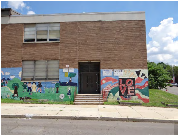
Photo 1: Looking NE at main (SW) façade entrance
