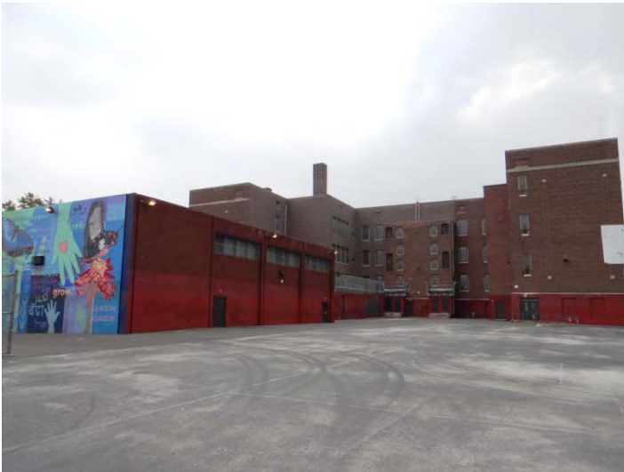
Photo 3: Looking NE W façade and S façade of addition
