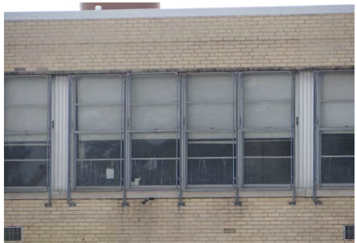
Photo 4: Detail, original windows
