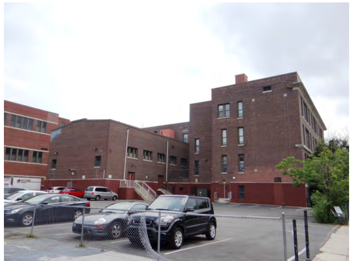
Photo 4: Looking S at rear (N) facade
