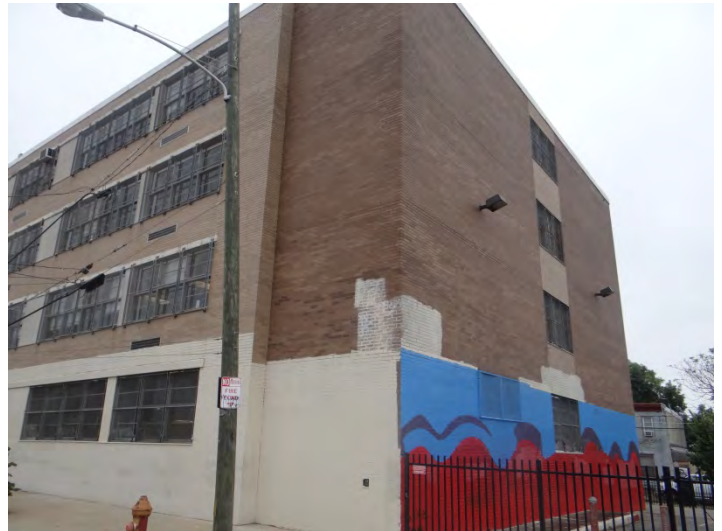
Photo 4: Looking NE at main (W, left) and S (right) facades
