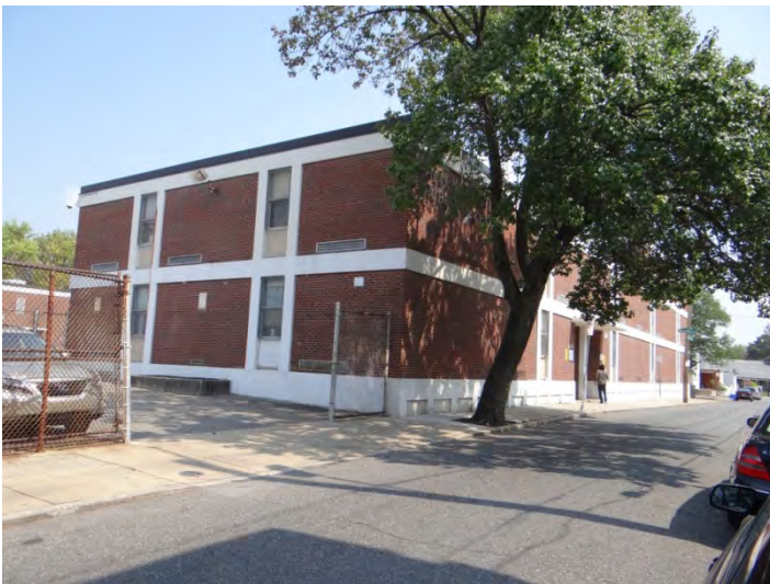
Photo 3: Looking NE at SW (right) and NW (left) facades
