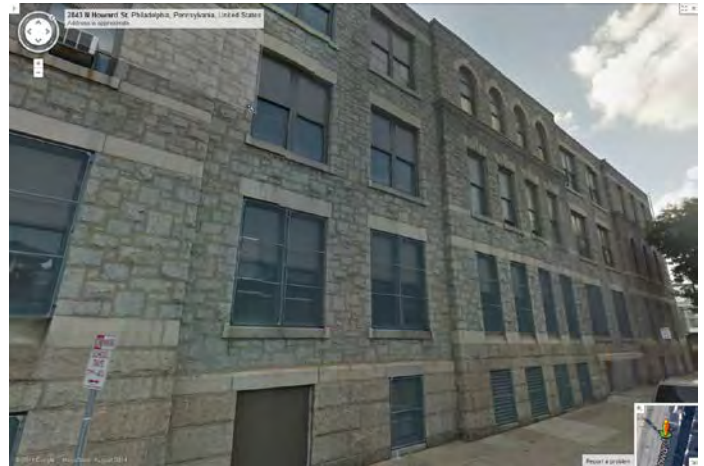
Photo 4: Looking N along W façade. Source: Google maps
