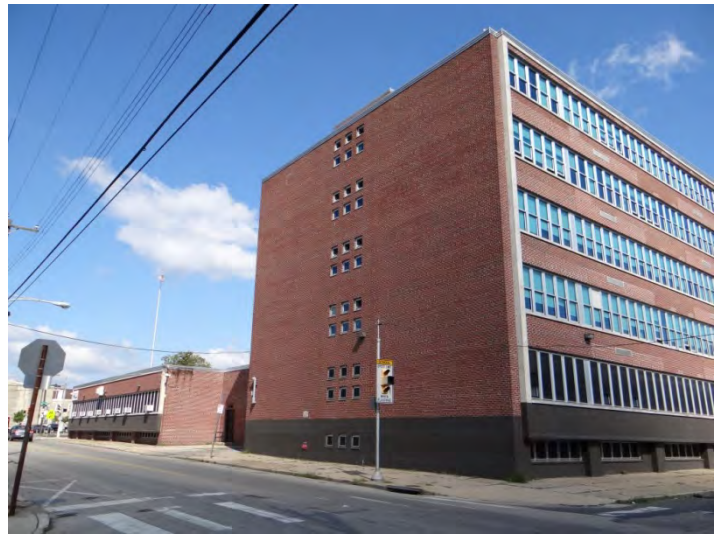
Photo 2: Looking NW at S (left) and E (right) façades
