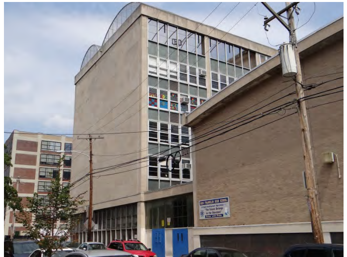
Photo 2: Looking NE at center of rear (W) facade
