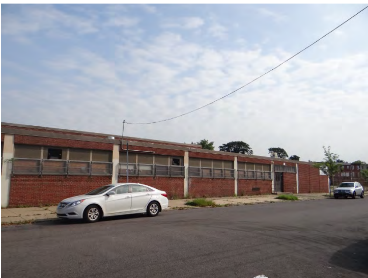
Photo 5: Looking N at S facade
