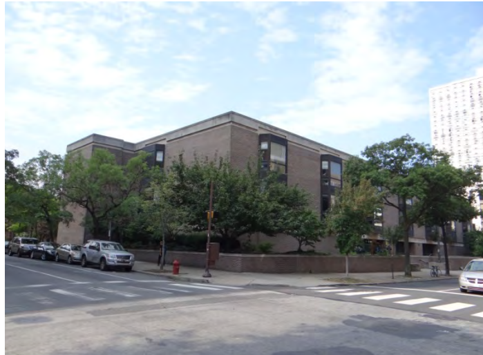
Photo 4: Looking SW at E (left) and main (N, right) facades
