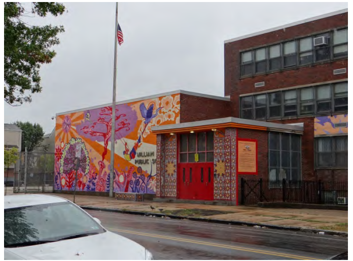
Photo 2: Looking SW at entrance on main (N) façade
