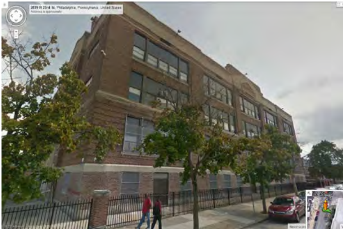
Photo 3: Looking SE at W façade. Source: Google Earth
