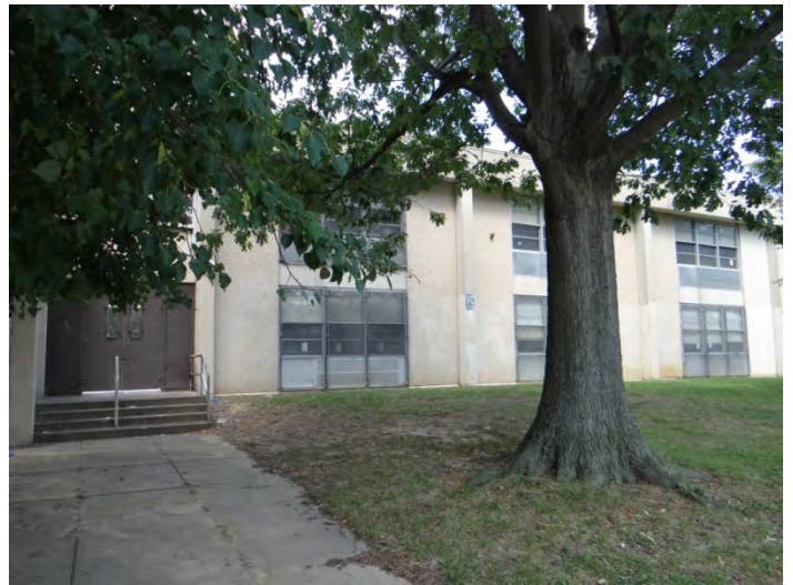
Photo 2: Looking N at main (SE) façade
