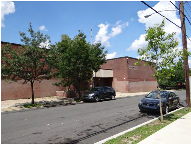
Photo 1: Looking NE at main (S) facade
