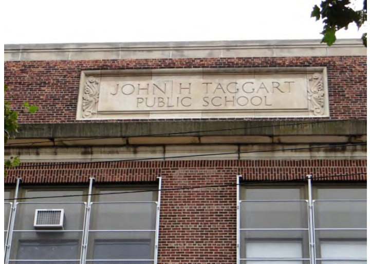
Photo 6: Looking W at E facade
