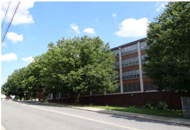
Photo 3: Looking SE at NW façade
