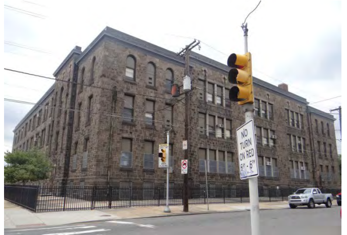
Photo 2: Looking NW at SE facade
