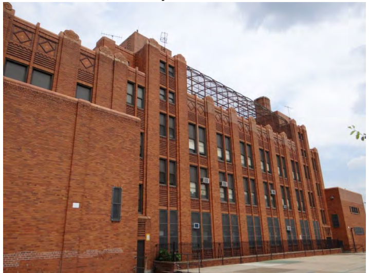
Photo 6: Looking NE at rear (S) facade
