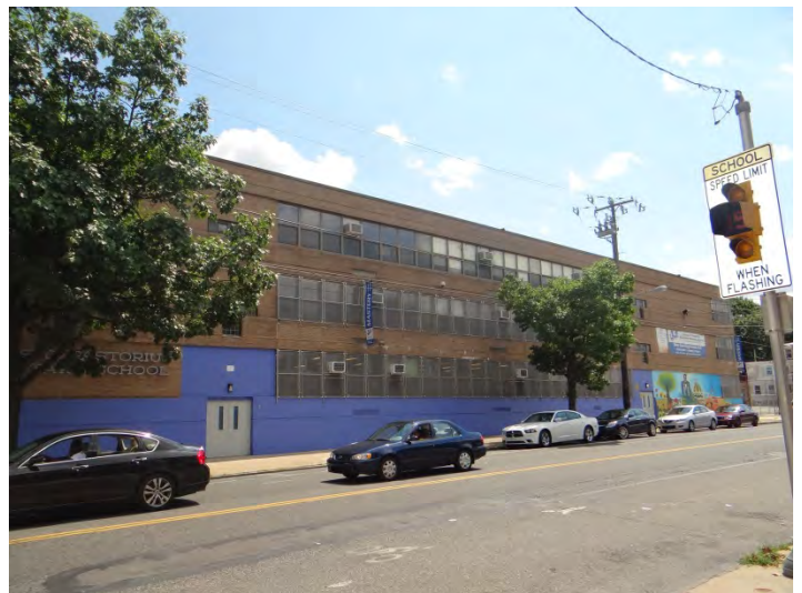
Photo 2: Looking SW along NW facade
