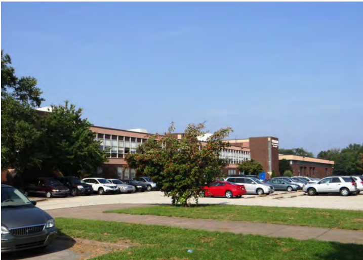
Photo 3: Looking N at center of main (NE) facade
