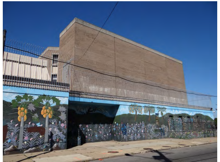
Photo 2: Looking N at E façade and main entrance
