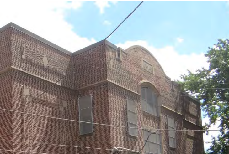
Photo 5: Looking NE at center bay of W facade
