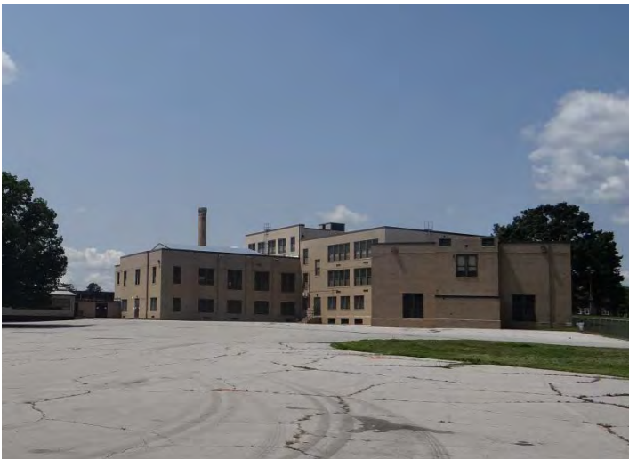
Photo 5: Looking NW at rear (S) facade
