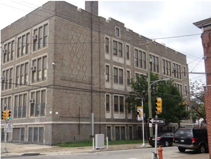
Photo 3: Looking NW at NE façade
