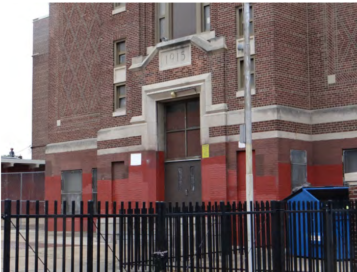
Photo 3: Looking NW at entrance on S facade
