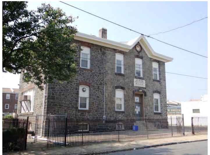
Photo 2: Looking SW at NE (center) and SE (left) facades
