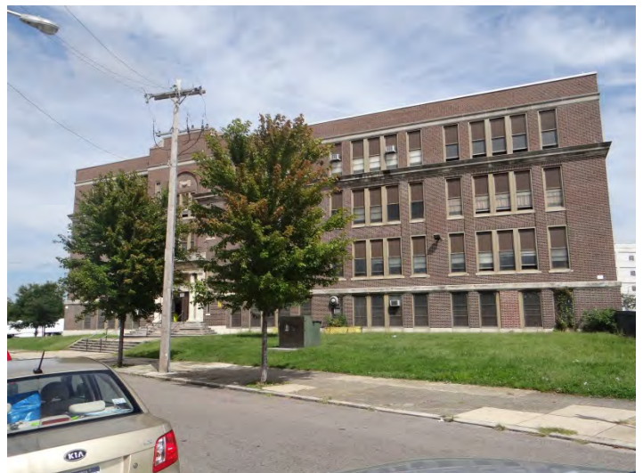
Photo 6: Looking N at S facade
