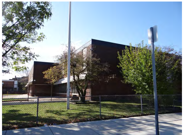
Photo 6: Looking S at E facade
