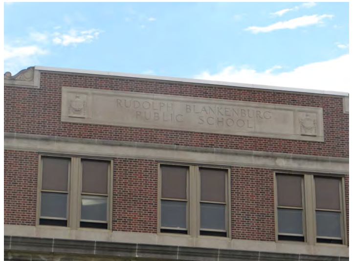
Photo 2: Detail, main (W) façade
