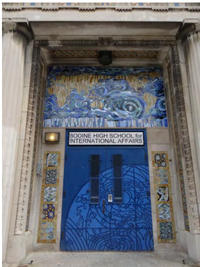
Photo 3: Looking E at main entrance on main (W) façade
