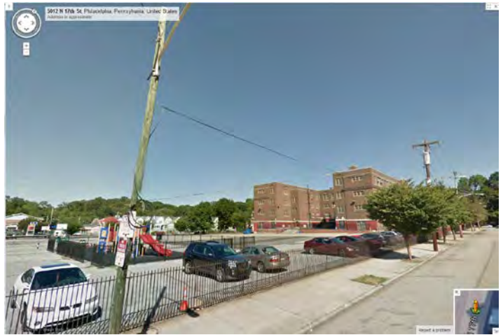
Photo 4: Looking NW at S facade
