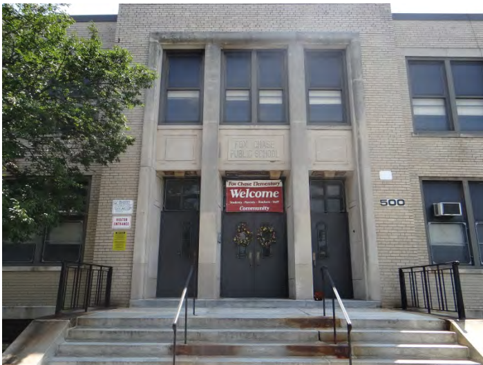
Photo 3: Looking S at main entrance on main (N) facade
