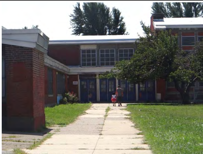
Photo 2: Detail, main entrance on main (NW) facade
