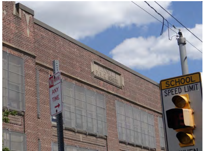
Photo 2: Looking NE at nameplate in center of S façade
