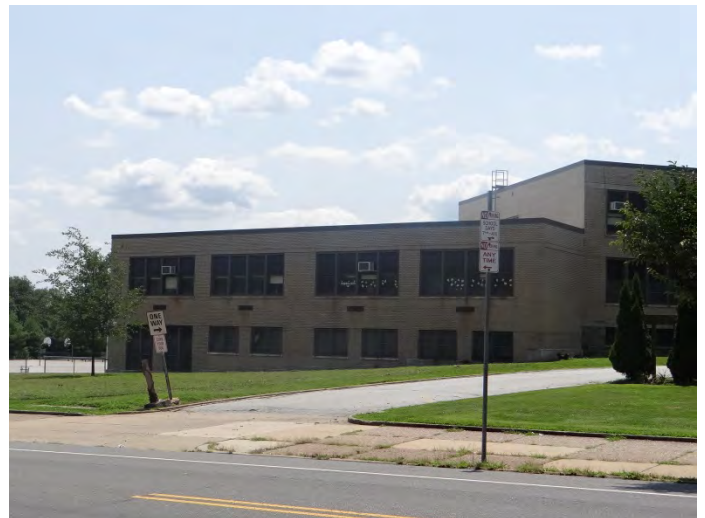
Photo 4: Looking SW at NE facade
