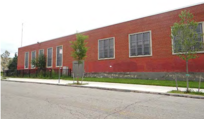
Photo 3: Looking E at NW façade
