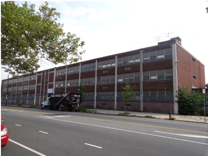
Photo 3: Looking E at S end of main (W) facade
