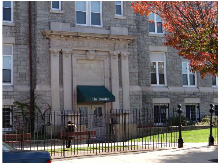
Photo 2: Looking NE at W facade
