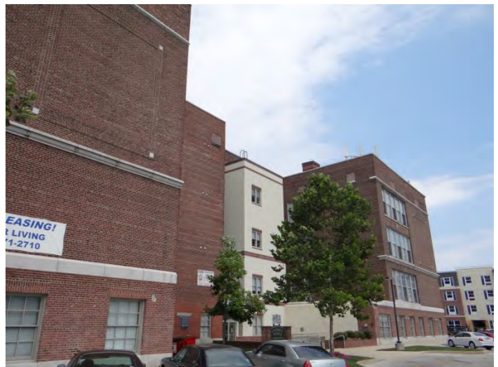
Photo 6: Looking N at S facade
