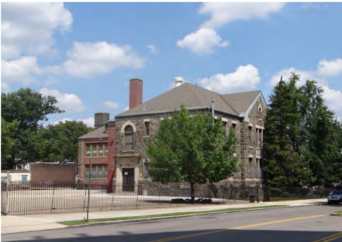
Photo 3: Looking NW at SE facade
