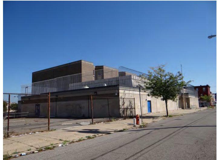
Photo 4: Looking NE at W at W (left) and S (right) facades
