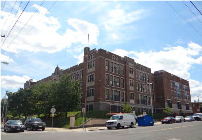
Photo 3: Looking SW at E (left) and N (right) facades
