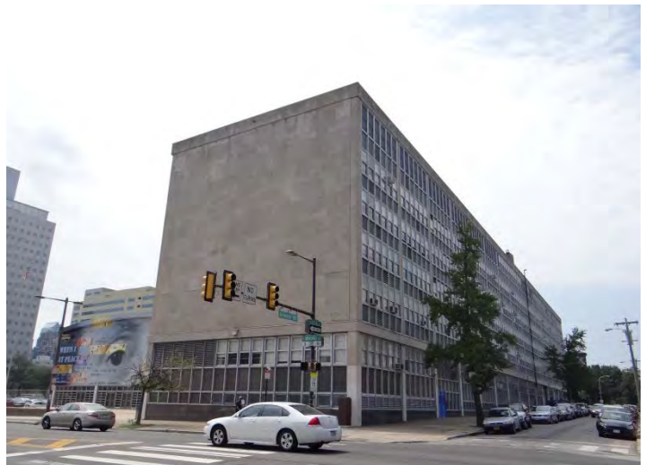
Photo 4: Looking SW at main (E, left) and N facades
