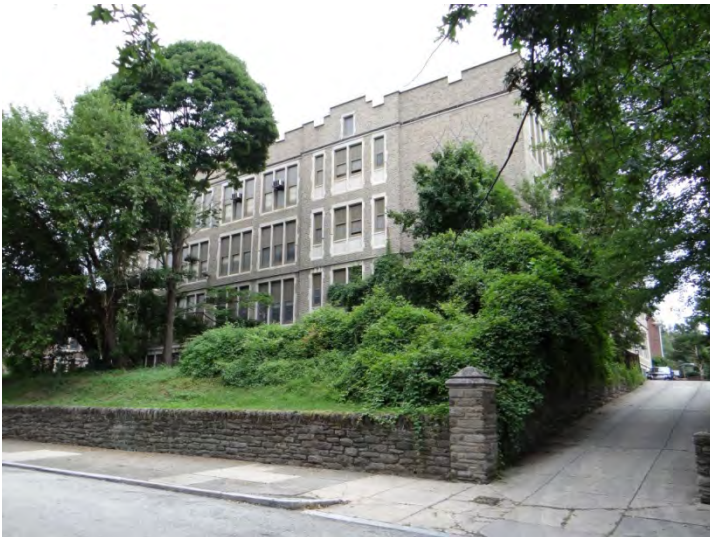
Photo 3: Looking W at NE façade
