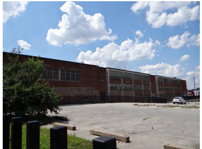
Photo 4: Looking NW at E facade
