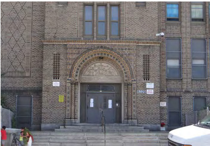
Photo 3: Looking SE at entrance at N end of main (NW) façade
