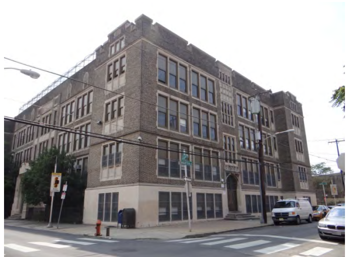
Photo 2: Looking SW at N façade
