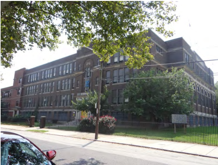
Photo 3: Looking S at NE façade
