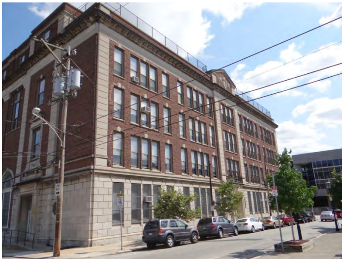
Photo 3: Looking SE at W facade
