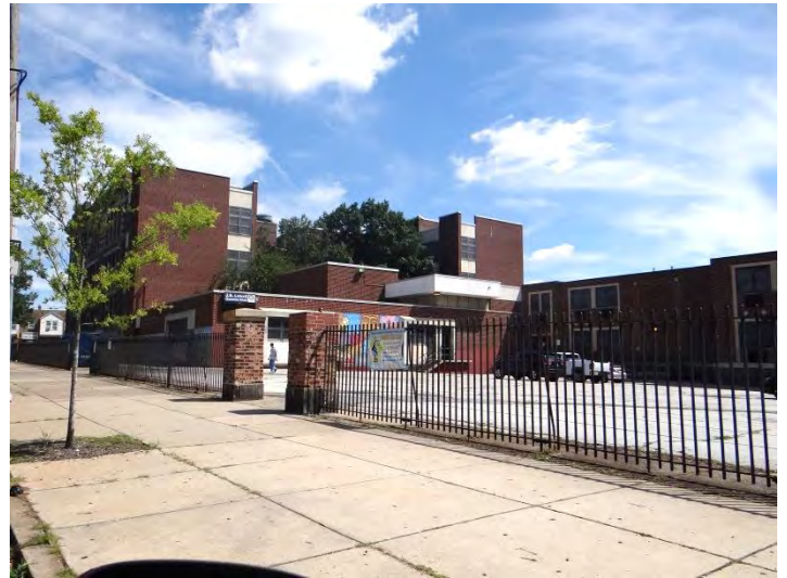
Photo 4: Looking NE at rear façade
