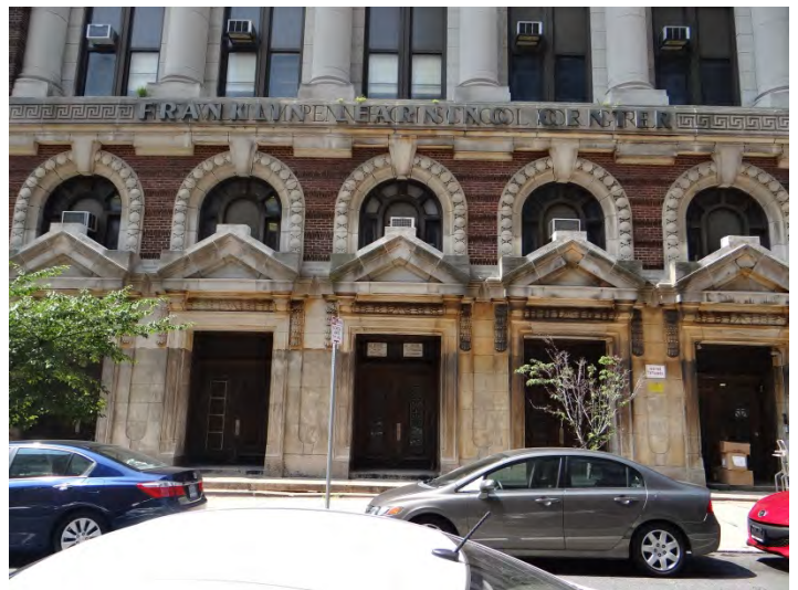
Photo 2: Looking W at main (E) façade entrances
