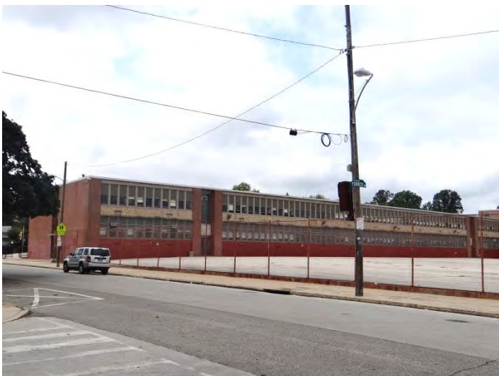
Photo 5: Looking SW at NE facade
