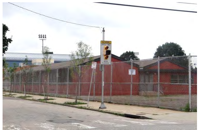
Photo 6: Looking N at portables at S end
