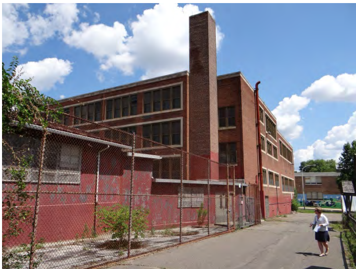
Photo 5: Looking N at SE façade of portable addition
