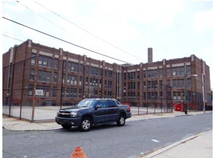
Photo 4: Looking SE at rear (W, left and N, right) facades
