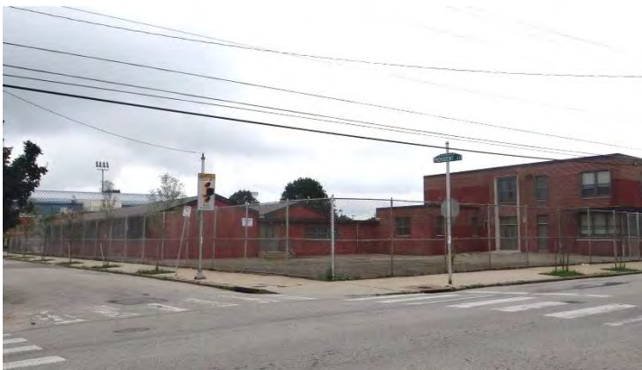
Photo 5: Looking NW at SW façade
