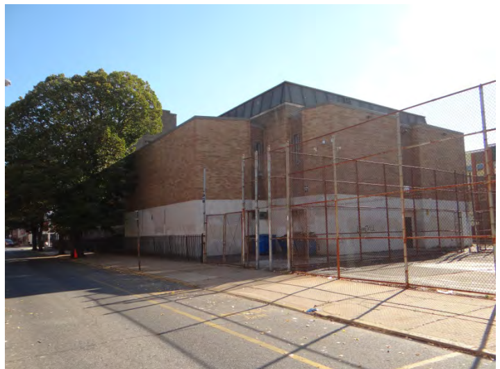
Photo 6: Looking NE at SW facade
