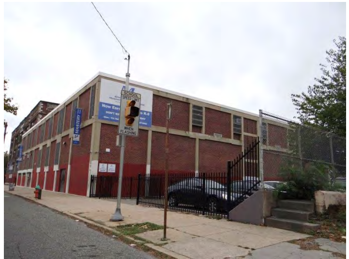
Photo 2: Looking NE at S (right) and W (left) facades of addition
