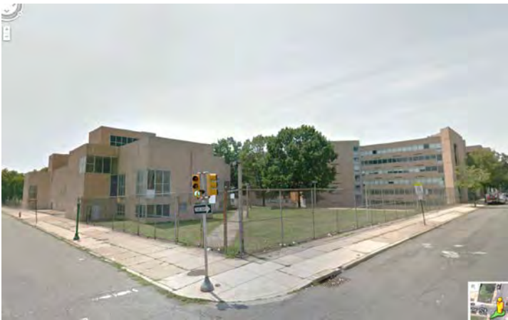
Photo 5: Looking SW at NE quadrant, E (right) and N (left) walls
