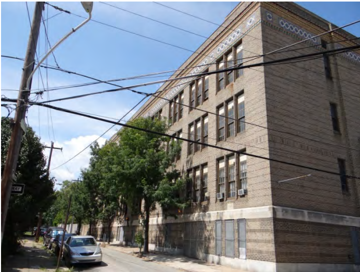
Photo 3: Looking NW at S facade
