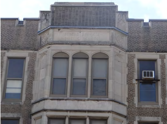
Photo 3: Looking S at N façade center bay
