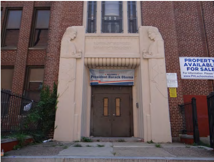
Photo 3: Entrance, main (NW) façade
