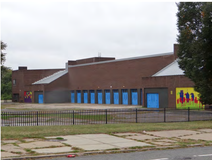
Photo 5: Looking NW at S facade
