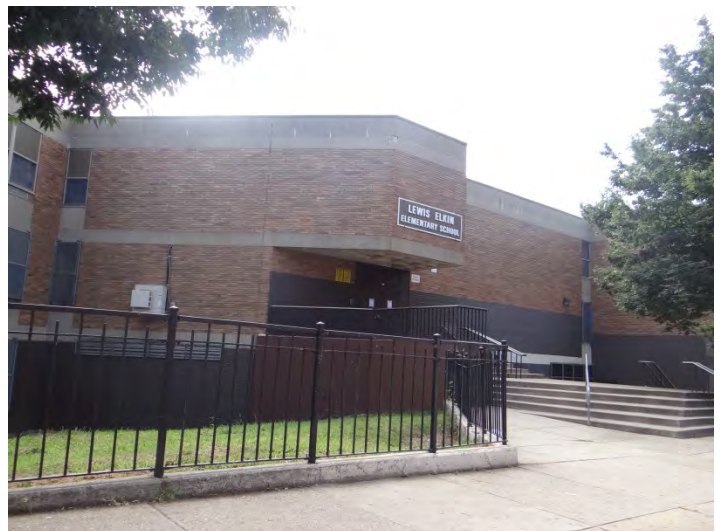
Photo 6: Looking SE at main entrance on W facade
