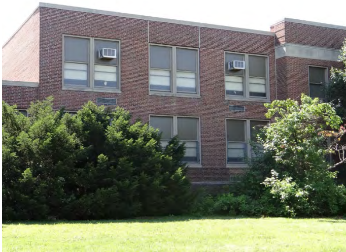
Photo 3: Looking E at N end of main (NW) facade
