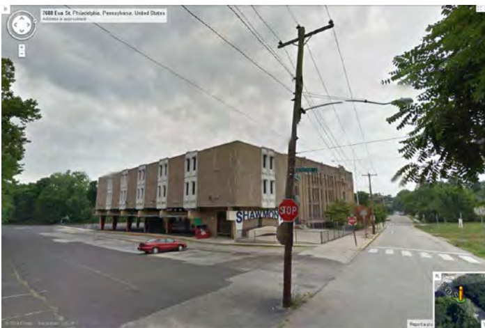
Photo 5: Looking NW at NE (right) and SE (left) facades
