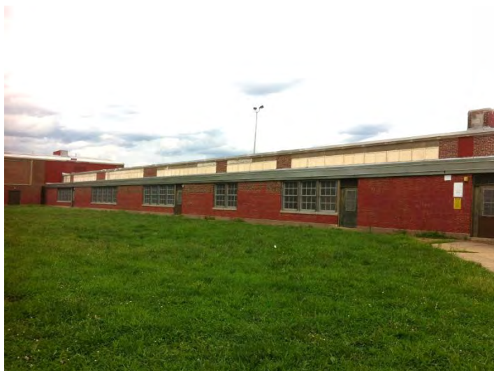
Photo 6: Typical classroom wing, N and S facades
