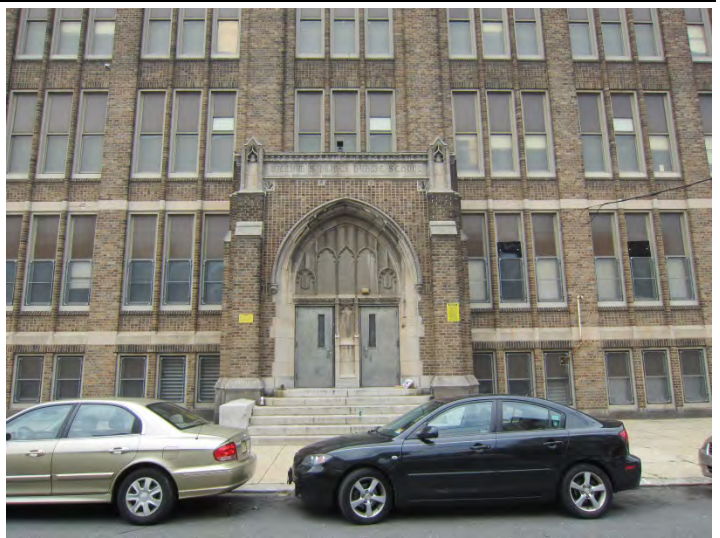
Photo 2: Looking W at E façade entrance
