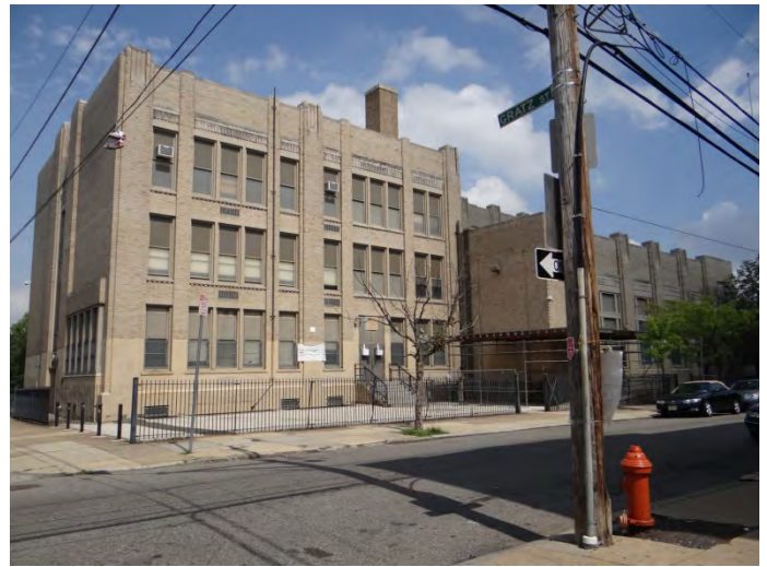
Photo 4: Looking NE at S façade (auditorium to right)
