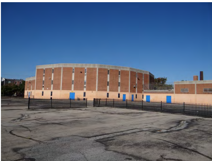
Photo 5: Looking W at E facade
