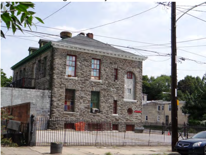
Photo 5: Looking NE at SW facade
