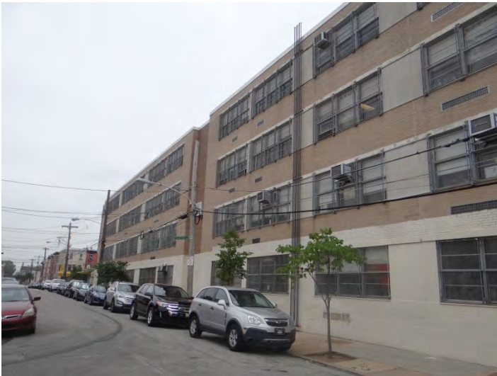
Photo 3: Looking NE at main (W) façade
