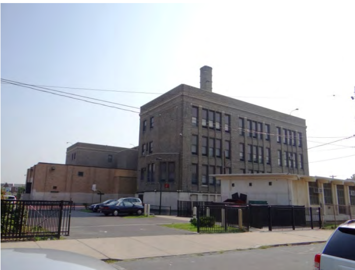
Photo 5: Looking SE at SW (right) and NW (left) facades
