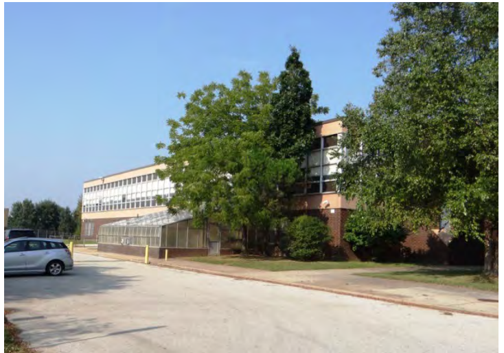
Photo 4: Looking NW at SE facade
