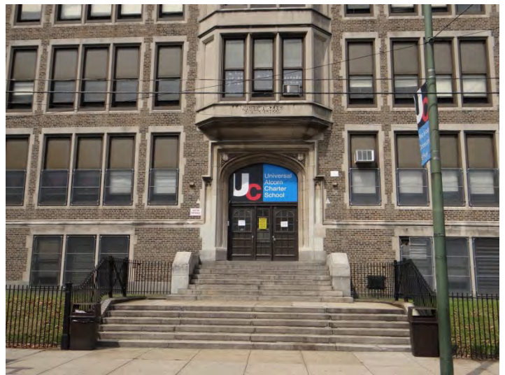
Photo 2: Looking W at E main entrance
