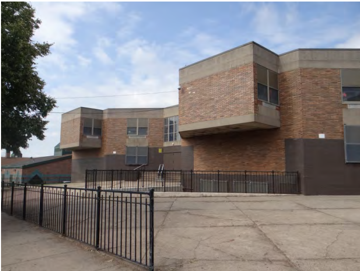
Photo 3: Looking SW at E facade
