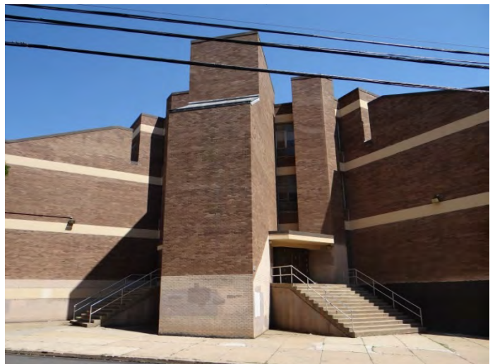
Photo 6: Looking N at S facade
