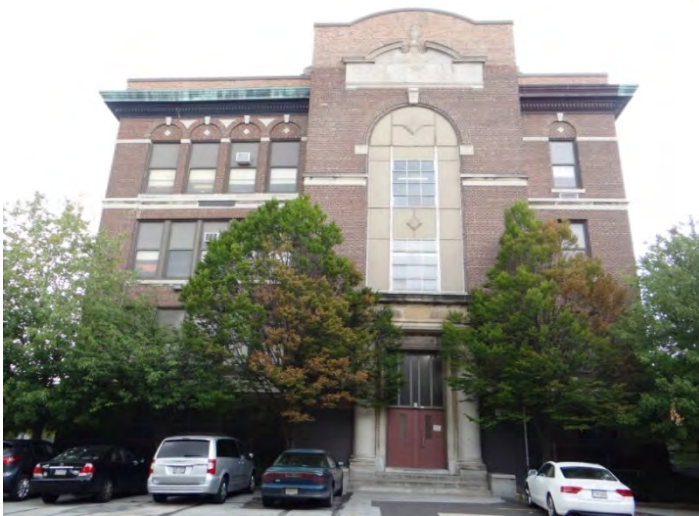
Photo 1: Looking E at W facade
