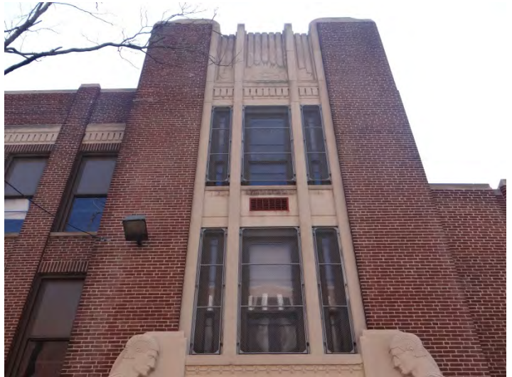
Photo 4: Entrance tower, main (NW) façade
