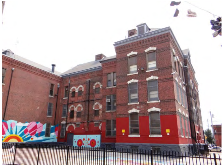
Photo 4: Looking S at N facade
