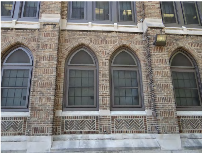
Photo 3: Looking SW at NE façade wall/window details
