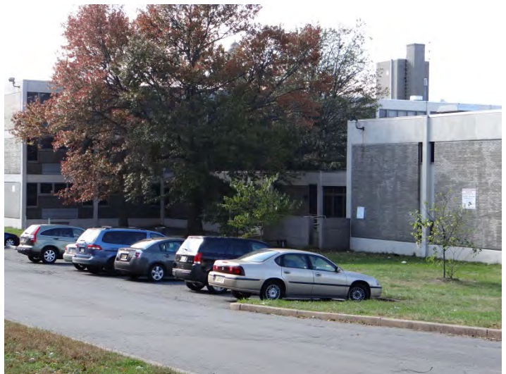
Photo 6: Looking SW at S end of E facade
