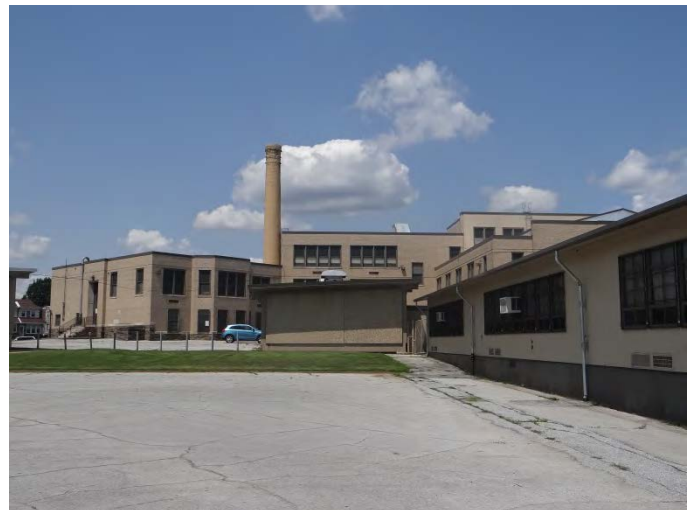
Photo 6: Looking NE at rear (S) facade
