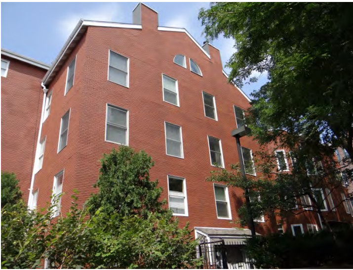
Photo 1: Looking NW at E facade
