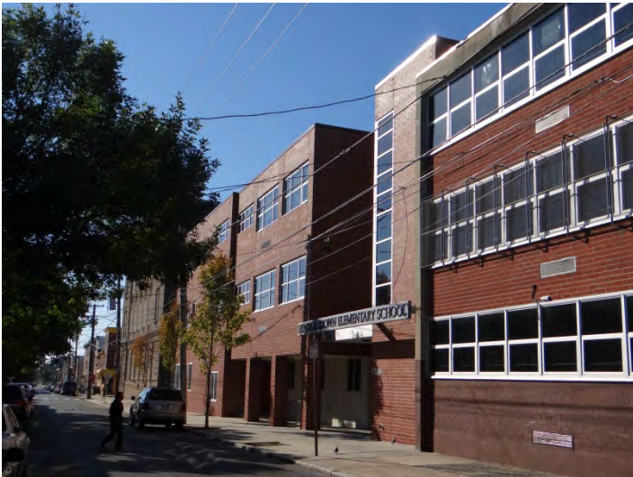
Photo 3: Looking S at center of NE façade
