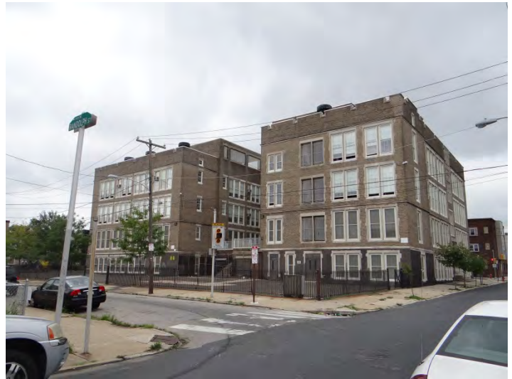
Photo 4: Looking SW at rear (E) façade
