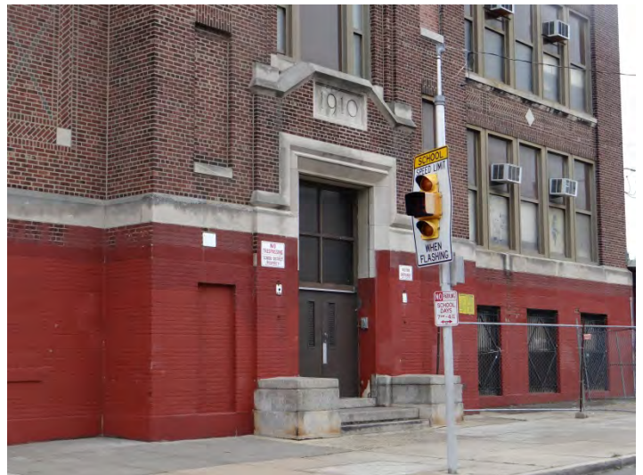
Photo 4: Looking W at entrance at N end of E façade
