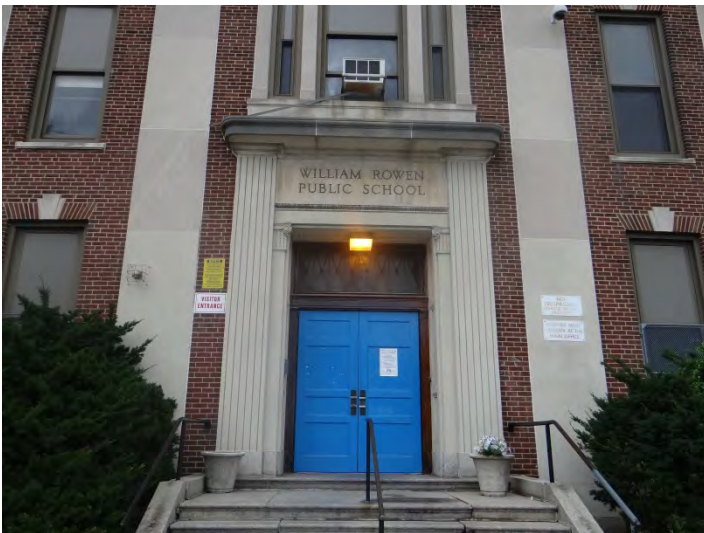
Photo 3: Looking E at entrance on main (W) facade
