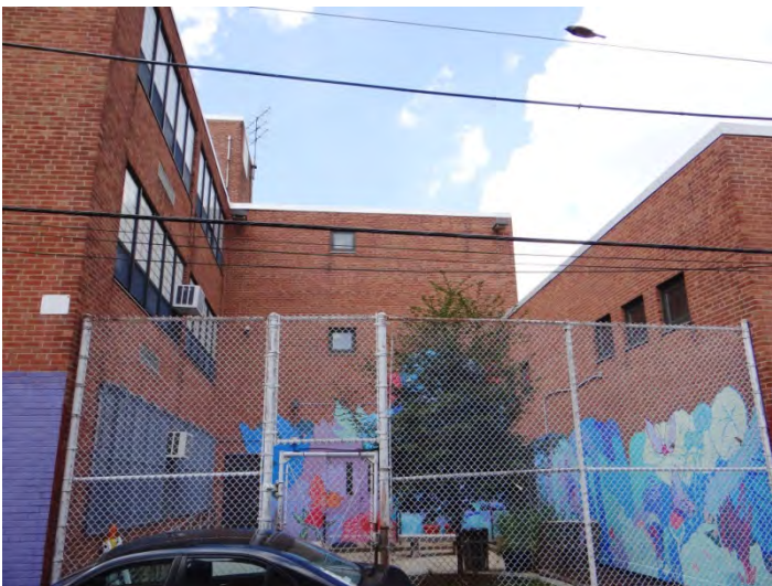
Photo 5: Looking N at E end of S façade
