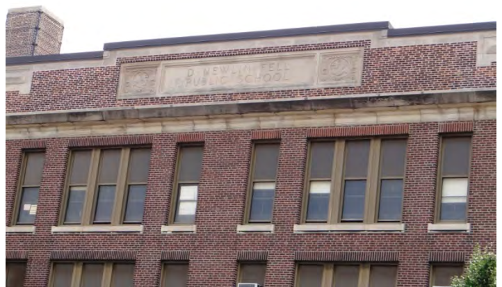
Photo 6: Looking S at main (N) façade
