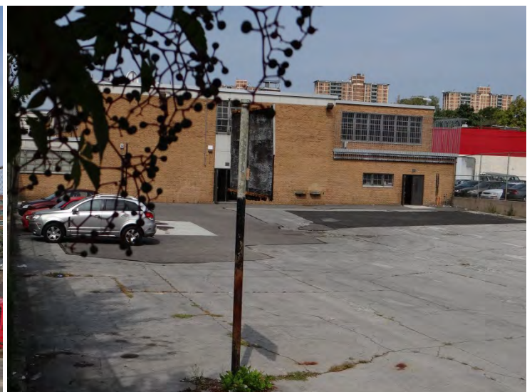
Photo 6: Looking W at E façade
