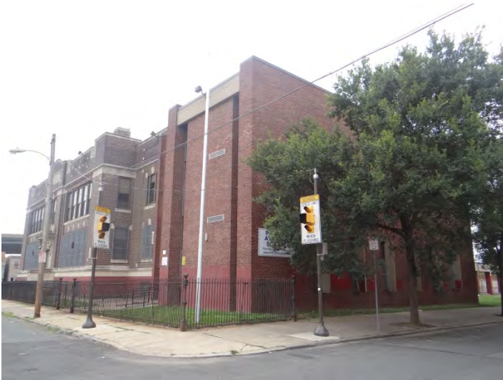
Photo 3: Looking S at main (NE, left) and NW (right) facades
