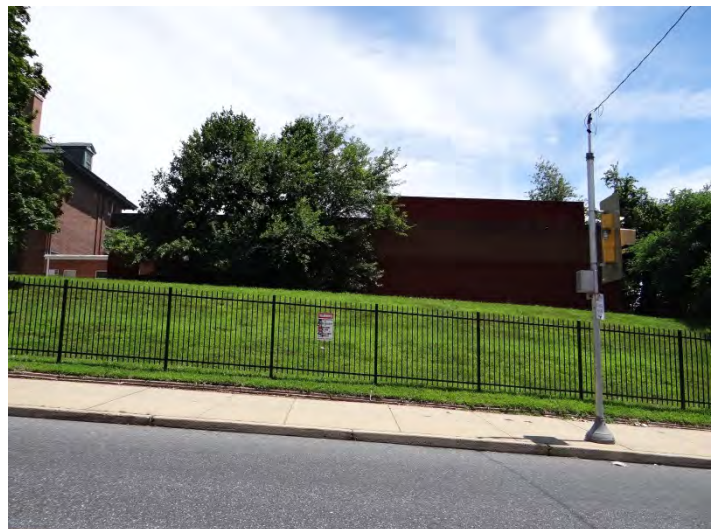
Photo 6: Looking SE at NW façade of addition to SW
