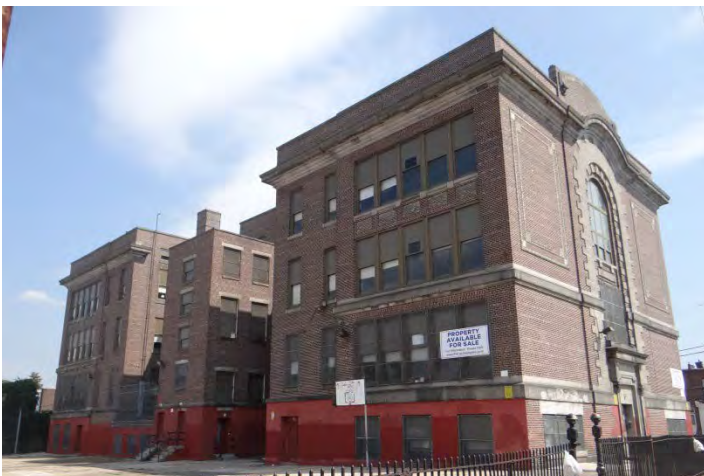
Photo 5: Looking NE at SW (left) and SE (right) facades
