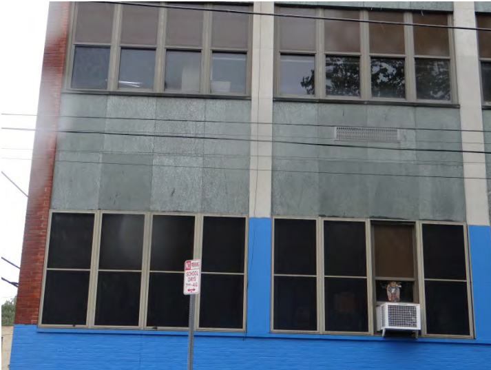
Photo 3: Looking S at main (N) façade window bay
