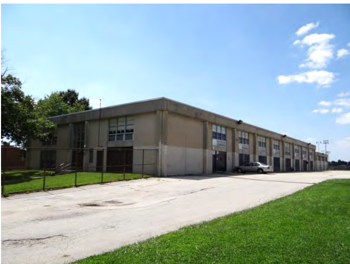
Photo 5: Looking S at NW (right) and NE (left) facades
