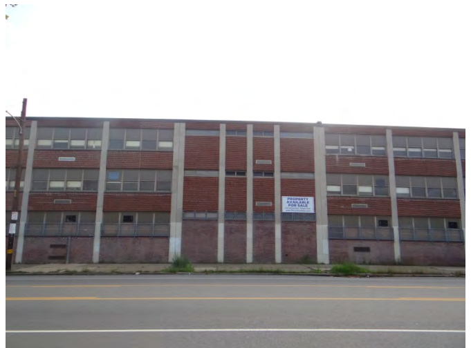
Photo 2: Looking E at center of main (W) facade
