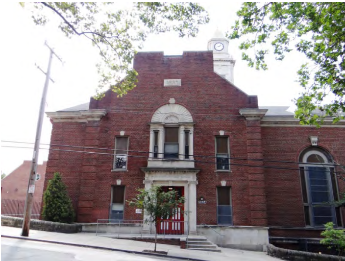
Photo 3: Looking SW at E end of NE facade
