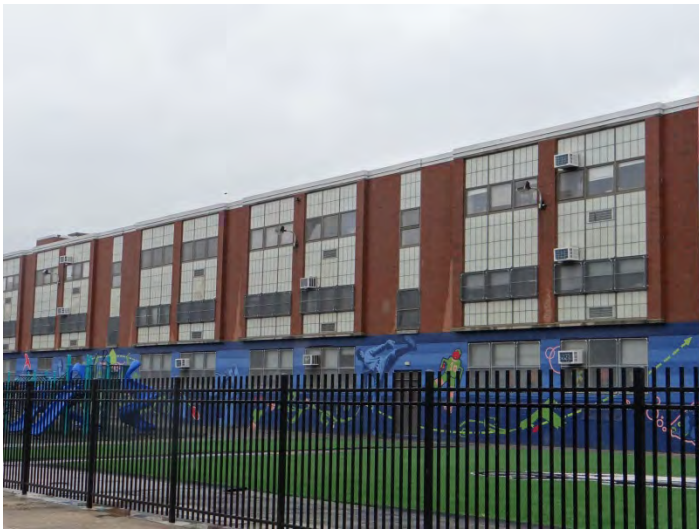
Photo 3: Looking SW at E facade
