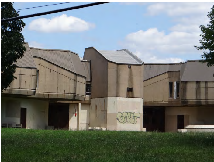
Photo 5: Looking NE at SW facade
