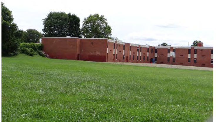
Photo 4: Looking SE at N (left) and W (right) facades
