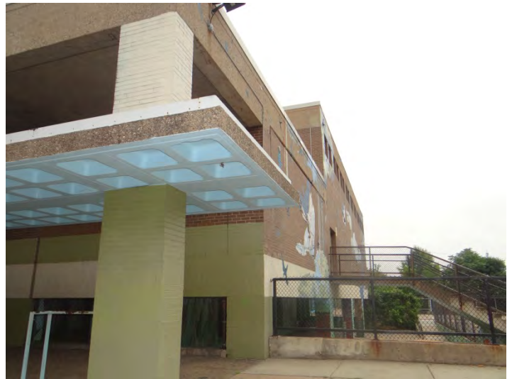
Photo 2: Looking NE at W corner of S facade
