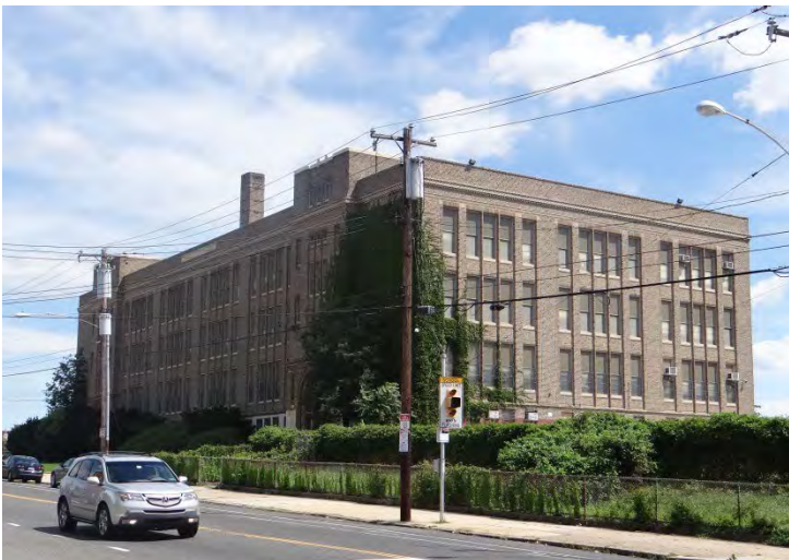
Photo 5: Looking NE at main (N, left) and S (right) facades
