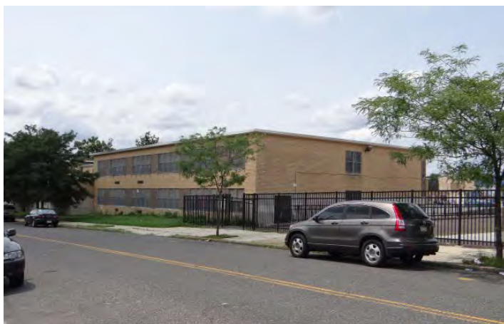
Photo 6: Looking W at rear (SE) facade
