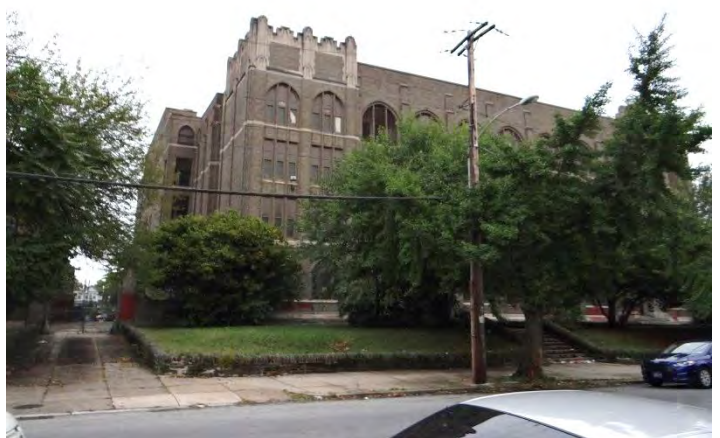
Photo 4: Looking SE at W (right) and rear (N, left) facades
