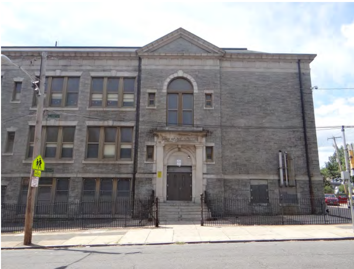
Photo 3: Looking W at E facade
