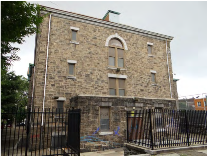
Photo 3: Looking W at E facade
