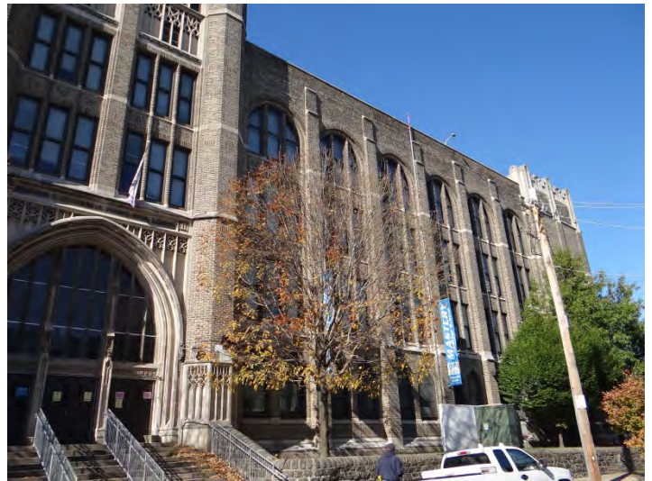
Photo 2: Looking NW at N end of main (E) facade
