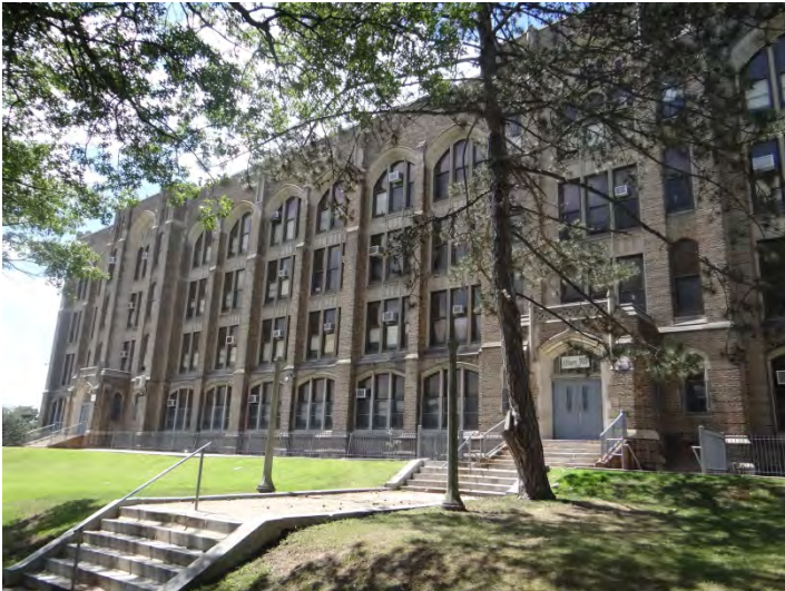
Photo 3: Looking SW at E facade
