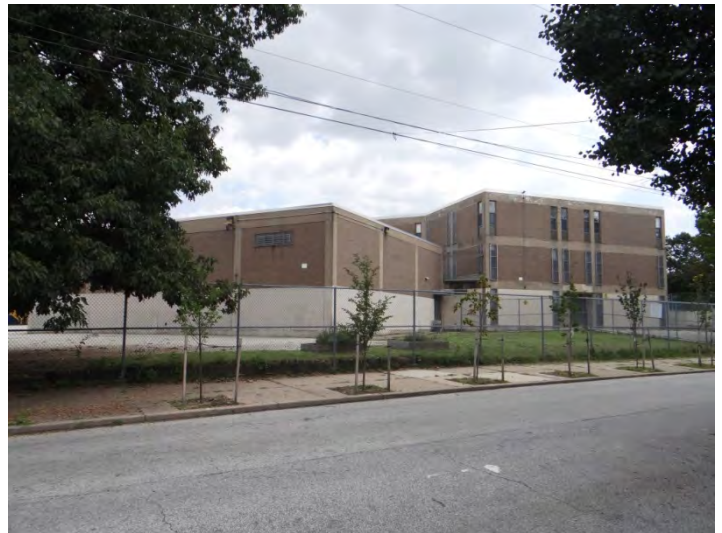
Photo 4: Looking E at W facade
