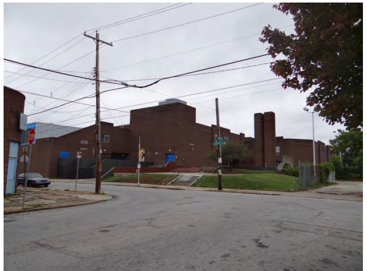
Photo 4: Looking NW at W facade
