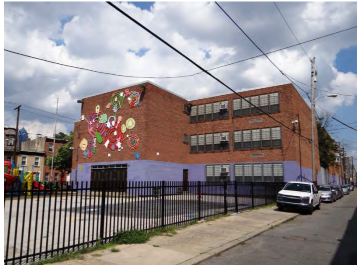
Photo 4: Looking NE at W façade
