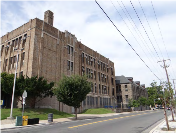
Photo 3: Looking NW at main (NE) facade
