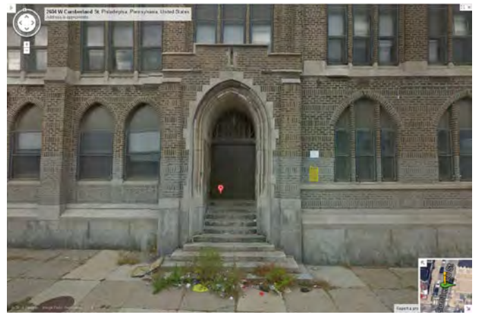
Photo 6: Looking E at entrance on W facade
