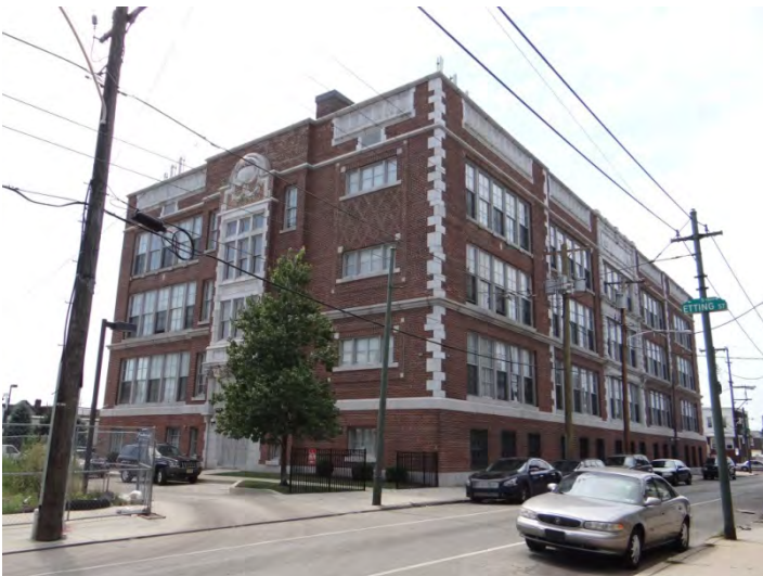
Photo 5: Looking SW at N (right) and E facades
