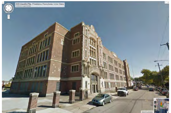
Photo 2: Looking SE at main (W, right) and N (left) facades. Source: Google Earth, August 2014
