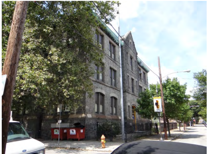
Photo 4: Looking NW at E facade
