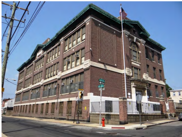
Photo 4: Looking NW at SW (left) and SE (right) facades
