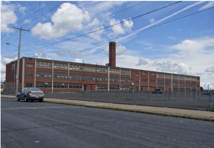
Photo 3: Looking E at SW facade
