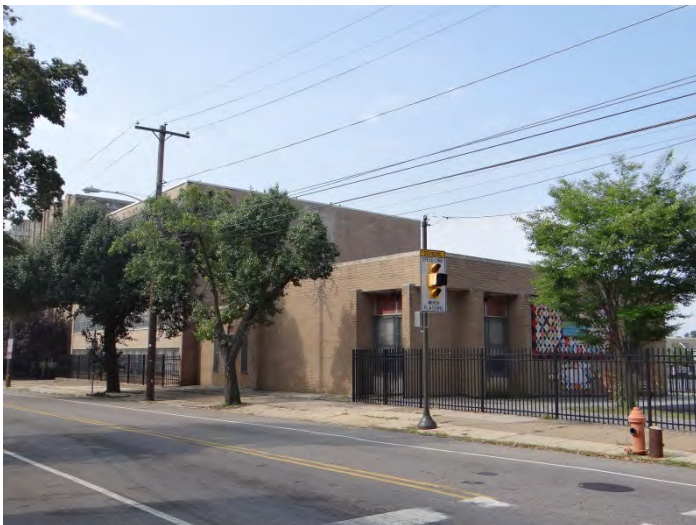
Photo 5: Looking SW at N façade of last addition
