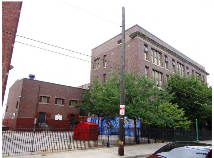
Photo 4: Looking NW at rear (S, left) and E (right) facades
