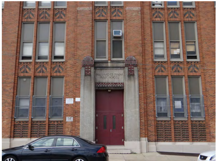
Photo 2: Looking W at N entrance on main (E) façade
