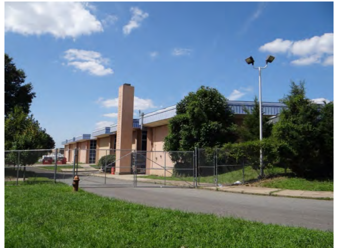
Photo 4: Looking SW at rear (E) facade
