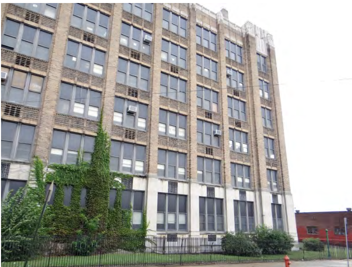
Photo 5: Looking SE at W façade
