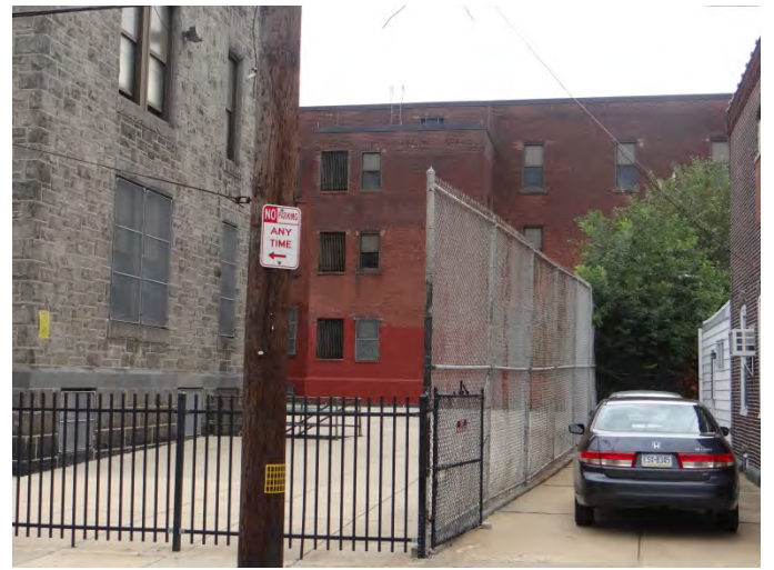
Photo 6: Looking SE at NW façade in rear courtyard
