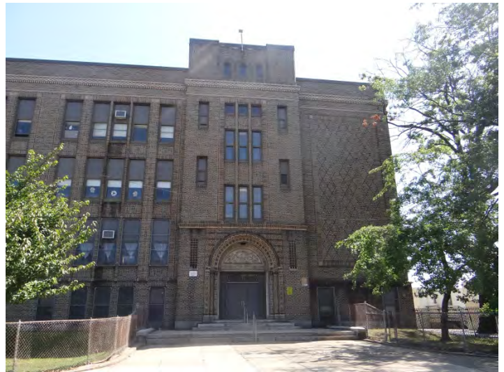
Photo 2: Looking SE at S end of main (NW) facade
