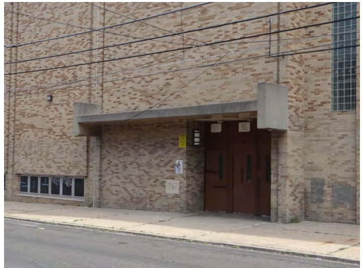
Photo 4: Looking NE at entrance at NW end of SW facade
