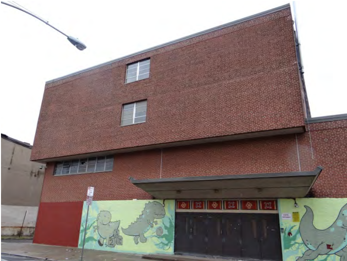
Photo 5: Looking NE at W facade
