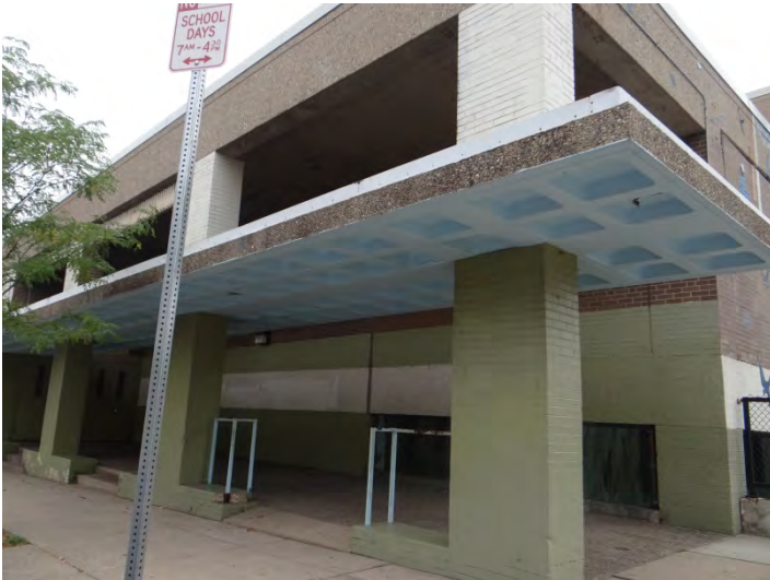
Photo 3: Looking NE at S corner of W facade
