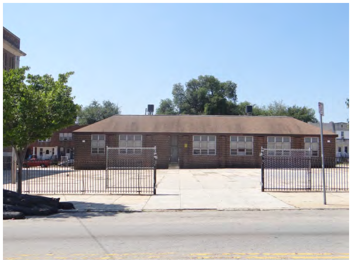
Photo 6: Looking SW at NE façade of annex building
