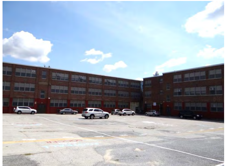
Photo 4: Looking SE at S (right) and W (left) facades
