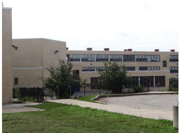
Photo 6: Looking SE at rear (N) facades
