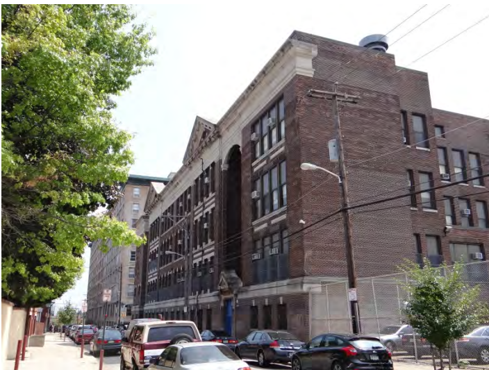
Photo 5: Looking SE at N facade
