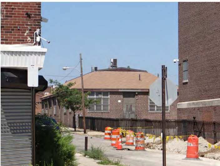
Photo 5: Looking NW at SE façade of annex building
