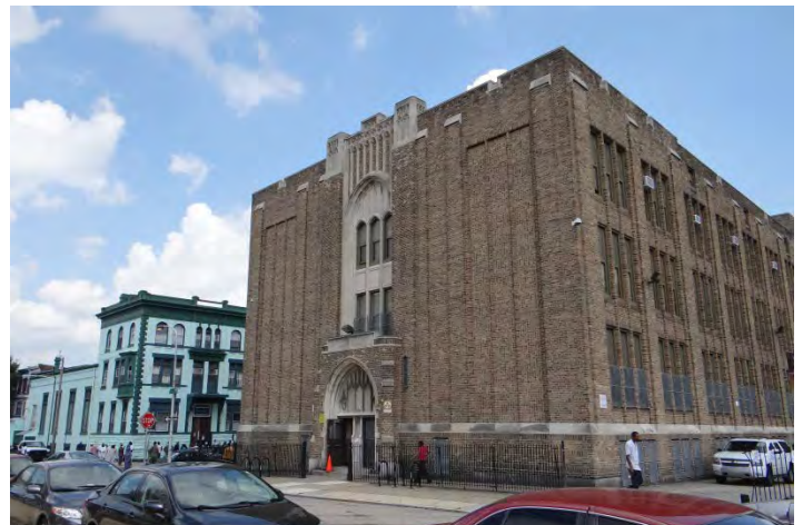
Photo 6: Looking E at W facade
