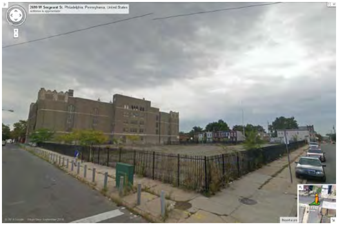
Photo 4: Looking SW at rear (N) facade
