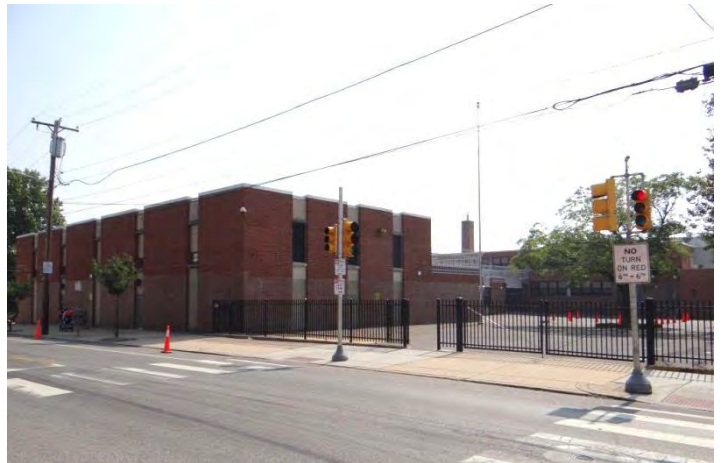
Photo 2: Looking E at NW (left) and SW (right) facades
