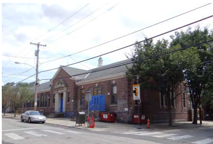
Photo 3: Looking SE at N facade
