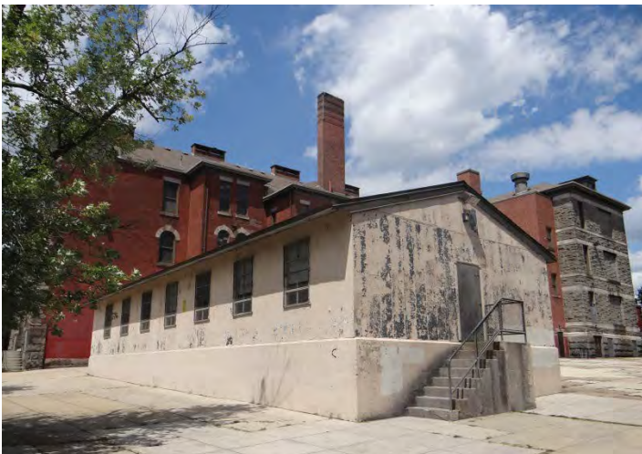
Photo 5: Looking N at SW facade
