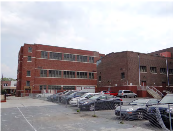
Photo 5: Looking E at W façade
