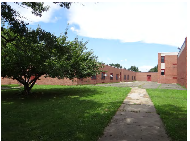
Photo 6: Looking N at W end of S facade
