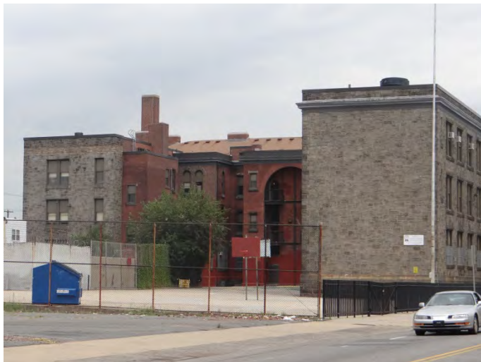
Photo 5: Looking NE at rear (W) facades and courtyard
