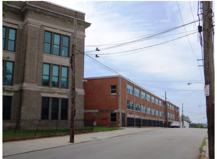
Photo 4: Looking W at NW façade of addition
