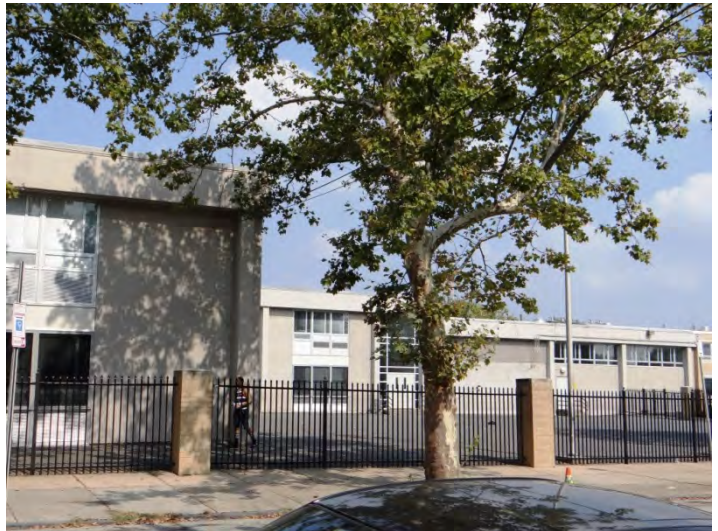
Photo 4: Looking E at SW facade
