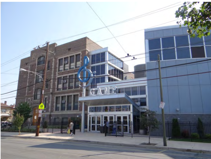
Photo 5: Looking NE at W façade
