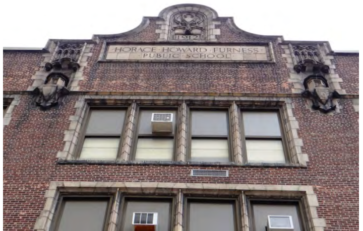
Photo 6: Looking W at E facade
