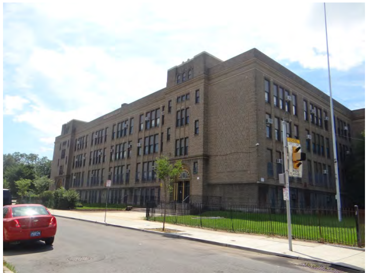
Photo 4: Looking SW at main (E, right) and N (left) facades
