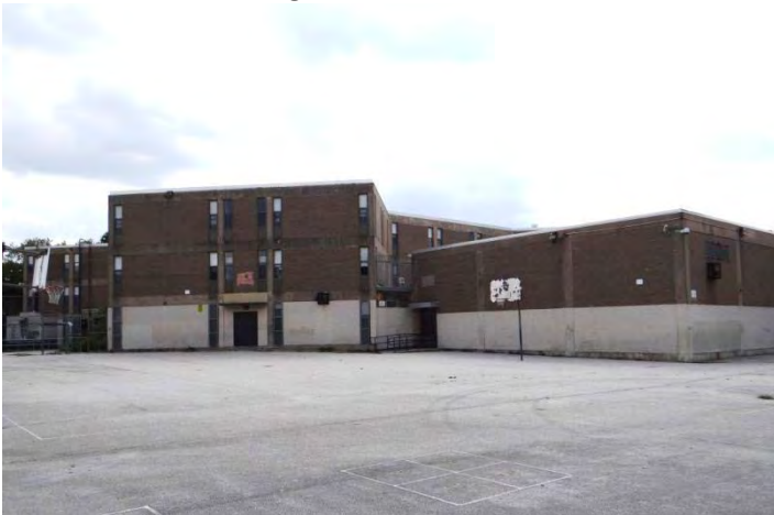
Photo 5: Looking SW at N facades
