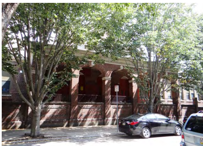
Photo 4: Looking E at center of W facade
