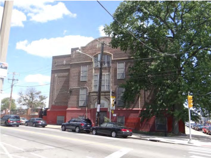
Photo 3: Looking E at W facade
