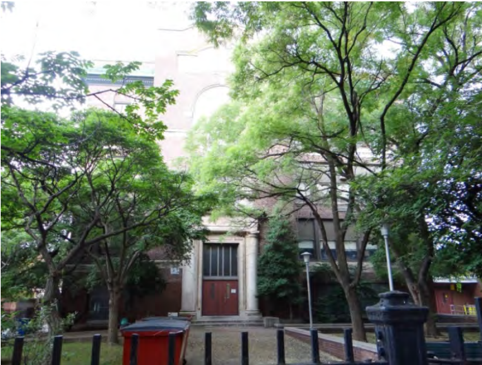
Photo 3: Looking W at E facade
