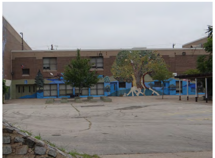
Photo 6: Looking N at S facade
