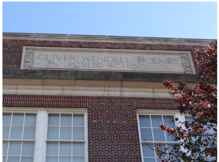
Photo 6: Looking E at W facade
