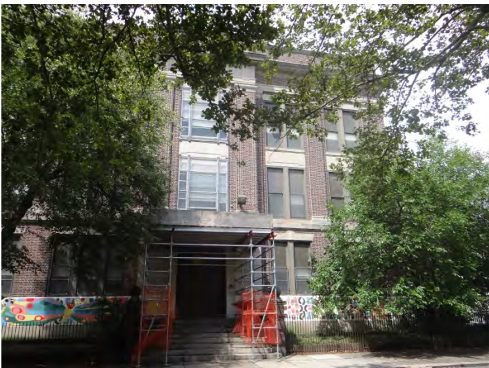
Photo 5: Looking E at W facade
