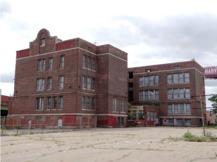
Photo 3: Looking SW at rear (N) façade
