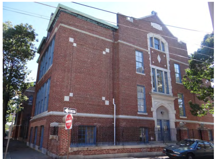
Photo 6: Looking SE at W facade
