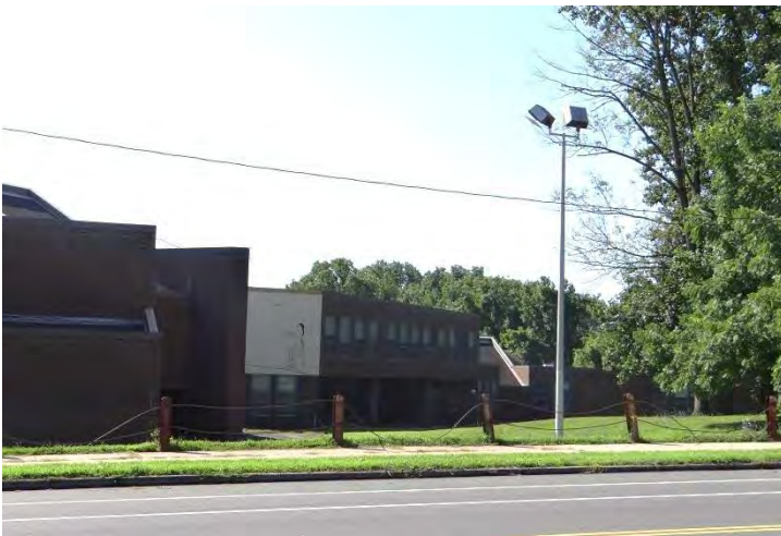
Photo 3: Looking S at N end of W facade
