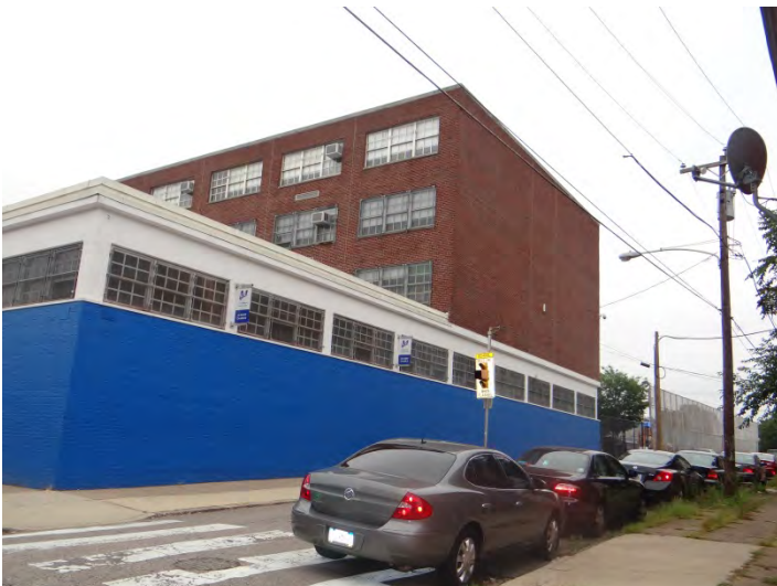
Photo 5: Looking SW at W (right) and N facades
