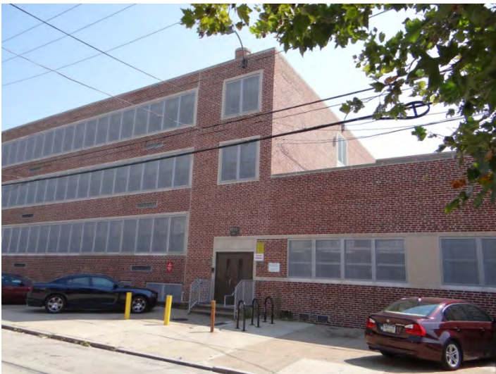
Photo 5: Looking NE at W facade
