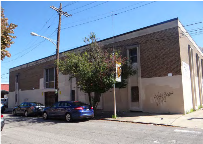
Photo 5: Looking NE at secondary building, W façade
