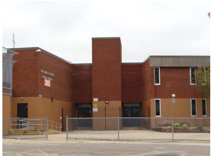
Photo 4: Looking W at main entrance on E facade
