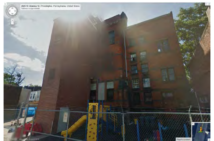
Photo 6: Looking SW at rear (E) facade
