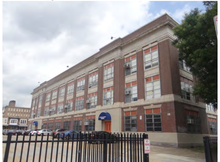
Photo 4: Looking N at SW façade
