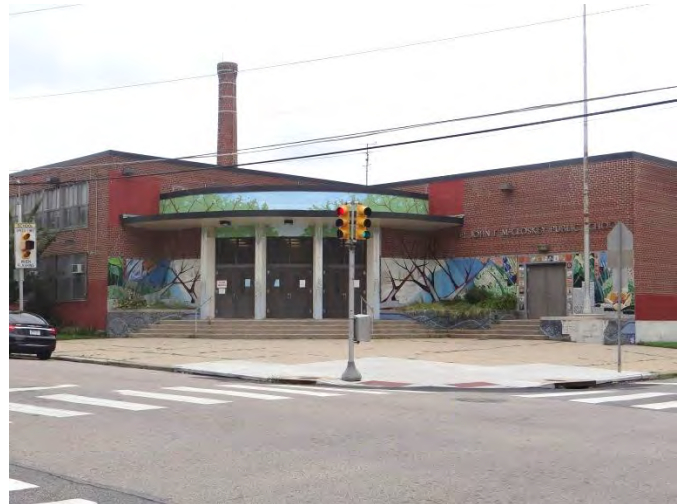
Photo 2: Looking W at main entrance at NE corner
