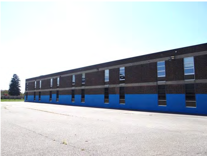
Photo 5: Looking S at NE facade
