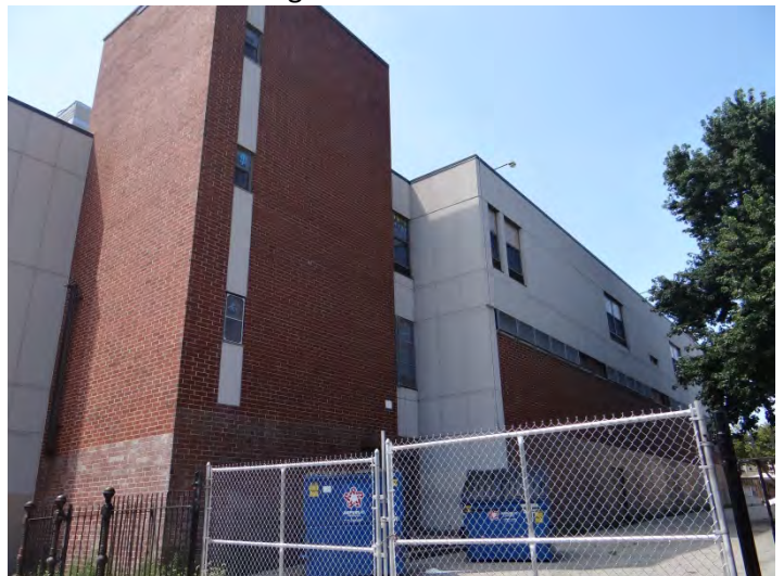
Photo 6: Looking W at NE facade
