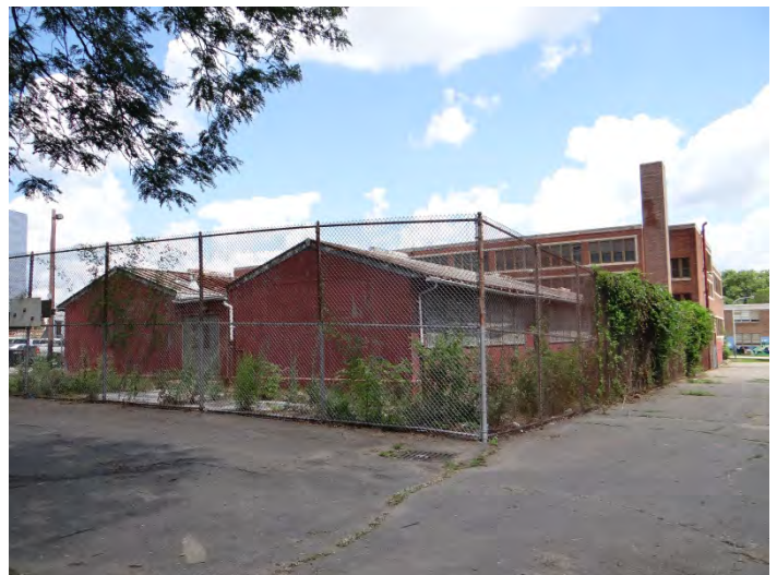
Photo 6: Looking N at S façade of portable addition
