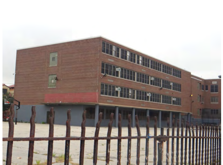
Photo 4: Looking SE at W façade of addition
