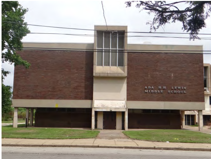
Photo 3: Looking NE at W corner of main (SW) facade
