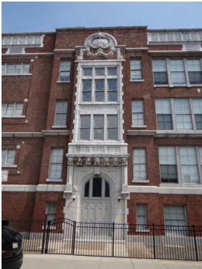
Photo 3: Looking E at W façade entrance
