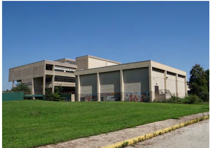
Photo 4: Looking NW at SW facade
