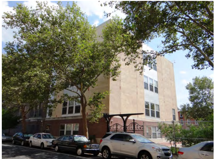
Photo 4: Looking SE at N (left) and W facades
