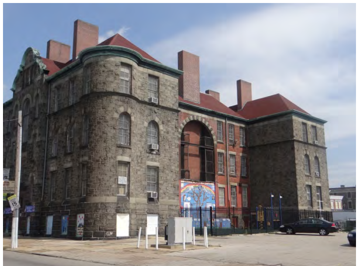
Photo 6: Looking N at rear (SE) facade
