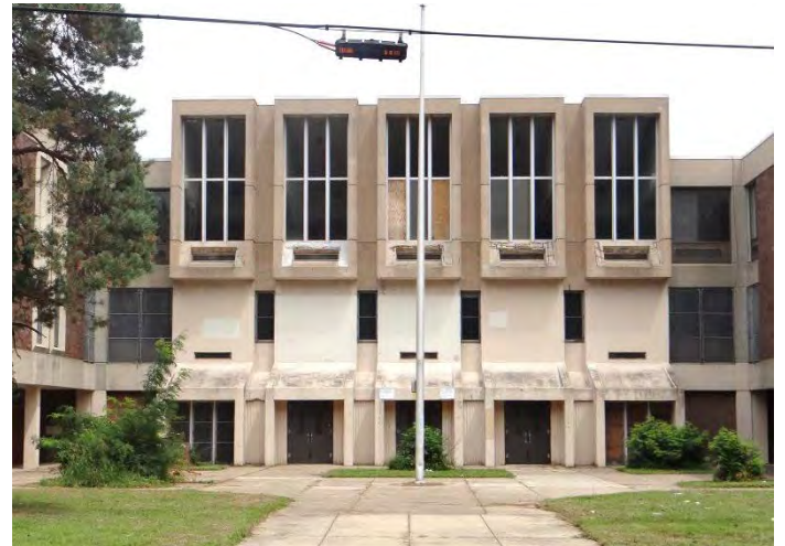
Photo 4: Looking NE at main entrance in center of main (SW) facade
