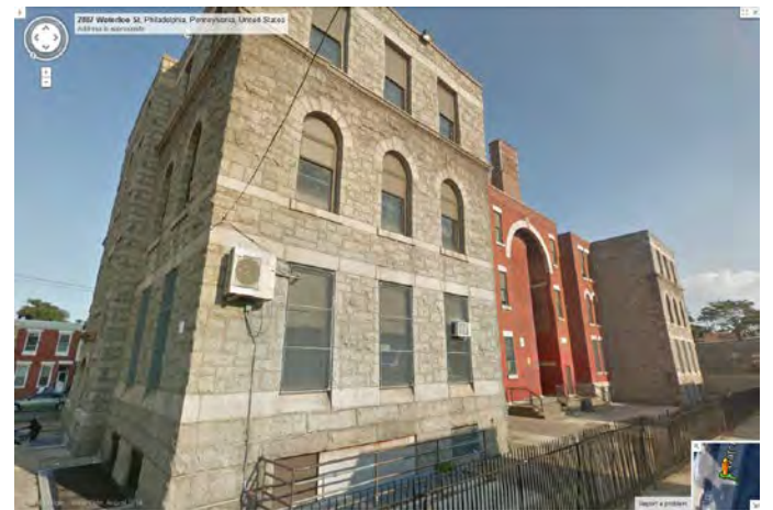
Photo 6: Looking SE at W façade. Source: Google maps
