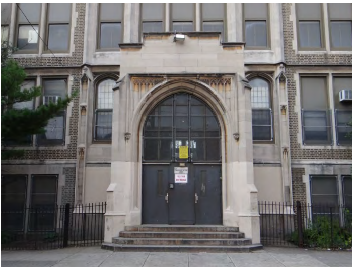
Photo 3: Looking W at E entrance
