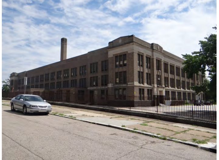
Photo 4: Looking SE at rear (NW, left) and SW facades
