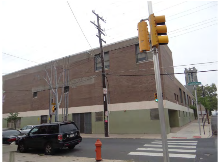
Photo 4: Looking SE at N (left) and W (right) facades
