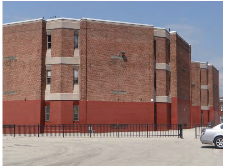
Photo 4: Looking NW at SE façade
