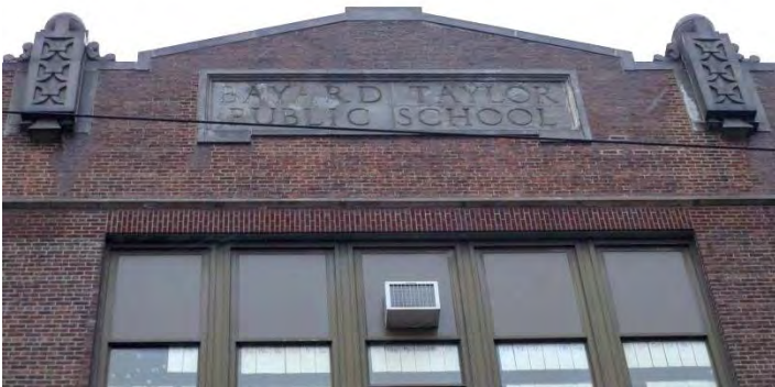
Photo 3: Looking W at nameplate on main (E) facade
