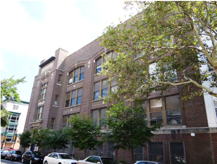
Photo 3: Looking SE at N façade
