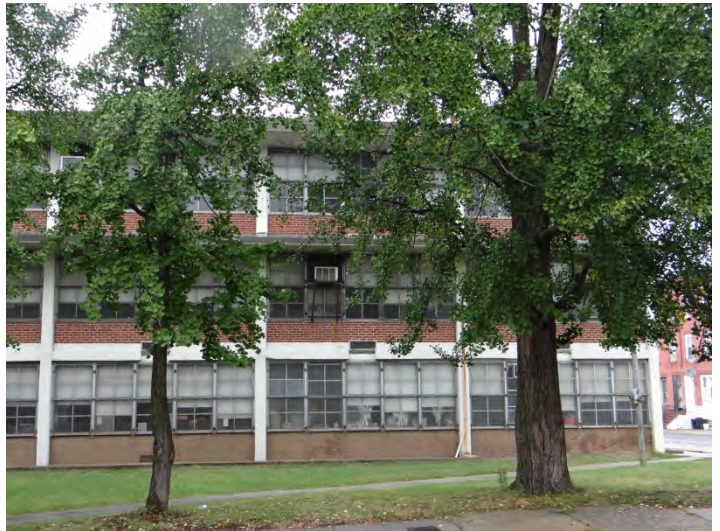
Photo 4: Looking N at E end of S façade
