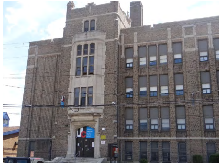
Photo 2: Looking SE at N entrance, main (NW) façade
