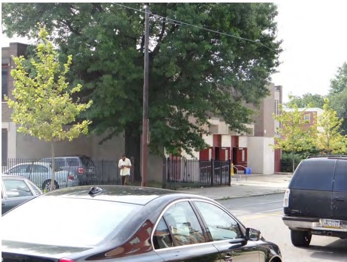
Photo 5: Looking SE at W façade
