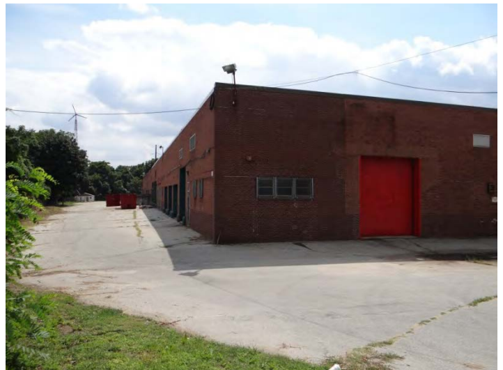
Photo 6: Looking SW at N (right) and E facades
