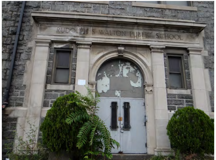
Photo 4: Looking N at entrance near E end of S façade
