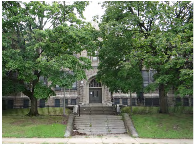
Photo 2: Looking NE at SW facade
