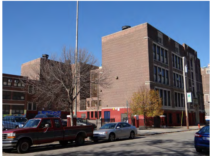
Photo 4: Looking NW at rear (S) facade
