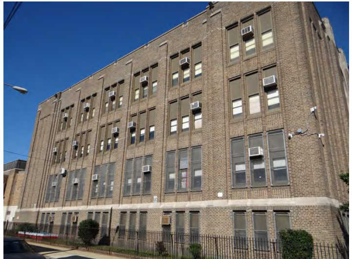
Photo 4: Looking NW at SE facade
