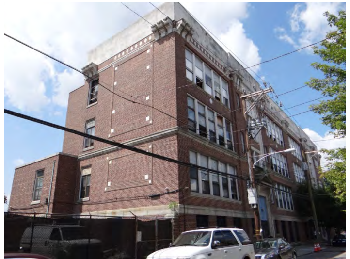
Photo 2: Looking SW at N (right) and E (left) facades
