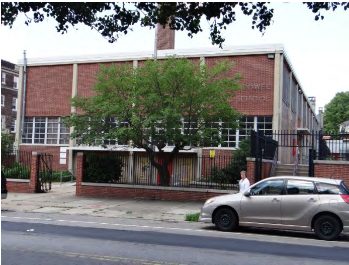
Photo 1: Looking N at main (S) facade
