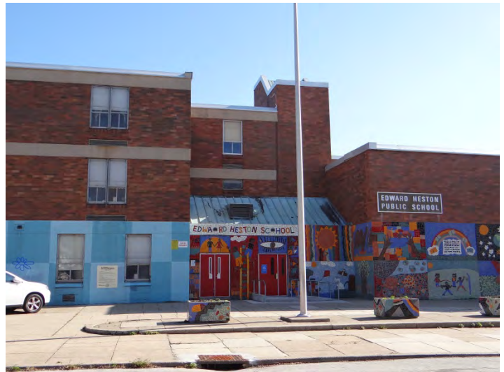
Photo 2: Looking E at main (W) façade entrance
