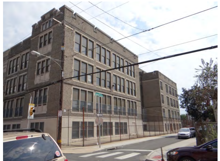
Photo 4: Looking E at W façade
