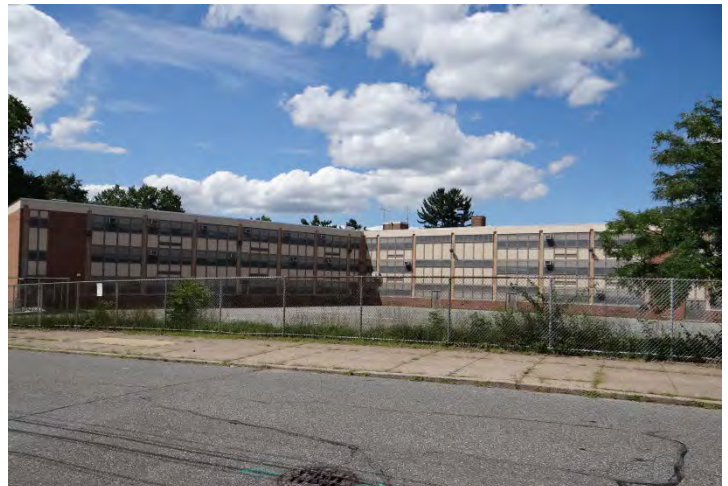
Photo 6: Looking NW at rear W (left) and S (right) facades
