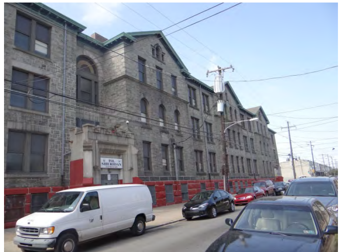
Photo 4: Looking SW at center of main (N) façade
