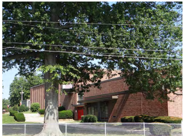
Photo 6: Looking NE at S end of main (SW) facade
