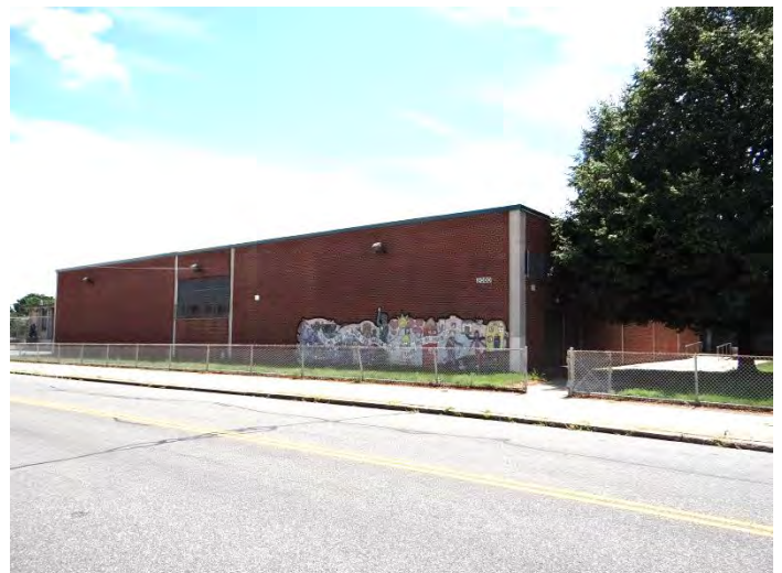
Photo 6: Looking SW at NE facade
