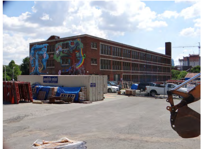
Photo 4: Looking E at rear (S) façade
