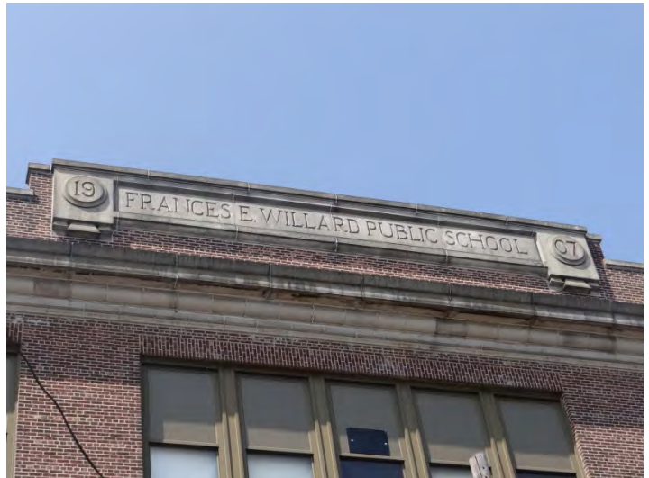
Photo 4: Looking W at name and datestone on NE facade
