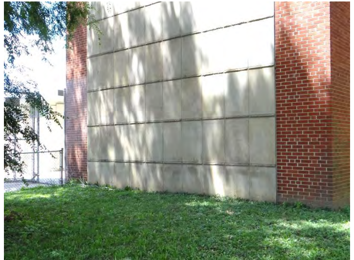
Photo 4: Detail, stone panel and brick wall construction
