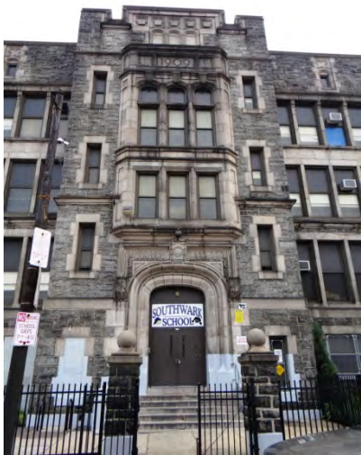
Photo 3: Looking E at main entrance on main (W) façade
