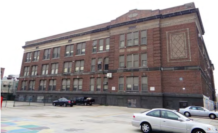
Photo 5: Looking NW at S façade
