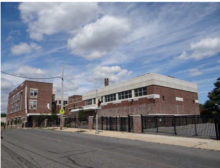
Photo 5: Looking NE at the W (left) and rear (S, right) facades
