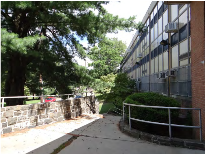
Photo 3: Looking E from main entrance on main (N) facade
