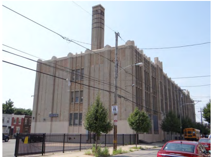
Photo 4: Looking SW at N (right) and E (center) facades
