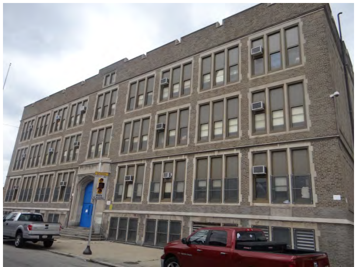
Photo 2: Looking N at main (SE) facade
