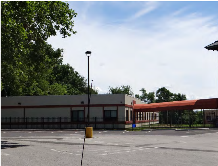
Photo 3: Looking E at modern additions to NE
