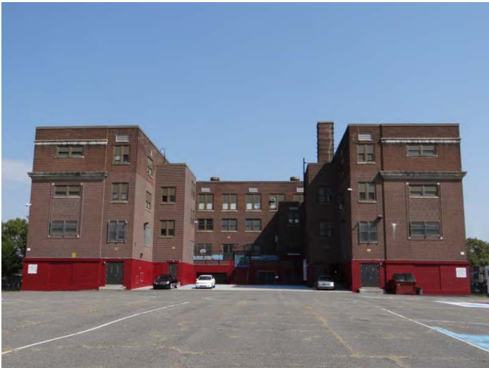
Photo 3: Looking N at S façade
