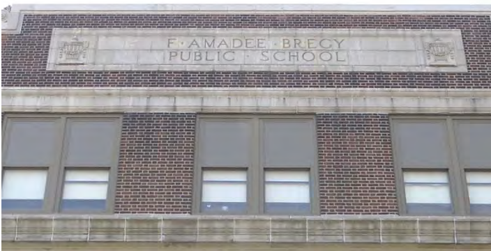
Photo 5: Looking S at N facade
