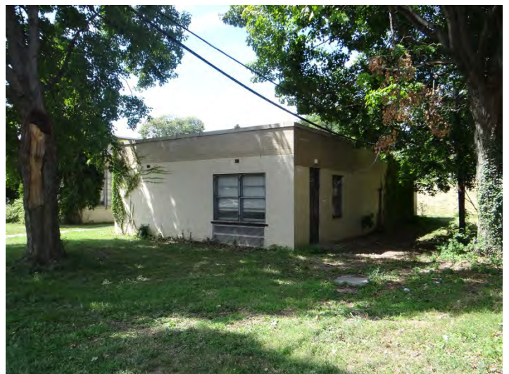
Photo 6: Looking NW at S façade of portable at N end of property
