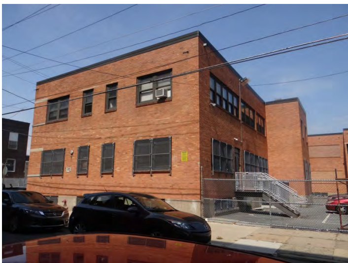
Photo 3: Looking W at SE (left) and NE (right) façades
