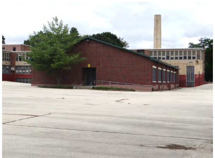
Photo 6: Looking W at NE facade
