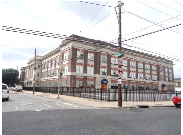
Photo 2: Looking W at main (SE, left) façade and NE (right) facades
