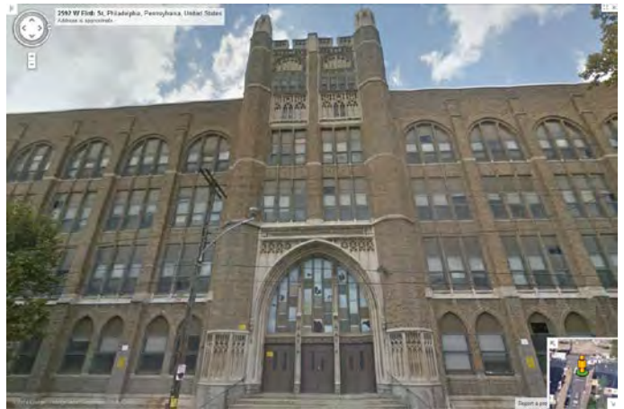
Photo 2: Looking N at main entrance on main (S) facade
