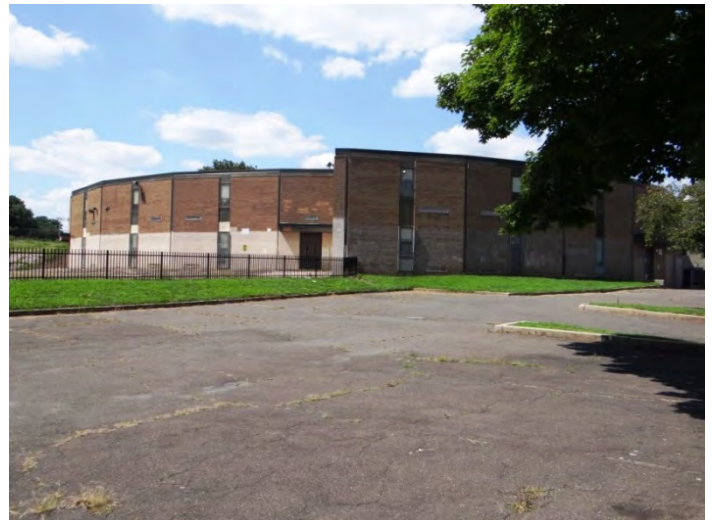
Photo 6: Looking W at E facade
