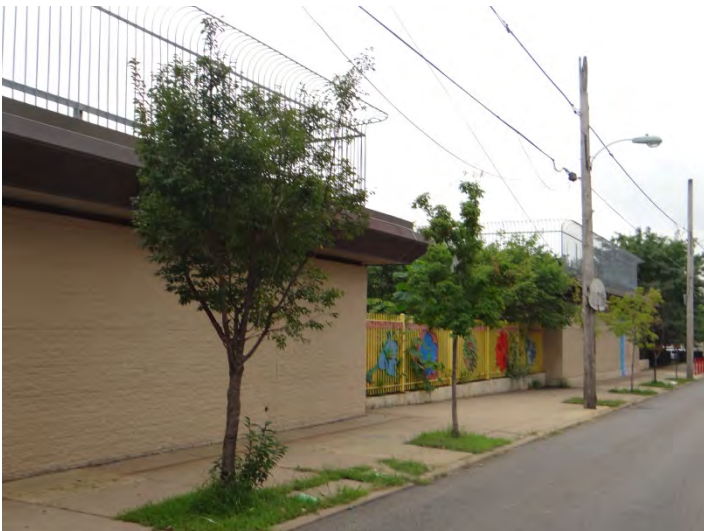
Photo 5: Looking SE at W facade
