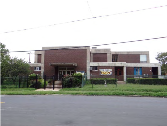
Photo 5: Looking W at NE facade
