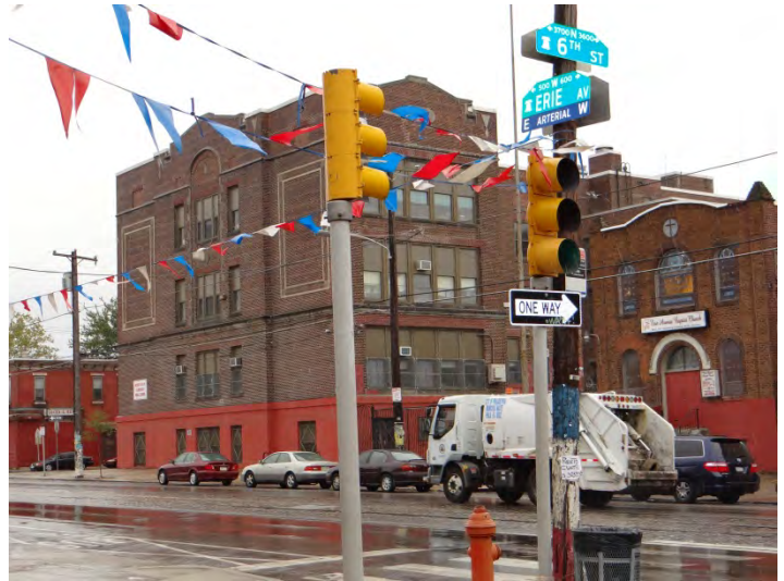
Photo 2: Looking SE at N (left) and main (E, right) facades
