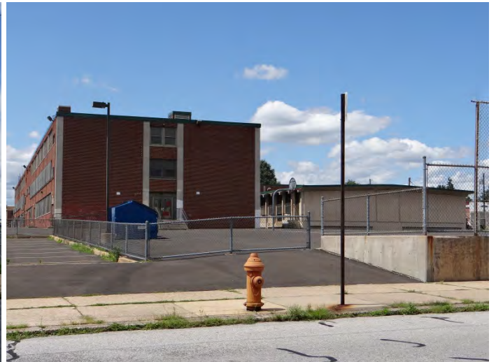
Photo 4: Looking NW at SE facade and portable
