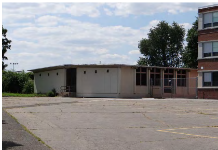
Photo 6: Looking SW at NE corner, rear building
