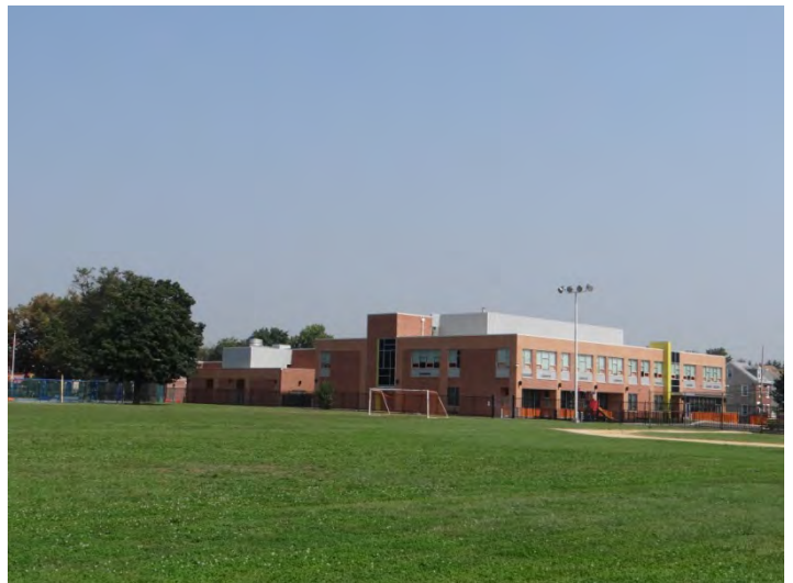
Photo 6: Looking NE at SW façade of recent addition
