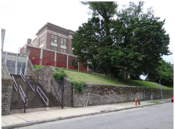
Photo 6: Looking W at NE facade
