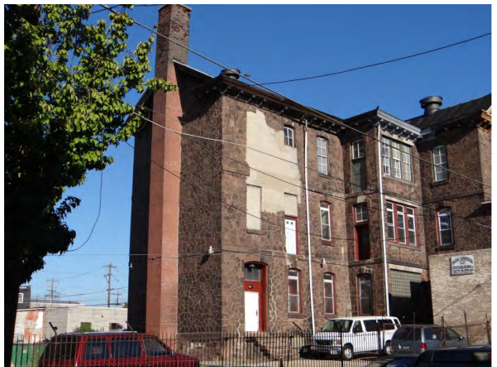
Photo 6: Looking NW at S half of E facade
