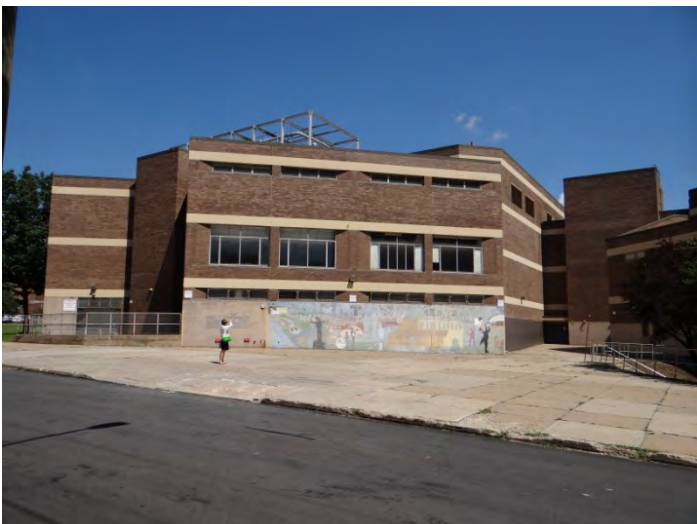
Photo 5: Looking NW at SW facade
