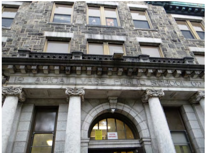
Photo 2: Looking E at W façade entrance
