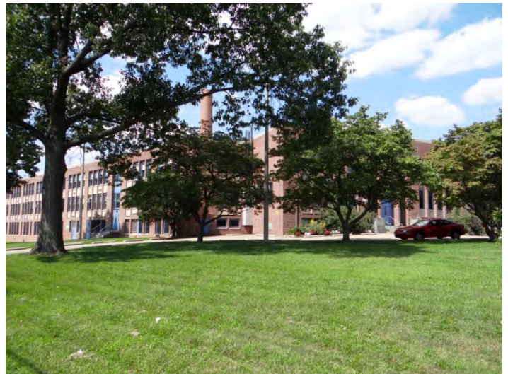
Photo 2: Looking NE at W (left) and main (SE) facades
