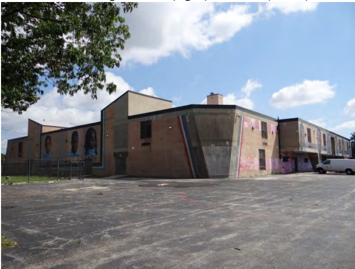
Photo 5: Looking NE at rear (S, right) and W (left) facade
