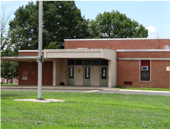
Photo 3: Looking W at main entrance on E facade
