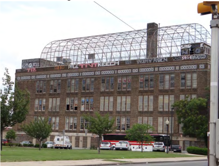
Photo 5: Looking S at N facade
