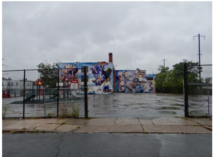
Photo 4: Looking SW at E facades
