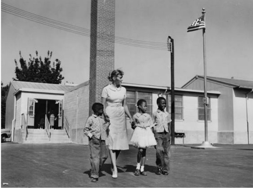
The Lehigh School, located at 31 st and Lehigh, was constructed entirely of portable classrooms. Photo, 1958. George D. McDowell Philadelphia Evening Bulletin Photographs, Urban Archives, Temple University.
