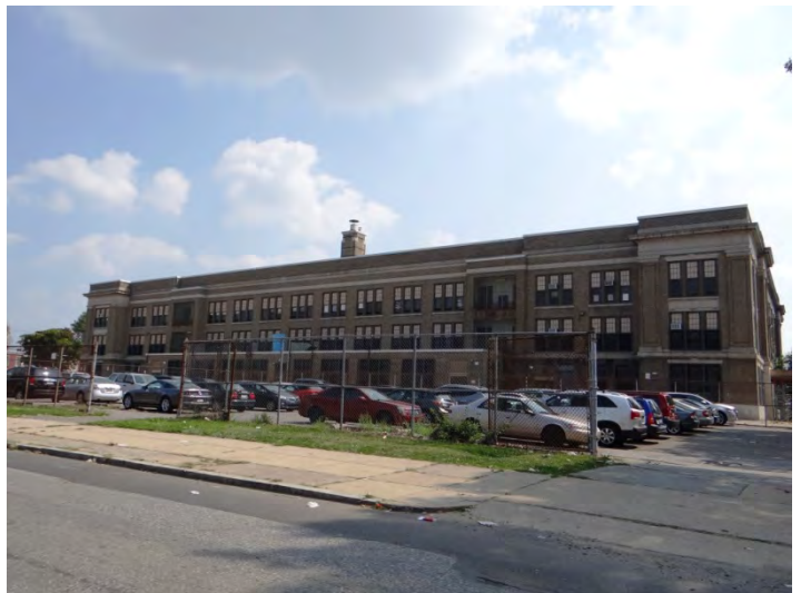
Photo 4: Looking S at N façade
