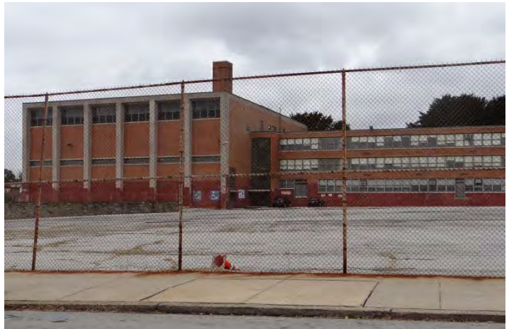
Photo 4: Looking NW at W end of SE facade
