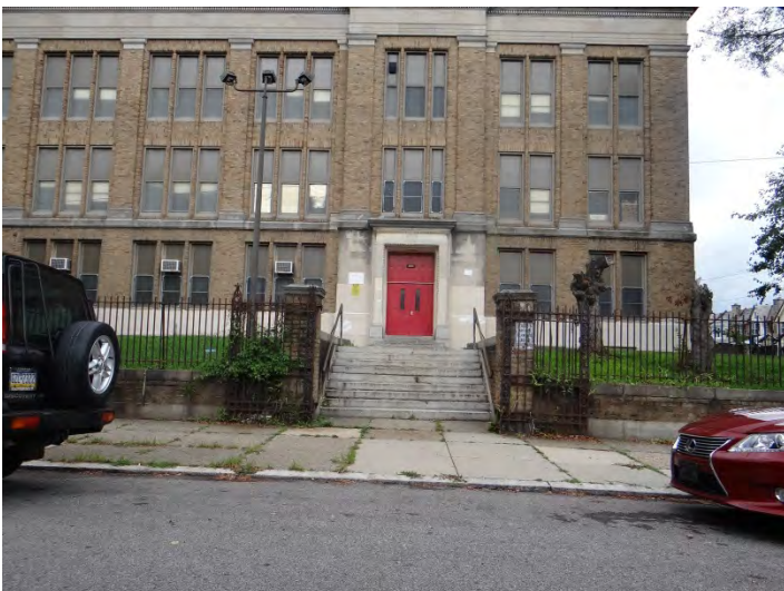
Photo 5: Looking W at N end of E façade
