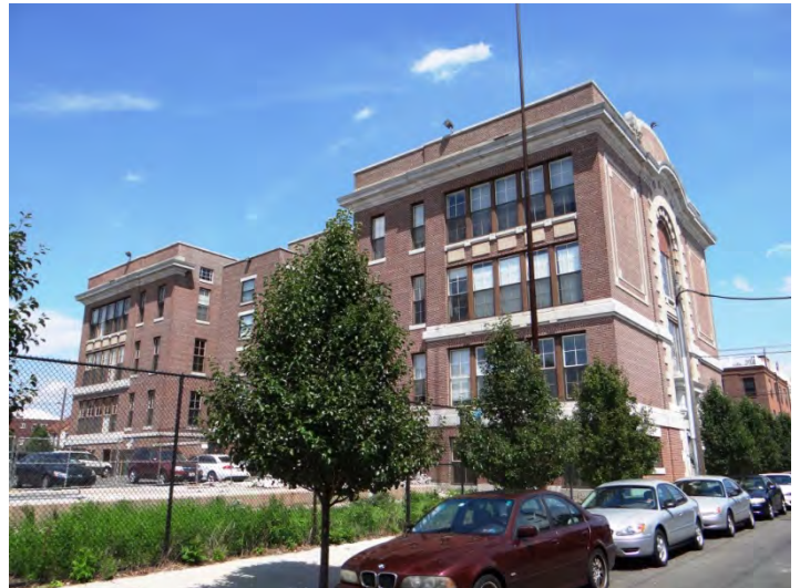
Photo 4: Looking NE at W facade
