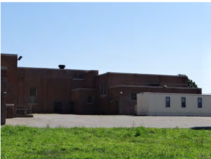
Photo 5: Looking N at SW façade
