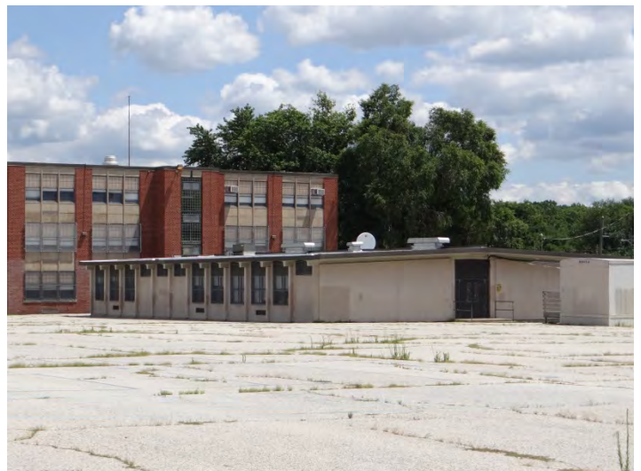
Photo 6: Looking NE at rear (NW) façade, S end
