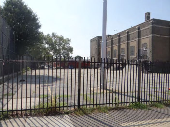
Photo 5: Looking SE at playground; rear (NE) facade at right
