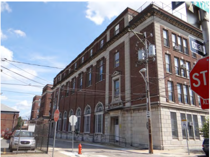
Photo 4: Looking E at N facade
