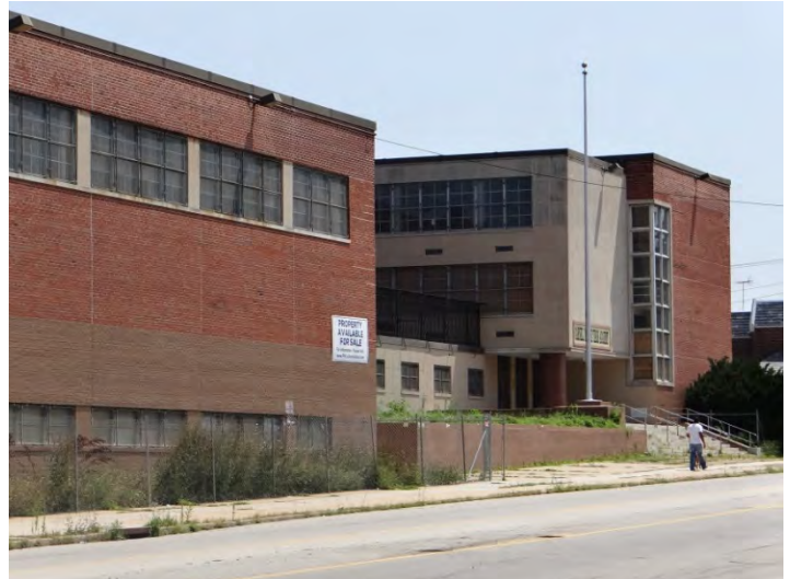
Photo 2: Looking SE at main (SW) facade
