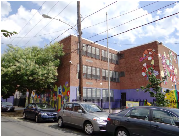
Photo 3: Looking SE at W façade
