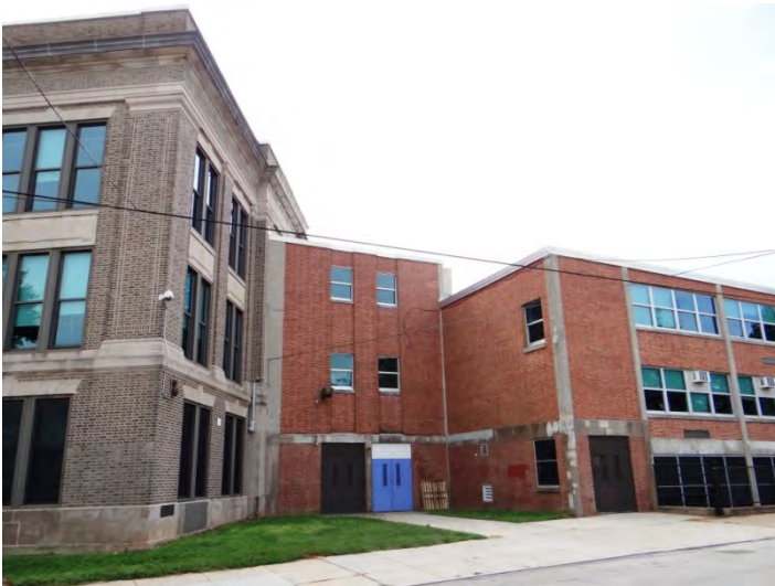
Photo 3: Looking S at addition hyphen on NW facade
