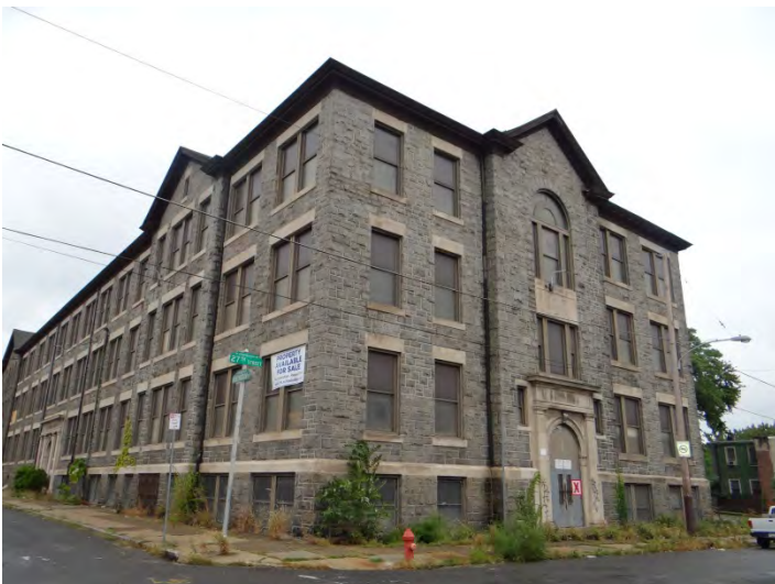
Photo 5: Looking NW at S (left) and E (right) facades
