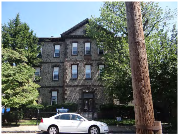
Photo 2: Looking NE at SW facade
