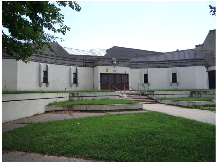
Photo 2: Looking SE at NW entrance
