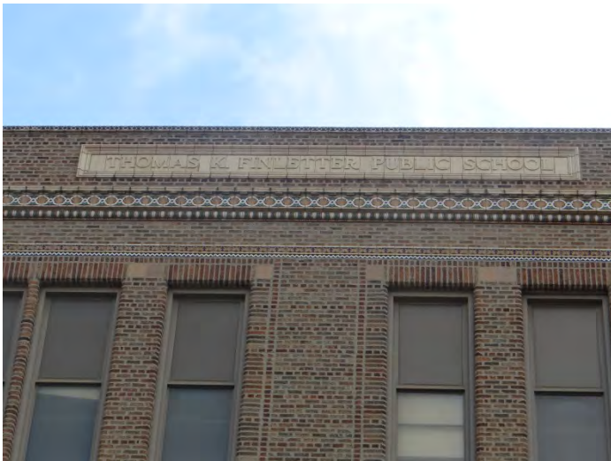
Photo 3: Looking E at nameplate on main (W) façade
