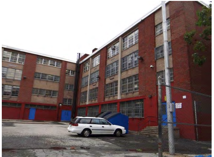
Photo 4: Looking SE at N facade
