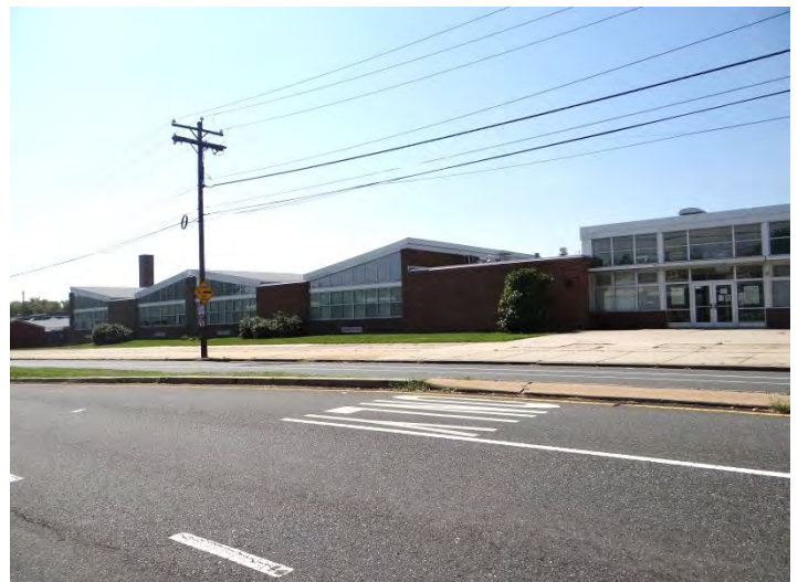
Photo 6: Looking SW at building at N corner of lot
