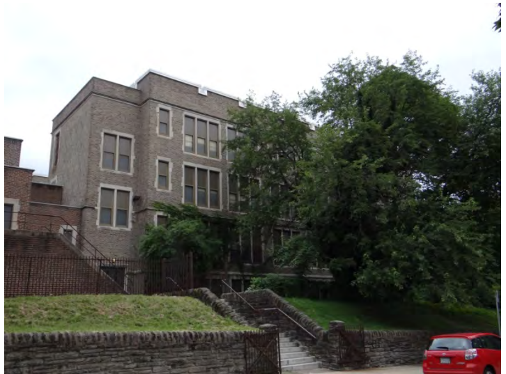
Photo 4: Looking E at SW facade
