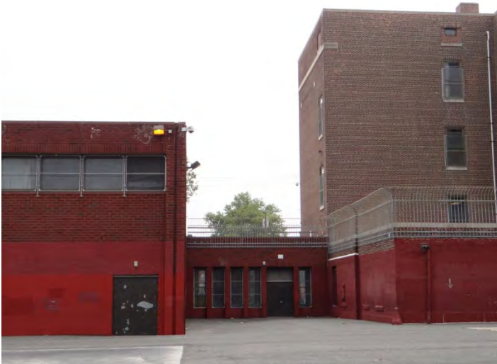
Photo 5: Looking N at addition hyphen
