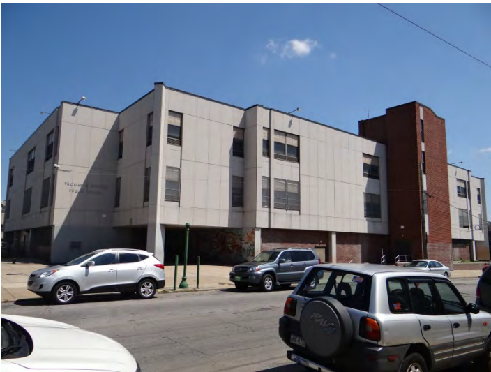
Photo 3: Looking NE at SW façade
