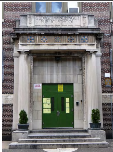
Photo 2: Looking N at main entrance on main (S) facade
