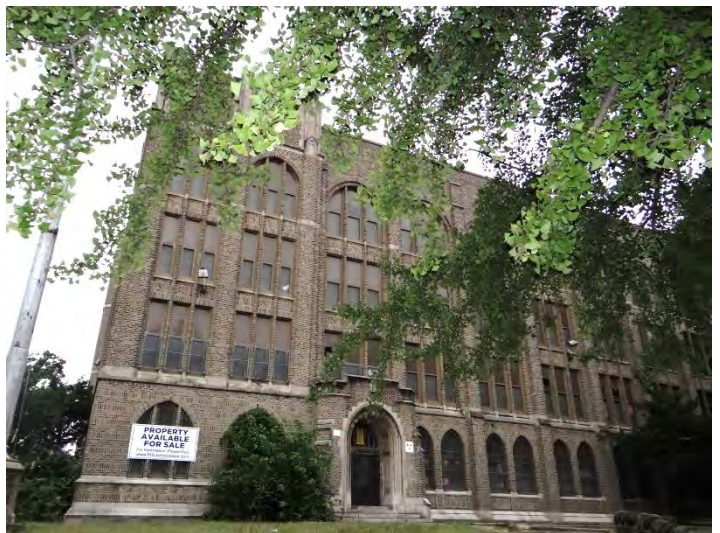
Photo 6: Looking W at E facade
