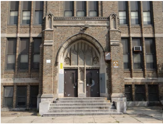
Photo 1: Looking N at main (S) facade
