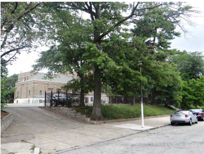
Photo 5: Looking N at rear (SW) facade
