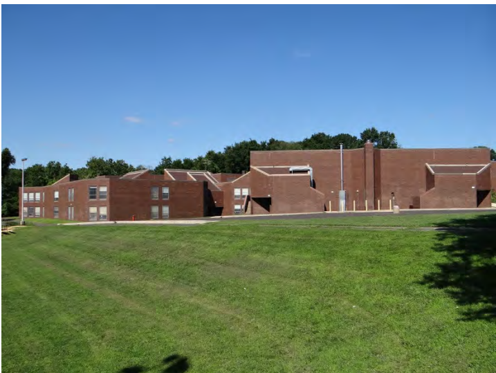
Photo 5: Looking W at S end of E facade
