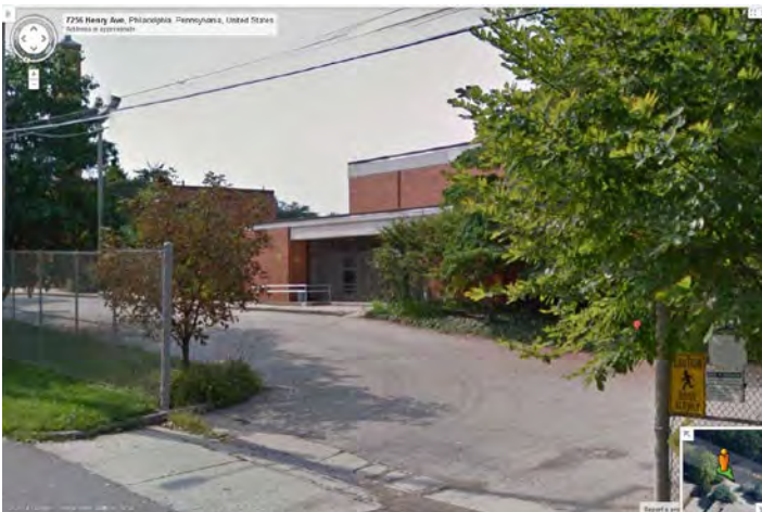
Photo 1: Looking SE at main (NE) façade of main building in center of complex on SW side of Henry Ave.
