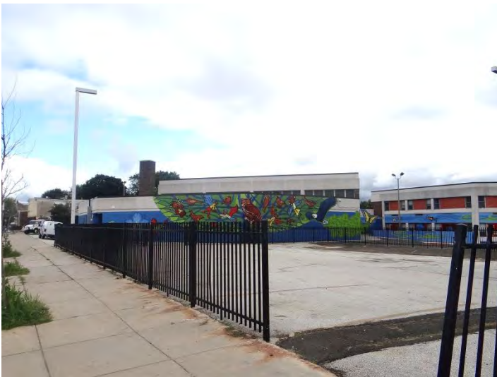
Photo 3: Looking NW at E façade
