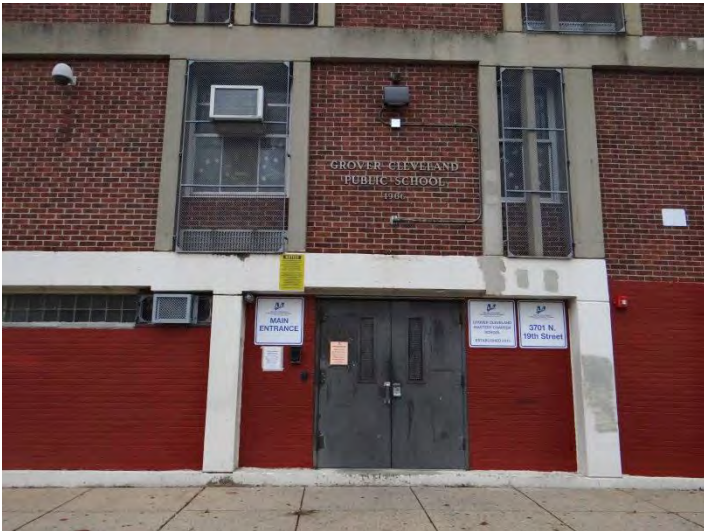
Photo 3: Looking E at entrance on W façade of addition
