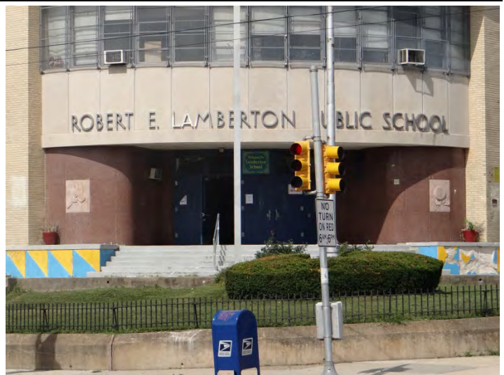
Photo 2: Detail, main entrance, E corner
