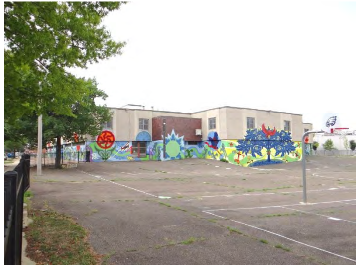
Photo 4: Looking SW at rear (N) façade
