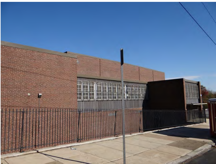
Photo 5: Looking NE at S façade of addition
