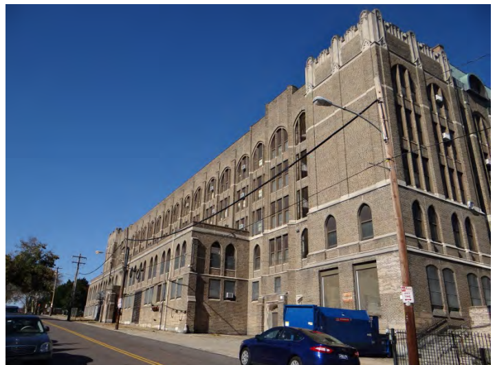
Photo 6: Looking NW at rear (S) façade of main building
