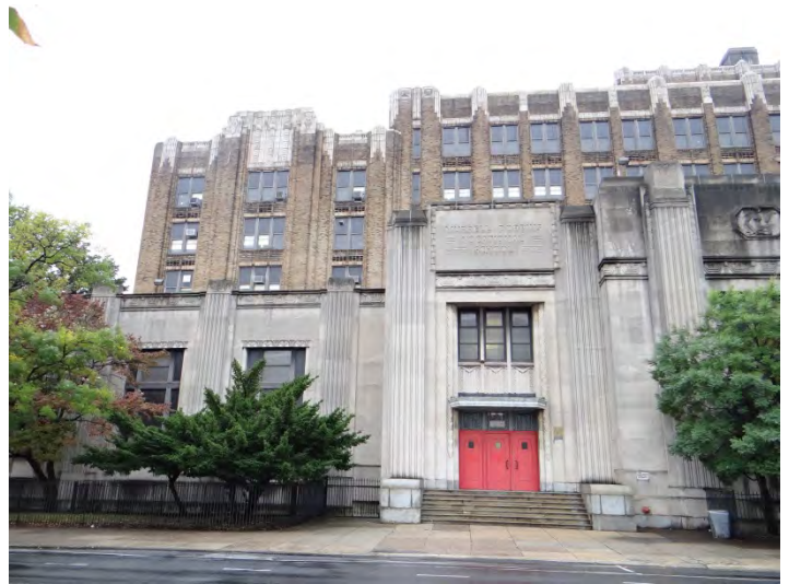
Photo 2: Looking S at E end of main (N) façade
