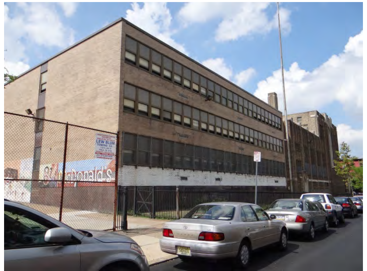
Photo 2: Looking N at S (left) and E (center) facades
