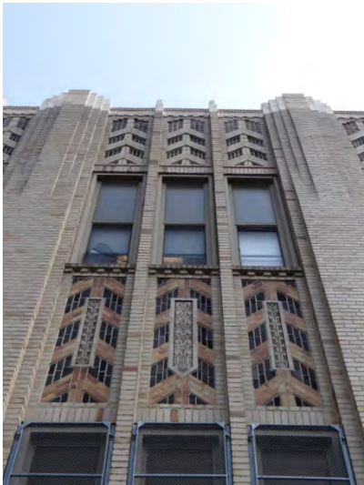
Photo 3: Looking S at N façade detailing
