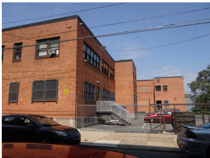
Photo 4: Looking NW at rear (NE) facade
