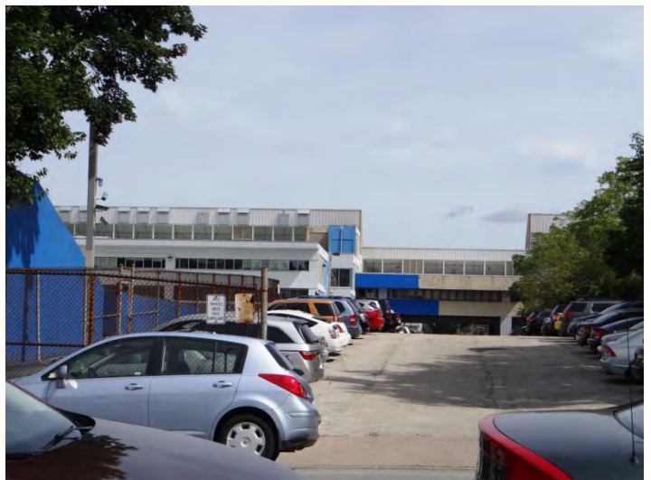
Photo 6: Looking NE at E end of SW facade
