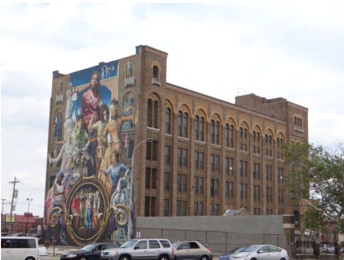
Photo 5: Looking NE at W (left) and main (S) facades
