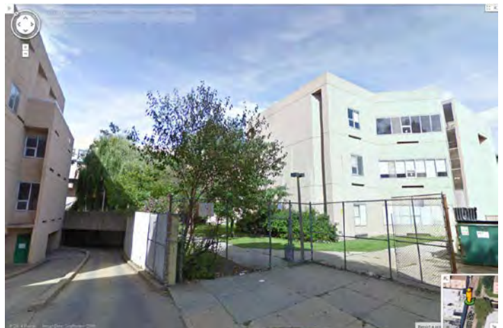
Photo 6: Looking N at SW quadrant
