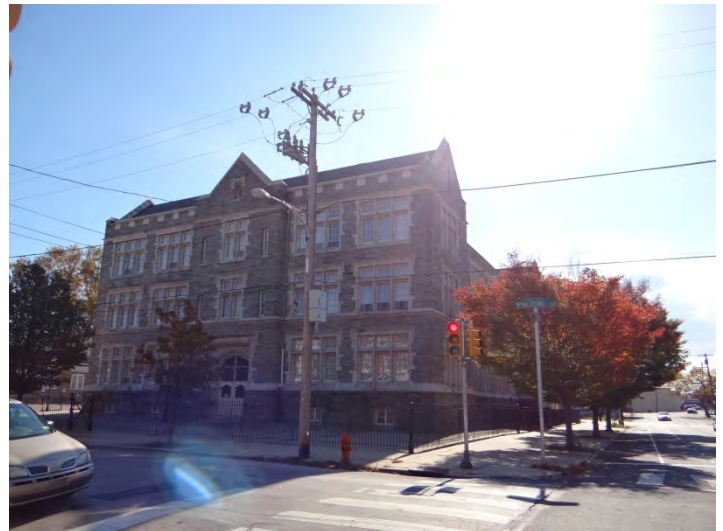
Photo 6: Looking S at N facade
