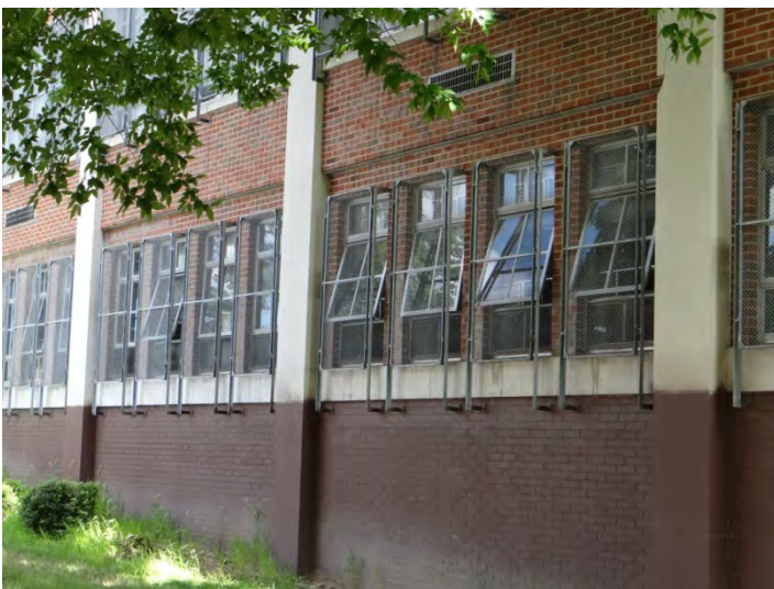
Photo 5: Detail, NW and SW façade windows
