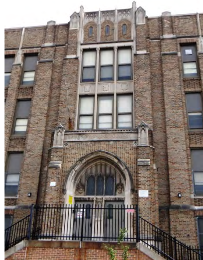
Photo 2: Looking NE at entrance on main (SW) facade
