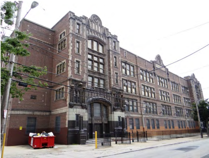
Photo 3: Looking NW at S end of main (E) façade
