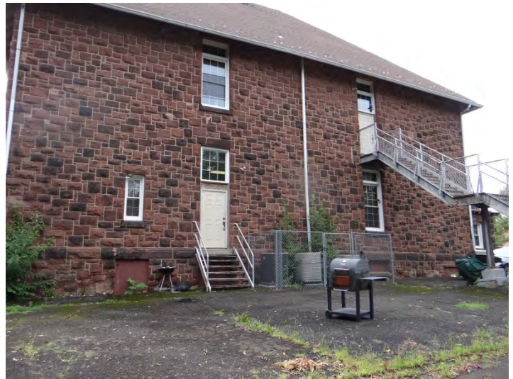
Photo 4: Looking SE at rear (NW) facade
