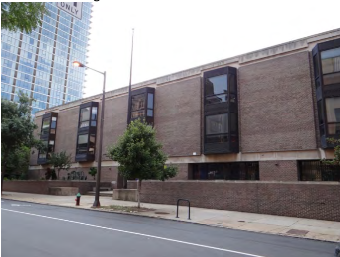
Photo 5: Looking S at main (N) facade
