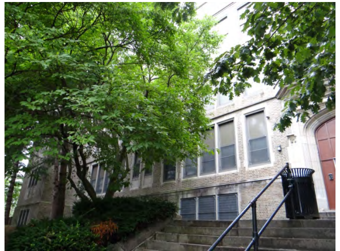
Photo 2: Looking W at S end of (main) SE facade
