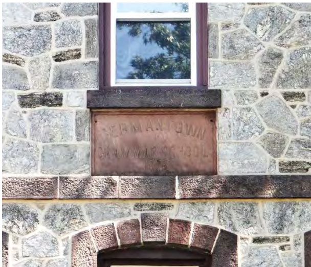
Photo 3: Detail, SW façade
