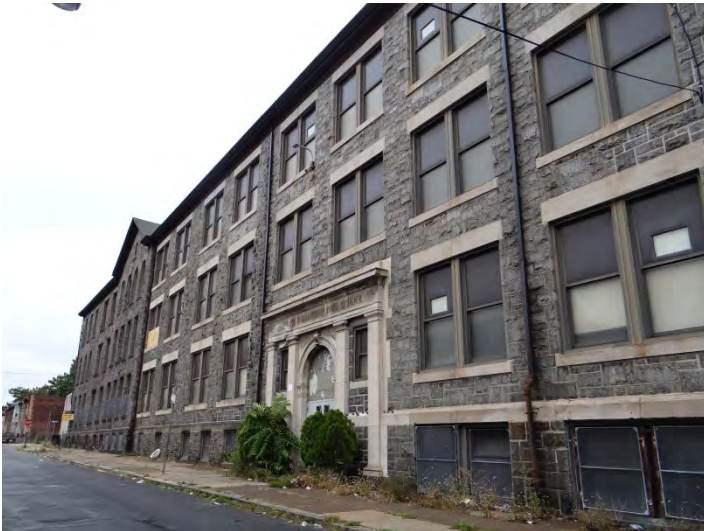
Photo 3: Looking NW at S façade near center of building
