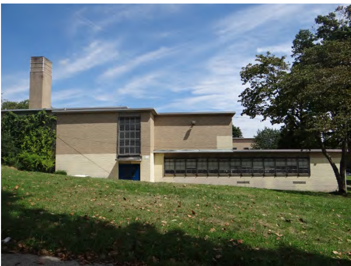
Photo 5: Looking NE at SW facade
