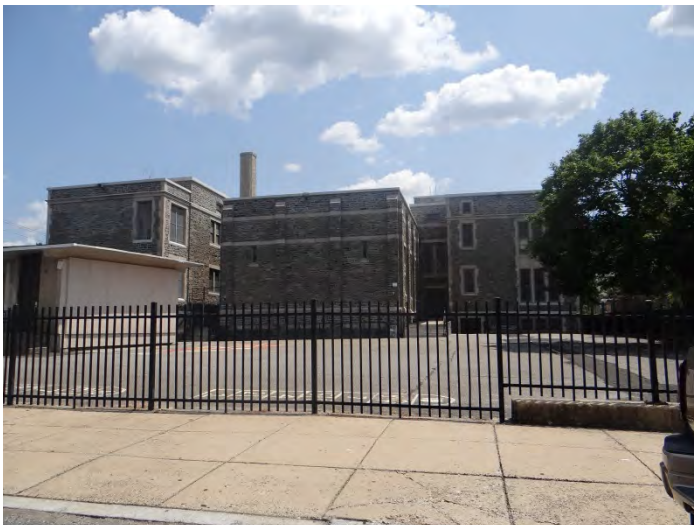
Photo 5: Looking SE at rear (NW) facade
