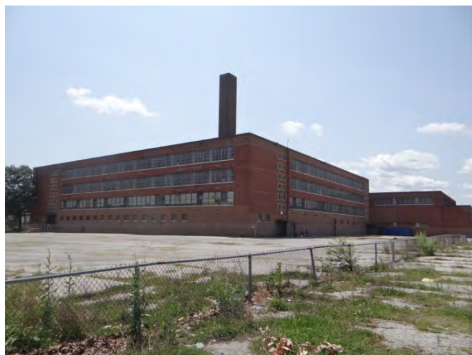
Photo 5: Looking S at rear (NE, left) and NW (right) facade
