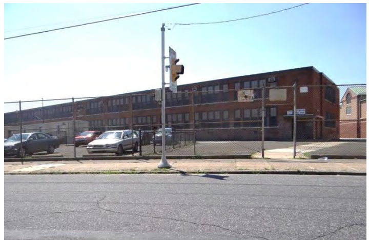
Photo 6: Looking NE at N end of SW facade
