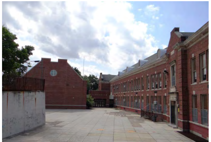
Photo 2: Looking W at SE facade
