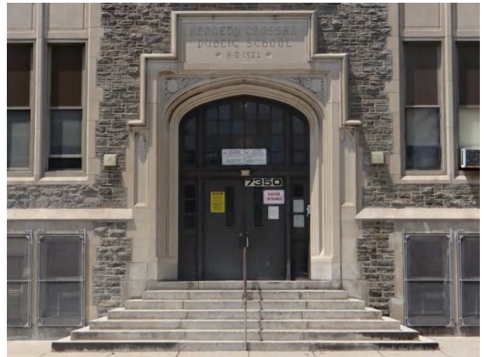
Photo 4: Looking NW at main entrance, main NW facade
