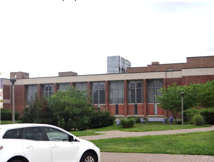
Photo 5: Looking S at center of main (NE) façade
