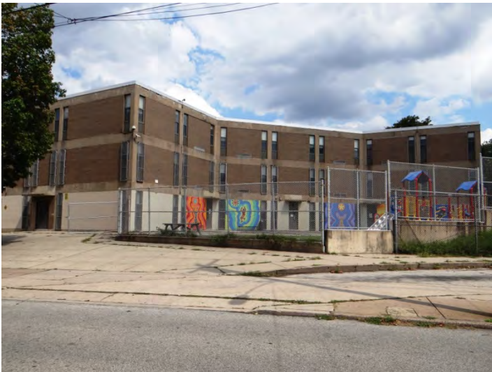
Photo 3: Looking NE at SW facade
