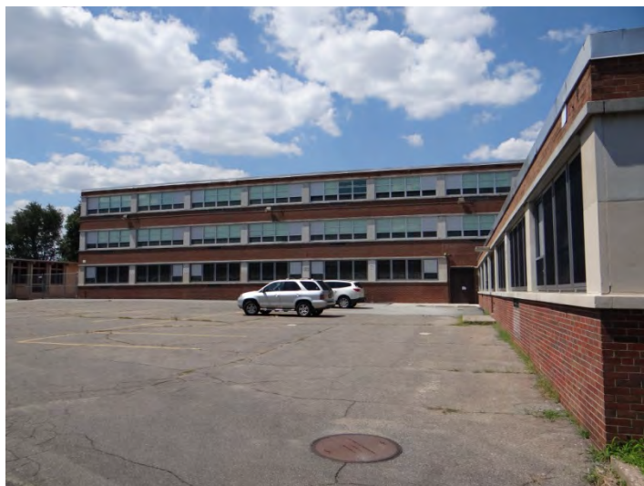
Photo 4: Looking NW at SE facades
