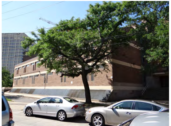
Photo 2: Looking SE at NE facade
