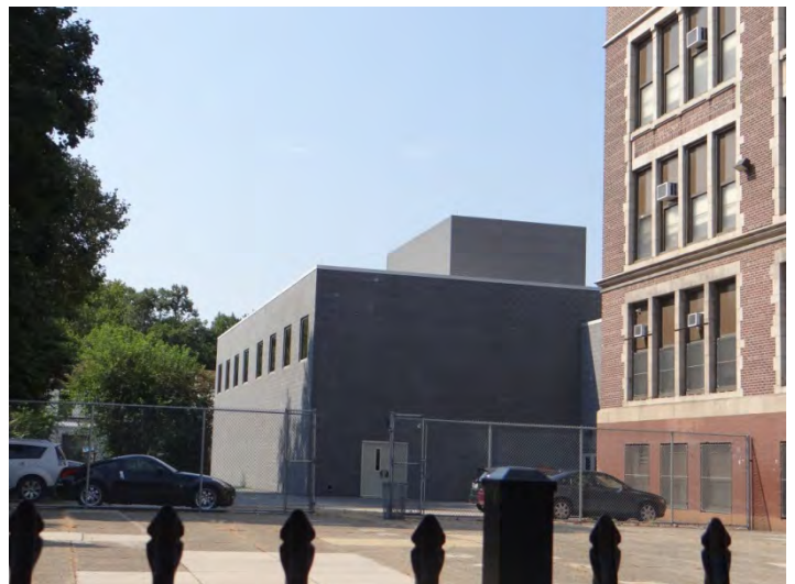
Photo 6: Looking S at E façade
