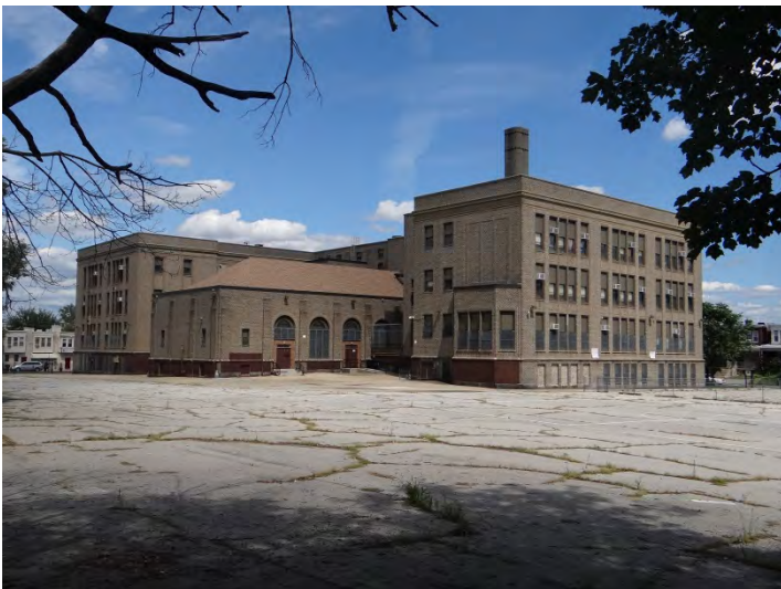
Photo 5: Looking NE at rear (W, left) and S (right) facades
