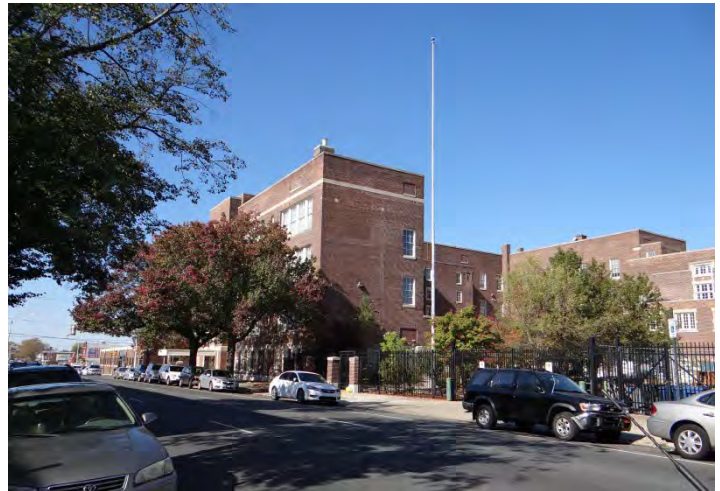
Photo 4: Looking NW at S (left) and E (right) facades
