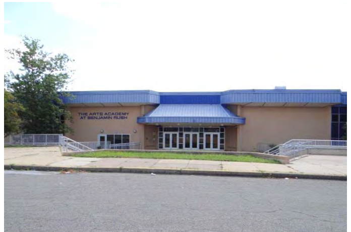
Photo 2: Looking E at main (W) facade
