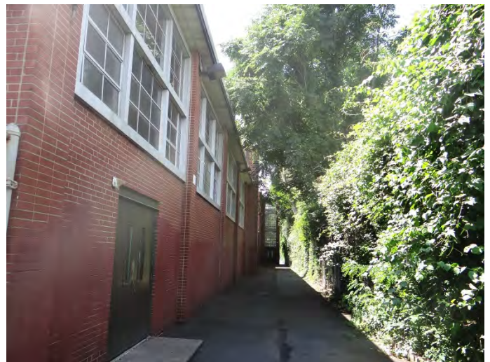
Photo 4: Looking SW at NW facade
