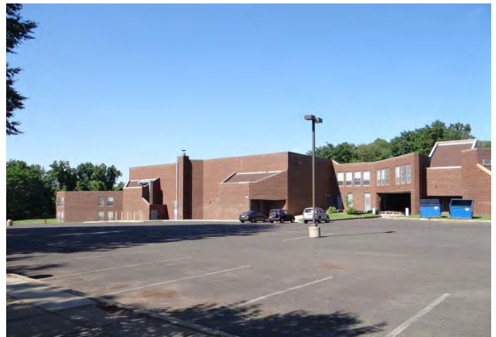
Photo 4: Looking W at E facade
