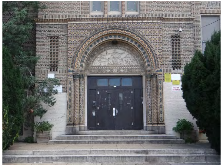
Photo 2: Looking E at entrance on main (W) façade
