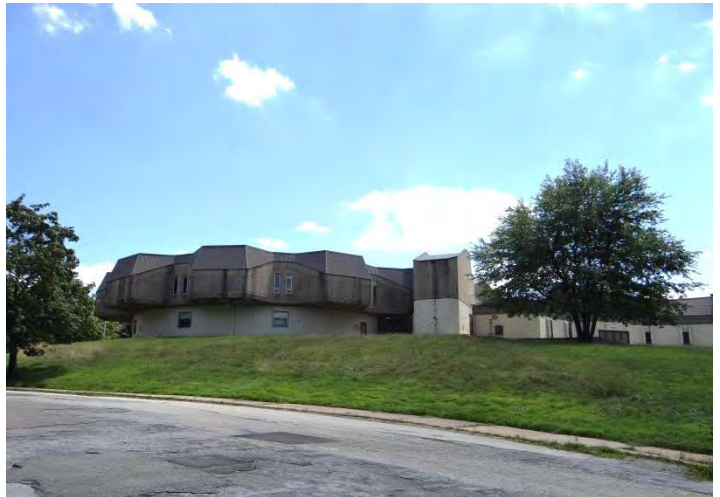
Photo 4: Looking E at NE corner of main (NW) facade
