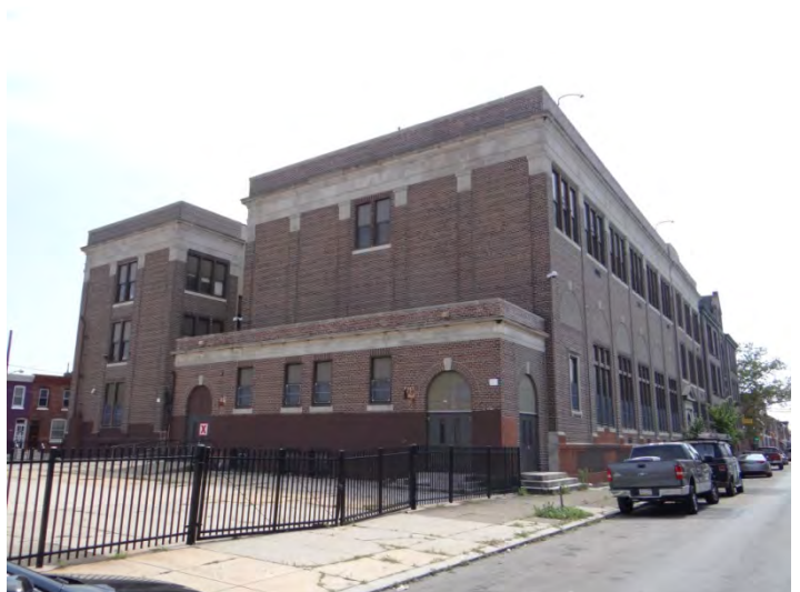
Photo 6: Looking SE at N (center) and W facades
