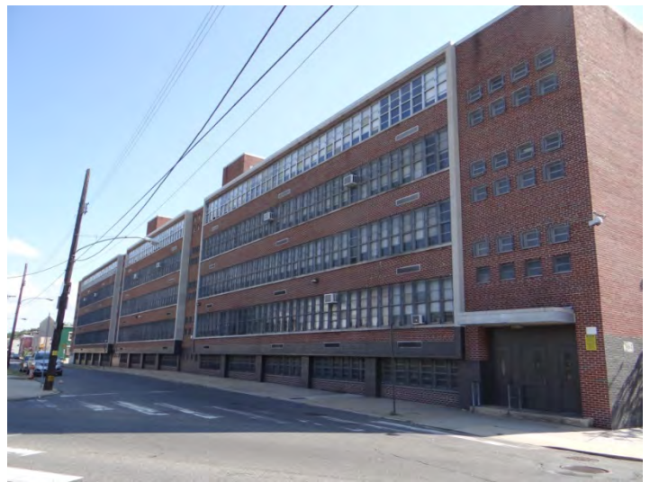
Photo 2: Looking NE at W facade
