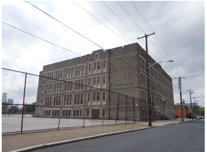
Photo 4: Looking SW at E façade (left) and main (N, right) façade
