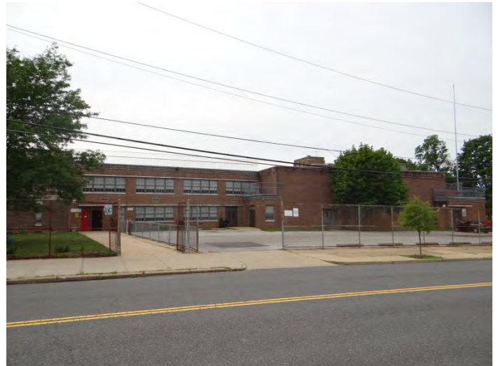
Photo 4: Looking E at center of NW facade
