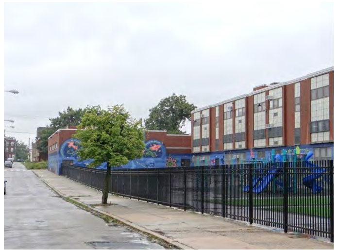
Photo 2: Looking SW at E façade
