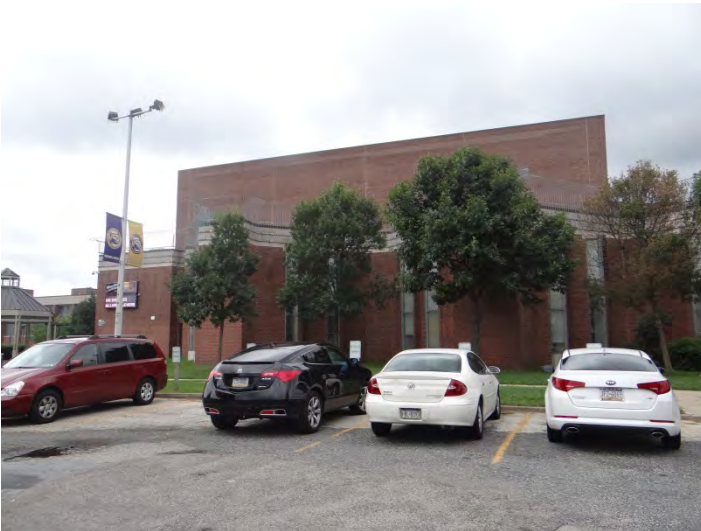
Photo 3: Looking SW at angled walls near NW corner of main (NE) facade
