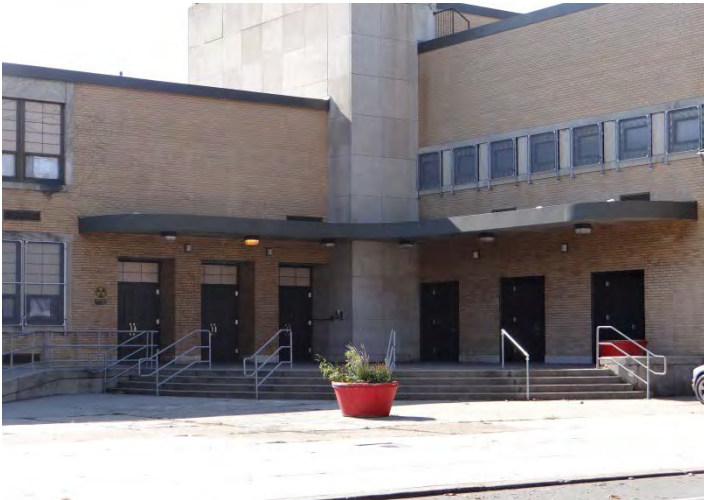
Photo 3: Looking SW at main entrance on main (N) facade
