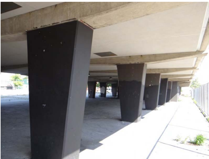
Photo 5: Looking N below N end of main wing
