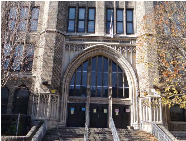
Photo 3: Looking W at entrance on main (E) façade
