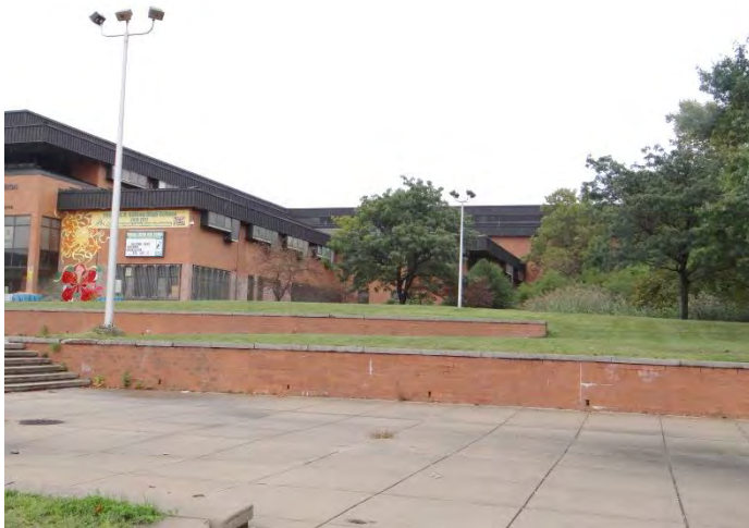
Photo 3: Looking N at S façade
