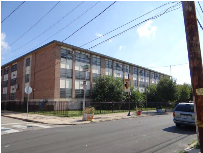
Photo 3: Looking NE at main (S) facade
