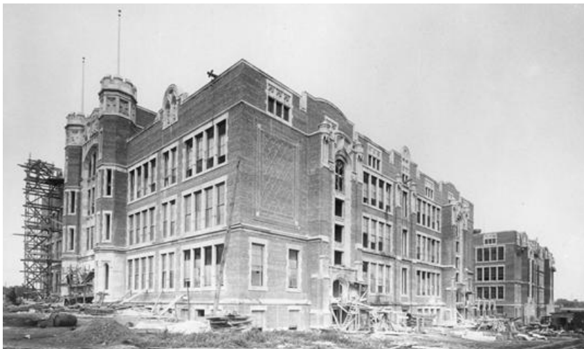
Construction of West Philadelphia High School, designed by SDP's chief architect Henry deCoursey Richards and completed in 1912. Philadelphia Department of Records, 1912.
