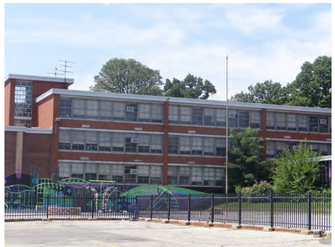
Photo 2: Looking SW at center of main (E) facade
