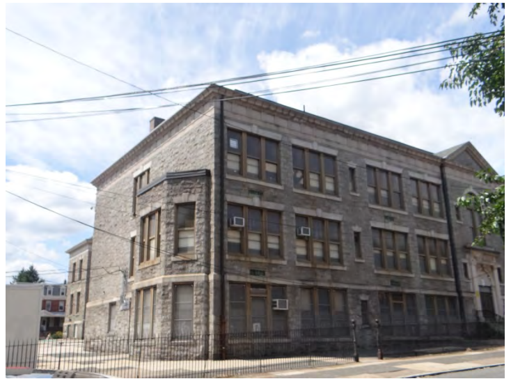
Photo 4: Looking NW at S (left) and E (right) facades
