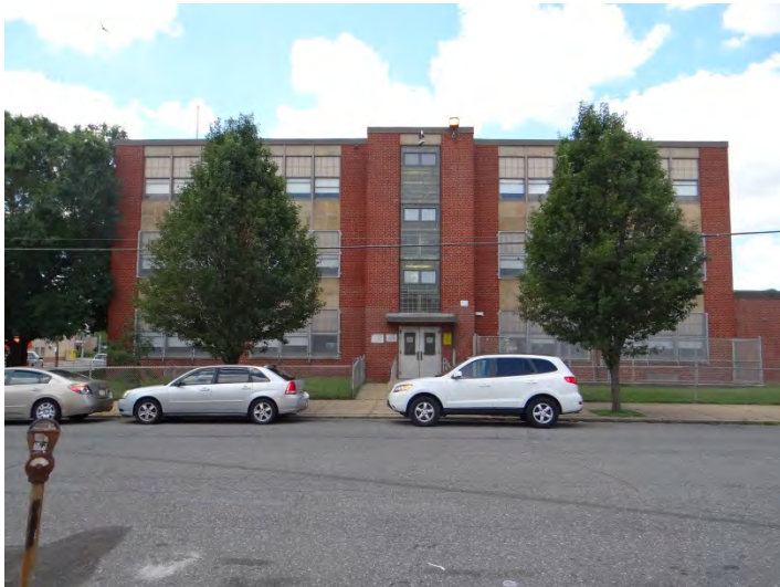
Photo 3: Looking S at NE façade
