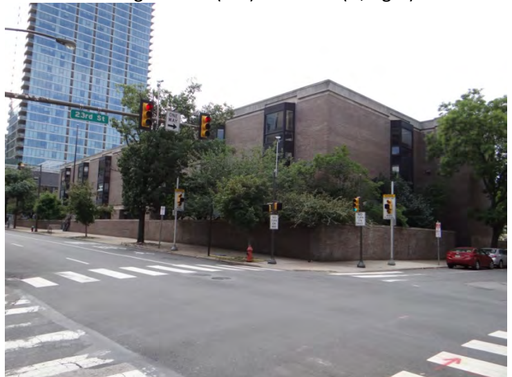
Photo 6: Looking SE at main (N) facade
