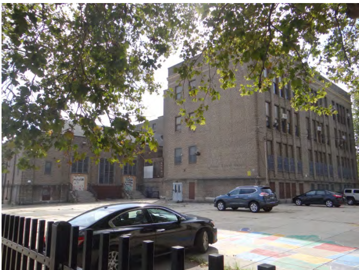
Photo 5: Looking SW at E façade
