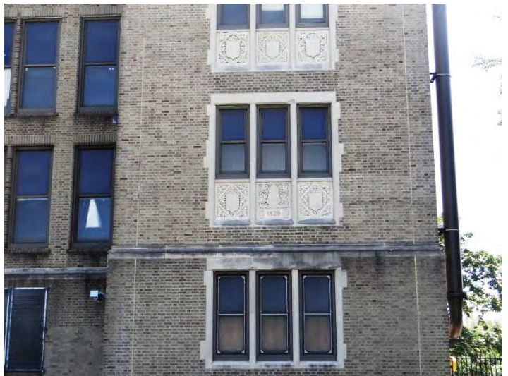
Photo 4: Detail, end bay, main (NW) façade
