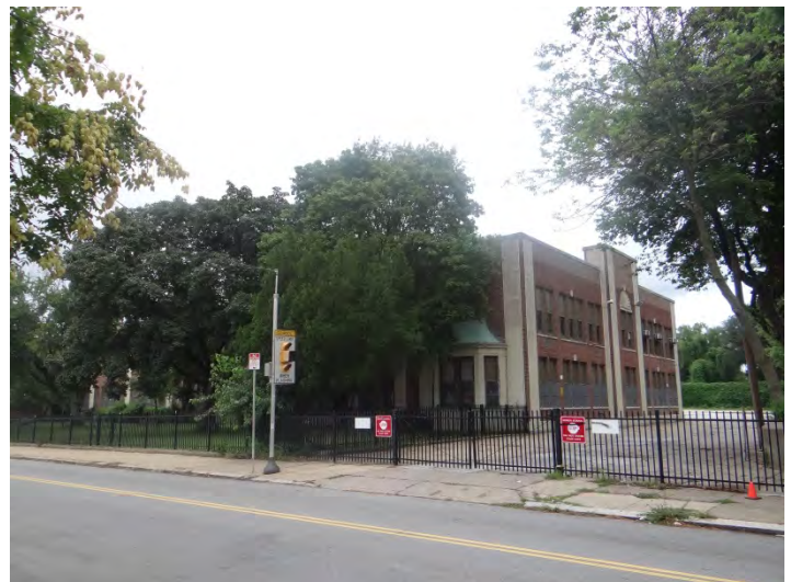
Photo 6: Looking NW at E facade
