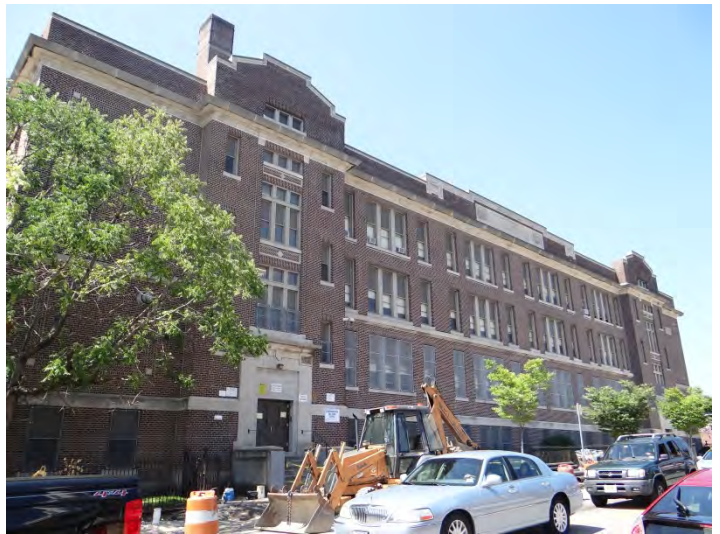
Photo 2: Looking W at N facade
