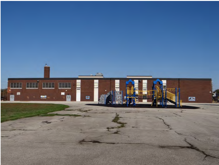
Photo 3: Looking N at rear (S) façade
