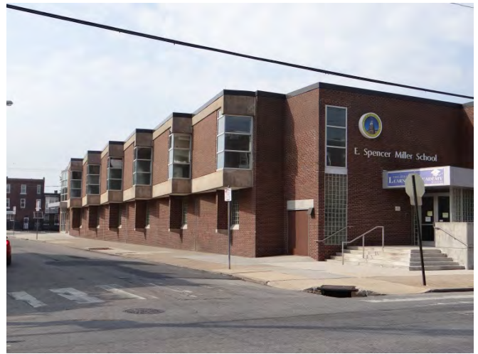
Photo 2: Looking S at E façade
