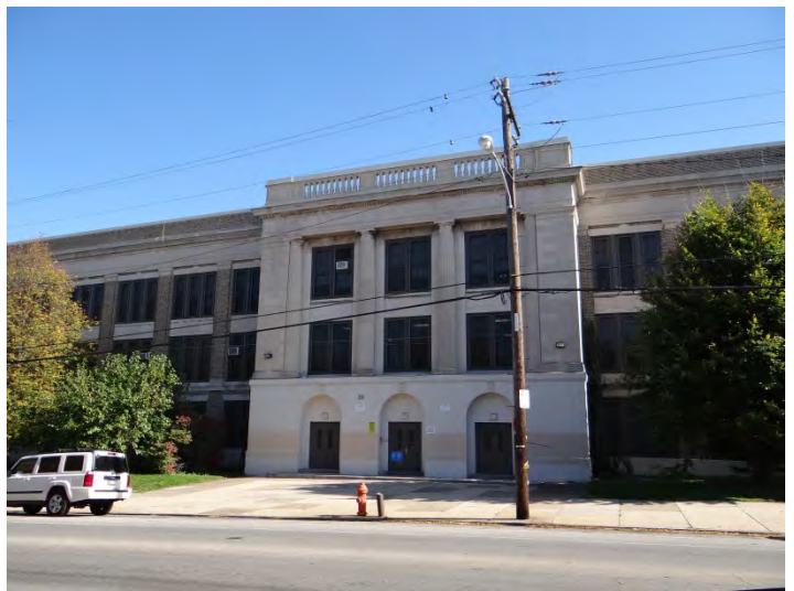
Photo 2: Looking E at main (W) facade
