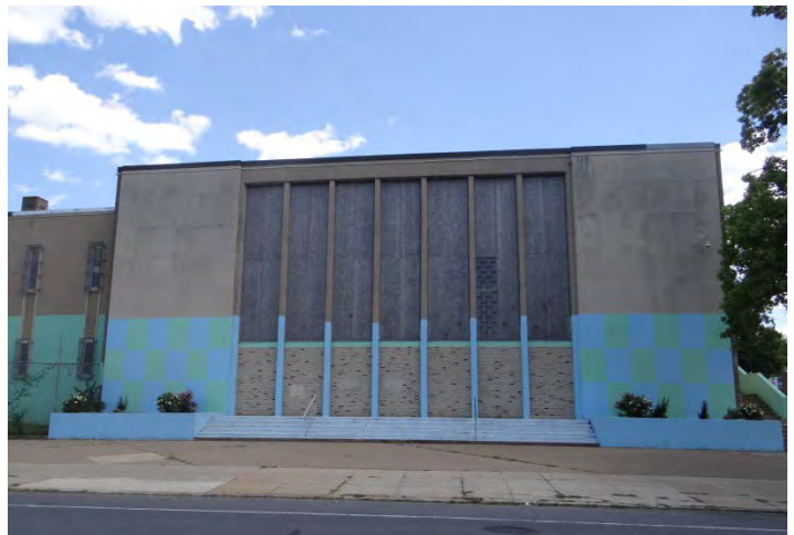
Photo 6: Looking E at W façade of 1960s addition
