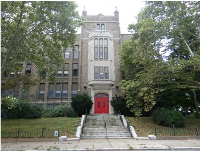
Photo 3: Looking SW at entrance at W end of NE facade
