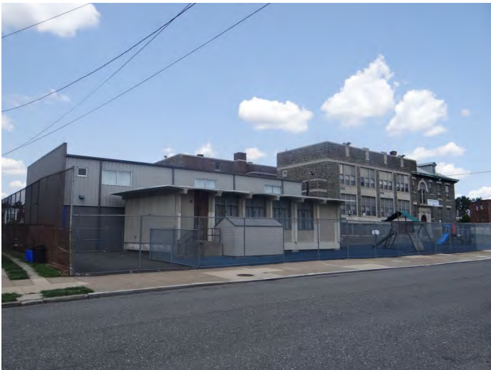
Photo 5: Looking N at S end of SE facade
