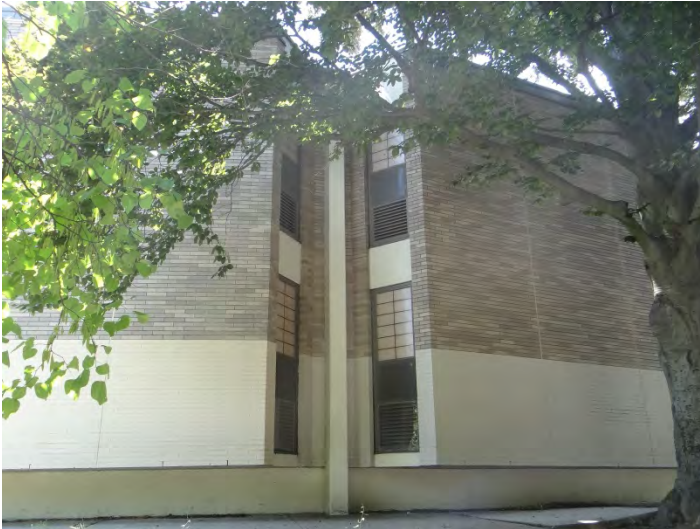
Photo 3: Typical window bay
