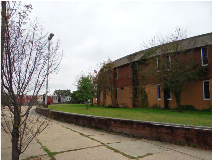
Photo 3: Looking E at N facade
