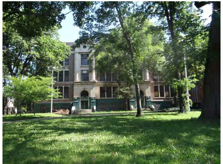
Photo 6: Looking NE at SW façade, W end
