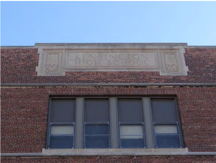
Photo 3: Looking NE at main (SW) façade
