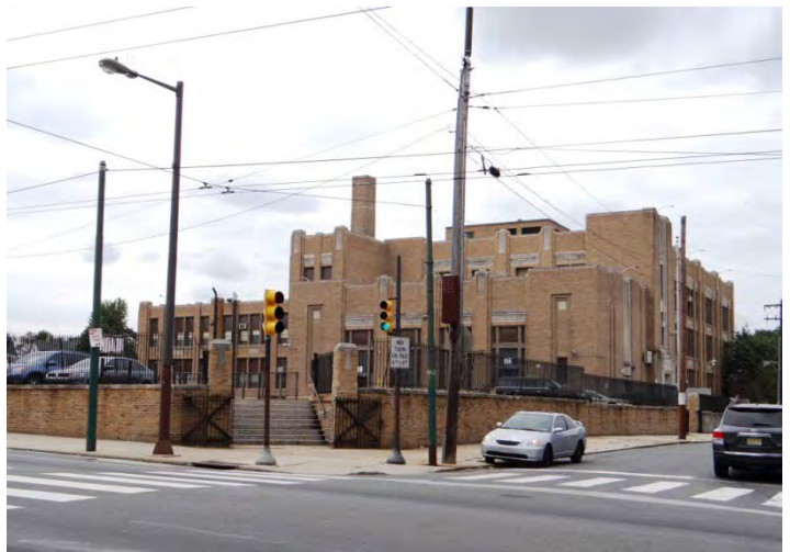
Photo 6: Looking NW at SE facade
