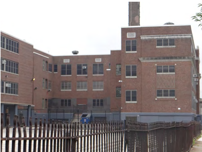
Photo 5: Looking S at rear (N) facade
