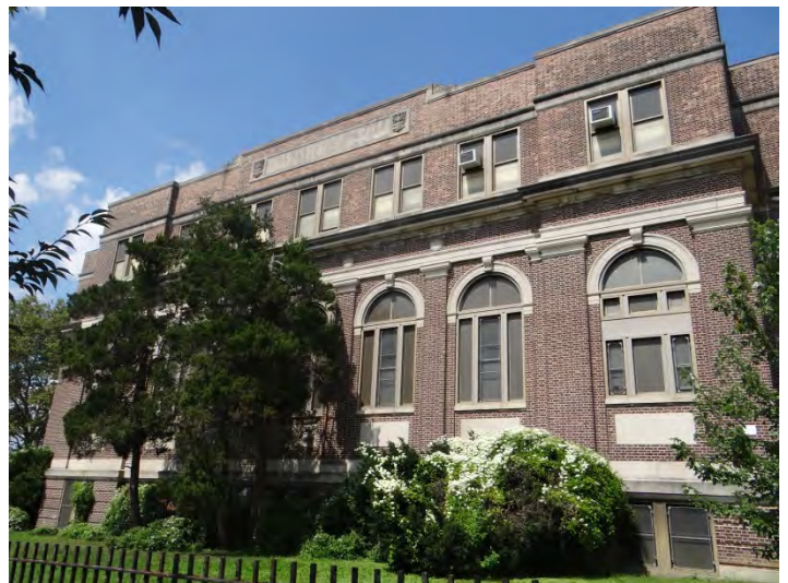
Photo 2: Looking NW at main (S) facade
