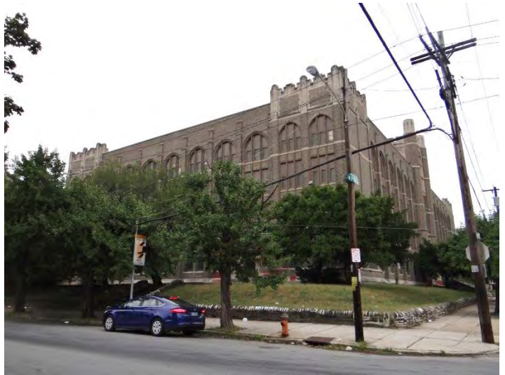
Photo 2: Looking NE at main (S, right) and W (left) facades
