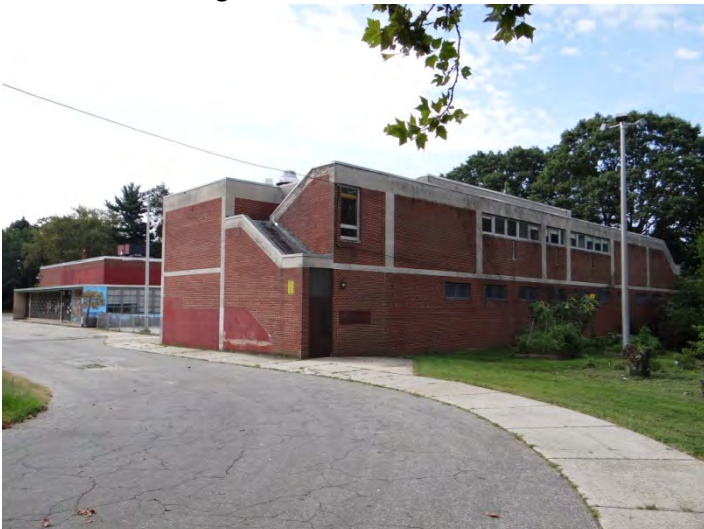
Photo 5: Looking S at NW facade
