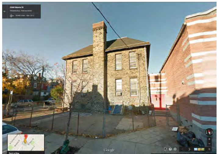
Photo 6: Looking NE at SW facade
