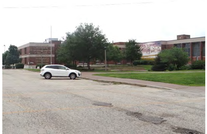
Photo 4: Looking SE at main (NE) facade
