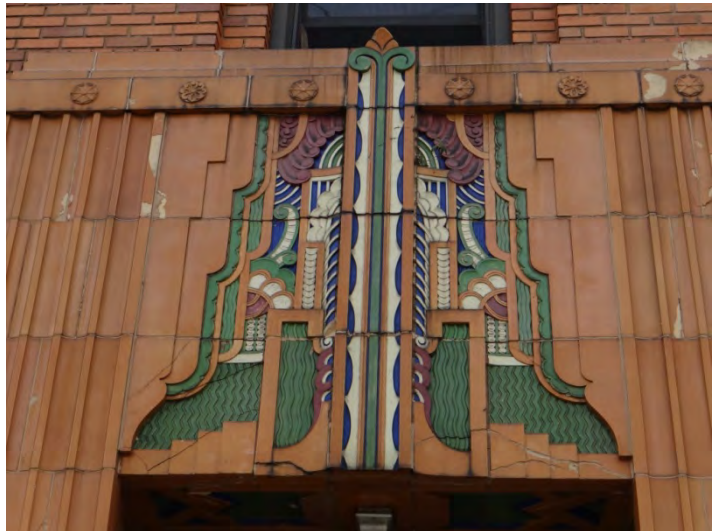
Photo 4: Detail, main façade entrance
