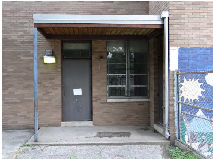
Photo 4: Looking E at NW façade entrance
