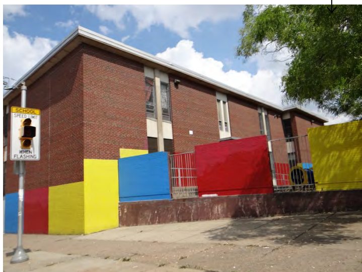
Photo 3: Looking NE at main (S, right) and W (left) facade
