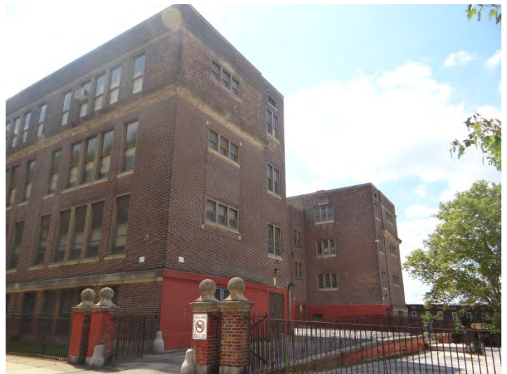
Photo 6: Looking SW at rear (N) facade
