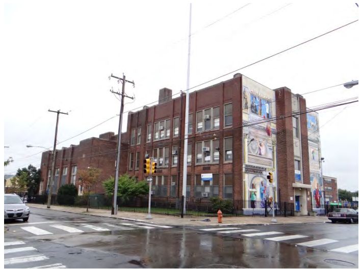
Photo 2: Looking SE at north (left) and W (right) facades
