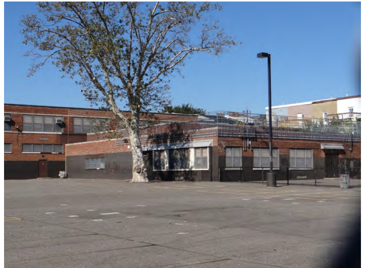
Photo 4: Looking N at N end of E facade
