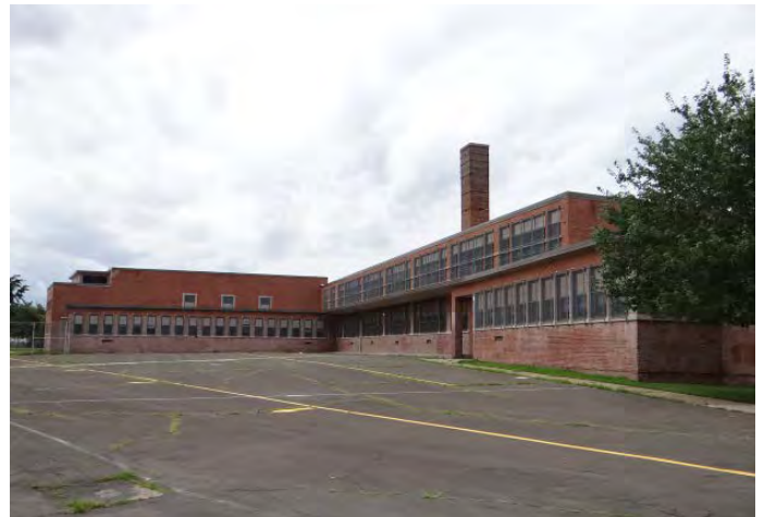
Photo 4: Looking W at SE facades
