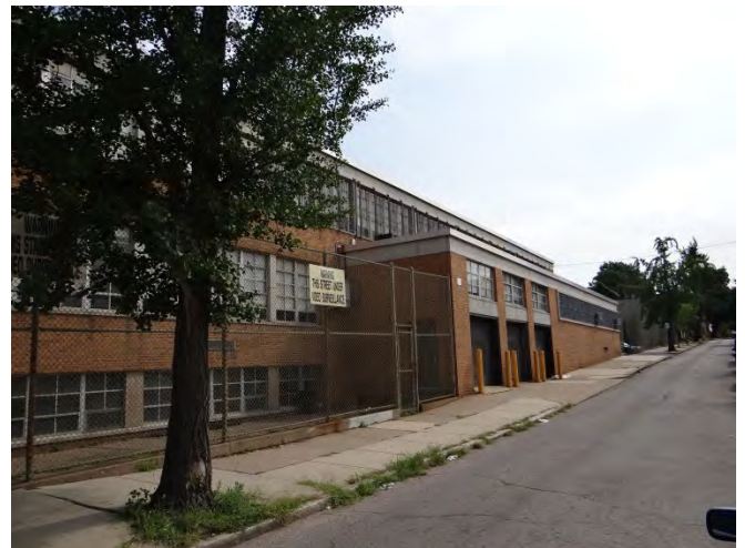
Photo 4: Looking NE at main (S) façade
