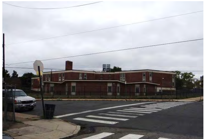
Photo 2: Looking SW at SW facade
