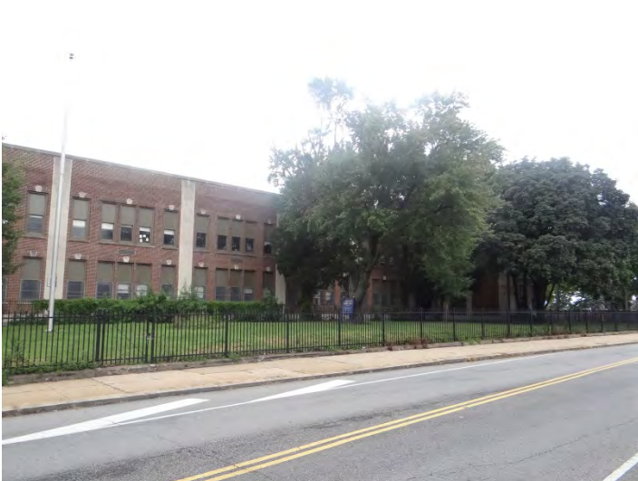
Photo 5: Looking NE at S facade
