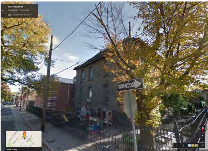
Photo 3: Looking S at NE façade
