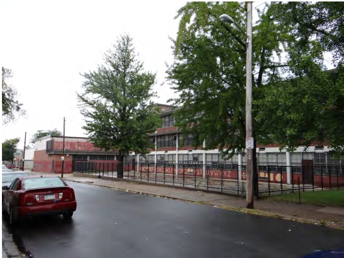
Photo 3: Looking NW at S facade
