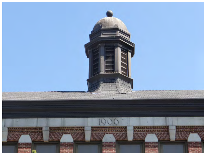
Photo 2: Detail, datestone, main (SW) facade
