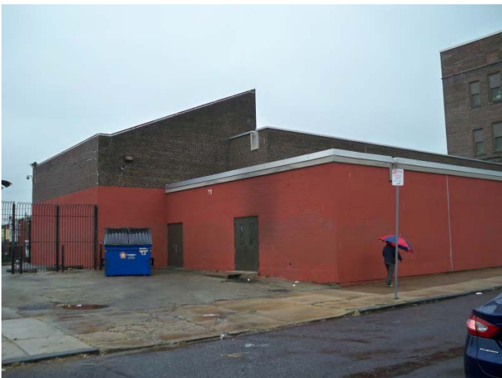
Photo 5: Looking NW at E (right) and S (left) facades of rear addition
