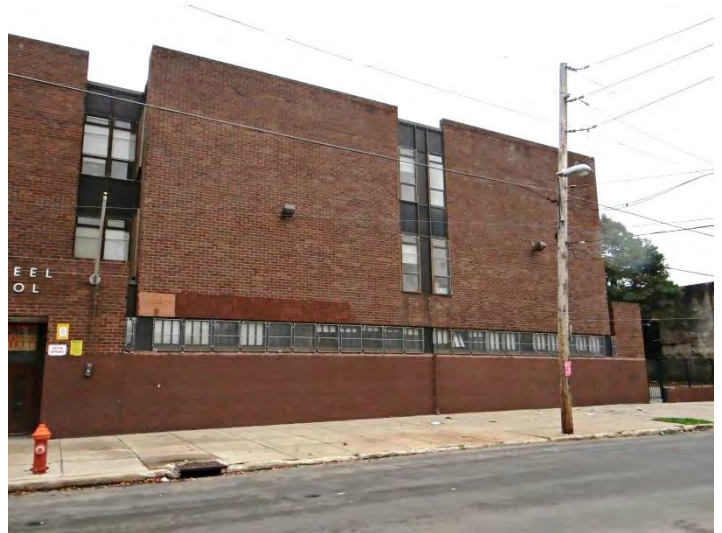
Photo 4: Looking NE at S end of main (SW) façade
