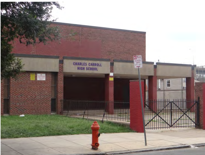
Photo 5: Looking SE at W end of NW façade
