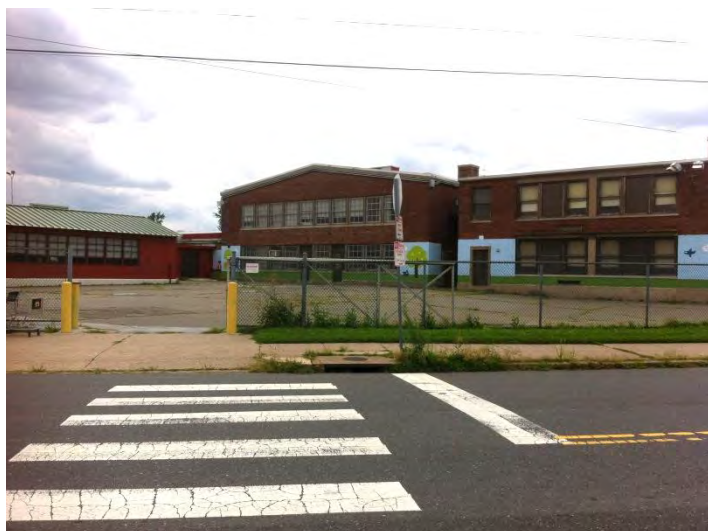
Photo 5: Looking SW at NE facades
