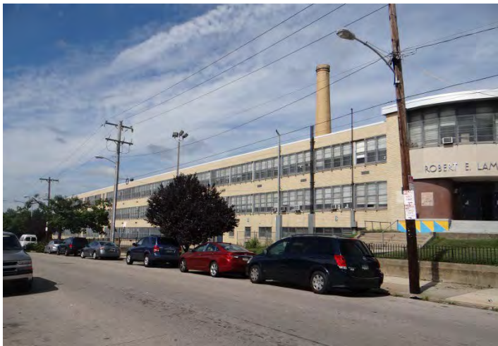
Photo 3: Looking W at SE façade
