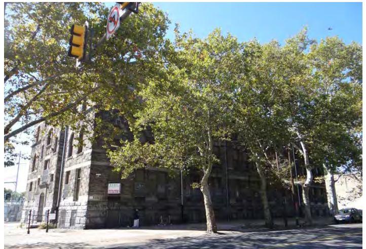
Photo 2: Looking SW at E (left) and N facades
