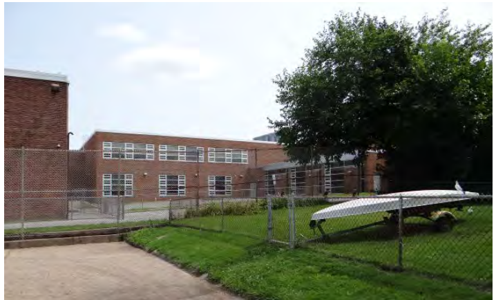
Photo 4: Looking NE at SW facade
