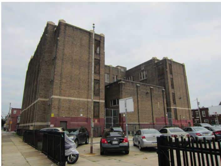
Photo 5: Looking SE at W façade
