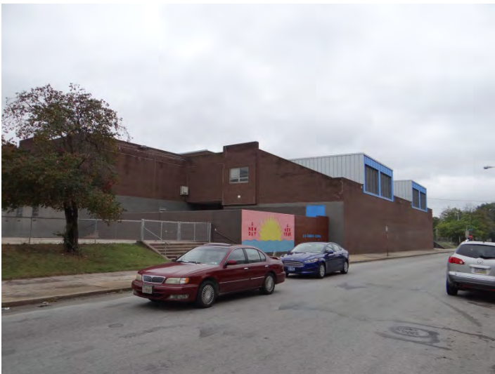
Photo 3: Looking SW at E facade
