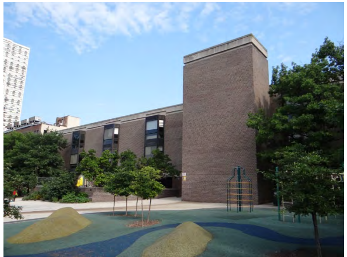
Photo 2: Looking N at rear (S) facade and playground
