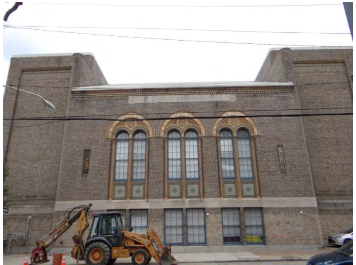
Photo 2: Looking SW at NE façade
