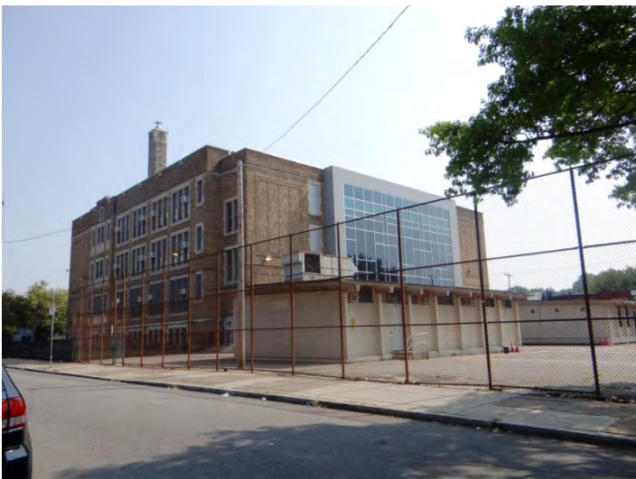
Photo 5: Looking NE at SW (right) and NW (left) facades
