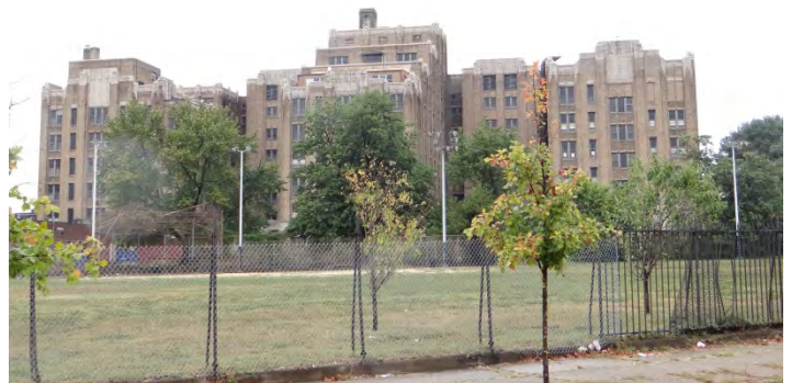
Photo 6: Looking N at rear (S) façade
