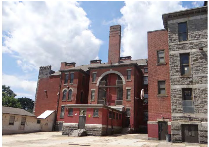
Photo 4: Looking W at SE facade
