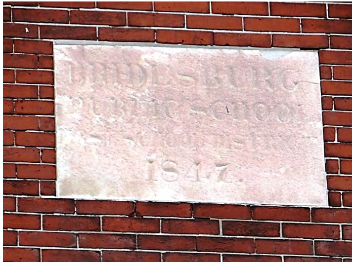
Photo 4: Looking SW at plaque on main (NE) facade
