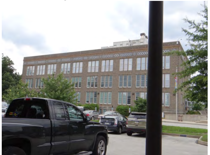
Photo 4: Looking SW at E facade
