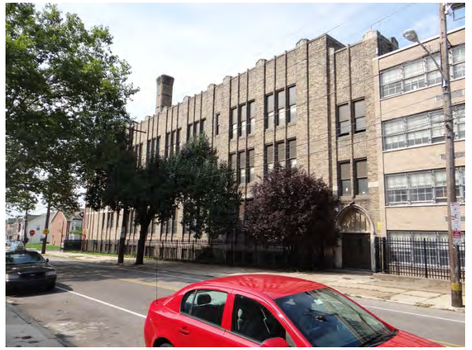
Photo 2: Looking SW at E facade
