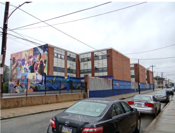
Photo 5: Looking SE at N (left) and W (right) facades
