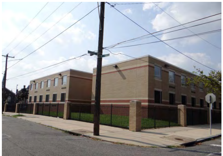
Photo 6: Looking W at SE and NE facades of addition
