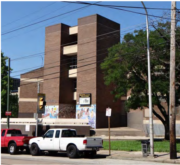
Photo 1: Looking SW at main (E) façade
