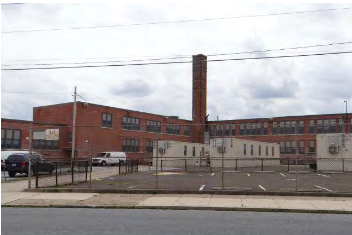
Photo 5: Looking W at NE facades
