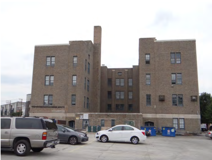
Photo 5: Looking NE at SW facade
