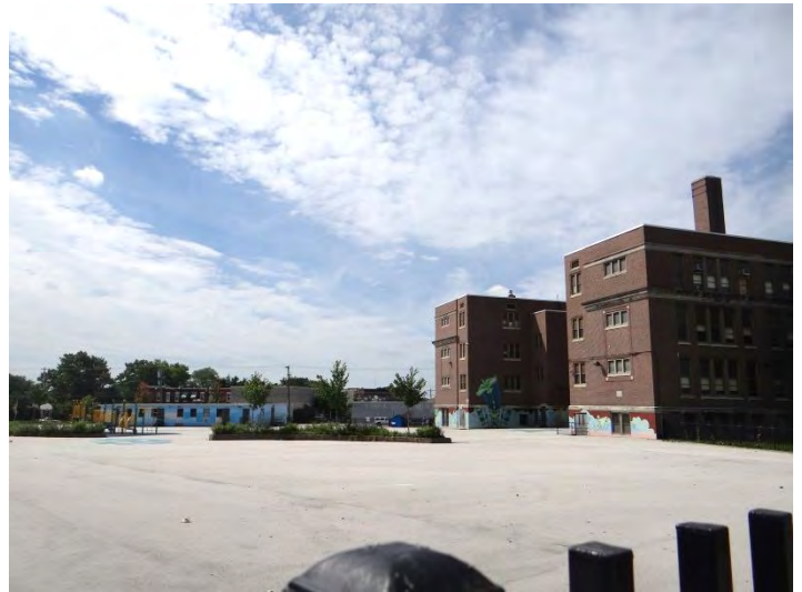
Photo 4: Looking W at rear (E) façade across playground
