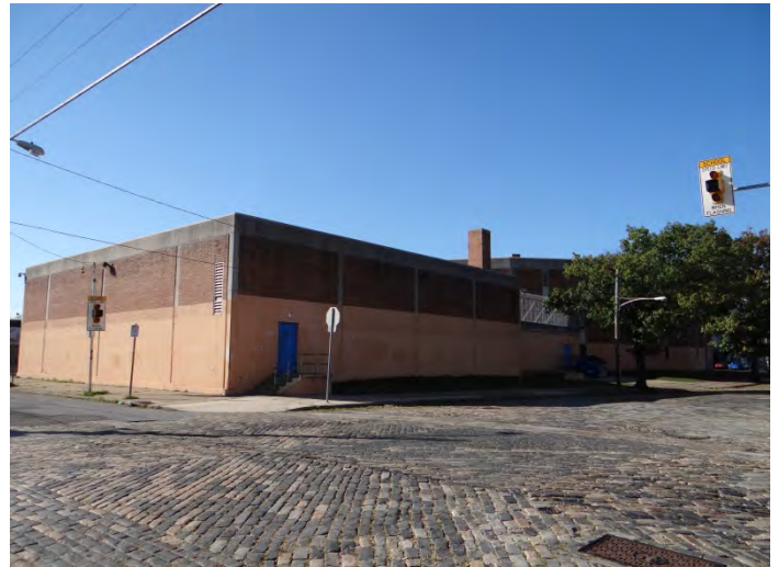
Photo 4: Looking S at N (right) and E (left) facades
