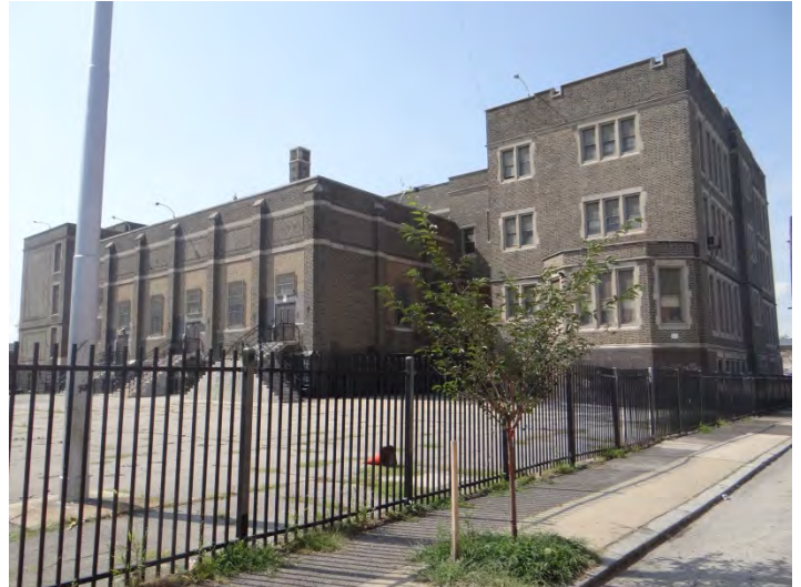
Photo 4: Looking SW at rear (NE) facade
