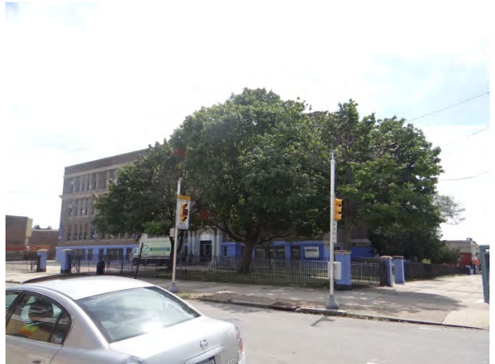
Photo 4: Looking SE at N facade
