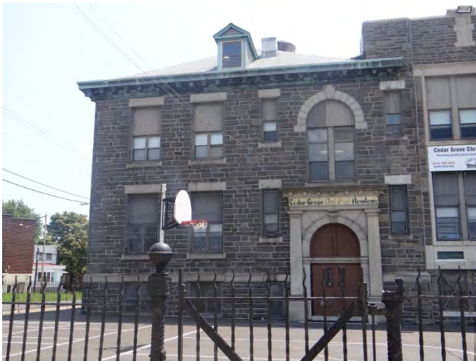
Photo 3: Looking SE at N end of NW facade
