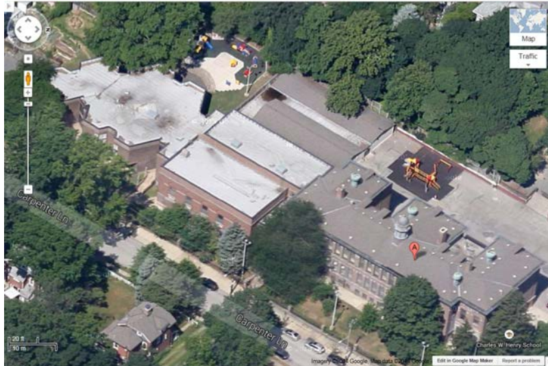
The Charles W. Henry Public School in the Mount Airy neighborhood was designed in 1908 by Henry deCourcy Richards. In the mid-1960s the size was dramatically increased with a Bornfreund and Cox addition (left half of the image). (2013 Google Earth aerial view)
