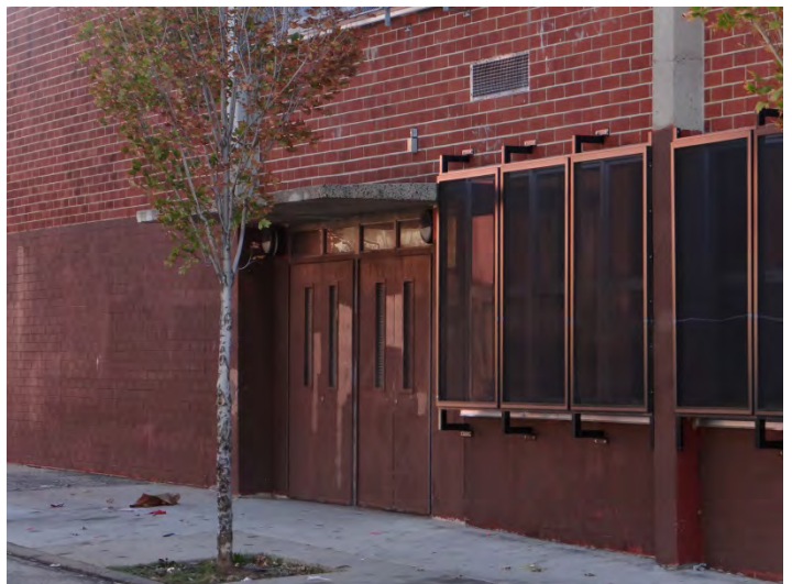
Photo 6: Looking NE at N end of SW facade
