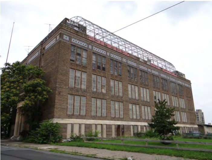
Photo 3: Looking NE at S facade
