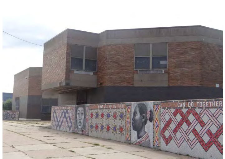
Photo 2: Looking E along N facade
