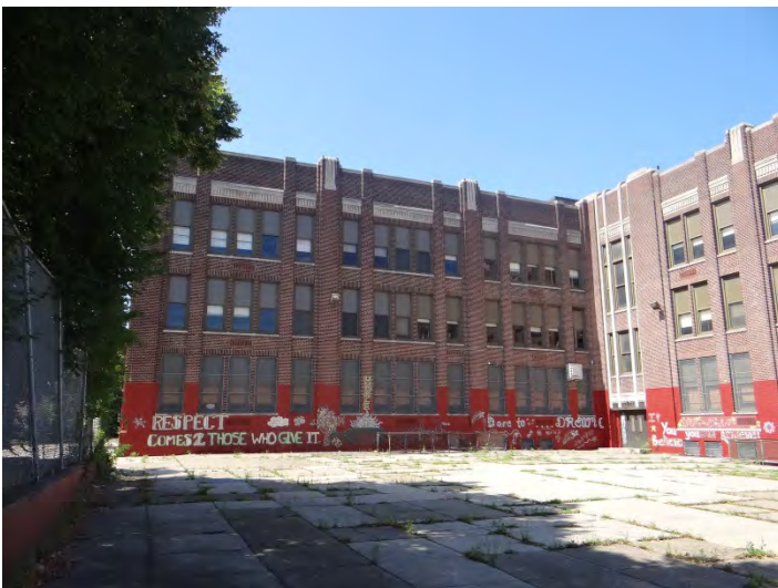
Photo 5: Looking W at E facades
