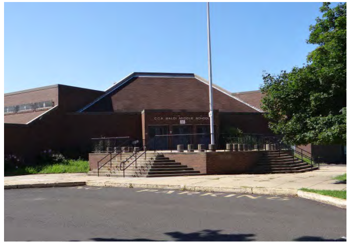
Photo 2: Looking SW at main entrance on main (N) facade
