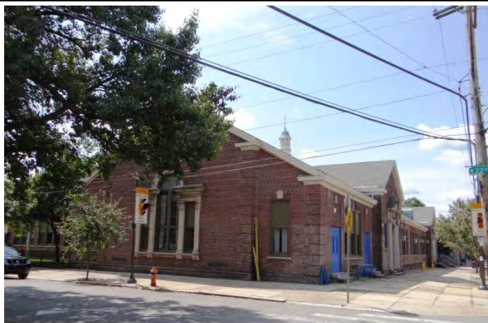
Photo 2: Looking SW at N (right) façade and E façade (left)
