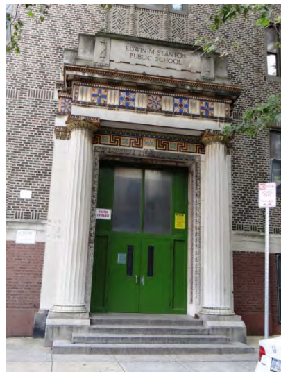
Photo 2: Looking E at main entrance on W façade
