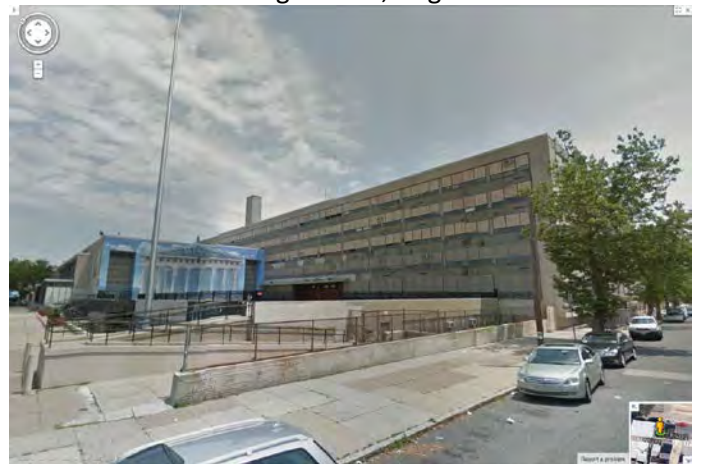
Photo 6: Looking NE at main (W) façade. Source: Google Earth, August 2014
