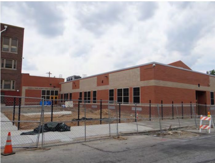
Photo 3: Looking NW at S façade of 2013 addition
