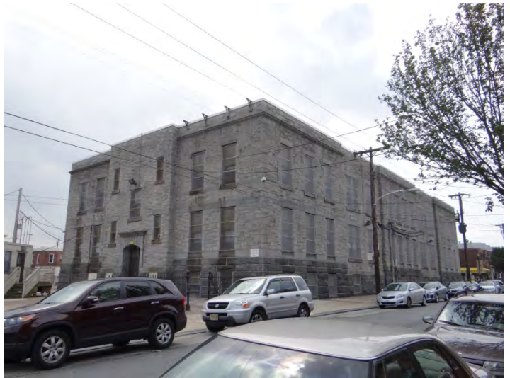
Photo 2: Looking SW at E (left) and N (right) facades
