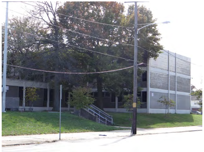
Photo 4: Looking S at S end of W facade
