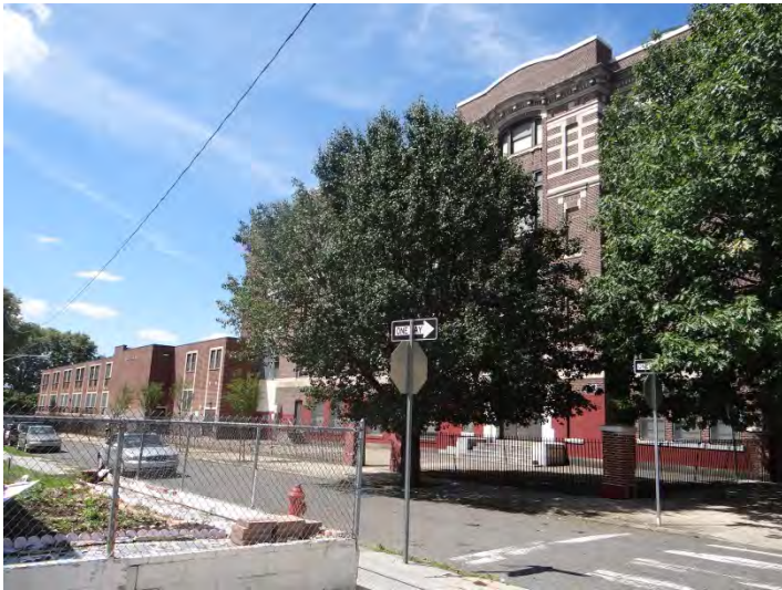
Photo 3: Looking SW at E façade, original building at right
