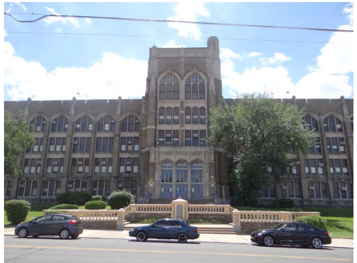
Photo 2: Looking S at main (N) façade
