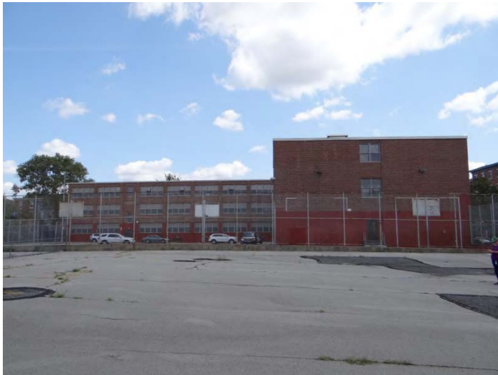
Photo 3: Looking E and rear (W) facades
