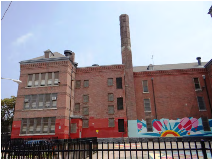
Photo 3: Looking E at N end of W facade
