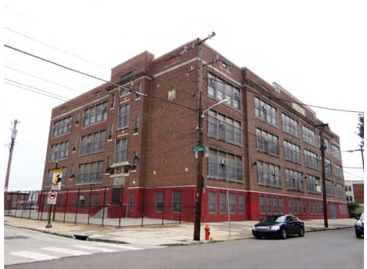
Photo 2: Looking NW at S (left) and E (right) facades
