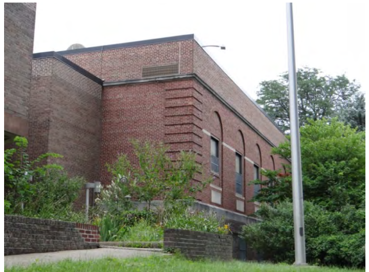
Photo 4: Looking NW at SE façade at SW end of school
