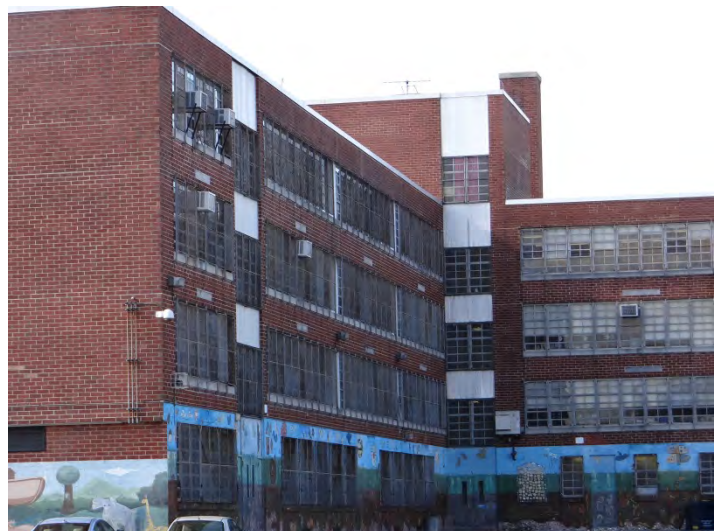
Photo 6: Looking SW at N façade
