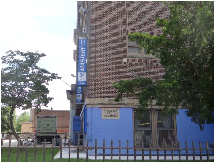
Photo 3: Looking E at datestone at N end of W facade
