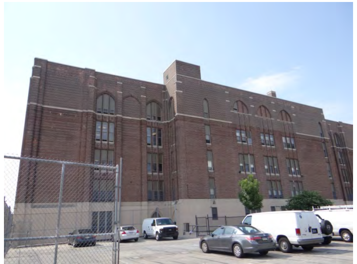
Photo 4: Looking NW at E facade
