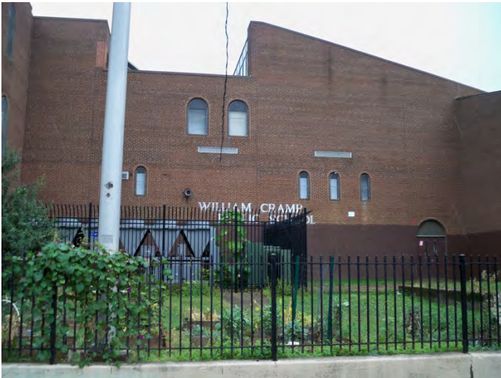
Photo 3: Looking E at W facade
