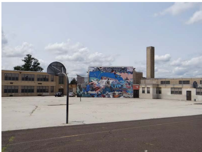
Photo 4: Looking W at NW corner of NE facades
