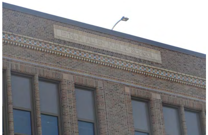
Photo 4: Looking S at main (NW) facade
