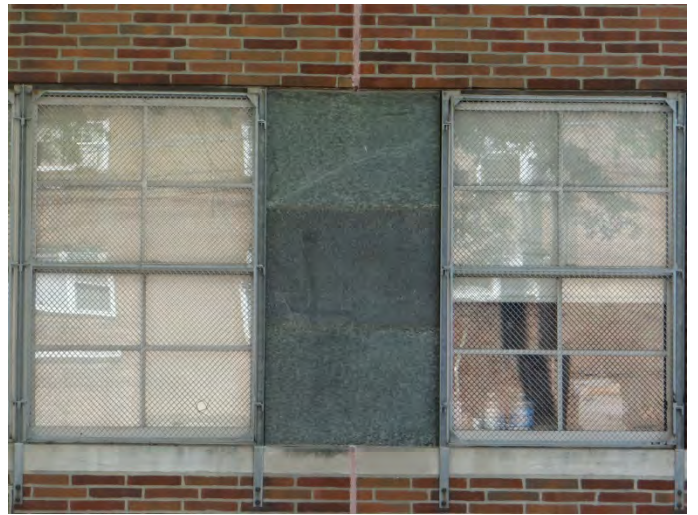
Photo 2: Detail, original windows and stone panels, typ.
