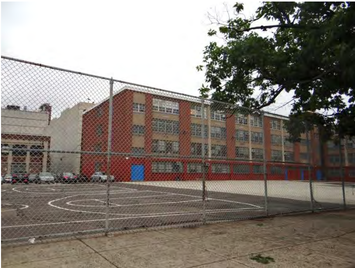
Photo 3: Looking SE at W façade
