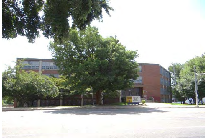
Photo 2: Looking E at NW façade
