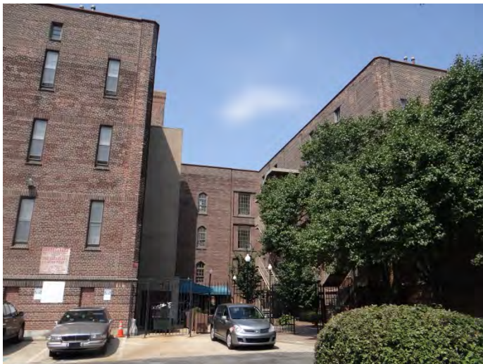
Photo 5: Looking W at E façade
