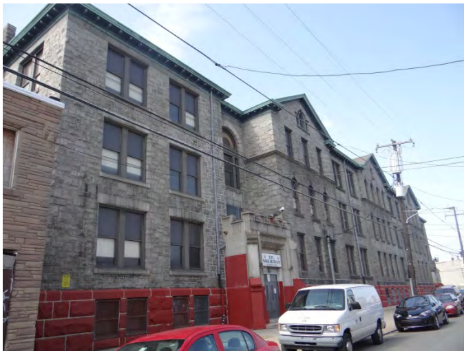
Photo 3: Looking SW at E end of main (N) façade
