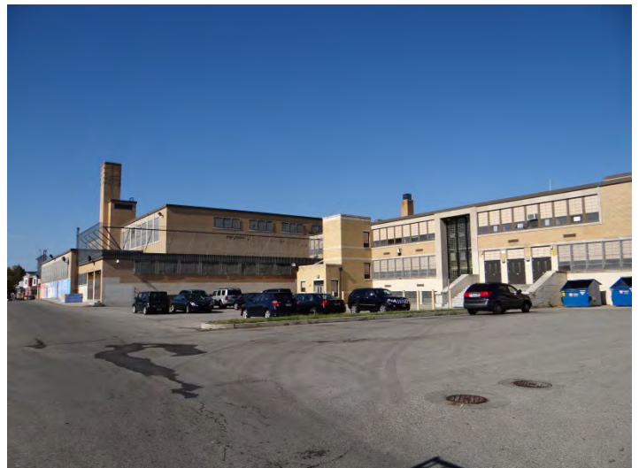
Photo 6: Looking NW at E corner of rear (S) facade
