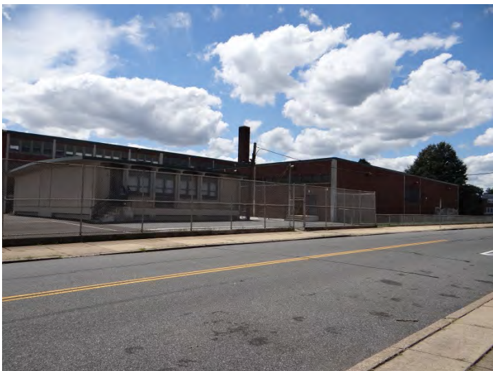
Photo 5: Looking W at E facade
