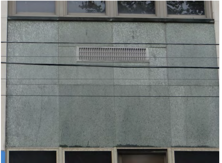
Photo 4: Detail, granite panels in window bays, typical
