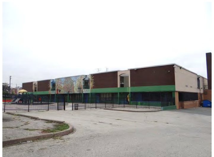
Photo 6: Looking SW at E facade
