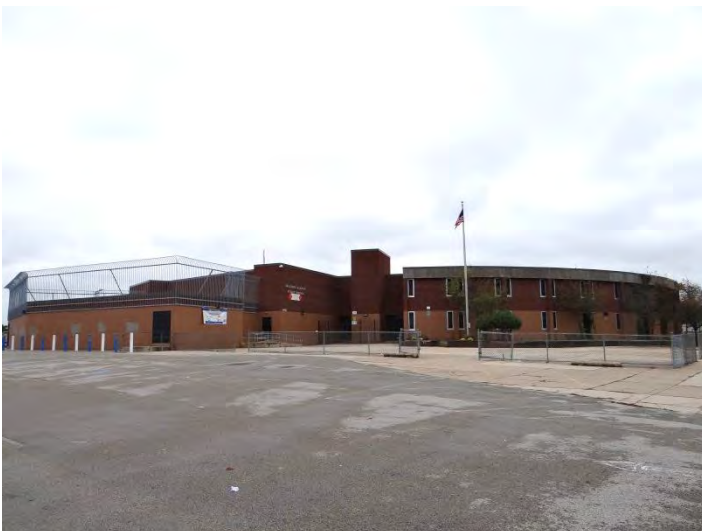
Photo 5: Looking NW at E façade and main entrance
