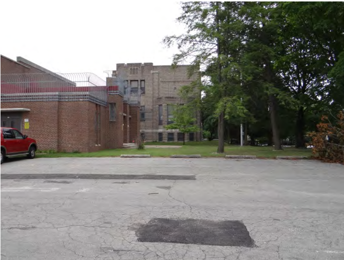
Photo 3: Looking E at W facade
