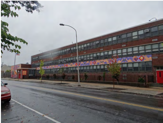
Photo 3: Looking E at main (N) façade
