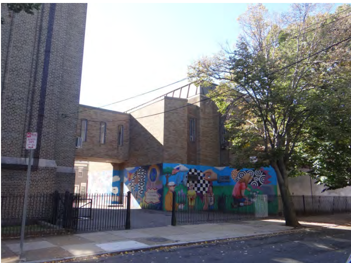
Photo 5: Looking SW at NW facade
