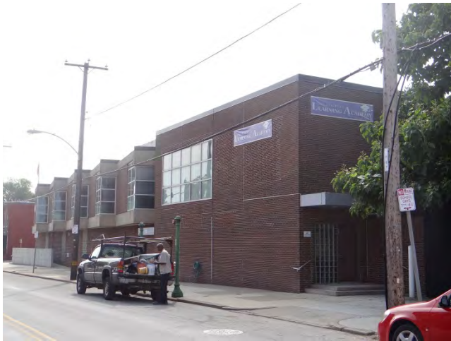
Photo 3: Looking SE at N façade
