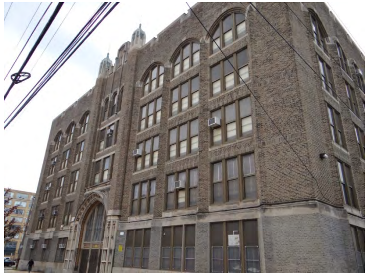
Photo 2: Looking W at E façade
