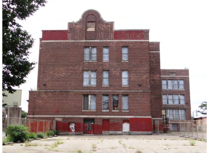
Photo 2: Looking W at E facade
