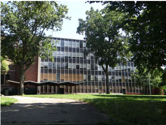
Photo 5: Looking NE at SW façade, E end
