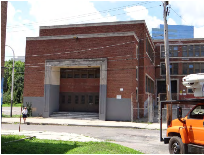
Photo 1: Looking SW at main (NE) façade
