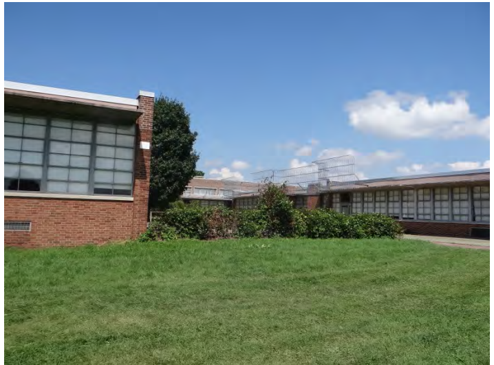
Photo 4: Looking NE at W end of S façade
