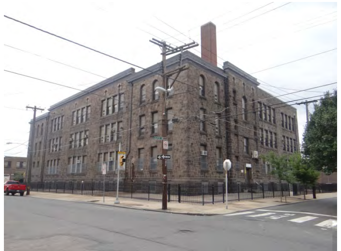
Photo 4: Looking S at NE (left) and NW (right) facades
