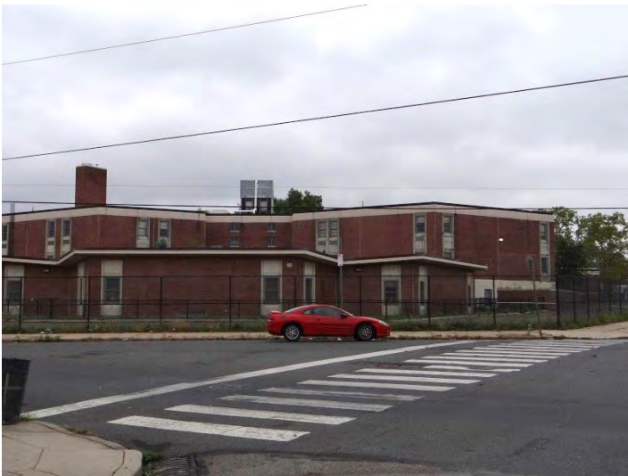
Photo 3: Looking W at N end of E facade
