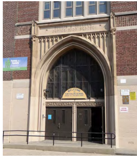
Photo 2: Looking E at W façade entrance
