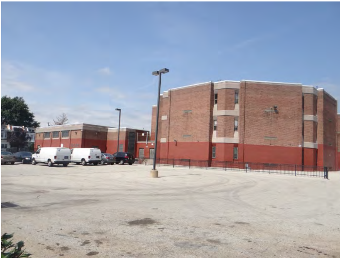
Photo 3: Looking NW at SE façade
