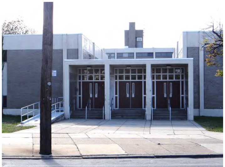
Photo 2: Looking S at main entrance on main (N) facade
