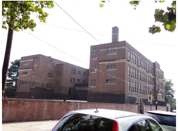
Photo 4: Looking S at NE facade
