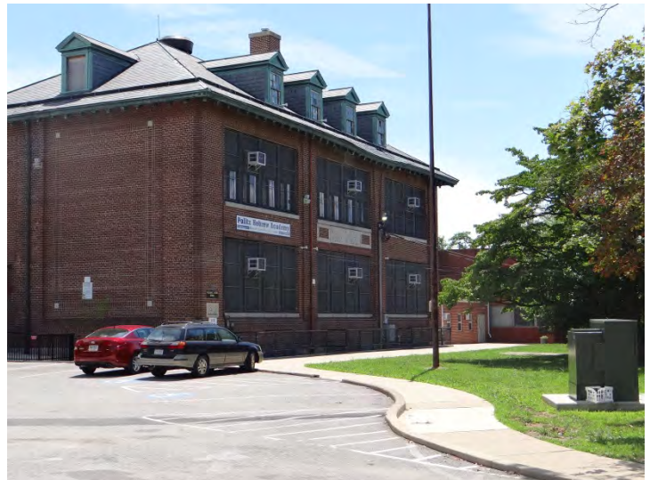
Photo 4: Looking S at NW façade of historic school
