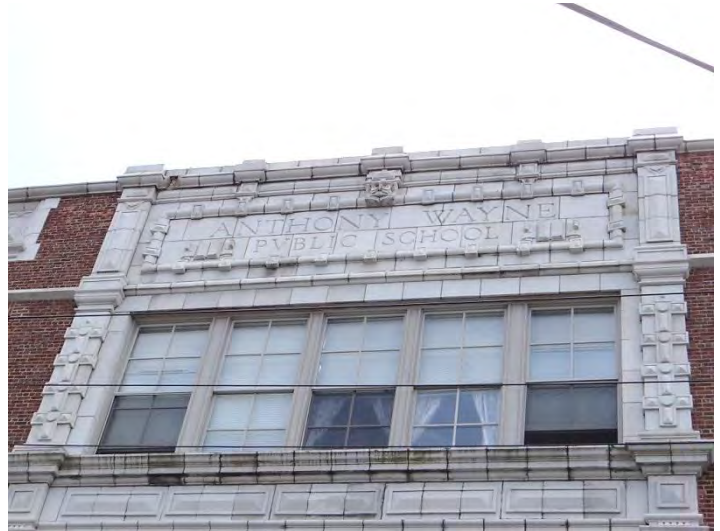
Photo 4: Looking S at N facade
