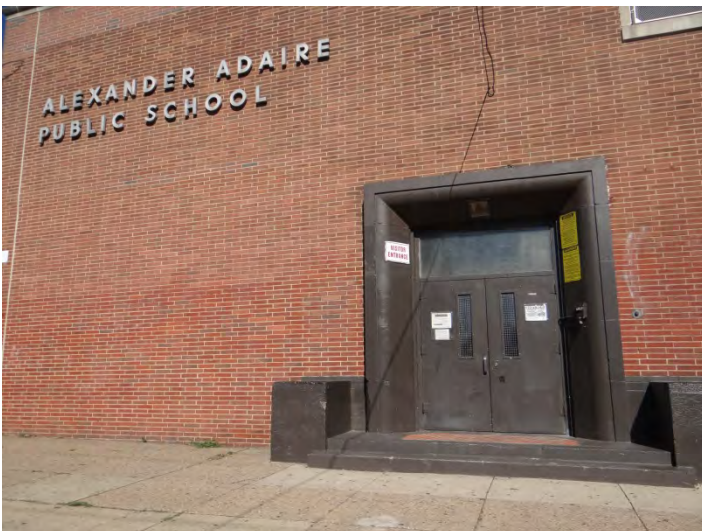
Photo 5: Looking N at entrance at W end of S facade
