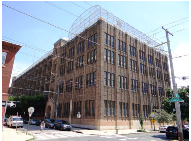
Photo 2: Looking SE at main (N, left) and W (right) facades
