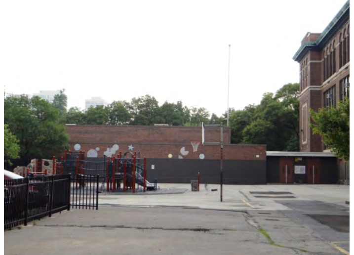
Photo 2: Looking E at W facade of addition
