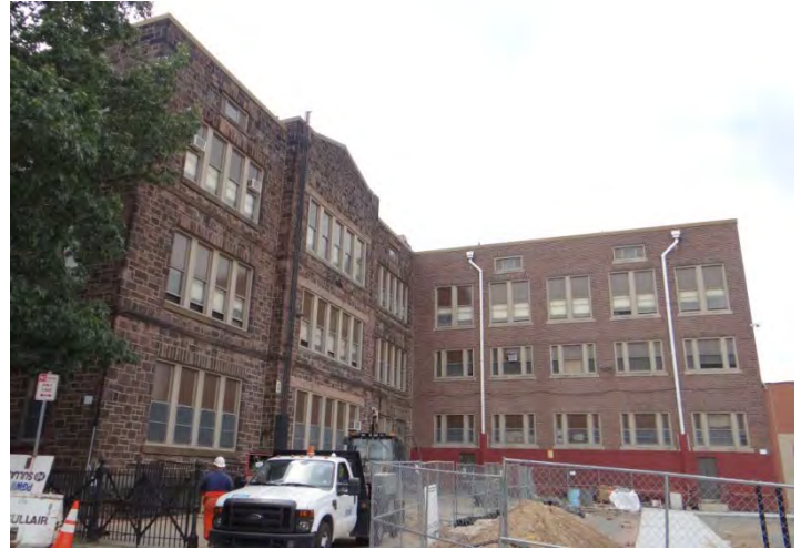
Photo 2: Looking SW at N (left) and E (right) facades
