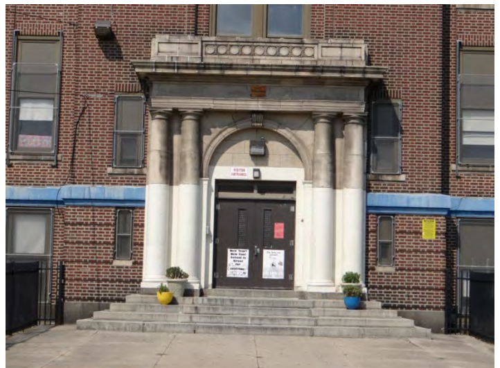
Photo 6: Typical entrance, E and W facades
