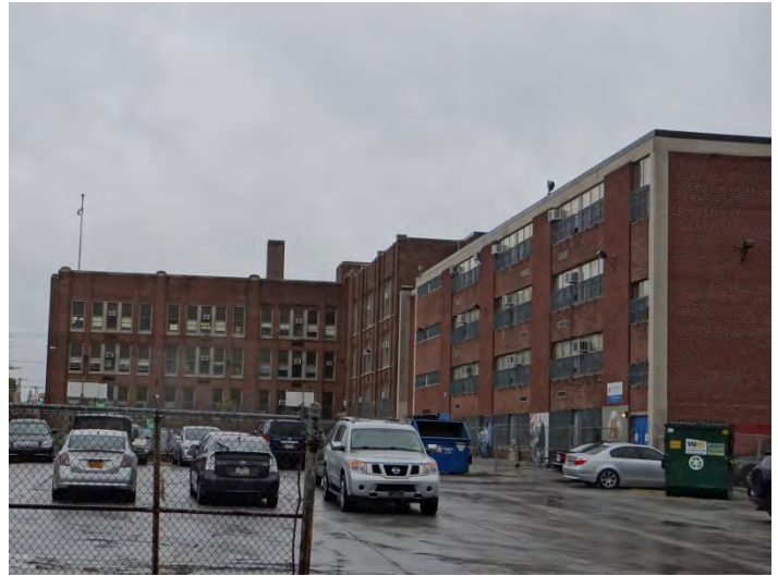
Photo 4: Looking NE at rear (S, left and W, right) facades
