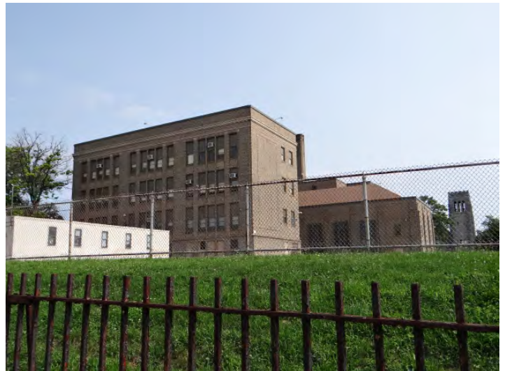
Photo 6: Looking N at SW (left) and rear (SE) facades
