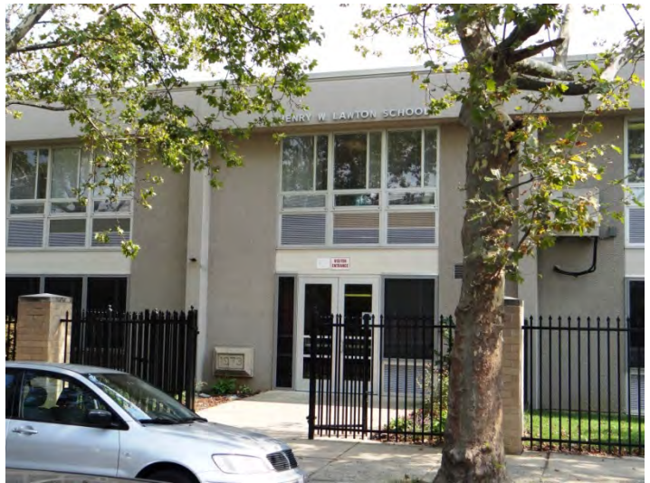
Photo 2: Looking SE at entrance on NW facade
