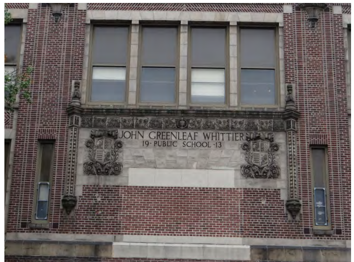
Photo 2: Looking E at former main entrance, W facade
