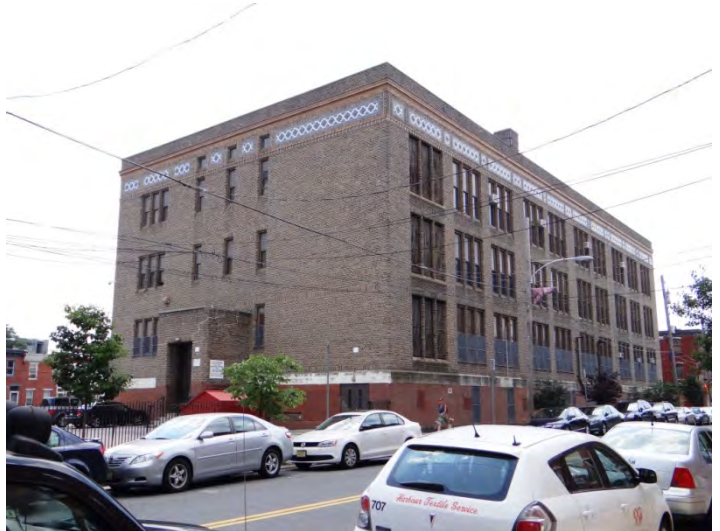
Photo 4: Looking SW at E (left) and N facades
