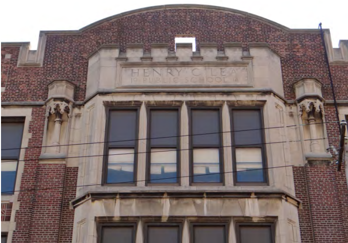
Photo 3: Looking S at center bay of main (N) façade
