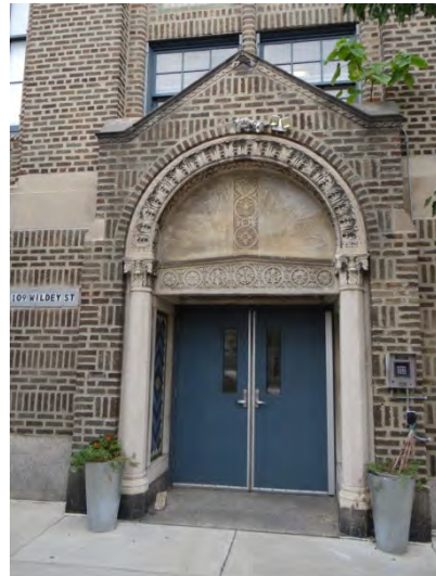
Photo 4: Looking NW at SE façade entrance
