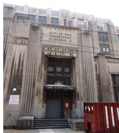
Photo 6: Looking S at W corner of main (N) facade
