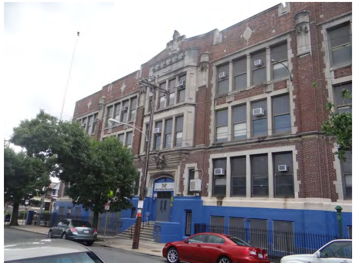
Photo 2: Looking SE at N facade
