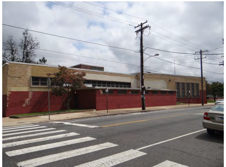
Photo 2: Looking NE at main (SW) facade
