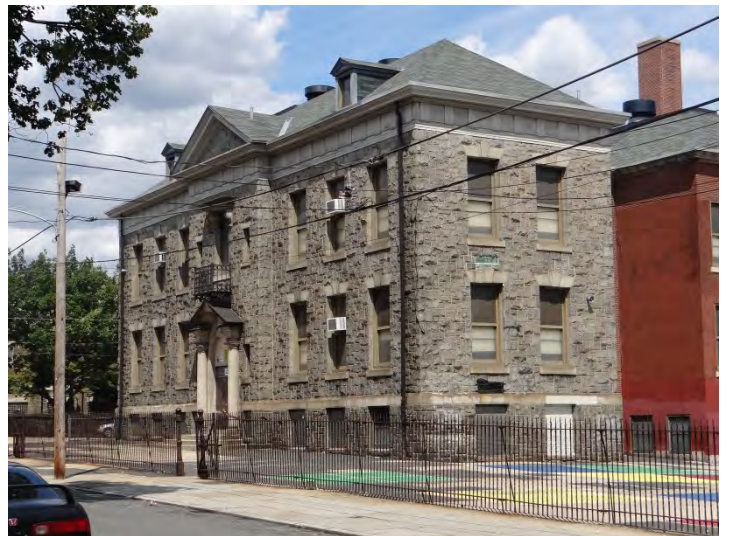
Photo 6: Looking NE at W facade
