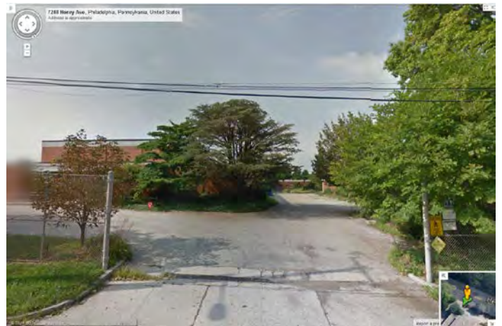
Photo 2: Looking SW at NW end of complex
