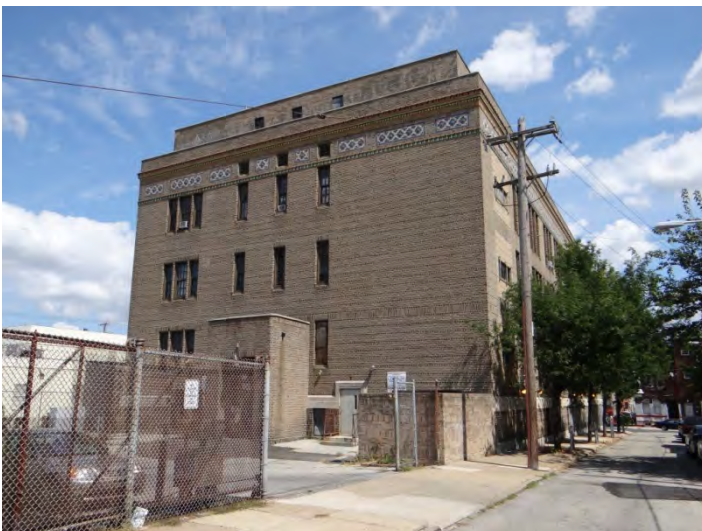
Photo 5: Looking NE at W facade
