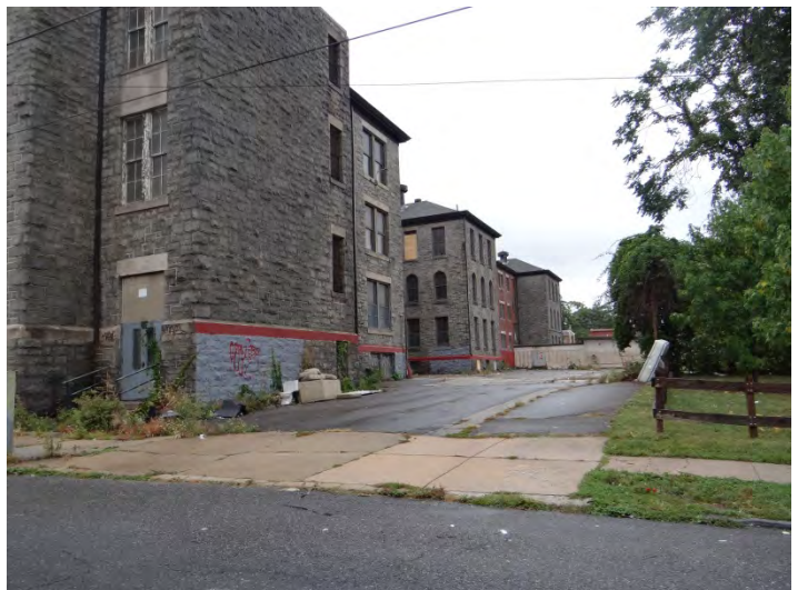
Photo 6: Looking W at N facade
