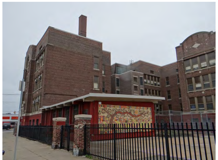
Photo 6: Looking NE at S (left) and W (right) facades
