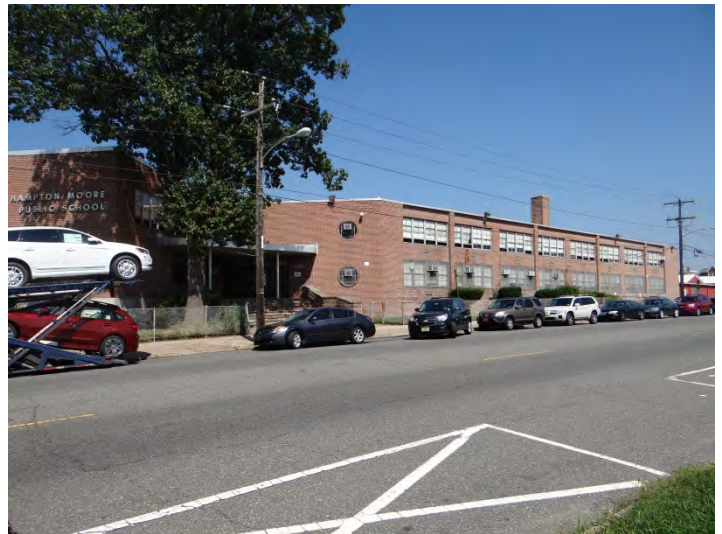
Photo 2: Looking NE at SE facade
