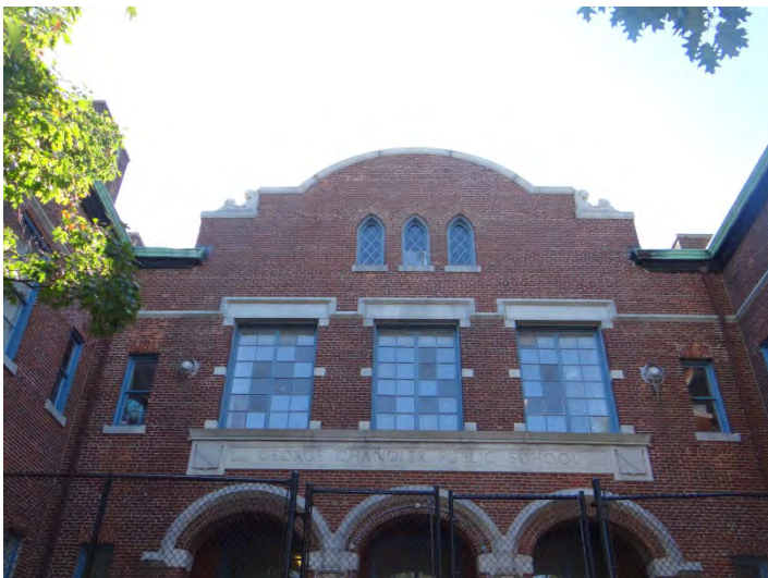
Photo 5: Looking S at center bays of N facade
