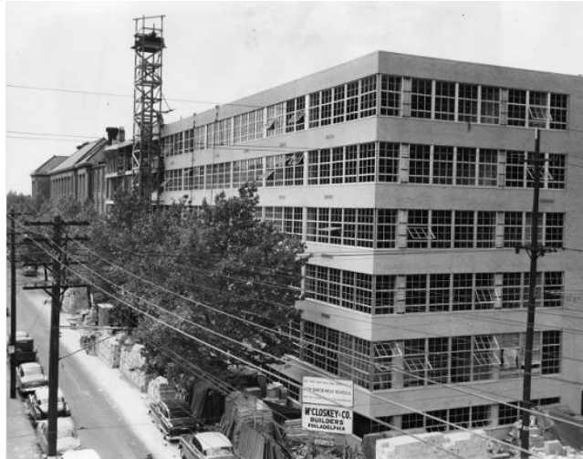
South Philadelphia High, designed by Davis, Dunlap, Carver, under construction in 1955. Strips of ribbon windows and simple rectangular massing are two character-defining features of International Style schools. George D. McDowell Philadelphia Evening Bulletin Photographs, Urban Archives, Temple University.
