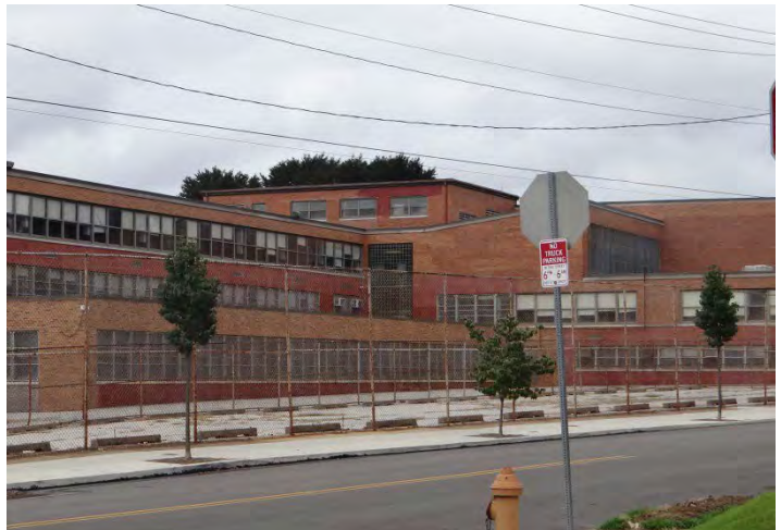
Photo 6: Looking SW at NE facade
