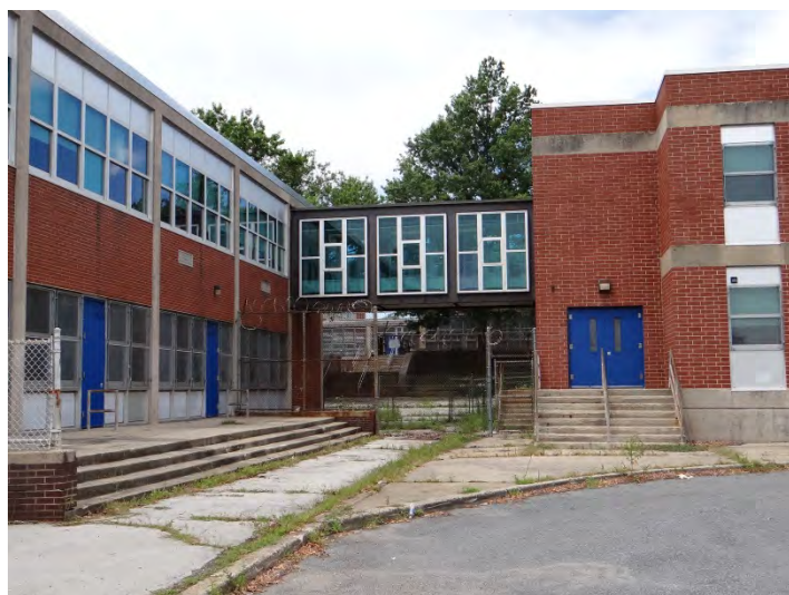
Photo 5: Looking W at N end of SE facade
