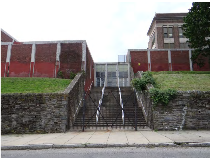
Photo 5: Looking SW at NE facade
