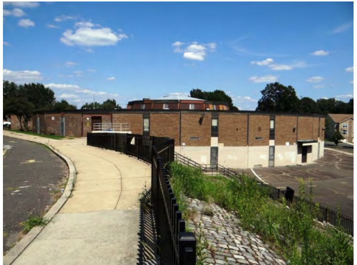
Photo 4: Looking NE at SW facade
