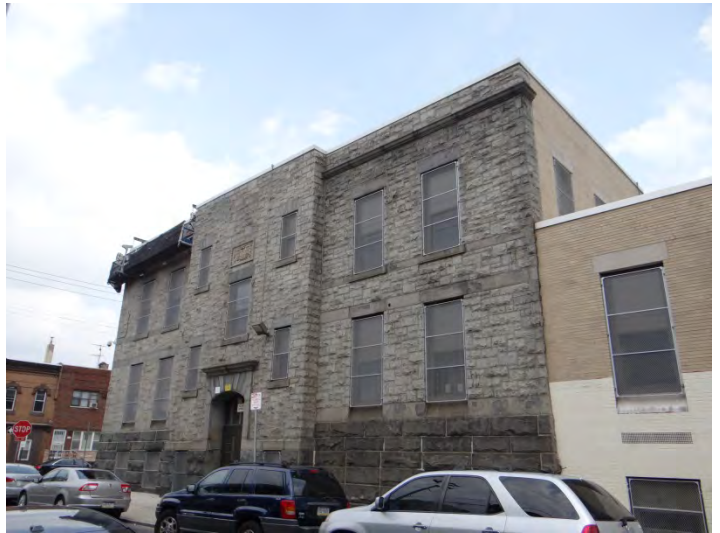
Photo 4: Looking NE at W facade
