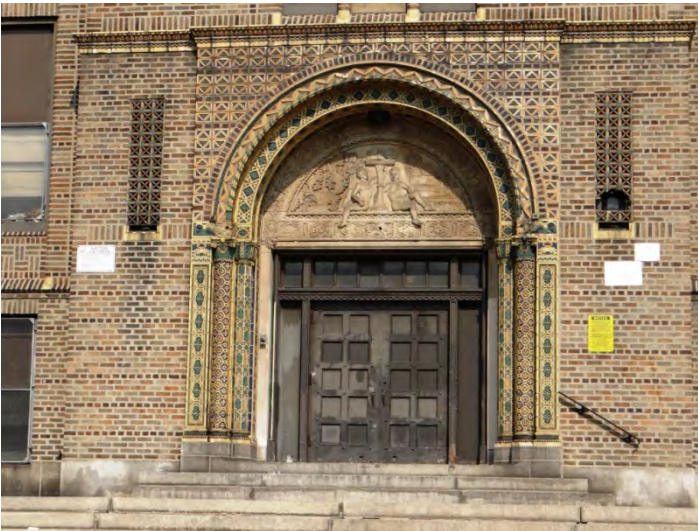
Photo 3: Looking NW at main (SE) façade entrance
