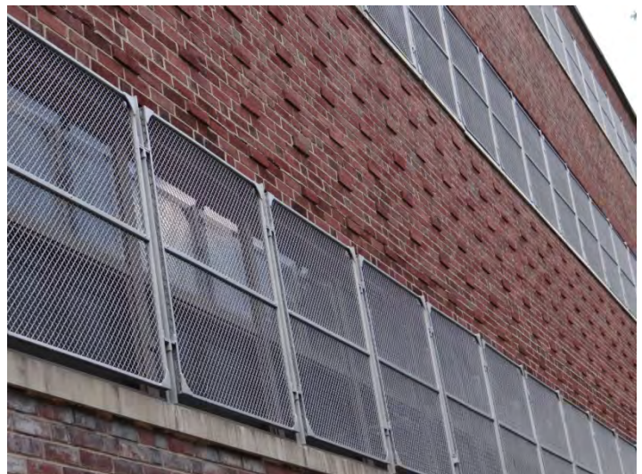
Photo 6: Detail, brickwork, E facade
