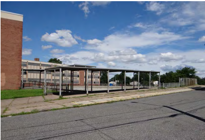
Photo 5: Looking NE at S façade bus canopy
