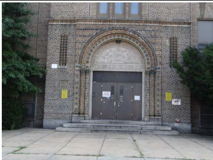
Photo 2: Looking SE at entrance on NW façade
