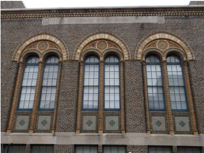
Photo 3: Detail, looking SW at NE facade
