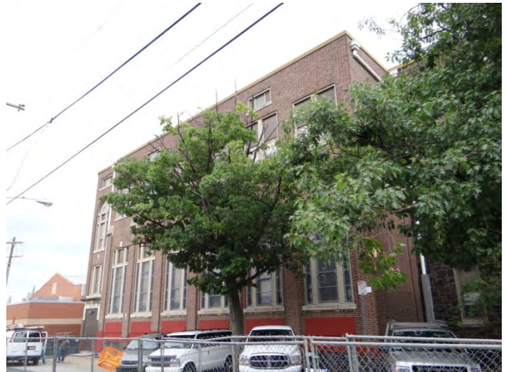
Photo 4: Looking NE at W façade
