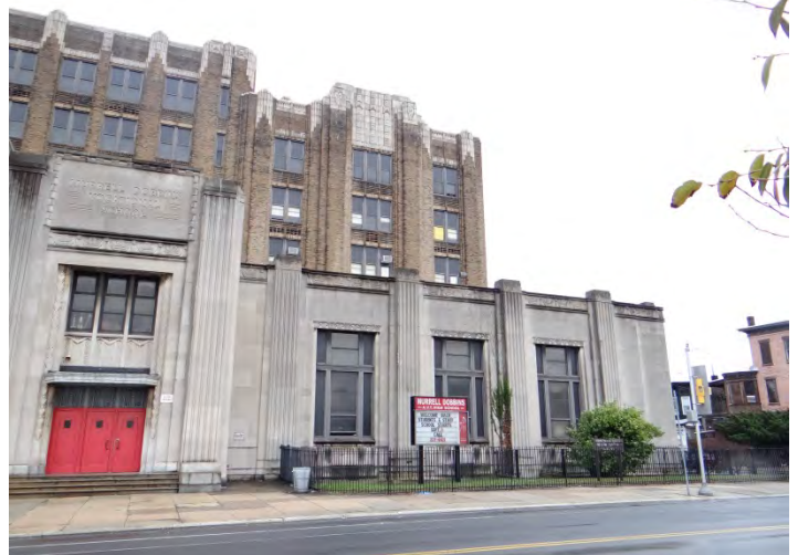
Photo 4: Looking SW at W end of main (N) façade
