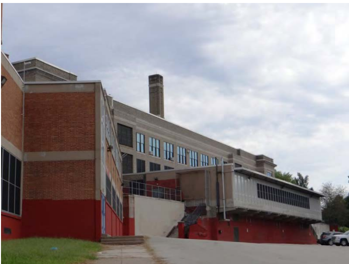
Photo 5: Looking N at rear (S) facade
