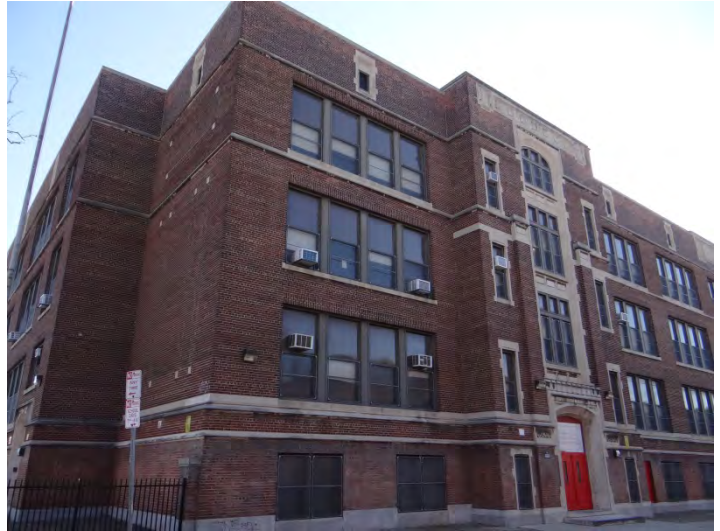
Photo 2: Looking SE at main (SE) facade
