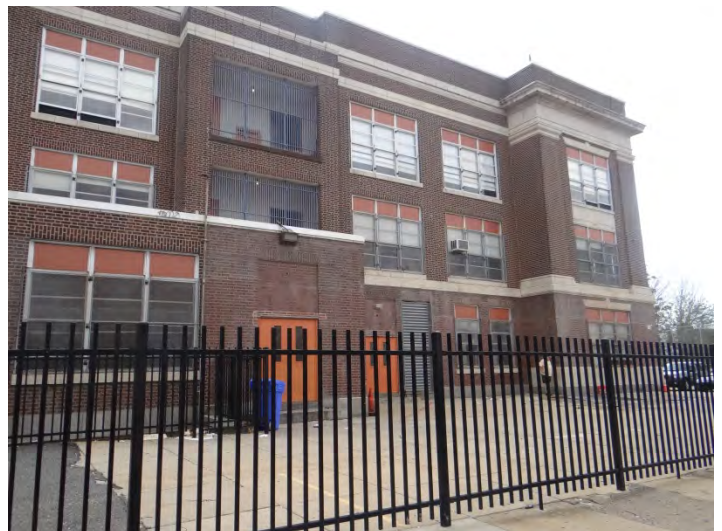
Photo 6: Looking SW at rear (NW) facade
