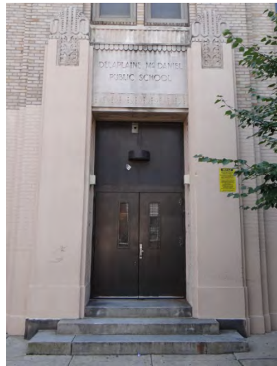
Photo 2: Looking S at N façade entrance
