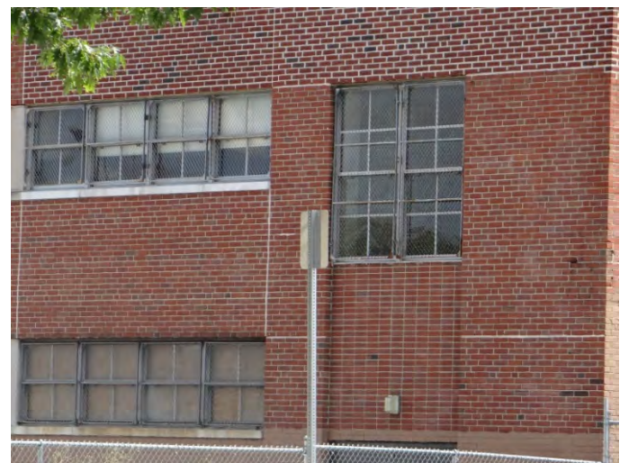
Photo 6: Detail, original metal windows, typical condition
