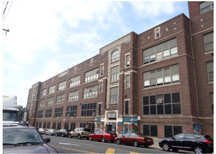
Photo 2: Looking SW at S end of main (E) facade
