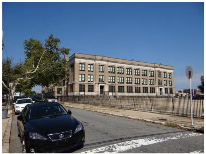
Photo 4: Looking NW at SE facade
