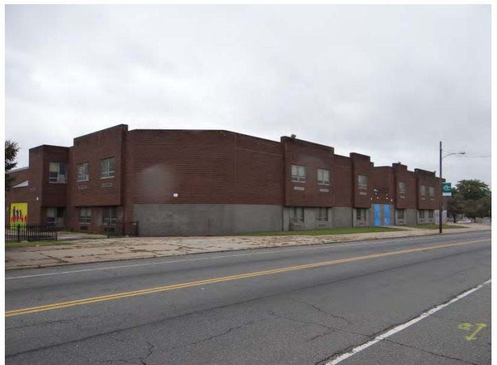
Photo 6: Looking NW at E facade
