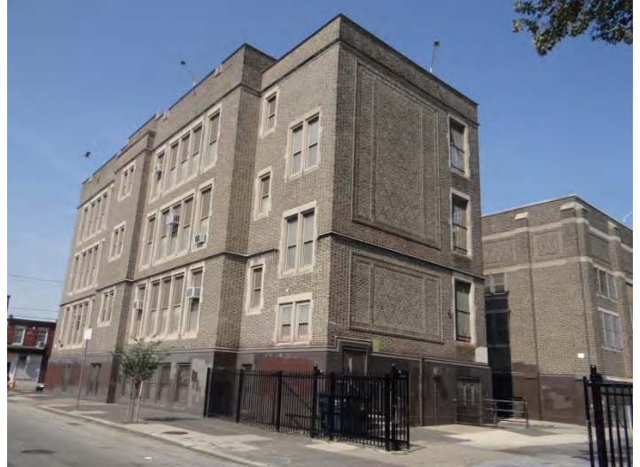
Photo 6: Looking W at SE facade
