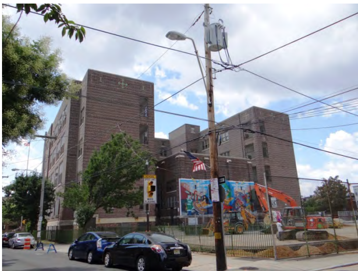
Photo 3: Looking SW at rear (N) façade
