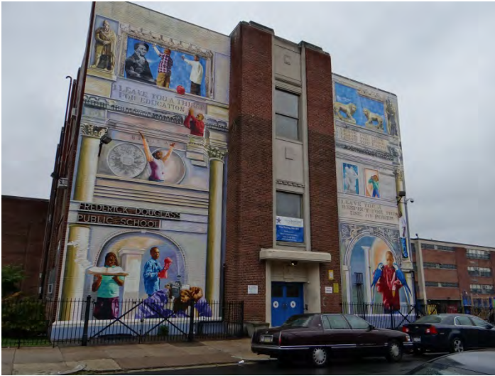
Photo 3: Looking E at W facade
