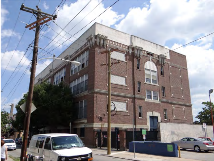
Photo 3: Looking N at W (left) and S (right) facades
