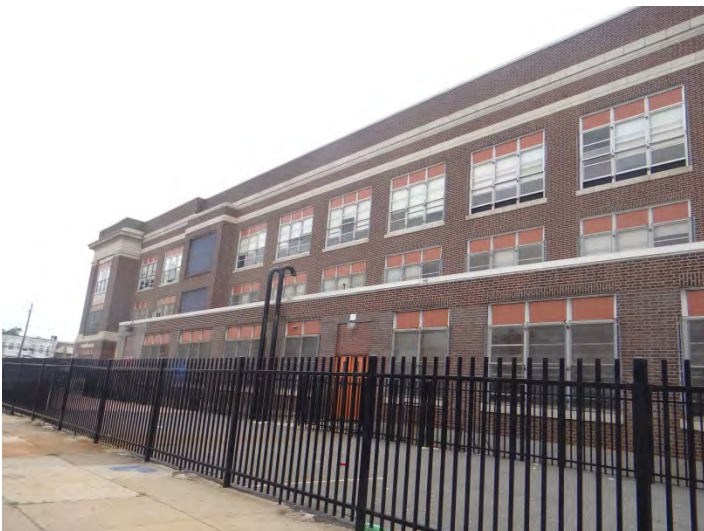
Photo 5: Looking E at rear (NW) facade
