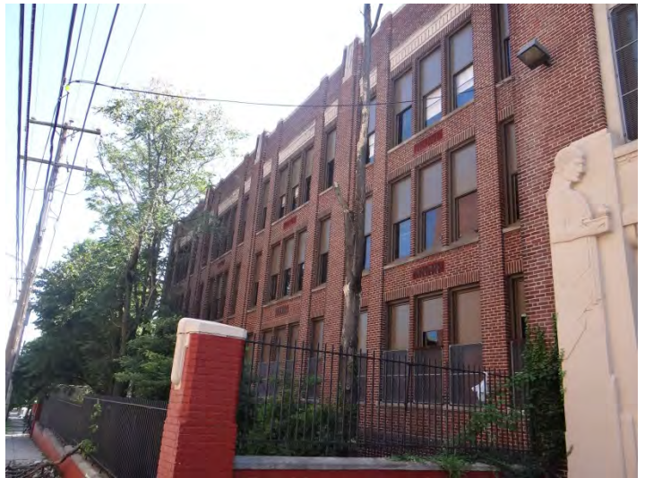
Photo 2: Looking N and main (NW) facade
