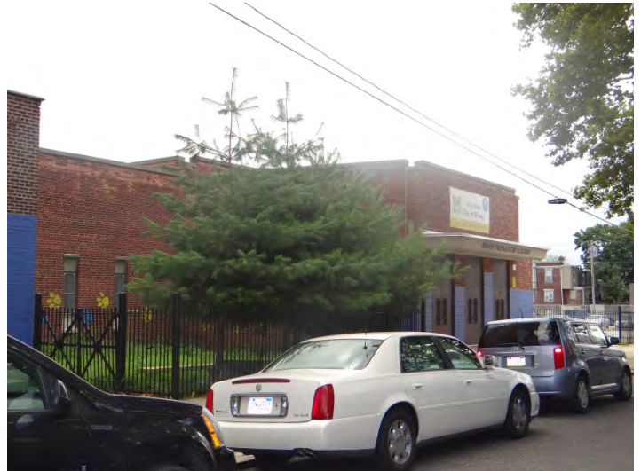
Photo 4: Looking S at W façade of rear addition
