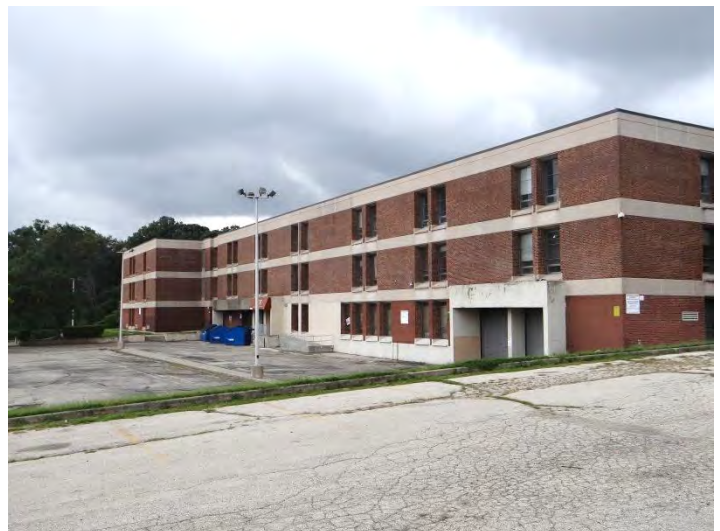
Photo 6: Looking W at SE facade
