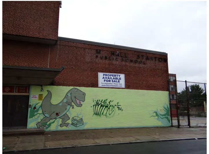
Photo 4: Looking SE at W facade
