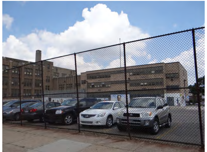
Photo 4: Looking NE at W facade
