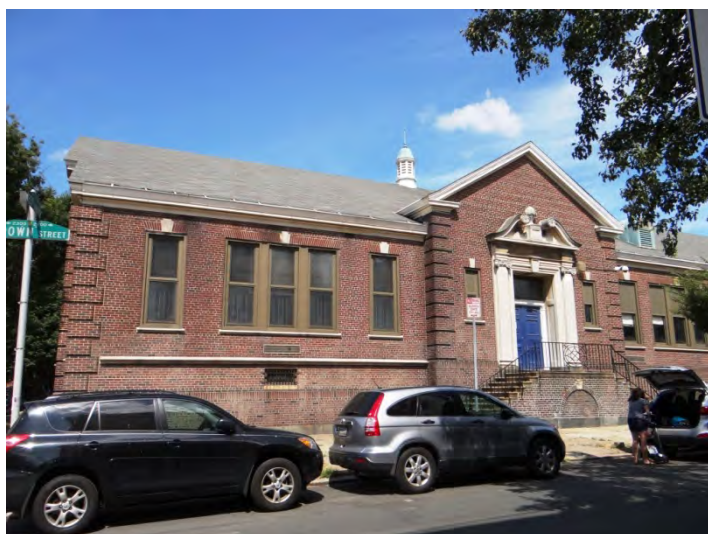
Photo 5: Looking N at W corner of S façade
