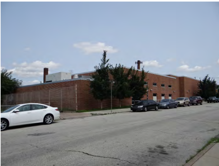
Photo 5: Looking N at SW (left) and SE facades
