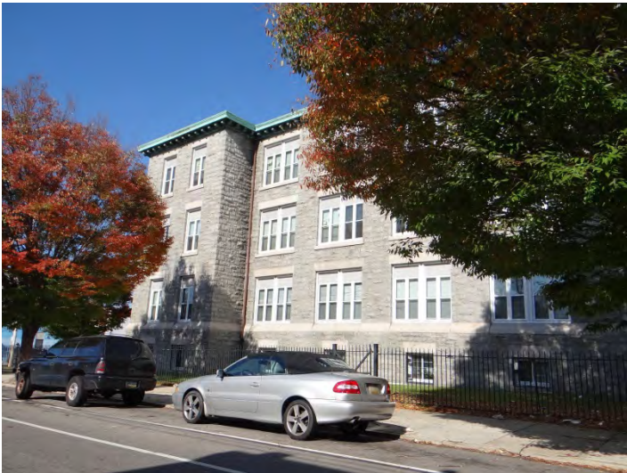
Photo 3: Looking NW at S facade
