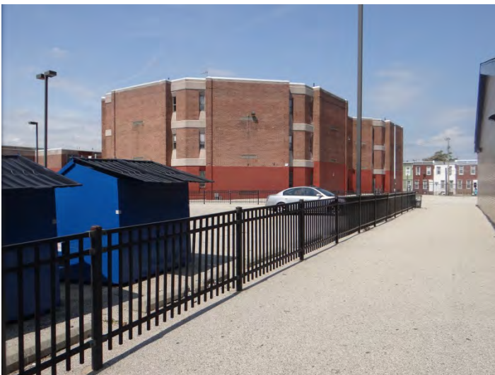
Photo 5: Looking N at SE (left) and NE (right) facades
