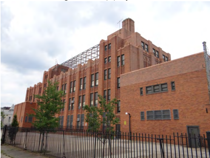
Photo 5: Looking NW at rear (S) façade
