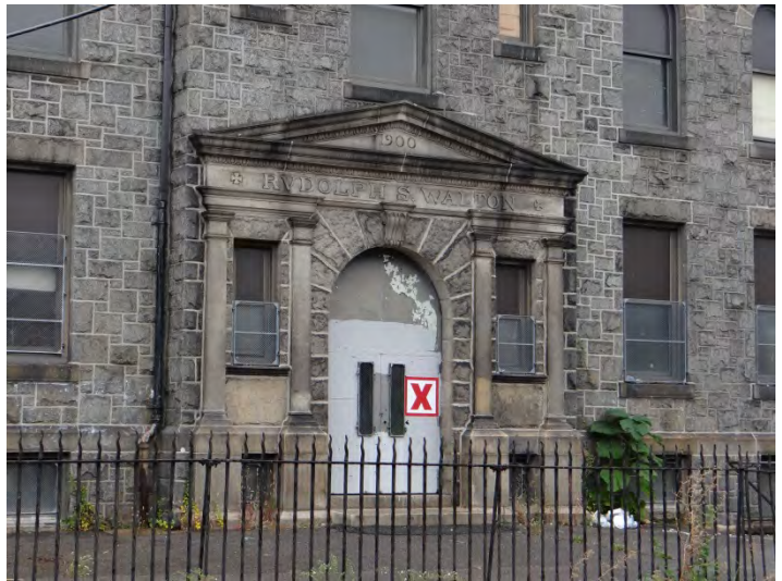
Photo 2: Looking E at entrance on W facade
