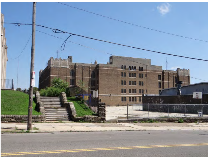
Photo 5: Looking NE at SW façade
