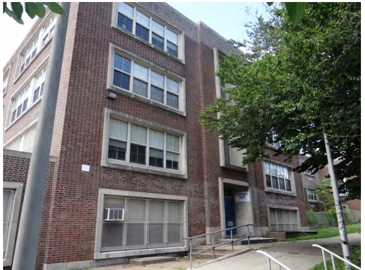
Photo 2: Looking NW at E facade
