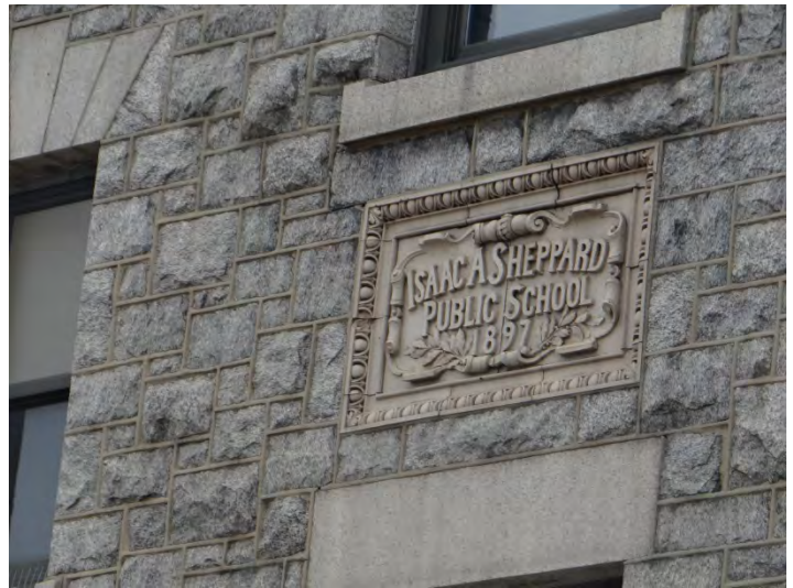
Photo 2: Detail, nameplate/datestone on N facade
