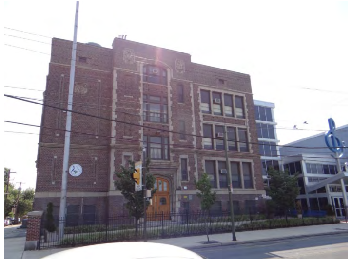
Photo 4: Looking E at W façade
