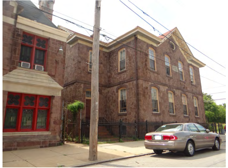
Photo 2: Looking S at N facade
