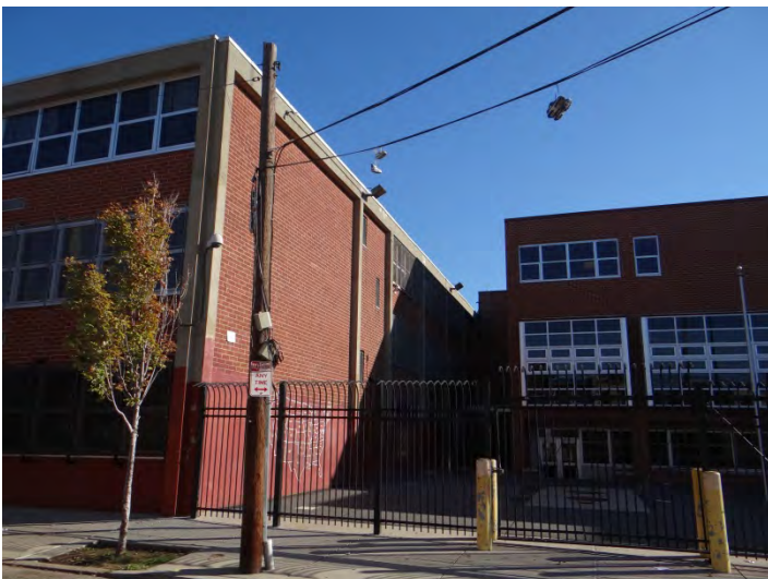
Photo 5: Looking E at center of SW facade
