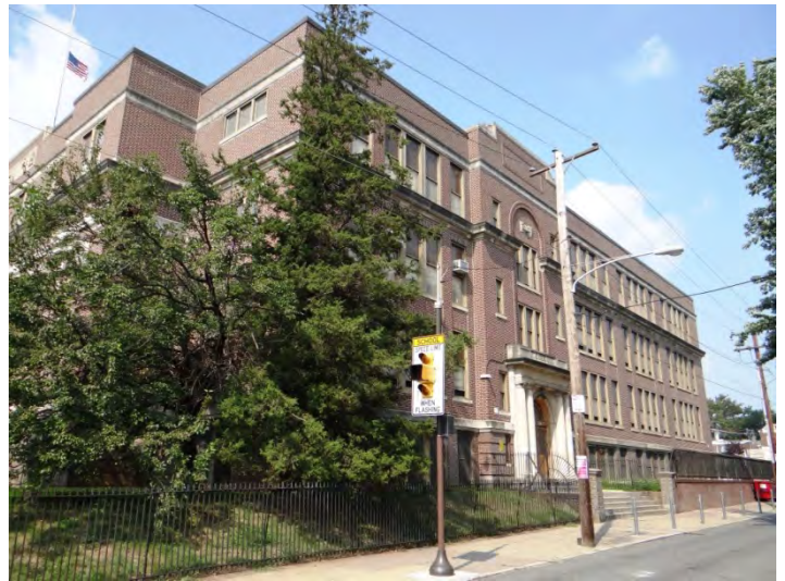
Photo 2: Looking NE at SE facade
