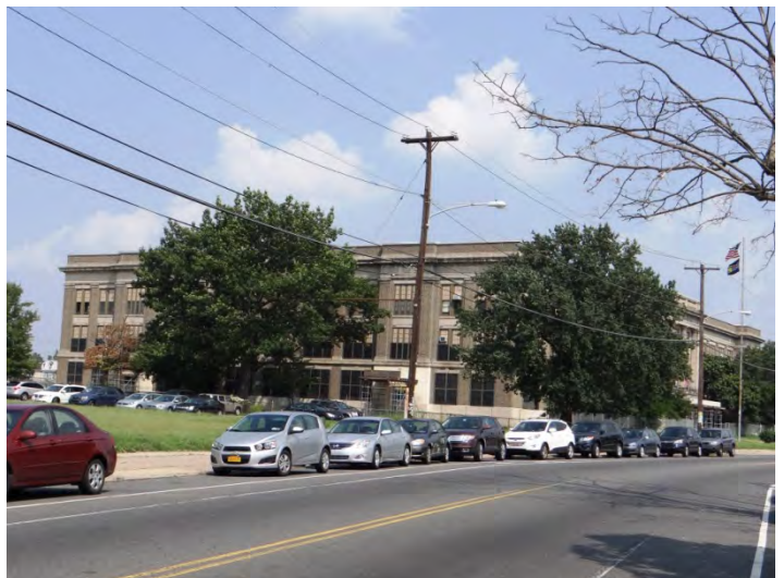
Photo 6: Looking NE at W facade
