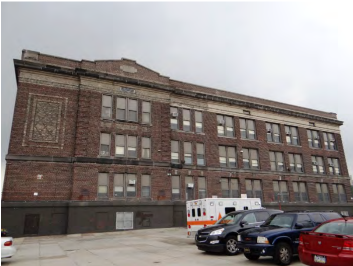
Photo 3: Looking S at N façade
