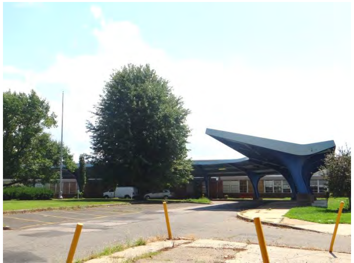
Photo 2: Looking S at N façade
