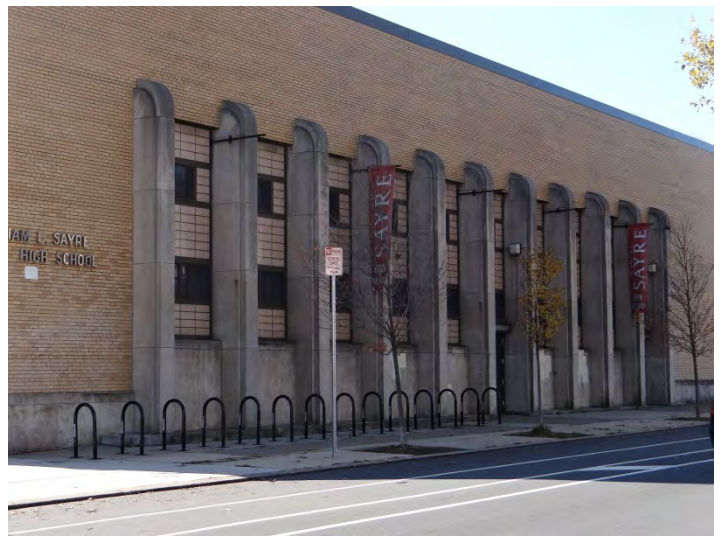
Photo 2: Looking SW at center of main (N) façade
