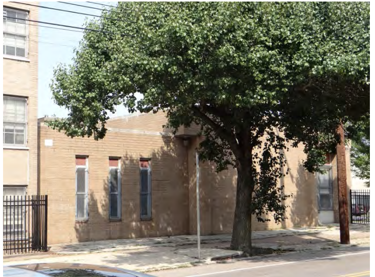
Photo 4: Looking NW at E façade of second addition
