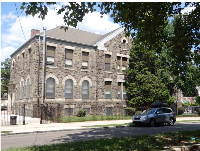
Photo 5: Looking NE at SW (left) and SE (right) facades
