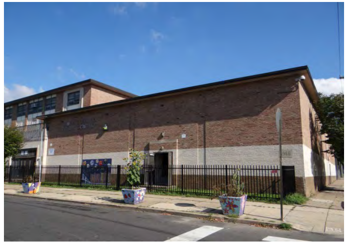
Photo 2: Looking N at main (S) façade of auditorium
