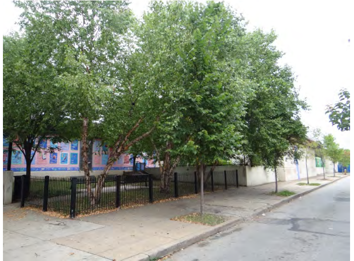
Photo 2: Looking NW at E façade
