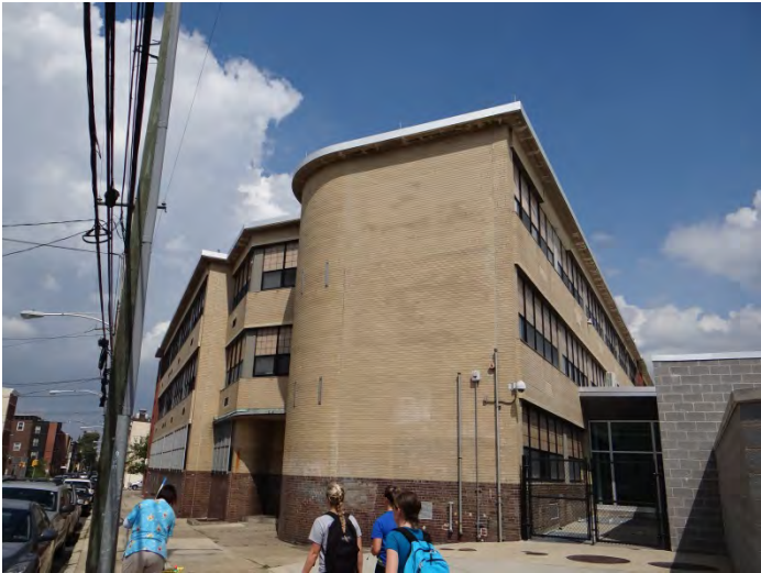
Photo 3: Looking NE at S end of NW façade
