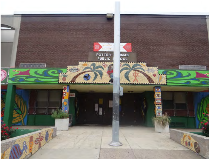
Photo 3: Looking E at main entrance on main (W) façade
