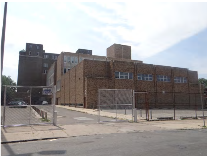
Photo 5: Looking S at rear (NW, right) and NE (left) facades
