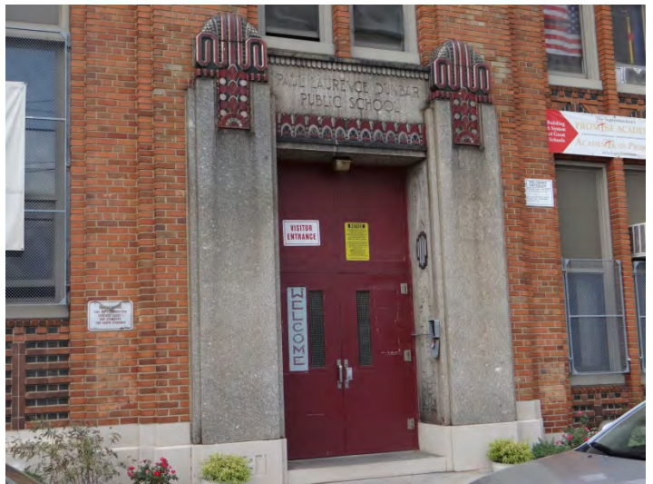
Photo 4: Looking NW at S entrance on main (E) facade
