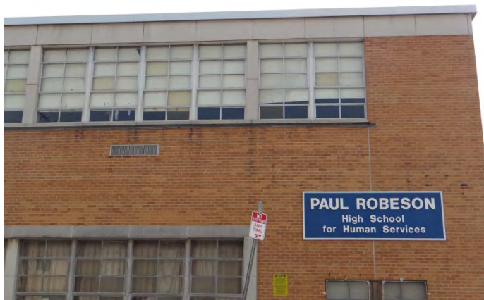
Photo 1: Looking E at W façade
