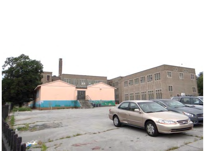
Photo 6: Looking W at rear (E) facade
