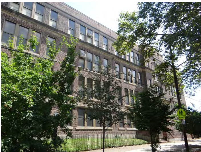
Photo 5: Looking SE at W facade
