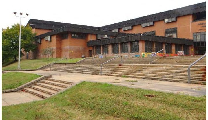
Photo 4: Looking W at S facade
