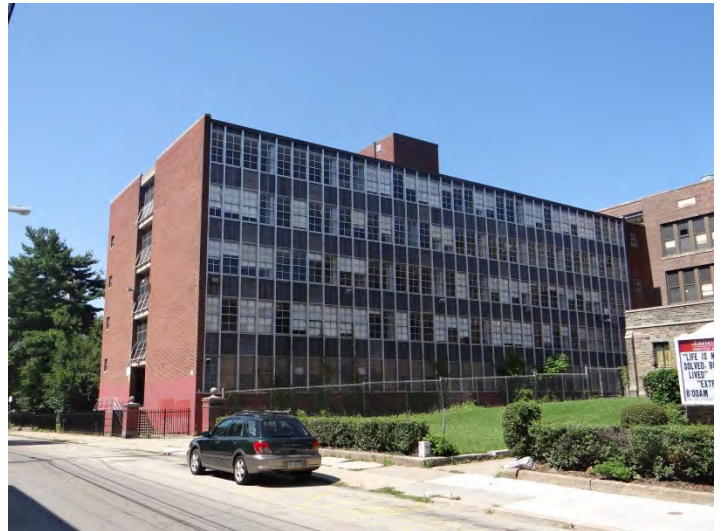
Photo 4: Looking W at S wing on SE facade
