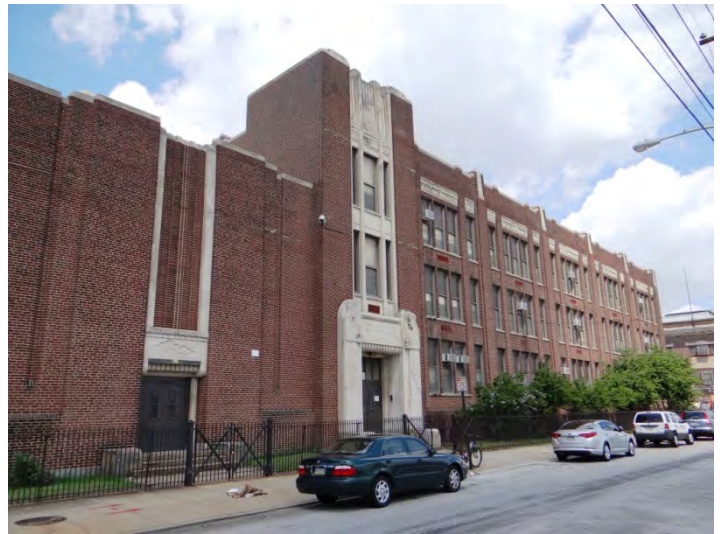
Photo 2: Looking NW at main (E) facade
