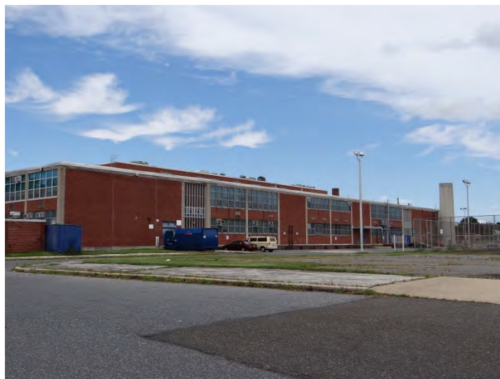
Photo 4: Looking NW at S end of SE facade
