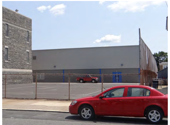
Photo 4: Looking SE at S end of NW facade
