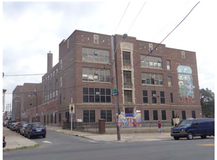
Photo 4: Looking N at W (left) and S (right) facades
