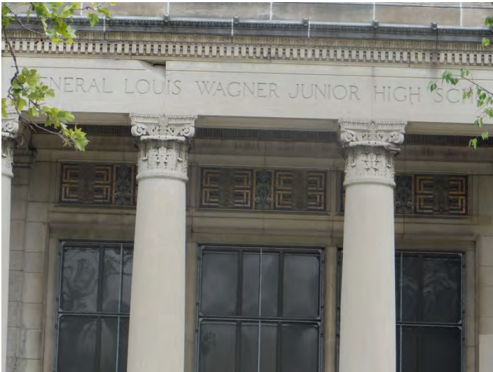
Photo 3: Looking N at main entrance detail on S façade
