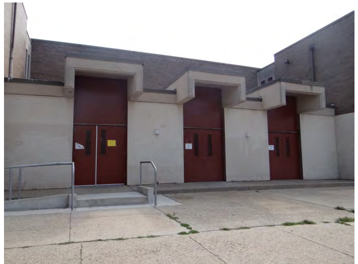
Photo 6: Looking E at W façade of addition
