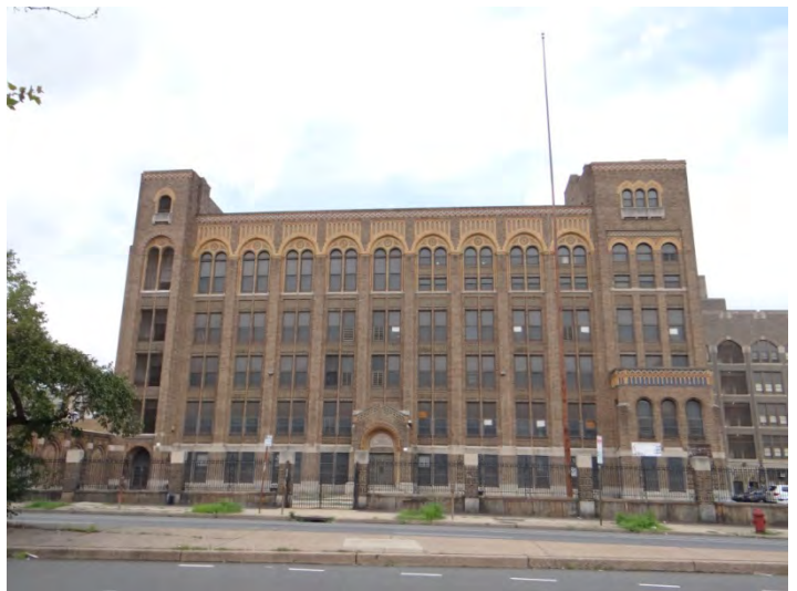
Photo 2: Looking N at main (S) façade
