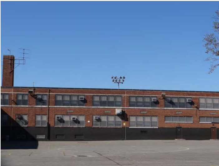
Photo 3: Looking W at center bays of E facade
