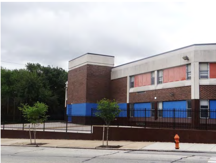
Photo 5: Looking S at NE façade
