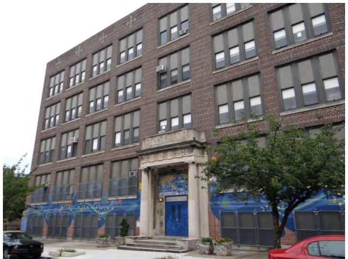
Photo 2: Looking NE at main (W) façade
