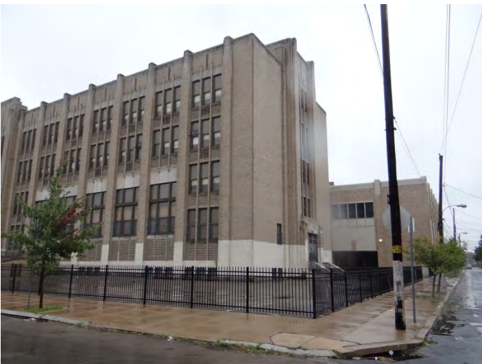
Photo 5: Looking NE at W (left) and rear (S) facades
