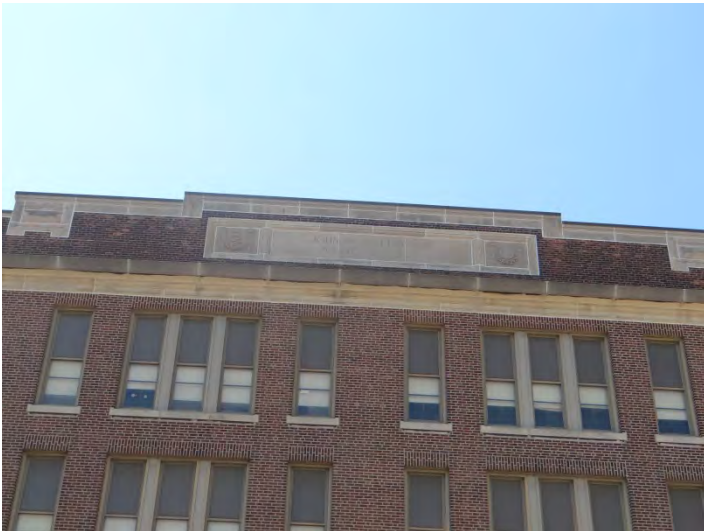
Photo 3: Looking SW at NE façade
