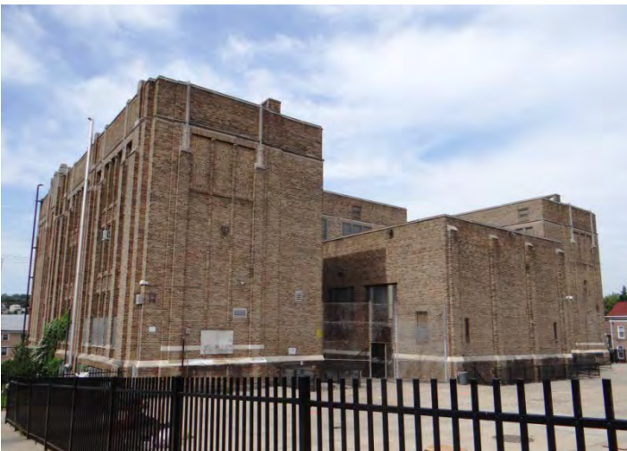
Photo 5: Looking NW at NE facade
