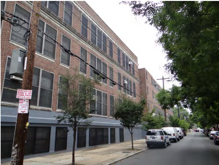
Photo 3: Looking NW at E facade
