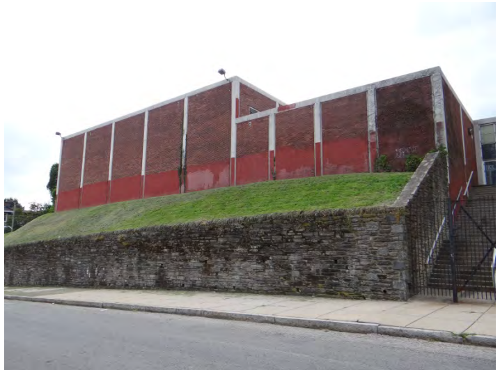
Photo 4: Looking S at NE facade
