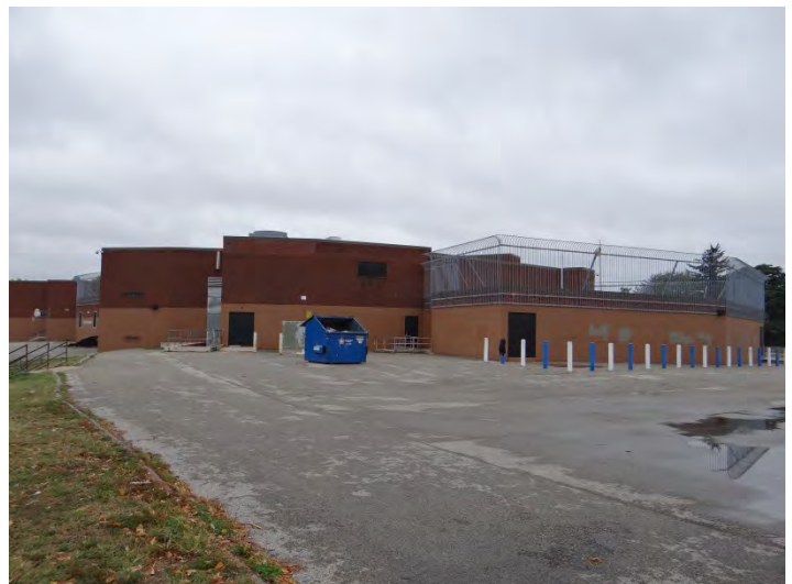
Photo 6: Looking N at SE corner
