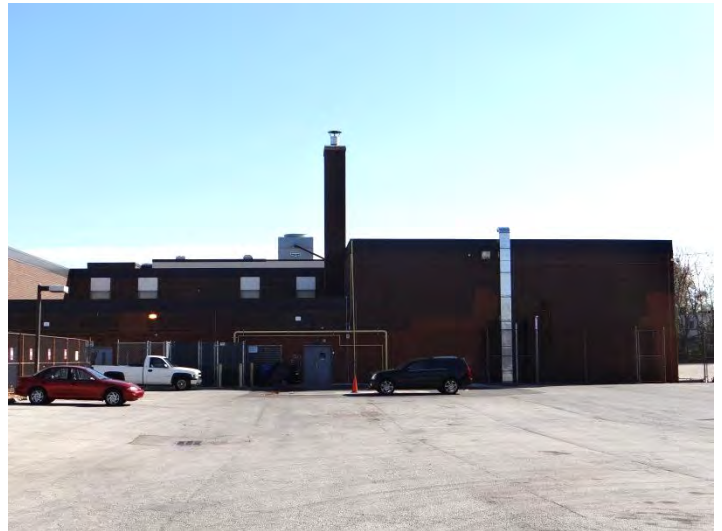
Photo 4: Looking E at S end of W facade
