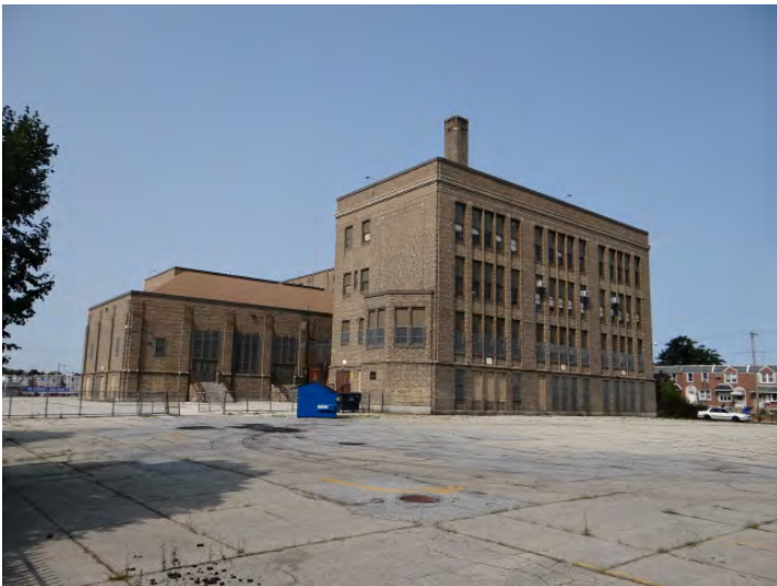
Photo 5: Looking W at NE (right) and rear (SE) facades
