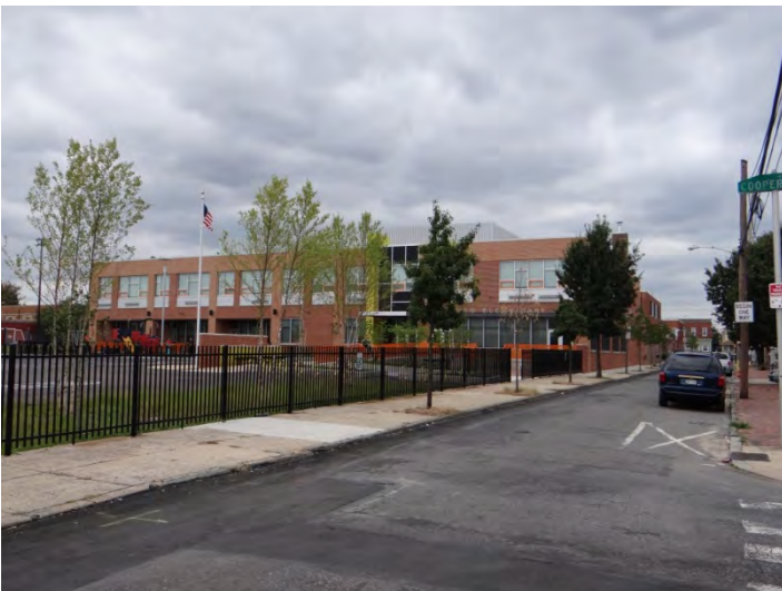
Photo 5: Looking NW at SE façade of recent addition
