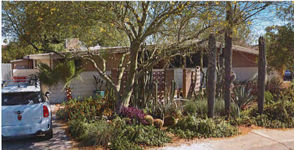
Fig. 3. House at 7307 E. Cypress St., 2018. Source: Google.
