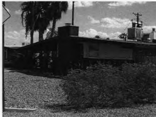
7325 Oak Street – Enclosed windows and addition of fireplace chimney on front of house are inappropriate modifications.
