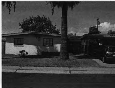
Hip roof style with casement windows. Recessed entry on side. Prominent carport.
