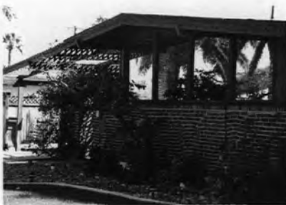
Typical use of glass across the front of the house with wood frames. Entrance is recessed. Clinker brick is used for detailing.
