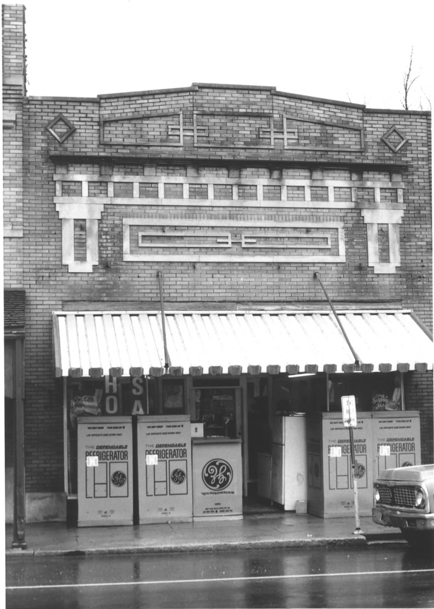
Hodgenville Commercial Historic District La Rue Co. Ky Photo 4
