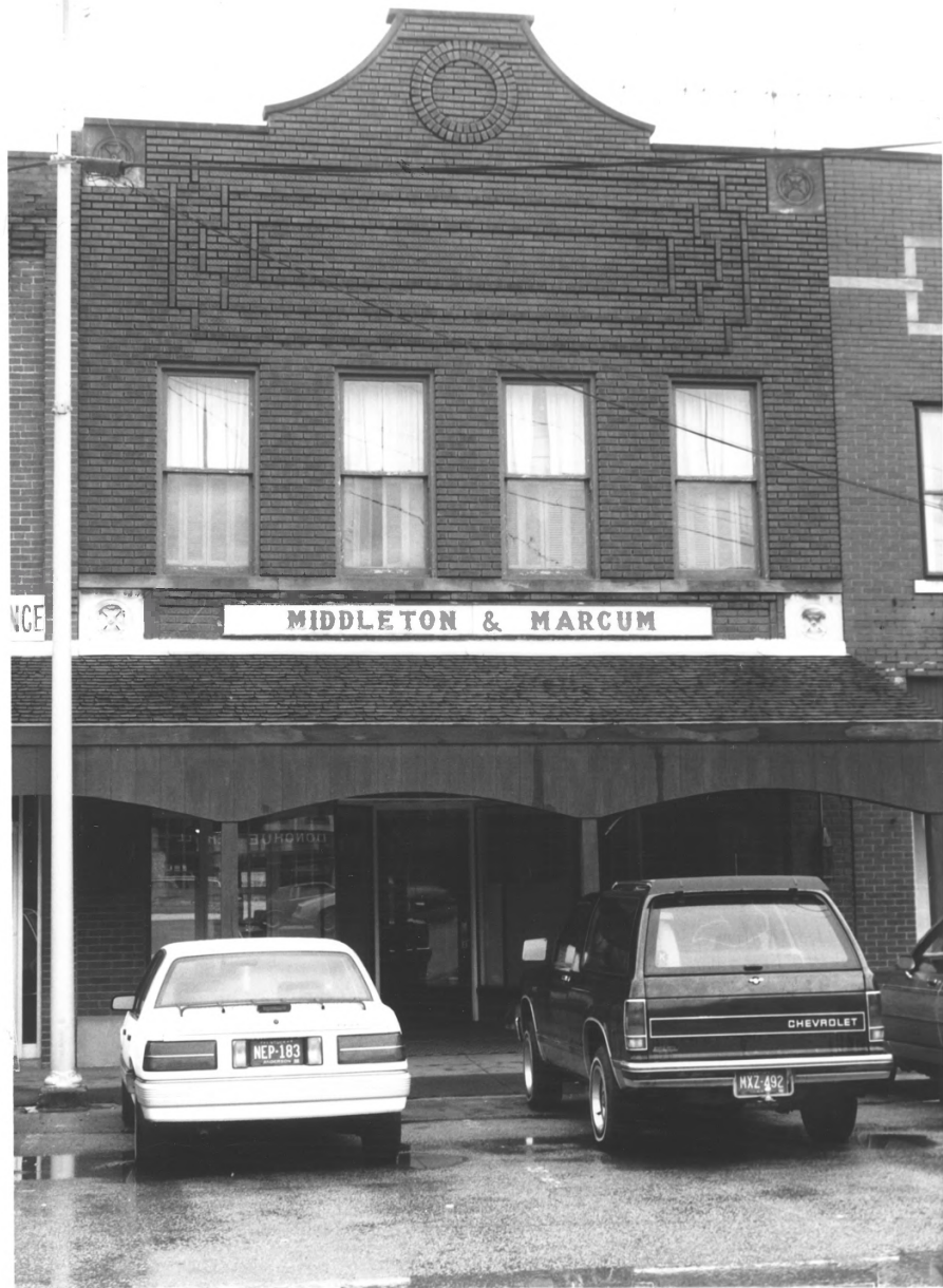
Holgenville Commercial Historic District - LaRue Co., Ky Photo 8
