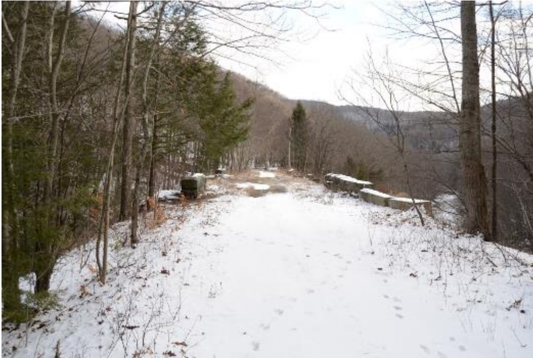
1. Western Railroad Roadbed and deck of Western Railroad Stone Arch Bridge No. 6 (Bridge No. 6) in the Westfield River gorge, looking southeast (downgrade, toward Worcester). John Daly, Public Archeology Laboratory (PAL), 2017.
