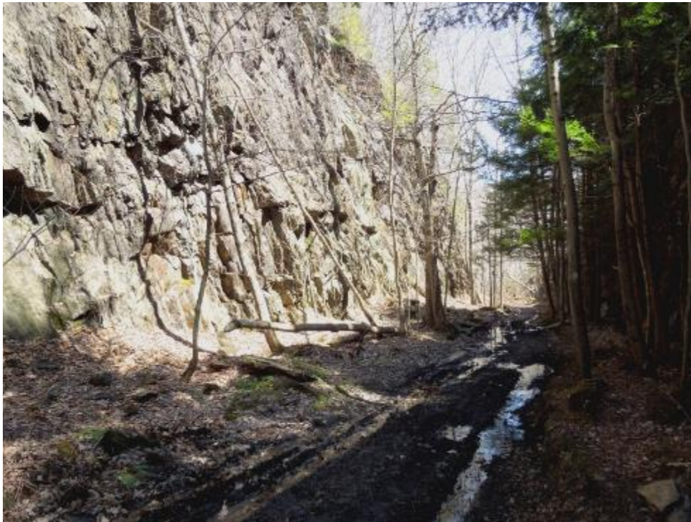
8. View of roadbed at narrow cut, looking northeast. Roger Reed, National Park Service (NPS), National Historic Landmarks Program, 2014.
