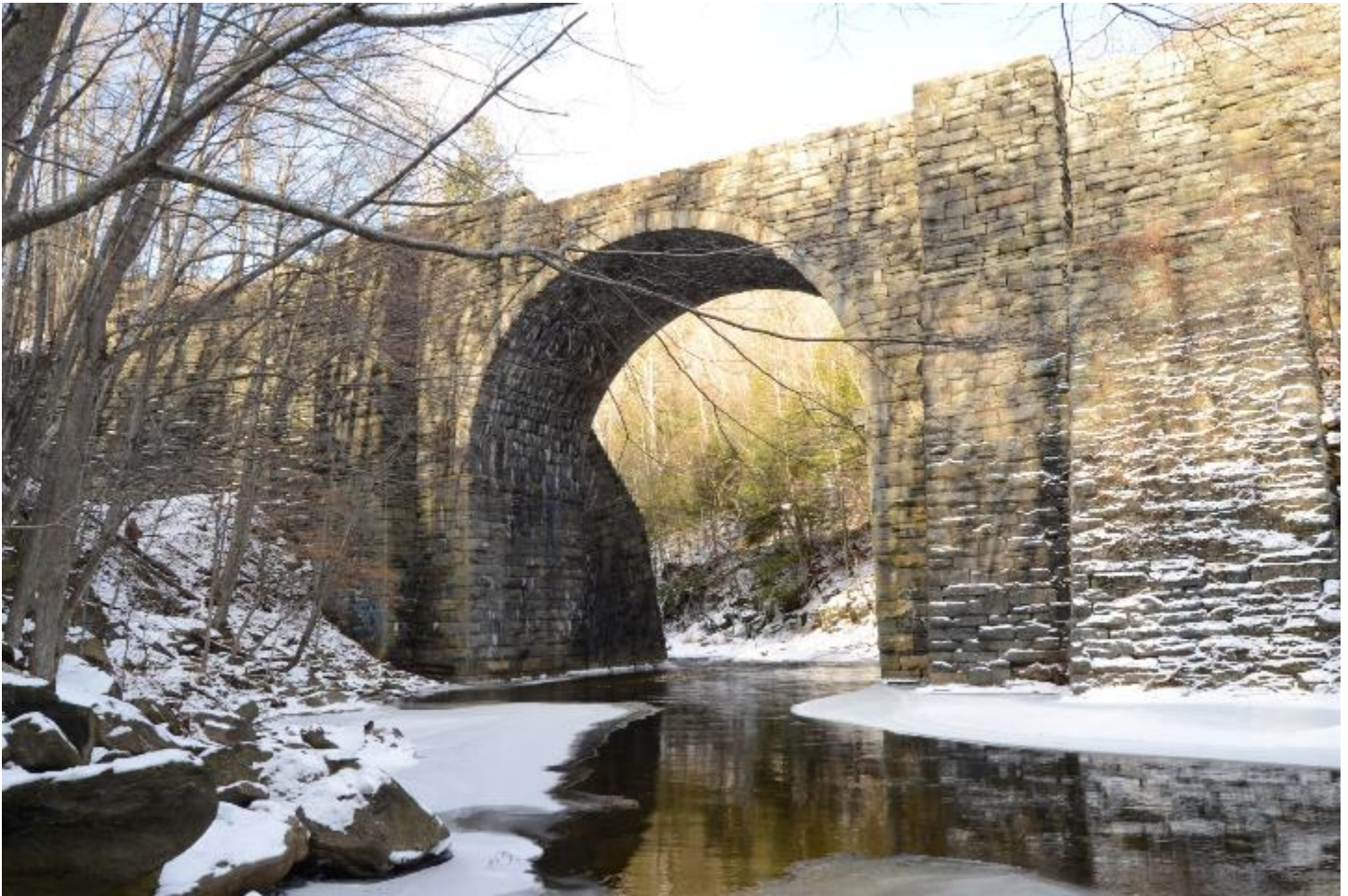
3. Southwest elevation of Bridge No. 6, looking north. John Daly, PAL, 2017.
