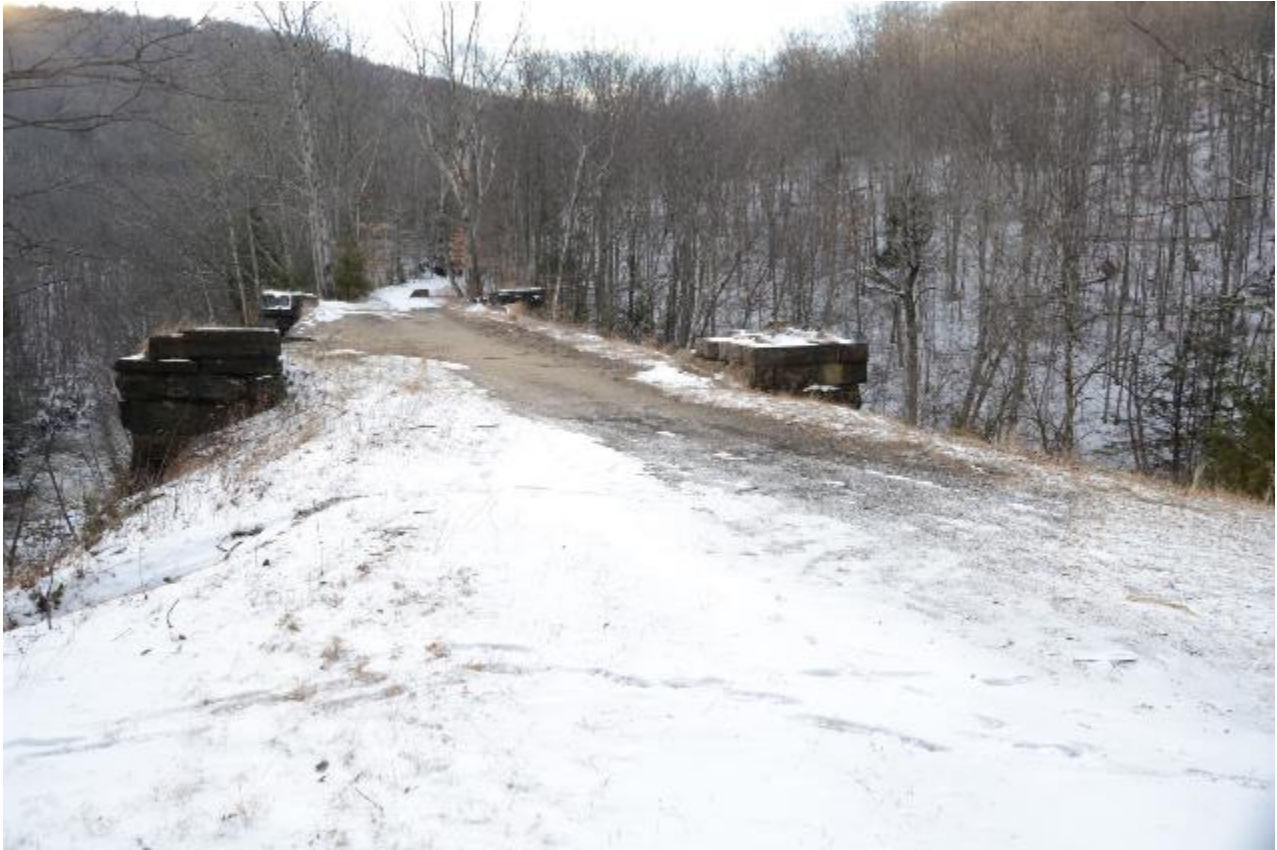
13. Deck view of Bridge No. 5, looking west. John Daly, PAL, 2017.
