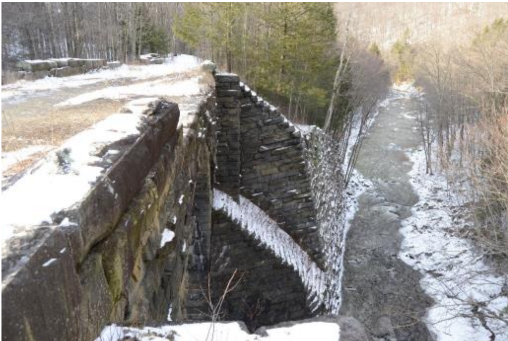
6. Buttresses and revetment/retaining wall at north corner of Bridge No. 6, looking northwest. John Daly, PAL, 2017.
