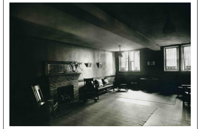
Figure 7. Downstairs Stage/Parlor, c. 1910.
