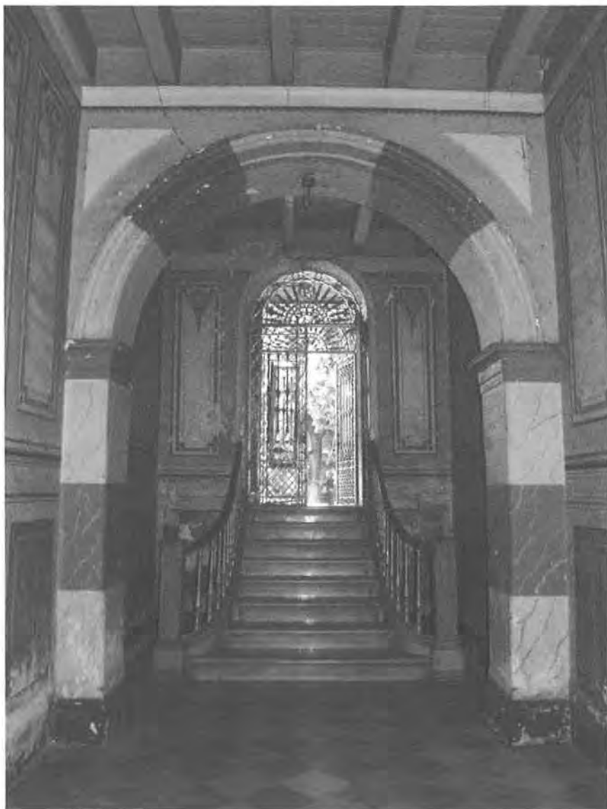
Fig. 4 Detail of zaguan, towards marble flared stair.
