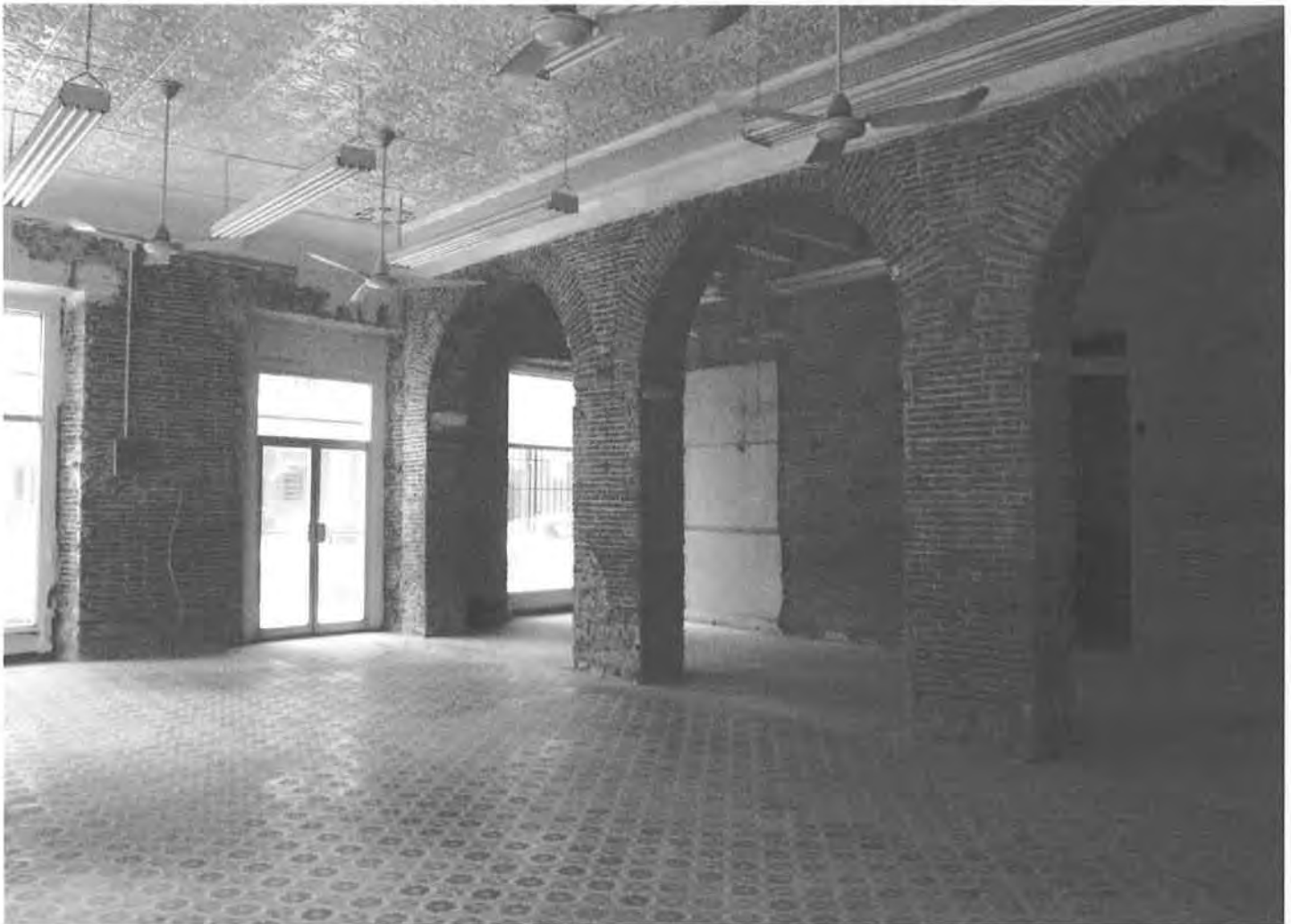
Fig. 3 Exposed brick walls, first floor.
