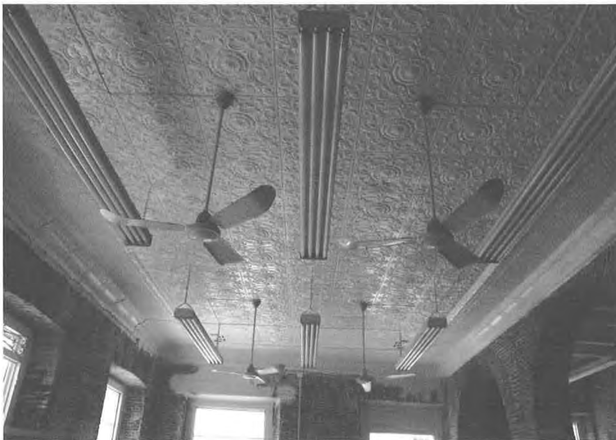
Fig. 2. Decorative tin panels, first floor.
