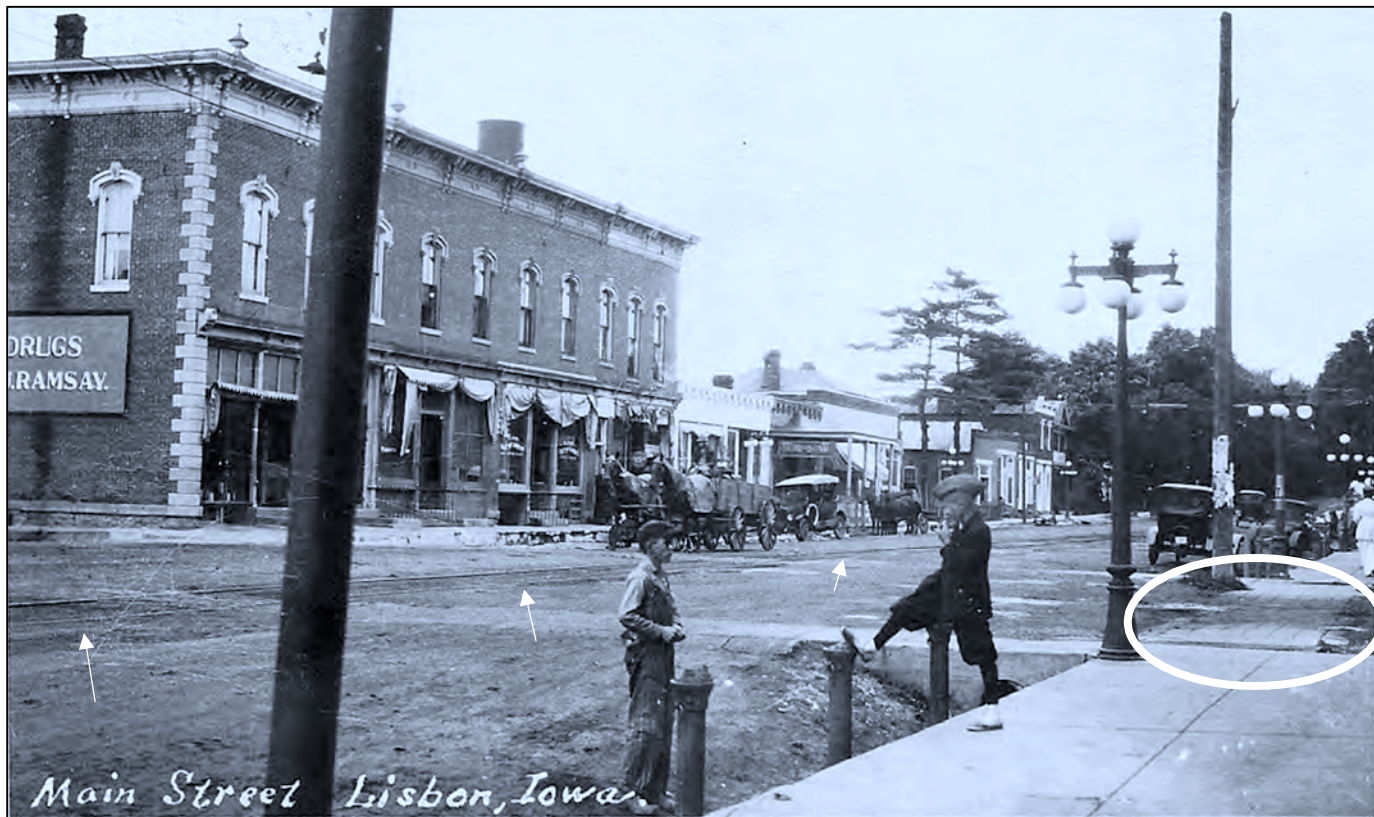
Figure 7. Photograph of Main Street in 1921 showing the interurban tracks (white arrows point to the tracks) in unpaved or macadam streets with a cobblestone cross walk on the south side of Main Street at the Washington Street intersection (circled). View is looking ENE. Note the concrete sidewalks and electric street lights, which were installed in 1912. Obtained from the Lisbon History Center collections.
