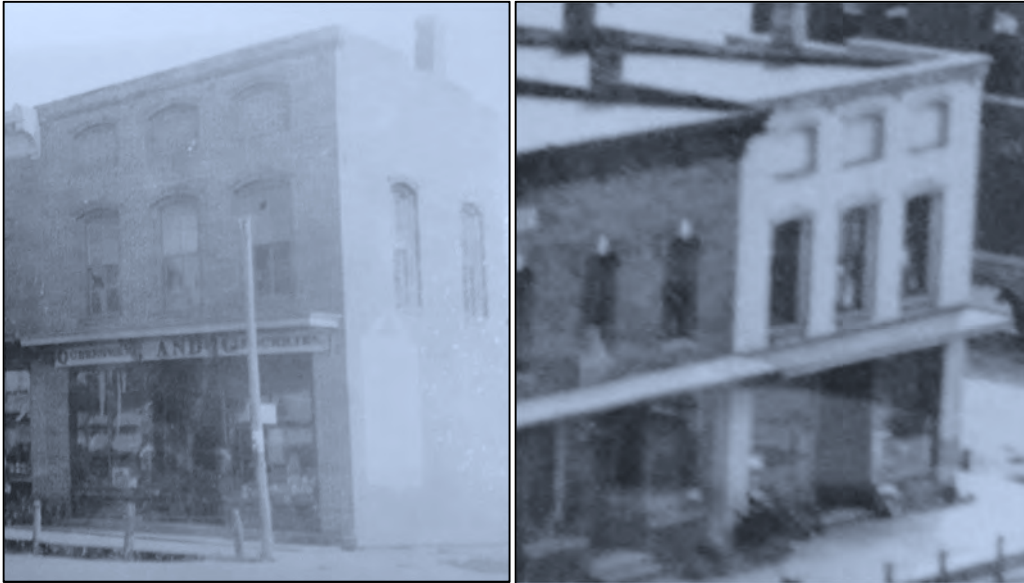
Left: Circa 1890 view of 101 E. Main looking SSE and showing the brick walls unpainted and the presence of the overhang with metal brackets above the storefront; Right: Circa 1909 view of 101 E. Main looking WSW (right) showing the painted exterior.
