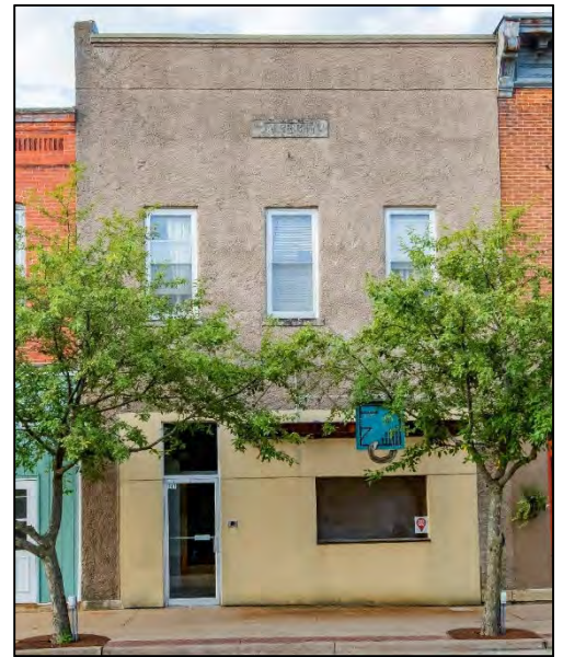
117 E. Main Street looking S, 6-10-2018.
