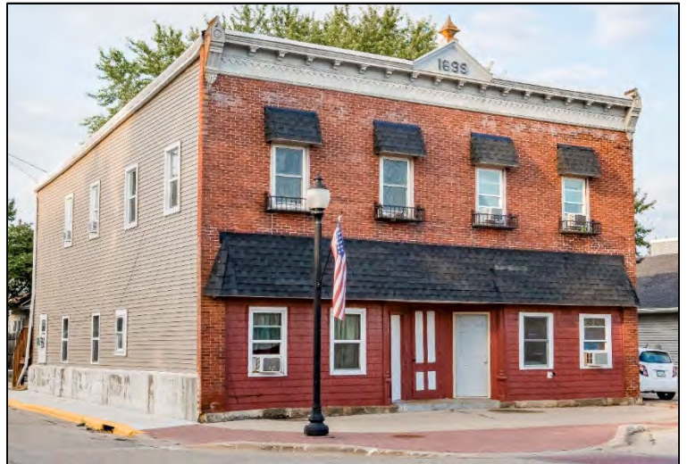
145 E. Main Street looking SSW, 6-10-2018.
