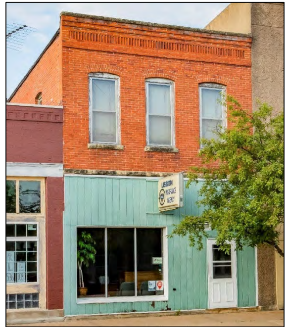
119 E. Main Street looking SSW, 6-10-2018.
