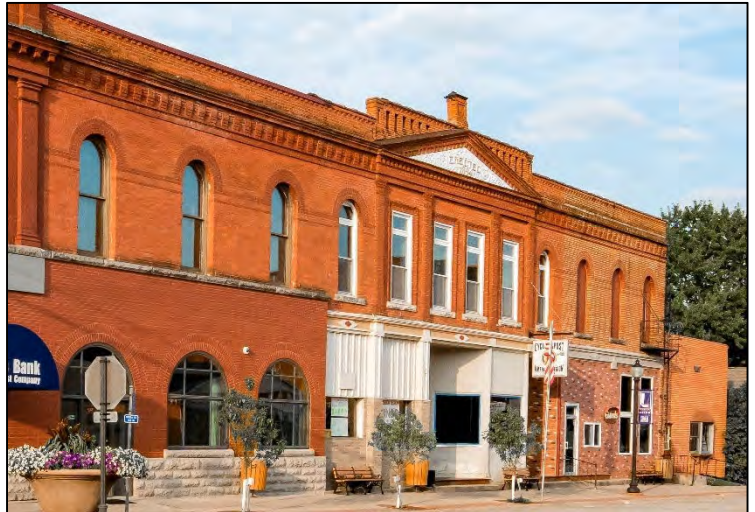
W1/2 103, 111-119 W. Main Street looking South, 6-10-2018.
