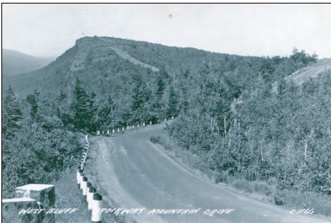
Figure 7. Historic Photograph (c.1940), View West from Beaver Dam Overlook of Wood Delineator Posts
