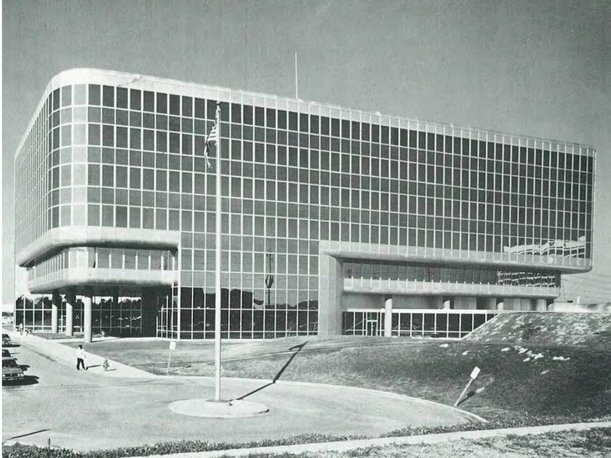
Figure H. View of the south façade of the Federal Building, ca. 1973. (Image from Cesar Pelli by John Pastier)
