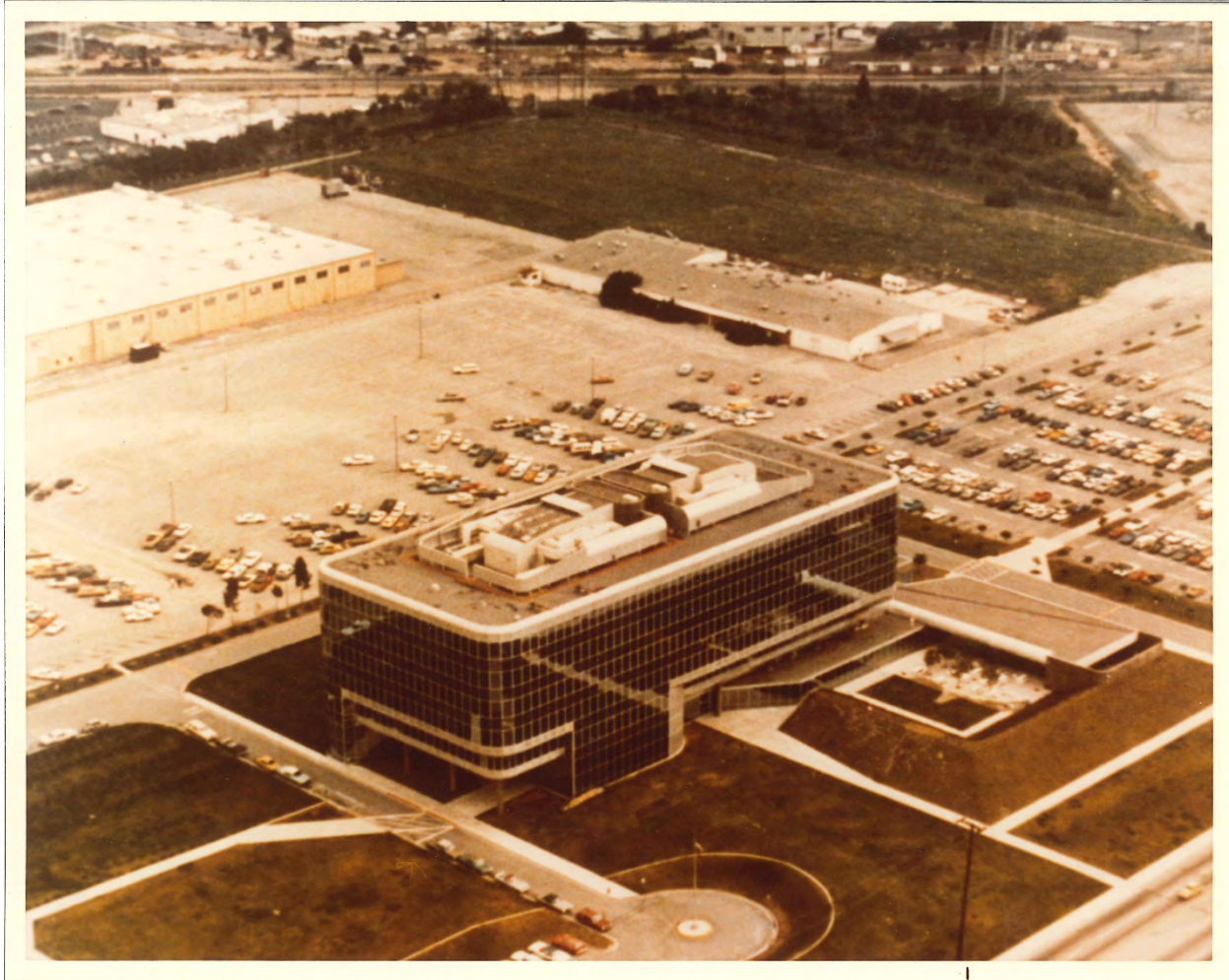
Figure J. Aerial of the Federal Building facing northeast at portions of the south and west façades, circa 1975. (Photograph courtesy of GSA)
