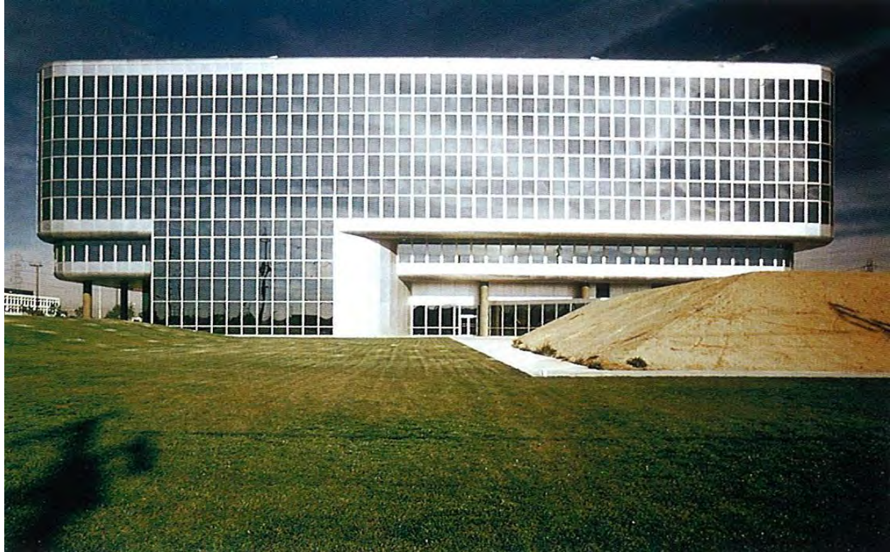
Figure I. South façade of the Federal Building shortly after completion in 1973. (Image from A.J. Lumsden: Selected and Current Works )
