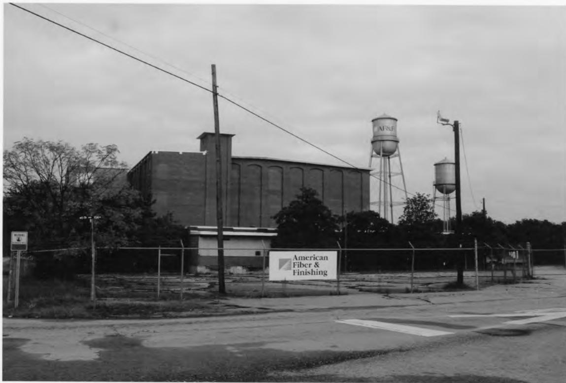
3. Oakland Mill 2802 Fair Avenue, Newberry Newberry County, South Carolina
