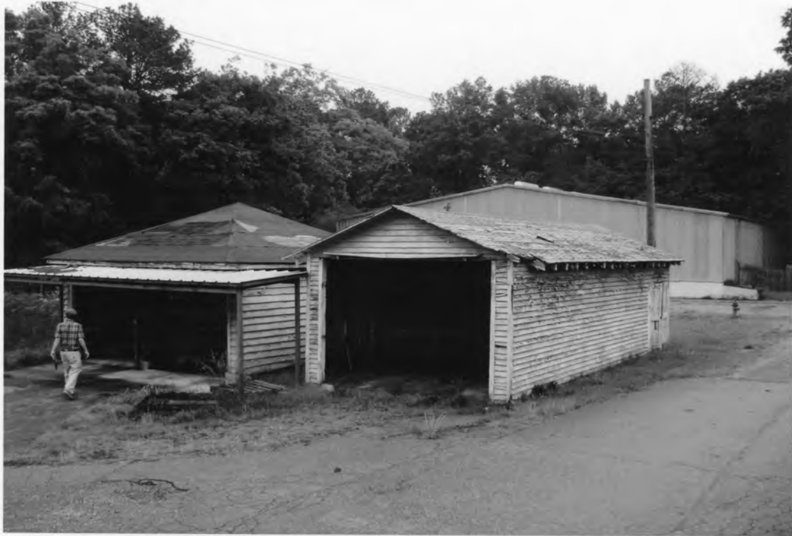
26. Oakland Mill 2802 Fair Avenue, Newberry Newberry County, South Carolina
