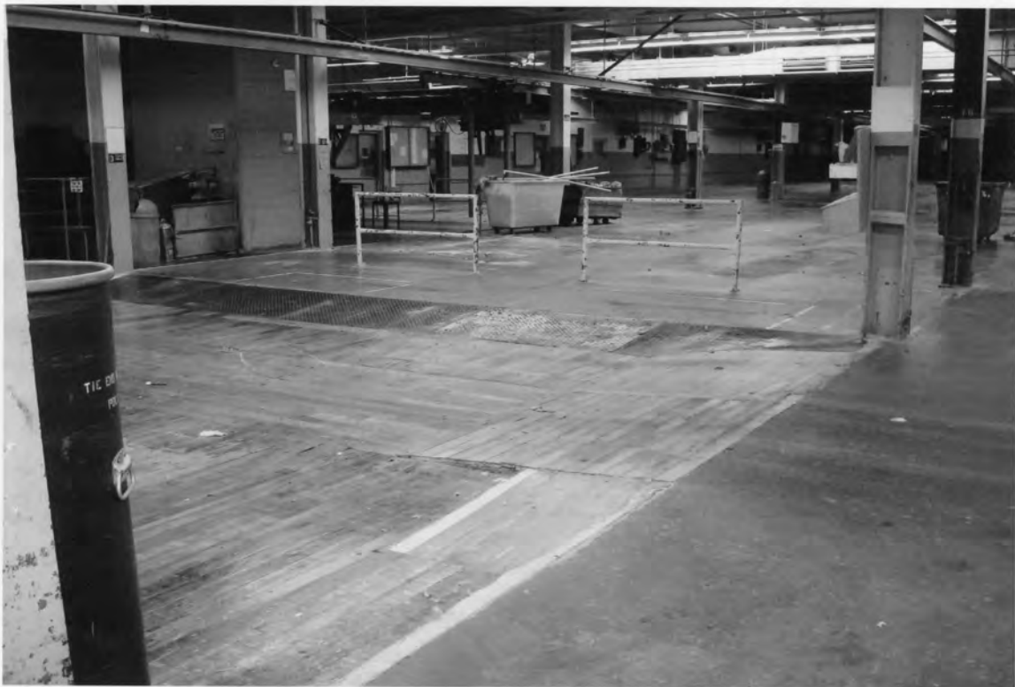
37. Oakland Mill 2802 Fair Avenue, Newberry Newberry County, South Carolina
