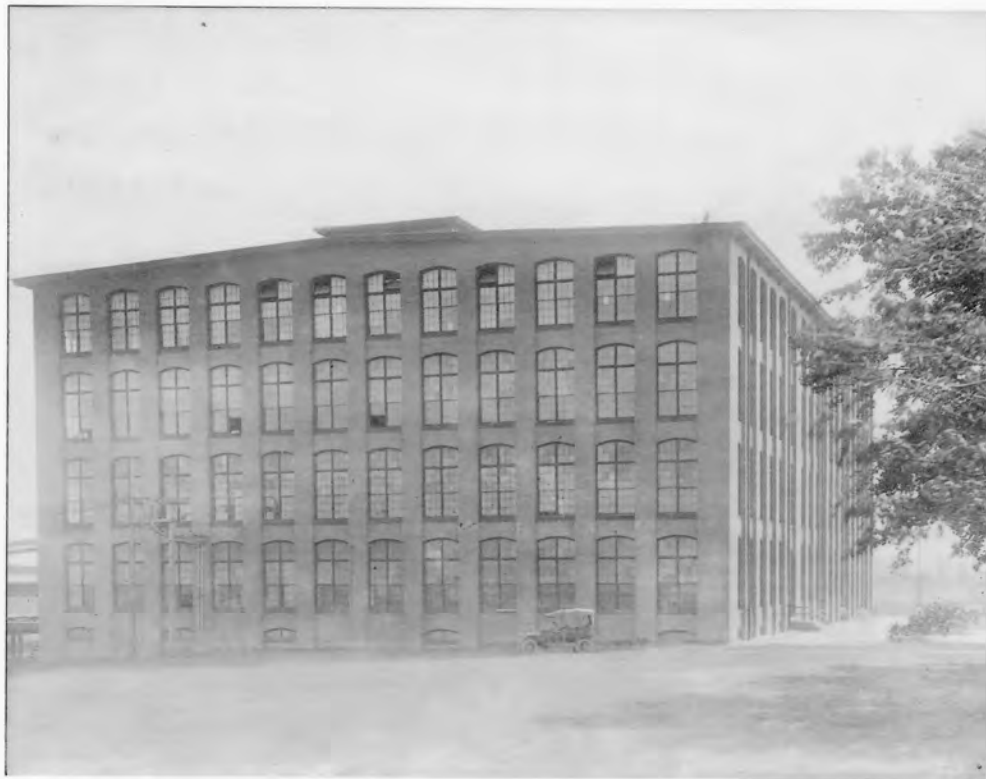
41. Oakland Mill 2802 Fair Avenue, Newberry Newberry County, South Carolina
