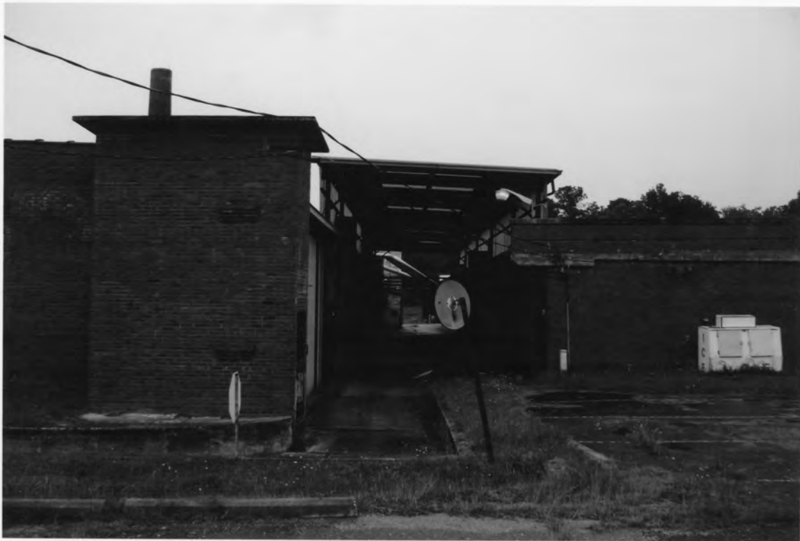
23. Oakland Mill 2802 Fair Avenue, Newberry Newberry County, South Carolina
