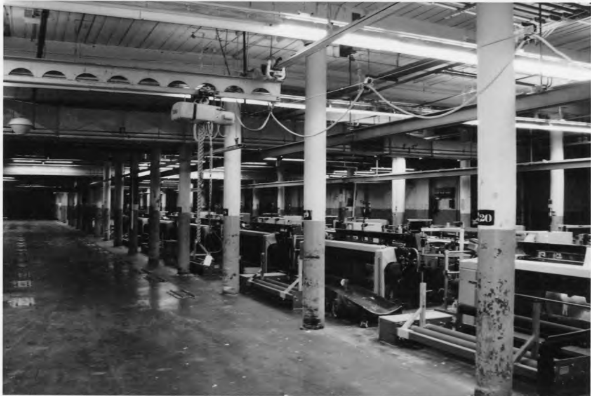
38. Oakland Mill 2802 Fair Avenue, Newberry Newberry County, South Carolina
