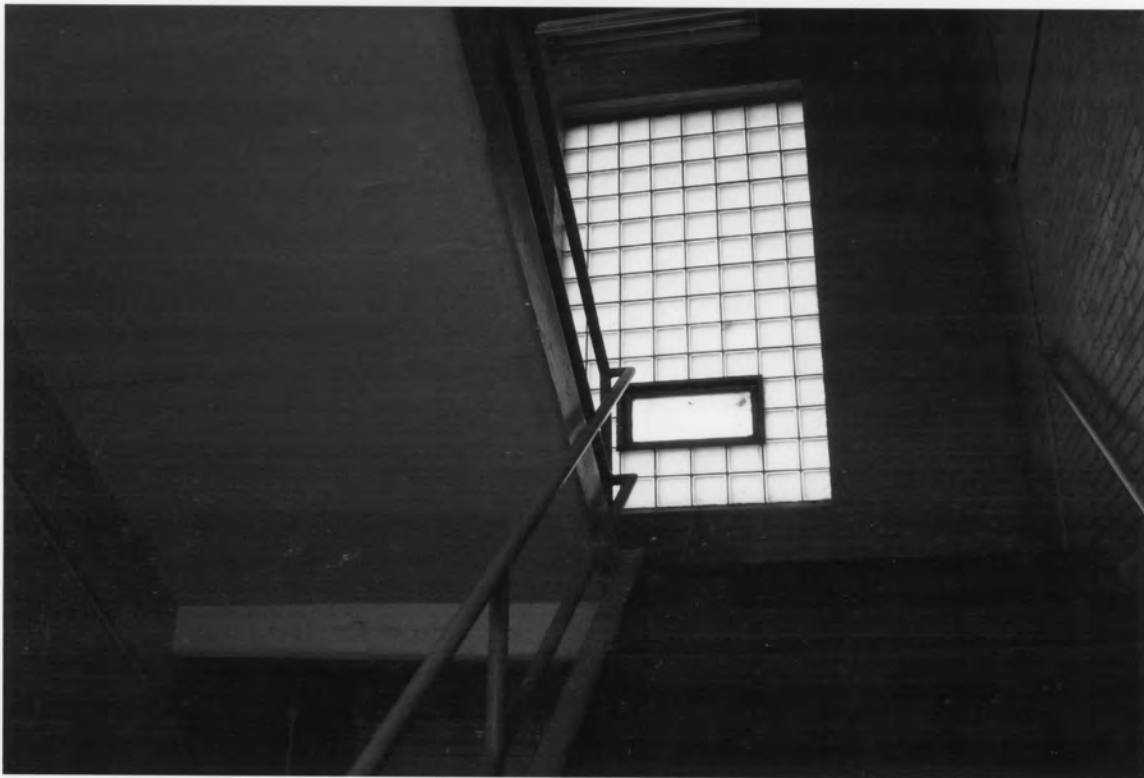
32. Oakland Mill 2802 Fair Avenue, Newberry Newberry County, South Carolina
