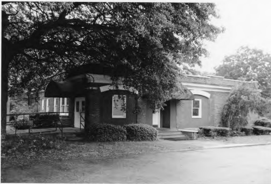
11. Oakland Mill 2802 Fair Avenue, Newberry Newberry County, South Carolina
