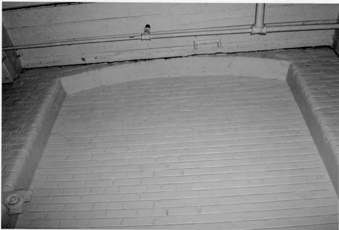
33. Oakland Mill 2802 Fair Avenue, Newberry Newberry County, South Carolina
