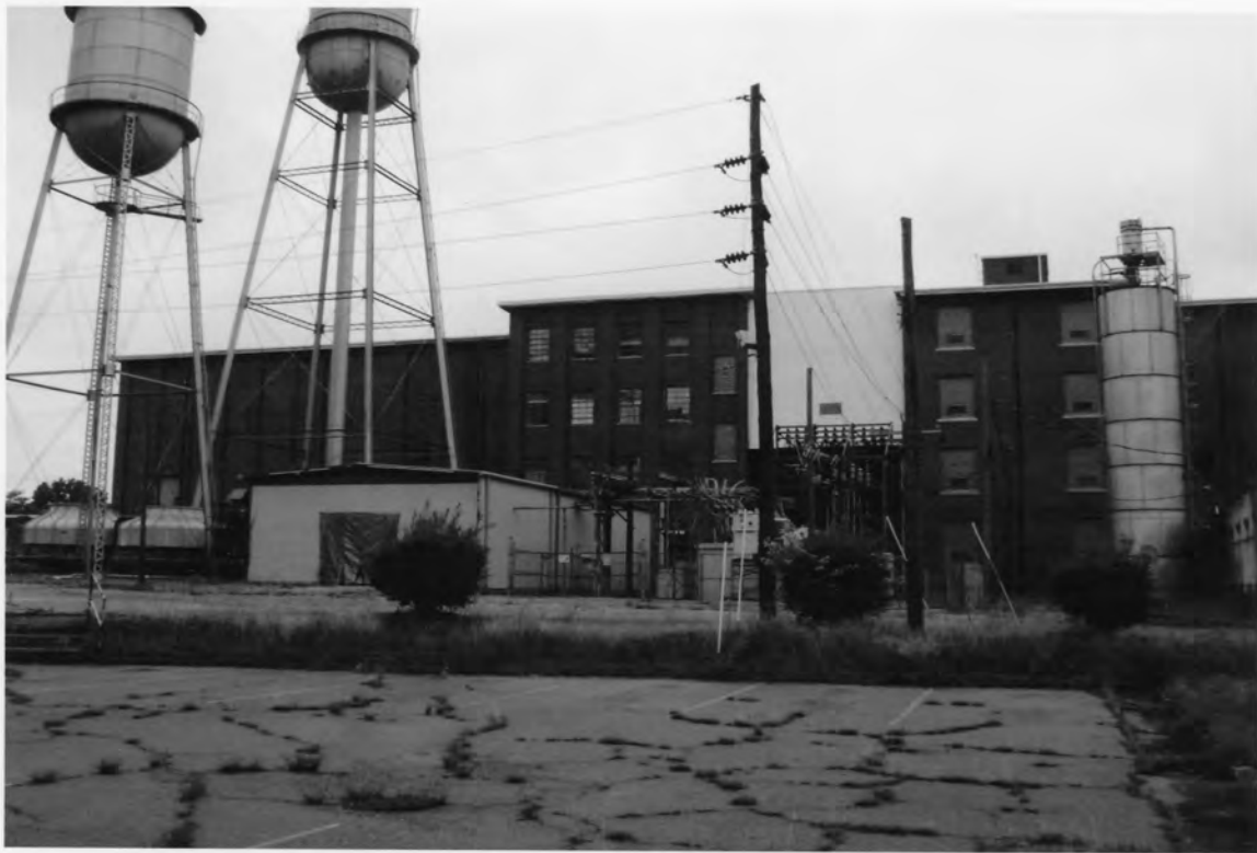
5. Oakland Mill 2802 Fair Avenue, Newberry Newberry County, South Carolina
