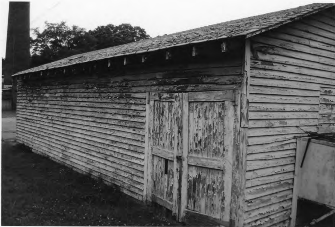
27. Oakland Mill 2802 Fair Avenue, Newberry Newberry County, South Carolina
