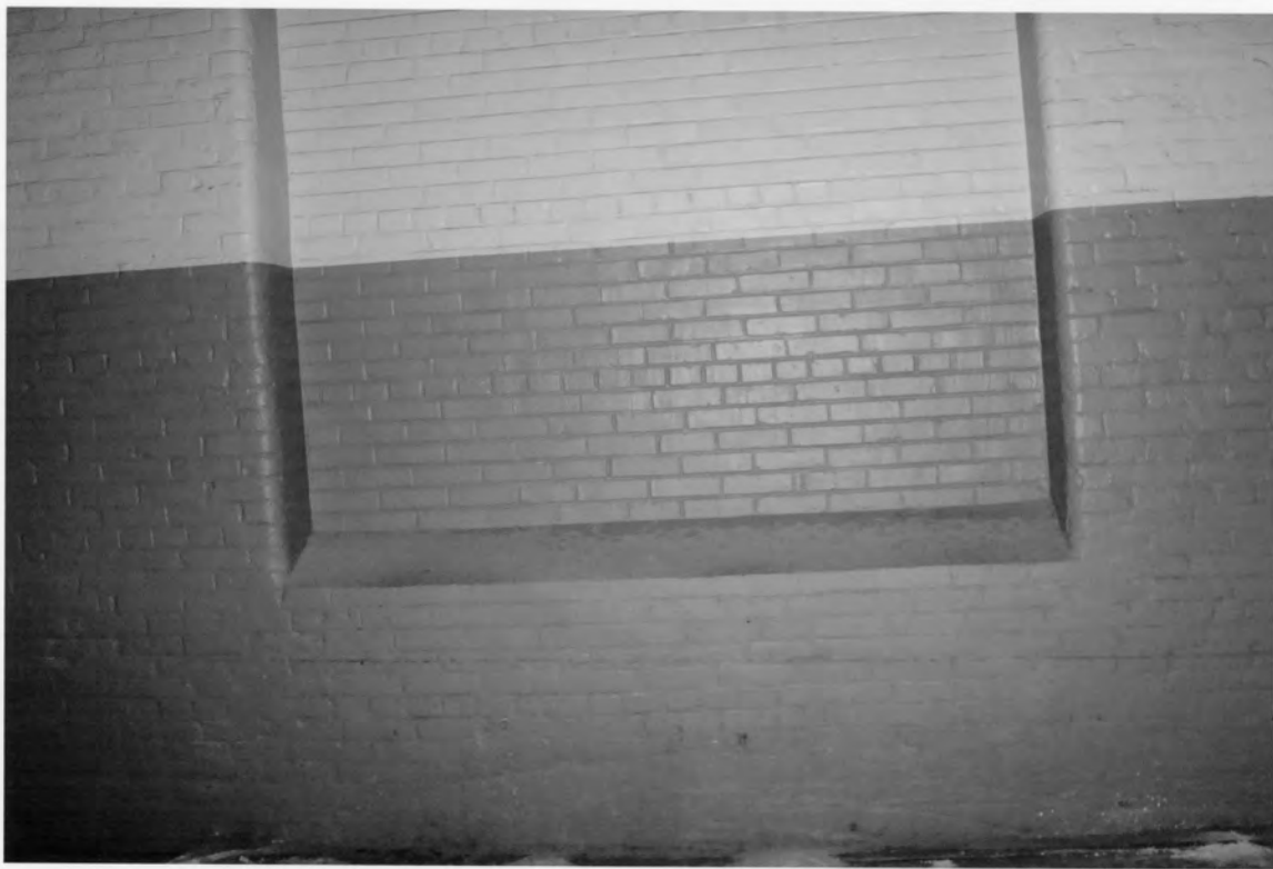
34. Oakland Mill 2802 Fair Avenue, Newberry Newberry County, South Carolina
