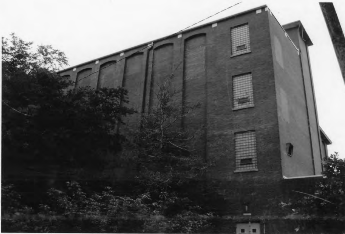
2. Oakland Mill 2802 Fair Avenue, Newberry Newberry County, South Carolina
