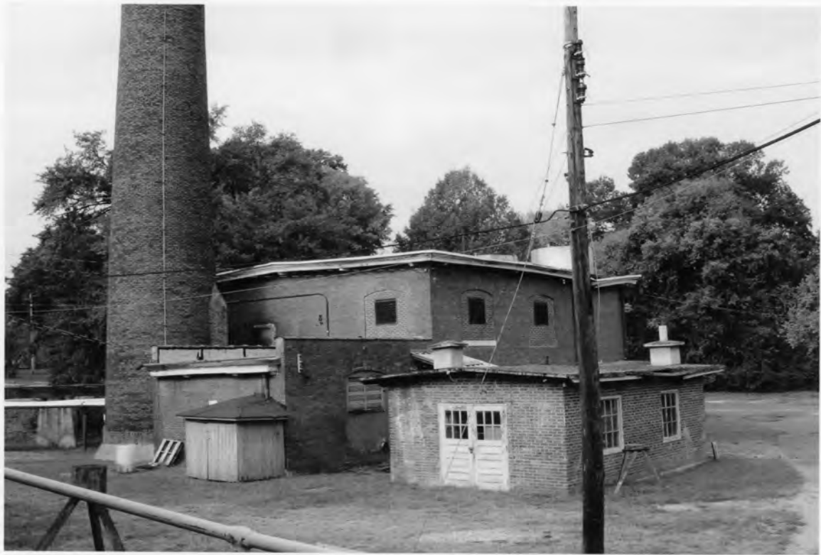
14. Oakland Mill 2802 Fair Avenue, Newberry Newberry County, South Carolina
