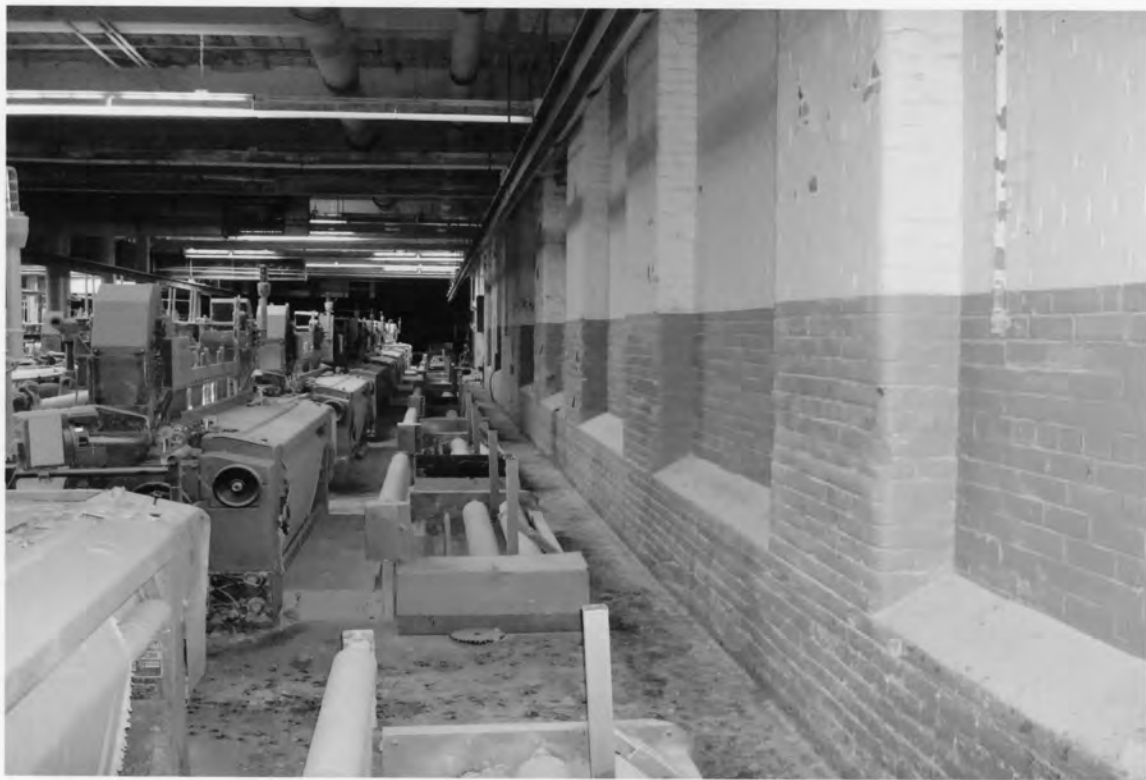
30. Oakland Mill 2802 Fair Avenue, Newberry Newberry County, South Carolina
