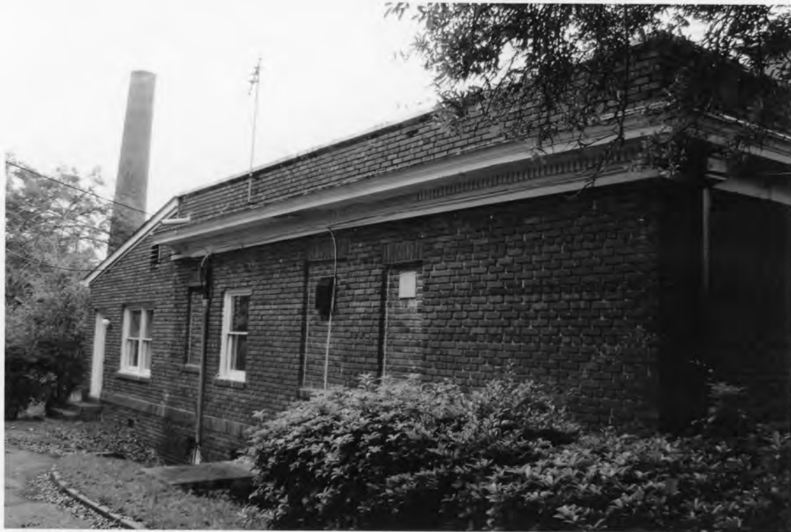
12. Oakland Mill 2802 Fair Avenue, Newberry Newberry County, South Carolina
