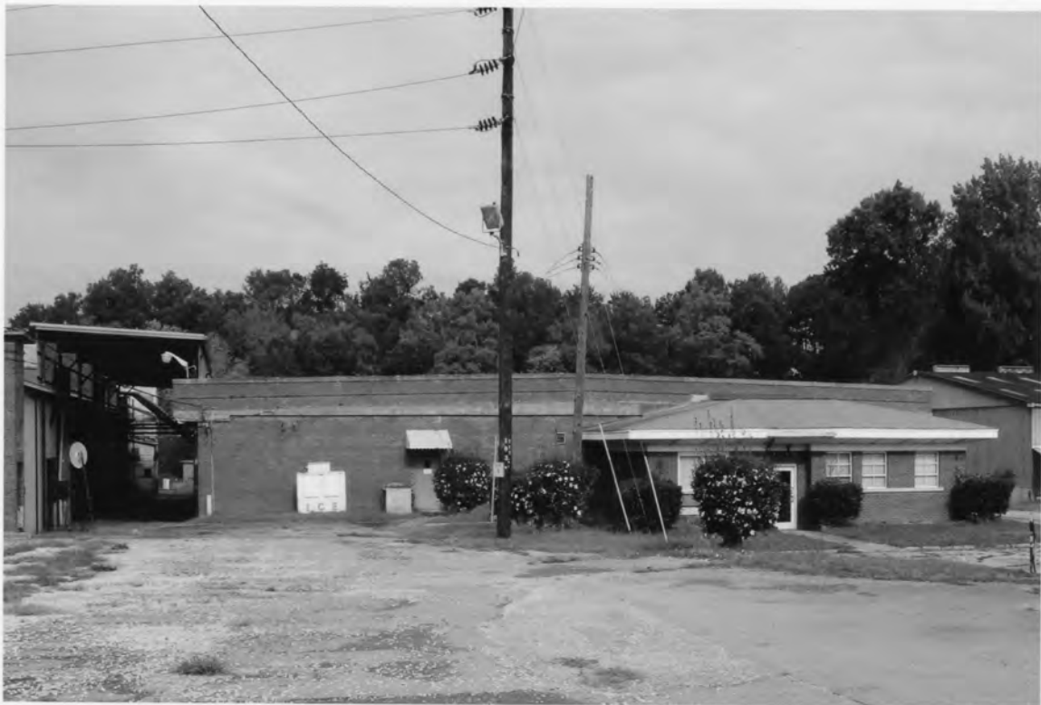
21. Oakland Mill 2802 Fair Avenue, Newberry Newberry County, South Carolina
