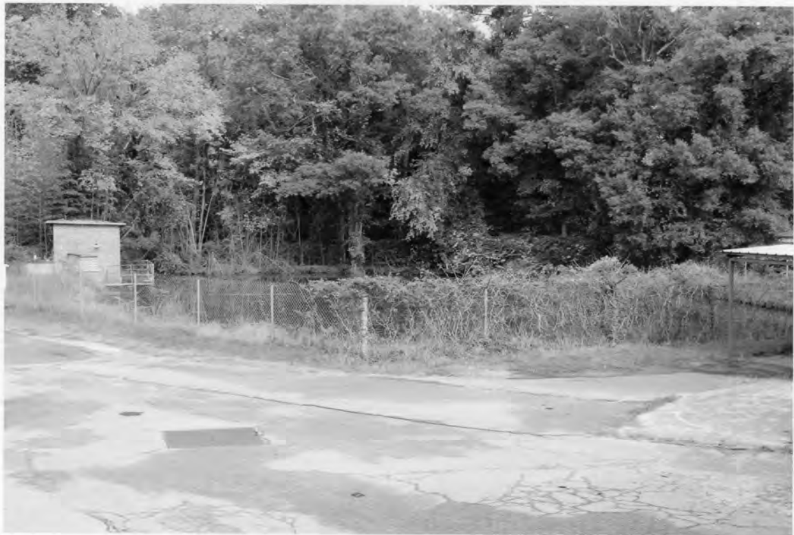
28. Oakland Mill 2802 Fair Avenue, Newberry Newberry County, South Carolina
