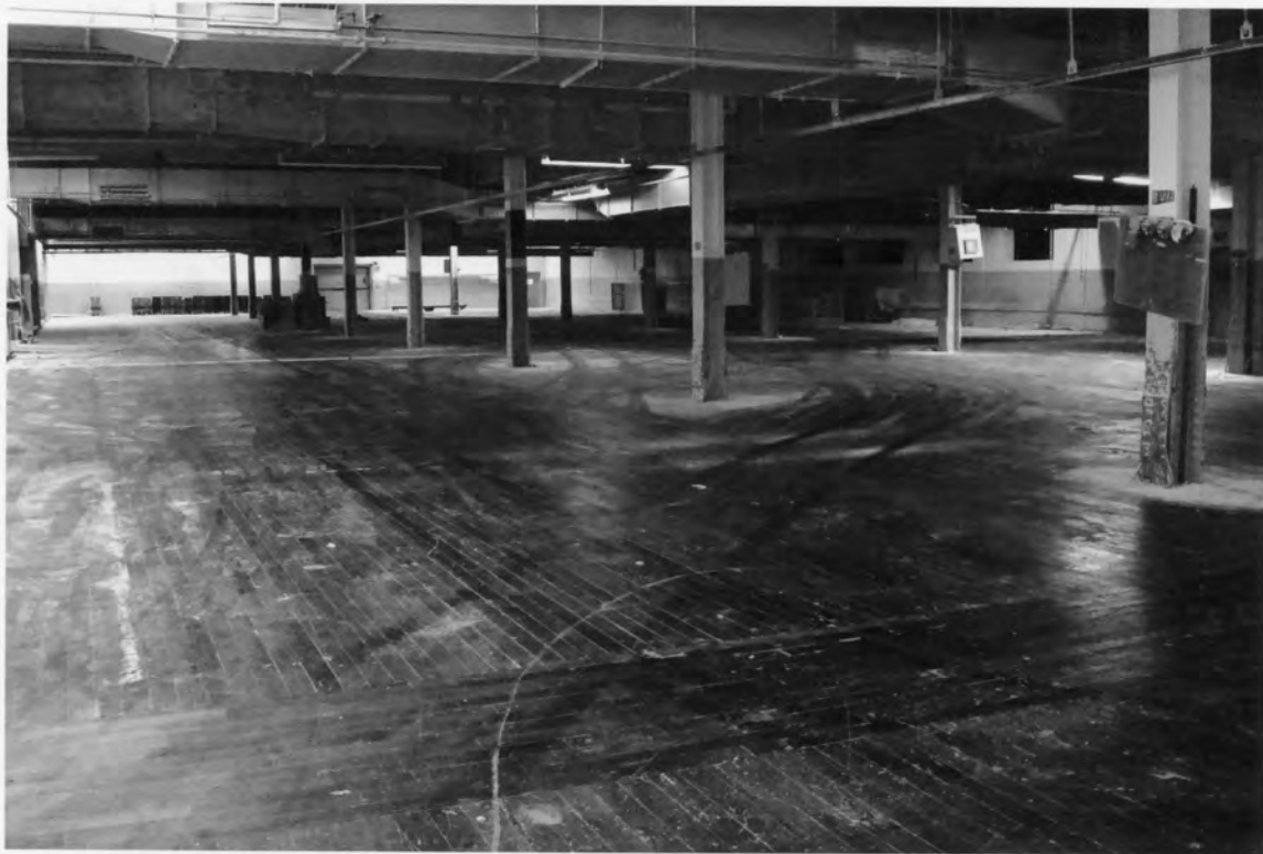
39. Oakland Mill 2802 Fair Avenue, Newberry Newberry County, South Carolina
