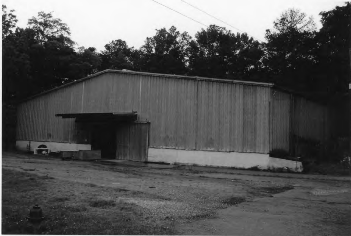
24. Oakland Mill 2802 Fair Avenue, Newberry Newberry County, South Carolina
