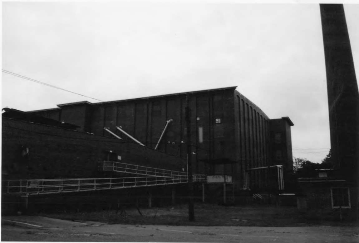
17. Oakland Mill 2802 Fair Avenue, Newberry Newberry County, South Carolina
