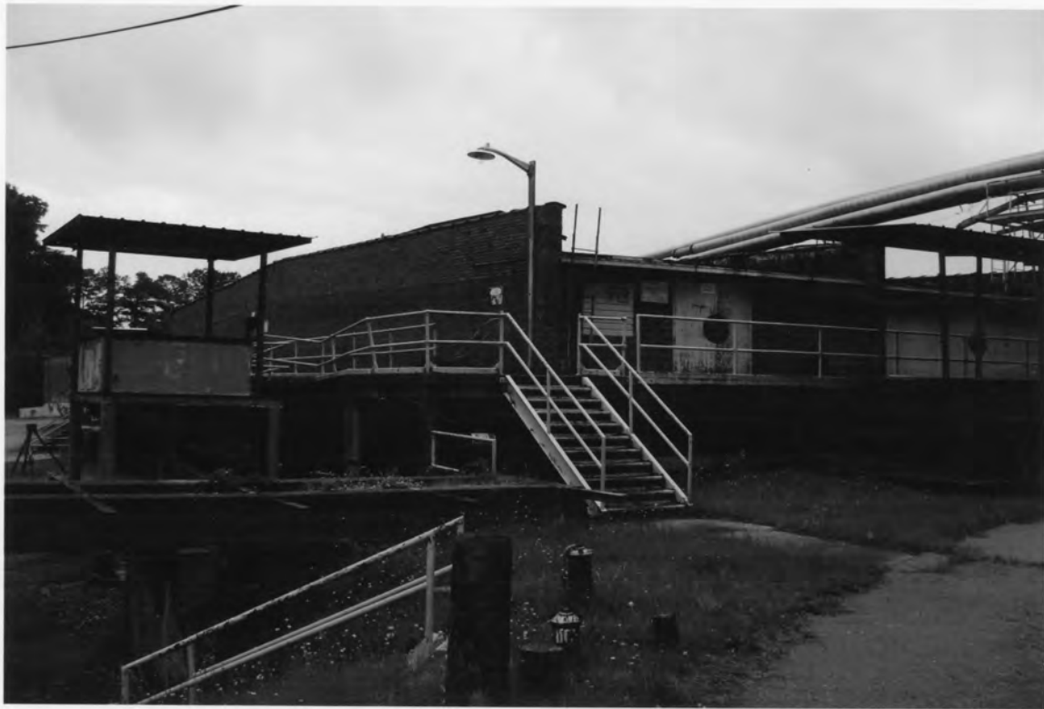
18. Oakland Mill 2802 Fair Avenue, Newberry Newberry County, South Carolina
