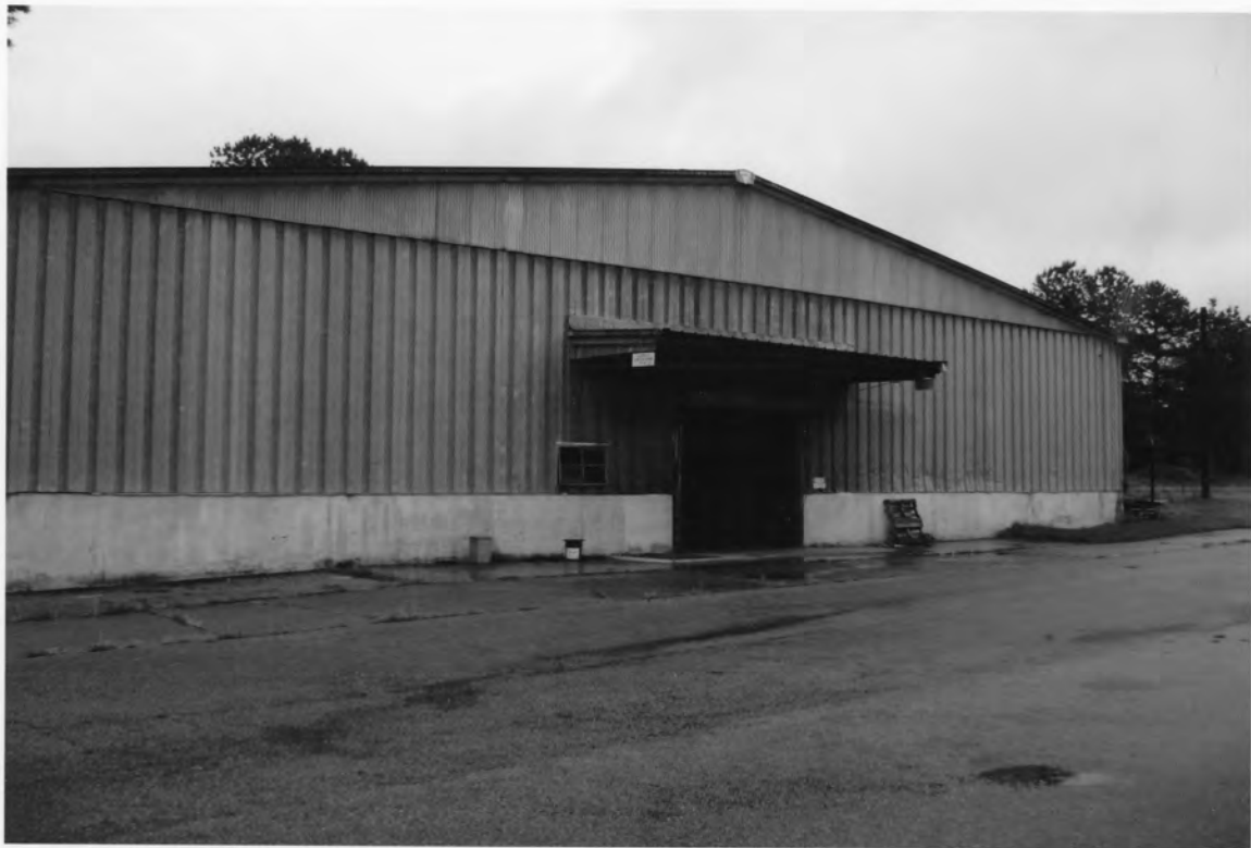
25. Oakland Mill 2802 Fair Avenue, Newberry Newberry County, South Carolina
