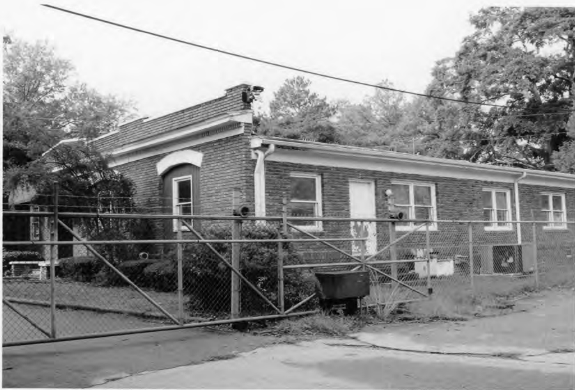
13. Oakland Mill 2802 Fair Avenue, Newberry Newberry County, South Carolina
