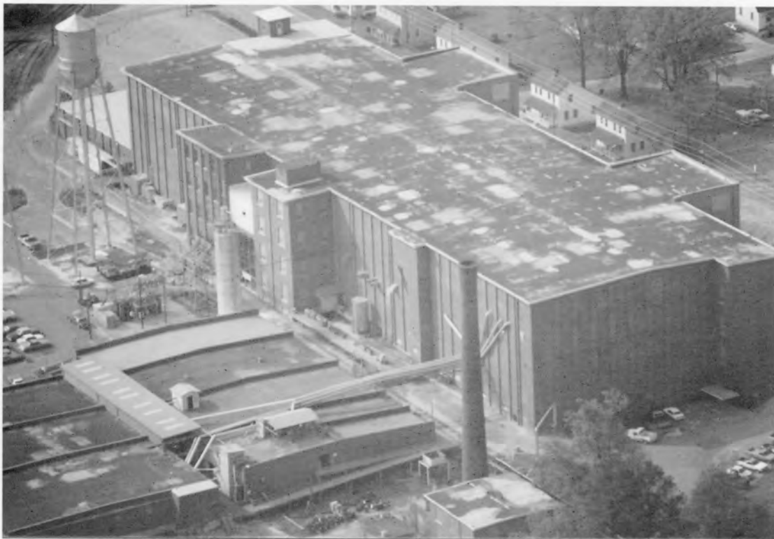
46. Oakland Mill 2802 Fair Avenue, Newberry Newberry County, South Carolina
