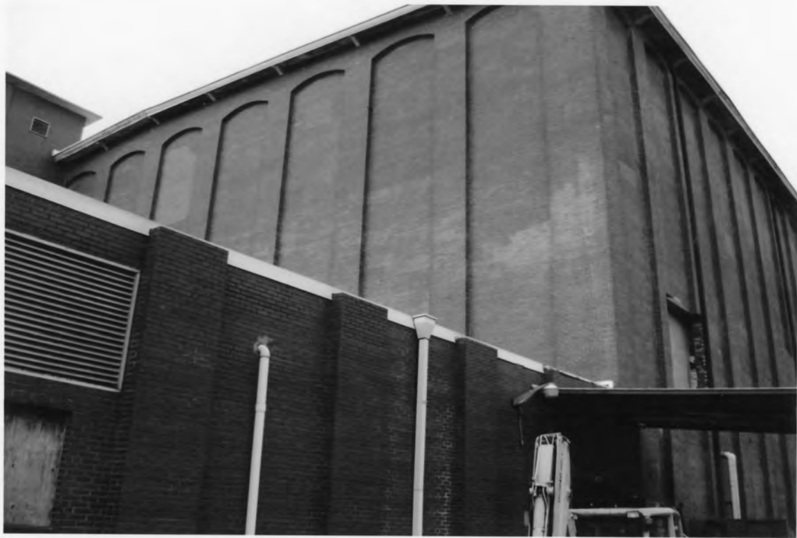
9. Oakland Mill 2802 Fair Avenue, Newberry Newberry County, South Carolina
