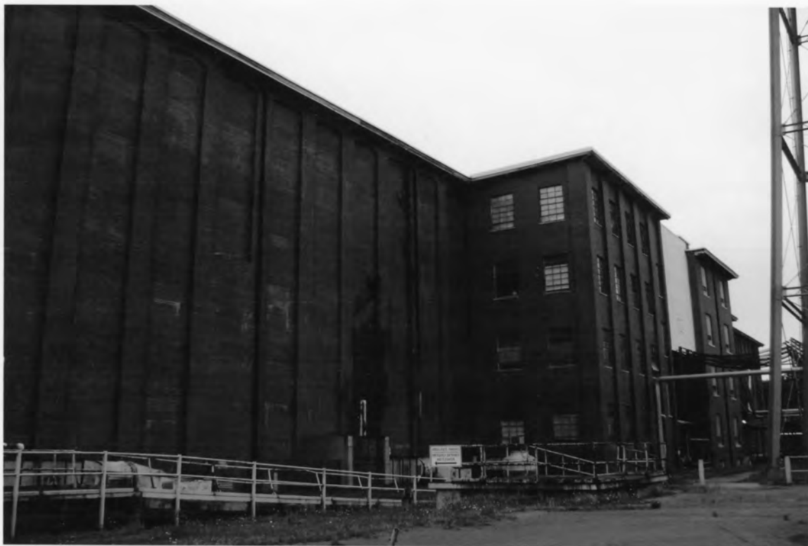
7. Oakland Mill 2802 Fair Avenue, Newberry Newberry County, South Carolina
