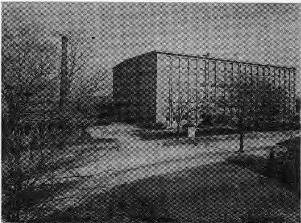
42. Oakland Mill 2802 Fair Avenue, Newberry Newberry County, South Carolina
