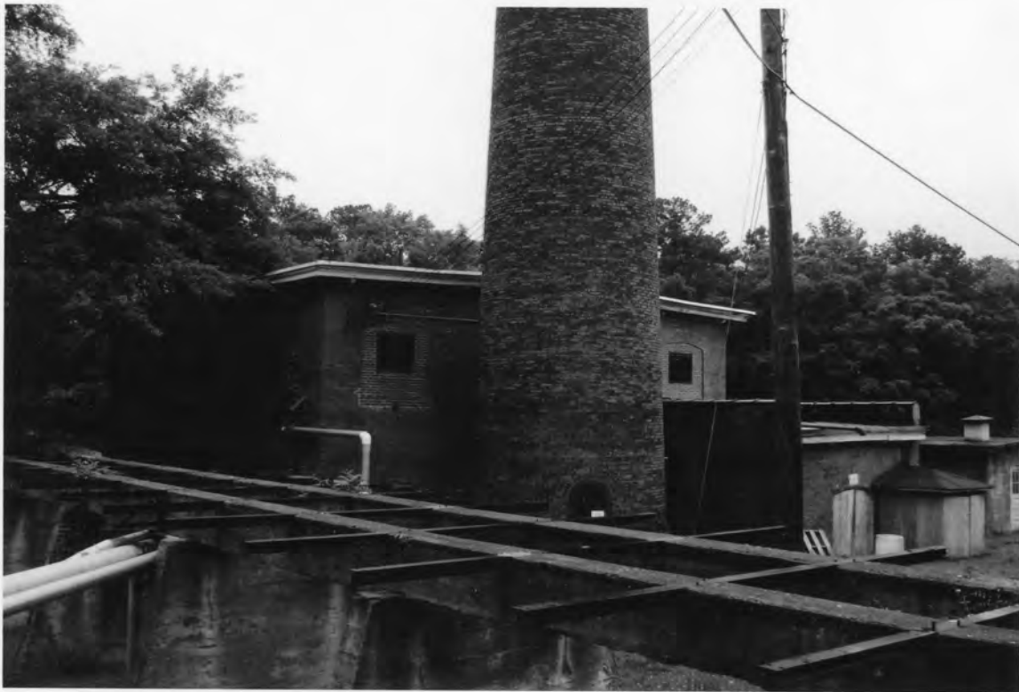
15. Oakland Mill 2802 Fair Avenue, Newberry Newberry County, South Carolina
