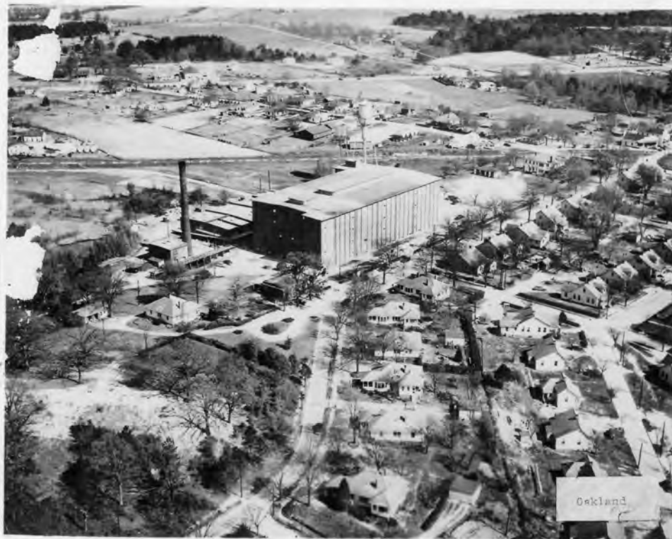
43. Oakland Mill 2802 Fair Avenue, Newberry Newberry County, South Carolina
