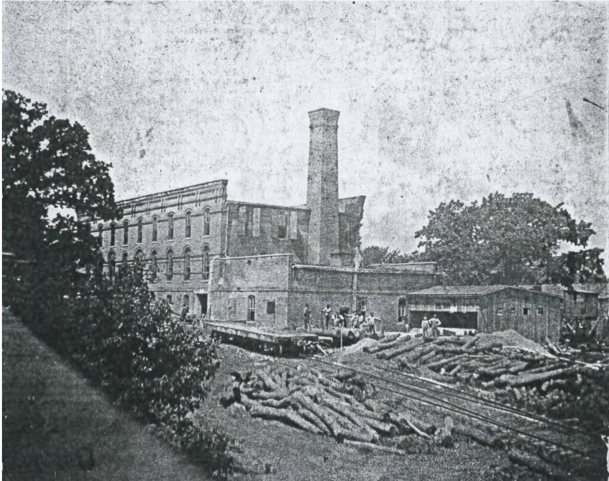
Fig. 1: South and east elevations of building during tenure of the American Manufacturing Company, c. 1910, looking northwest. Railroad spur, east elevation storage shed, full chimney stack, and one-story extension of building housing the furnace system and coal room visible. (Source: The History Center, Linn County Historical Society.)
