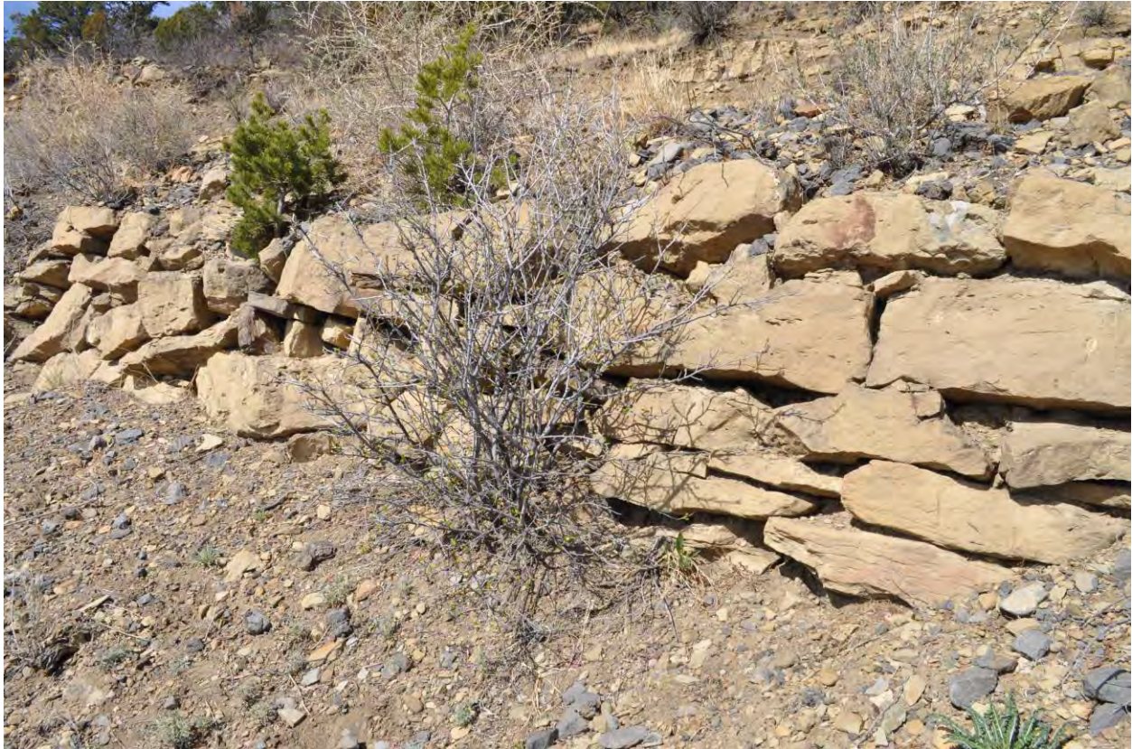
10 of 16: Rock retaining wall, Section 1, photographer facing northwest
