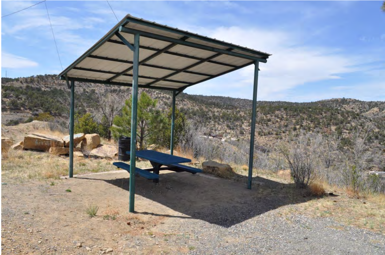
6 of 16: Picnic shelter at Goat Hill Park, photographer facing south.
