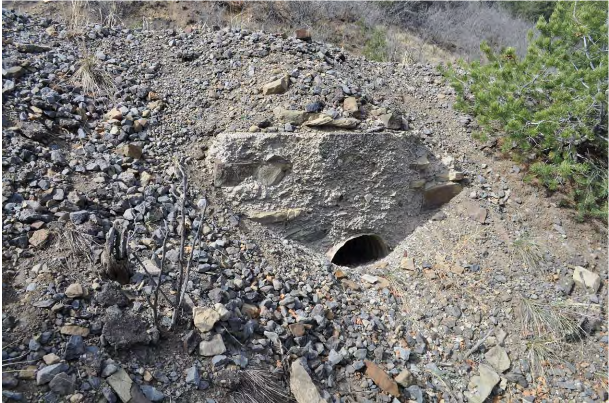
8 of 16: 1920 corrugated metal culvert with concrete headwall, photographer facing north.
