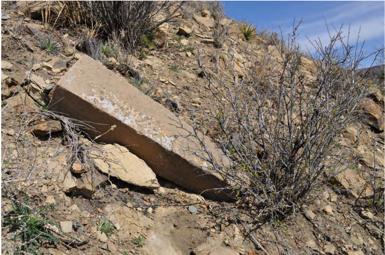
11 of 16: 1908 concrete guard post, photographer facing north.
