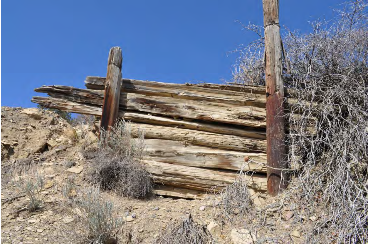
9 of 16: Wood cribbing retaining wall, photographer facing north.
