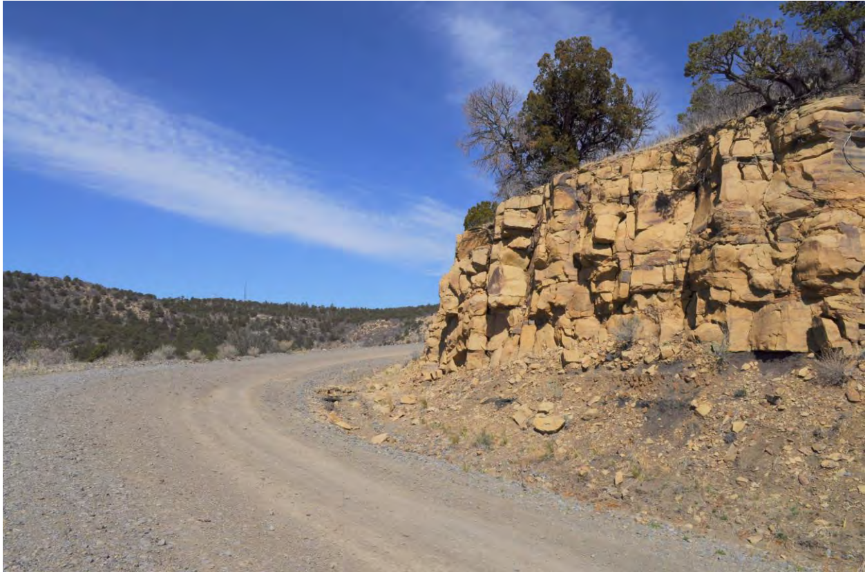
13 of 16: Rock cut of grade ascending ridge, photographer facing southwest.
