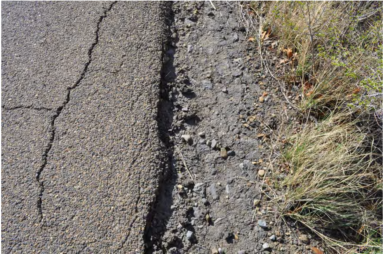
1 of 16: Modern and bituminous macadam paving, photographer facing southeast.
