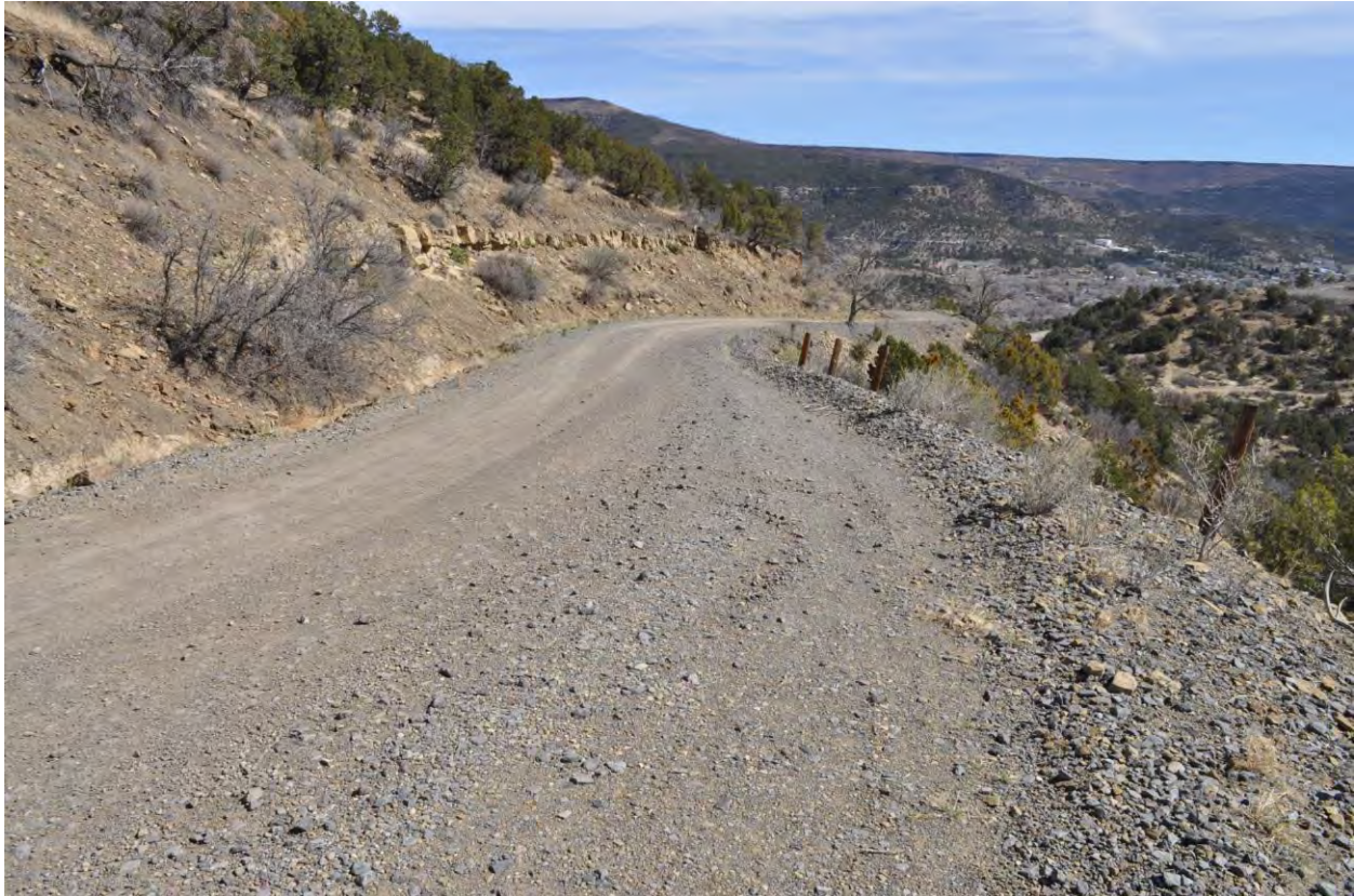
12 of 16: Grade ascending ridge, photographer facing northeast.
