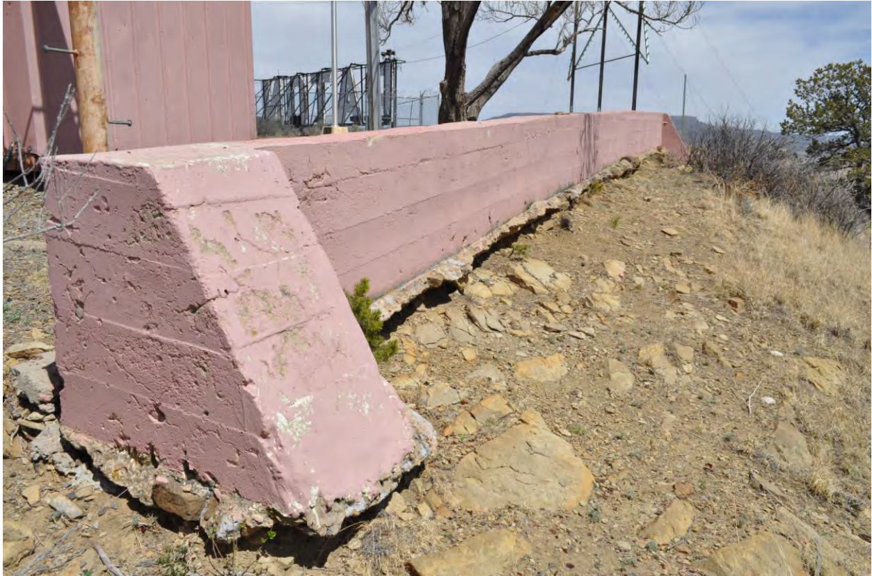
4 of 16: Concrete barrier, photographer facing northeast.
