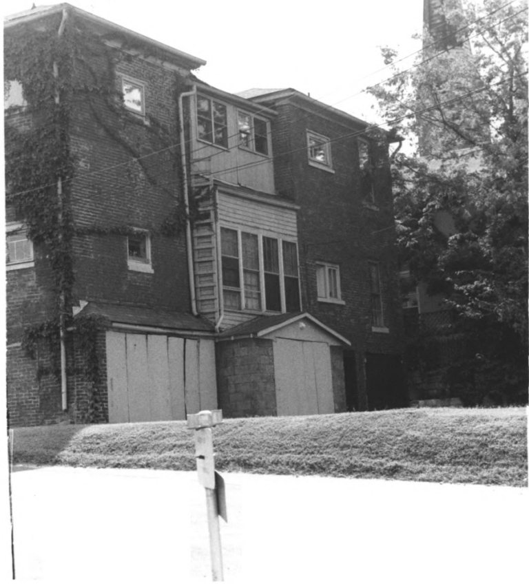
FIRST PRESBYTERIAN CHURCH MANSE MONTGOMERY COUNTY, TN
