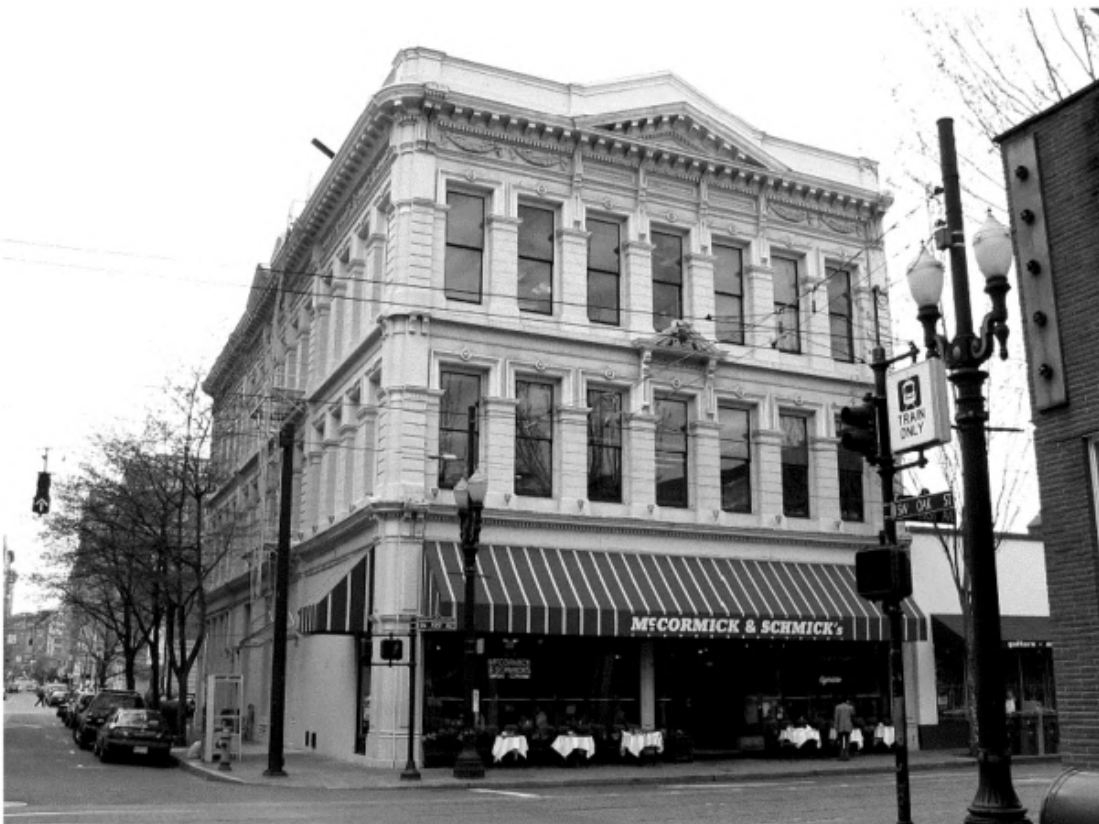
C13: Failing Building, 235 SW 1 st Ave., looking northwest. Bureau of Planning, 2005.
