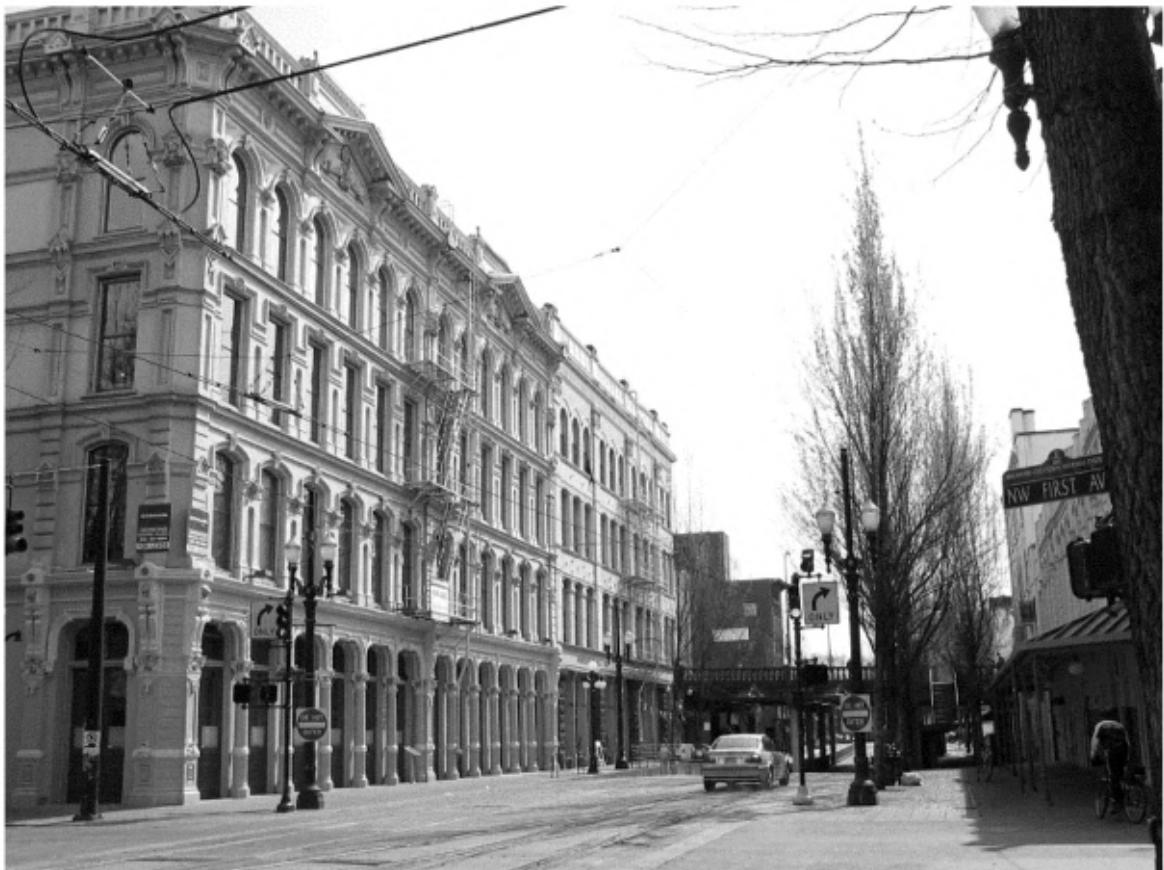
C1: NW 1 st Ave. looking south from NW Couch. 2005. Bureau of Planning.
