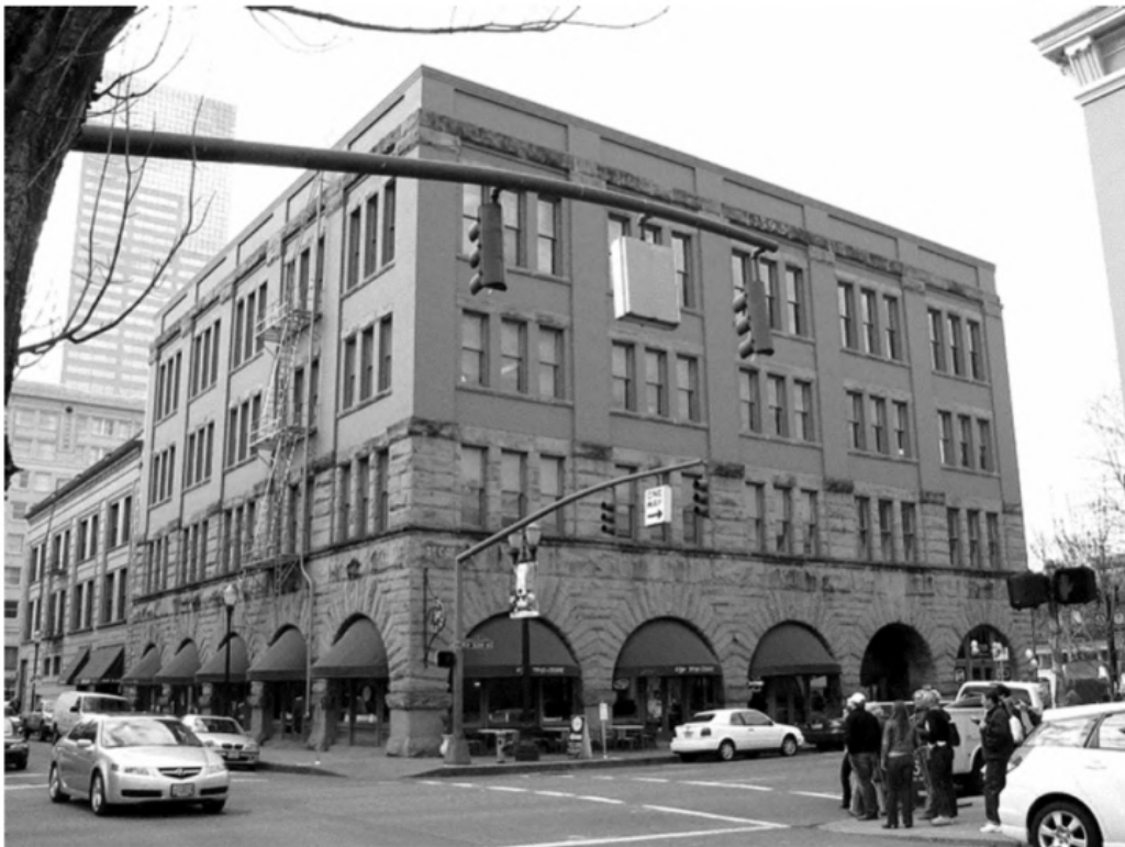
C10: Haseltine Building, 133 SW 2 nd Ave., looking northwest. Bureau of Planning, 2005.
