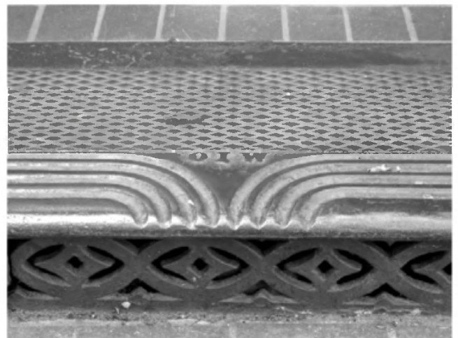
Delschneider Building (1859, detail of Oregon Iron Works mark), 71 SW Oak (#90), right.
