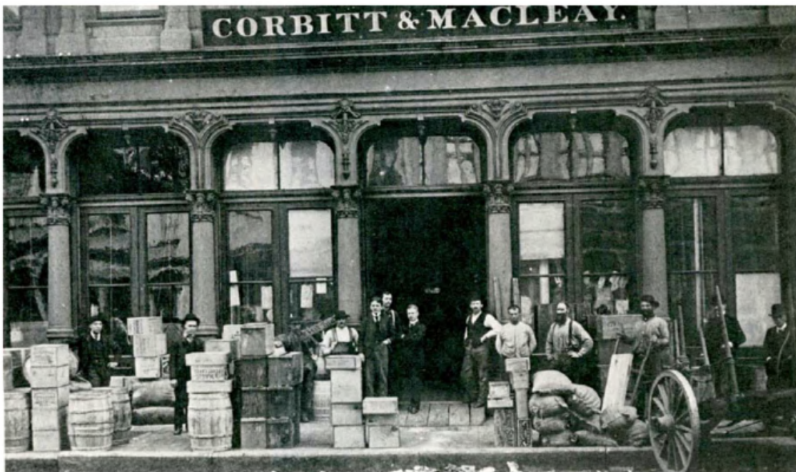
S6: Starr Block (SW Front Ave., between Oak & Pine—demolished), west façade from Front St. Photographer unknown, 1885. Oregon Historical Society.
