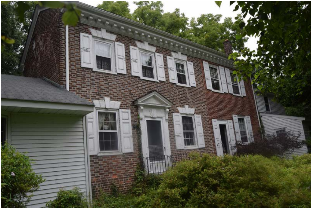
Photo 3. General view of the southeast façade toward northeast.
