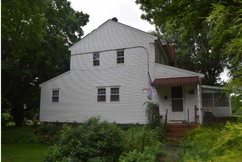
Photo 9. Northeast side of house toward southwest.
