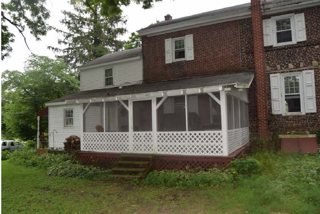
Photo 11. West end of northwest (rear) elevation toward southeast.
