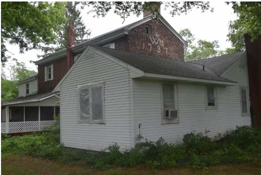
Photo 10. Southwest and northwest elevations of 1958 addition toward south.
