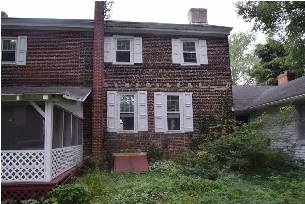
Photo 12. Southwest end of northwest (rear) elevation toward southeast.
