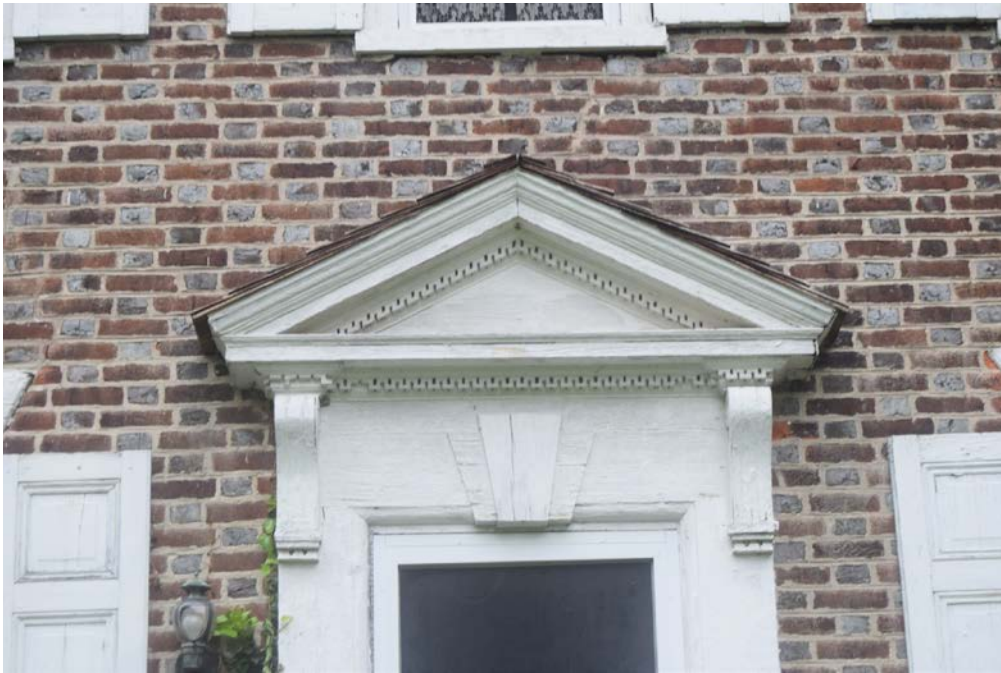
Photo 7. Close-up of entry pediment showing punch and gouge work toward northwest.
