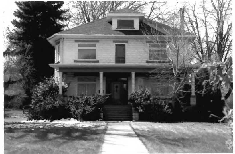
2564 E. Evergreen Avenue Photograph 18
