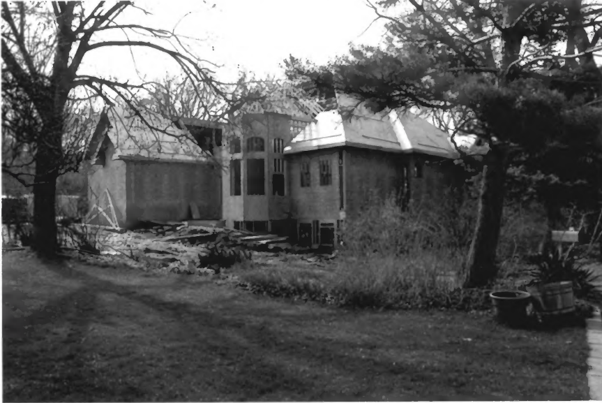
2448 E. Evergreen Avenue (under construction 2006) Photograph 9
