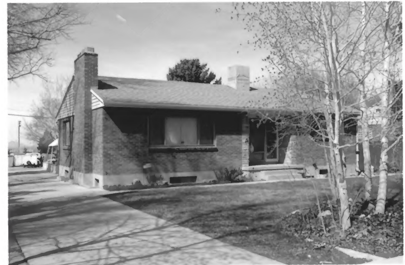
3366 S. Pioneer Street Photograph 40
