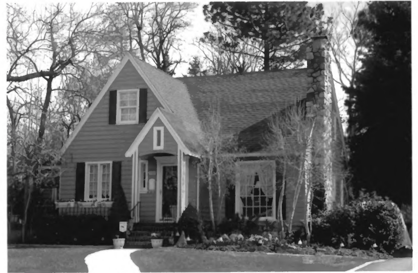
2360 E. Evergreen Avenue Photograph 26
