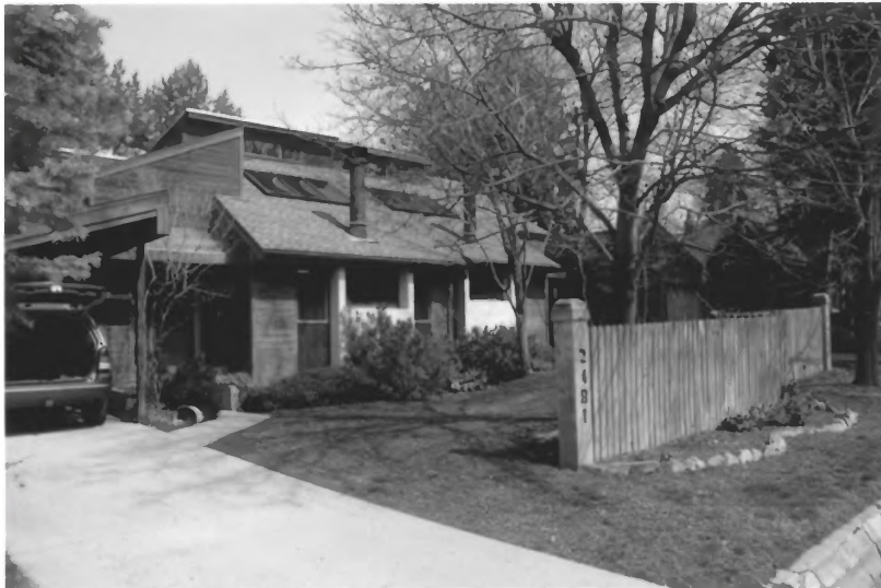
2481-2485 E. Evergreen Avenue Photograph 47
