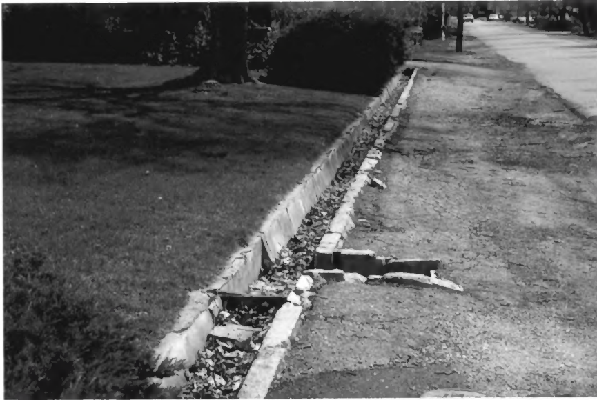
3325 S. Oakwood Street (stone-lined gutter/ditch) Photograph 5
