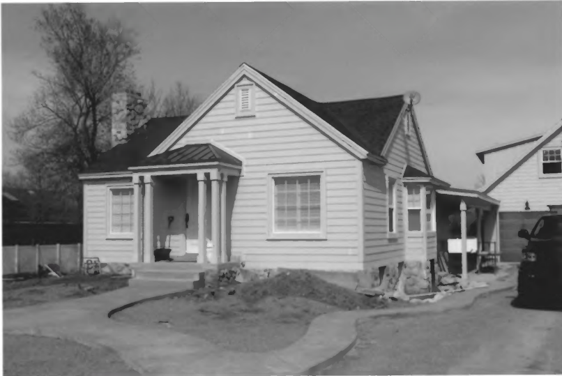
2511 E. Evergreen Avenue Photograph 37
