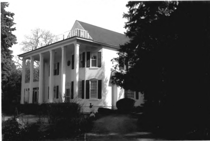
2661 E. Evergreen Avenue Photograph 15
