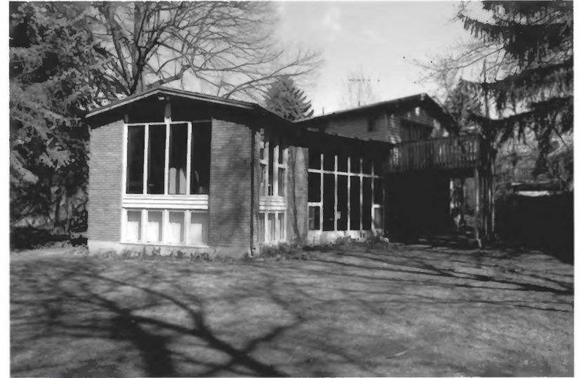
2584 E. Evergreen Avenue Photograph 46
