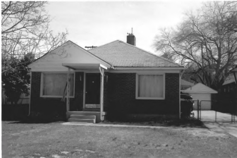
3335 S. Pioneer Street Photograph 35
