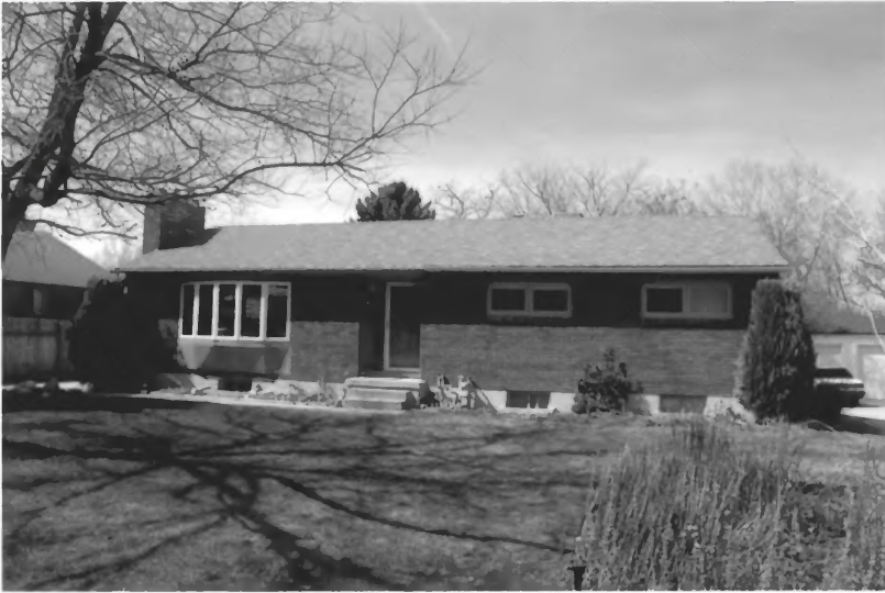
3336 S. Pioneer Street Photograph 41
