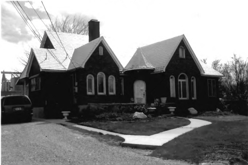
2324 E. Evergreen Avenue Photograph 23
