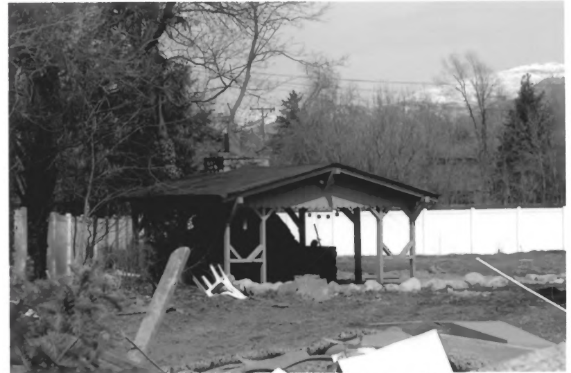
2511 E. Evergreen Avenue (picnic pavilion in rear) Photograph 38
