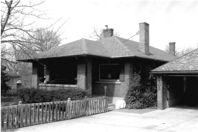
2405 E. Evergreen Avenue Photograph 21
