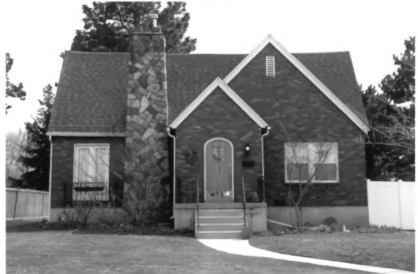
2342 E. Evergreen Avenue Photograph 24
