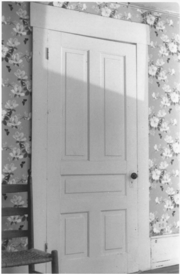
Farrar Homestead Shelbyville vicinity, Bedford Co., TN
