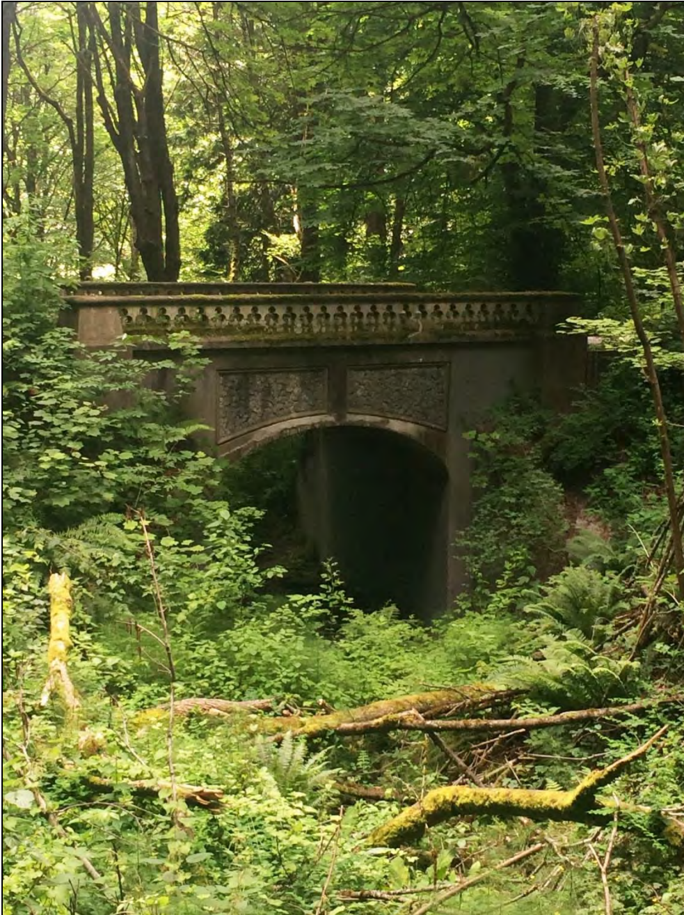
No. 0010, looking west at the bridge (June 15, 2018).
