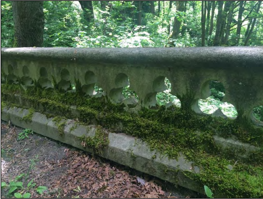
No. 0011, detail view of the bridge, east balustrade (June 15, 2018).
