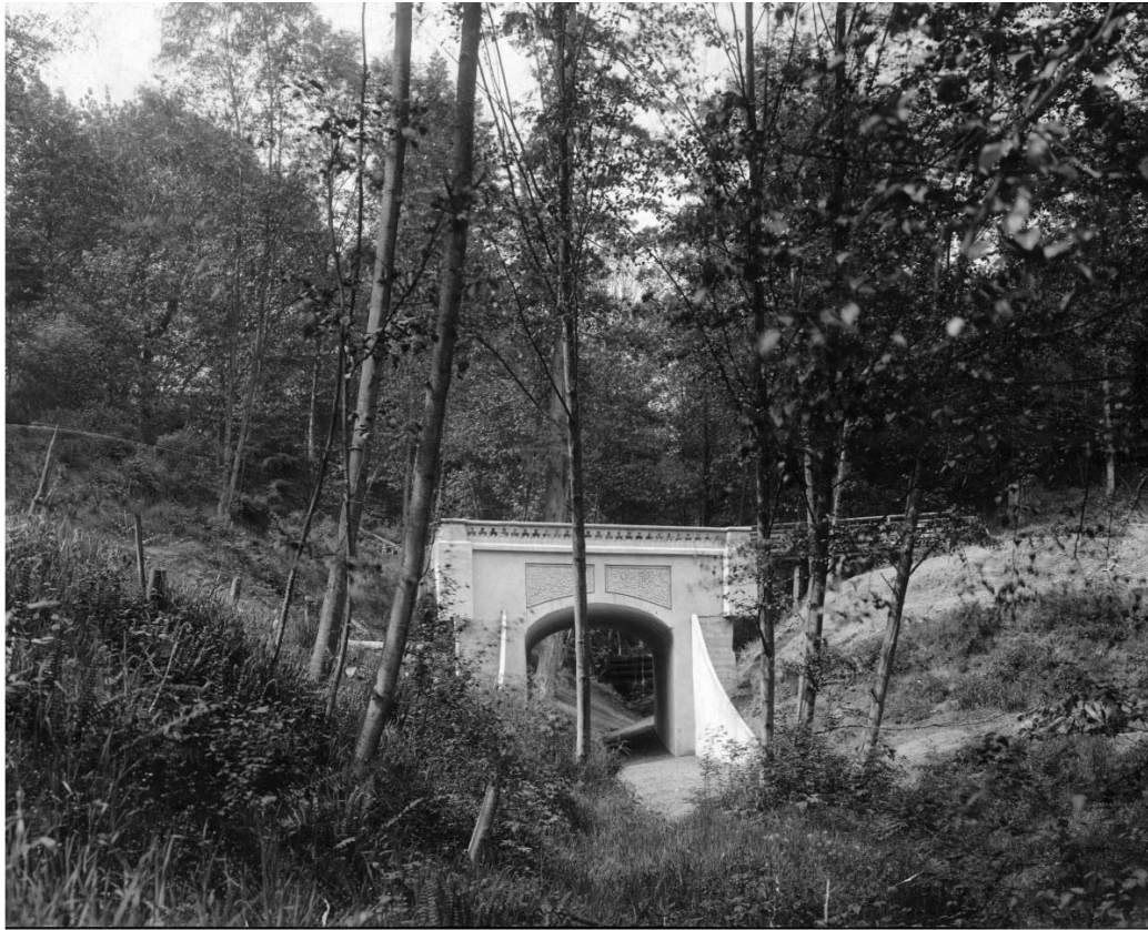
View looking generally northwest at the bridge under construction in ca. 1909. The boulevard does not appear, though grading anticipates its construction (SMA, Item 29052).
