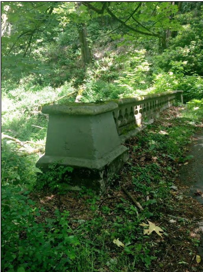
No. 0012, detail view of the west balustrade (June 15, 2018).
