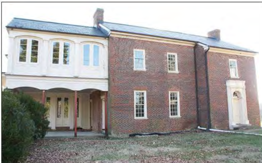
Figure 2: Façade of the Spencer Buford House in 2015.
