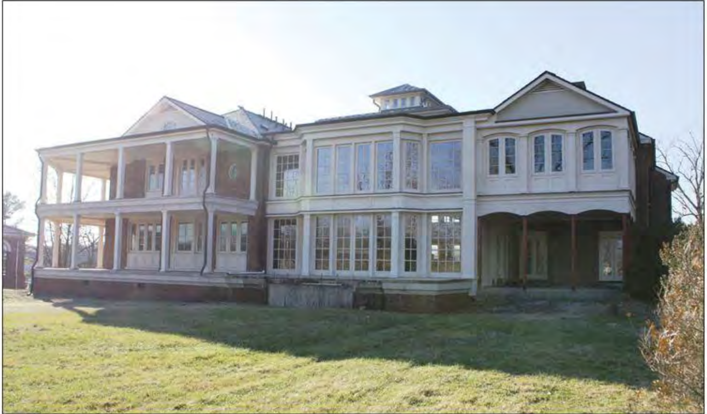
Figure 10: South elevation in 2015.
