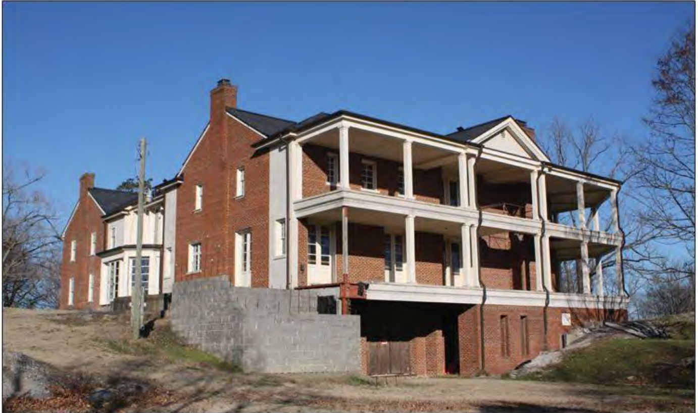
Figure 8: West and south elevations in 2015.
