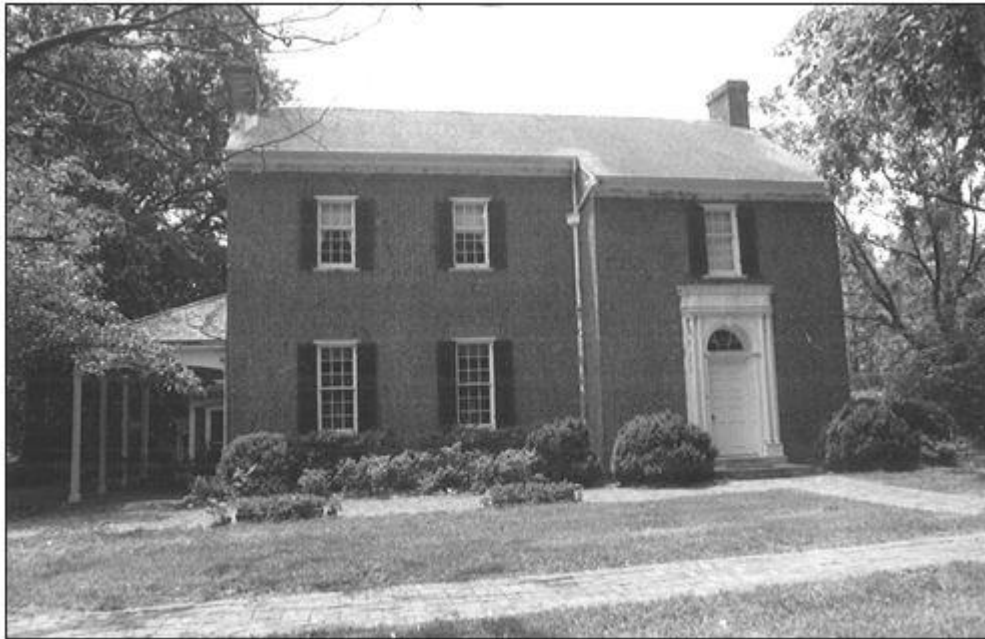
Figure 1: Façade of the Spencer Buford House in 1988 at the time of National Register listing.
