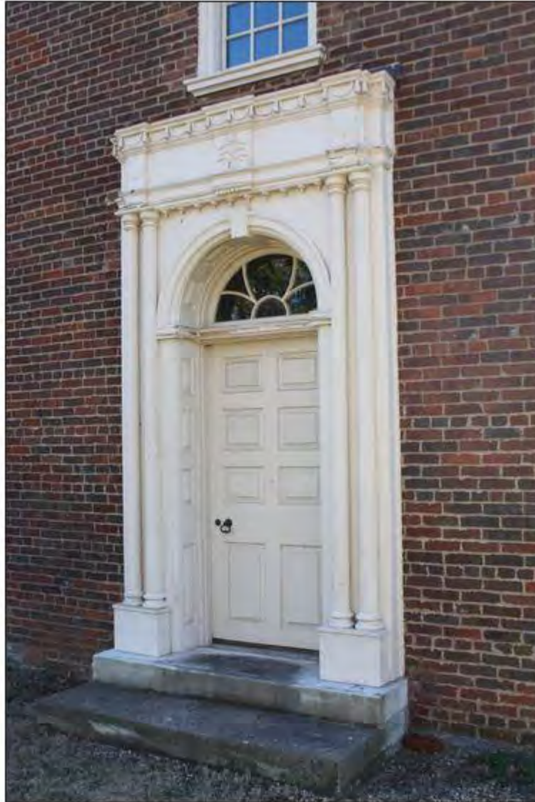
Figure 3: Main Entry of the Spencer Buford House in 2015
