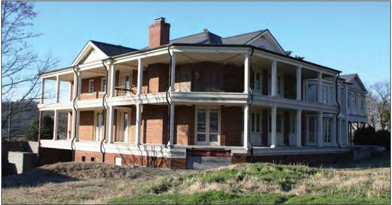
Figure 9: South and east elevations in 2015.
