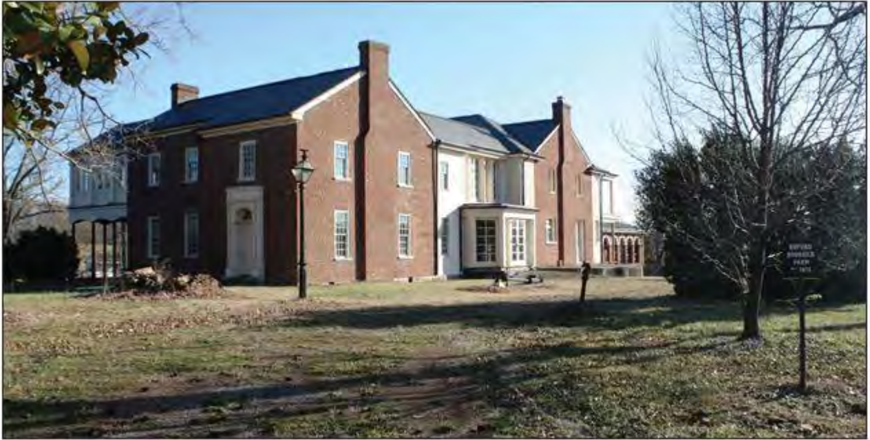
Figure 5: North façade and west elevation of the Spencer Buford House in 2015.
