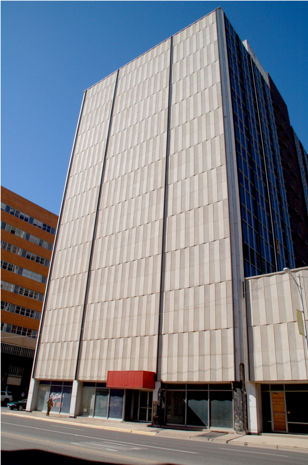
# 3 - Exterior view, east elevation, camera facing southwest
