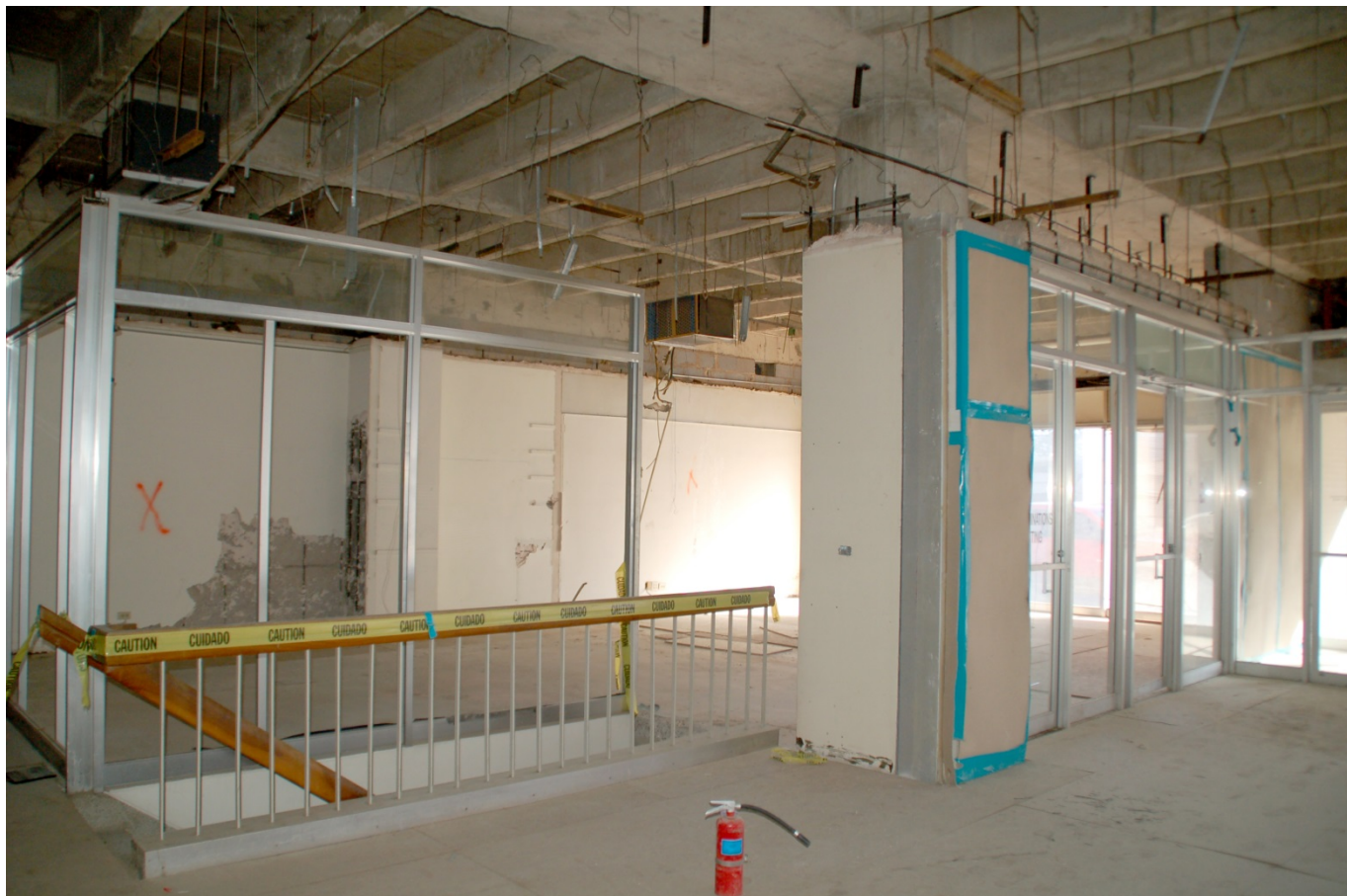
# 13 - Interior view, east corridor and staircase leading to basement, camera facing northeast
