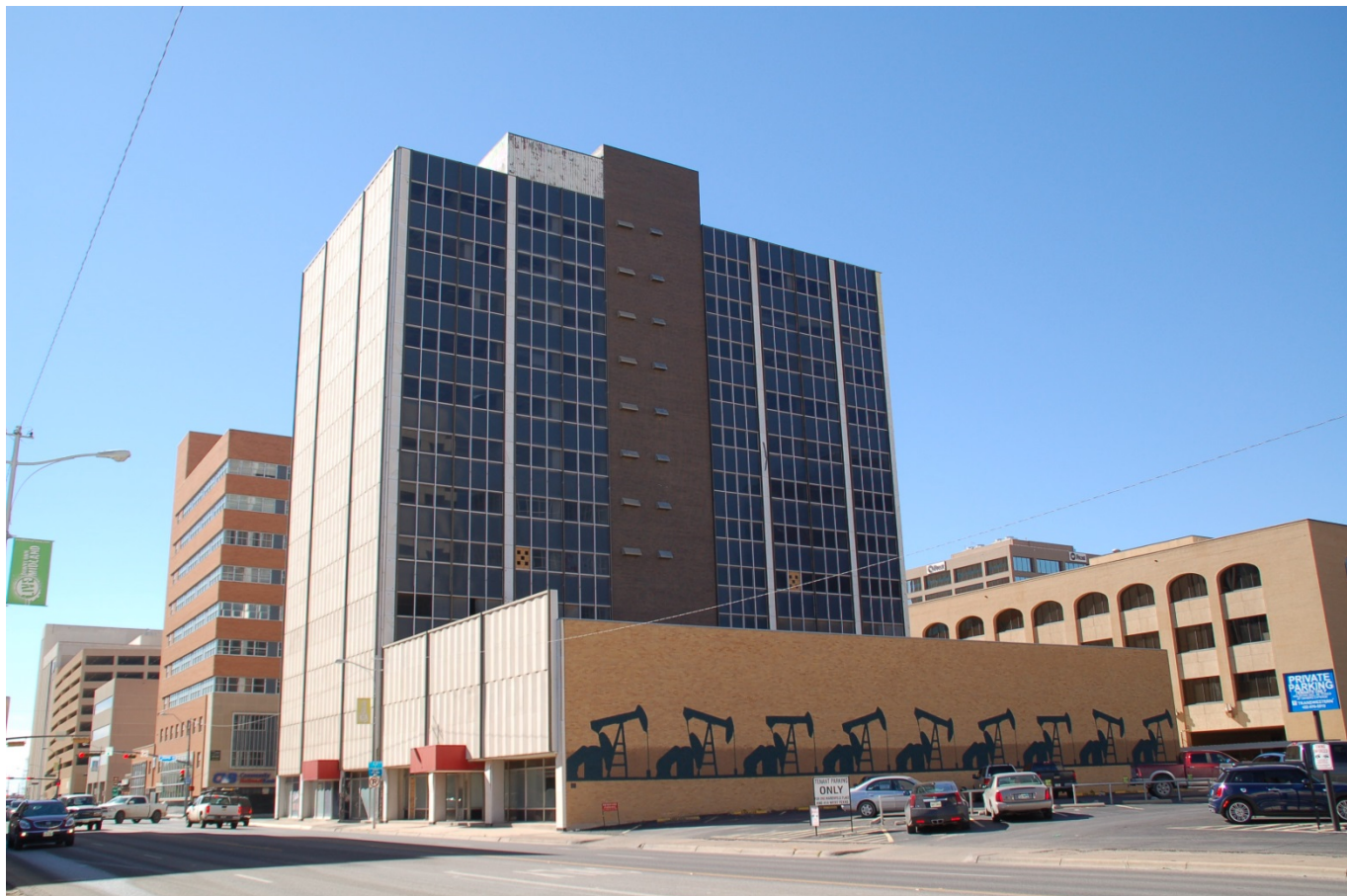
# 4 - Exterior view, east and north elevations, camera facing southwest
