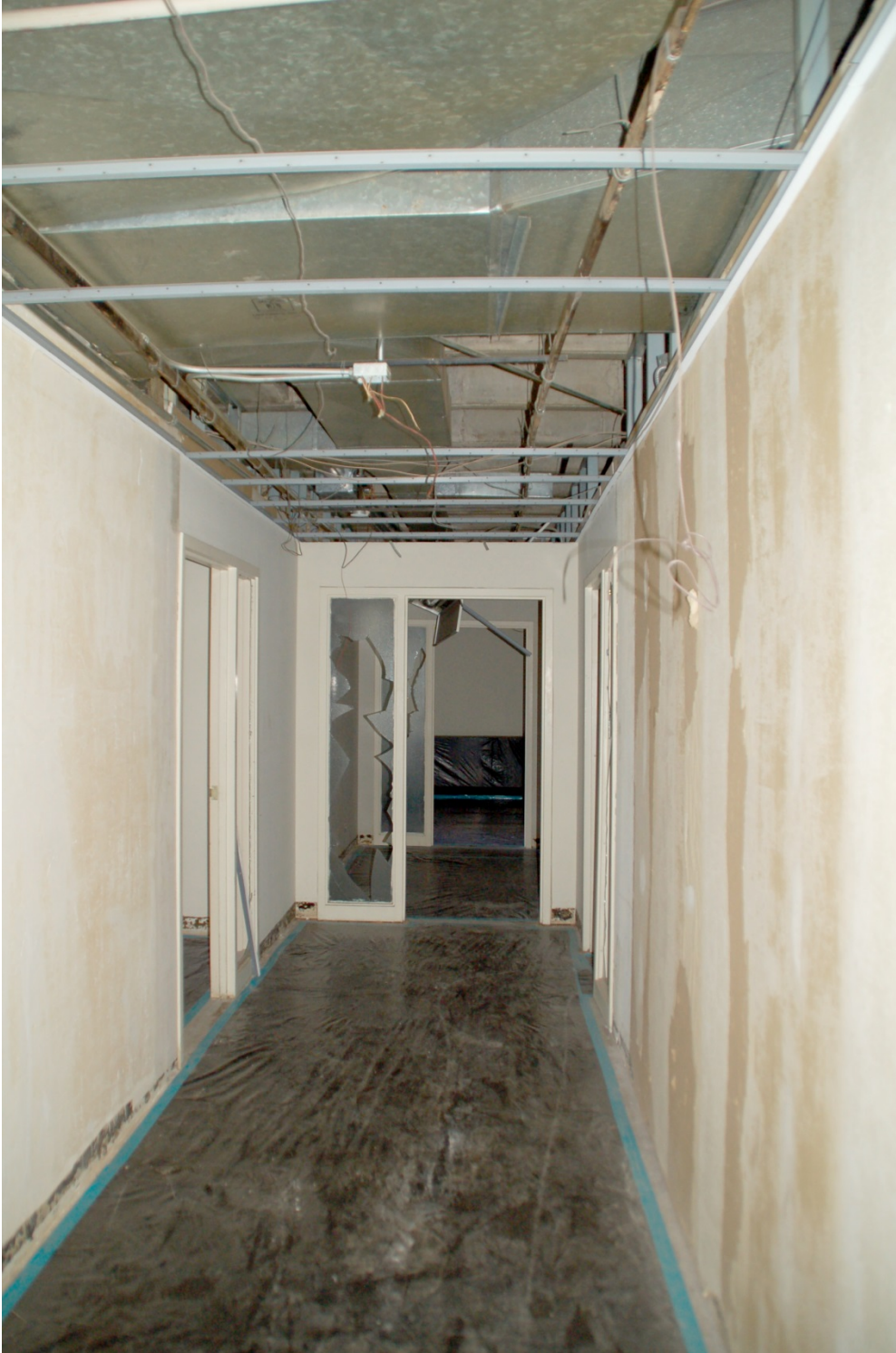
# 17 - Interior view, typical upper-floor corridor (sixth floor), camera facing east
