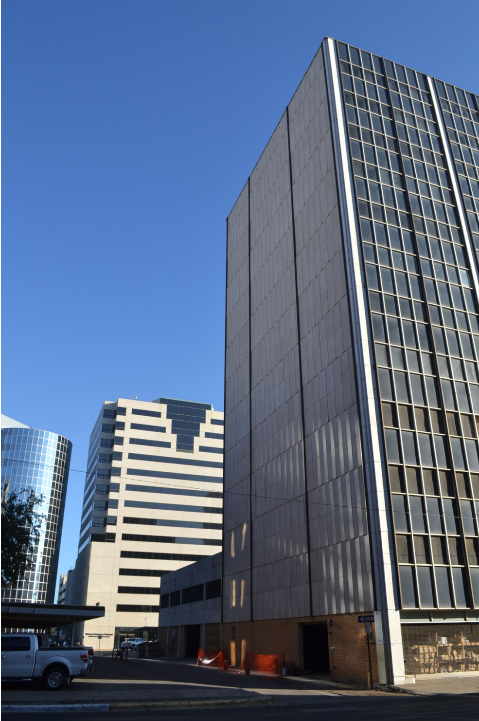
# 6 - Exterior view, west elevation, camera facing northeast
