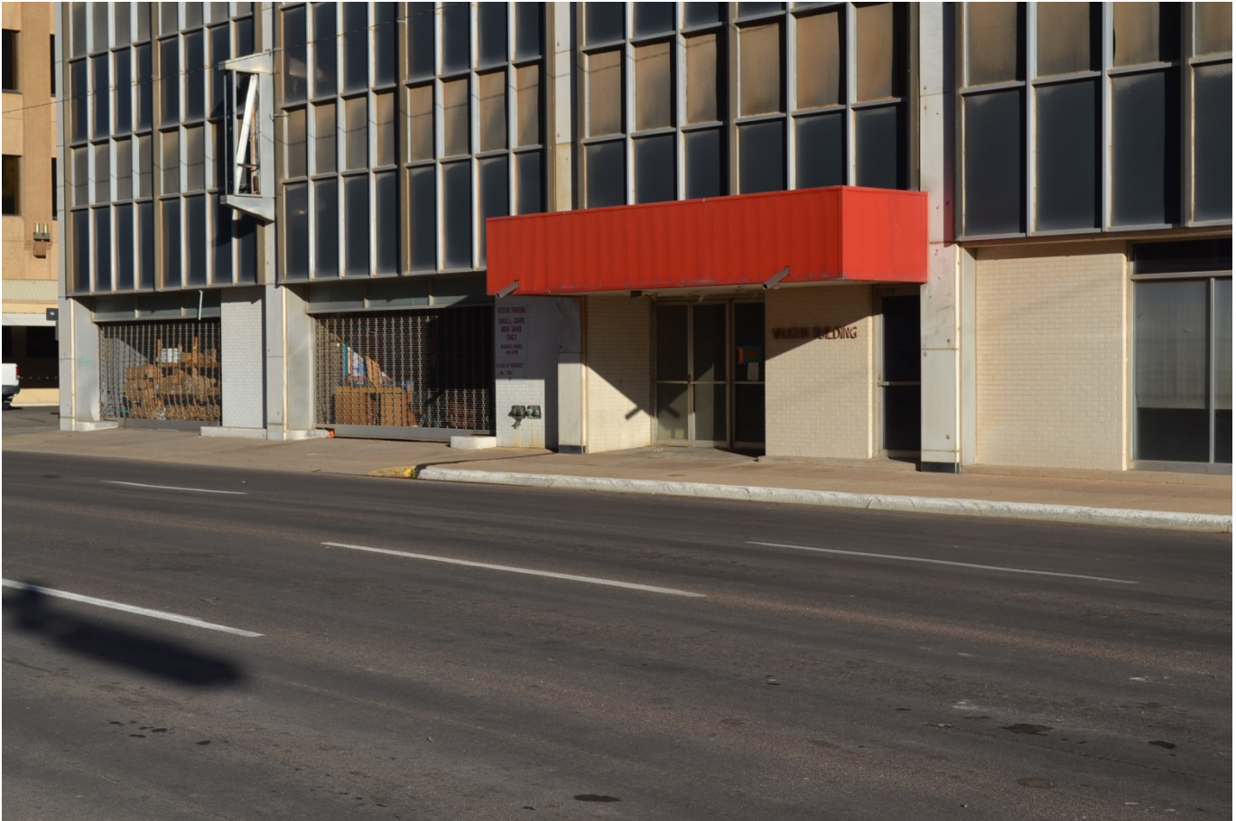
# 8 - Detail view, south elevation, main building pedestrian and garage entrances, camera facing northwest
