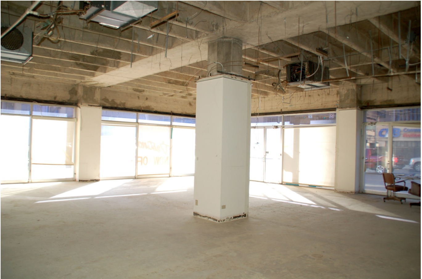
# 14 - Interior view, typical first-floor retail space, camera facing southeast
