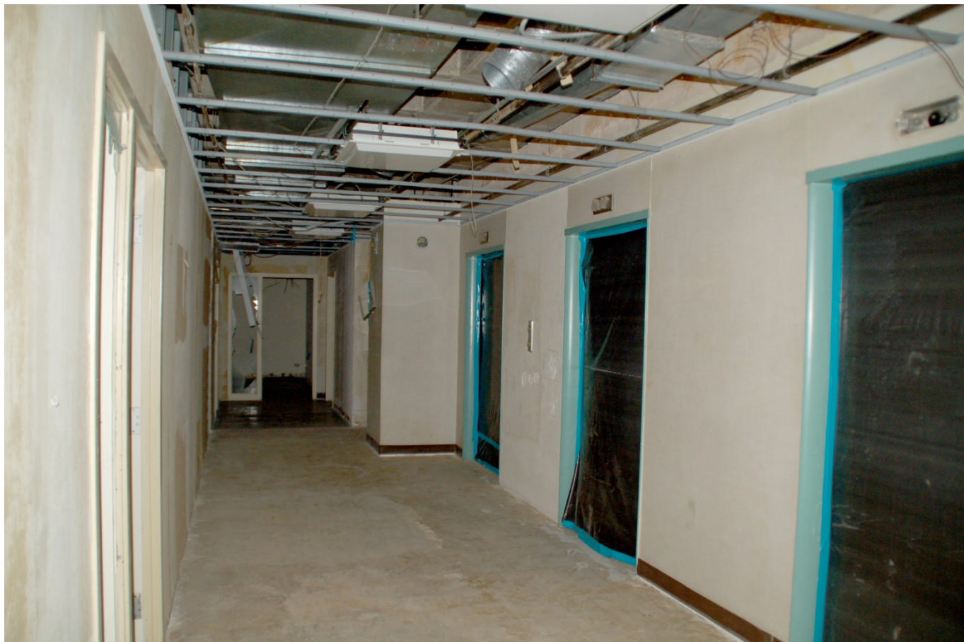
# 16 - Interior view, typical upper-floor elevator lobby (sixth floor), camera facing west
